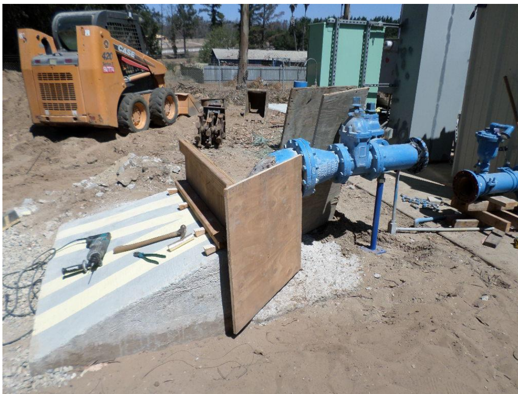
Forming thrust block for above ground piping adjustments.
