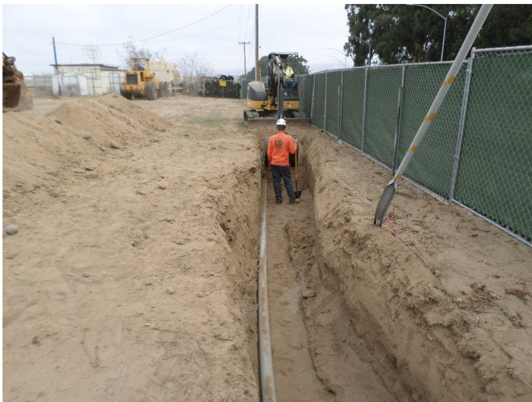
Exposing 4-inch Verizon conduit which runs along the side of the vaults.
