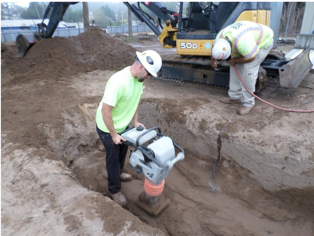
Backfill and compaction over the hot tap connection of the 12-inch waterline and 1-inch copper site waterline.
