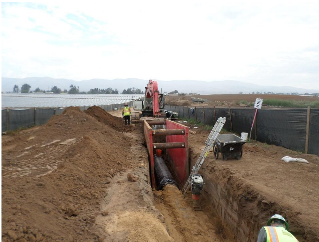
Spiess backfilling and compacting over 24-inch DIP in access road.
