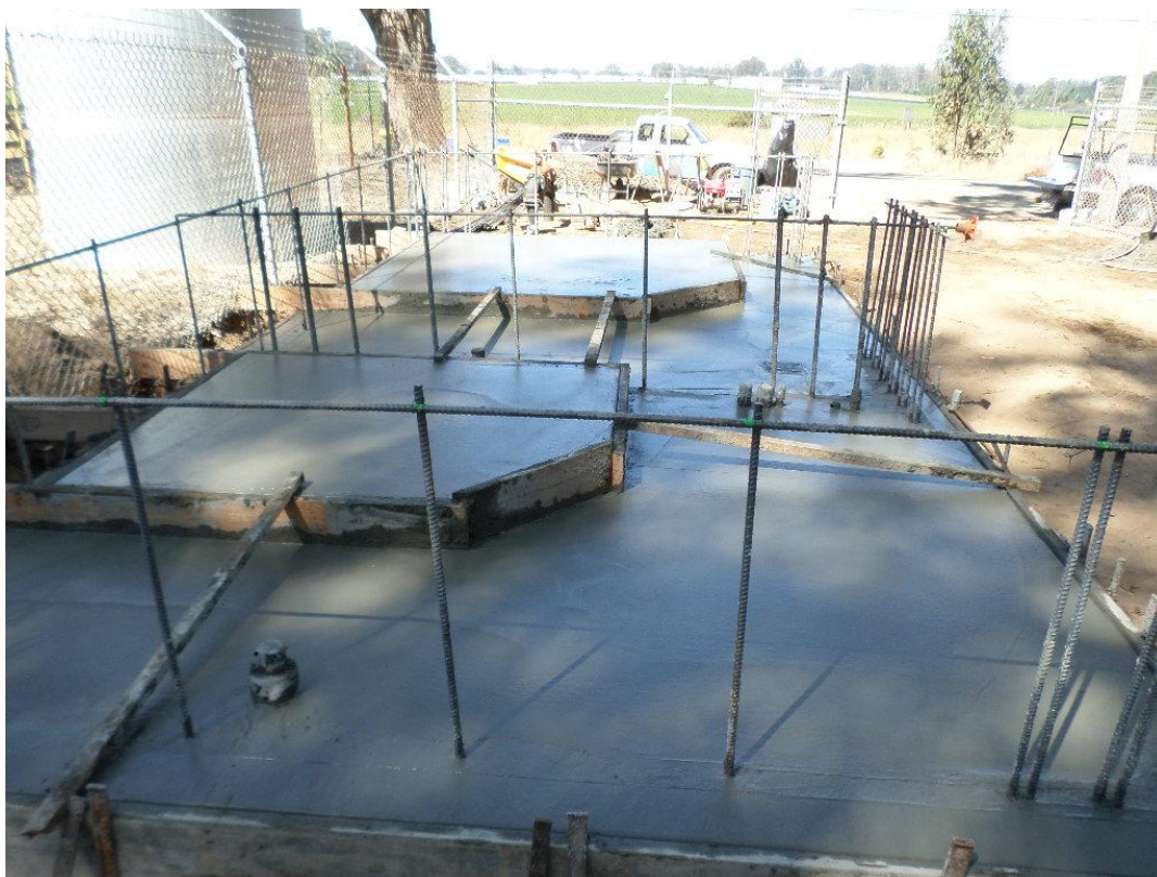
Finished chemical tank slab.
