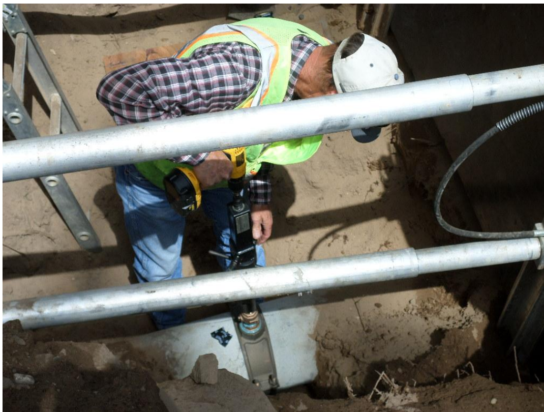
Vicker's Backhoe performing the hot tap of the existing 12-inch waterline to connect the 1-inch copper site waterline.
