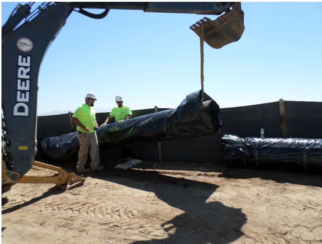
Spiess wrapping 24-inch DIP for installation along access road.
