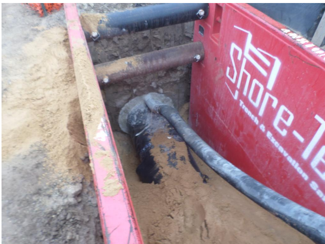
Filling annular space inside the 36-inch casing pipe with sand.
