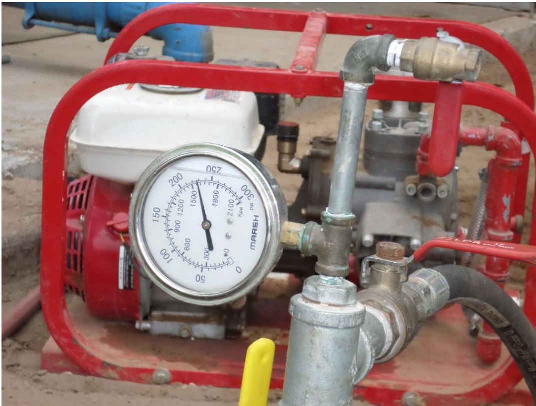
Pressure testing the new 1-inch copper site waterline.
