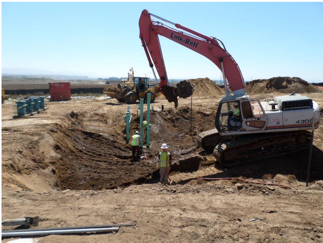
Spiess completing installation of the pipe extensions to the future tanks with backfill and compaction testing by Fugro.
