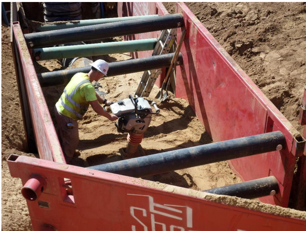
Spiess backfilling and compacting over the pipe extension for the future tank.
