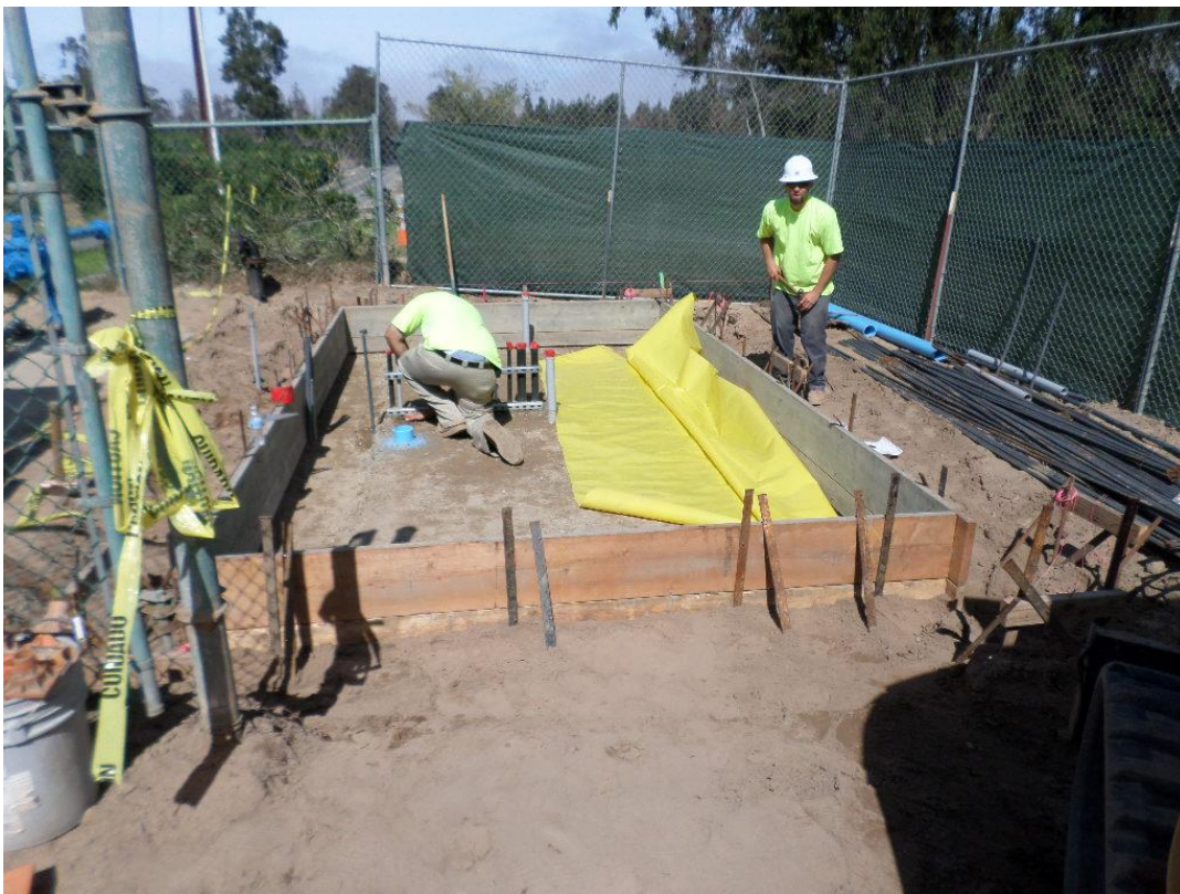
Spiess completing chemical building slab forms and installing vapor barrier.
