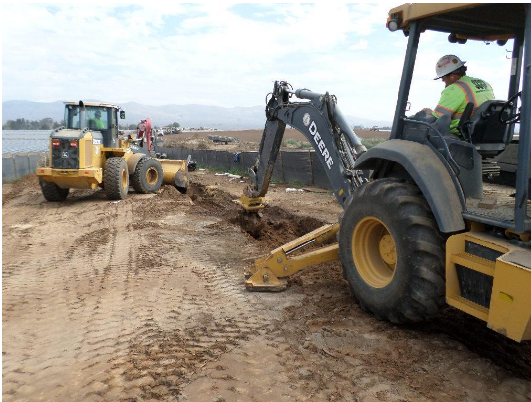
Backfilling and compacting over 24-inch DIP in access road.
