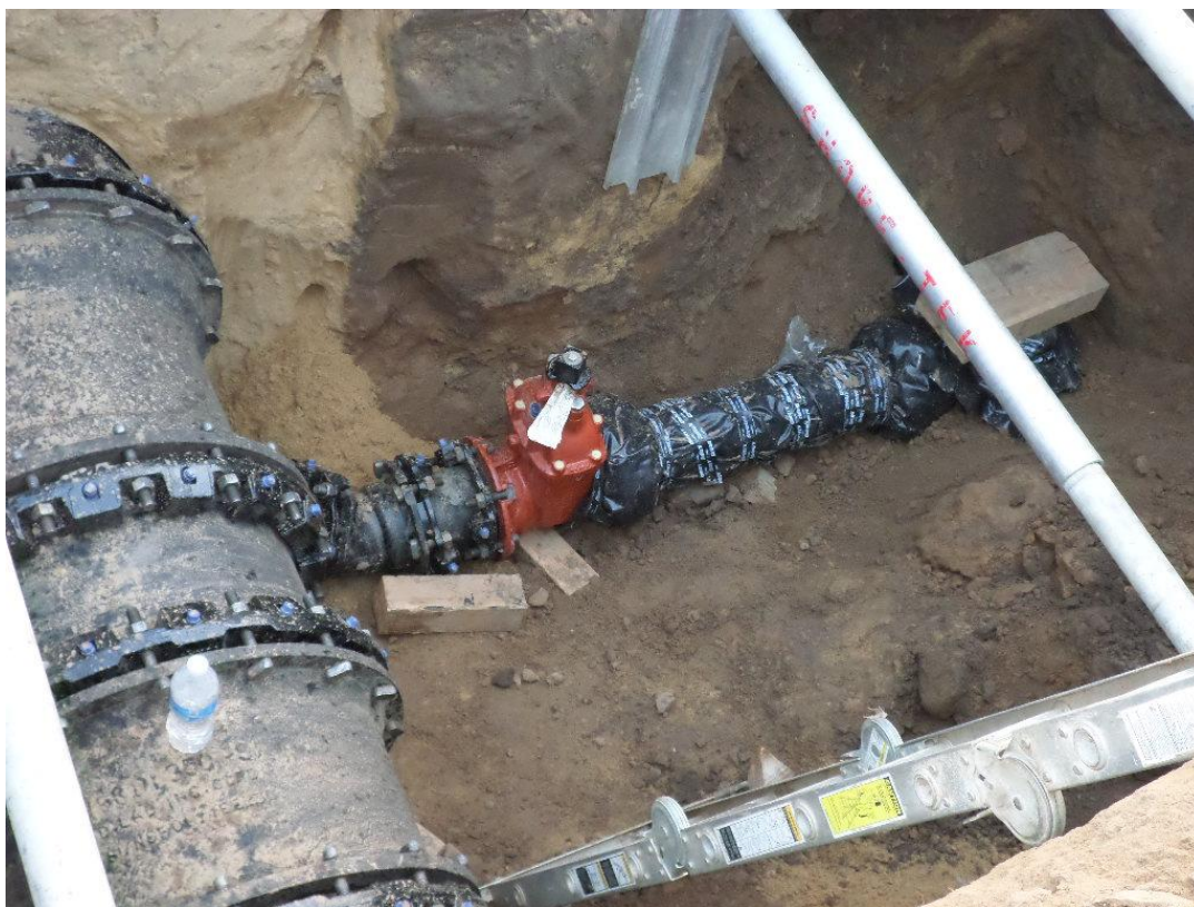
Installing 6-inch blow-off on 24-inch DIP in access road.
