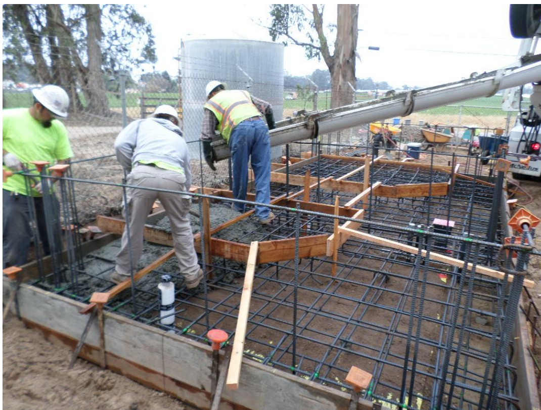
Spiess pouring concrete for chemical building slab.
