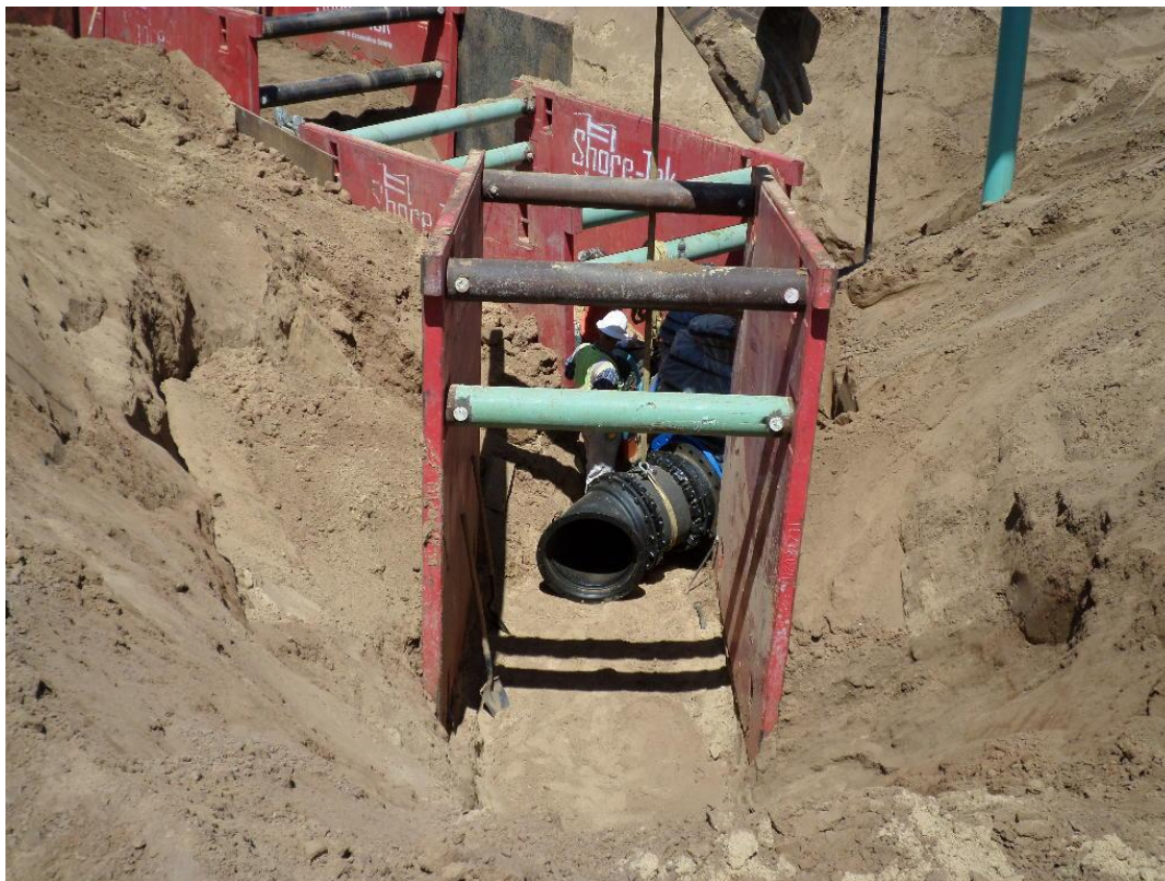
Spiess installing pipe extension to future tank.
