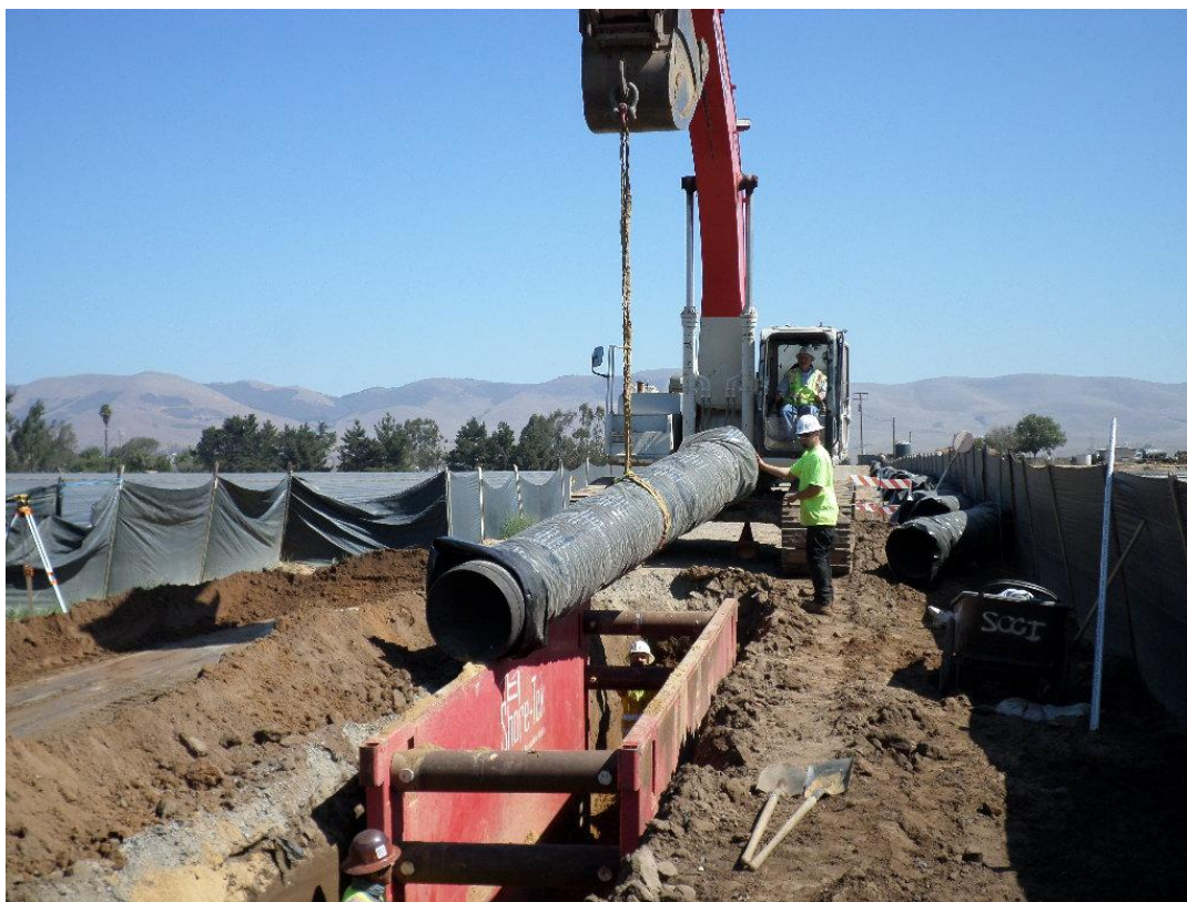
Installing 24-inch DIP in access road.
