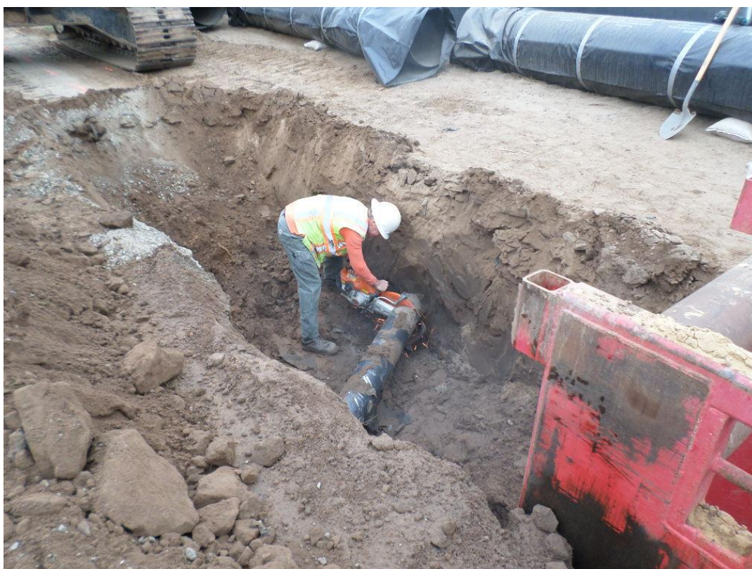
Spiess cutting out abandoned 8-inch gas main from trench.
