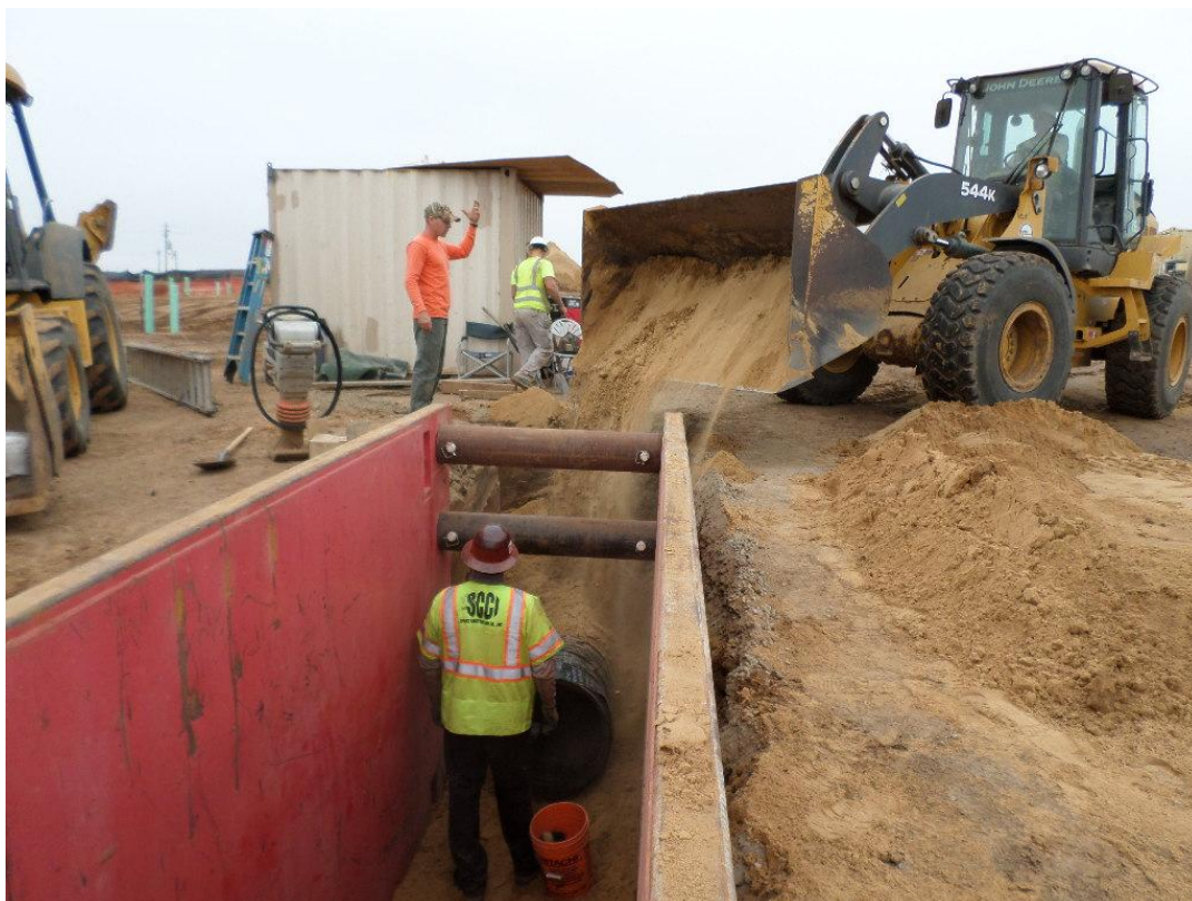
Spiess backfilling the 24-inch DIP as they start installing the pipe along the access road.
