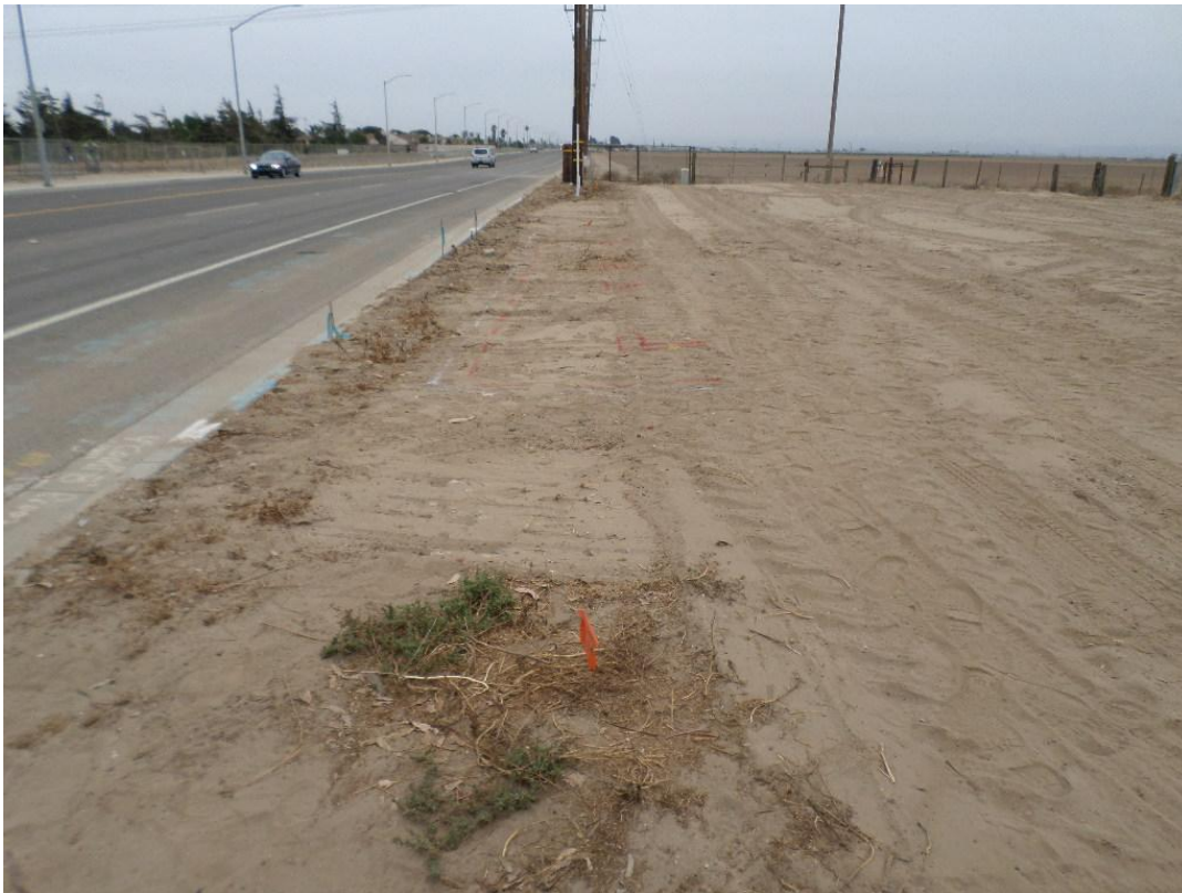
Site cleared and grubbed and the vault locations laid out.
