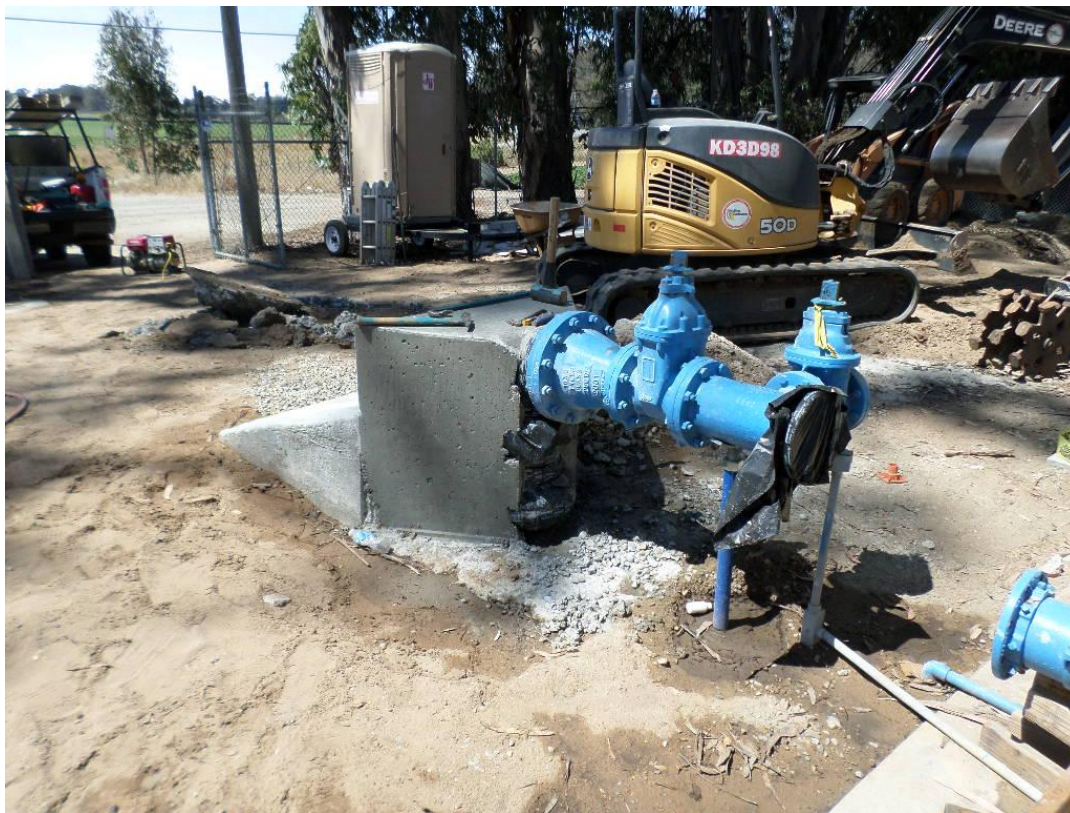
Forms removed from thrust block.
