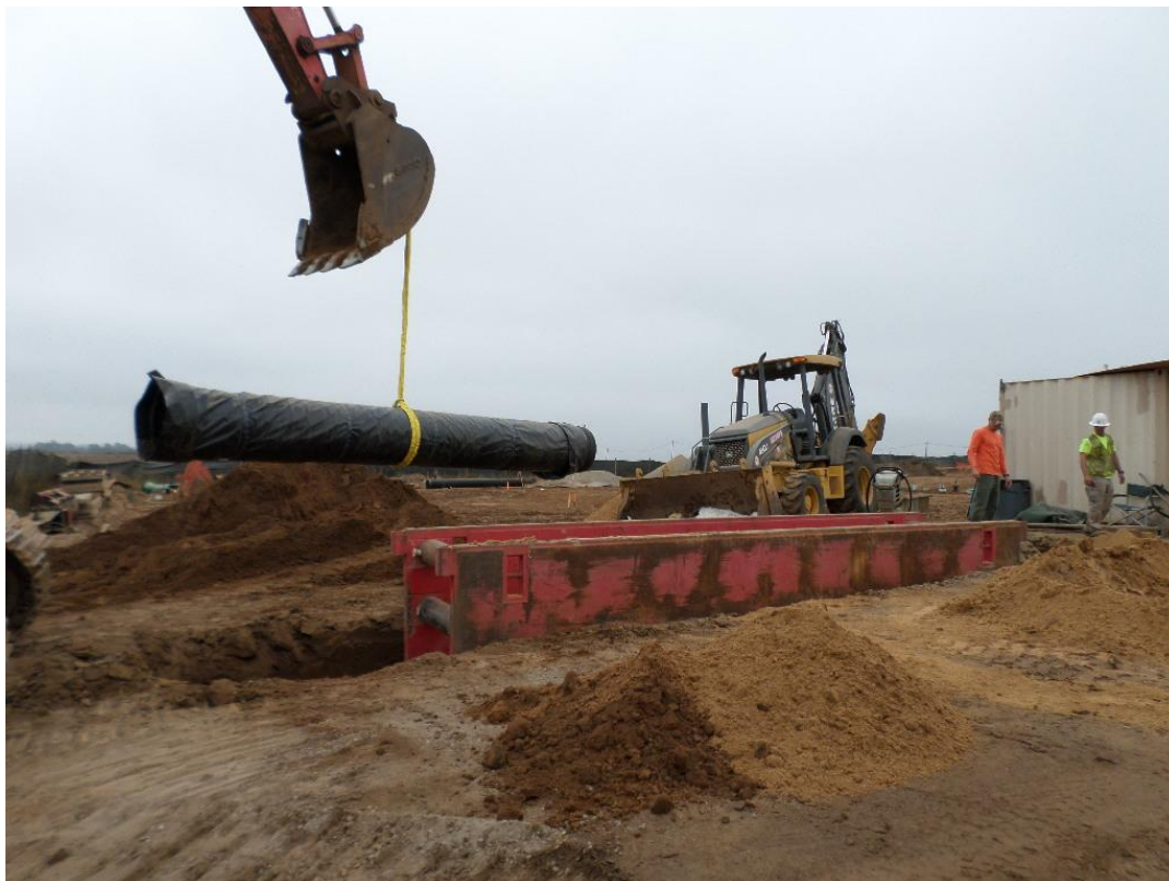
Spiess installing 24-inch DIP from near the pump station down access road.
