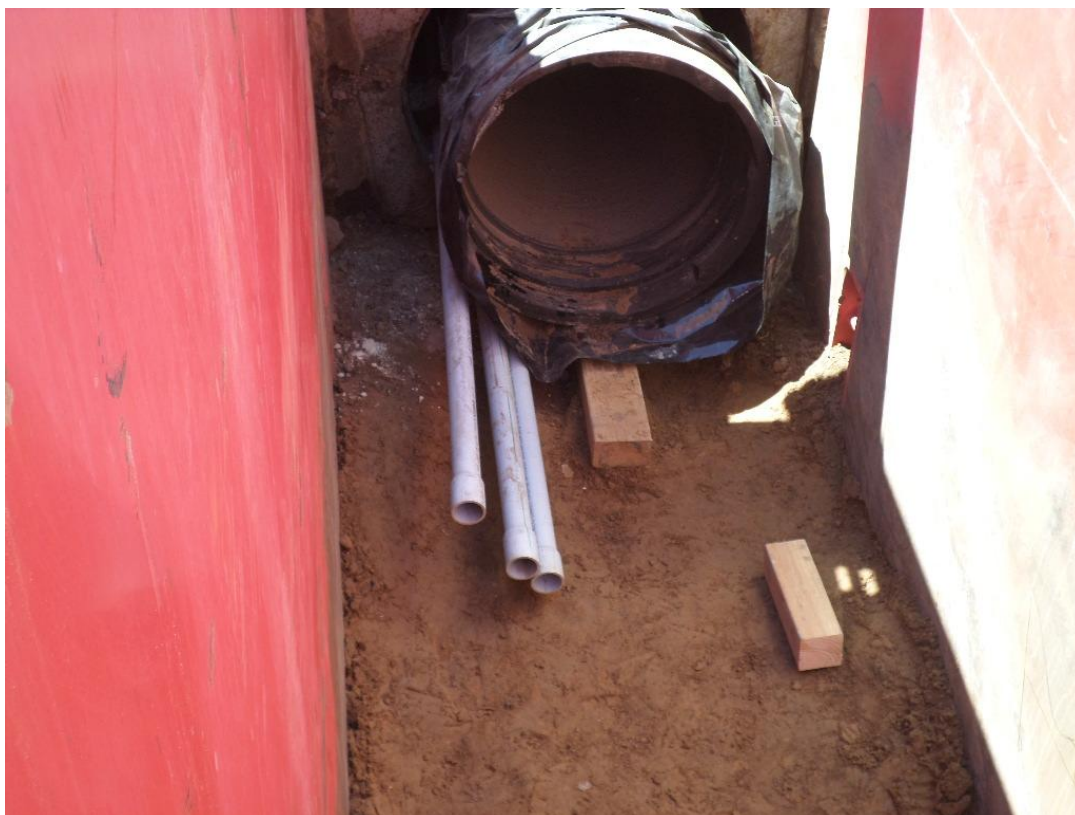
24-inch DIP installed inside casing with three 2-inch conduits for AT&T.
