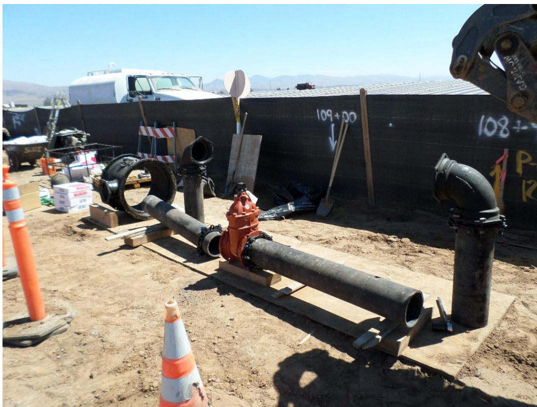
Spiess assembling 8-inch bypass piping.
