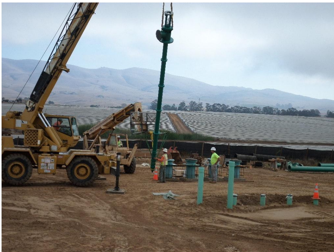
Spiess installing vertical turbine pumps.
