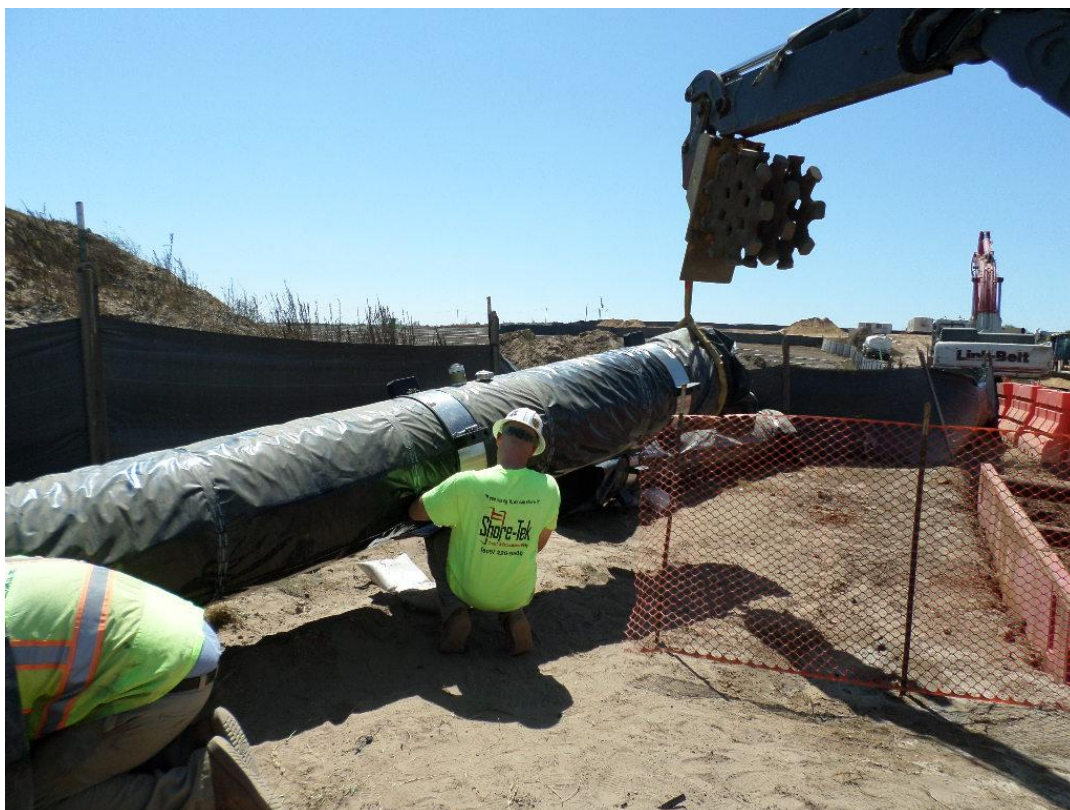
Spies installing pipe spacers on 24-inch DIP to insert the pipe inside of 36-inch steel casing under culverts.
