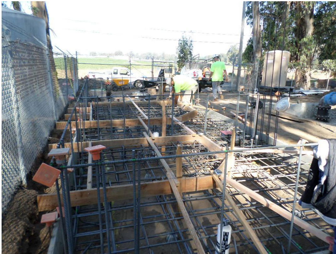
Spiess forming the chemical tank pad.
