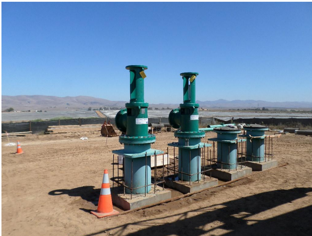
Vertical turbine pumps installed in pump shafts.
