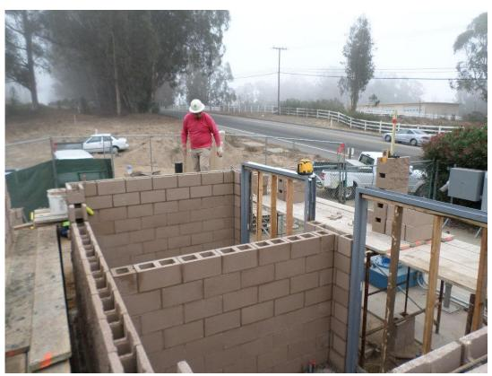
Rocky Boydston Masonry installing second course of block walls at chemical building.
