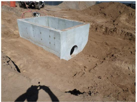
Spiess backfilling around the metering vault.
