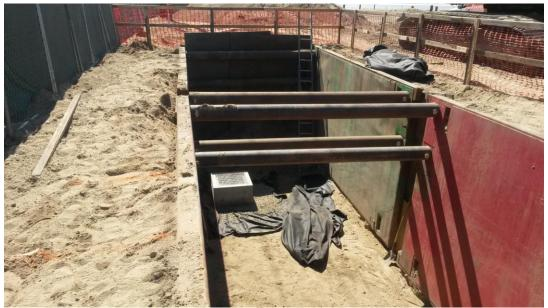
Sump boxes positioned and set for vault placement.
