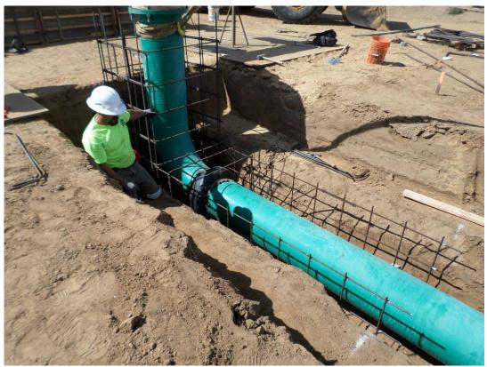
Spiess placing setting discharge pipe inside rebar cage for concrete encasement.
