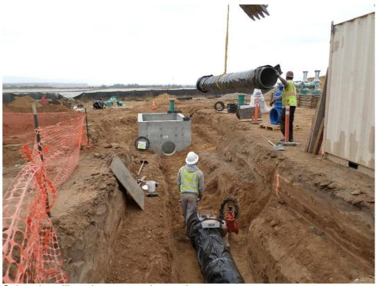
Spiess installing pipe to metering vault.
