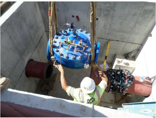
Spiess installing flow control valve.
