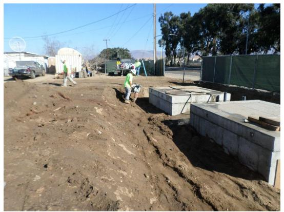
Spiess completing backfill and compaction around vaults.
