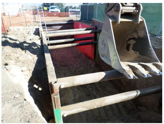
Spiess installing shoring for vaults excavation.
