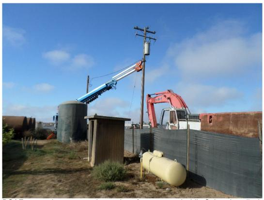
PG&E supporting power pole at edge of access road while Spiess installs the 24-inch DIP.
