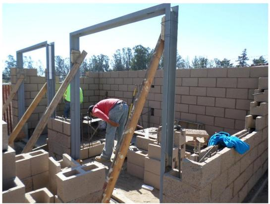
Door frames set by Spiess and Rocky Boydston Masonry constructing block walls at the chemical building up to 5'-4".
