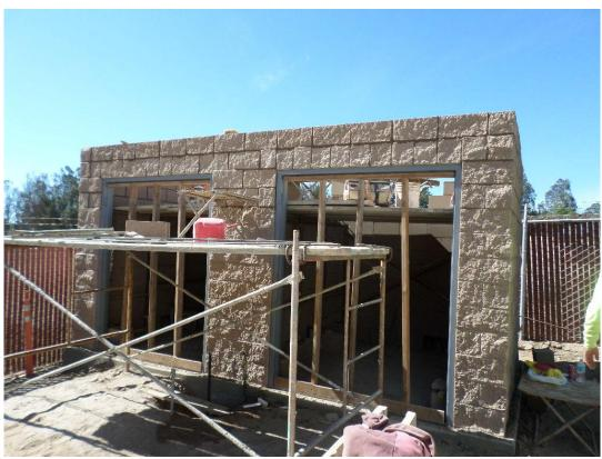
Final course of masonry being completed for the chemical building.
