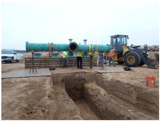
Spiess aligning manifold and excavating for discharge pipe and encasement.
