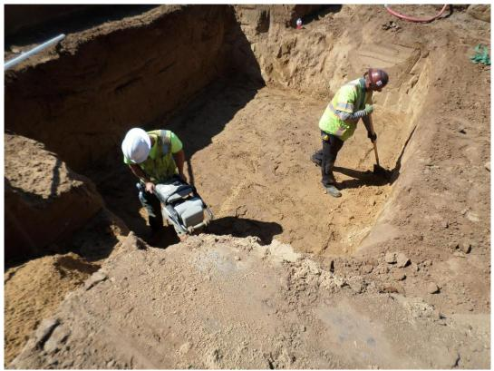
Spiess compacting subgrade for the metering vault.
