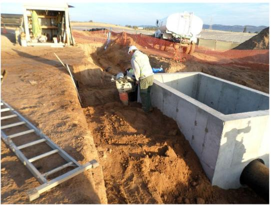
Spiess compacting around the metering vault.
