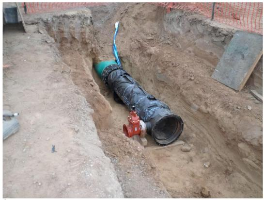
Spiess installing piping toward metering vault.
