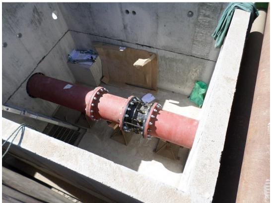
Spiess assembling piping in metering vault.
