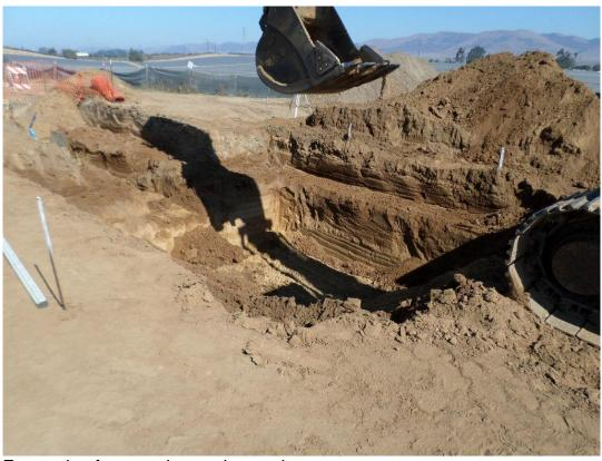
Excavating for metering station vault.
