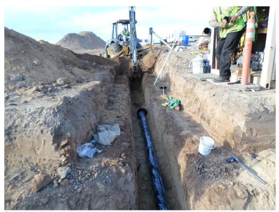
Spiess installing 6-inch DIP for the fire hydrant located on site.
