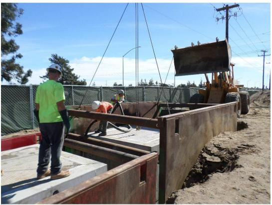
Spiess pouring slurry around vaults for backfill.
