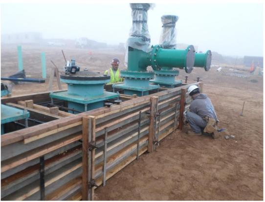
Forms installed for pump pedestals.
