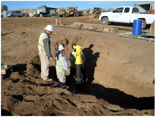
Spiess installing the fire hydrant.
