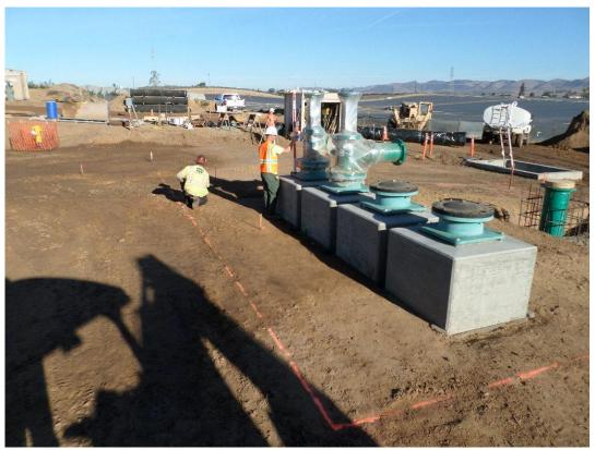
Pump pedestals poured and forms removed. Spiess laying out pump station building foundation.
