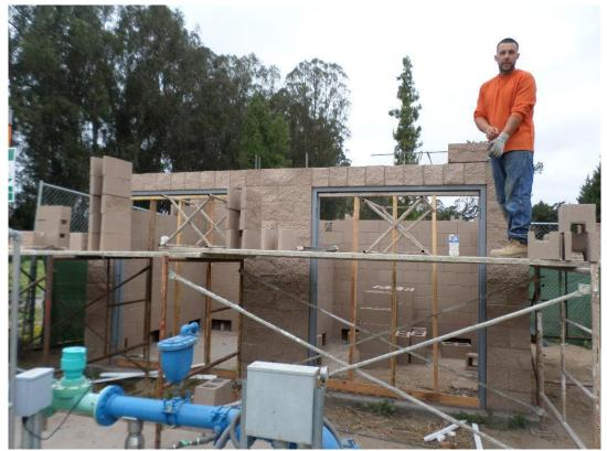
Rocky Boydston Masonry installing second course of block walls at chemical building.
