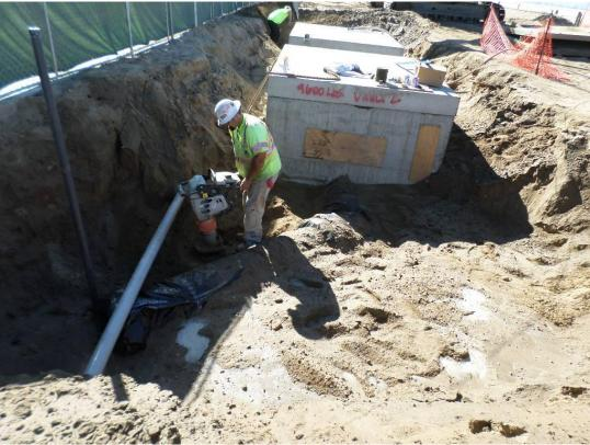
Piping to and from vaults installed and Spiess backfilling and compacting around piping and 4-inch Verizon line.
