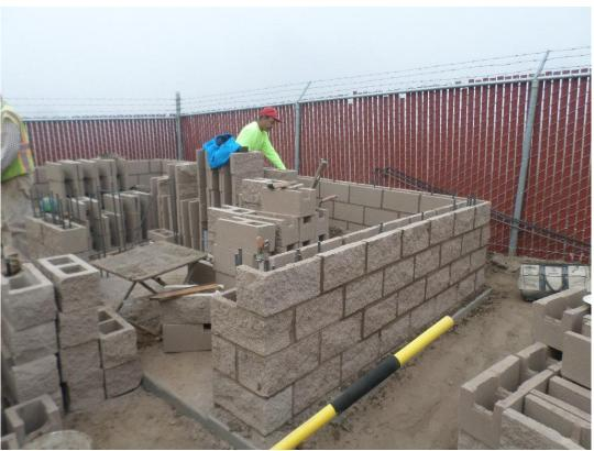
Rocky Boydston Masonry installing first course of block walls for the chemical building.
