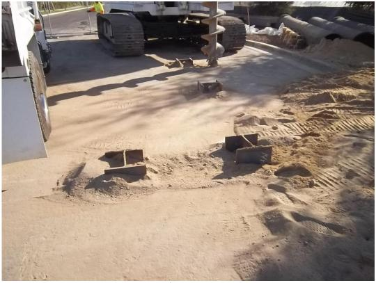
I-beams in place in Blosser Road for steel plate supports in the receiving pit.
