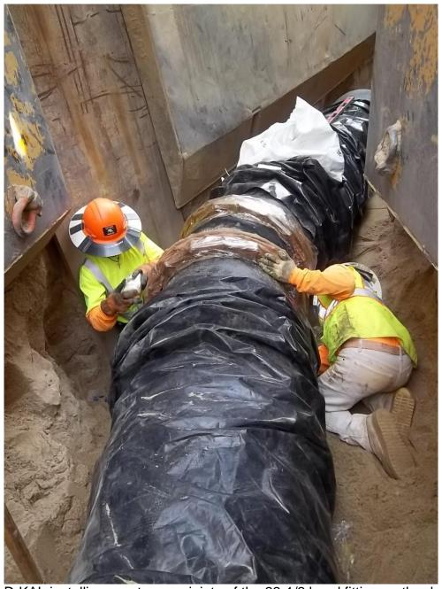
D-KAL installing wax tape on joints of the 22-1/2 bend fitting on the deep trench pipe.
