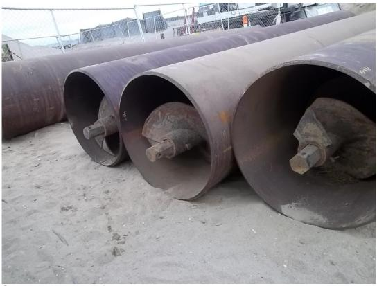
Steel casing staged for installing into bore and jack pit, with auger sections inside.
