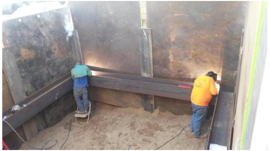
D-KAL welding horizontal supports for shoring inside receiving pit.
