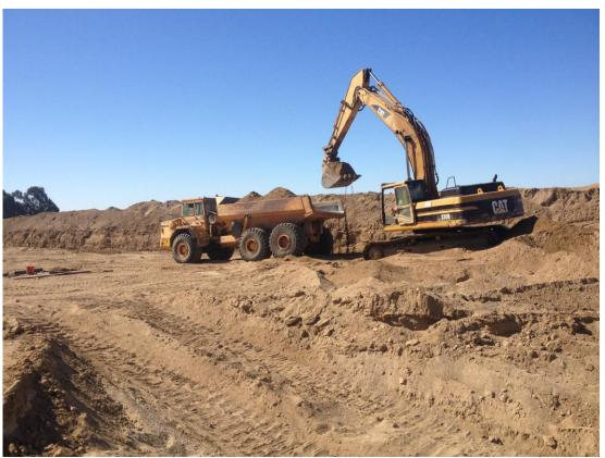
D-KAL hauling native material off-site to be screened and returned for use as backfill.
