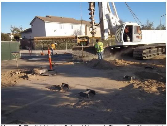
Meyers Drilling finishing installation of I-beams in Blosser Road for steel plate supports in receiving pit.
