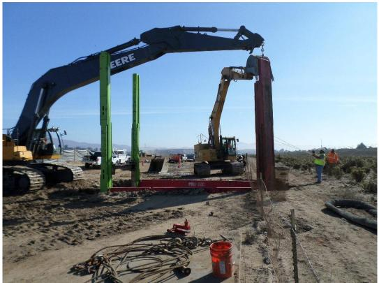
D-KAL excavating bore and jack pit and installing slip shoring.
