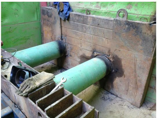
Pacific Boring installing back brace located behind the bore and jack machine.
