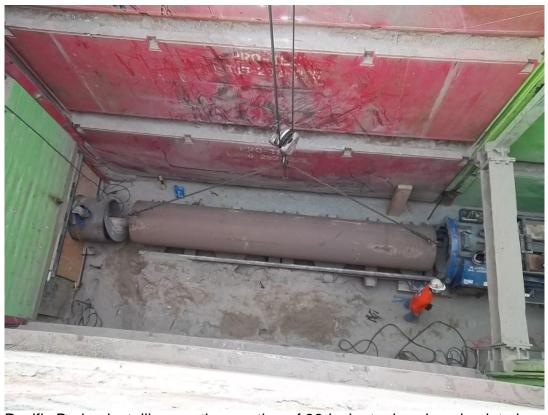
Pacific Boring installing another section of 36-inch steel casing pipe into bore and jack pit.
