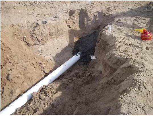
D-KAL pouring temporary thrust blocks on relocated irrigation line.
