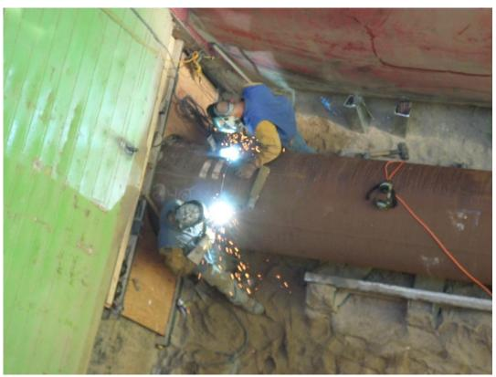
Pacific Boring welding another section of 36-inch casing to the one installed.
