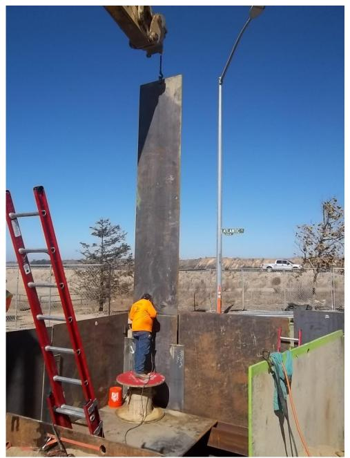
D-KAL welding second layer of steel plates at receiving pit.
