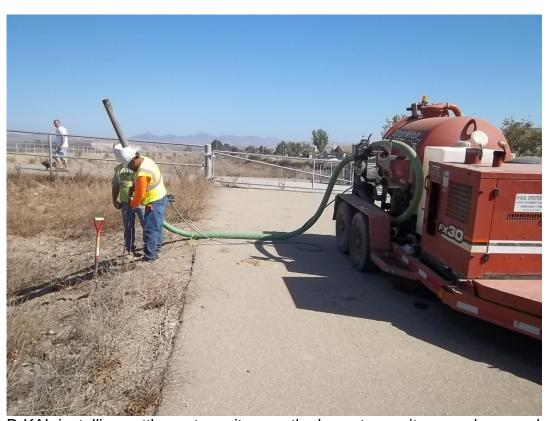
D-KAL installing settlement monitors on the levee to monitor any changes during the bore and jack operation.
