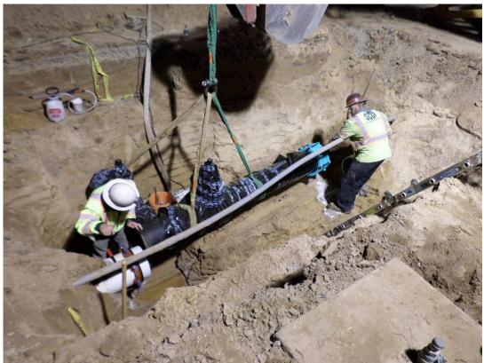
Spiess installing the first section of the bypass on the existing 12-inch PVC pipe.
