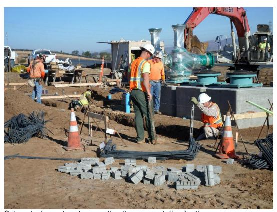
Spiess laying out and excavating the pump station footing.
