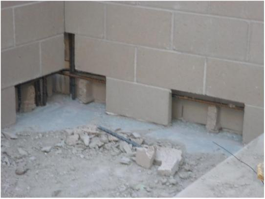
Boydston Masonry cleaning out the block walls in preparation for grouting.
