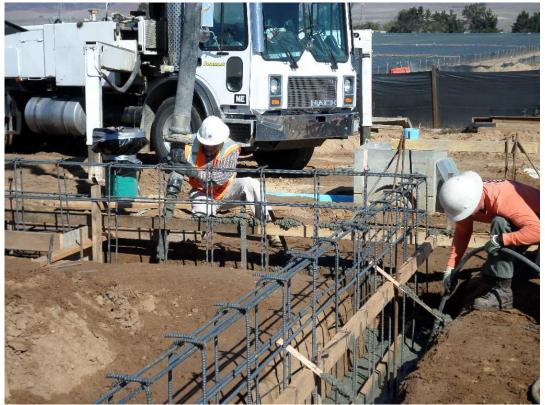
Spiess pouring the exterior footings for the pump station.
