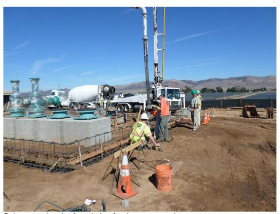
Spiess pouring the foundation for the pump station.
