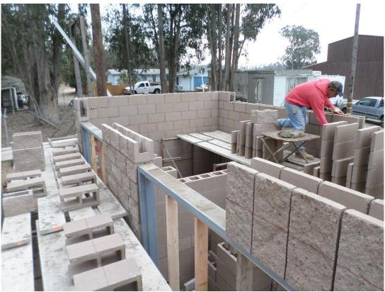
Boydston Masonry installing final course for walls at the chemical building.
