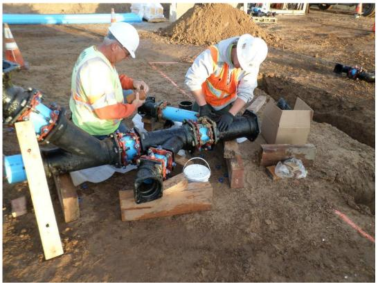
Applying wax tape to drain piping.
