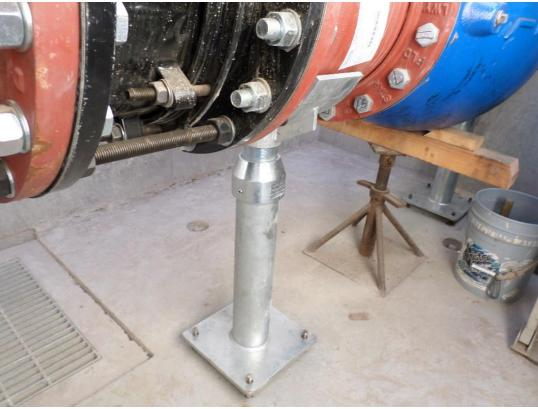
Pipe supports being installed inside the metering vaults.
