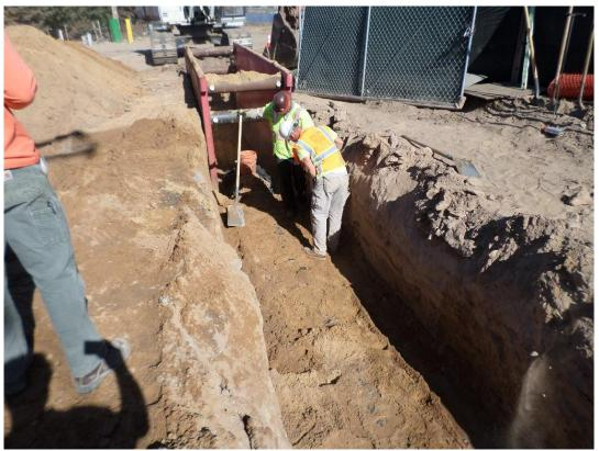
Spiess compacting last section of 24-inch DIP installed in the access road.
