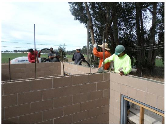
Boydston Masonry grouting walls of chemical building.
