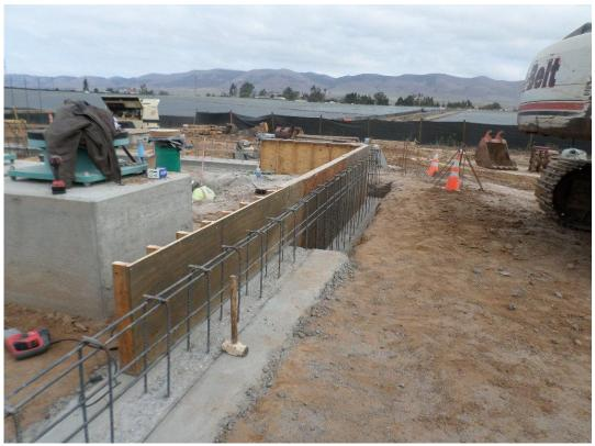
Spiess forming the stem wall for the pump station.
