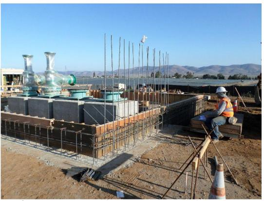
Vista Steel installing more reinforcing at the stem walls of the pump station.
