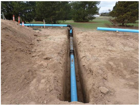
Spiess installing the 8-inch PVC bypass line.
