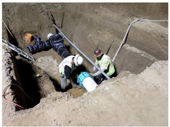
Spiess installing second section of the bypass on the existing 12-inch PVC waterline.
