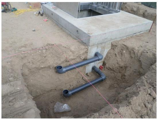
Vent pipes installed at the metering vaults.
