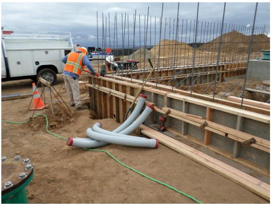
Spiess forming stem wall and St. Dennis Electric installing conduit underneath the future pump station slab.
