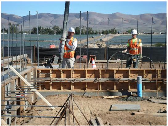
Spiess pouring the stem walls at the pump station.
