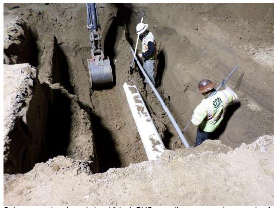
Spiess exposing the existing 12-inch PVC waterline at second connection for the bypass.
