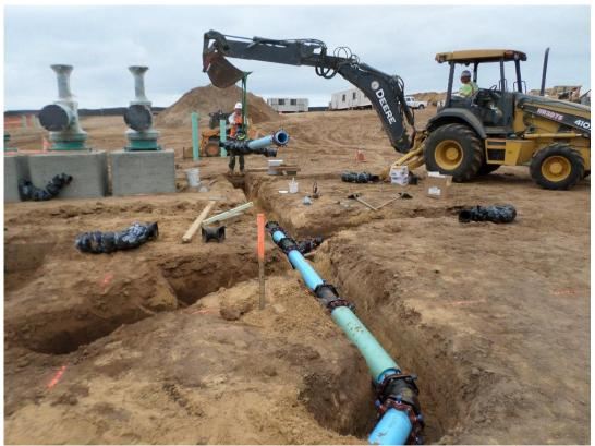
Spiess installing drain pipe for underneath the pump station slab.
