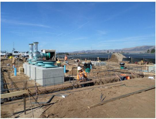
Vista Steel installing reinforcing for the pump station footing and stem wall.
