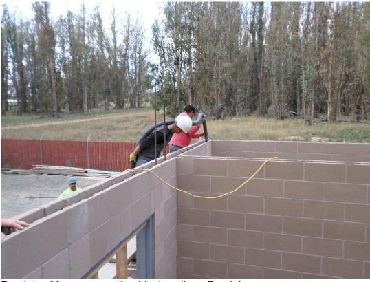
Boydston Masonry grouting block walls at Sundale.
