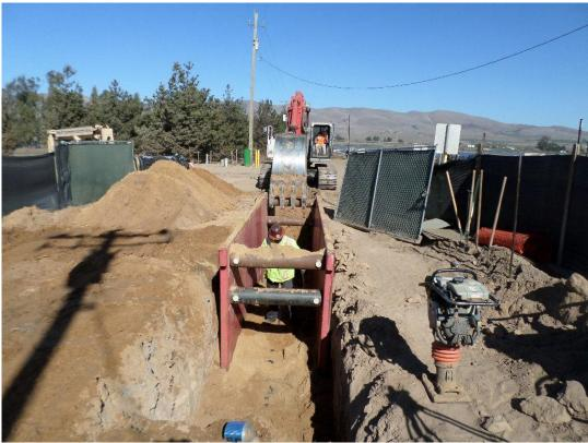
Spiess finishing installation of the 24-inch DIP in the access road.
