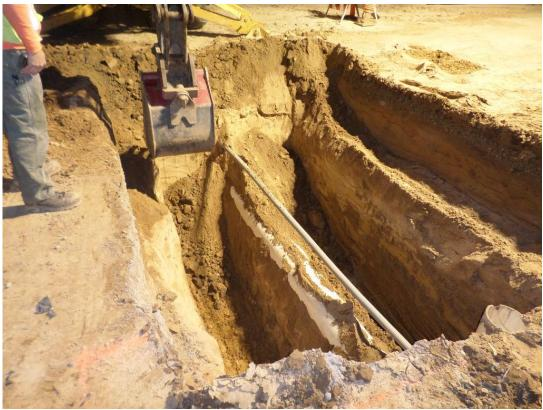
Spiess exposing the 12-inch PVC waterline for installing the temporary bypass.
