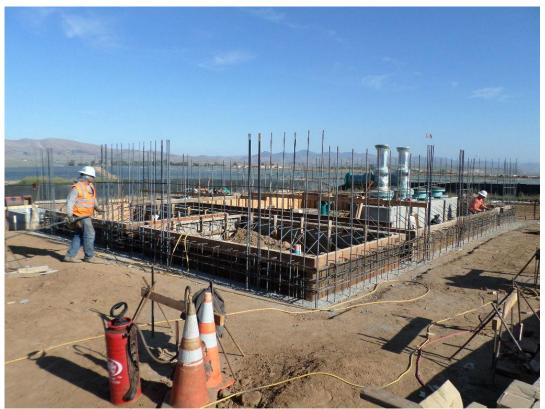
Vista Steel installing reinforcing at the pump station stem walls.
