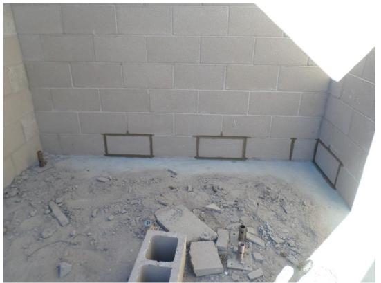
Clean out cells in block walls sealed and ready for grouting.
