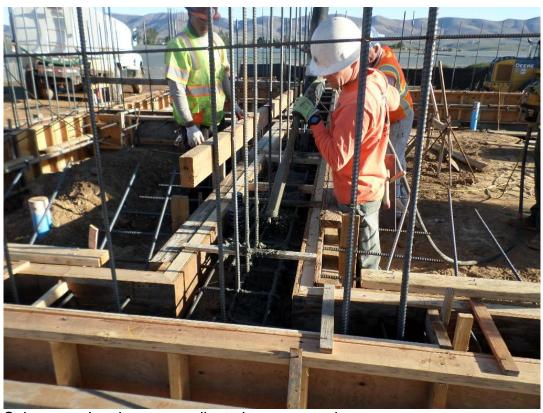
Spiess pouring the stem walls at the pump station.
