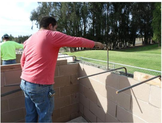
Boydston Masonry grouting walls and installing rebar for connection to future roof.
