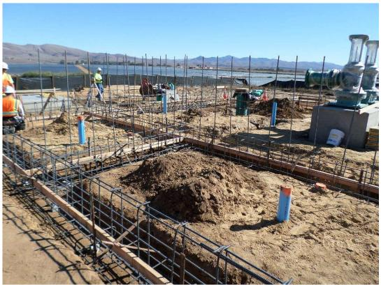
Installing forms for pump station foundation.
