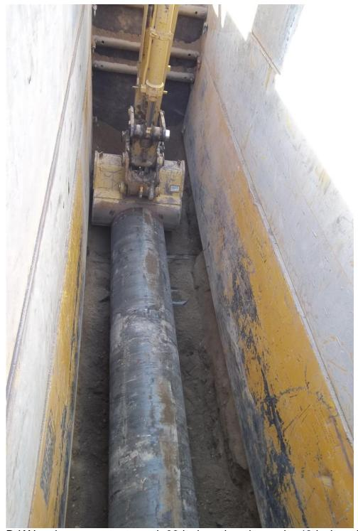
D-KAL using excavator to push 36-inch casing pipe under 48-inch and 72-inch storm drain pipes.
