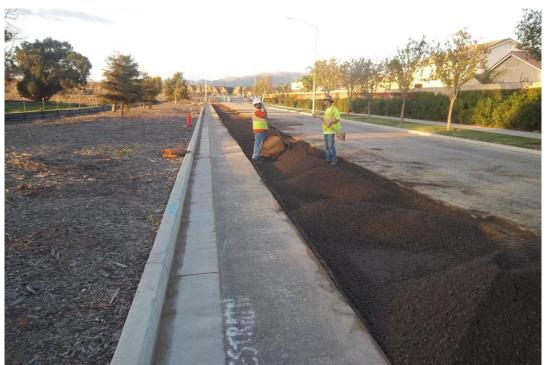
D-KAL spreading base over trench in preparation for final paving.
