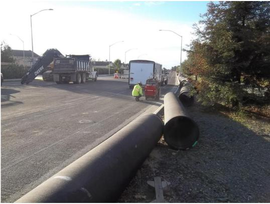
D-KAL sawcutting existing pavement for trench excavation.
