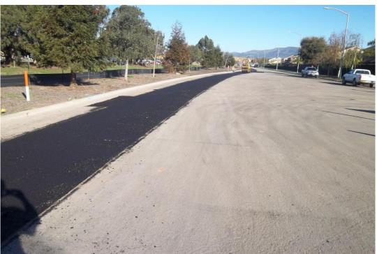
Ramsey Asphalt rolling final pavement over trench.
