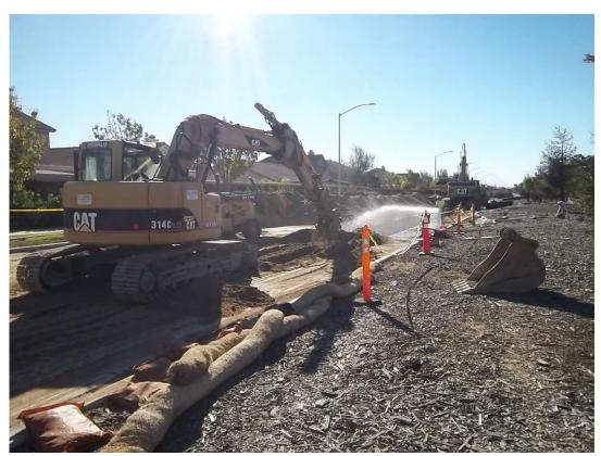
D-KAL compacting backfill in trench.
