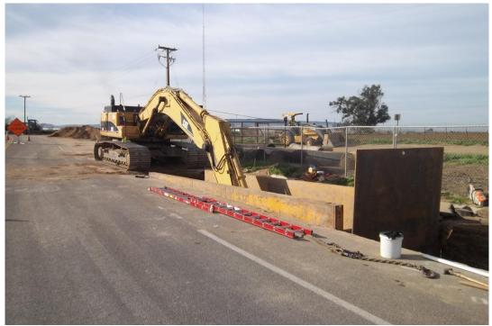
D-KAL using excavator to push 36-inch casing under storm drain pipes in Blosser Road.
