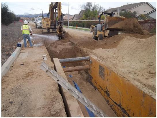
D-KAL backfilling and compacting trench.
