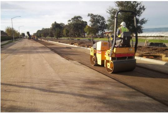
D-KAL compacting base prior to final paving.
