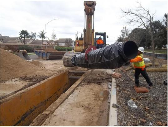
D-KAL installing a section of 24-inch DIP.
