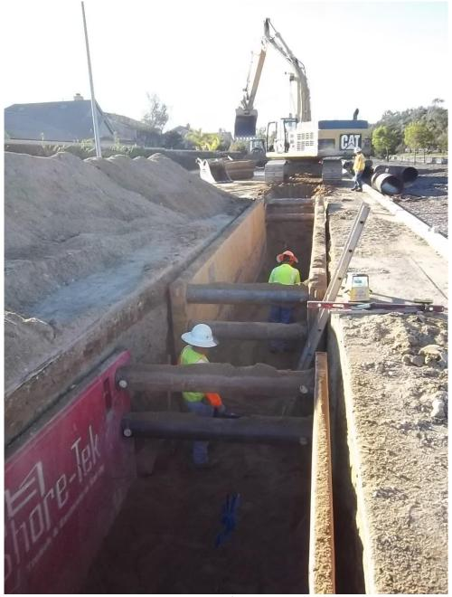
D-KAL installing pipe going south of receiving pit in Blosser Road.
