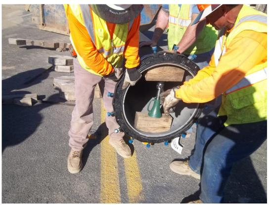
D-KAL using pipe jacking method to get pipe end to fit inside megalug for butterfly valve installation.
