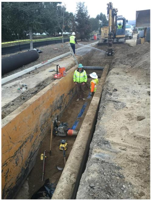
Fugro on site taking compaction tests.
