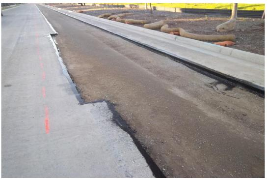
Edges of existing pavement oiled in preparation for final paving.
