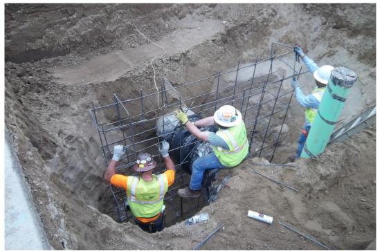
D-KAL installing reinforcing for thrust collar for butterfly valve at Station 42+42.
