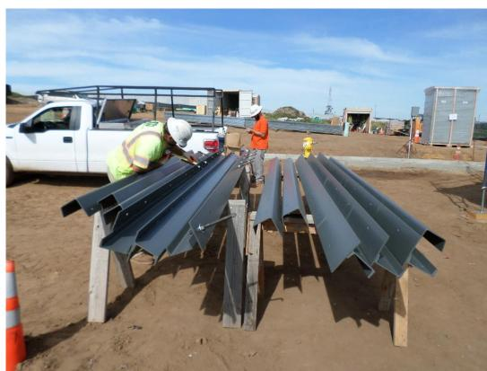
Spiess attaching bolts to roof steel plates.
