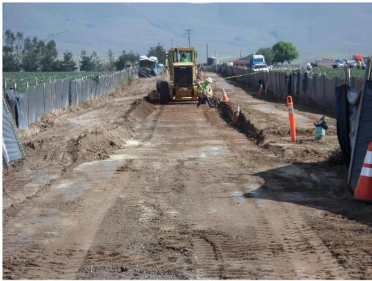
Spiess cutting the access road to subgrade to build permanent access road.
