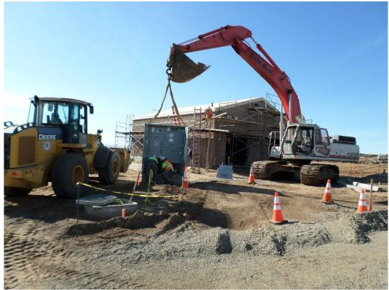
St. Denis Electric installing PG&E metering station.
