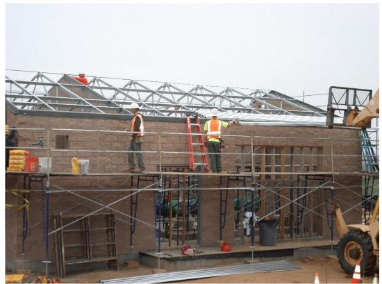
Spiess installing the steel deck for the roof.
