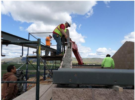
Spiess setting steel roof plates during final wall grout.
