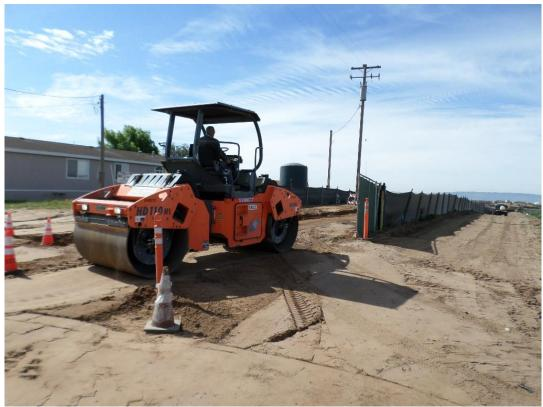
Spiess compacting subgrade to construct permanent access road.
