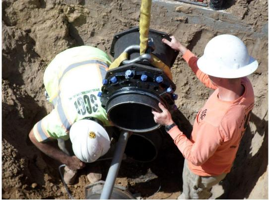
Spiess making the final tie-in to the 12-inch water line at the PRV vault.
