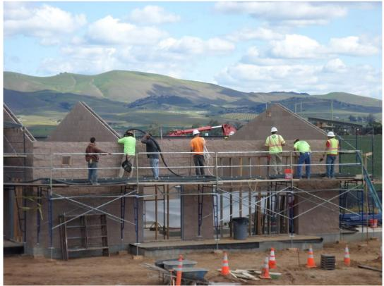
Boydston Masonry pouring final grout while Spiess set steel plates for roof.
