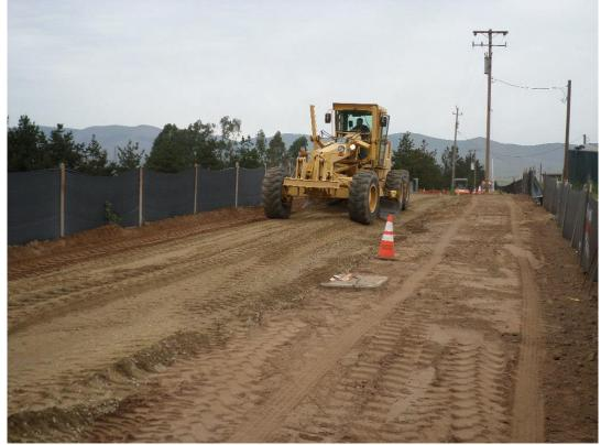
Spiess placing base to construct permanent access road.
