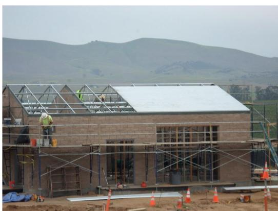
Spiess installing the steel deck for the roof.
