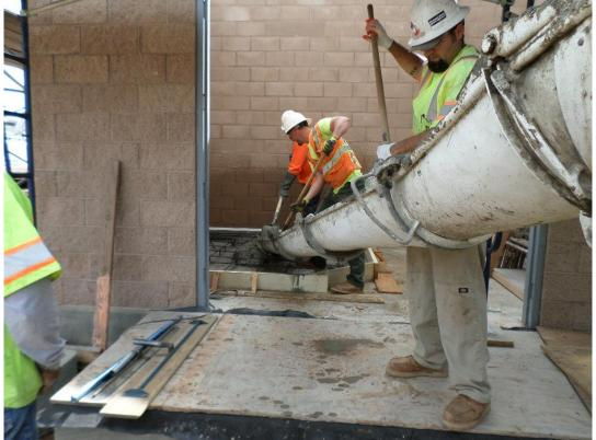
Spiess pouring chemical tank pad in Sodium Hypochlorite Room at pump station.
