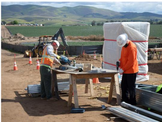
Spiess fabricating steel framing for roof at pump station.
