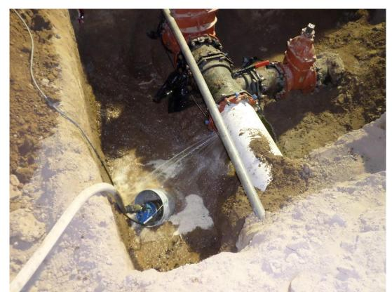
Spiess performing night work to drain the District's existing 12-inch water line and remove tee used for temporary bypass.
