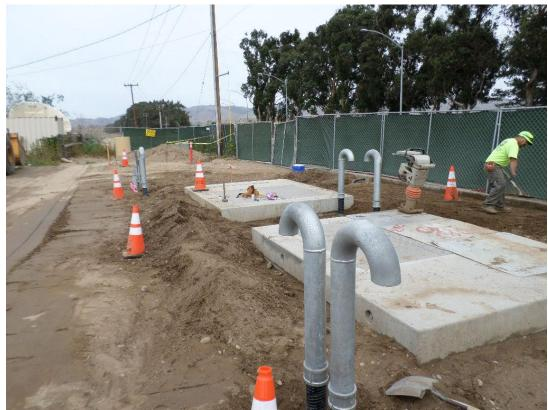
Spiess installing vent piping at metering vaults.
