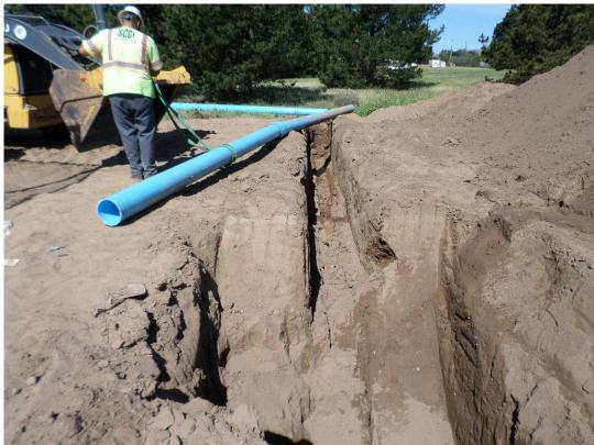
Removing temporary bypass piping after the final tie-in was completed at the PRV vaults.
