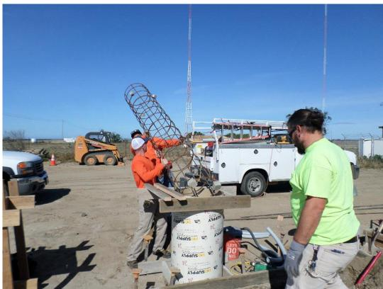
Spiess installing forms and reinforcement for light pole base.
