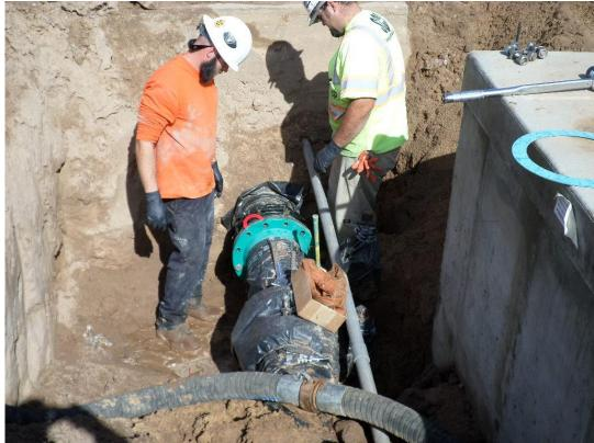
Spiess removing the test plate from piping at the PRV vault.
