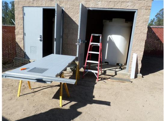
Doors being trimmed by manufacturer to make final fit with door frame.
