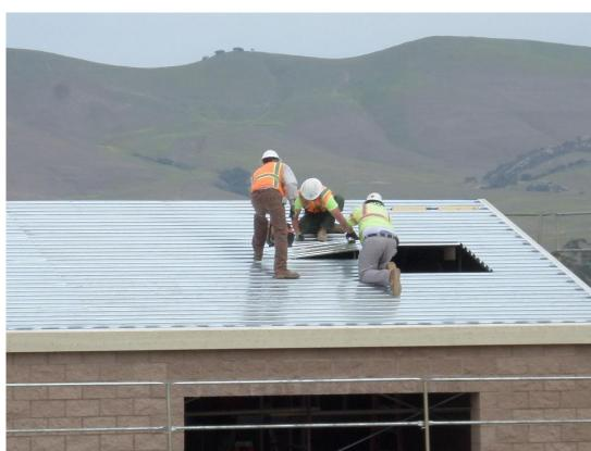
Spiess cutting openings for roof hatches.
