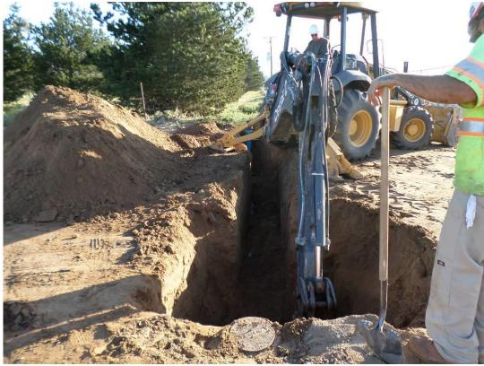
Spiess excavating to remove temporary bypass piping at PRV vault.
