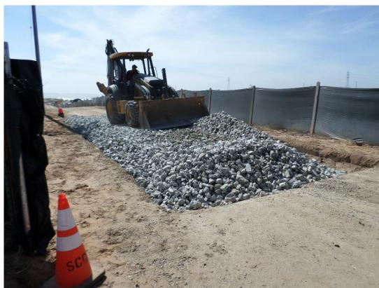
Spiess installing tracking control at the beginning of the permanent access road.
