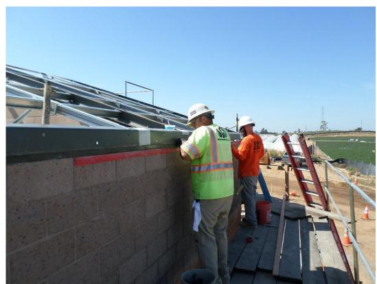
Spiess dry packing grout under steel roof frame plate.
