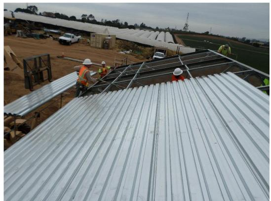
Spiess installing the roof deck at the pump station.
