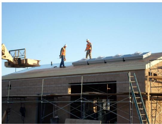
Spiess installing plywood sheeting on pump station roof around hatches.
