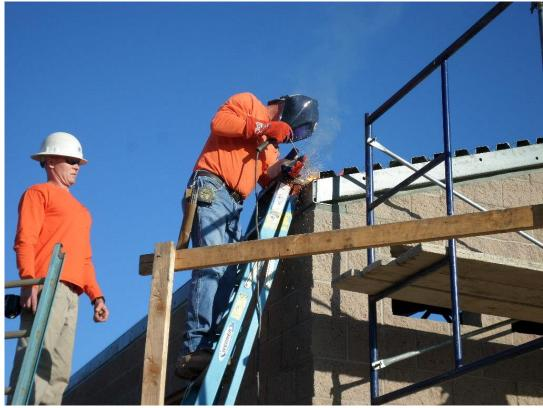
Puddle welding at steel roof plates.
