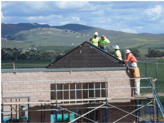
Spiess installing steel roof plates during final wall grout.
