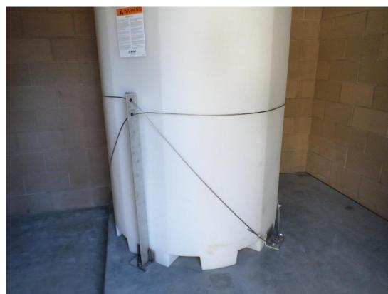
Chemical tank installed with tie-downs.
