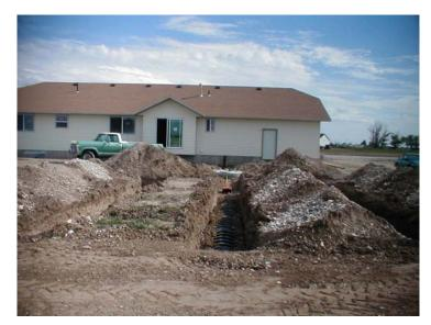
After the septic tank has settled out solids, clarified wastewater is dispersed through perforated pipes into the soil. Soil is the key to clean water. It acts as a physical strainer, chemical renovator and biological recycler for the wastewater passing through it.
