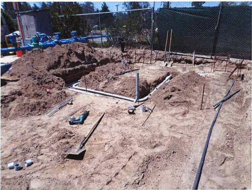
Spiess installing underslab piping.
