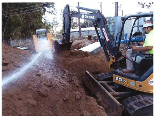
Spiess backfilling and compacting under the future chemical building slab.
