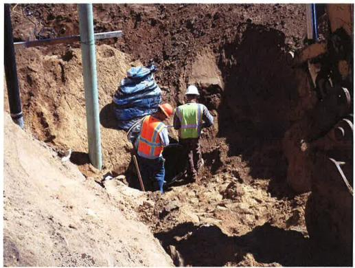
Spiess installing flange adapter on 24-inch DIP.
