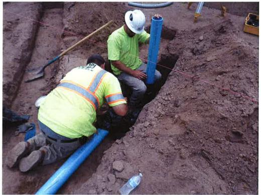
Spiess installing 4-inch drain line.
