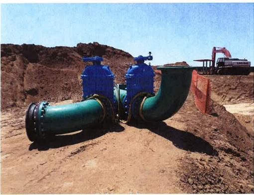
Pig outlet assembled and ready to set into place.
