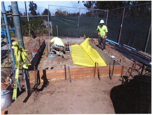
Spiess installing underslab vapor barrier.
