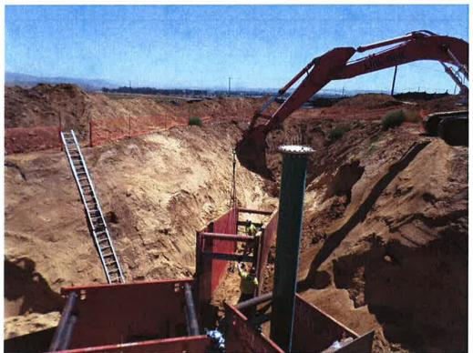
Spiess removing shoring around the pig launch and riser.
