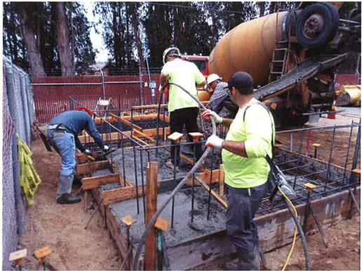
Spiess placing concrete for chemical building slab.
