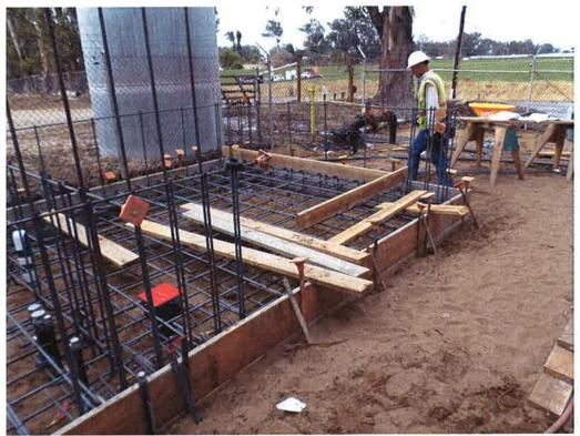
Spiess forming equipment pads on top of chemical building slab.
