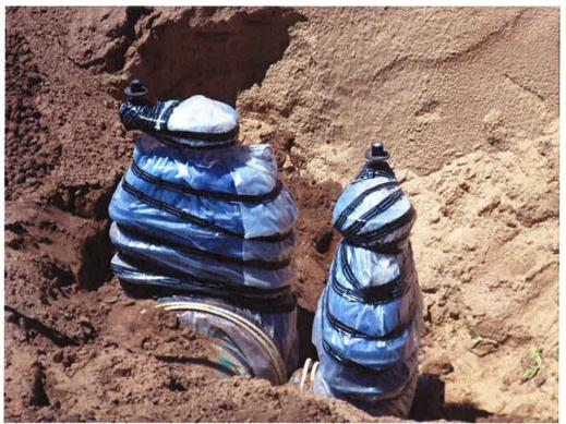
Spiess wrapping valves with plastic before backfilling.
