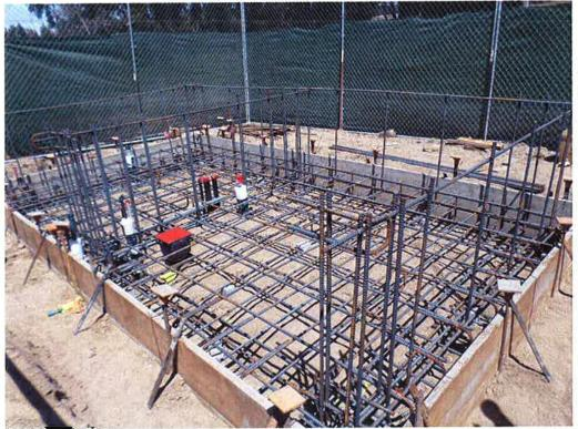
Reinforcing installed for chemical building slab.
