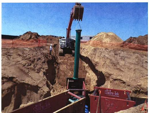
Spiess setting the pig launcher riser.
