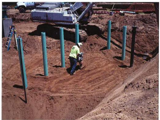
Spiess compacting around the valve can risers.
