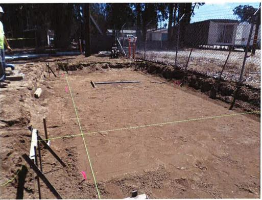
Laying out the chemical building slab foundation.
