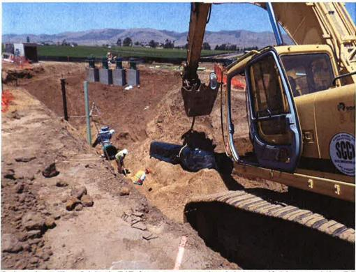
Spiess installing 24-inch DIP from pump station inlet manifold toward the BP #1 connection.
