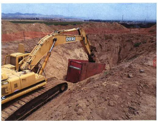
Spiess setting shoring for installing 24-inch DIP for future connection to the HDPE pipe installed as part of Bid Package #1.
