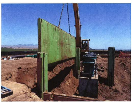
Removing shoring from around the pump cans.
