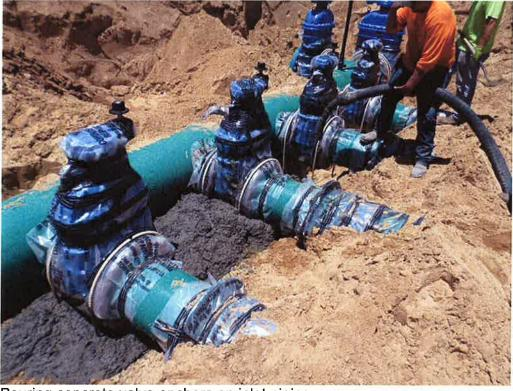
Pouring concrete valve anchors on inlet piping.
