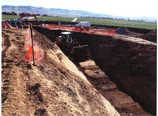
Spiess backfilling over 24-inch DIP.
