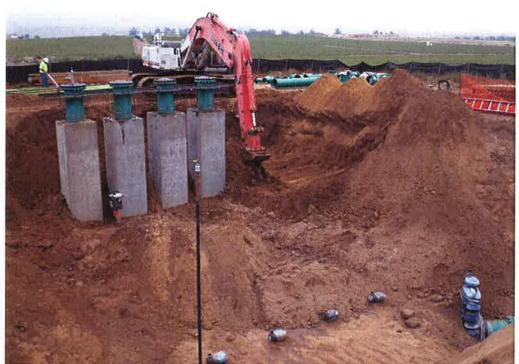
Spiess continuing backfill around the pump cans.
