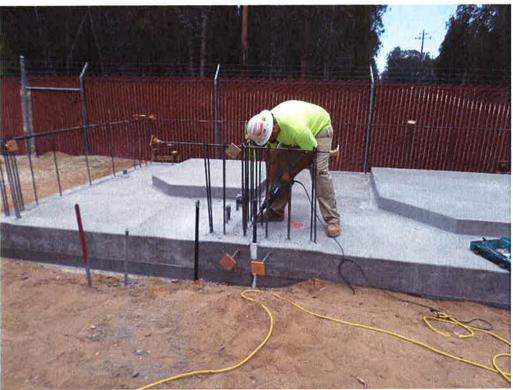
Spiess roughening concrete on building slab in preparation for placement of the concrete block.
