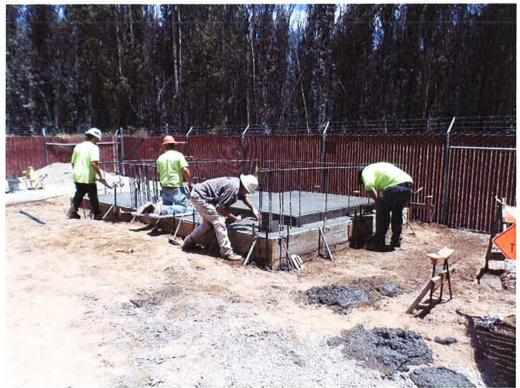
Spiess finishing concrete at chemical building slab.
