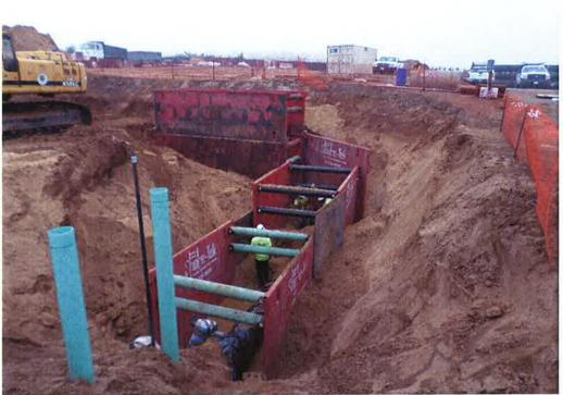
Spiess installing pipe extension to future tank outlet piping.
