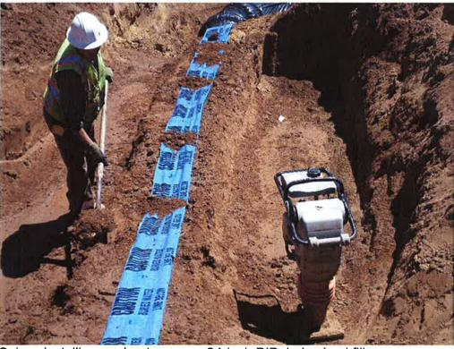
Spiess installing marker tape over 24-inch DIP during backfill.
