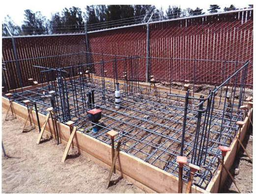
Spiess subcontractor Vista Steel installing reinforcing for chemical building slab.
