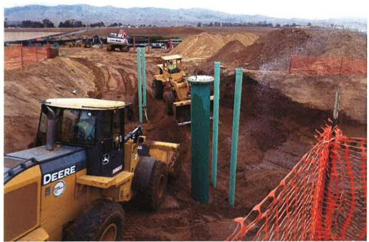
Spiess backfilling around installed valve can risers.
