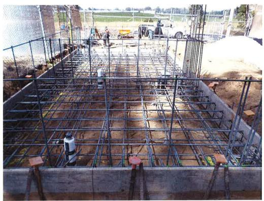
Chemical pad reinforcing installed by Vista Steel.
