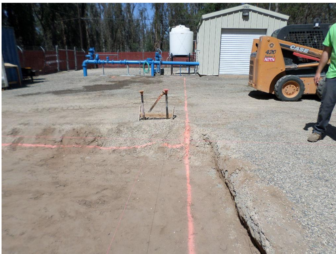
Laying out pipe trenches.
