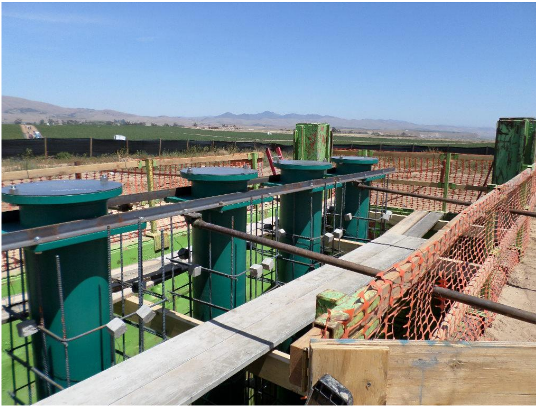
Spiess installing stabilizing structure/bracing to the tops of the pump cans.
