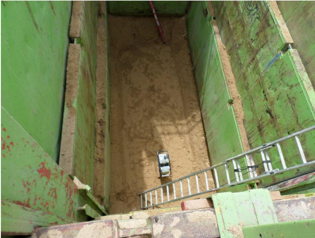
Spiess compacting the bottom of the excavation for the pump cans approximately 23 feet below grade.
