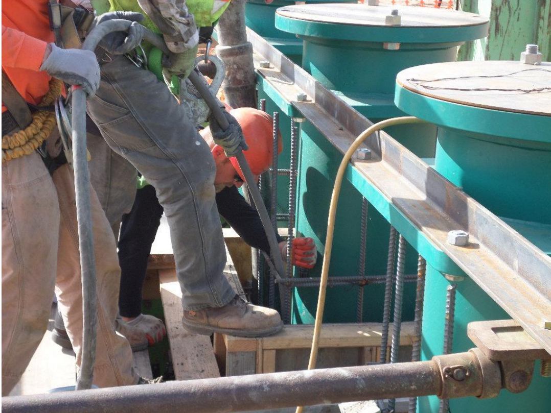
Spiess monitoring and vibrating concrete placement during pour of pump can encasements.
