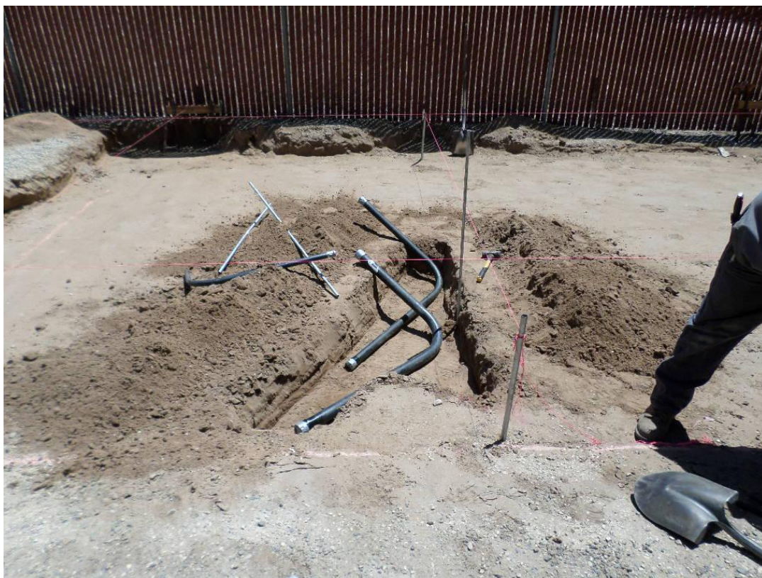
St. Dennis Electric starting underslab conduit installation.
