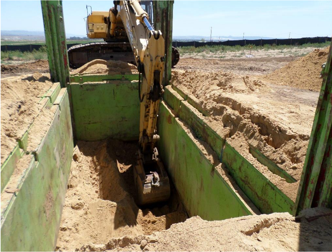
Spiess excavating inside shoring for pump can installation.
