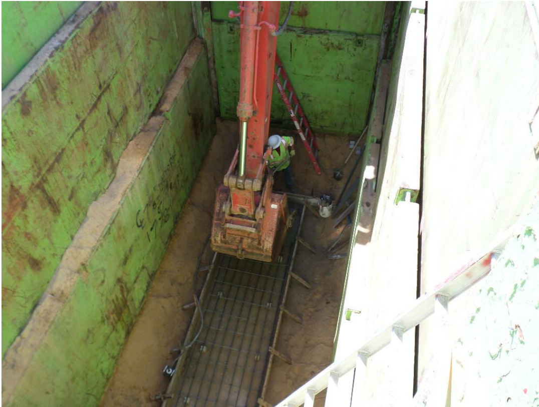
Spiess using excavator to place concrete for slab to set pump cans on top of.
