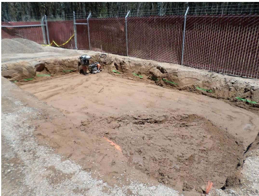
Spieß over excavating and compacting for slab under the chemical building.
