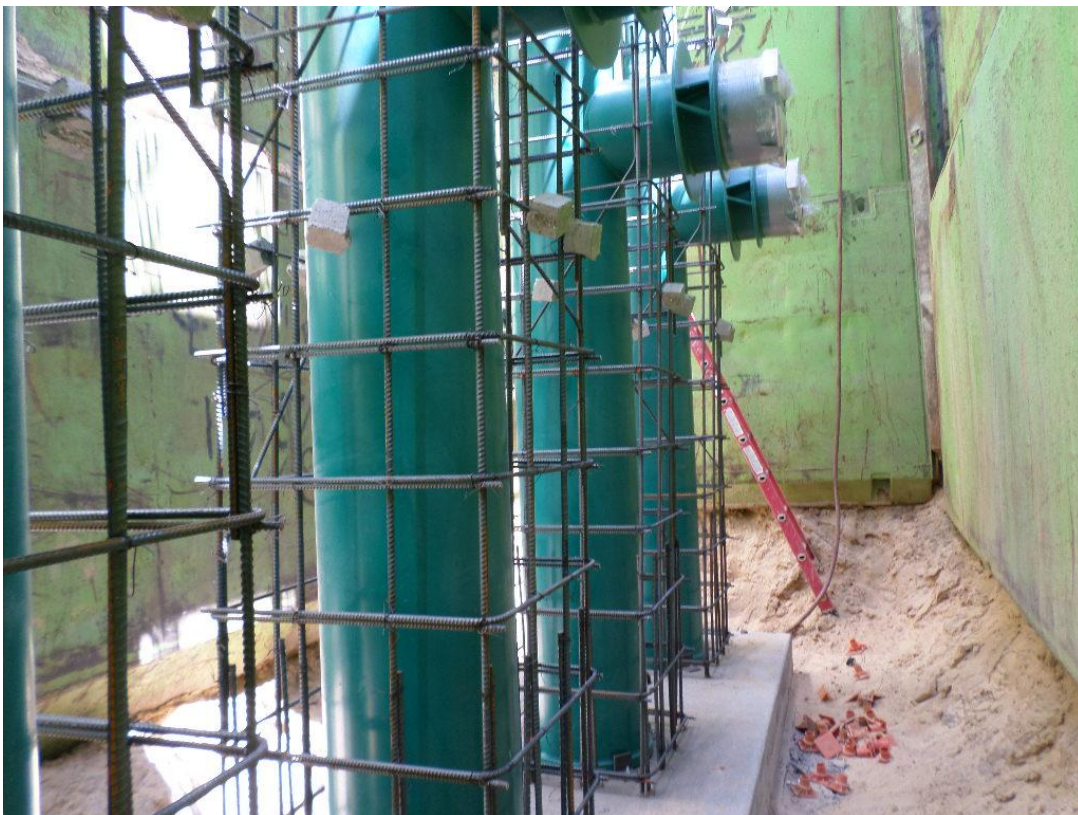
Reinforcing being installed for pump can encasements by Spiess subcontractor Valley Steel.
