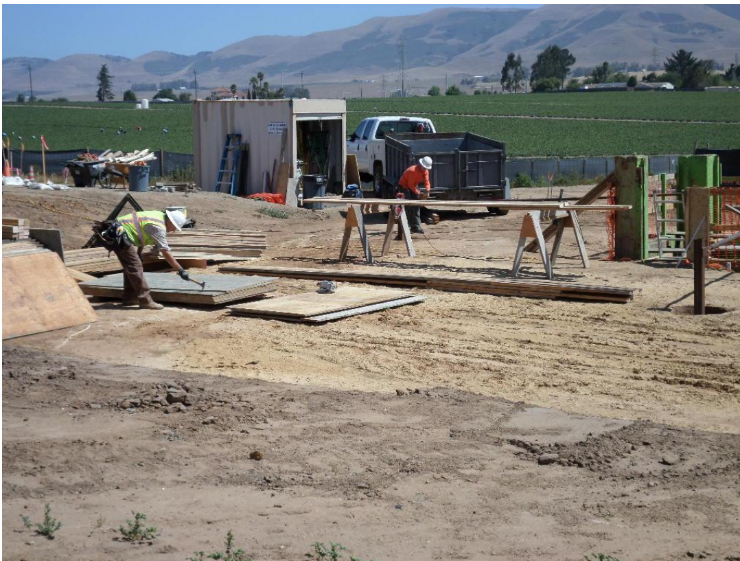
Spiess constructing forms for pump can encasements.
