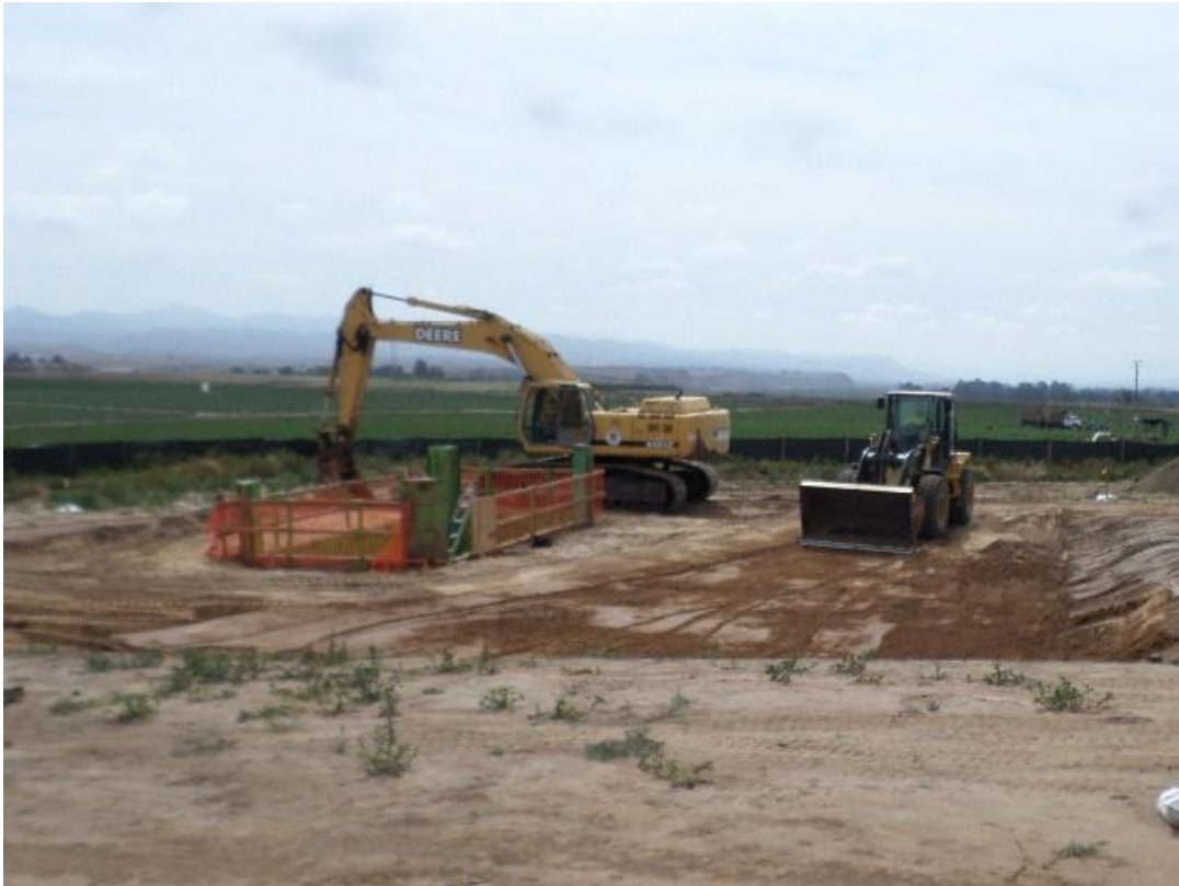
Spiess grading around excavation to prepare for installing supports to stabilize the pump cans when they are set.
