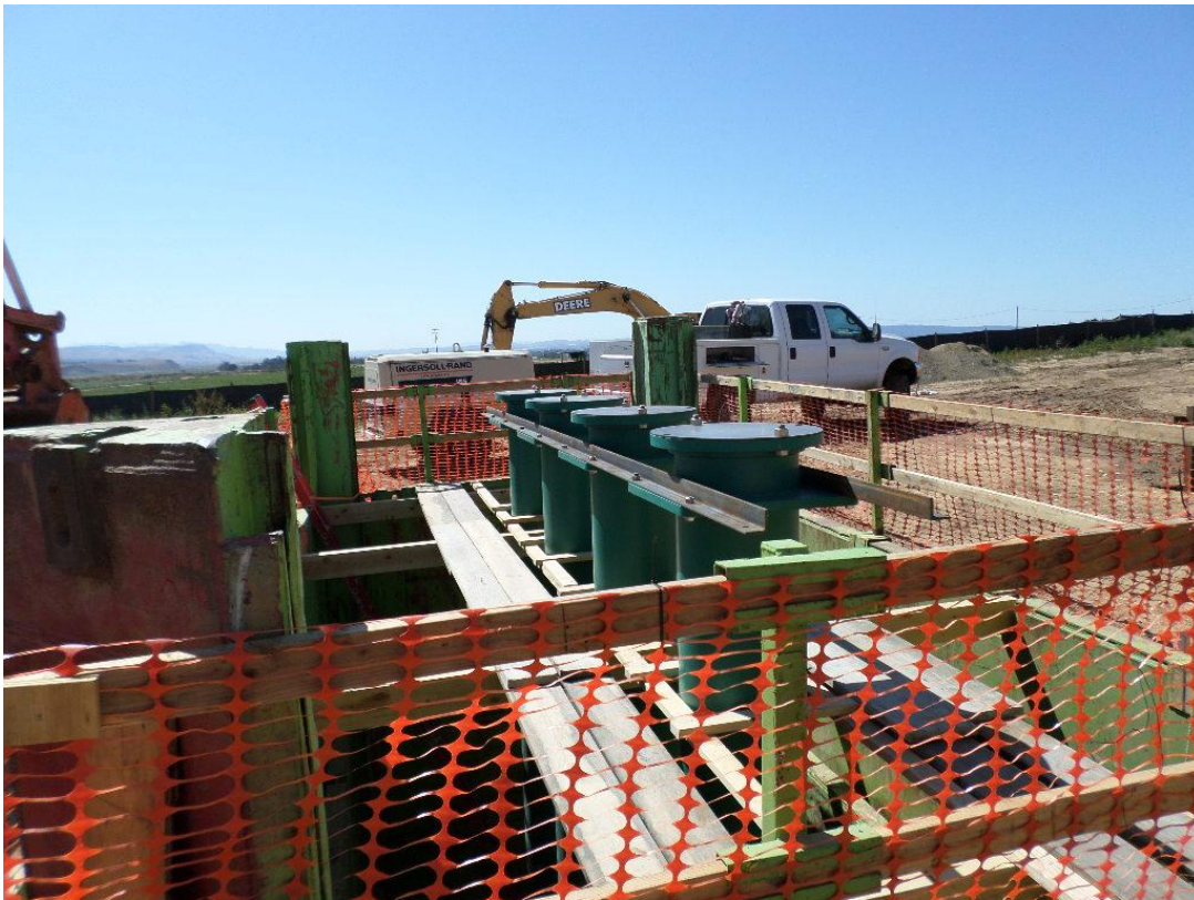
Spiess using steel angle iron to secure spacing of the pump can tops.
