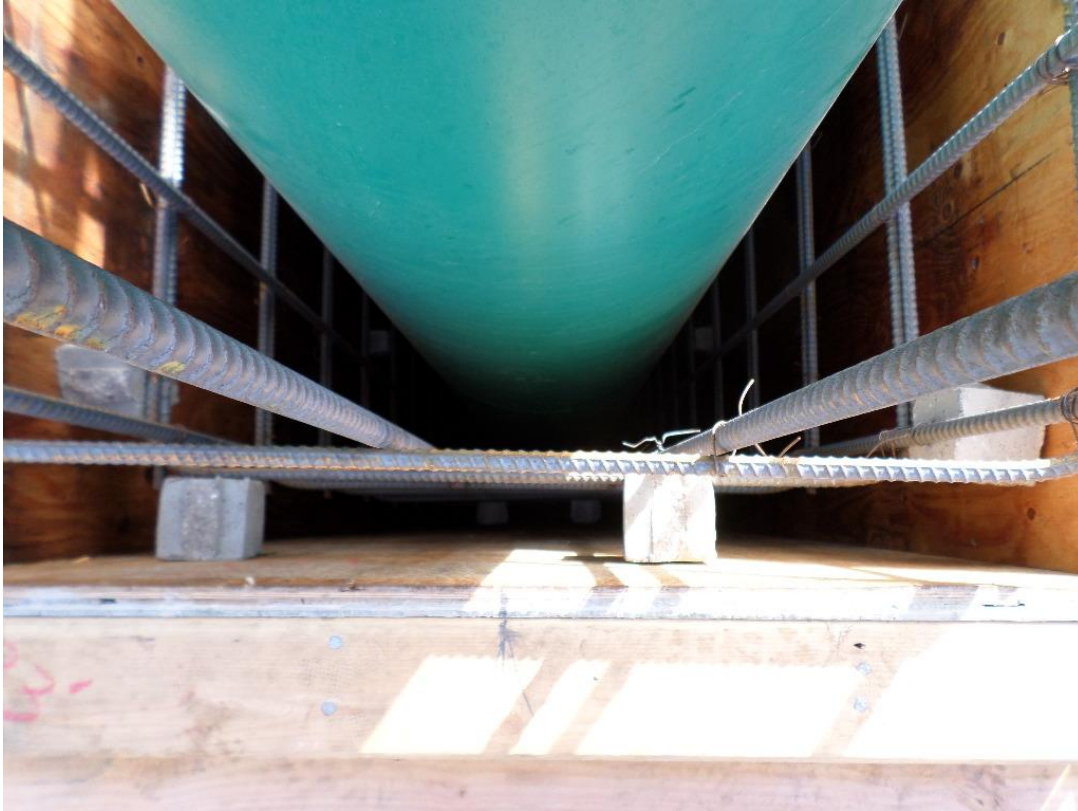
MNS verifying rebar and form spacing prior to Spiess pouring pump can encasements.
