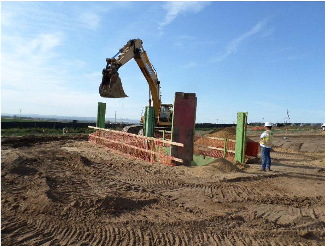
Spiess continuing excavation for pump cans and installing vertical shoring with shoring representative on site from Shoring Tech.
