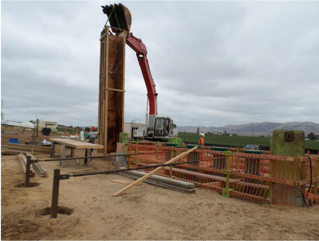
Spiess installing pump can encasement forms.
