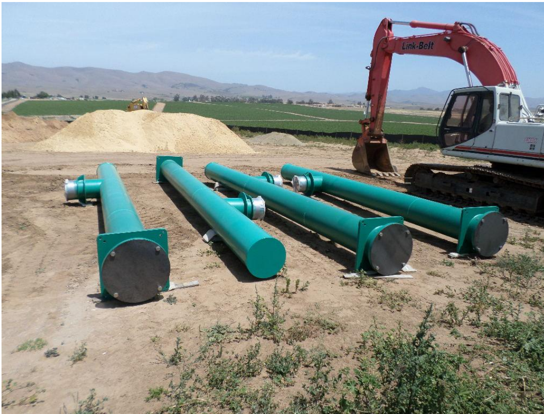
Pump cans delivered to site and coating inspected for thickness and any damage.
