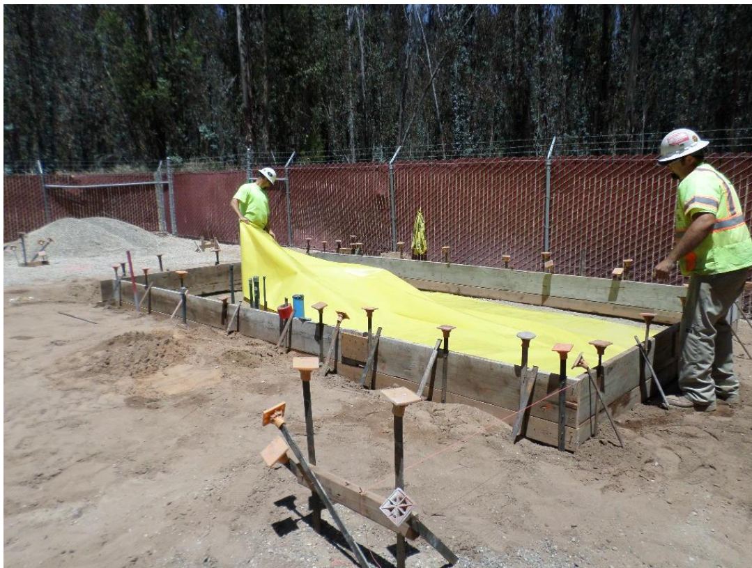
Spiess placing underslab vapor barrier at Chemical Building slab.
