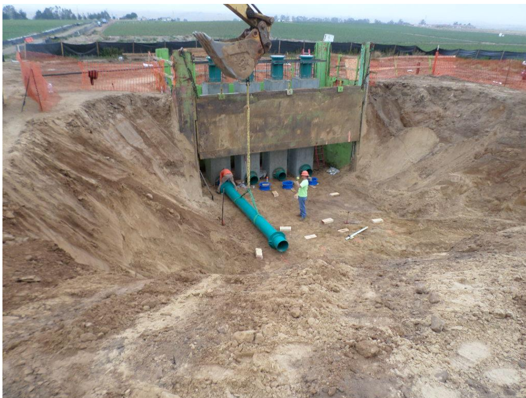
Spieß starting installation of 16-inch coated steel suction piping.
