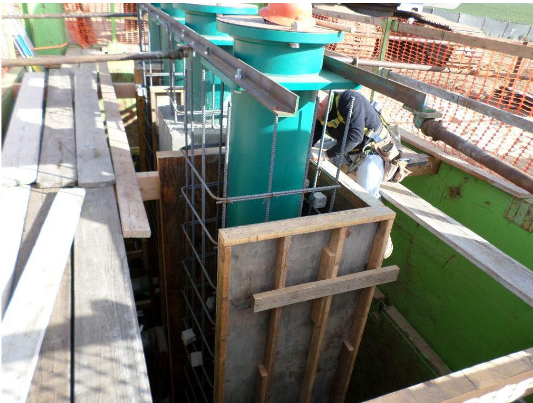
Spiess installing forms for pouring encasements at around the last two pump cans.
