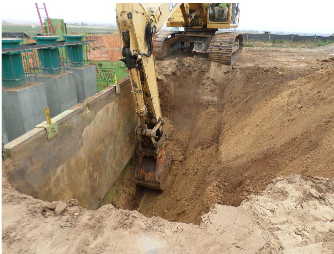
Spiess excavating and cutting back sides for installation of the suction piping and manifold.
