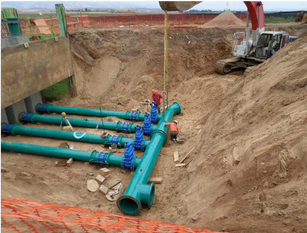
Spiess installing 24-inch manifold onto 16-inch valves.
