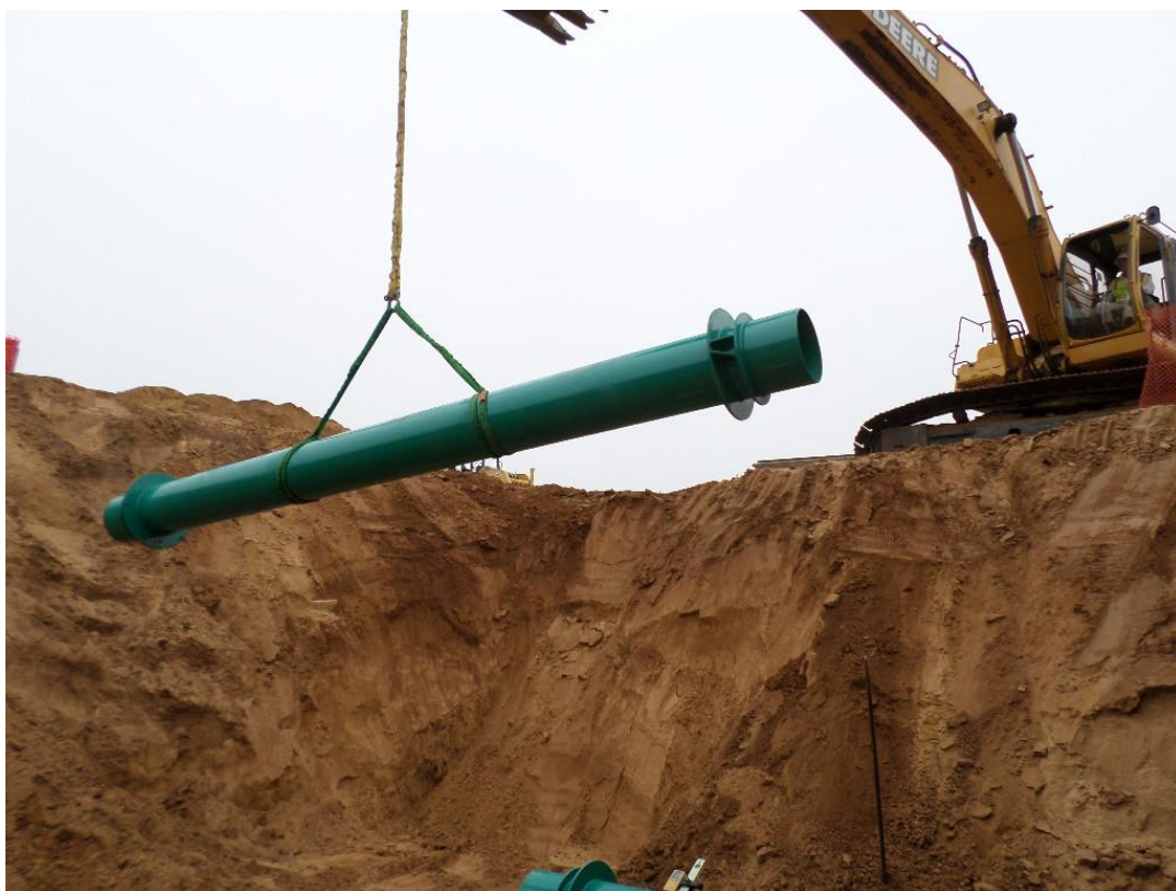
Installing suction piping.
