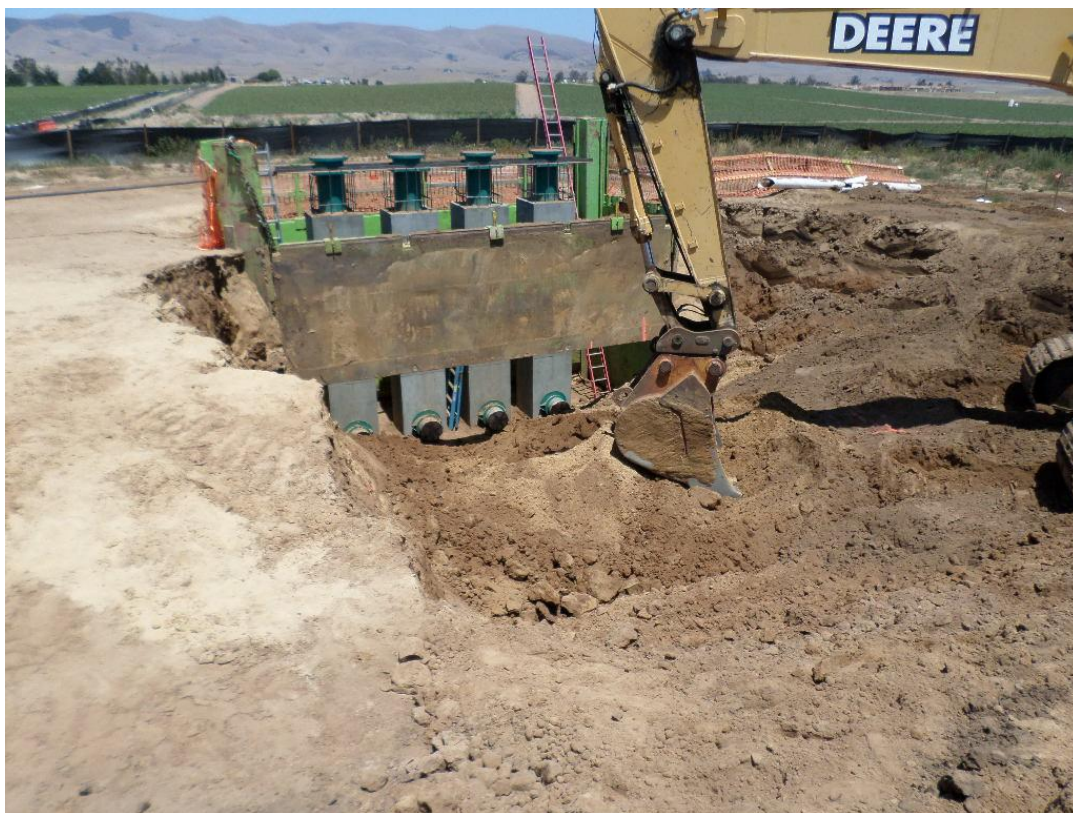
Spiess continuing work on the open cut for installation of the suction pipe and manifold.
