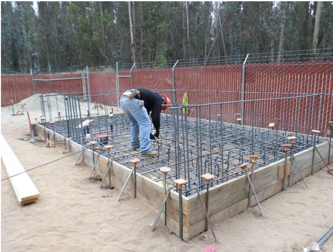
Vista Steel finishing installation of reinforcement at Chemical Building slab.
