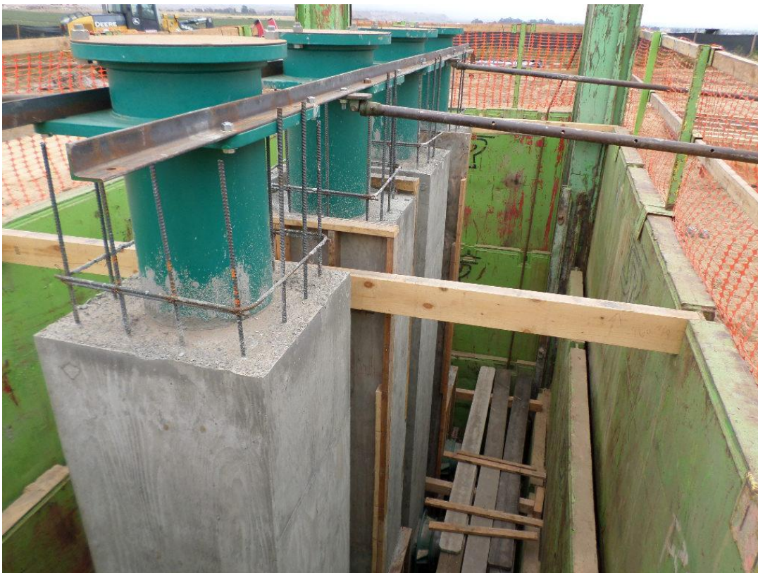
Stripping forms from second pump can encasement pour.
