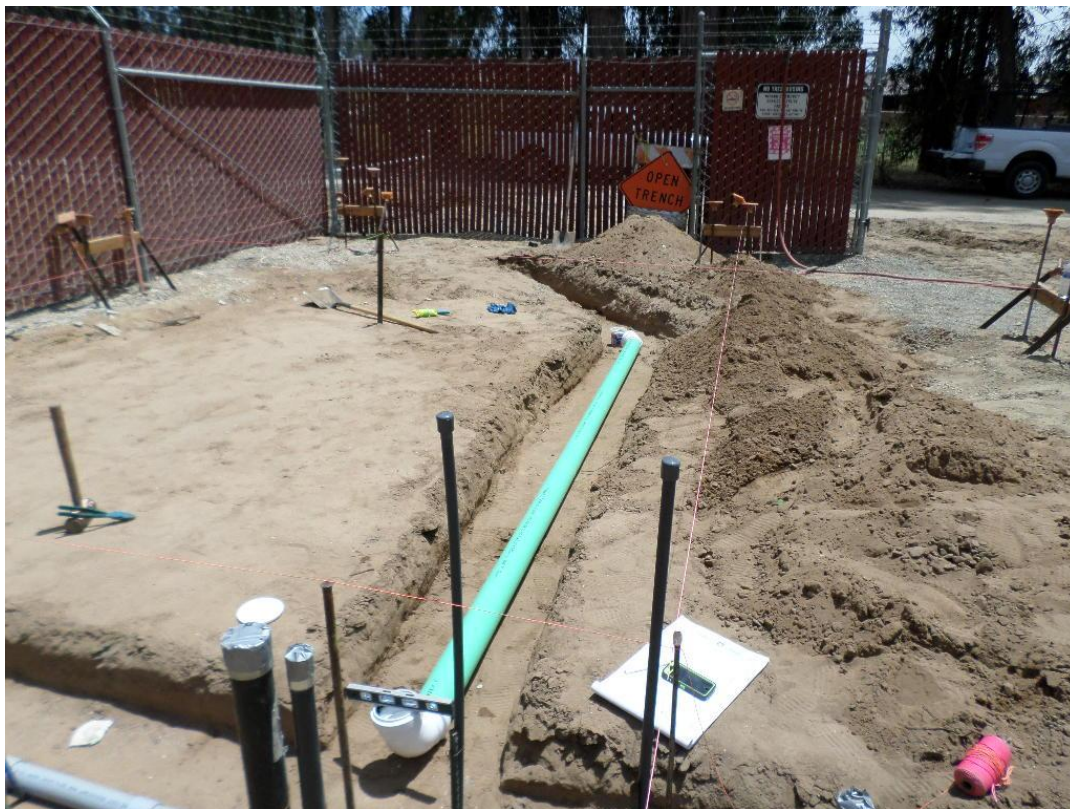
Spieß installing 4-inch PVC drain piping under the Chemical Building slab.
