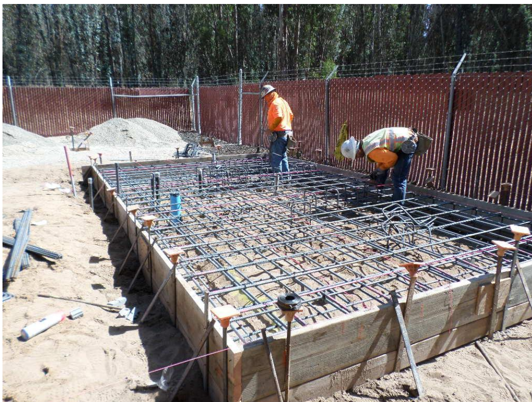
Vista Steel installing reinforcing at Chemical Building.
