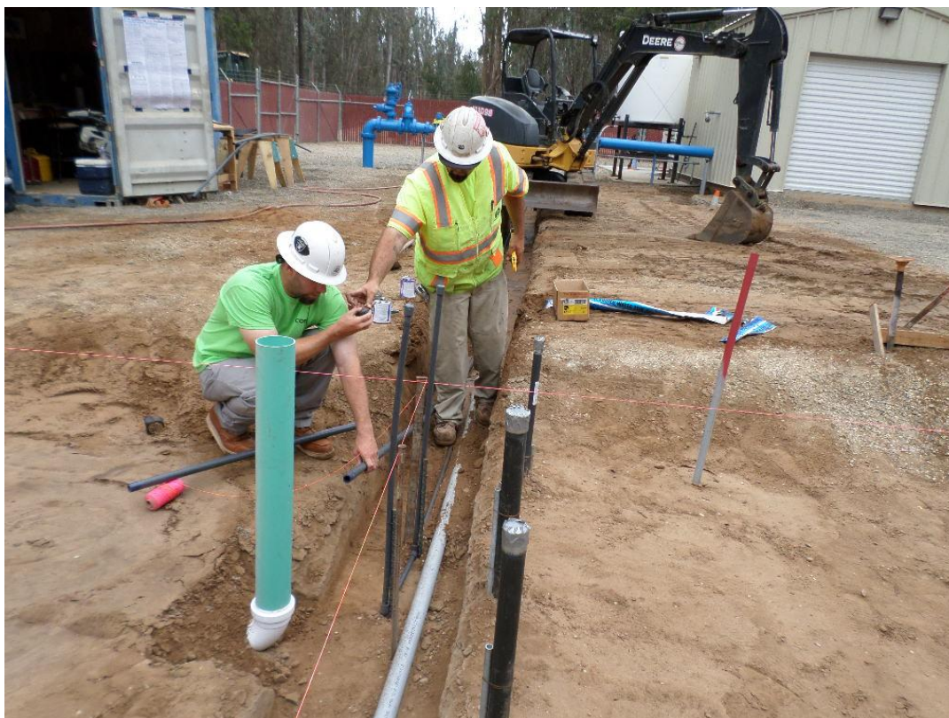
Spieß installing 1/2-inch PVC plant water line and 2-inch PVC chemical tubing line.
