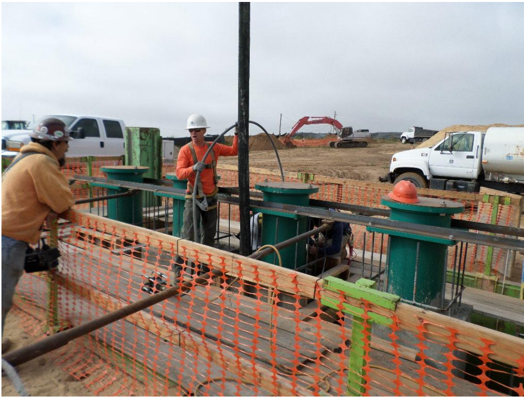
Spiess pouring last two pump can encasements.
