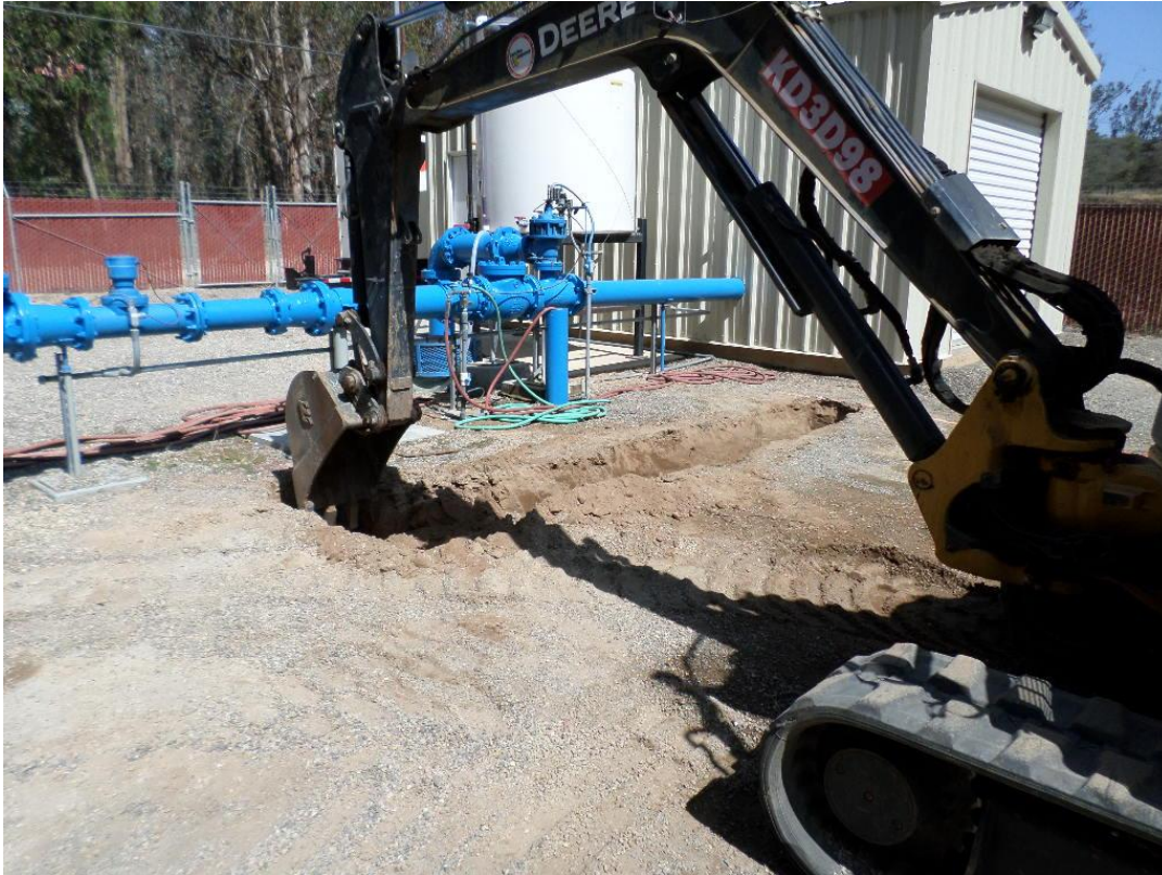
Spiess excavating to install plant water pipe.
