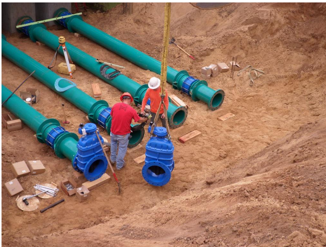
Spiess installing 16-inch valves.
