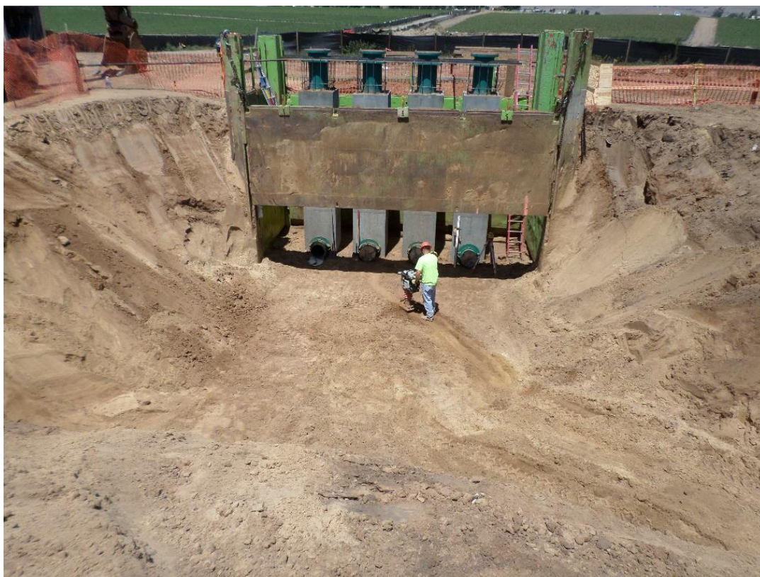
Compacting subgrade under future suction piping.
