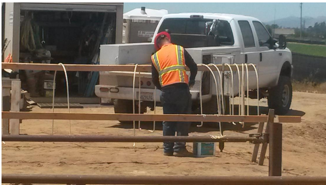
Spiess coating rebar for valve anchors.
