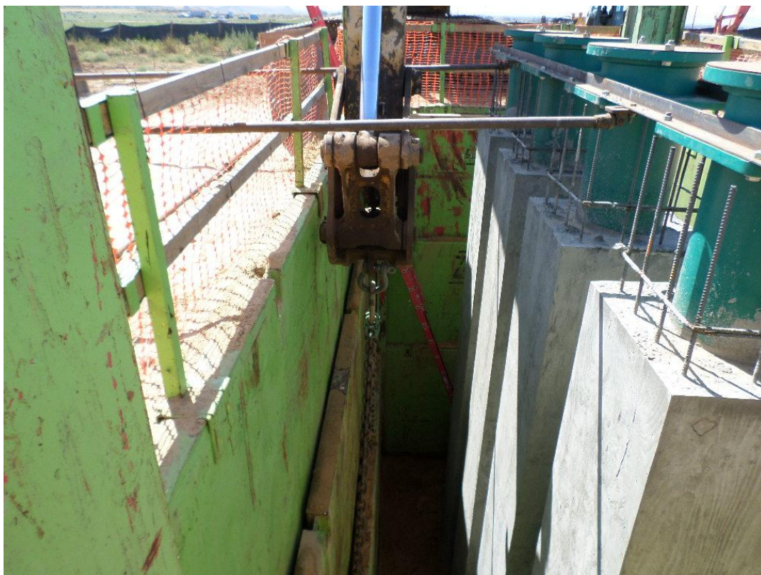
Spiess raising slip shoring from around the pump cans with the excavator.
