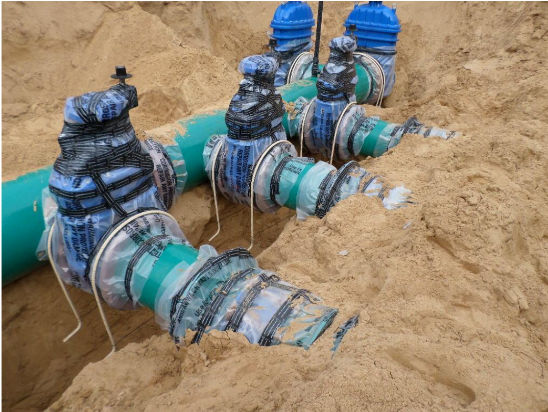
Spiess excavating for concrete blocks and placing epoxy rebar anchors over valves on inlet piping.
