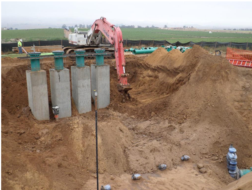
Spiess continuing backfill around the pump cans.
