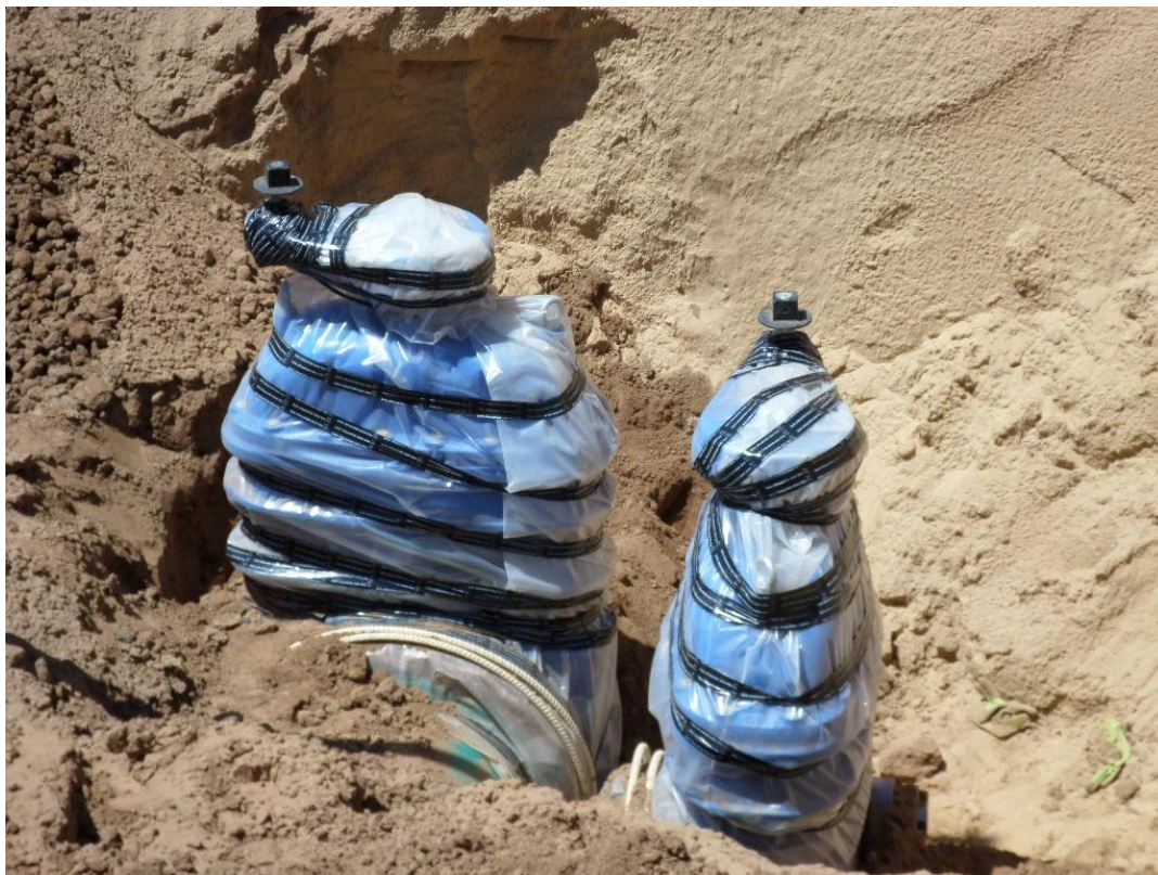
Spiess wrapping valves with plastic before backfilling.
