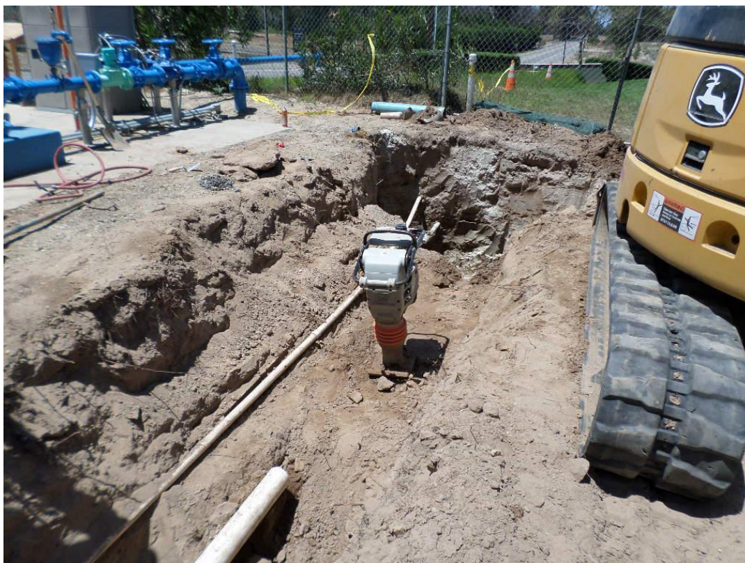
Spiess relocating existing 1-1/2-inch Irrigation line and 4-inch drain line which interfere with the future structures.
