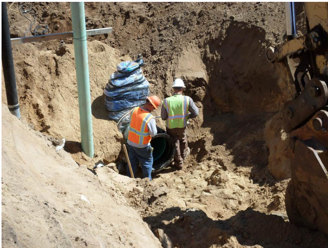
Spiess installing flange adapter on 24-inch DIP.
