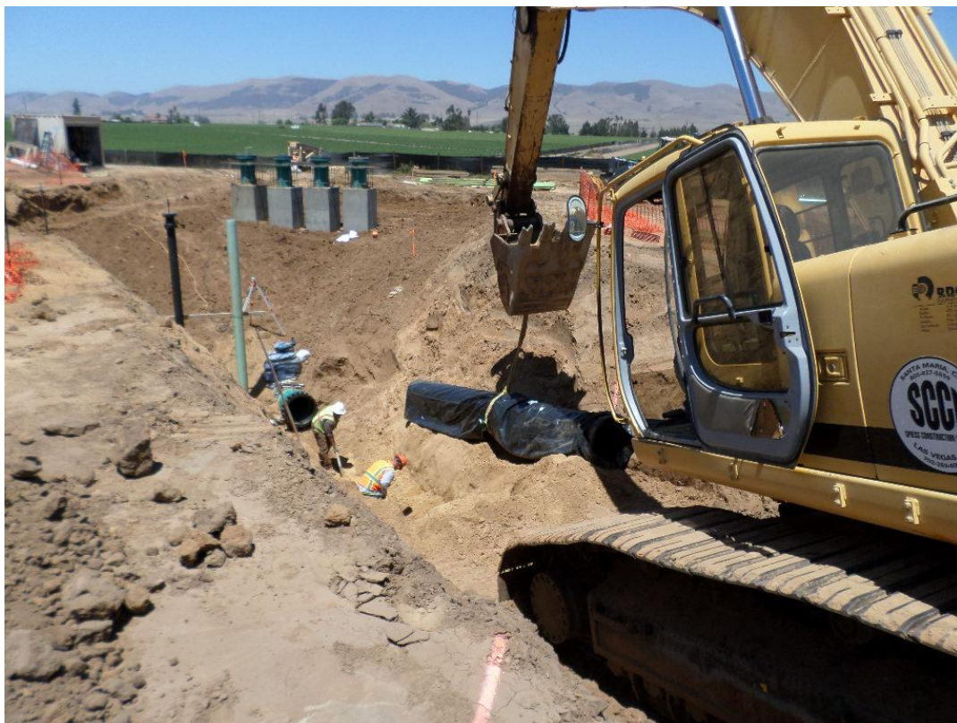
Spiess installing 24-inch DIP from pump station inlet manifold toward the BP #1 connection.
