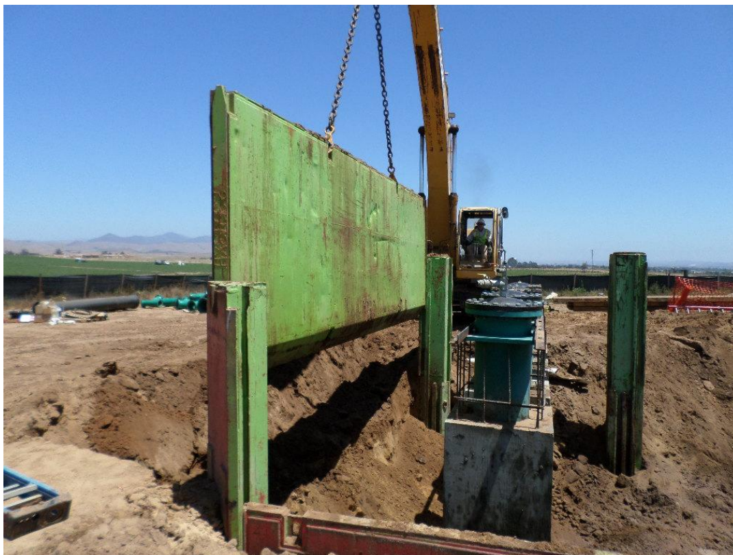
Removing shoring from around the pump cans.
