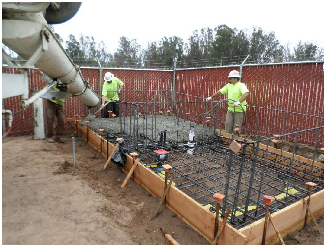
Spiess pouring chemical building slab.
