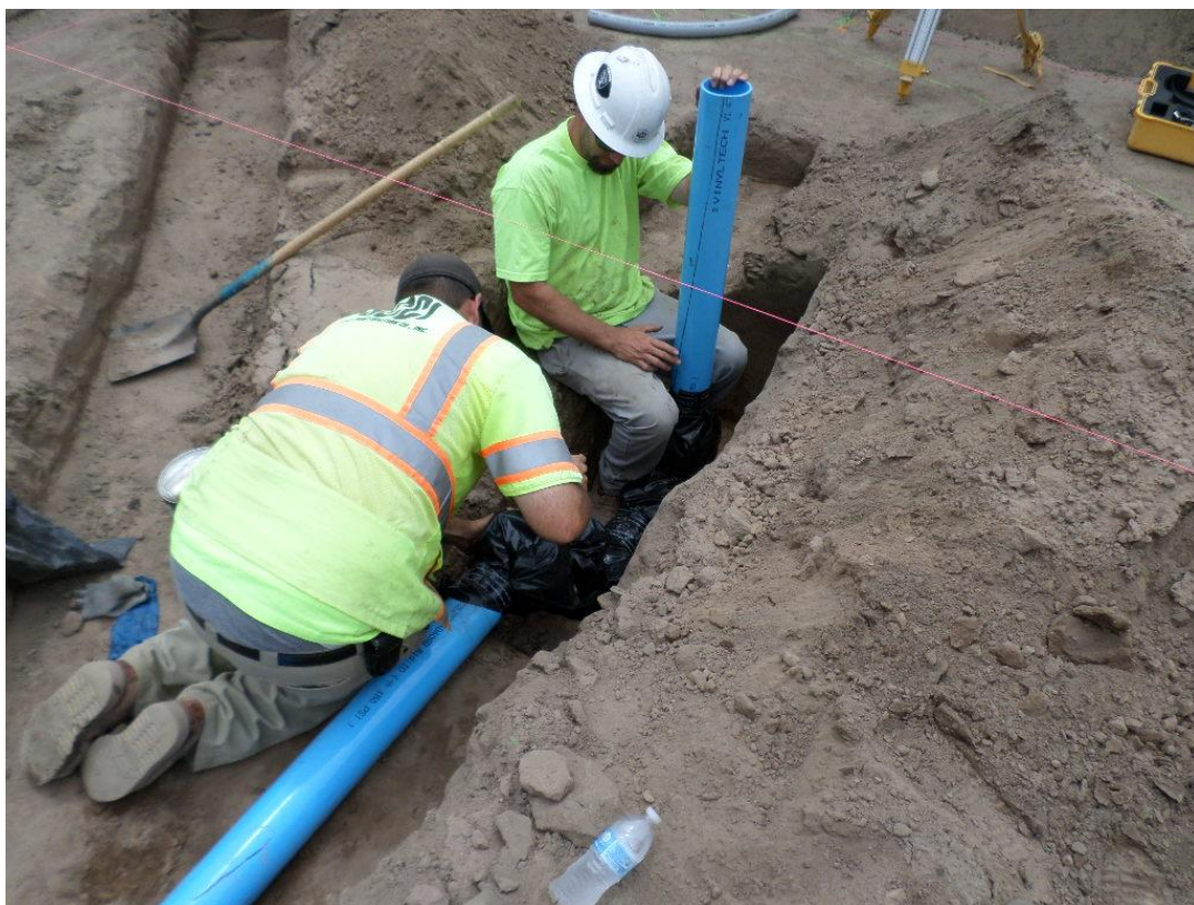
Spiess installing 4-inch drain line.
