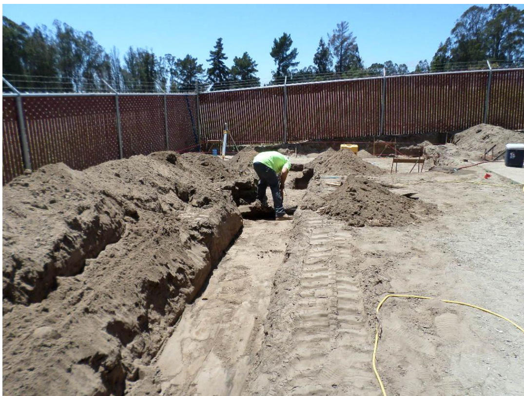
Spiess trenching for site piping.
