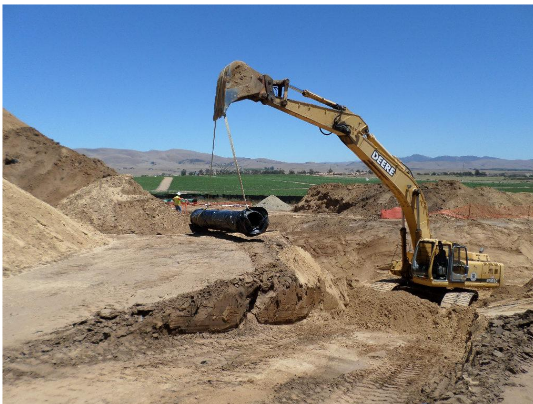
Spiess installing 24-inch DIP.
