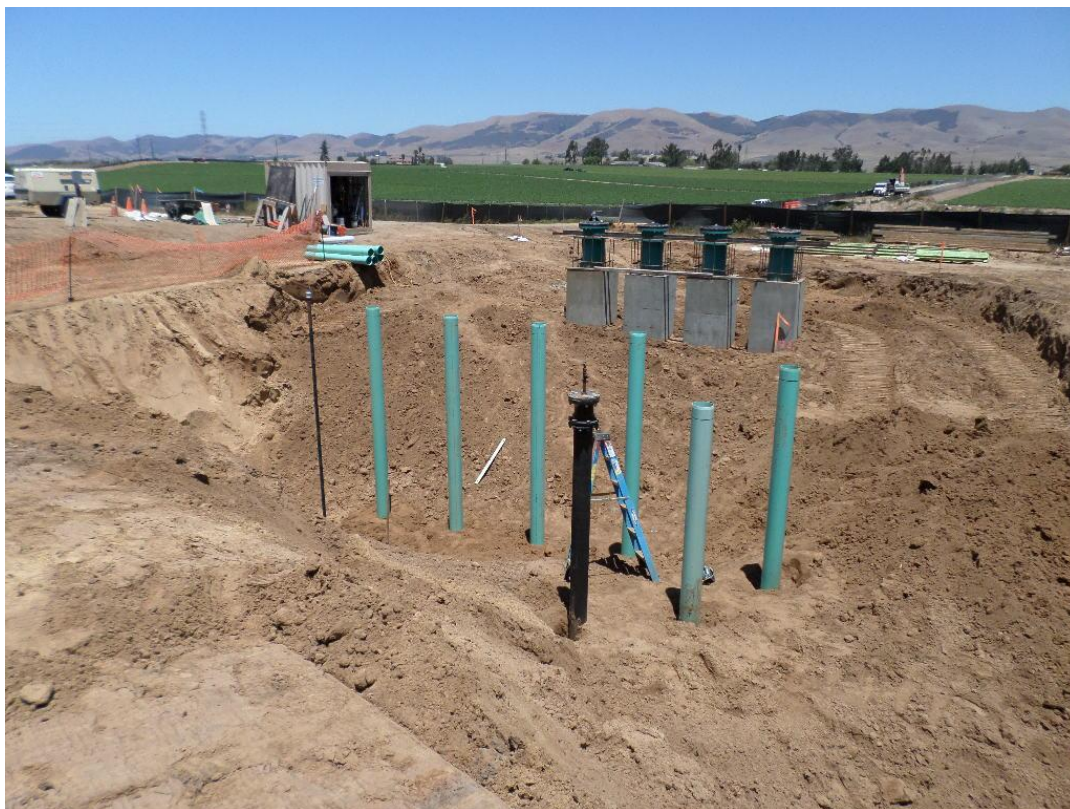
Spiess installing valve can risers on inlet manifold.
