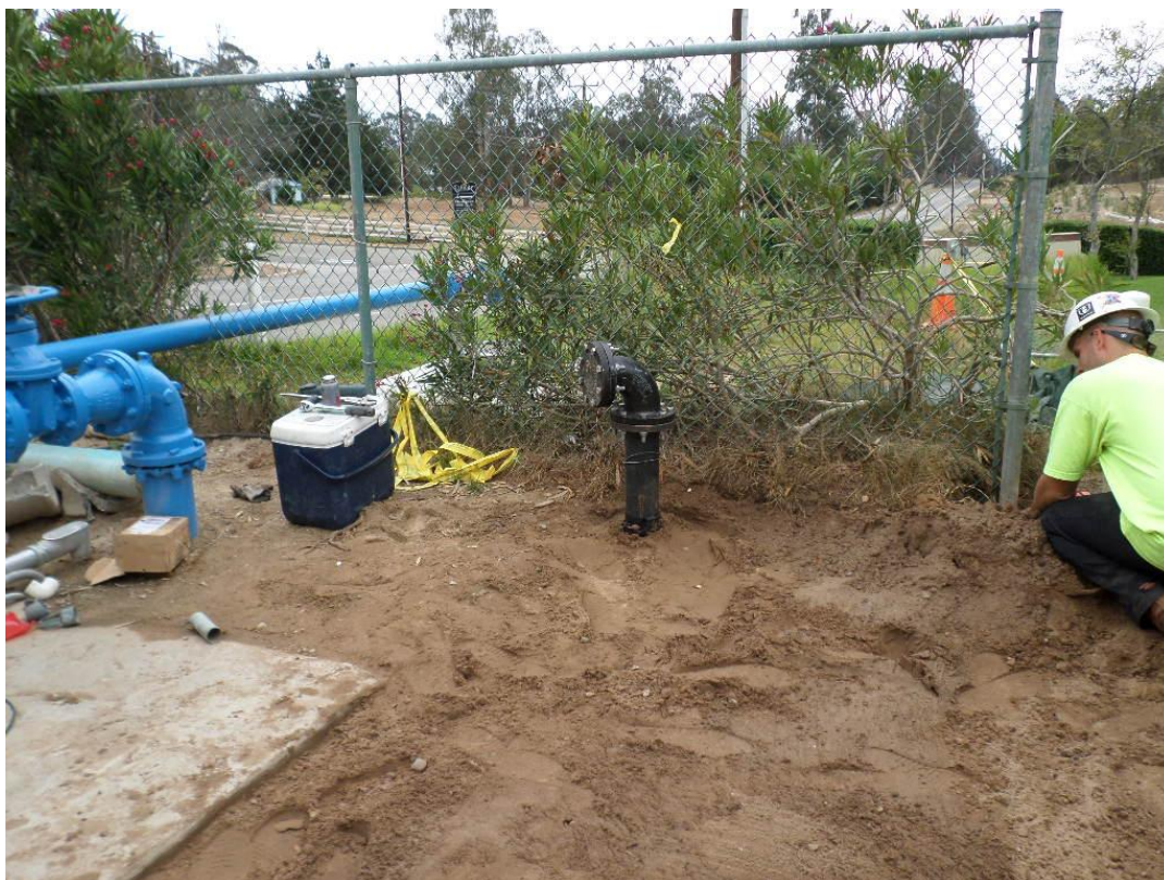
Relocated 4-inch riser.
