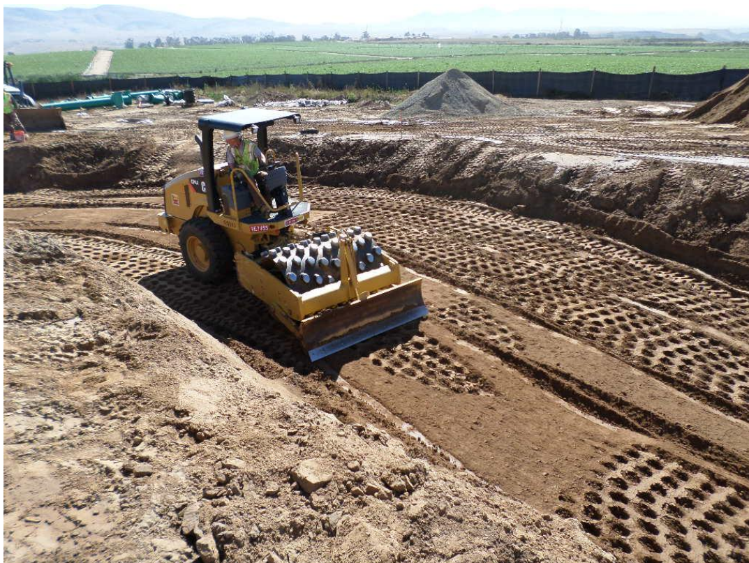
Spiess compacting over 24-inch DIP.
