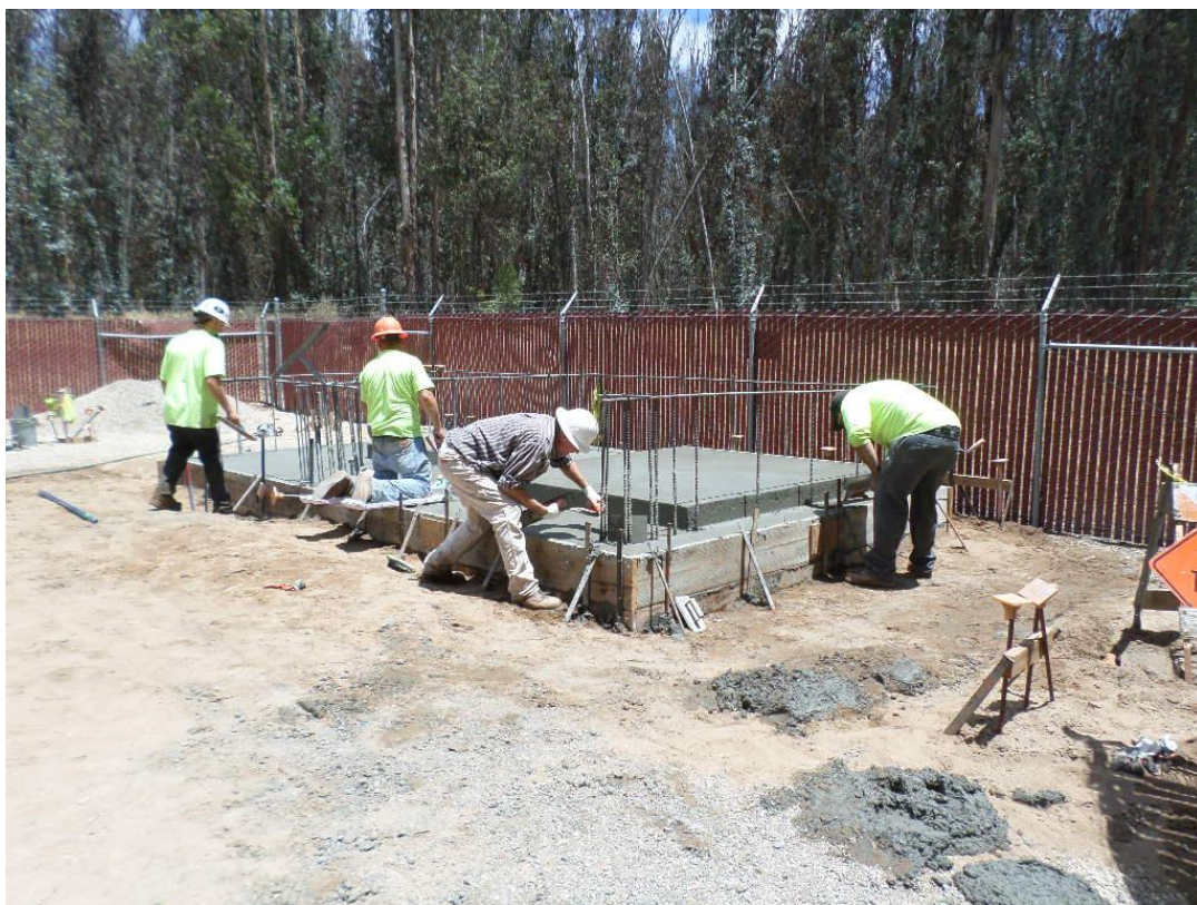
Spiess finishing concrete at chemical building slab.
