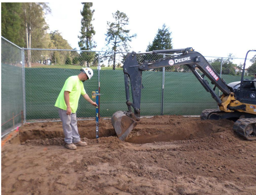
Spiess over excavating for the chemical building slab.
