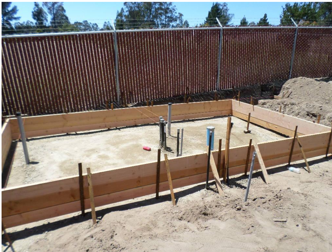
Spiess forming chemical building slab.
