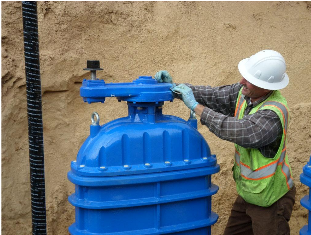
Spiess abrading valve in preparation for coating touch-up before backfill.
