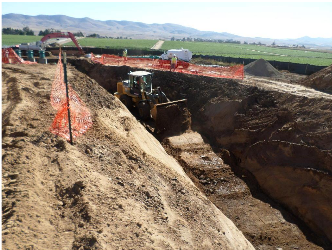
Spiess backfilling over 24-inch DIP.
