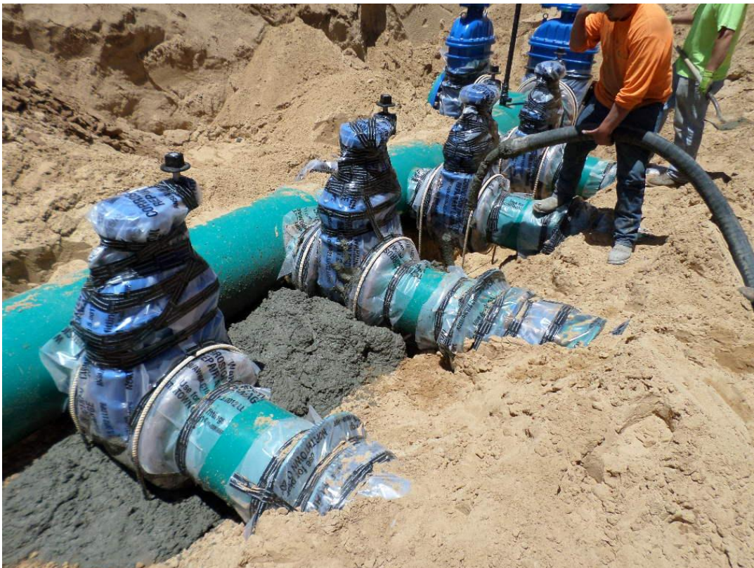
Pouring concrete valve anchors on inlet piping.
