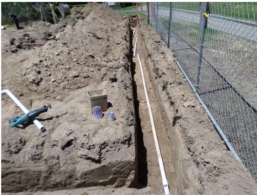
Spiess relocating 1-1/2-inch irrigation line.
