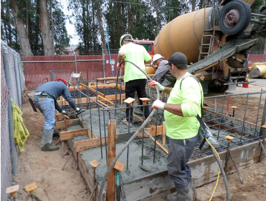
Spiess placing concrete for chemical building slab.
