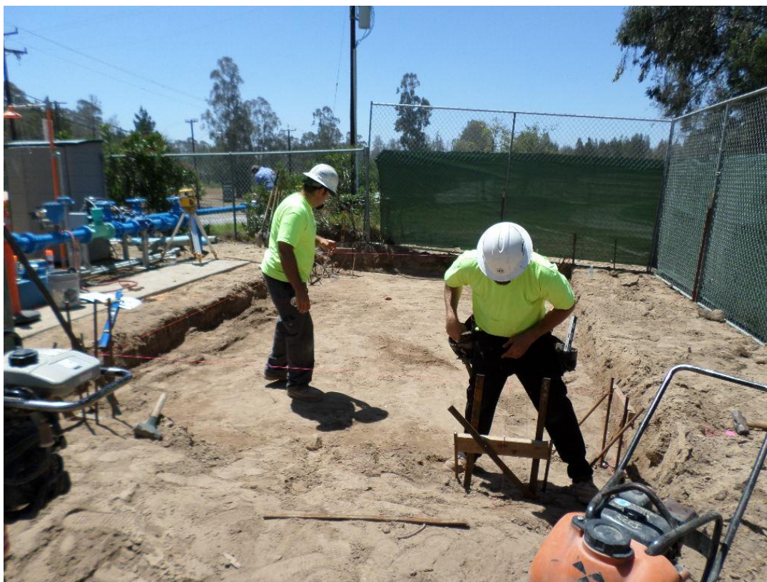
Spiess laying out the chemical building slab.
