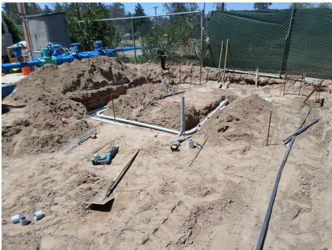
Spiess installing underslab piping.
