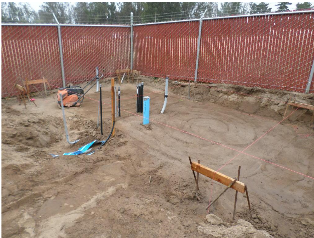
Compacting pipe trenches under future chemical building slab.
