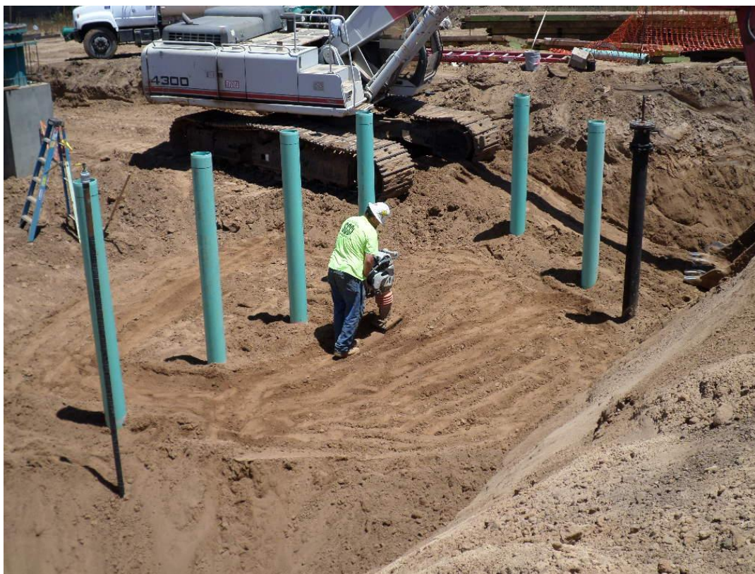
Spiess compacting around the valve can risers.
