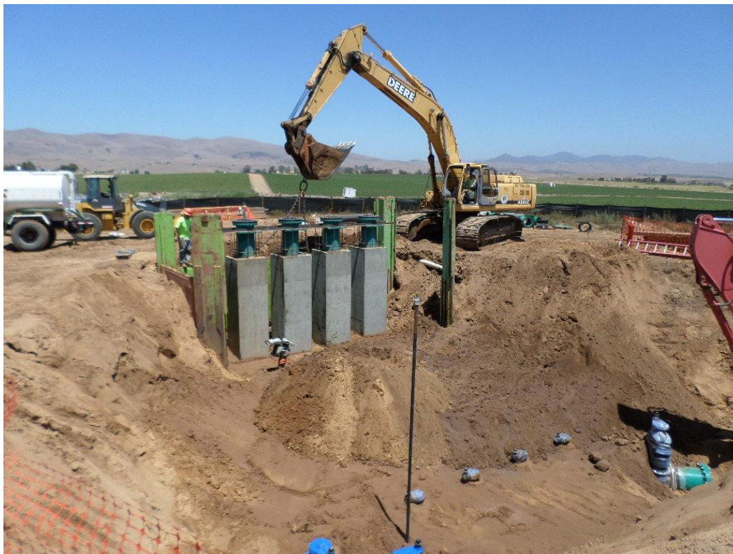
Spiess removing shoring plates at pump cans.
