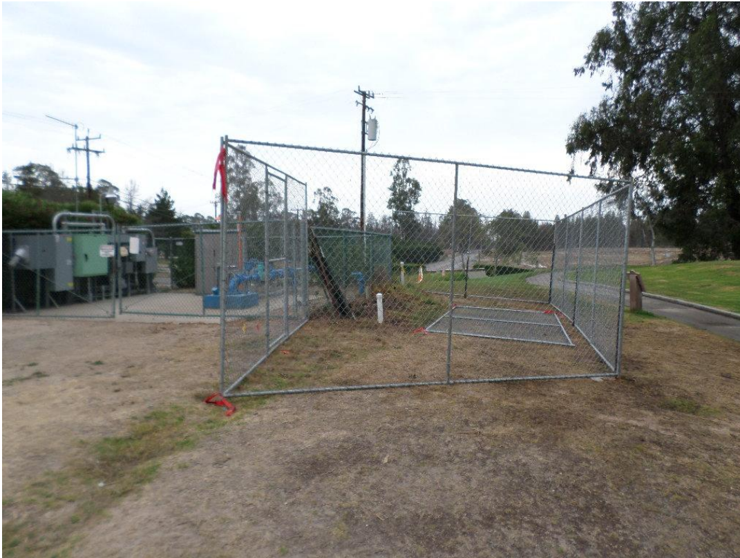
Installing temporary fencing to expand site.
