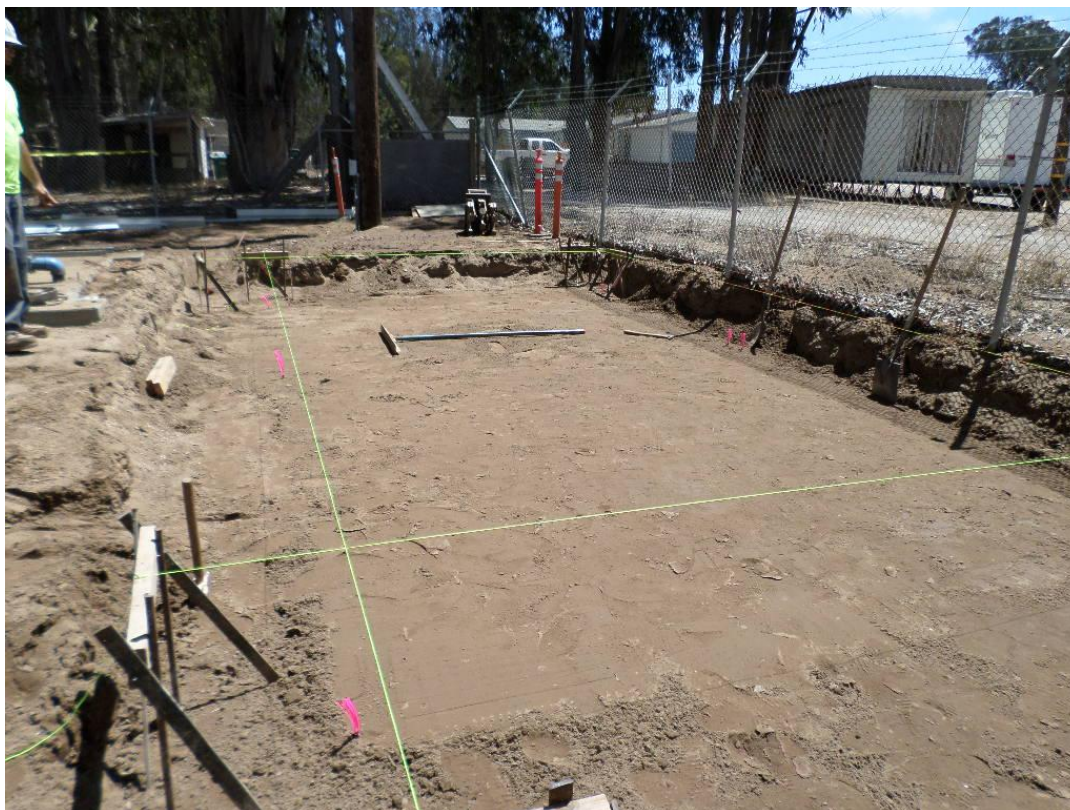
Laying out the chemical building slab foundation.
