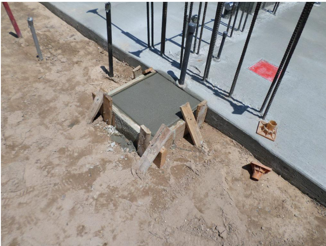
Eyewash station pad installed.
