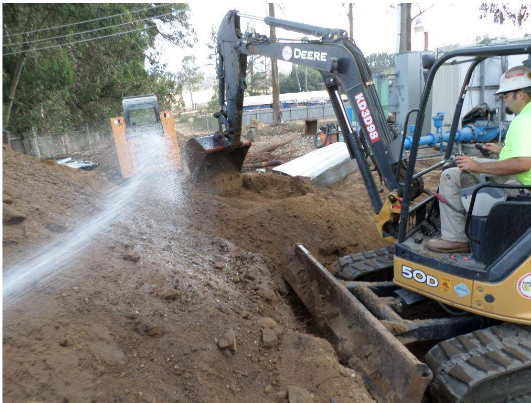
Spieß backfilling and compacting under the future chemical building slab.
