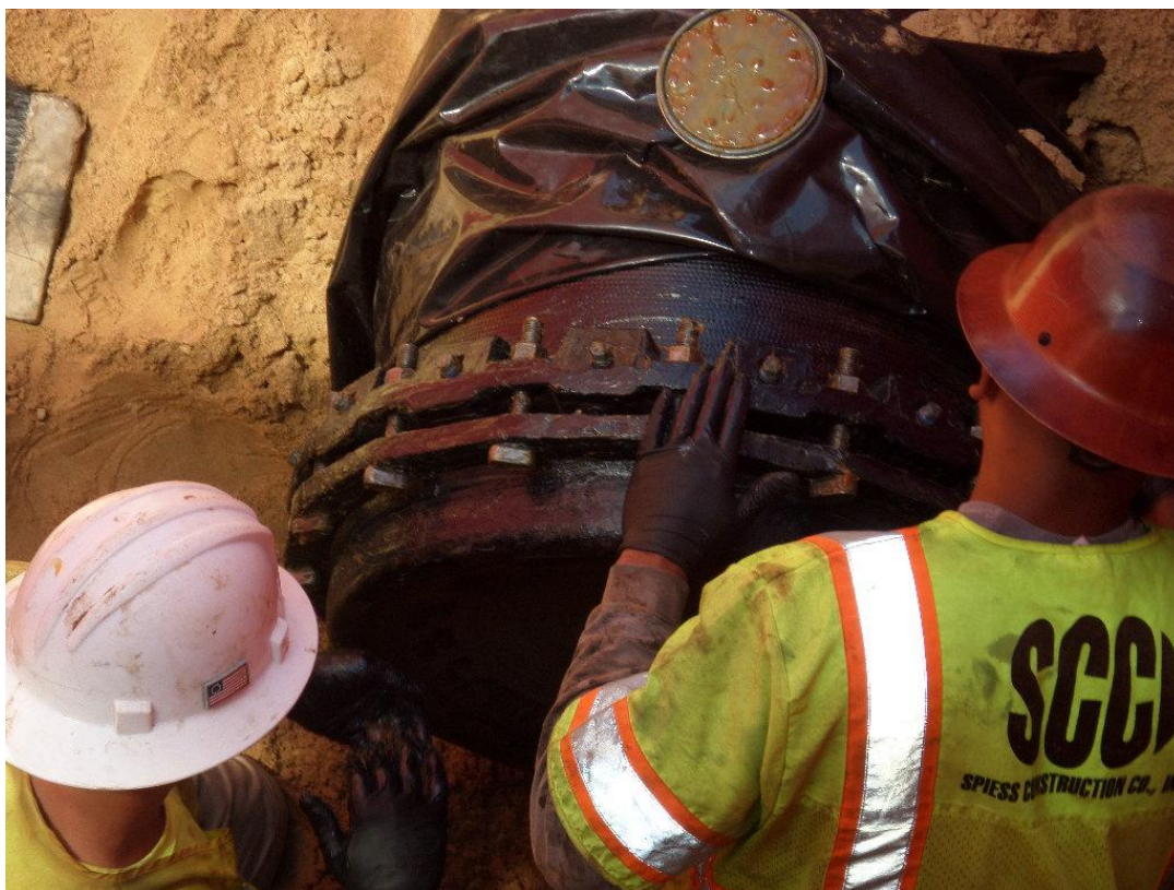
Spiess applying wax tape to bolted connection on the DIP pipe for the future tank outlet.
