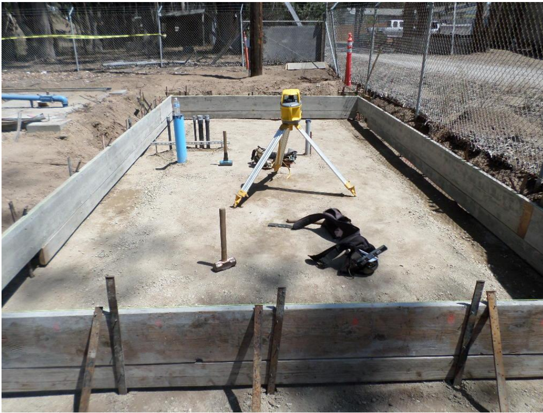
Forming the chemical building slab foundation.
