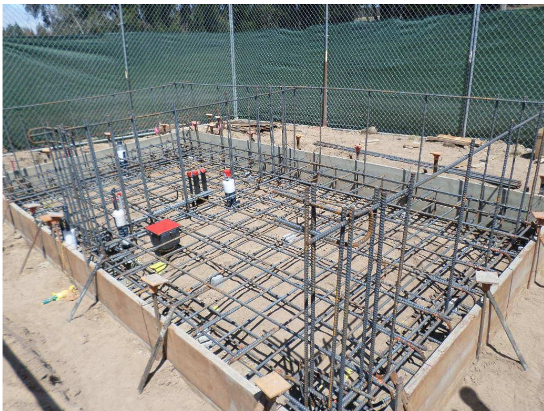
Reinforcing installed for chemical building slab.
