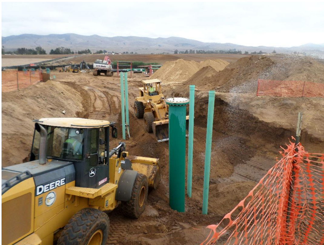
Spiess backfilling around installed valve can risers.
