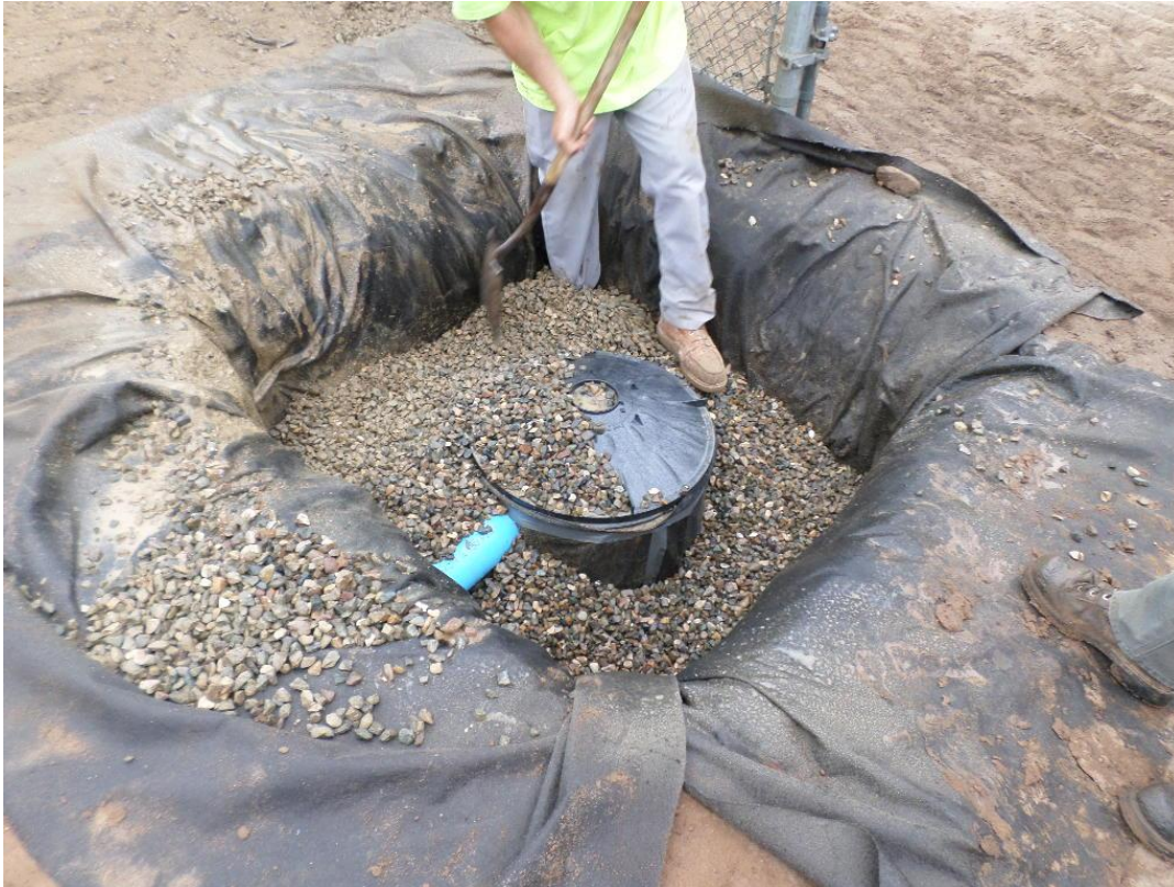
Spiess installing drywell at Via Concha.
