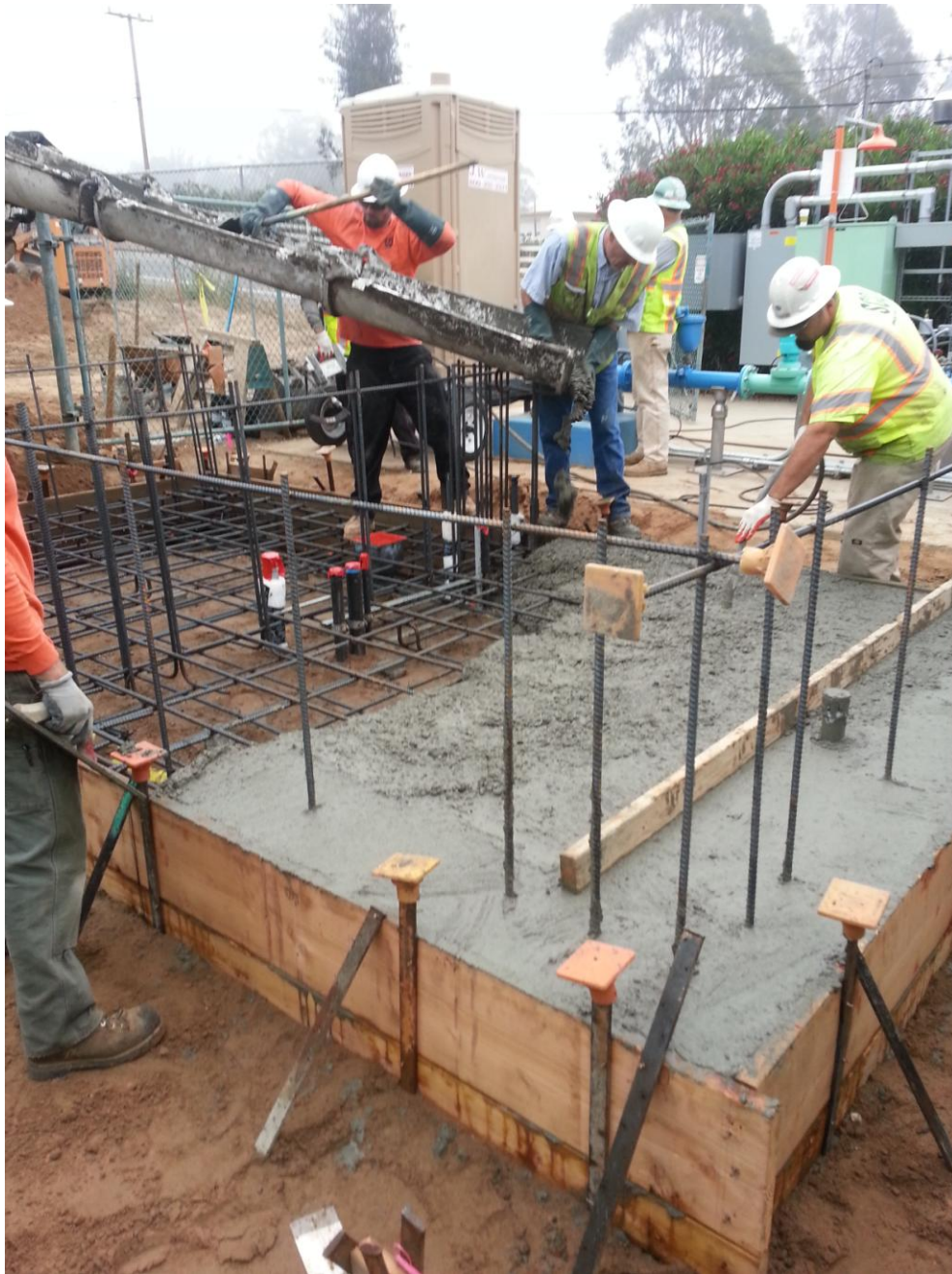
Spiess pouring the chemical building slab.
