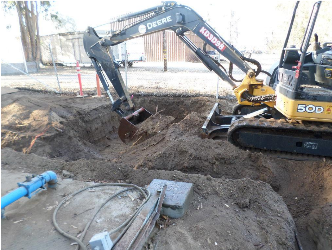
Spiess over excavating native material under the future chemical building slab.
