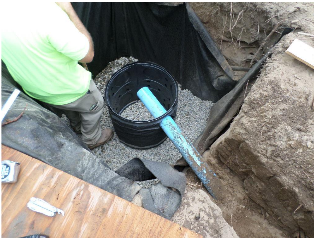
Spiess installing drywell.
