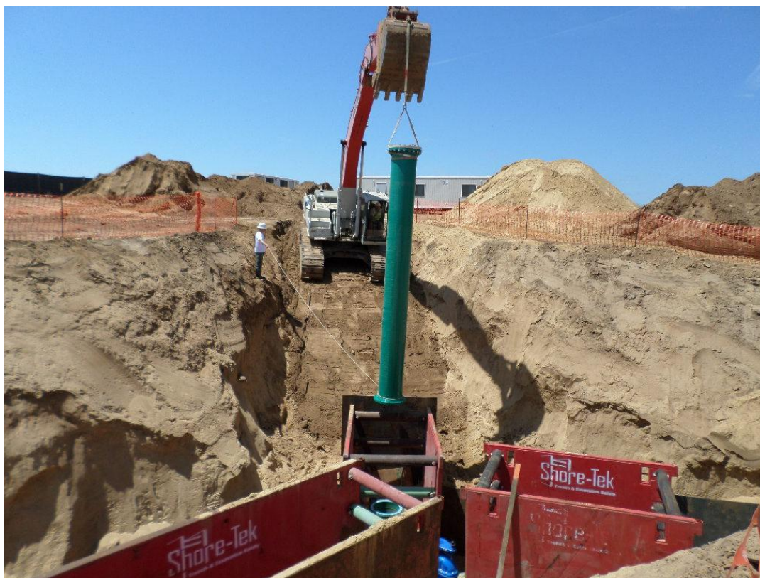
Spiess setting the pig launcher riser.
