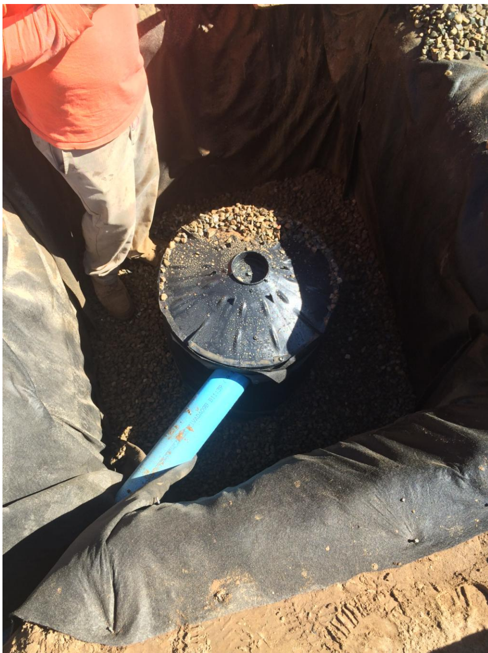
Spiess installing the drywell.
