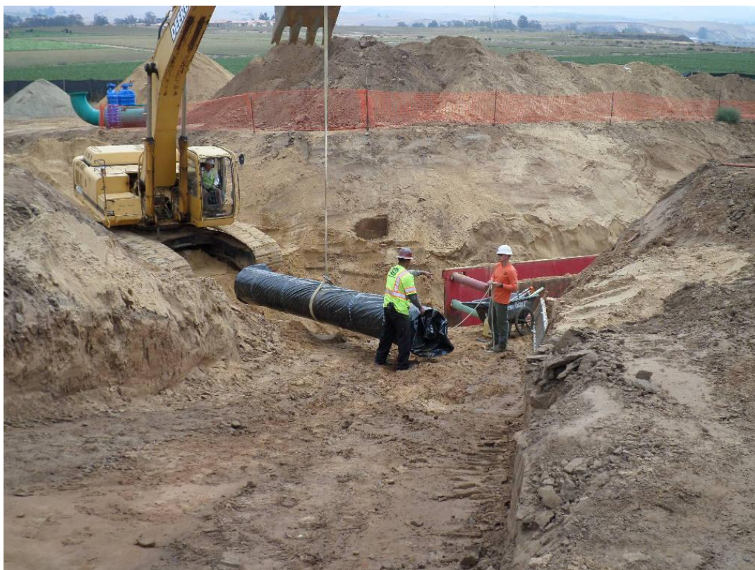
Spiess installing the 24-inch DIP.
