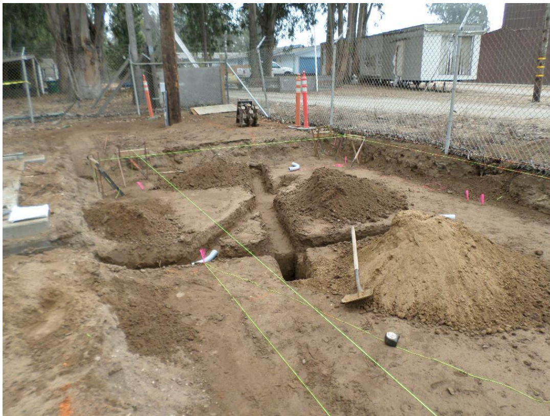
Trenching for underslab piping.
