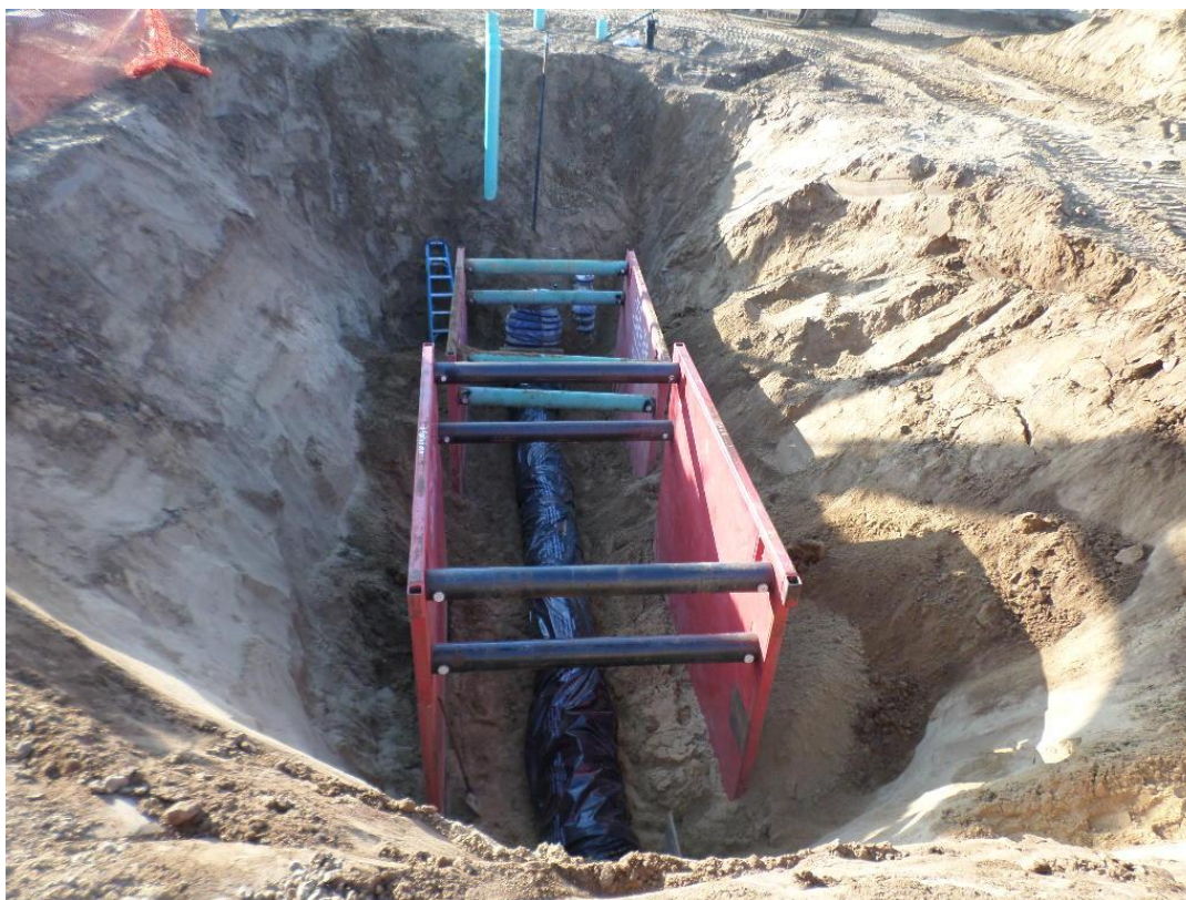
Spiess installing pipe extension to future tank outlet piping.
