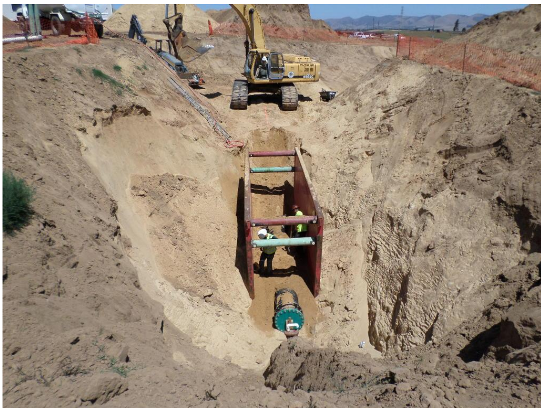
End of 24-inch DIP which will be connected to the HDPE in the future.
