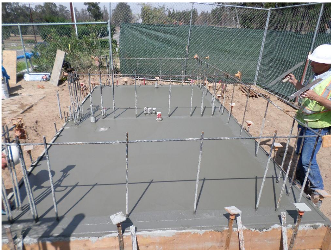
Spiess finishing the chemical building slab.
