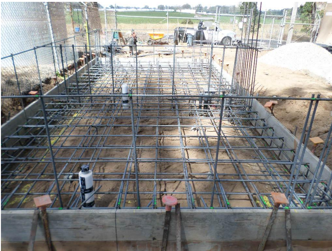
Chemical pad reinforcing installed by Vista Steel.
