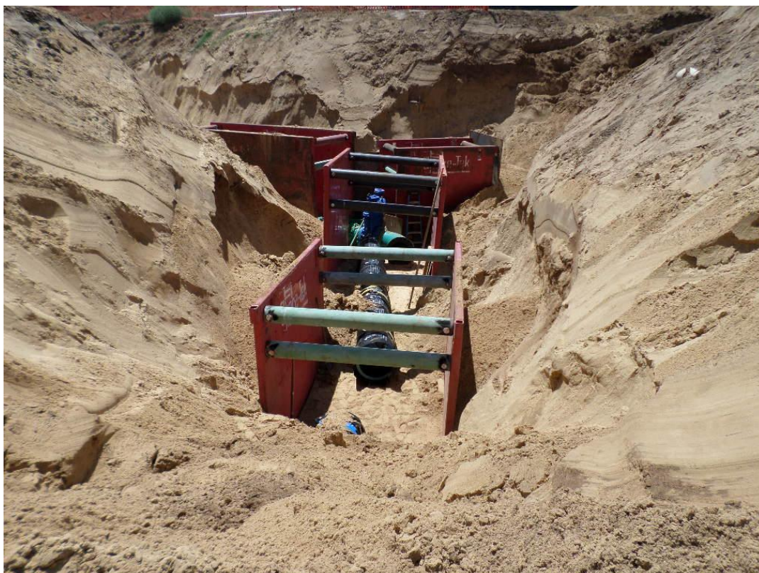
Spiess installing the 24-inch DIP around the pig launcher.
