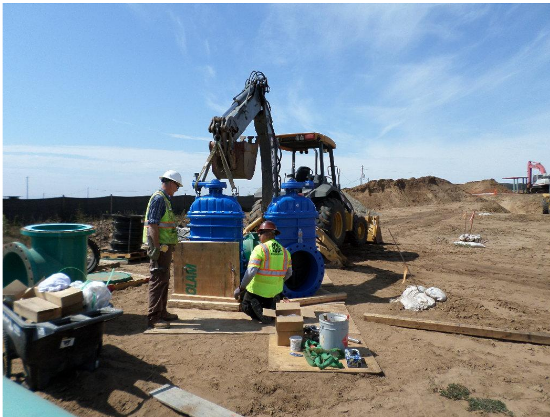
Spiess bolting up 24-inch valves.
