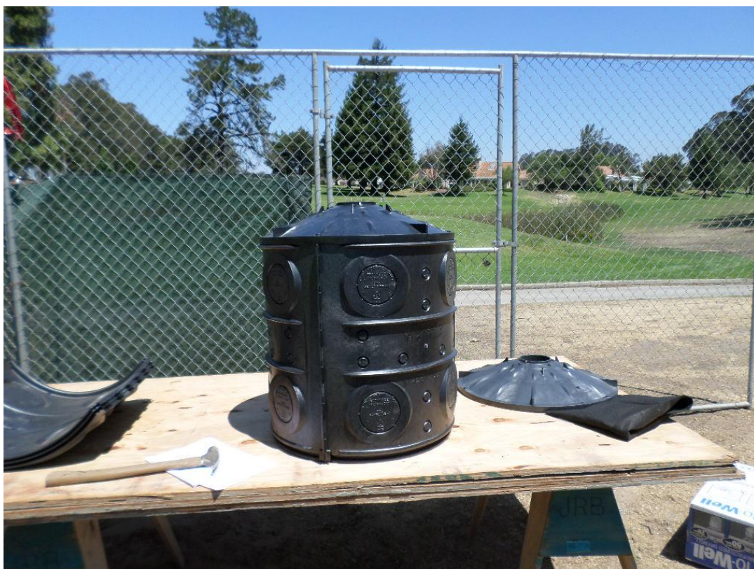
Assembling the drywell.
