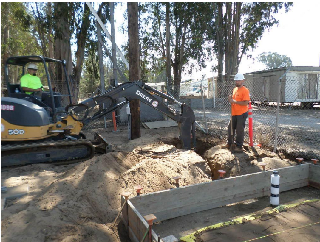
Spiess excavating for drywell.
