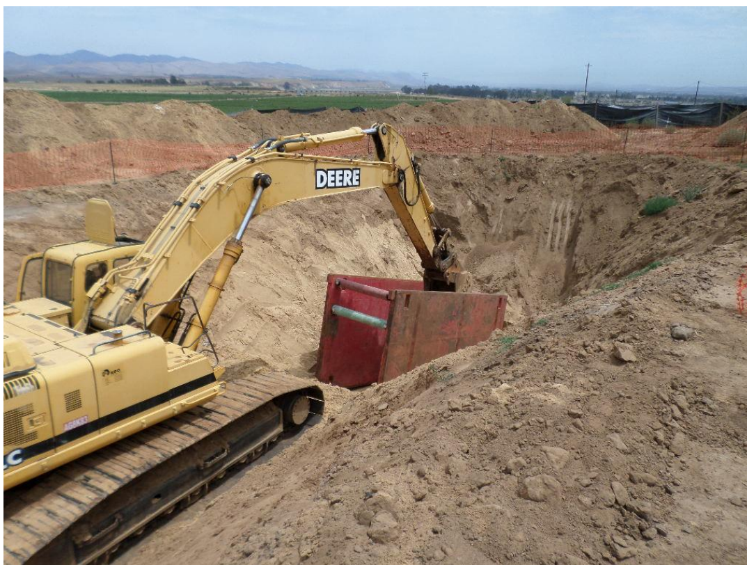
Spiess setting shoring for installing 24-inch DIP for future connection to the HDPE pipe installed as part of Bid Package #1.
