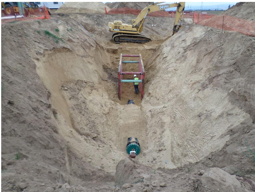
Spiess continuing installation of 24-inch DIP from the future connection point at the HDPE pipe to the pump station inlet manifold.
