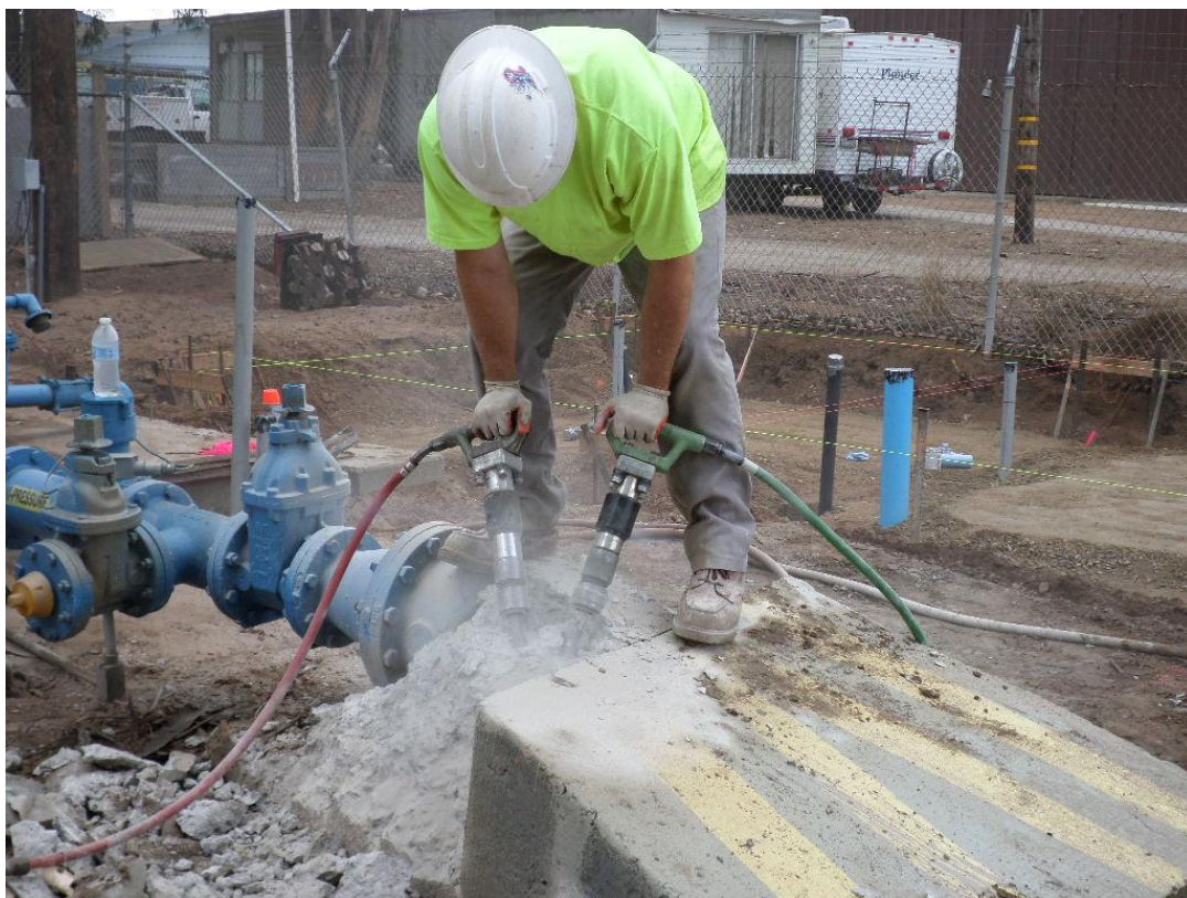
Spiess performing demolition of existing thrust block for installation of pipe riser.
