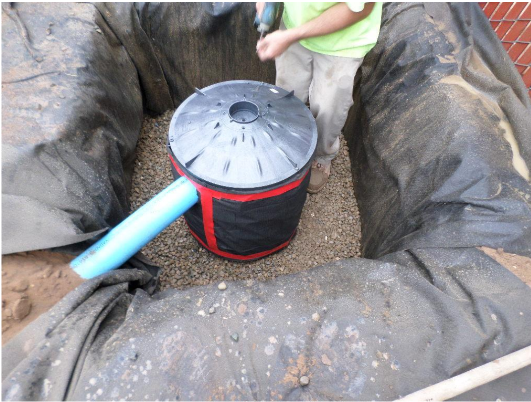
Spiess installing the drywell at Sundale.
