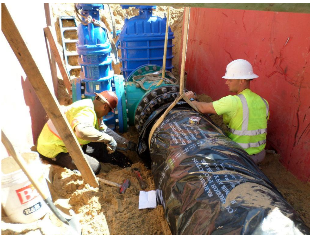
Spiess connection the 24-inch DIP to the "tee".
