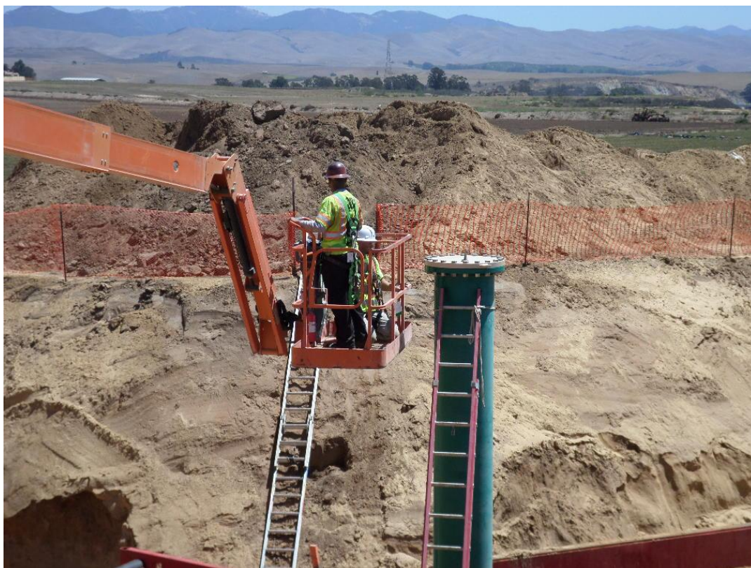
Spiess tightening bolts at the top of the pig launcher riser during pressure testing.
