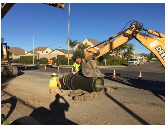
D-KAL bolting together a 45 degree elbow and pup for the storm drain crossing.
