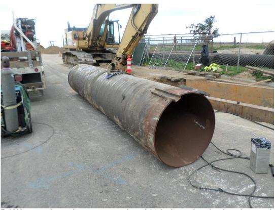
D-KAL preparing to lower next section of 36-inch steel casing into the trench for pushing under the 72-inch storm drain crossing.
