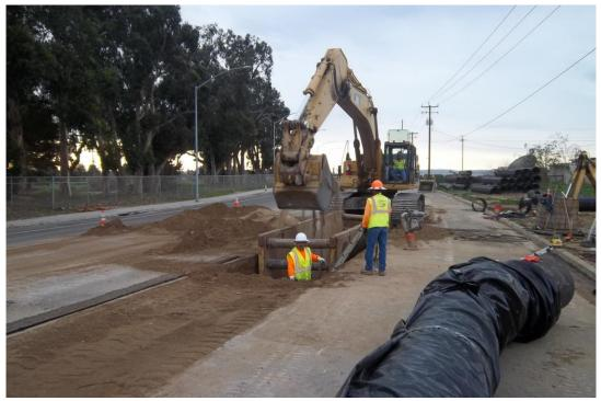
Trench excavation at 12-inch storm drain crossing.
