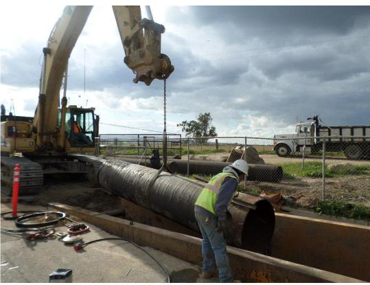
D-KAL lowering next section of 36-inch steel casing into the trench.
