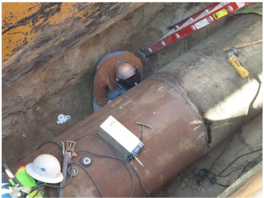
D-KAL welding 36-inch steel casing section to casing end at 72-inch storm drain crossing.
