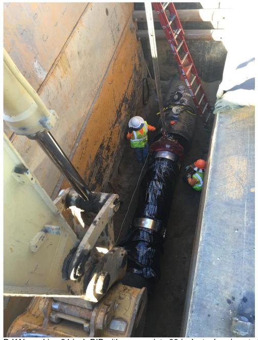
D-KAL pushing 24-inch DIP with spacers into 36-inch steel casing at storm drain crossings.
