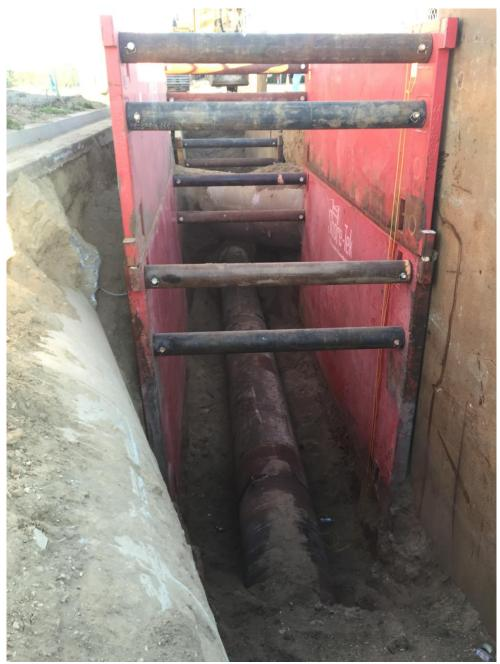
Steel casing installed under the 48-inch storm drain.
