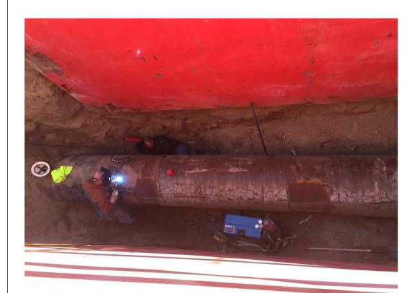
Welding casing section in trench.
