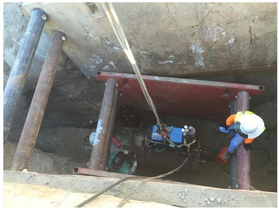
D-KAL welding last section of 36-inch steel casing.
