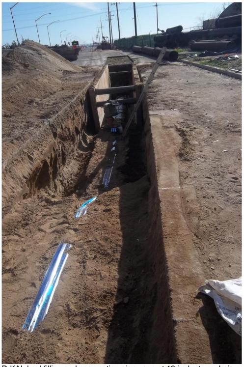
D-KAL backfilling and compacting pipe zone at 12-inch storm drain crossing.
