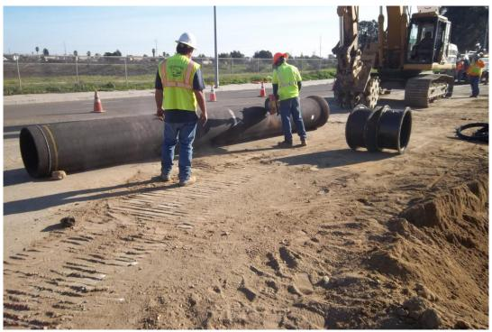
D-KAL cutting section of 24-inch DIP to connect the north end of the storm drain crossing to the pipe already installed.
