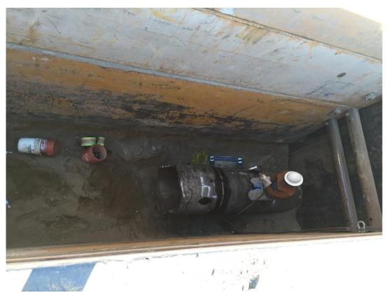
D-KAL cutting off the end of the 36-inch steel casing where it was damaged by the excavator during pushing underneath the 72-inch storm drain crossing.
