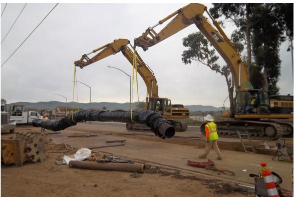
D-KAL installing 24-inch DIP over 12-inch storm drain.
