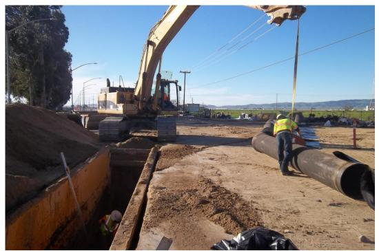
D-KAL continuing installation of 24-inch DIP south past the 48-inch and 72-inch storm drain crossings.
