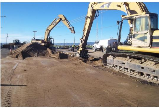
D-KAL compacting trench over 24-inch DIP.
