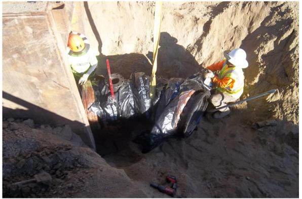
D-KAL installing 45 degree bend off 24-inch DIP to connect to the Flow Metering Station.
