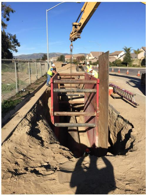
Installing casing section inside trench shields.
