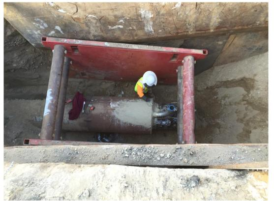
Installing bulkheads at the end of the casing pipe for filling the casing with sand.
