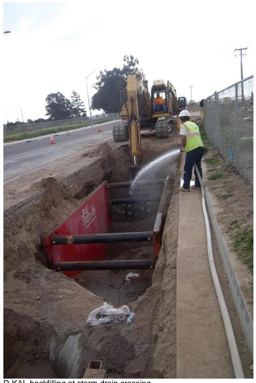
D-KAL backfilling at storm drain crossing.
