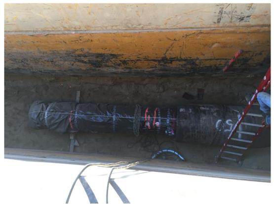
24-inch DIP pushed through 36-inch steel casing.
