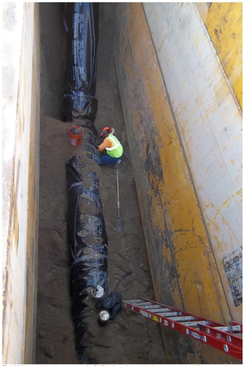
D-KAL continuing 24-inch DIP pipe installation at ends of storm drain crossings.
