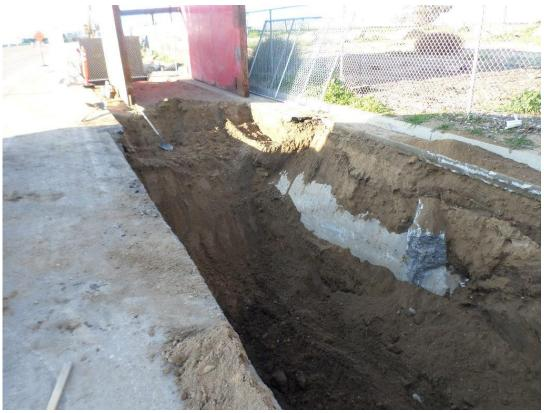
D-KAL excavation the open trench between the 48-inch and 72-inch storm drain crossings.
