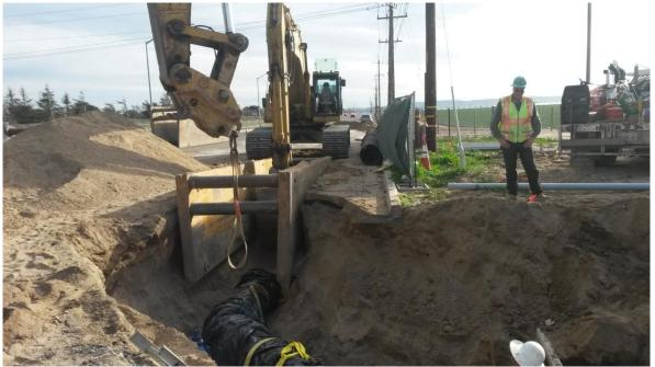
Fugro on site for compaction testing during connections to the Flow Metering Station.
