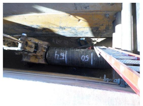
D-KAL using excavator to push the 36-inch steel casing underneath the 72-inch storm drain crossing.
