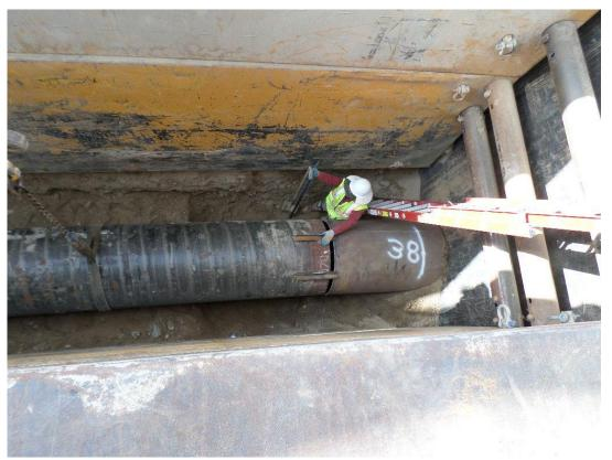
D-KAL lining up the next section of 36-inch steel casing for welding to the portion already pushed underneath the 72-inch storm drain crossing.
