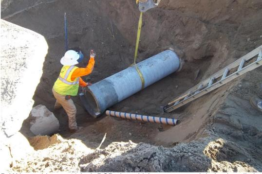
D-KAL repairing an 18-inch RCP pipe which was removed during installation of the 36-inch casing.
