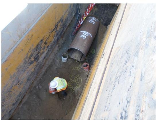
D-KAL removing spoils from inside casing end as it is pushed by the excavator under the 72-inch storm drain crossing.
