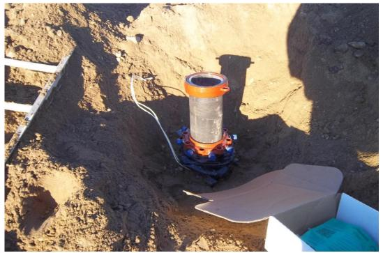
D-KAL installing collar and megalugs at the top of the blow-off at the storm drain crossings.
