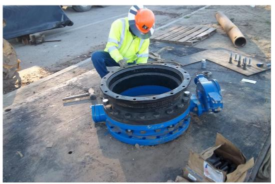
D-KAL bolting MJ adapters to both sides of a 24-inch butterfly valve.
