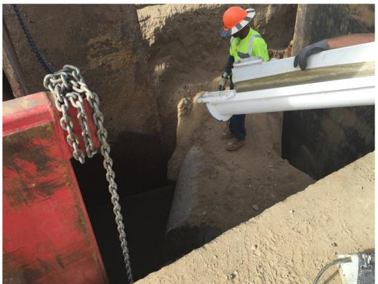
D-KAL pouring a 2 sack slurry around the 48-inch storm drain.
