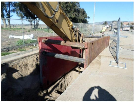
Excavating and installing trench shields between the 48-inch and 72-inch storm drain crossings.
