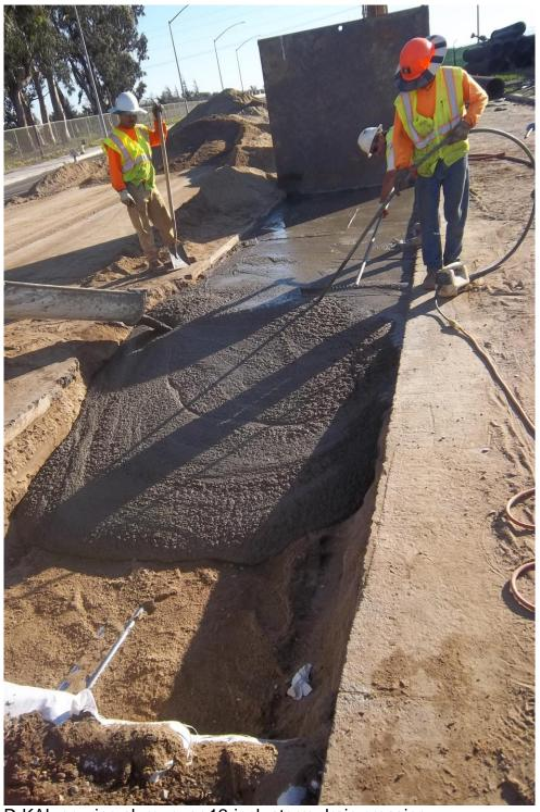
D-KAL pouring slurry over 12-inch storm drain crossing.
