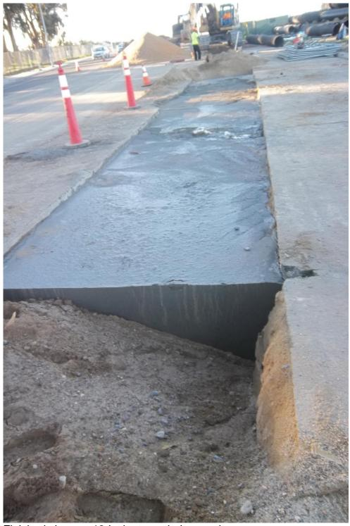
Finished slurry at 12-inch storm drain crossing.
