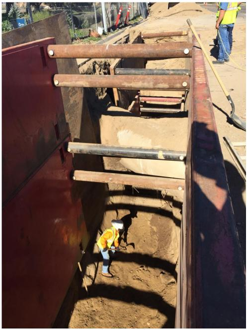
D-KAL leveling the bottom of the trench for installing the casing between the 48-inch and 72-inch storm drain crossings.
