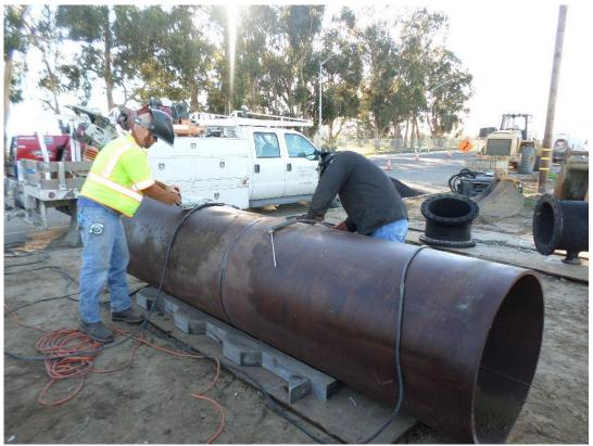
D-KAL welding a section of the 36-inch casing for installing underneath the 48-inch and 72-inch storm drain crossings.
