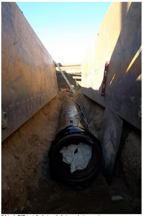
24-inch DIP installed at end of storm drain crossing.
