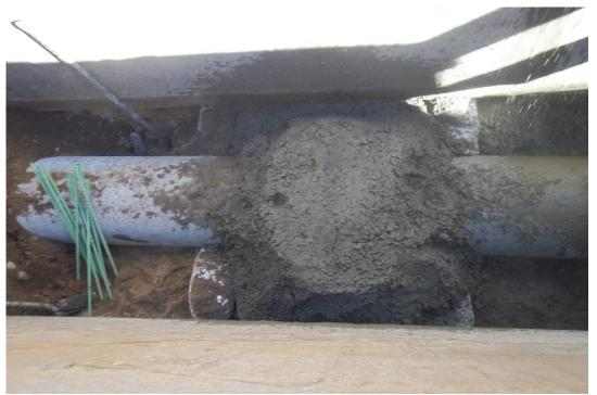
Concrete collar poured at both connections of the new and existing storm drain.
