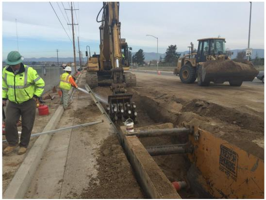
D-KAL continuing compaction over 24-inch DIP.
