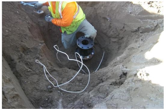
D-KAL installing 4-inch reducer on the 24 X 6-inch tee for the CAV, Station 5+33.
