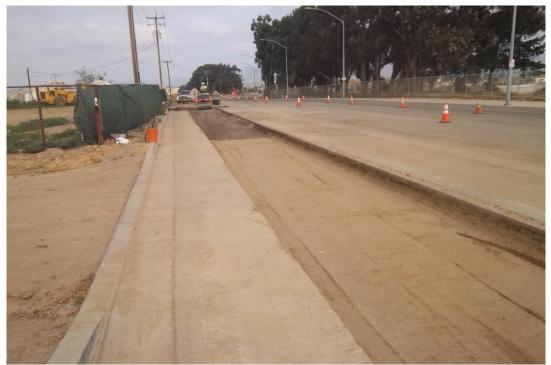
D-KAL prepping trench for paving by removing top backfill, compacting sub-base and spreading and compacting AB.
