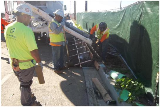
D-KAL pouring concrete for curb and gutter repair along Blosser Road.
