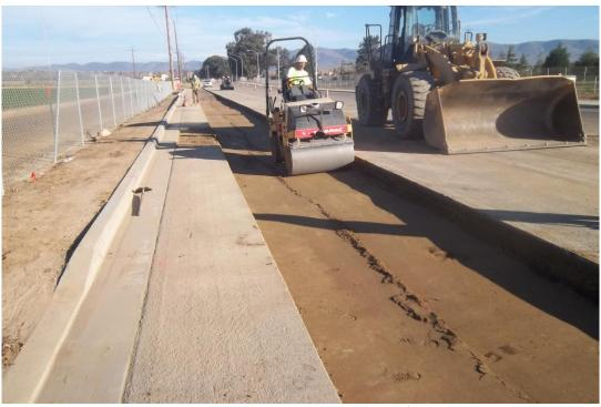
D-KAL compacting base over trench in preparation for aggregate base.
