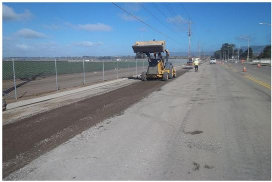
D-KAL spreading aggregate base over trench in preparation for compaction and paving.
