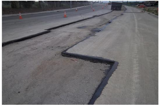
Trench ready for paving with aggregate base compacted and edges oiled.
