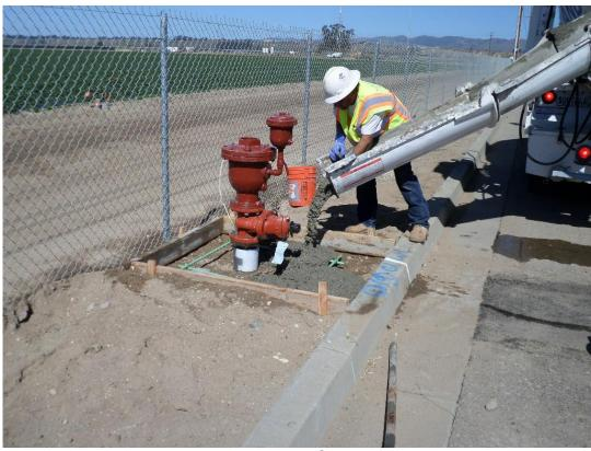
D-KAL pouring the concrete pads at the CAV's.
