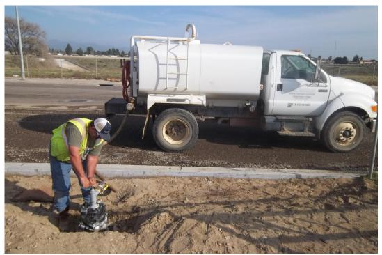
D-KAL using water truck to contain water from flushing the blow-offs and CAV's.
