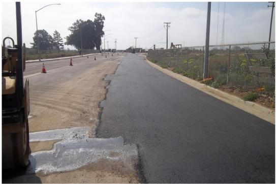
Ramsey Paving completing second lift of paving over trench in Blosser Road.
