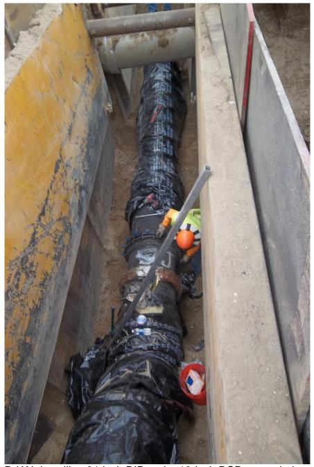
D-KAL installing 24-inch DIP under 18-inch RCP storm drain, approximate Station 12+00.
