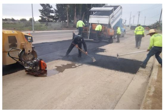
Ramsey Paving placing AC in Blosser Road to complete trench paving to near Taylor Street.
