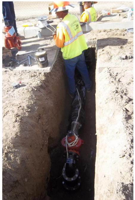
Gate valve installed for CAV at Station 5+33.
