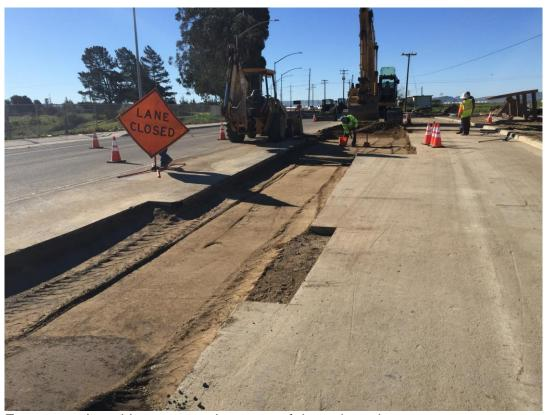
Furgro on site taking compaction tests of the subgrade.
