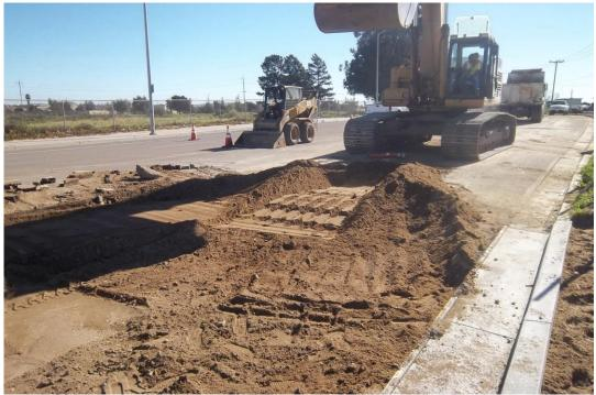
D-KAL backfilling and compacting over the relocated storm drain in Blosser Road.
