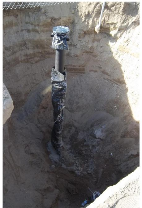
Blow-off and riser installed at the end of the pipe for testing, Station 1+07.
