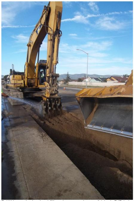
D-KAL continuing backfill and compaction as 24-inch DIP is installed.
