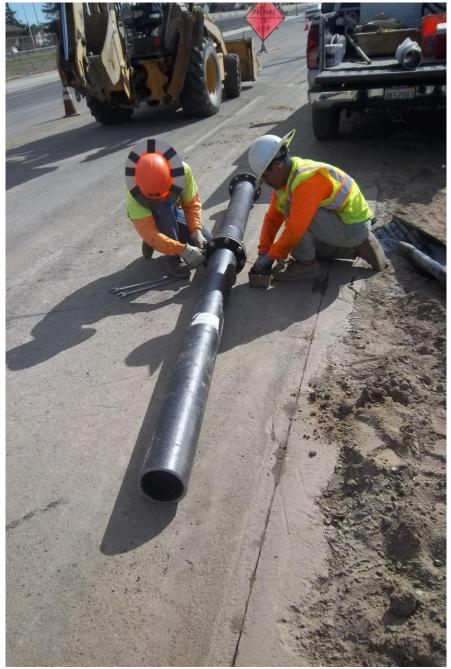
D-KAL putting together the riser for the blow-off at the end of the pipe.
