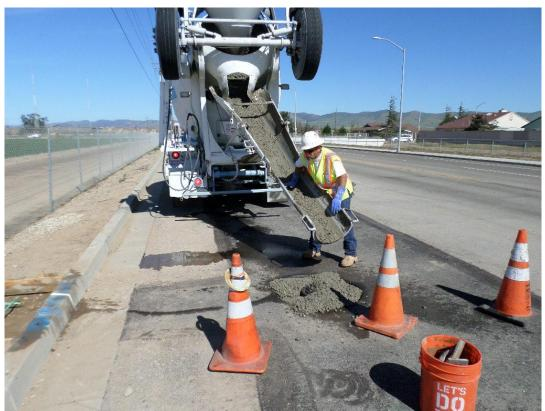
D-KAL pouring the concrete rings around the valve cans.
