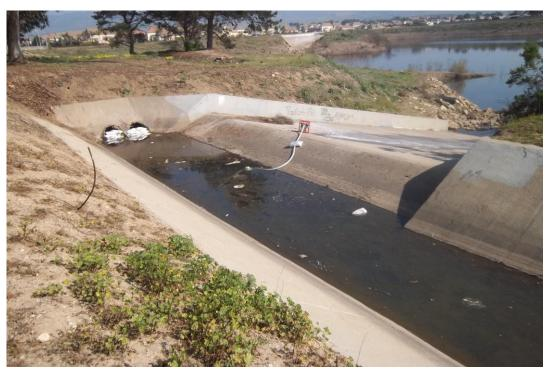
Dechlorinated water released into the storm drain channel being pumped over the spillway into the detention basin for percolating back into the ground water.
