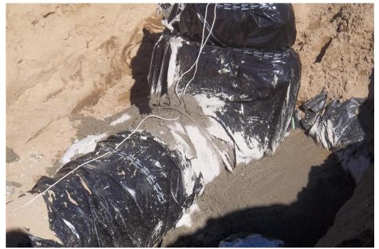
Concrete pad poured under 24-inch gate valve on pig launcher.
