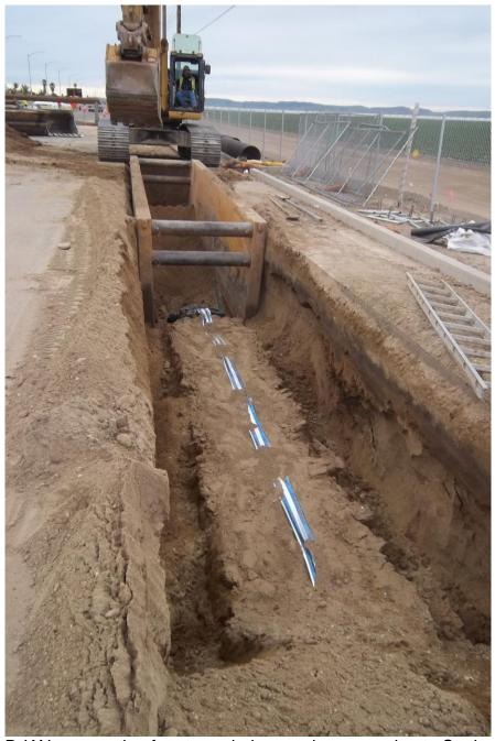
D-KAL excavating for storm drain crossing approximate Station 12+00.
