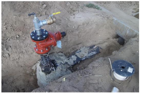
Concrete thrust block under 90 degree riser and gate valve.
