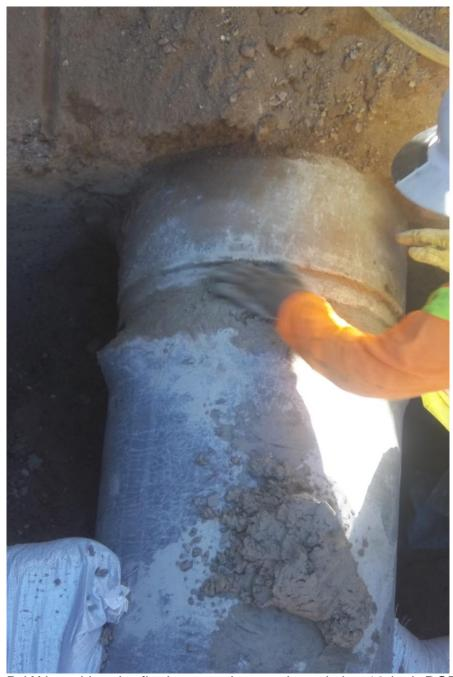
D-KAL making the final connections to the existing 18-inch RCP storm drain with the new and relocated storm drain.
