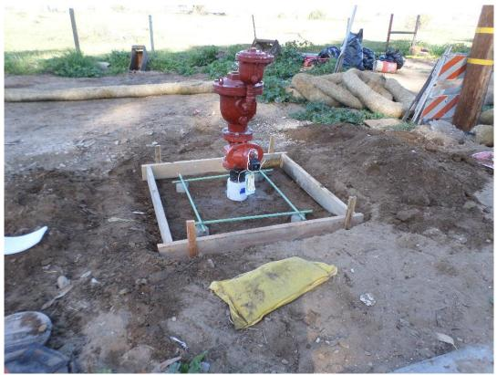
D-KAL installing concrete pads around CAV's.
