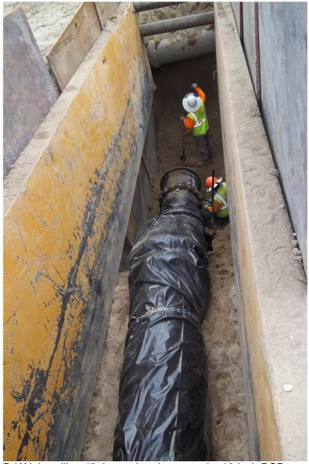
D-KAL installing 45 degree bend to go under 18-inch RCP storm drain crossing.
