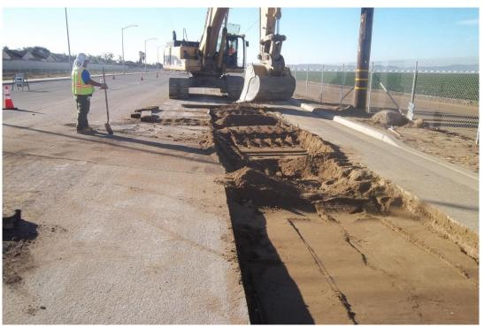
Remvoving existing AC at trench edges where it was sawcut to prepare for final paving, and excavating down for installing AB and asphalt.
