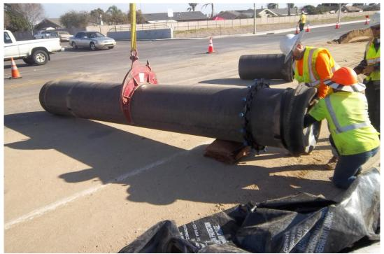
D-KAL installing the blind flange on the end of the last piece of pipe at Taylor Street.
