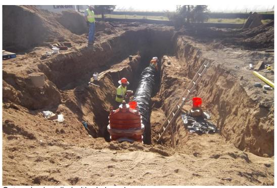
Gate valve installed with pig launcher.
