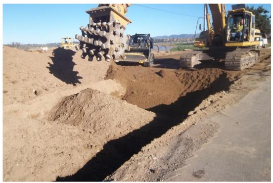
D-KAL removing the existing 18-inch RCP storm drain in Blosser Road which was located too close to the new waterline, and backfilling and compacting the native material as it is removed.
