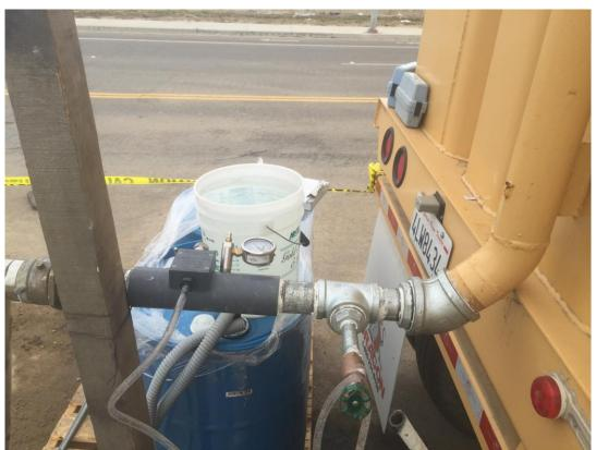
Sodium hyplchlorite injection and monitoring for dechlorinating water flushed from 24-inchDIP into Baker tank.
