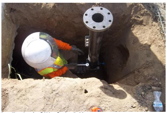
Installing riser for CAV at Station 5+33.
