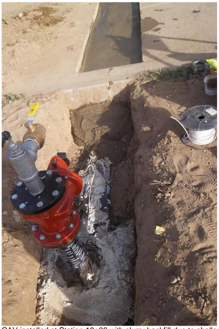
CAV installed at Station 18+06 with slurry backfill due to shallow depth of pipe.
