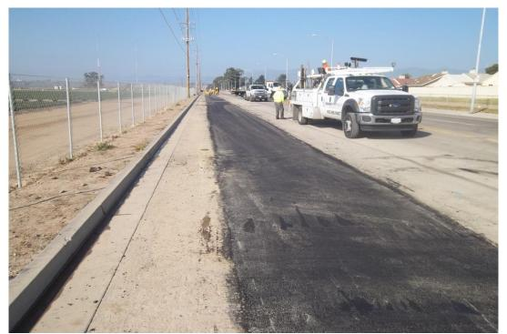
Ramsey paving completing paving of trench in Blosser to near the end at Taylor.
