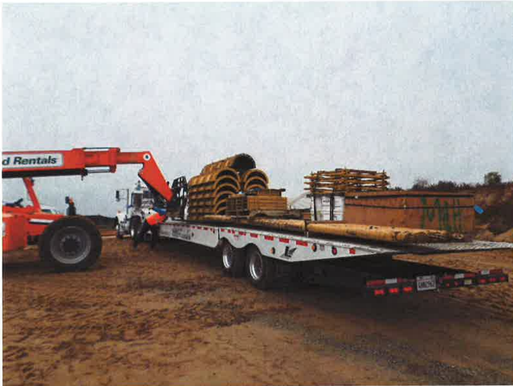
Wall and column forms being delivered to site.
