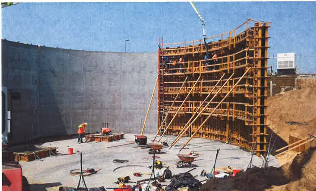
PHC performing third wall pour.
