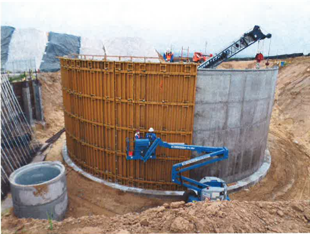
Removing form ties from the second wall pour the following day.
