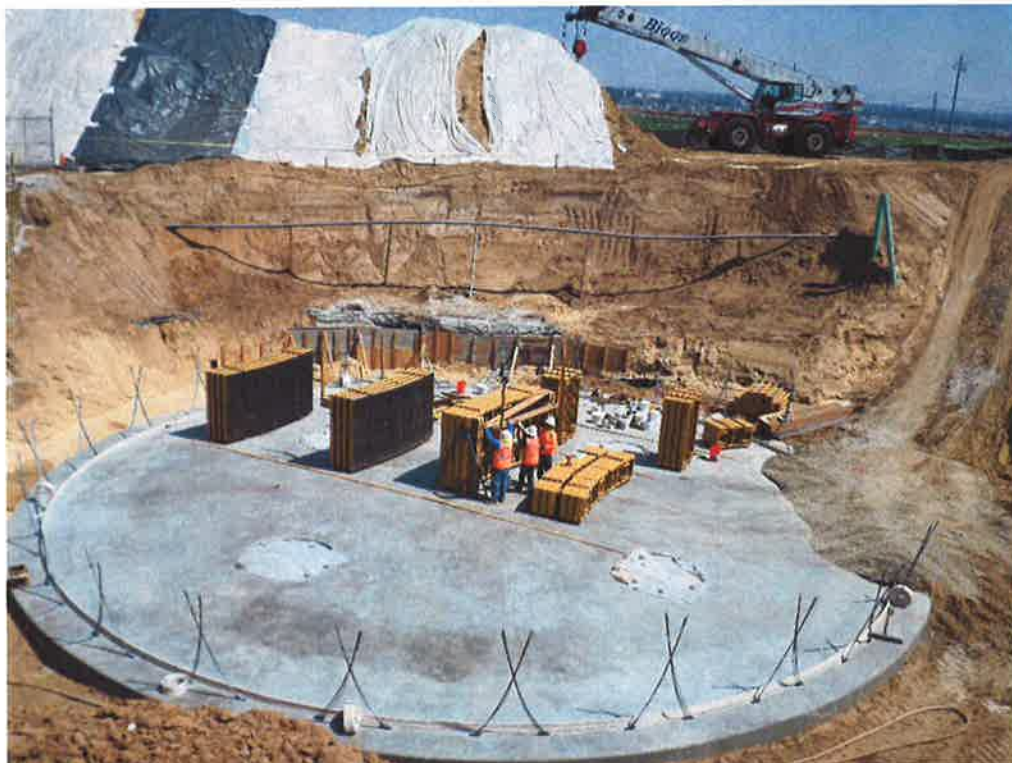
PHC staging wall forms.
