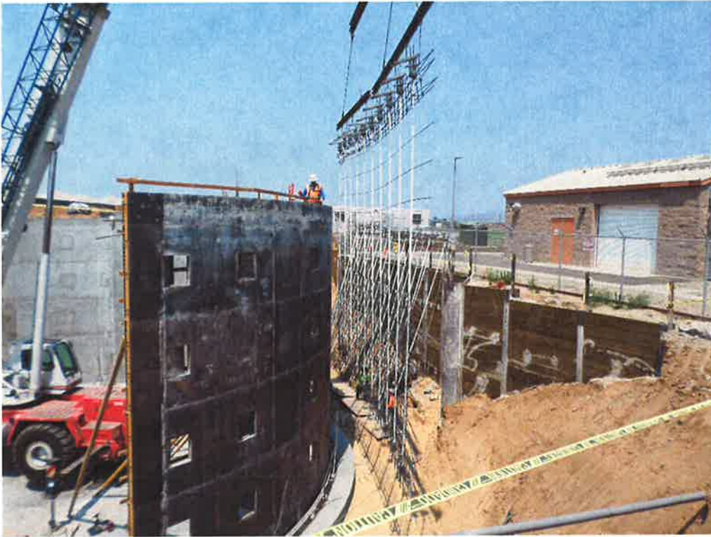
PHC moving reinforcing into place for third wall pour.
