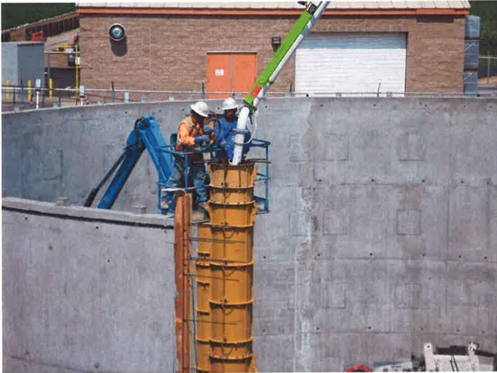
PHC pouring columns during fourth wall pour.
