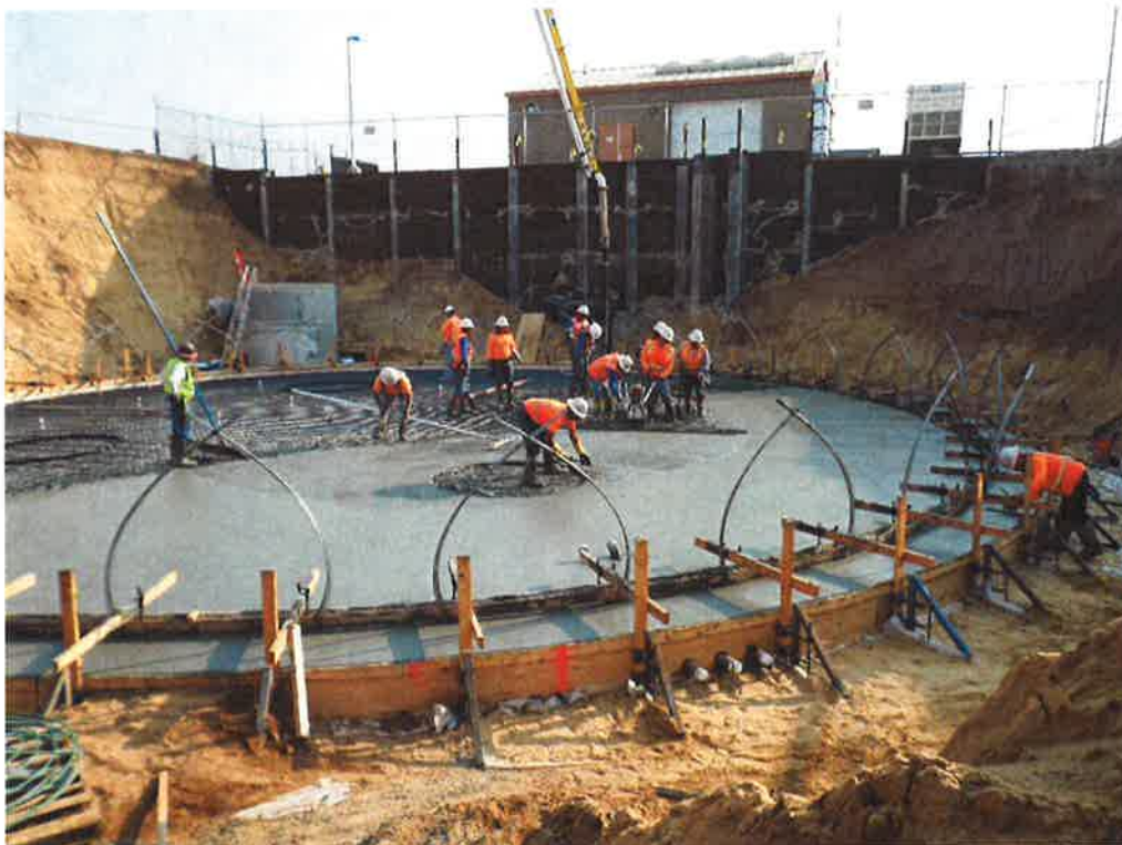
PHC pouring and finishing concrete for the tank slab.
