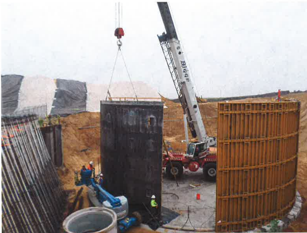
PHC removing interior wall forms from first wall pour the following day and setting forms in place for the second wall pour 48 hours later.
