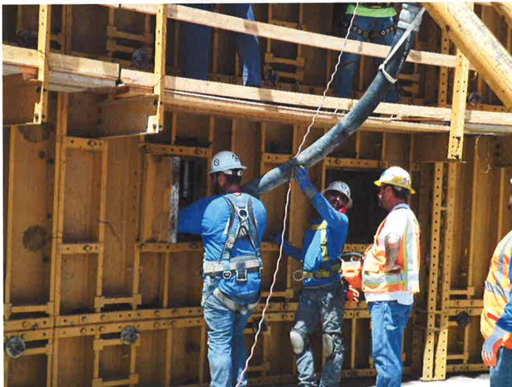
PHC starting first wall pour at ground level using windows in forms to place concrete.
