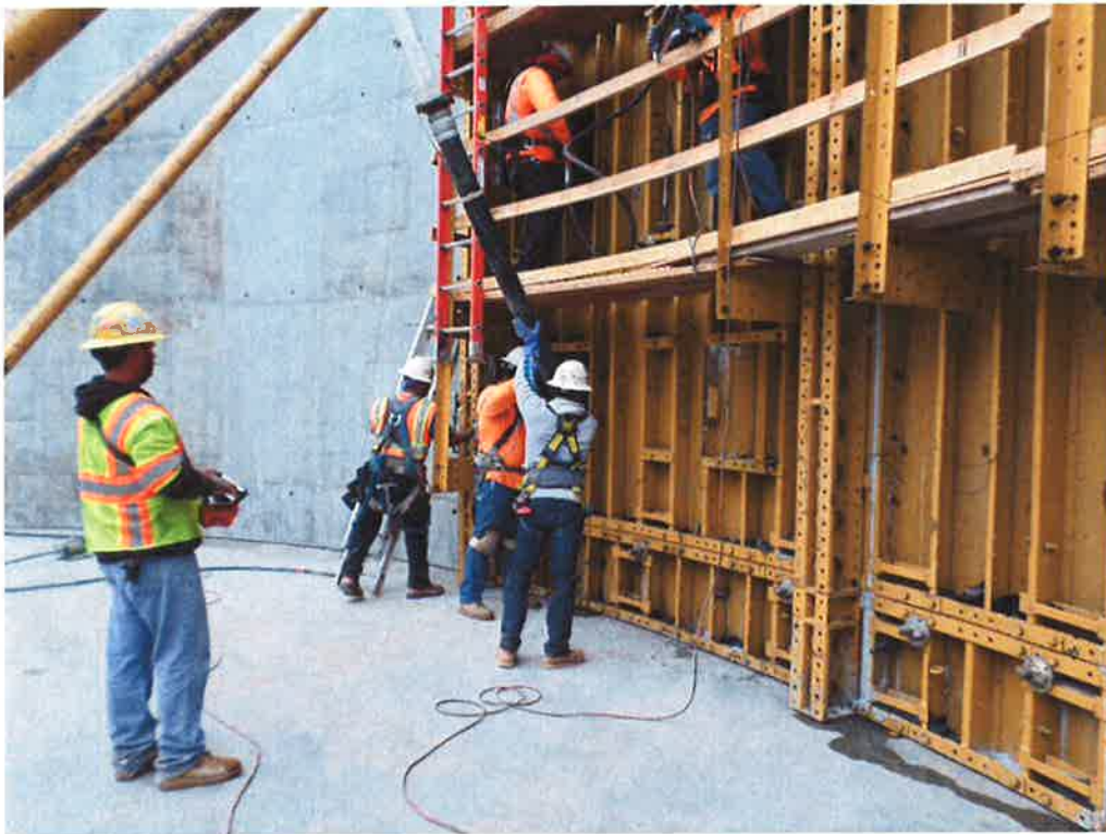
Concrete pump operator and PHC pouring second wall.
