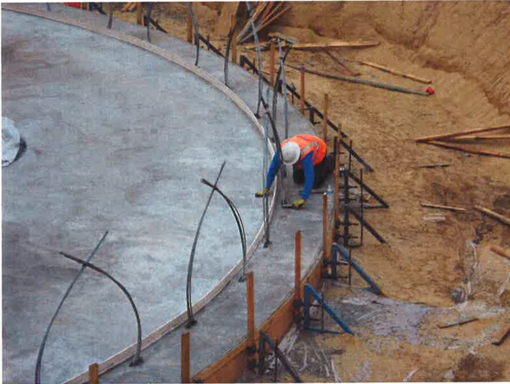
PHC cleaning up the water stop and concrete slab after stripping the template.
