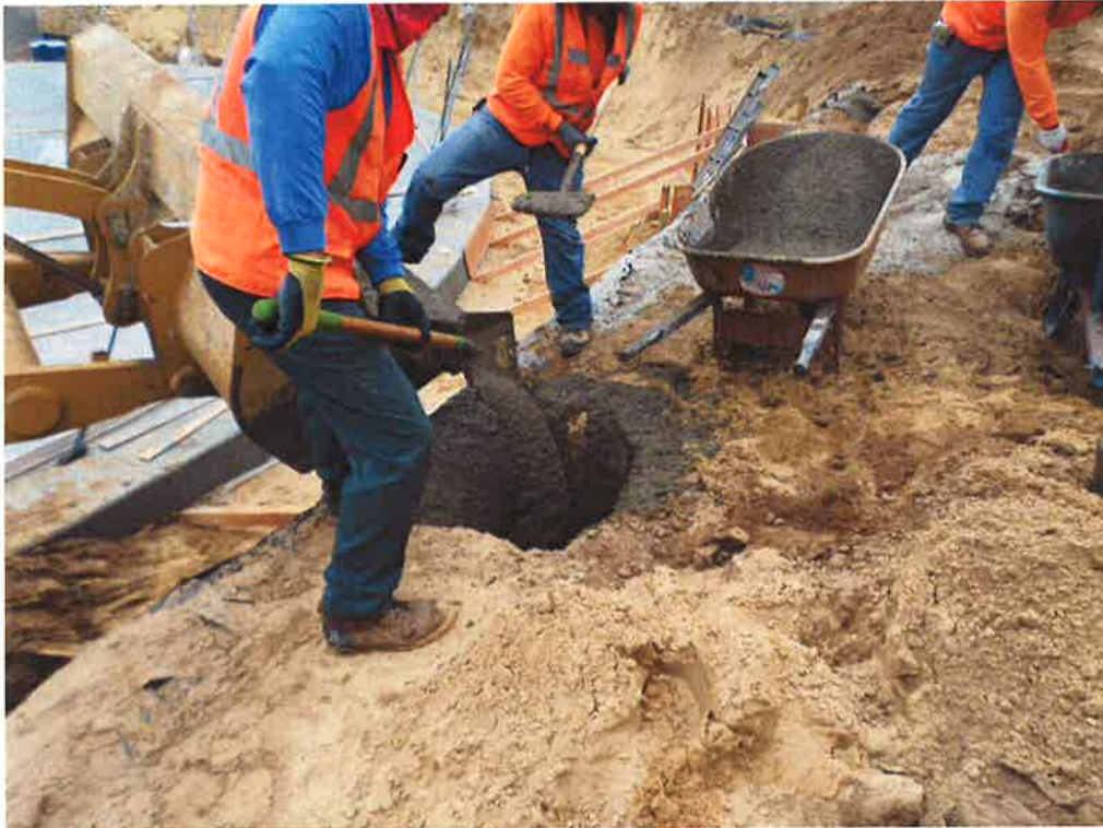
PHC pouring slurry behind plywood and underneath 24-inch inlet pipe to provide a support for the pipe and stabilize material below pipe.
