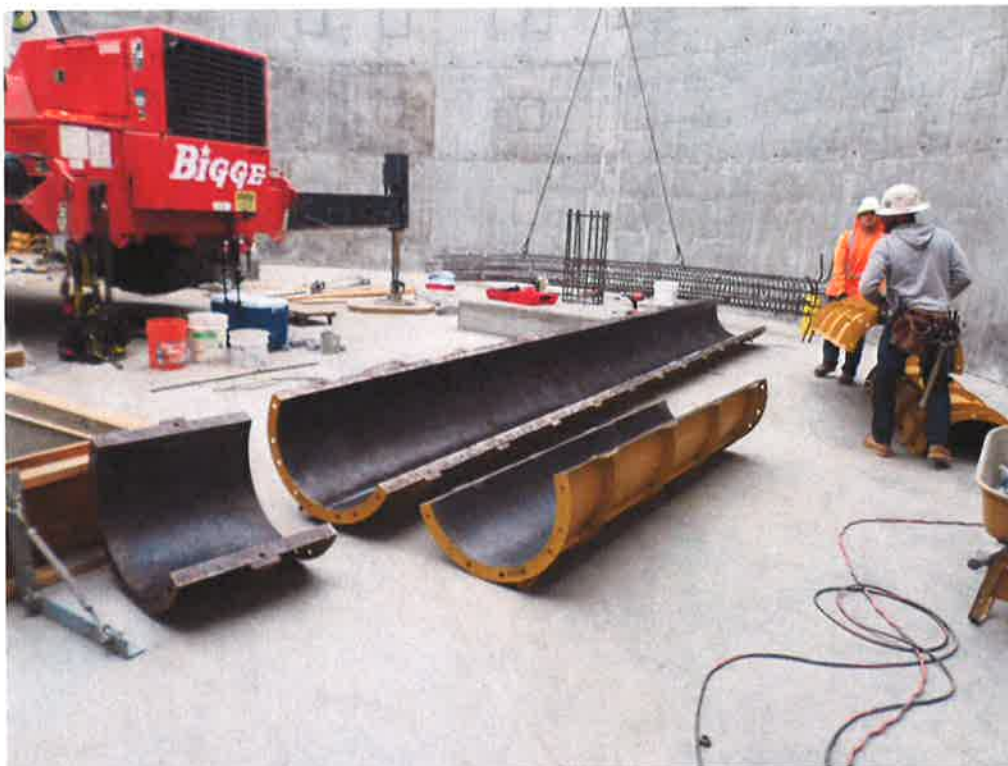
Assembling column forms.
