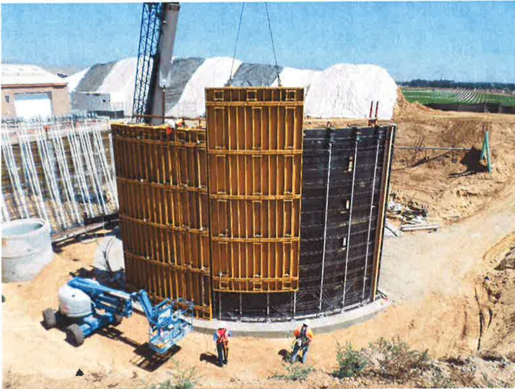
PHC setting exterior wall forms into place.
