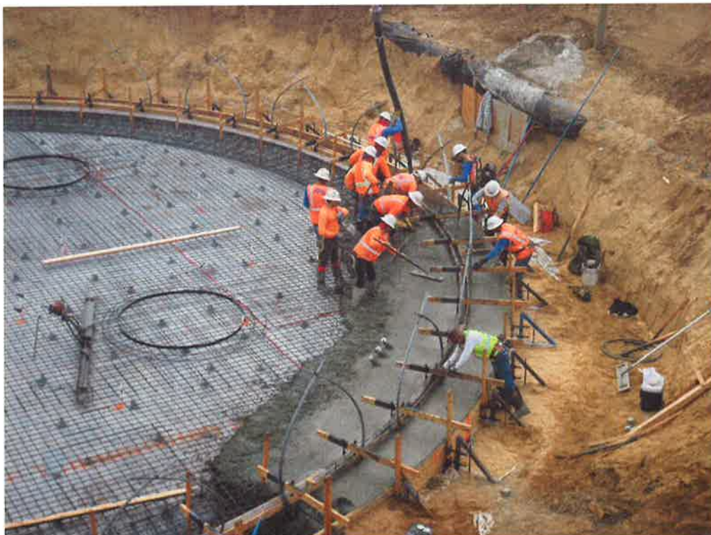
PHC pouring concrete for tank slab.
