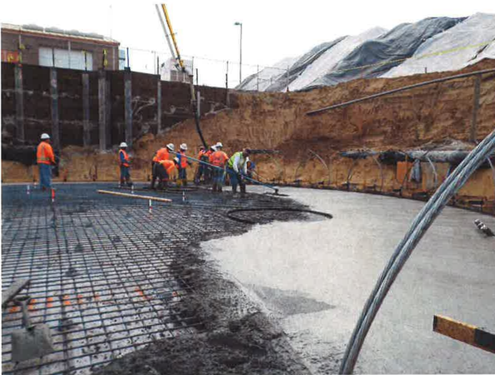
PHC pouring and finishing concrete for tank slab.
