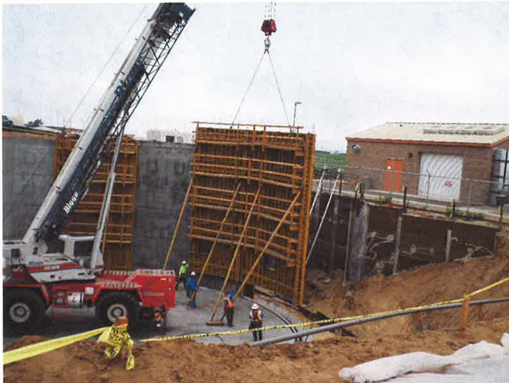
PHC removing wall forms from the second concrete pour.
