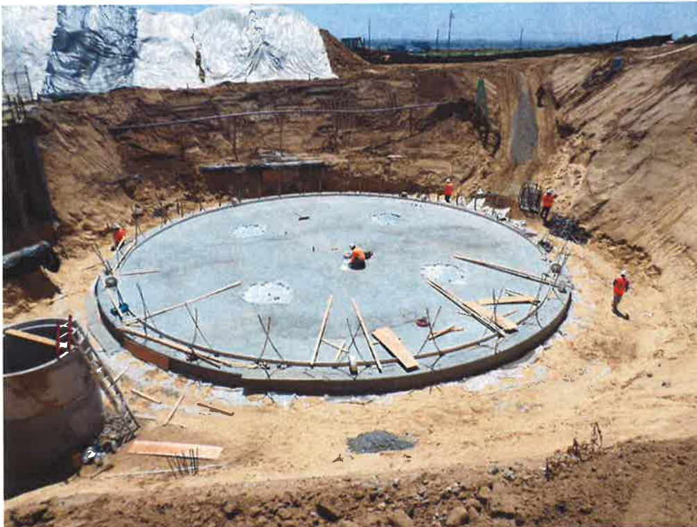
PHC stripping forms from concrete slab pour.
