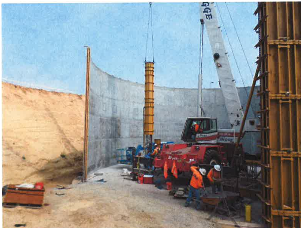
Setting column forms and reinforcing into place.
