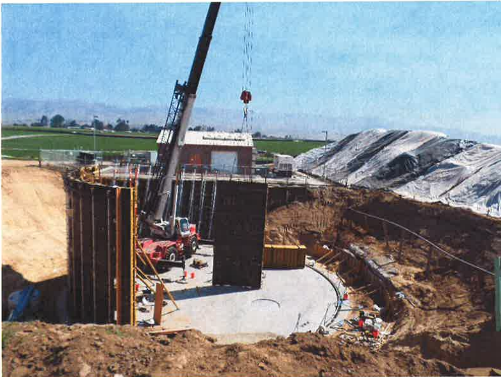
PHC moving exterior wall forms for the first wall pour into place.
