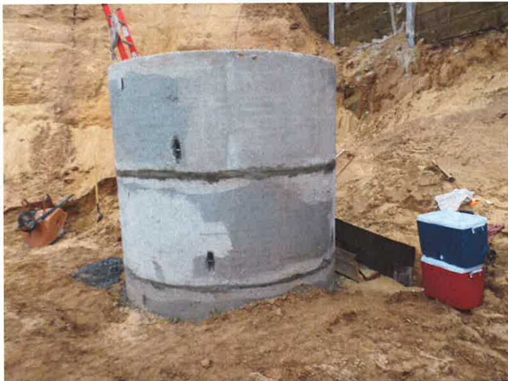
Patching joints at the manhole.
