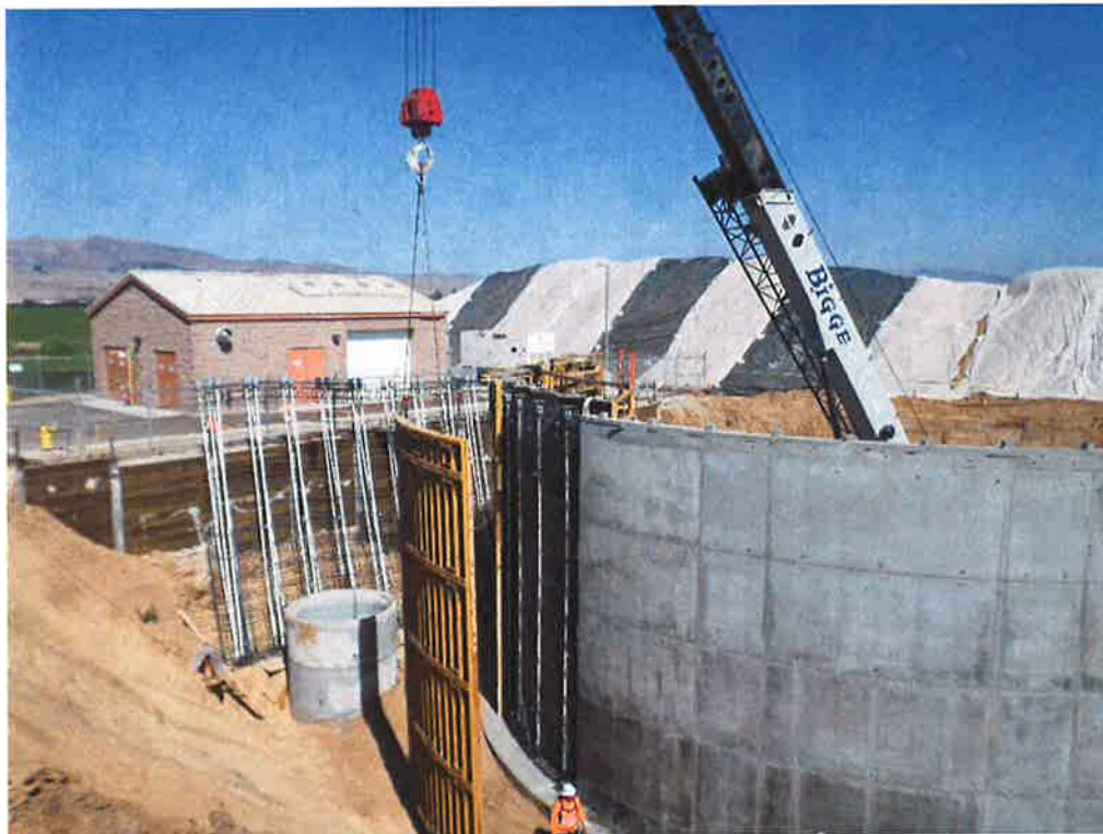
Moving exterior forms into place for the second wall pour.
