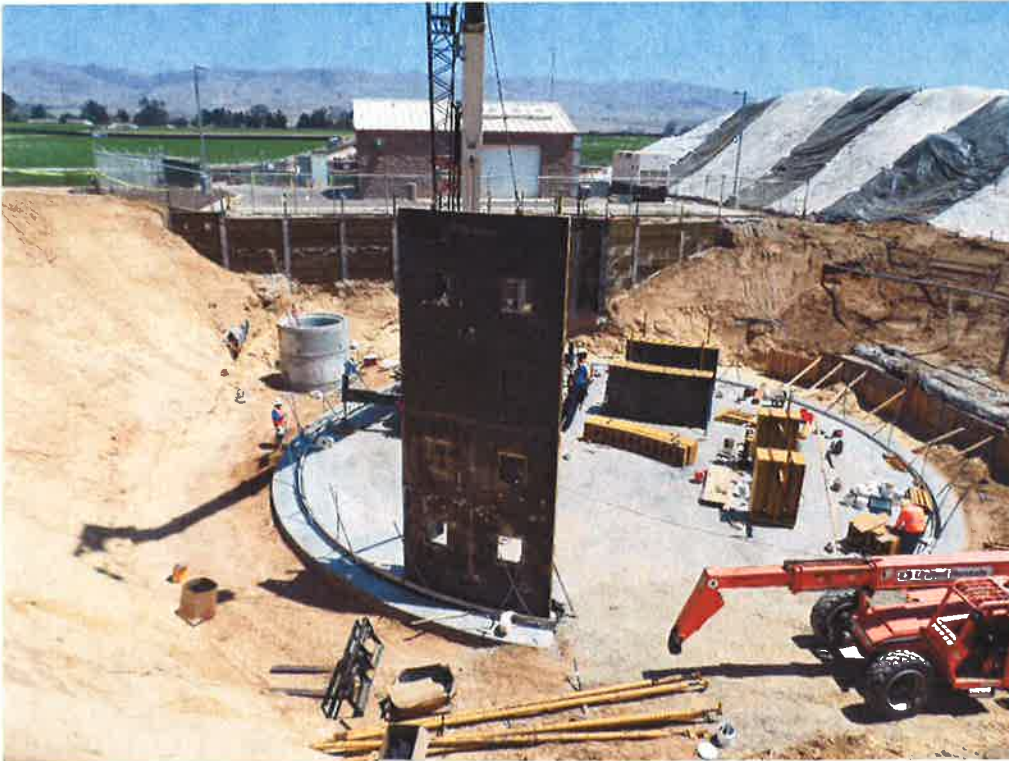
PHC setting the interior wall forms for the first wall pour.
