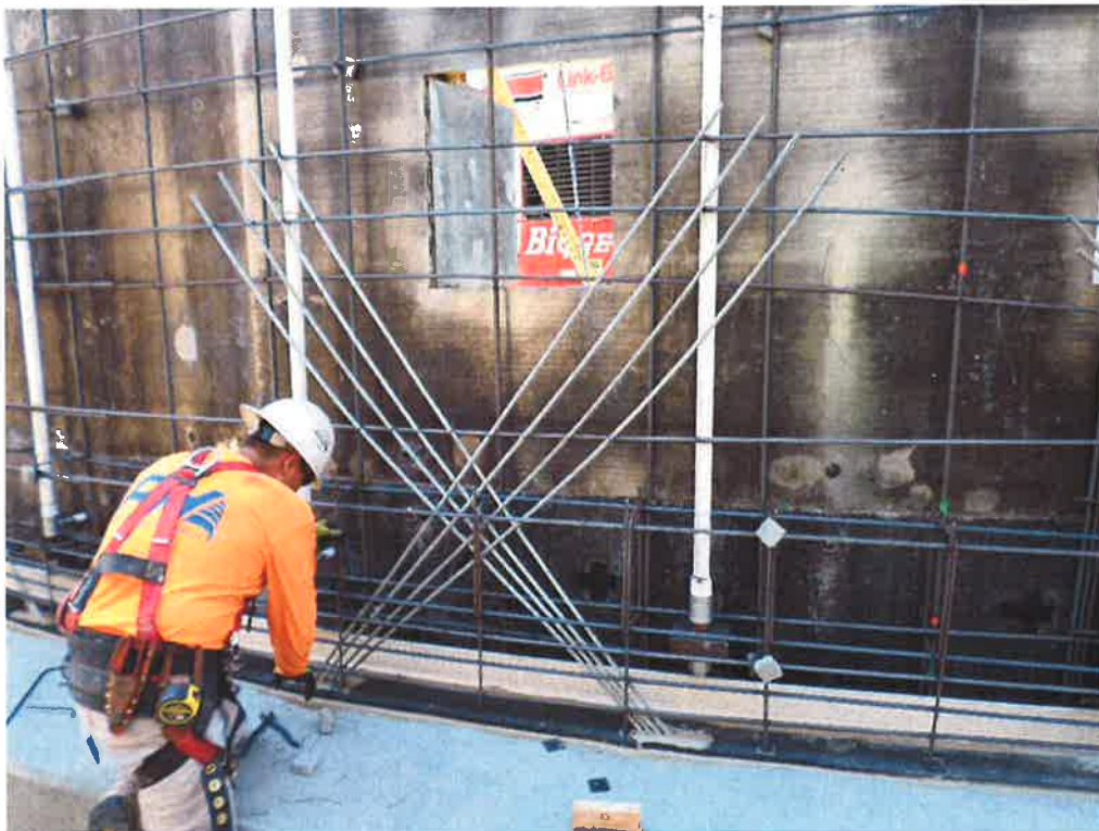
PHC tying off seismic cables to reinforcing for third wall pour.
