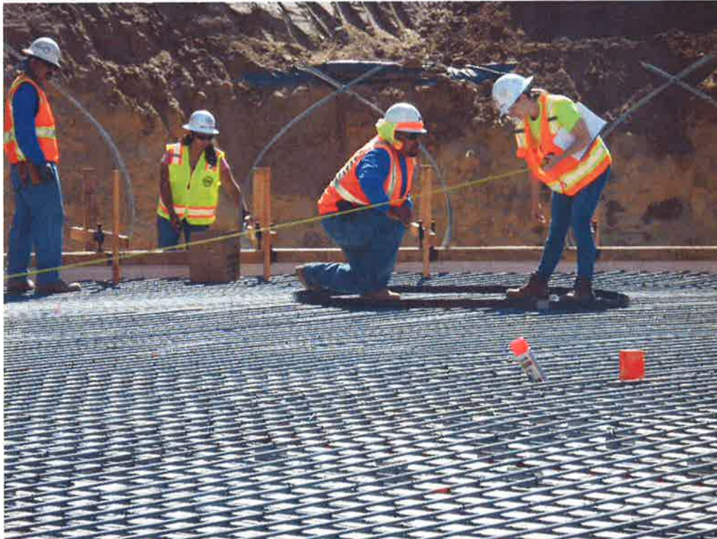
DN Tank inspectors reviewing reinforcing before concrete pour of tank slab.
