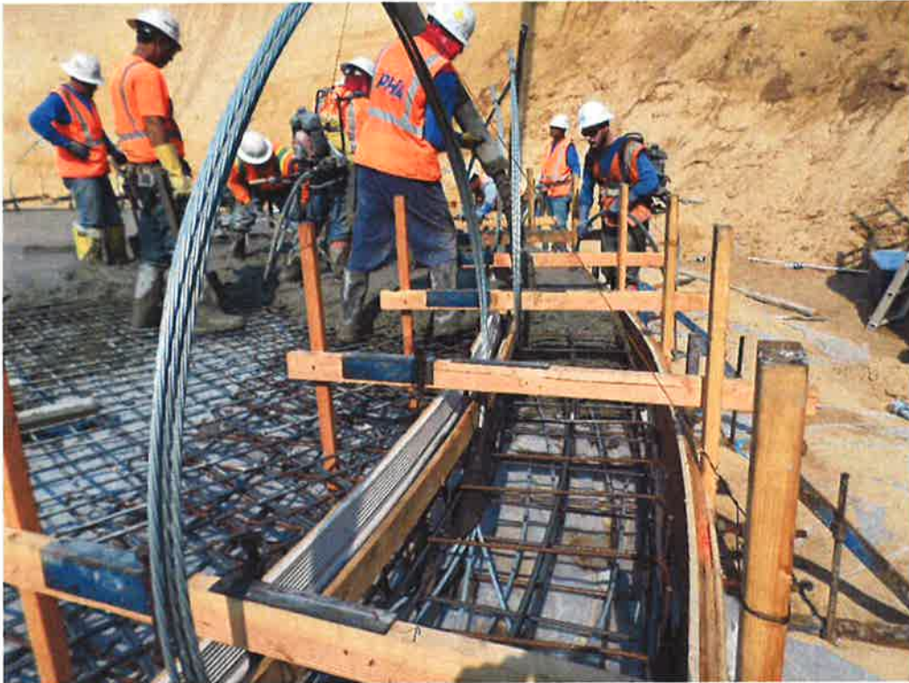
PHC pouring footing around concrete slab for reservoir.
