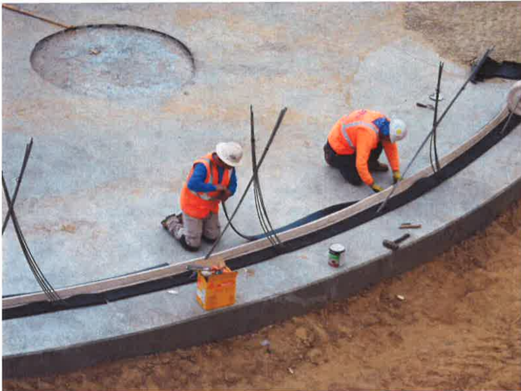
PHC installing bearing pad for walls.
