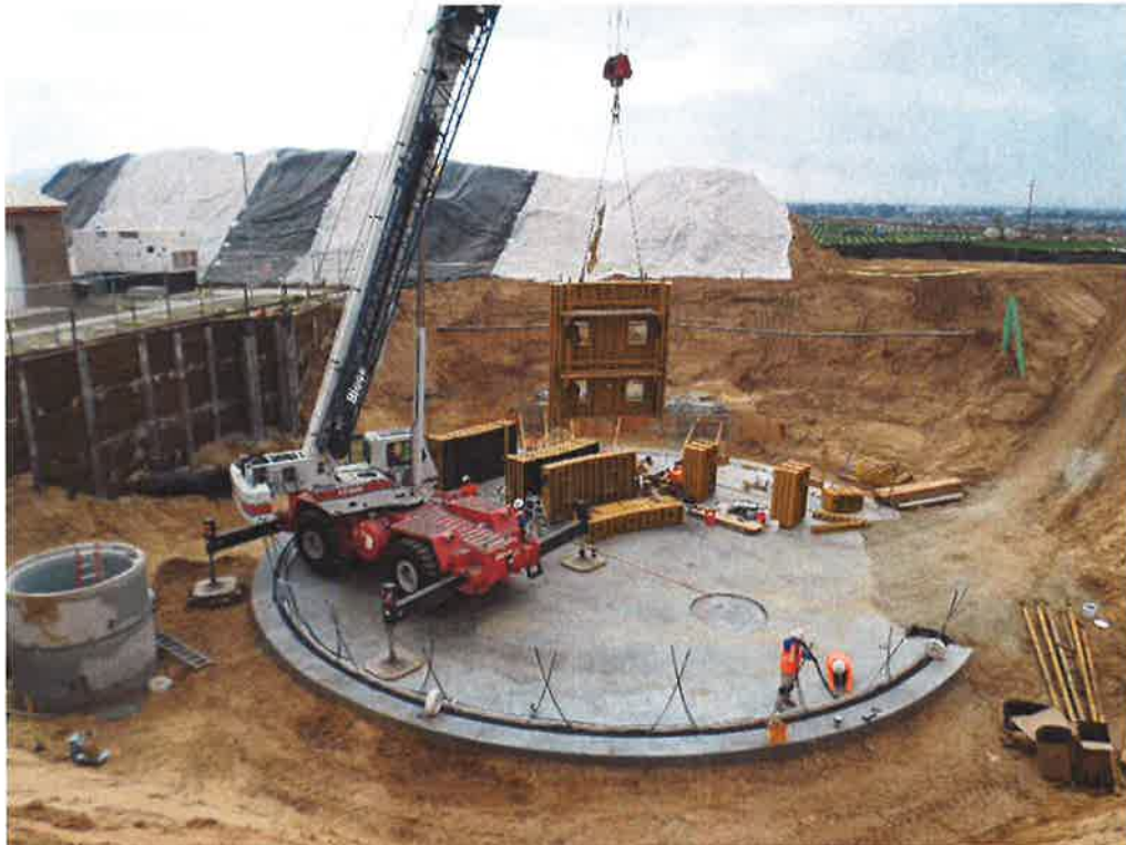
PHC assembling the forms for the reservoir walls.
