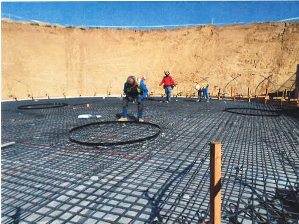
Monroy Steel correcting reinforcing clearances.
