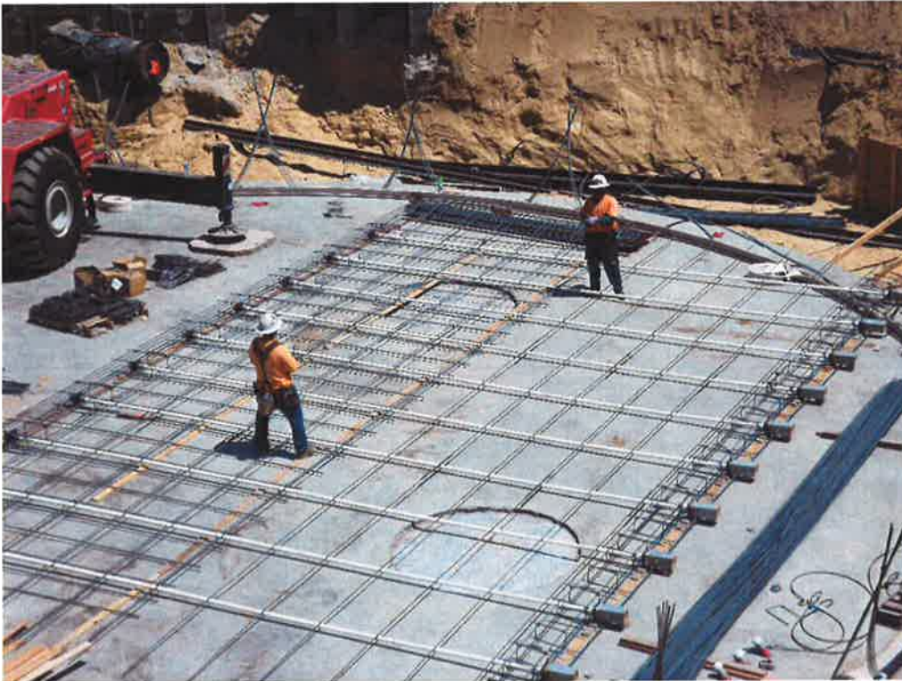
Monroy Steel tying wall reinforcing for the first wall pour.
