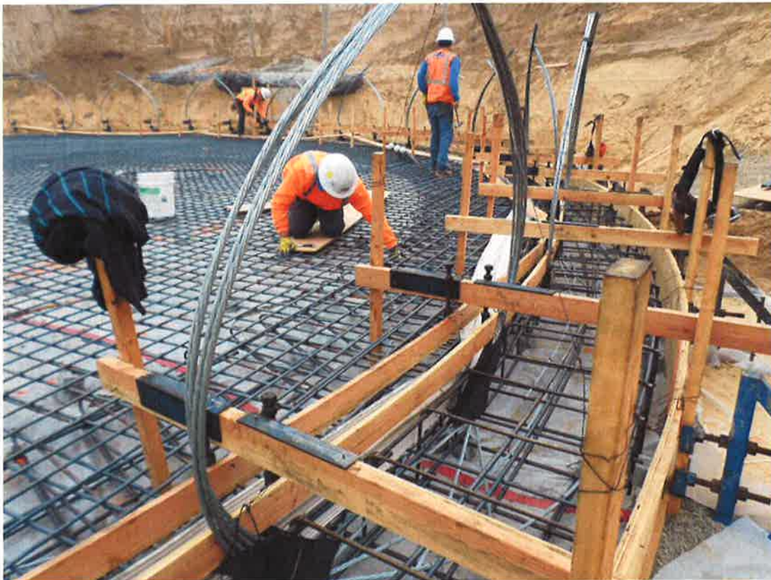
Monroy Steel correcting clearances of reinforcing.
