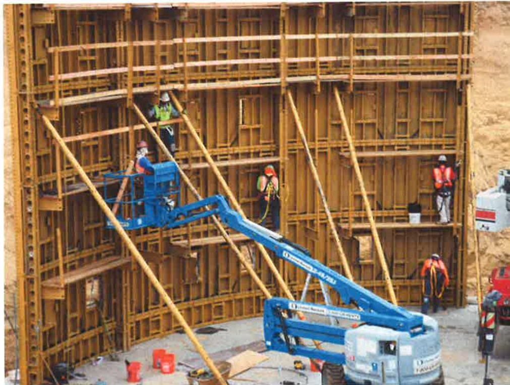
PHC tightening bolts to secure wall forms and installing wall planks.
