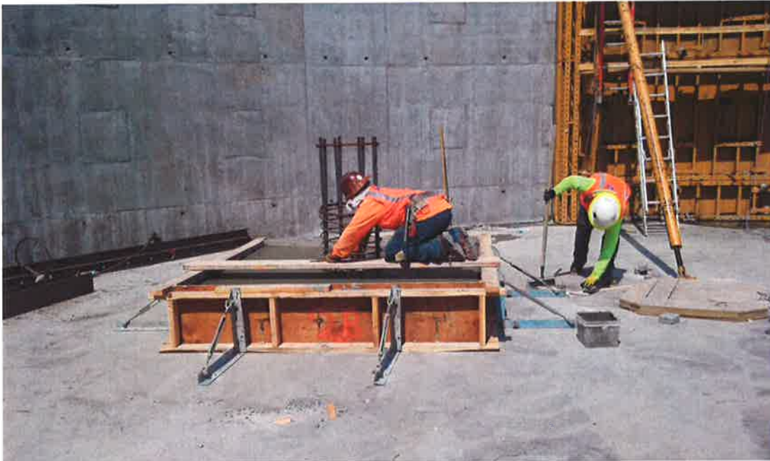
PHC pouring base for concrete columns.
