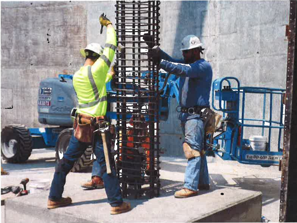
PHC setting column forms and reinforcing into place on column base.
