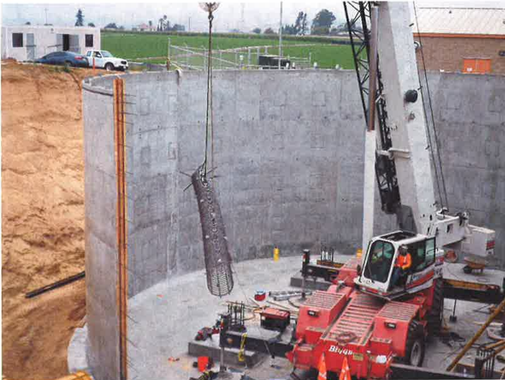
PHC lowering column reinforcing to the reservoir slab.
