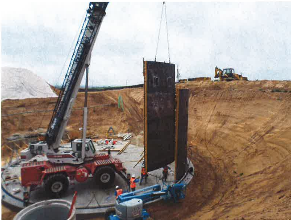
PHC assembling the wall interior wall forms for the first wall pour.
