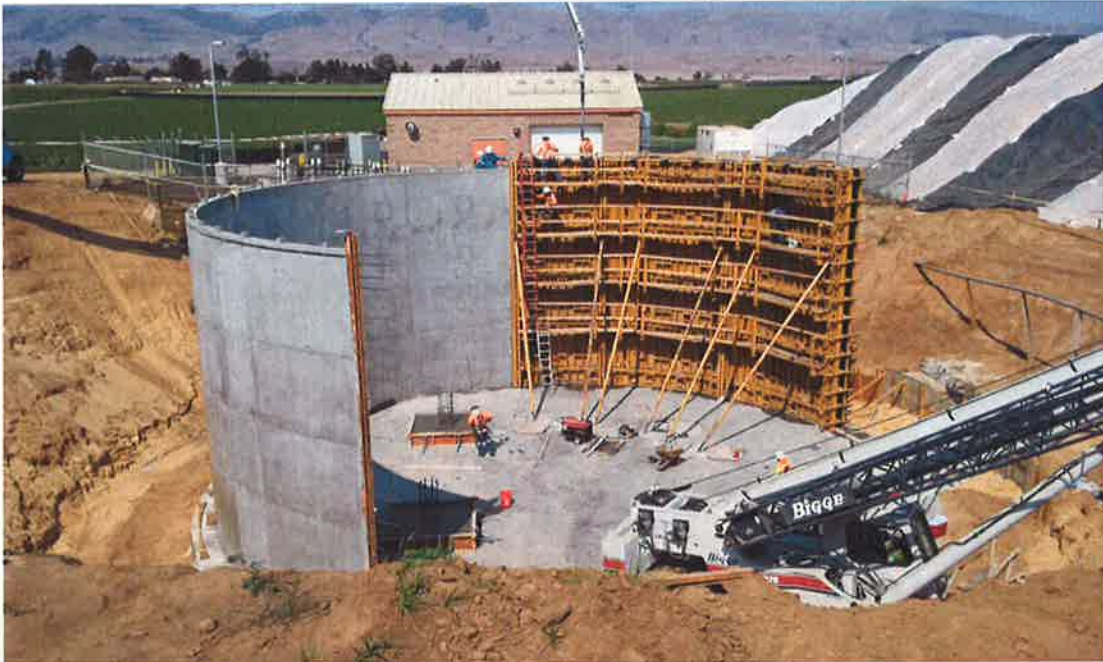
PHC completing third wall pour.
