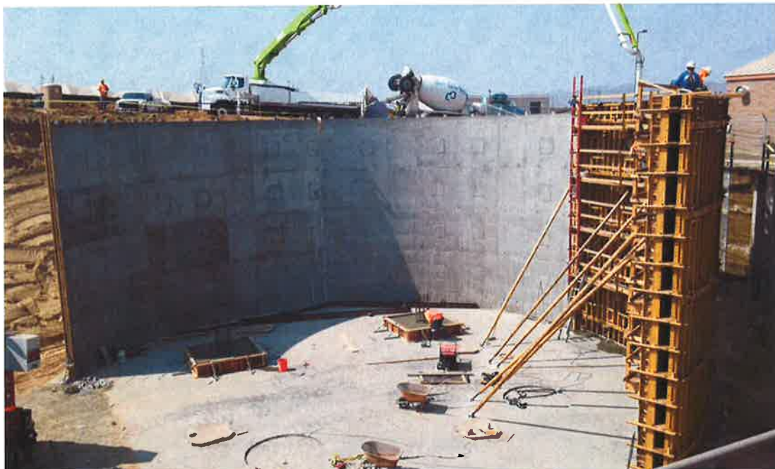
PHC completing third wall pour.
