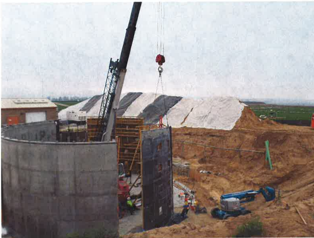
Removing wall forms from the second wall pour and setting them into place for the third wall pour the following day.
