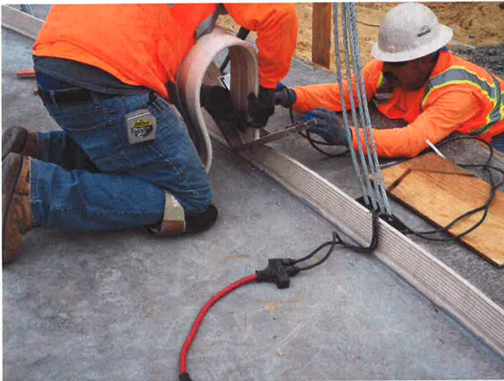
Heat welding water stops.
