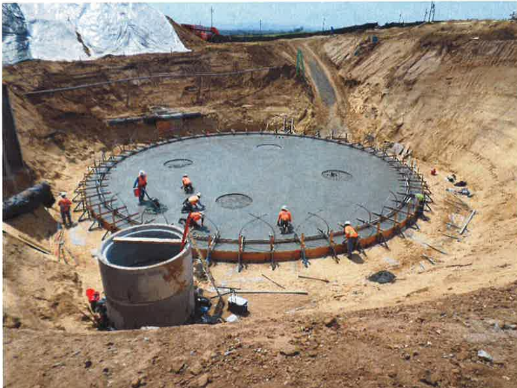
PHC completing finish work on reservoir slab concrete pour.
