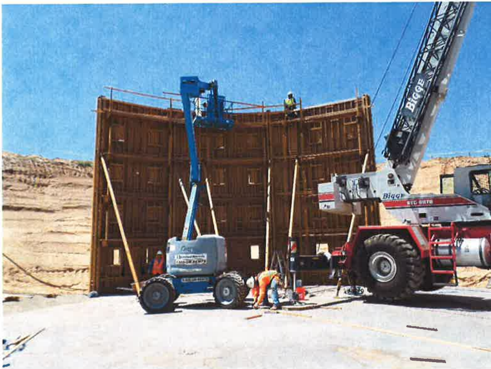
PHC assembling the wall forms for the first wall pour.
