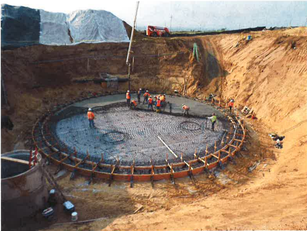
PHC pouring concrete for tank slab.
