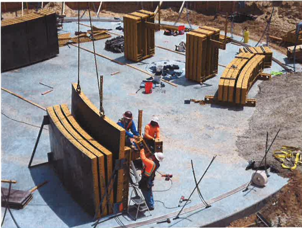
PHC starting assembly of reservoir wall forms.
