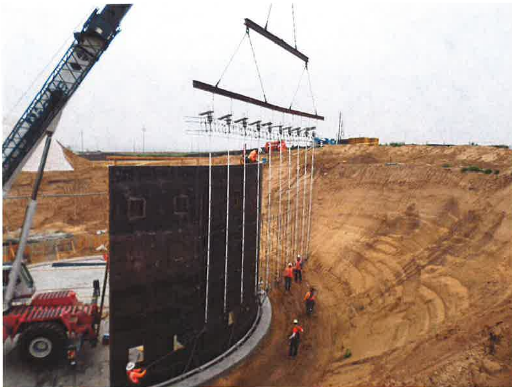
Moving wall reinforcing into place for the first wall pour.
