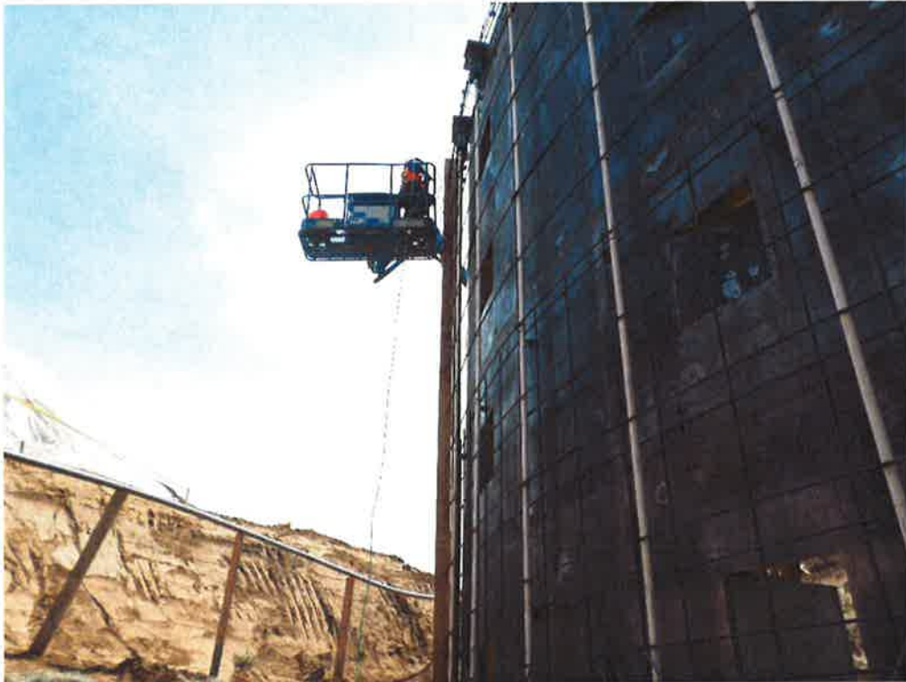
PHC installing water stop and bulkhead for third wall pour.
