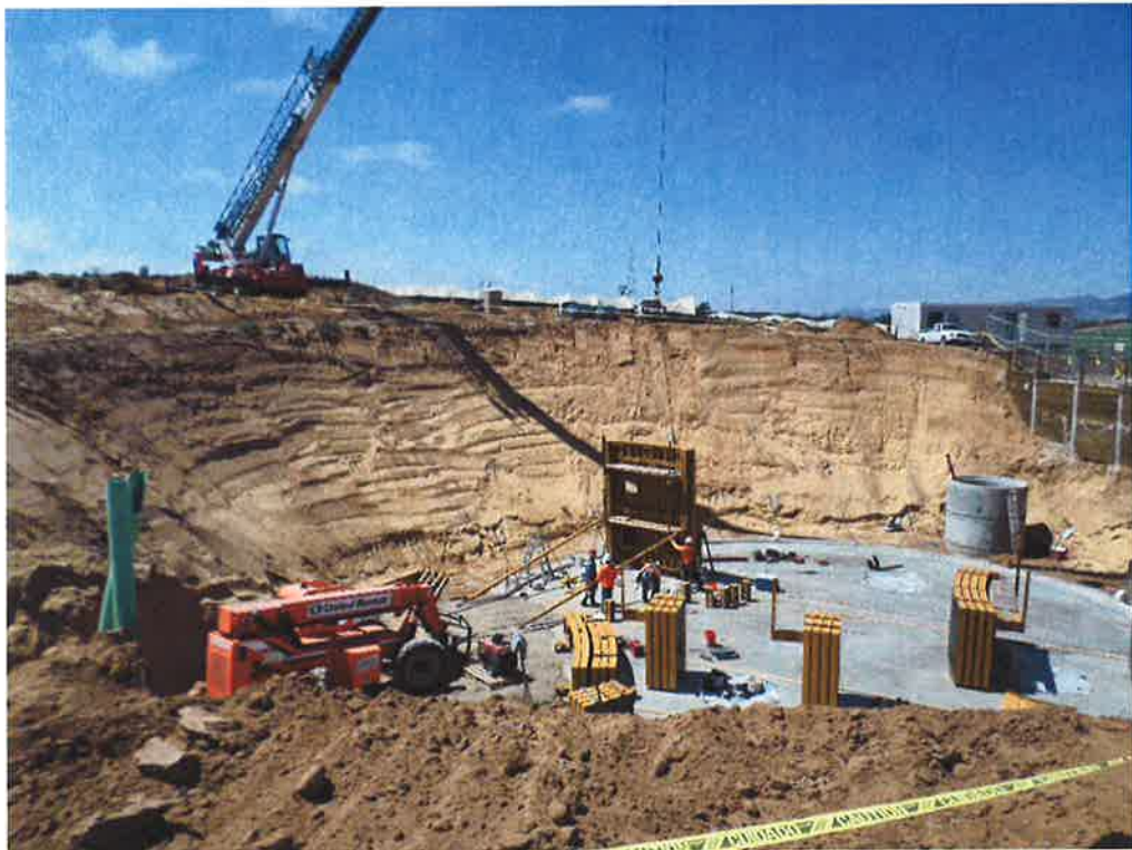
PHC assembling reservoir wall forms.
