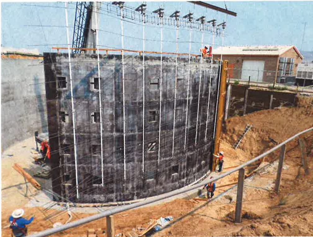
PHC moving reinforcement into place for the fourth wall pour.
