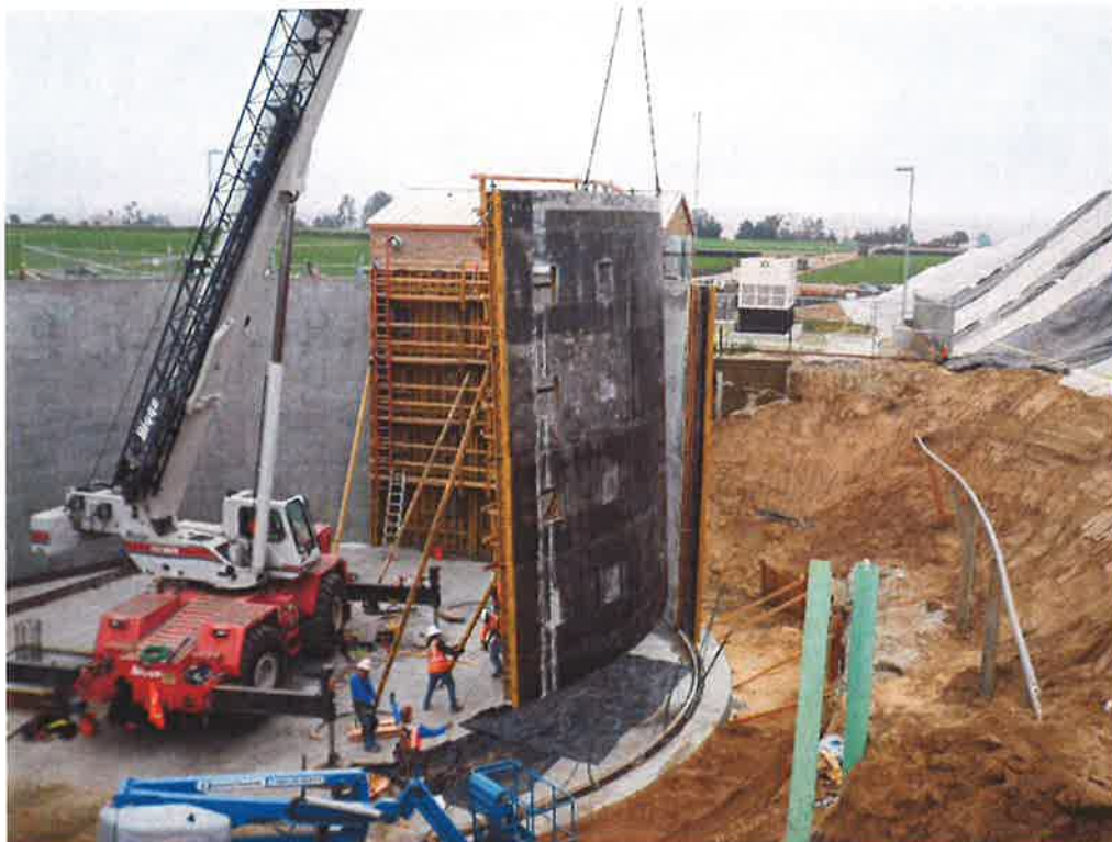
Removing forms the day after the third wall pour and setting into place for the fourth wall pour.
