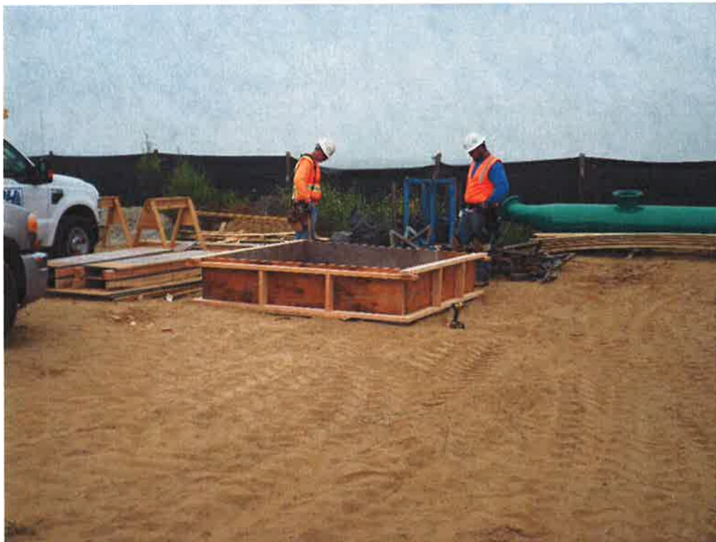
PHC constructing forms for column bases.
