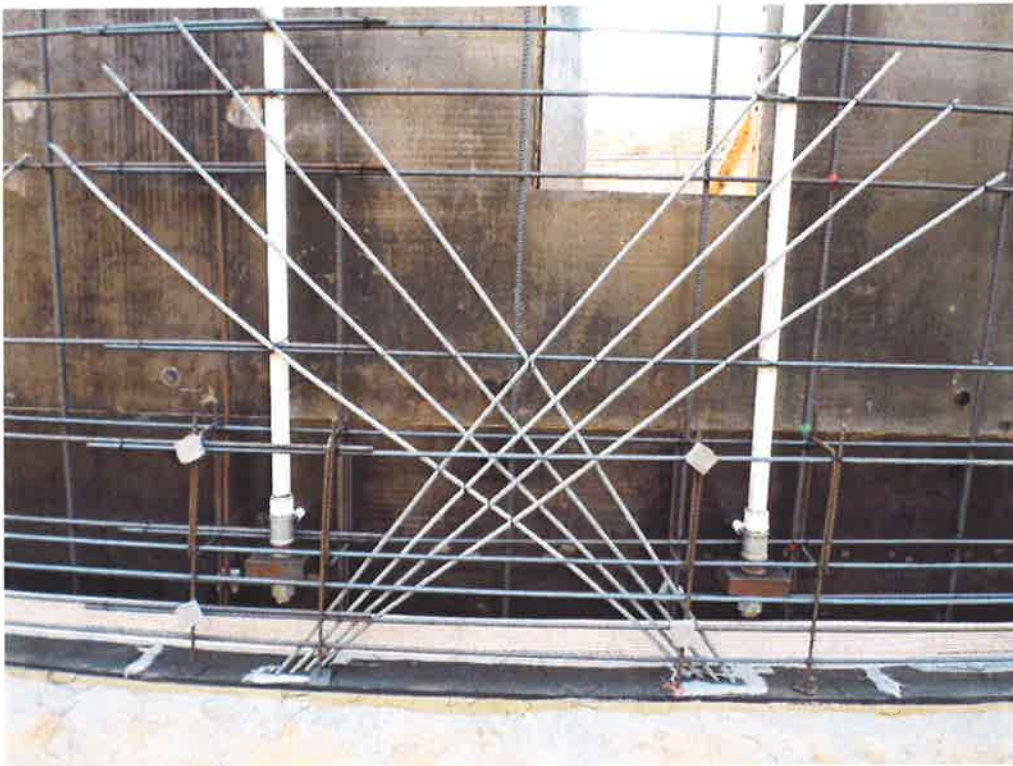
Wall reinforcing tied off to seismic cables.
