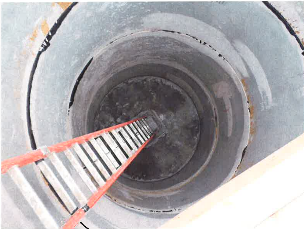
Sloped floor poured inside manhole.
