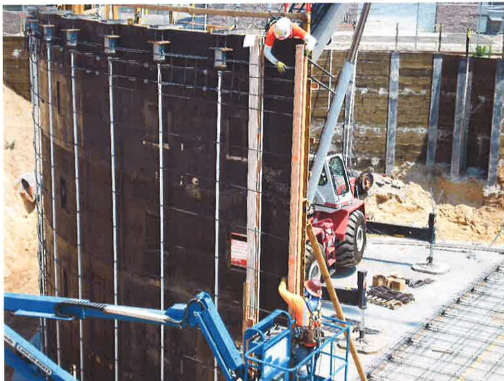
PHC installing the bulkheads and the water stop.
