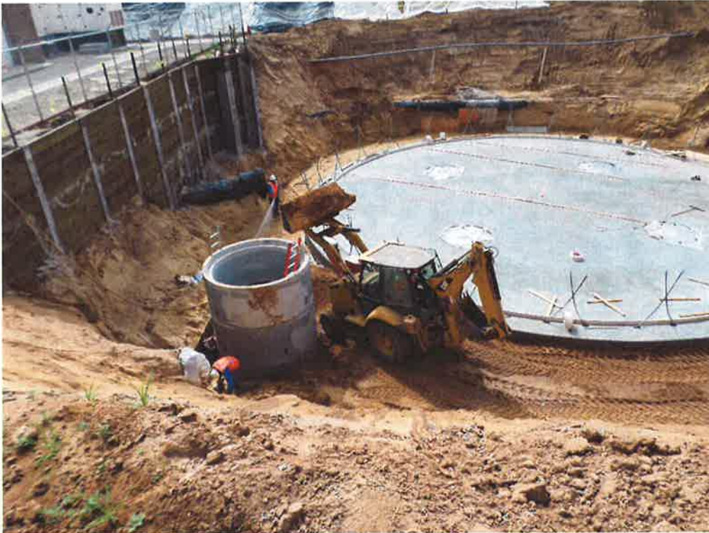
PHC placing native material around the outside of the slab and the manhole after form stripping.
