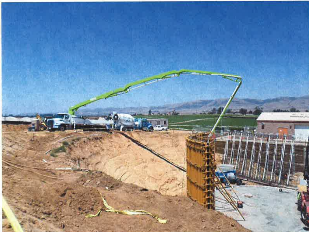
Concrete pump used for first wall pour.
