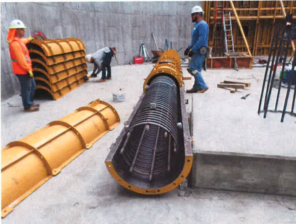
Reinforcing installed inside column form.
