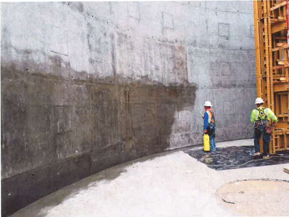
PHC spraying curing compound after interior wall form is removed.
