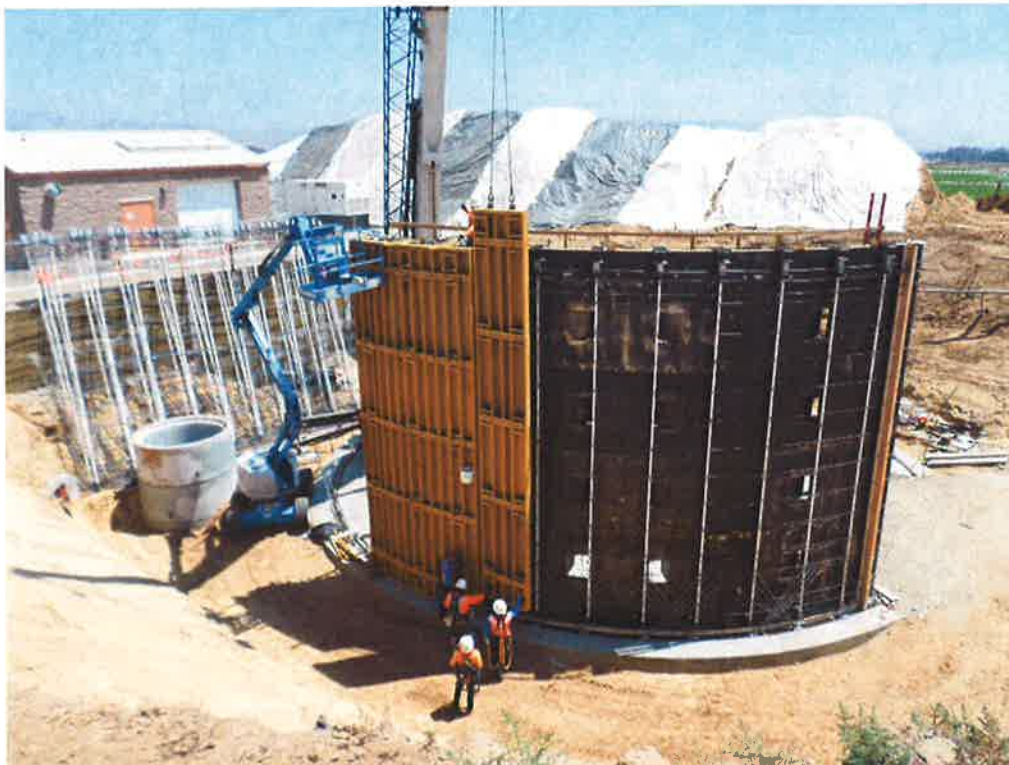
PHC moving exterior wall forms into place for the first wall pour.
