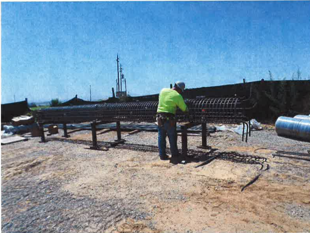
Monroy Steel tying reinforcing for concrete columns inside reservoir.
