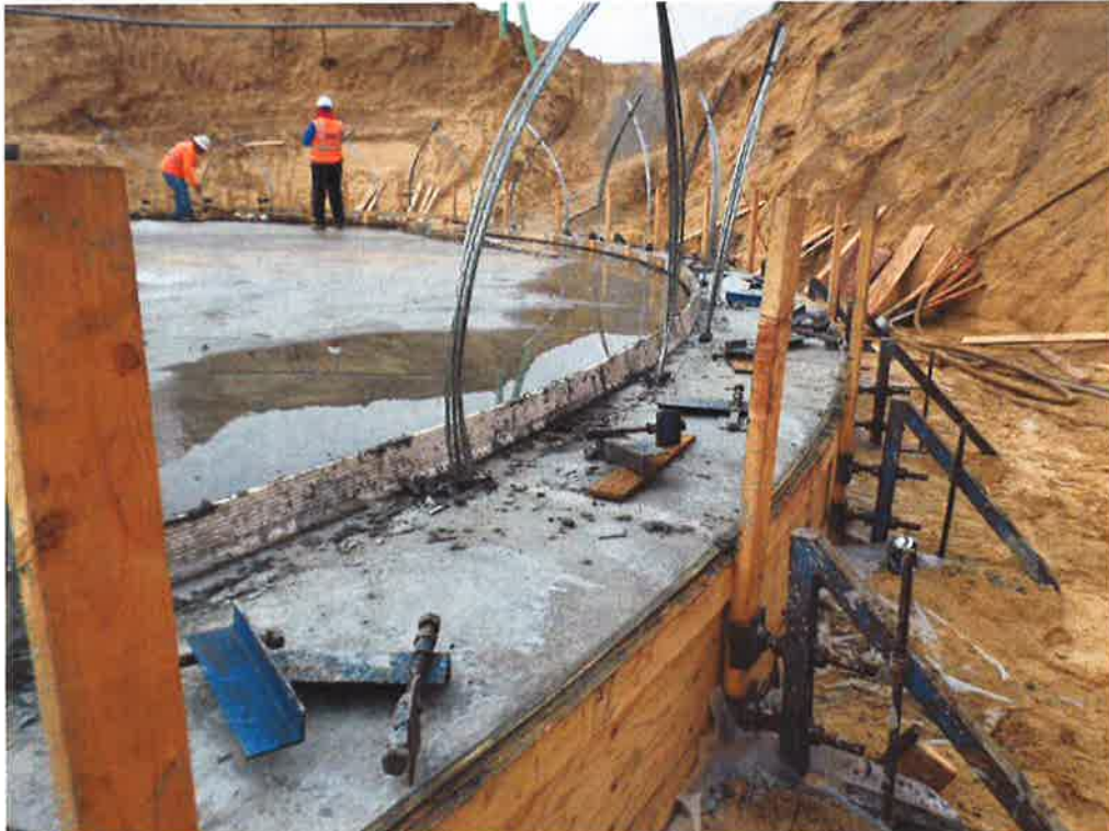
PHC stripping the water stop template after the reservoir slab concrete pour.
