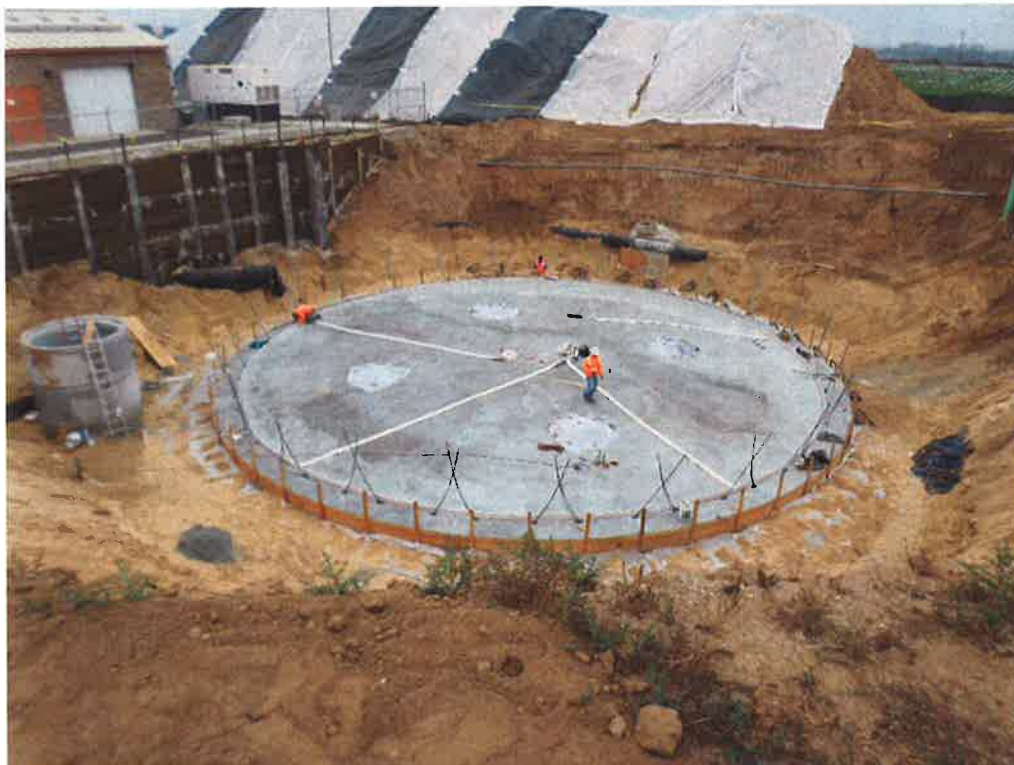
PHC laying out water stop for wall construction joints.
