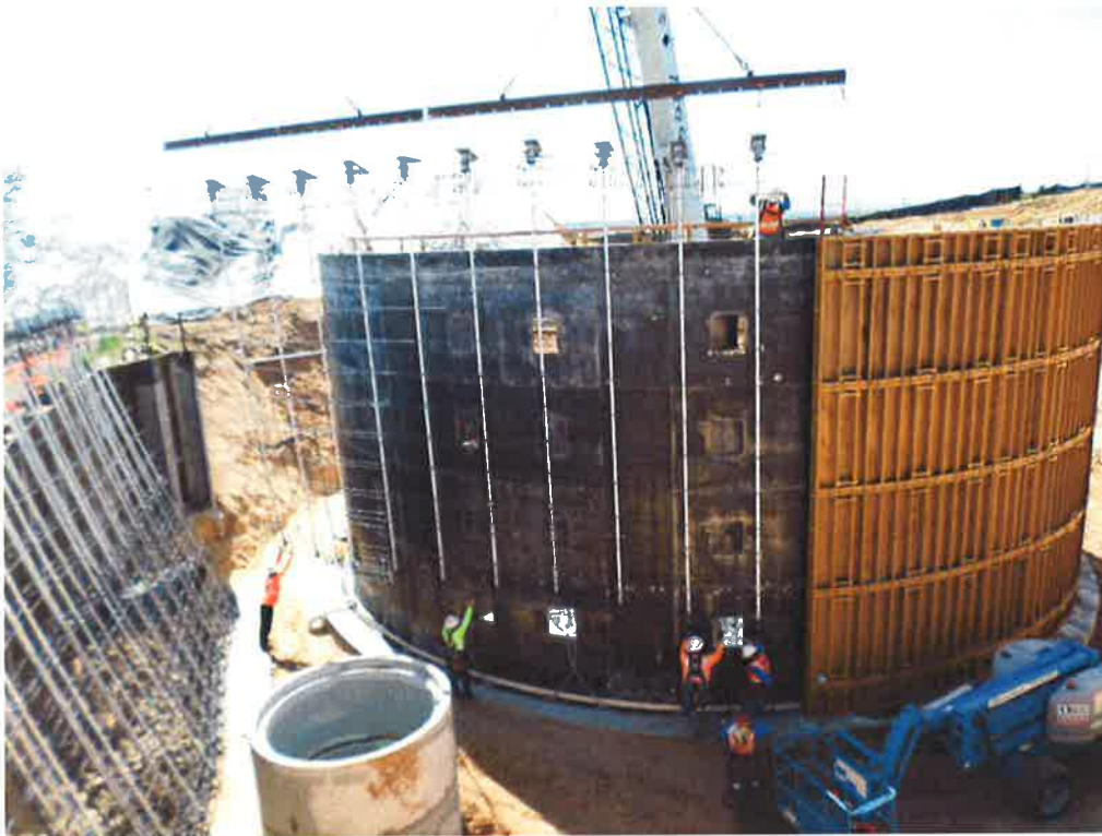
Placing reinforcement for the second wall pour.
