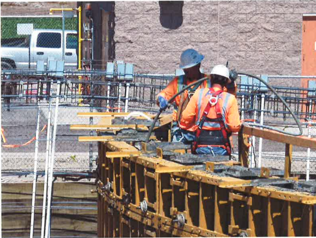
PHC finishing first wall pour, vibrating concrete along the top of the wall.
