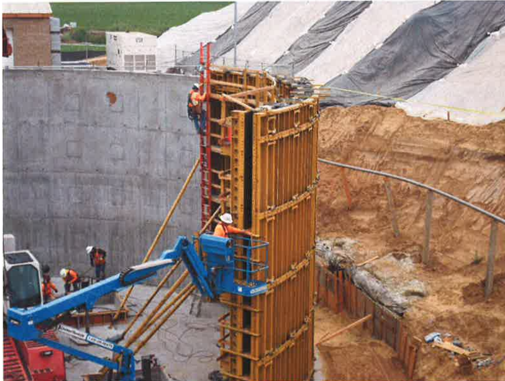
PHC securing the ends of the forms for the fourth wall pour.
