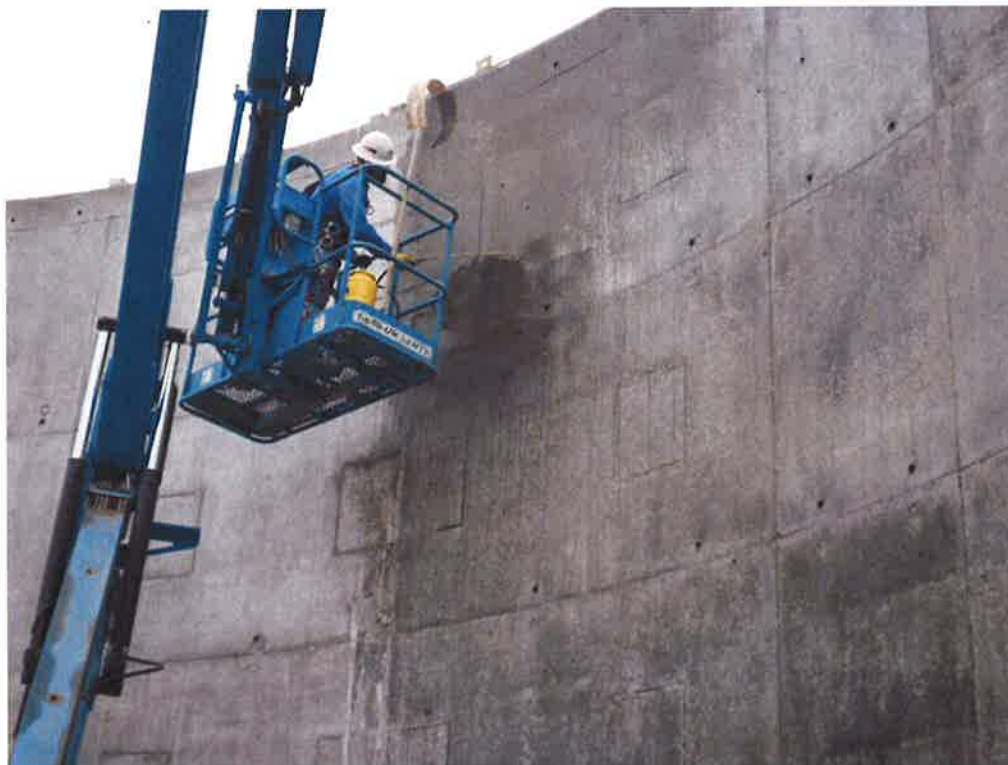
PHC spraying curing compound on second wall pour when forms are removed.
