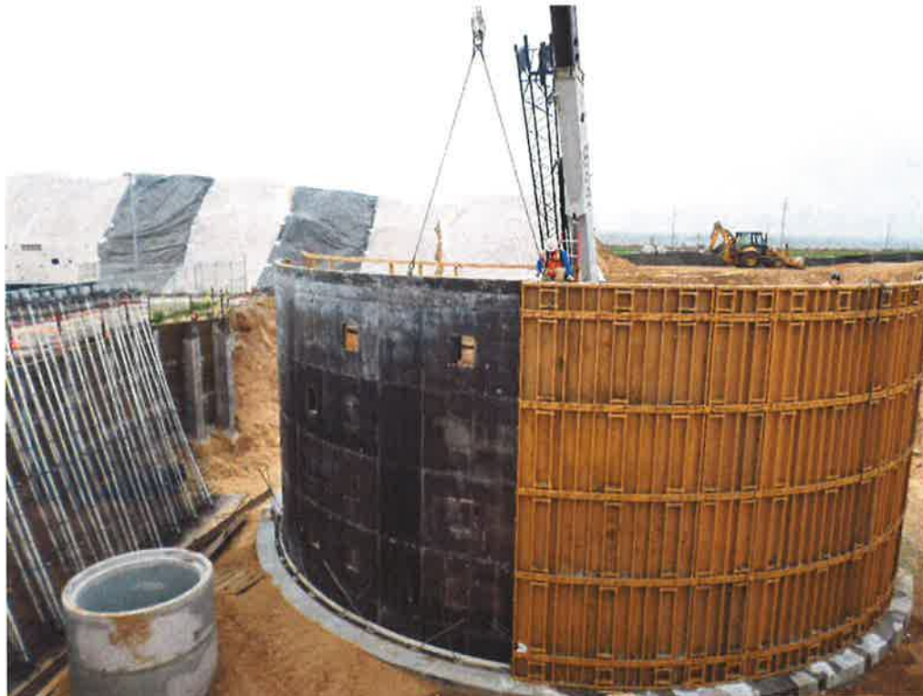
PHC setting interior wall forms for the second wall pour.
