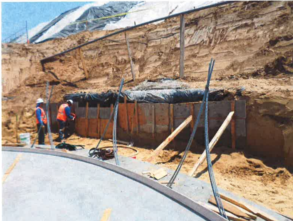
PHC stabilizing material underneath 24-inch inlet pipe.
