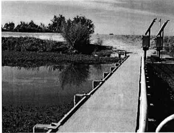
Sack Dam on the San Joaquin River is sinking six inches a year because of subsidence, according to the US Geological Survey. Photo by Amy Quinton/Capital Public Radio, November 2013
