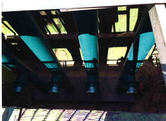
Pump Can Installation - Bottom
