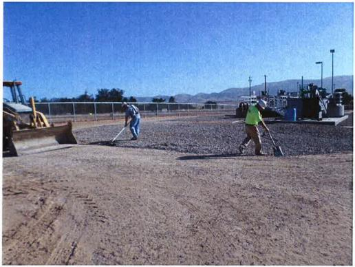
Cushman spreading ¾-inch rock around the Headworks.
