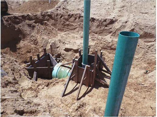
Forming thrust block at cleanout.
