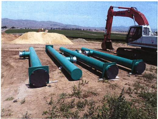
Pump cans delivered to site and coating inspected for thickness and any damage.
