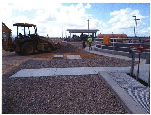
Spreading ¾-inch rock around the clarifiers.
