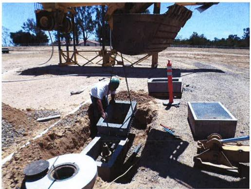
Cushman installing 2-inch meter on the treated water line for the site.
