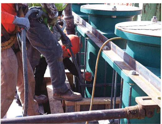
Spiess monitoring and vibrating concrete placement during pour of pump can encasements.
