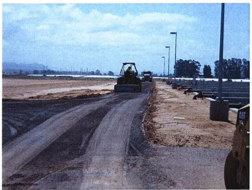
Mark Switzer Excavating completing new site roads with placement of aggregate base.
