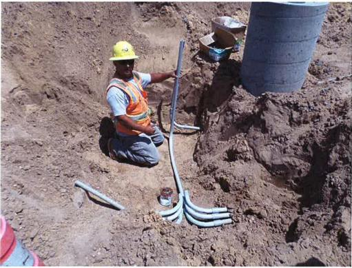
Bergelectric installing conduit to remaining street lights.
