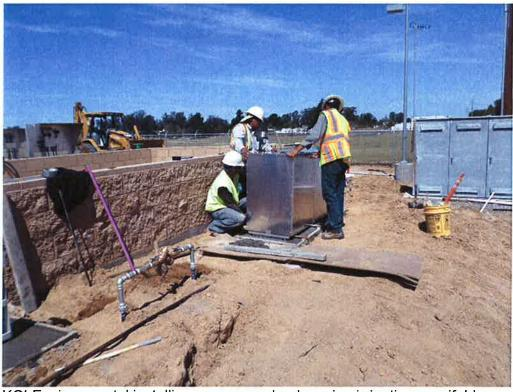
KCI Environmental installing cover over landscaping irrigation manifold.
