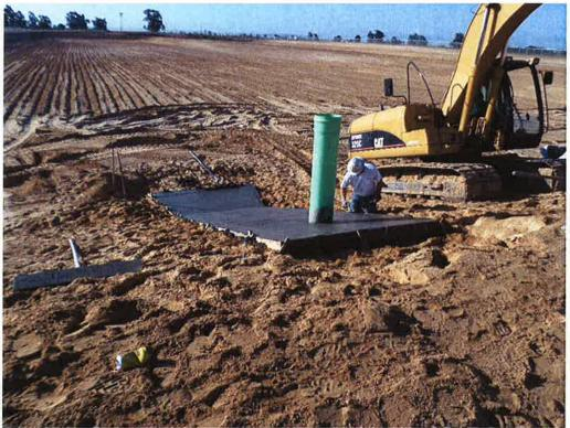
Cushman finishing concrete discharge pads at Ponds 9 & 10.
