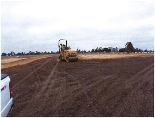
Switzer Excavating compacting aggregate base material for new site roads.
