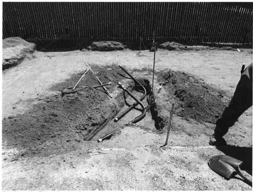
St. Dennis Electric starting underslab conduit installation.
