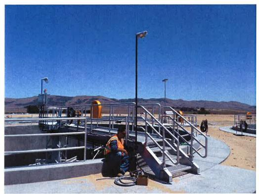
Bergelectric installing lights at clarifier stairs.
