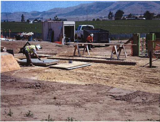
Spiess constructing forms for pump can encasements.
