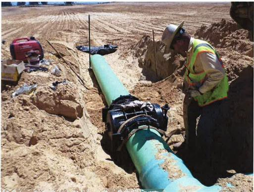
Cushman applying wax tape to bolts on valve of new 18-inch line.
