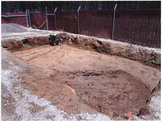
Spiess over excavating and compacting for slab under the chemical building.
