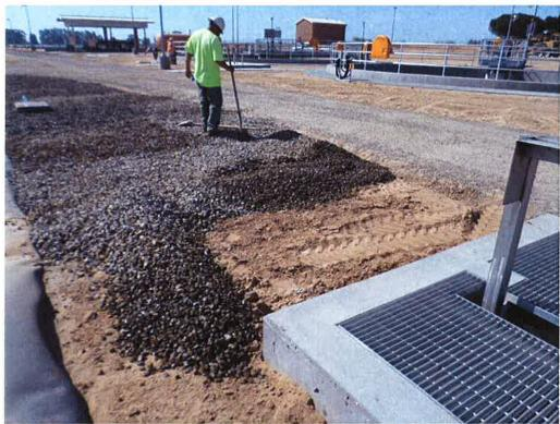
Placing ¾-inch rock around Aeration Basin #1 and the Emergency Holding Basin.
