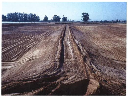
Switzer cutting new road between Ponds 9 & 10 to subgrade.
