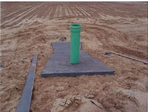
Completed concrete discharge pad after forms are removed.
