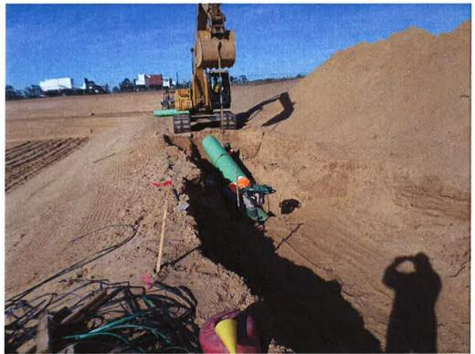
Cushman installing 24-inch SE pipe at new ponds.
