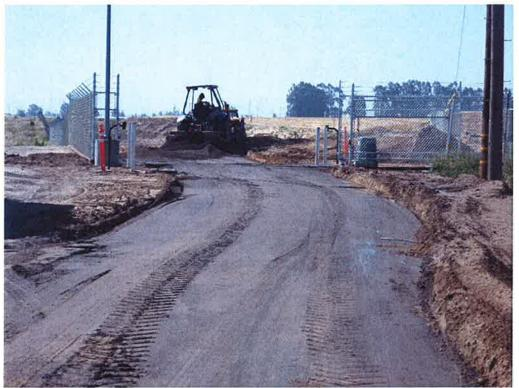
Switzer placing aggregate base for new road at site entry.
