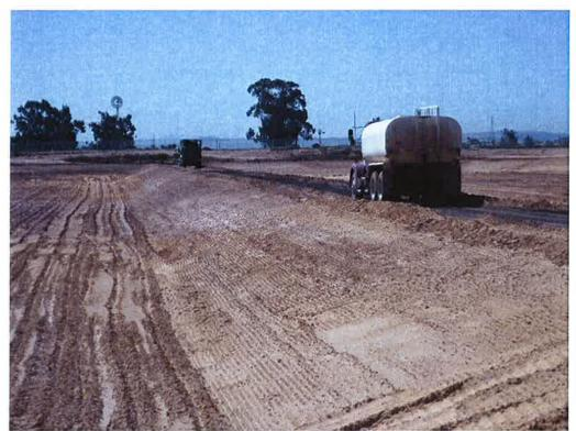
Switzer watering down aggregate base on road between Ponds 9 & 10.
