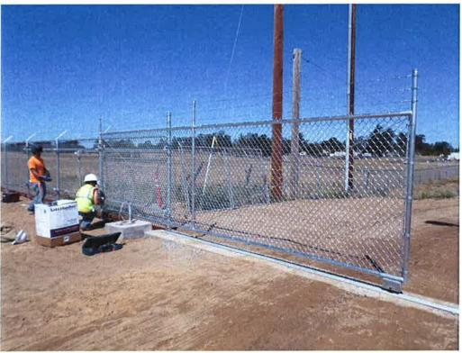
Valley Fencing installing new sliding and automated gate to site entry.
