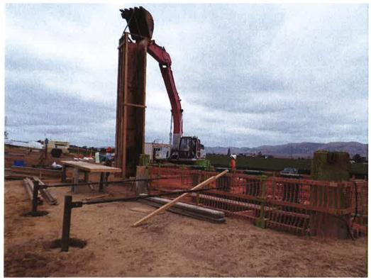
Spiess installing pump can encasement forms.
