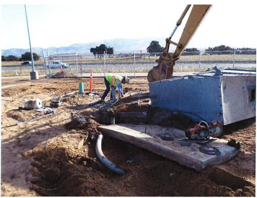
Cushman demolishing existing MCC panel and concrete slab at site entrance.
