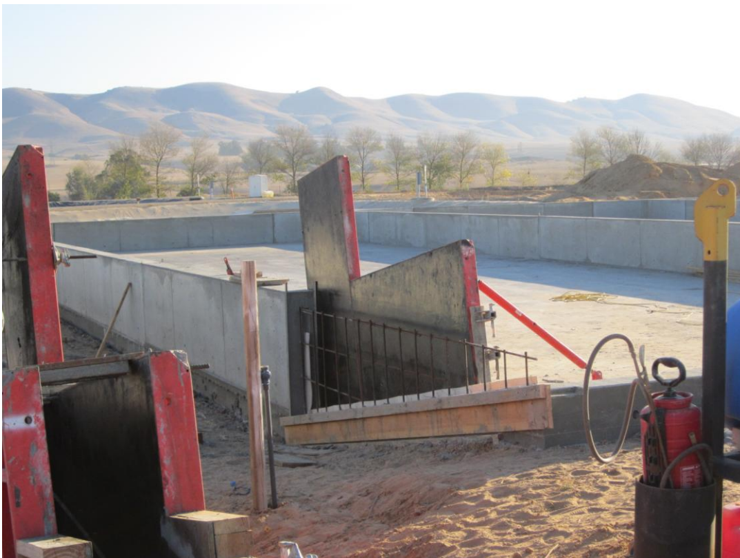
Cushman installing wall forms for ramp walls at Sludge Drying Beds.
