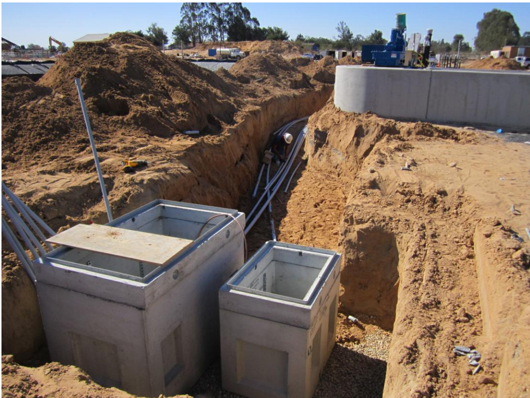
Installing more conduit for DB 02.
