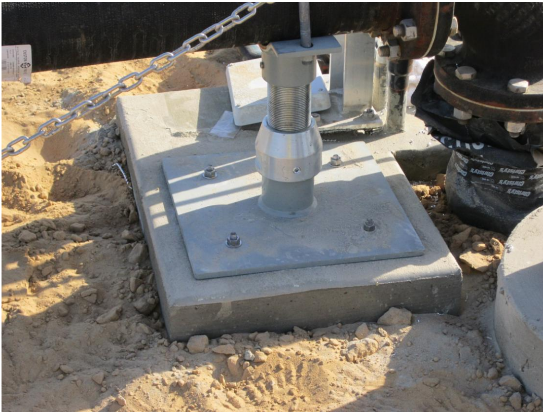
Installing AR pipe supports.
