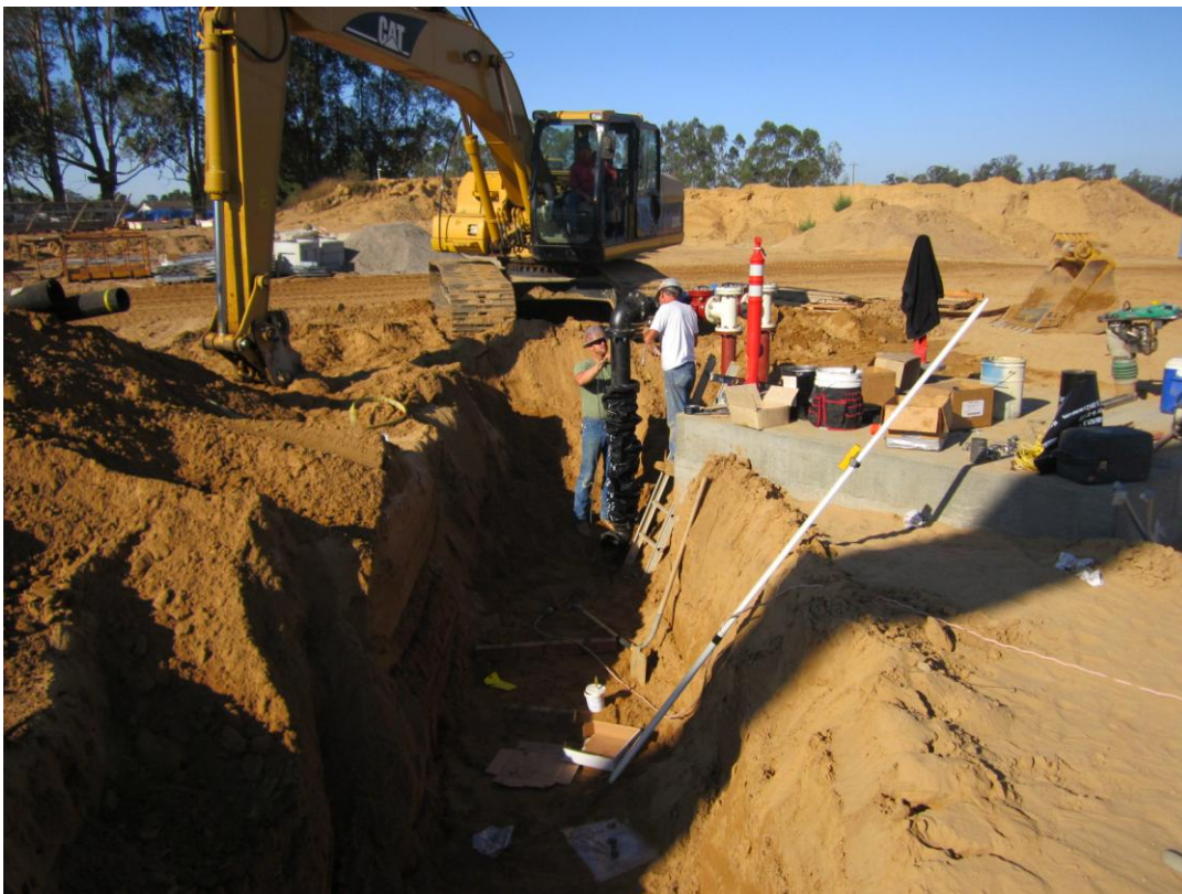
Installing SC piping at the Scum Well Pump Station.
