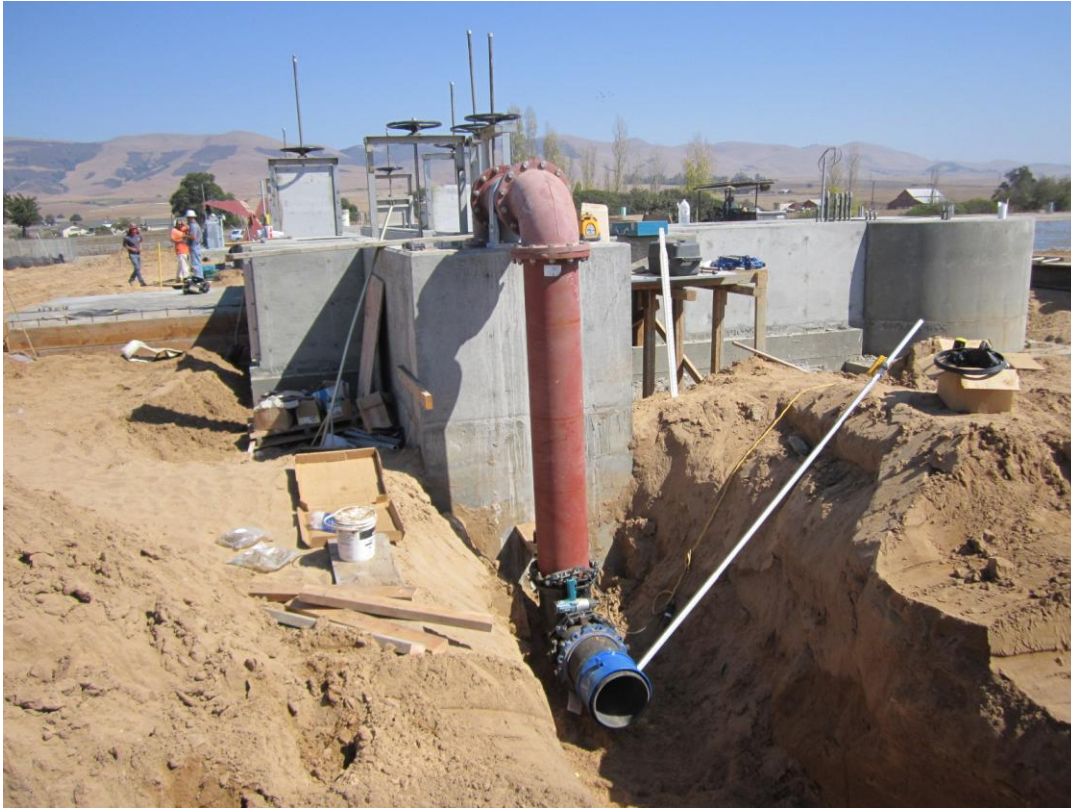
Installing 12-inch RAS piping from the Headworks.
