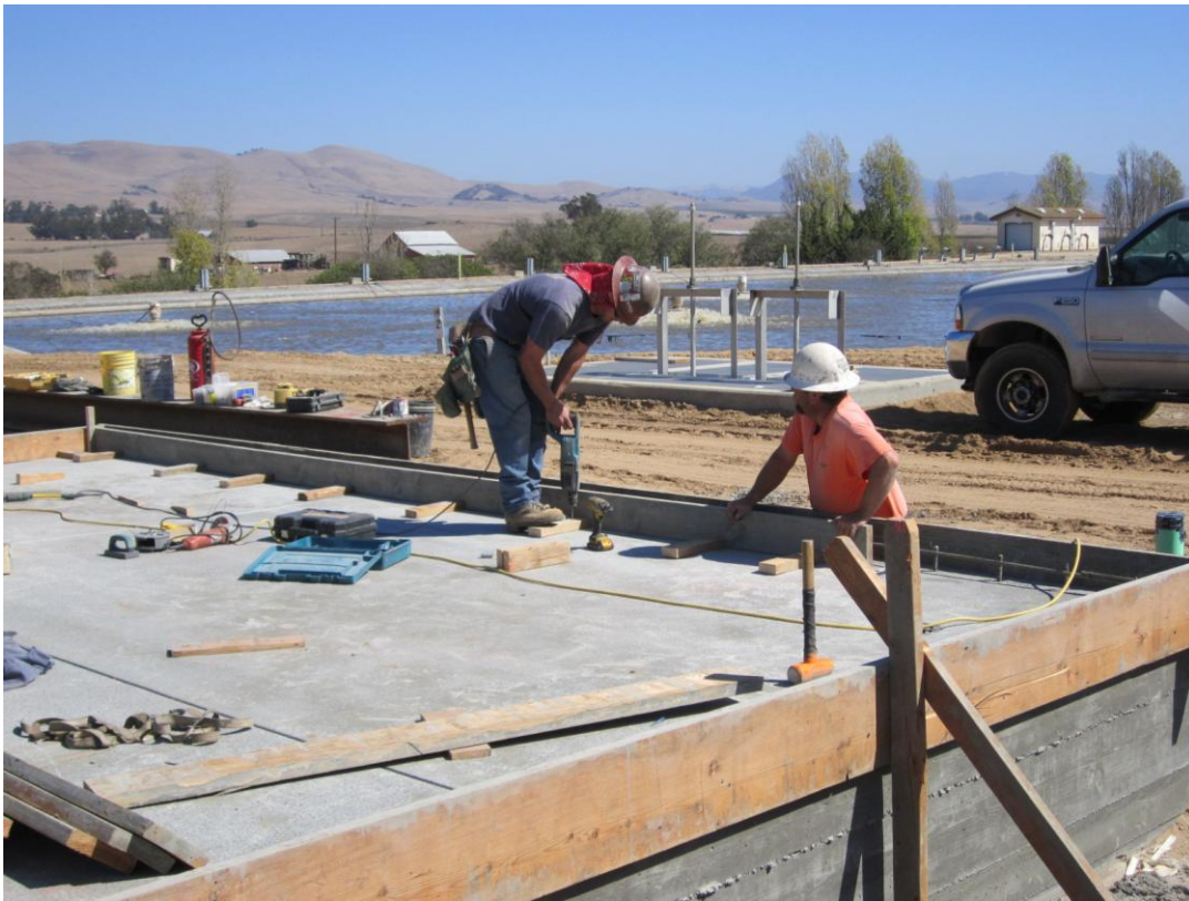
Cushman installing forms for curb at Grit Classifier slab.
