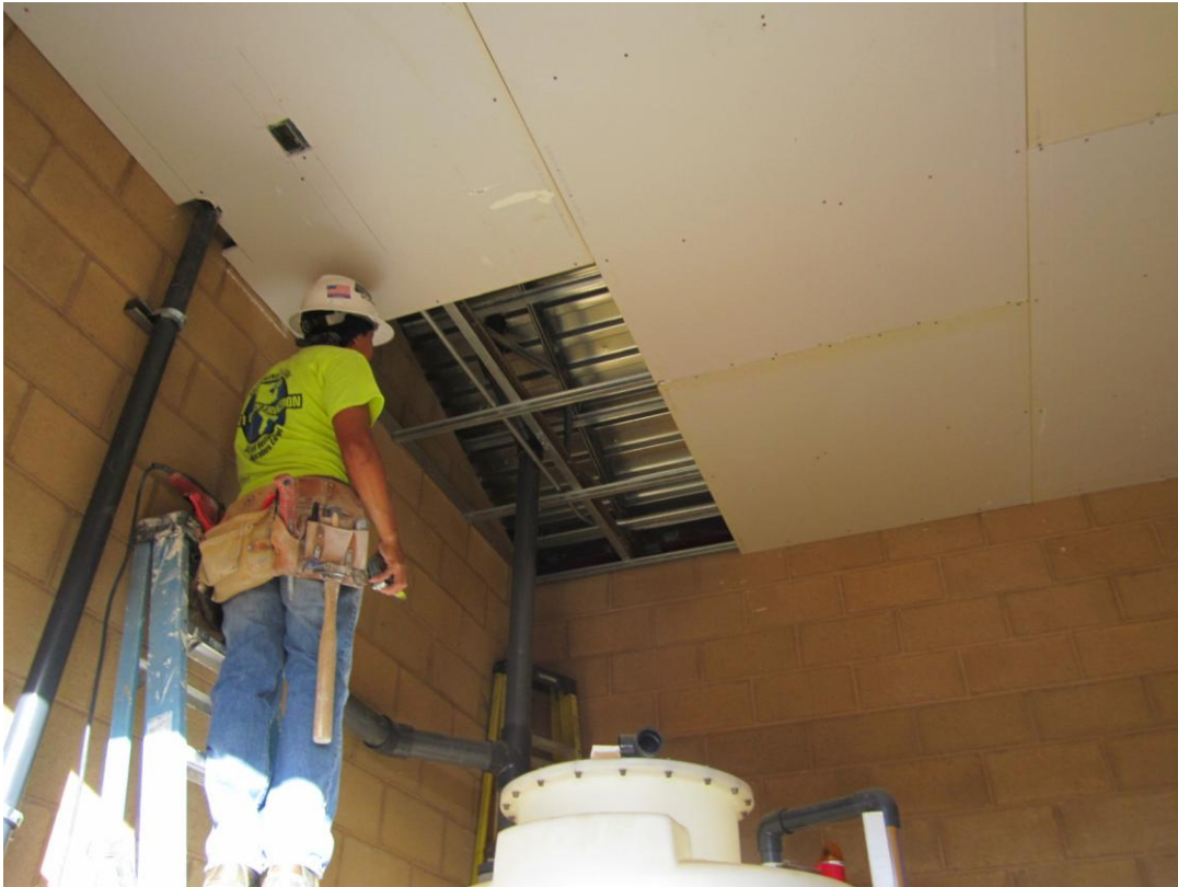
AIT completing installation of drywall inside the Sodium Hypochlorite Storage building.
