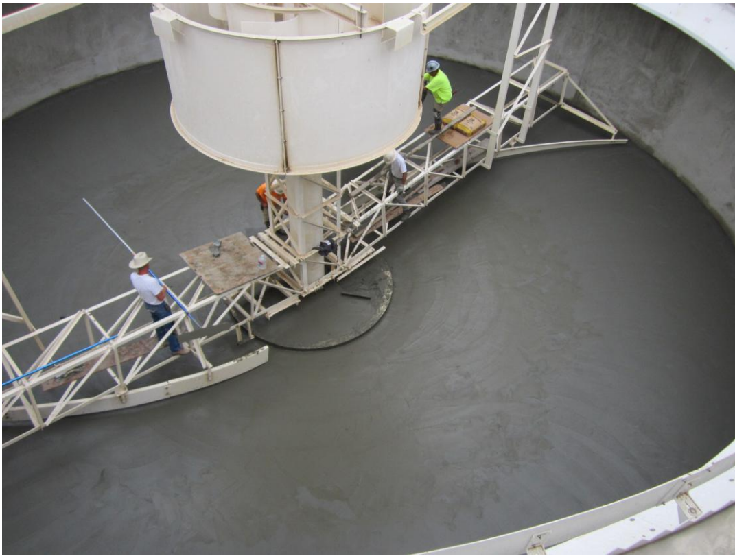
Finishing grouting in Clarifier #1.
