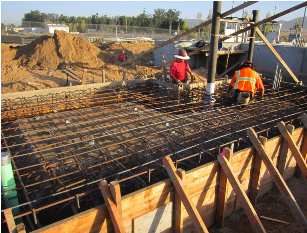
Reinforcing and forms installed for the Grit Classifier slab.
