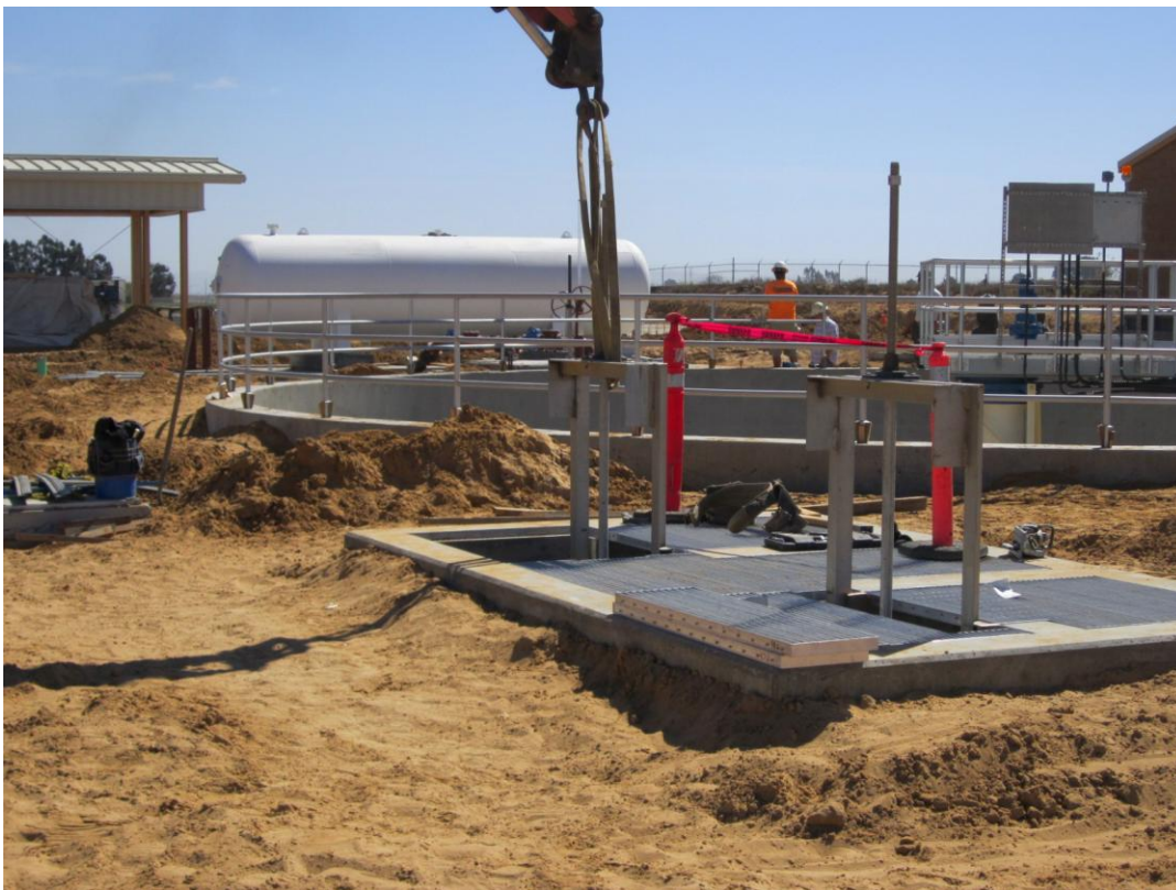
Installing slide gates at Distribution Box #2.
