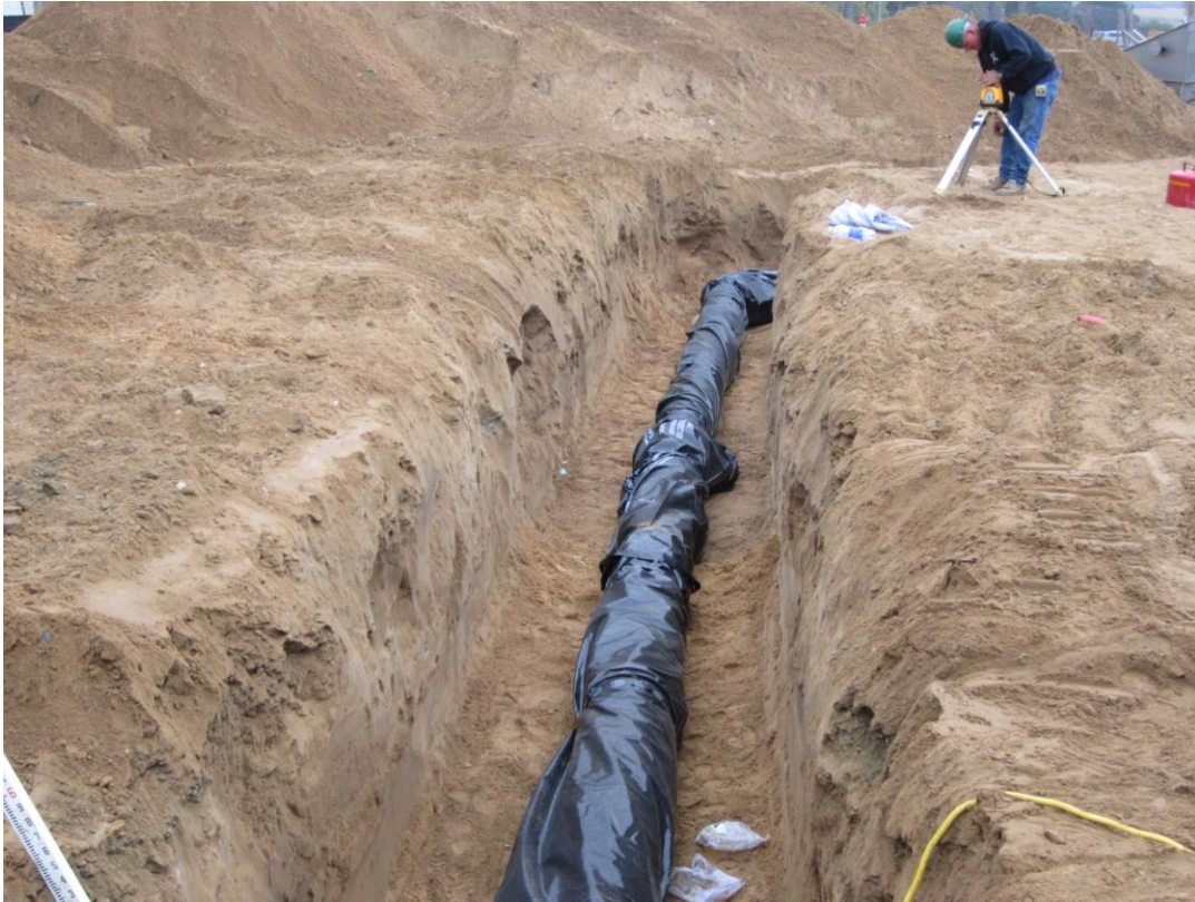
Cushman installing 12-inch RAS piping from the Headworks.
