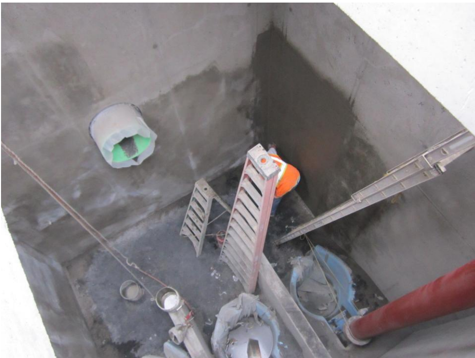
KNK Coating applying non-shrink grout to the inside of the Influent Pump Station in preparation for applying the Carboline coating.
