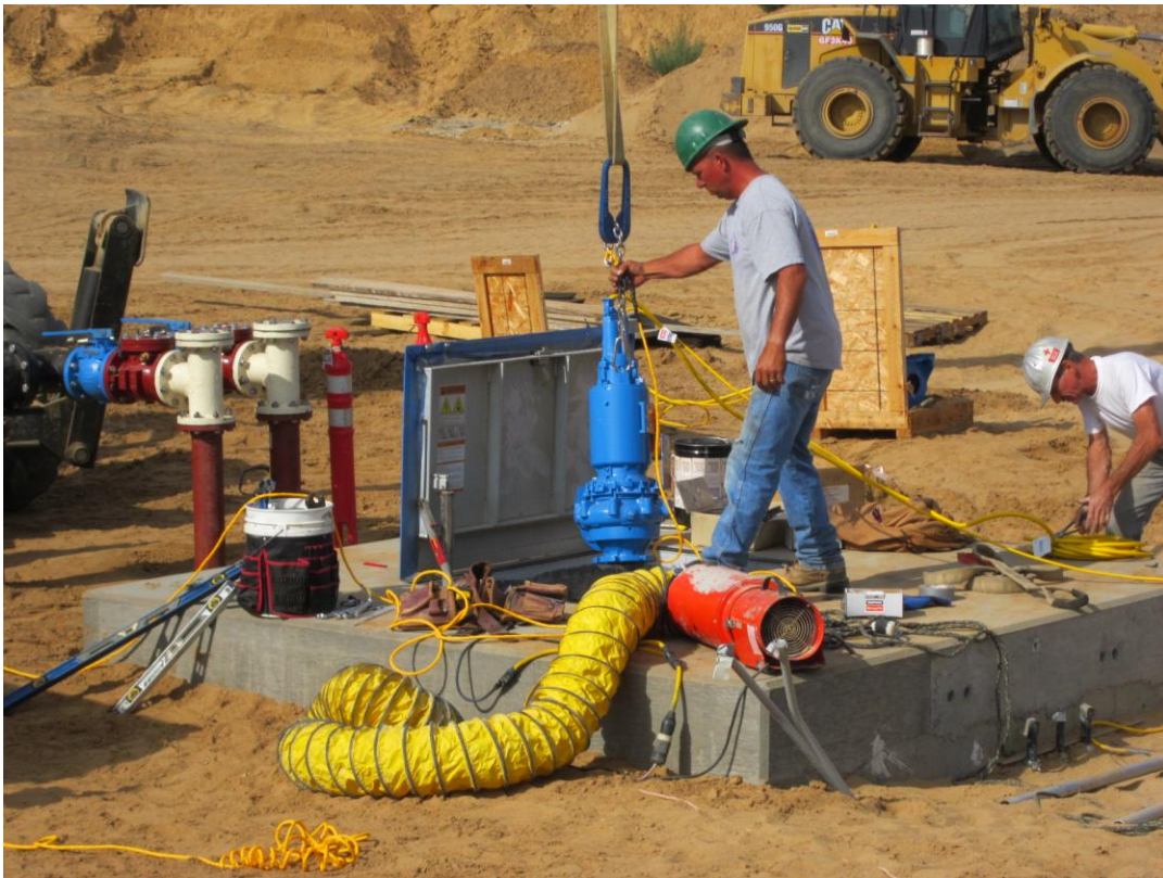
Cushman installing the pump inside the Scum Well.
