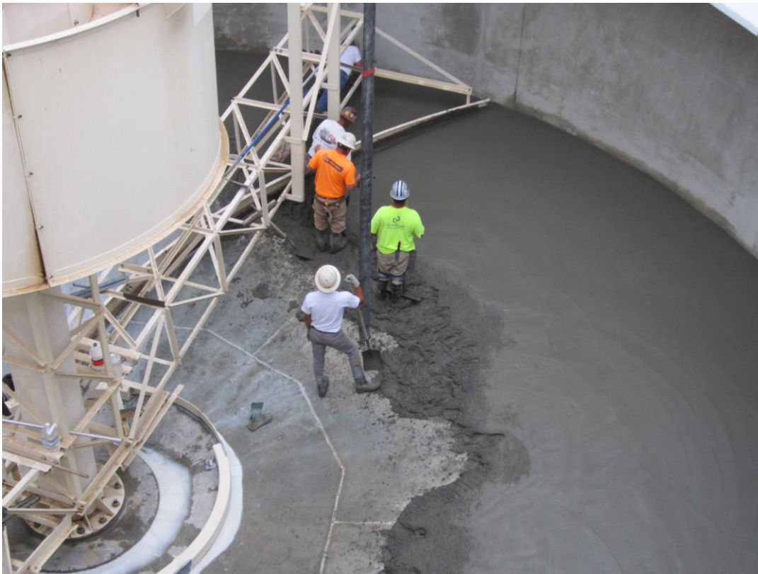
Cushman spreading grout in Clarifier #1.
