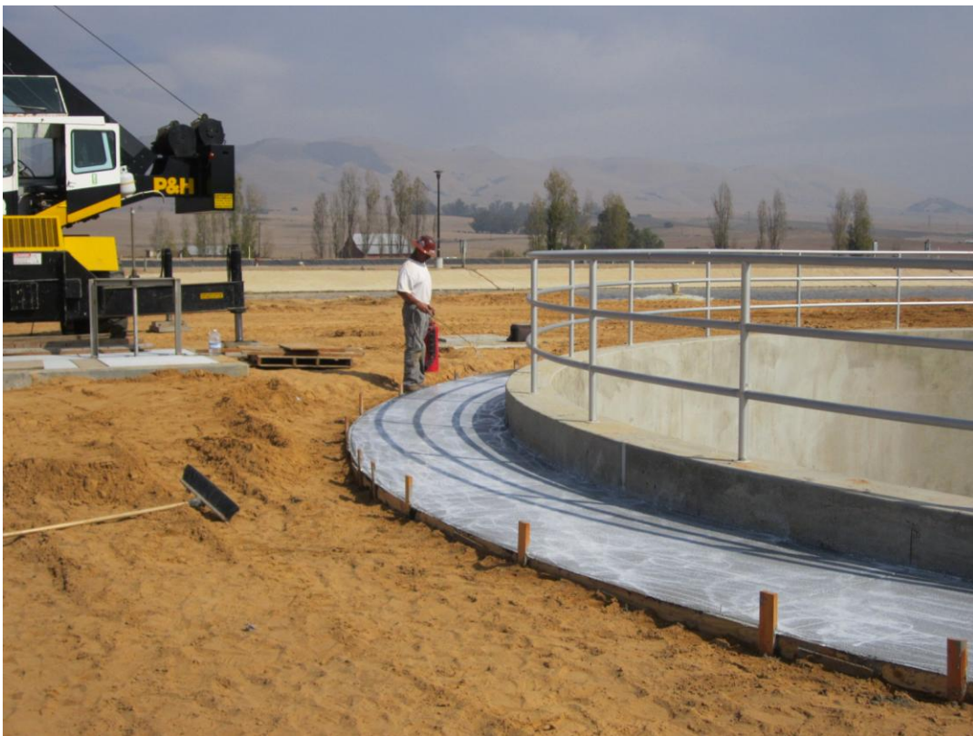
Cushman spraying curing compound on sidewalk around Clarifier #1.
