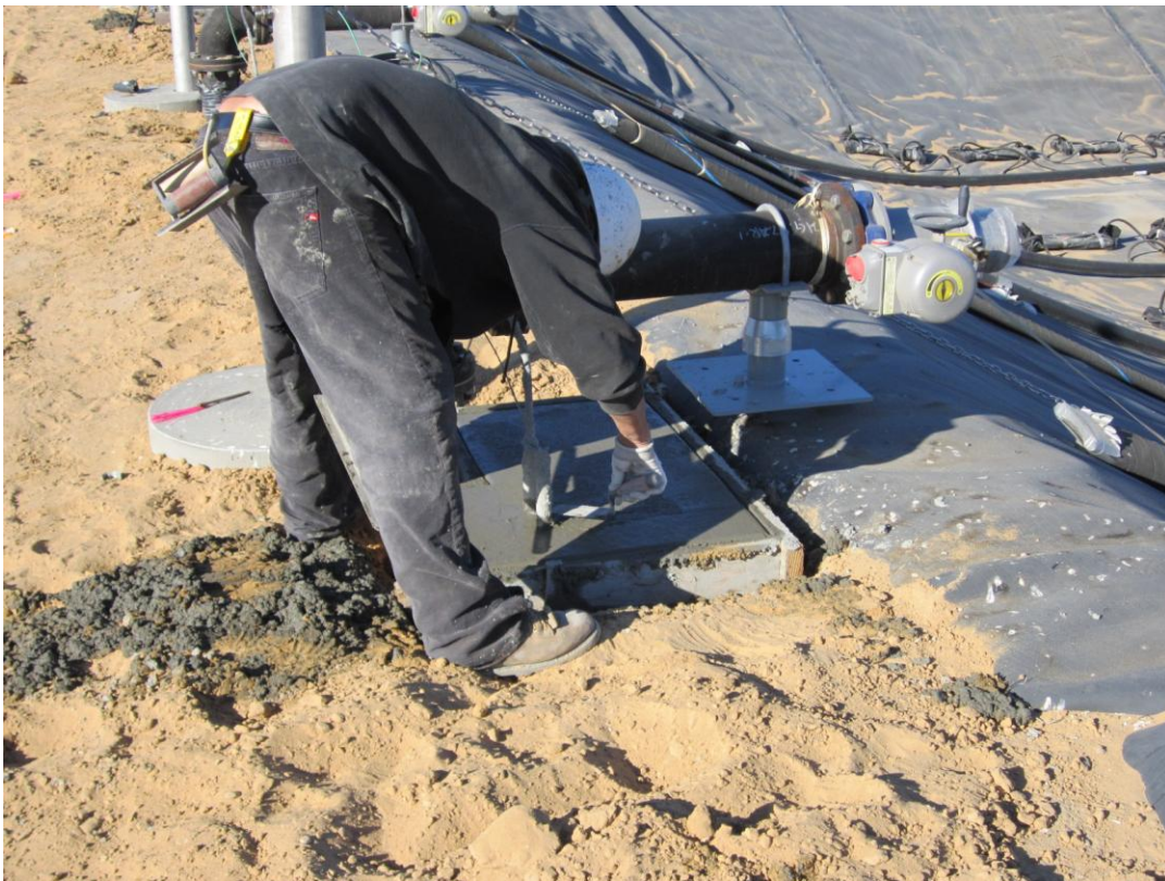
Cushman pouring pipe support pads for AR piping at the Aeration Basin.
