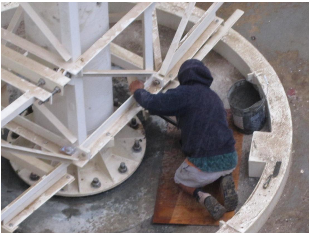
Cushman grouting center column of clarifiers.
