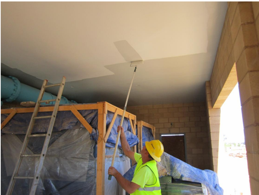
KNK Coating finishing painting of the ceiling in the blower room.
