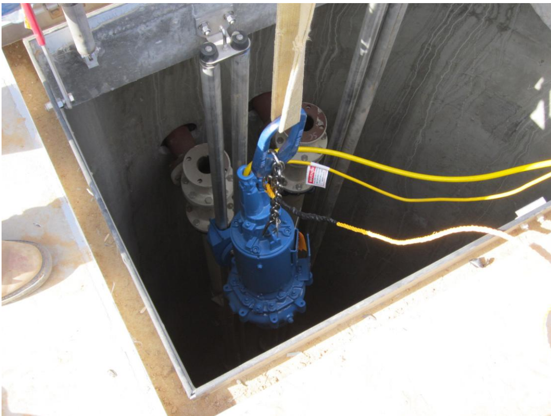
Pump and guide rails being installed inside the Scum Well.
