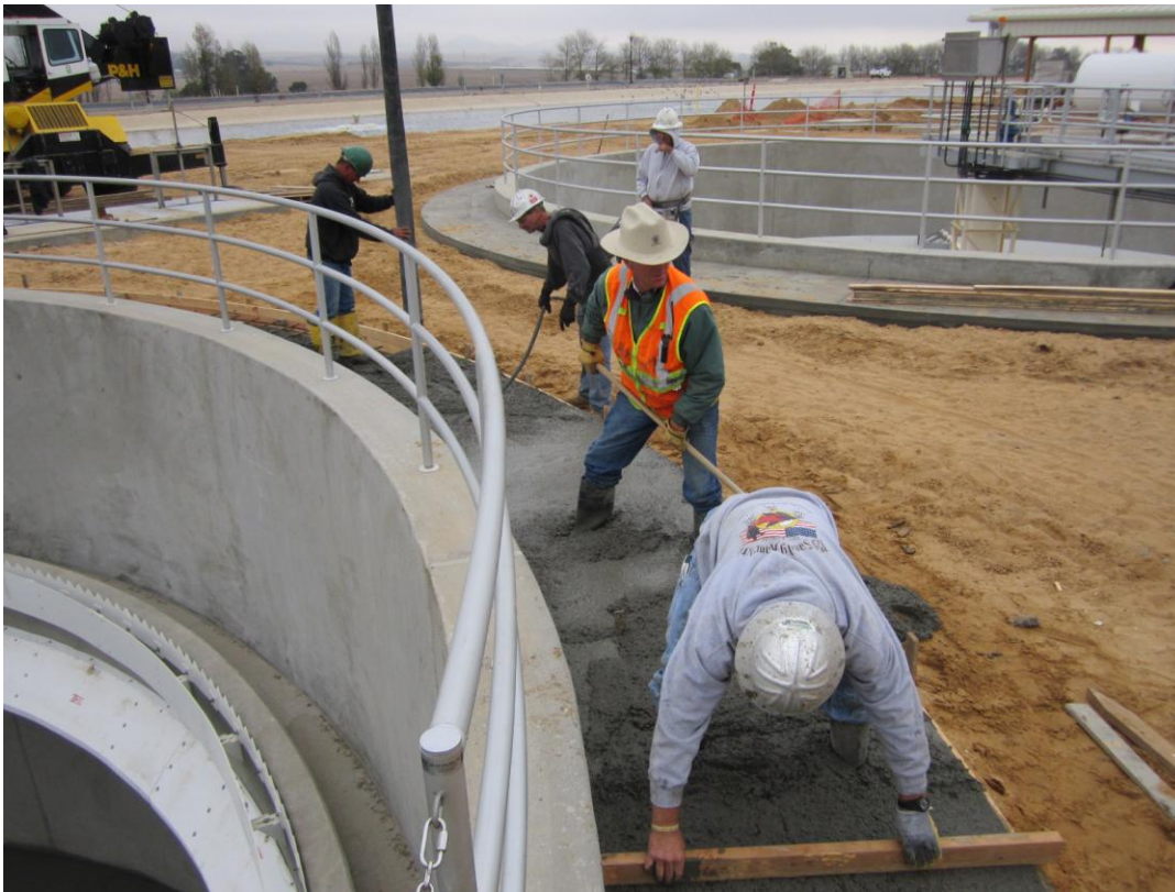
Cushman pouring concrete sidewalk around Clarifier #2.
