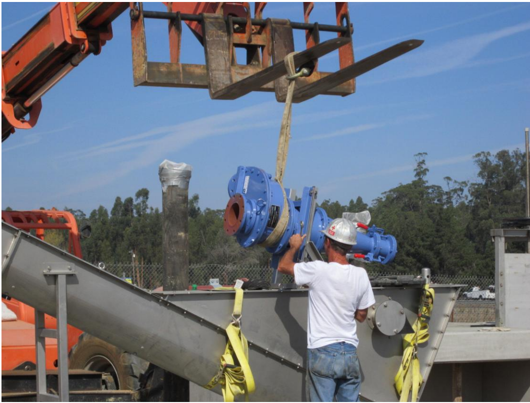
Installing Grit Classifier motor.
