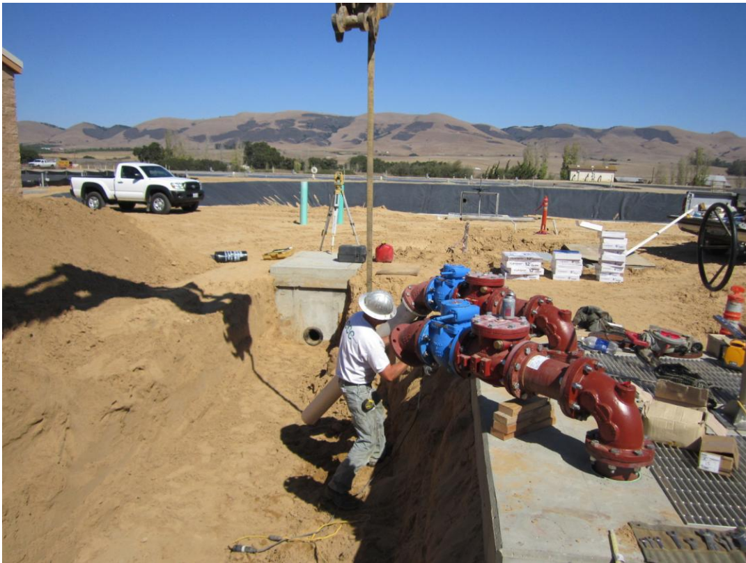
Cushman installing valves and piping at RAS/WAS Pump Station #1.
