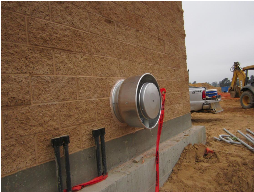
Exhaust fan installed by Long's Construction at Sodium Hypochlorite Storage building.
