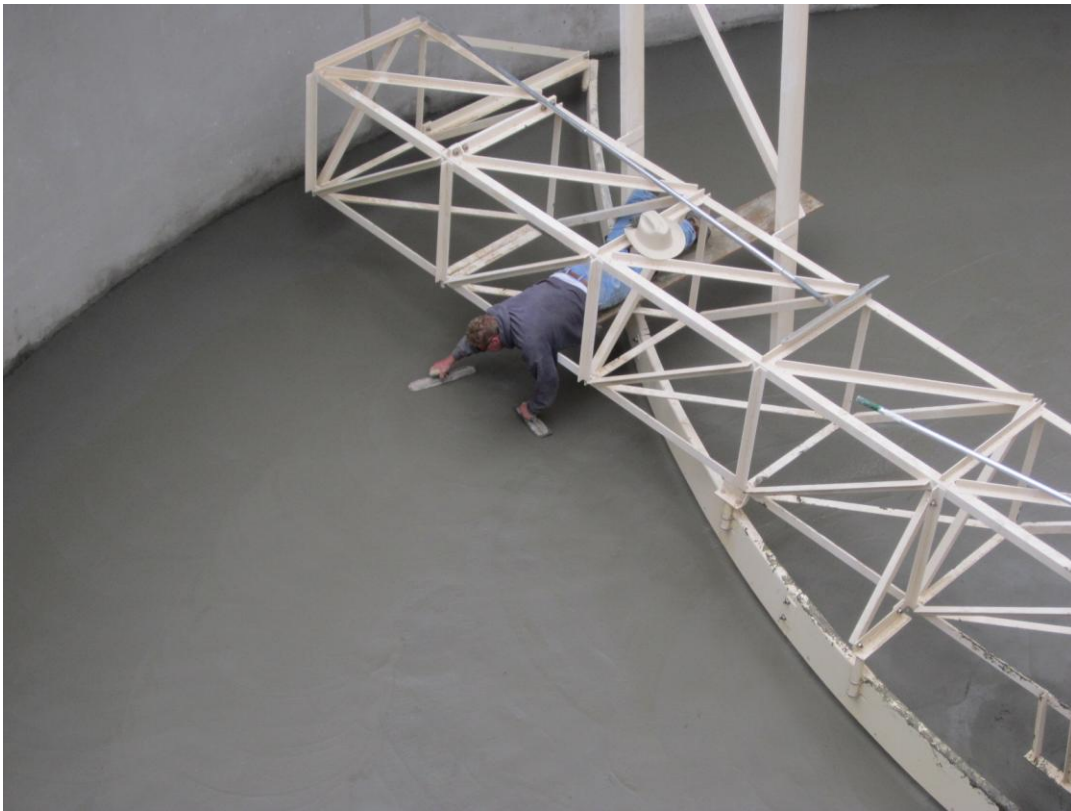
Cushman finishing grout pour in bottom of Clarifier #2.
