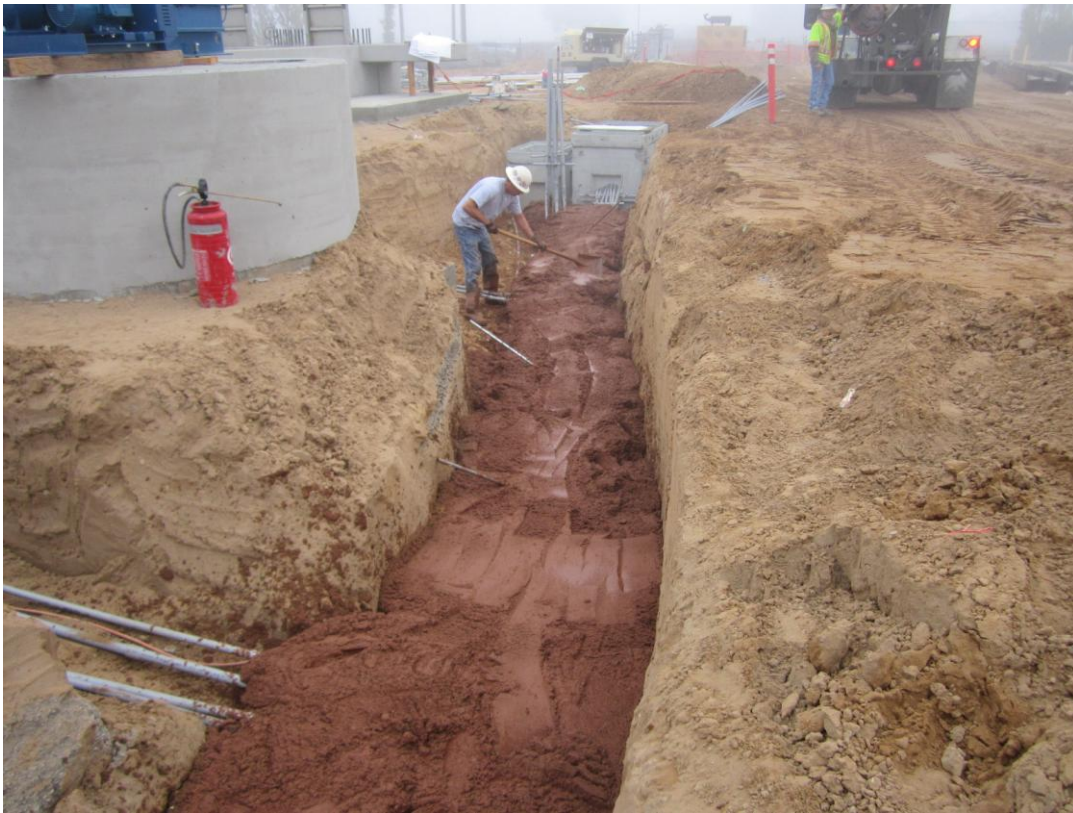
Bergelectric placing red slurry over DB 02.
