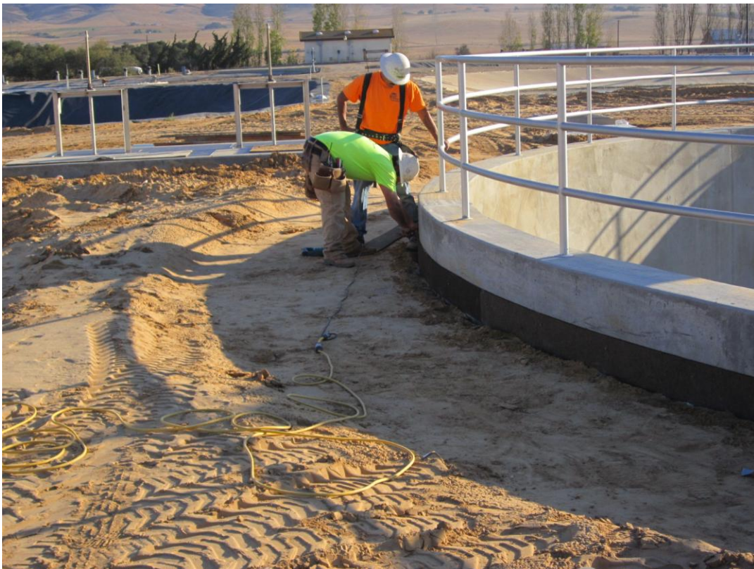
Cushman installing expansion material around Clarifier # 1.
