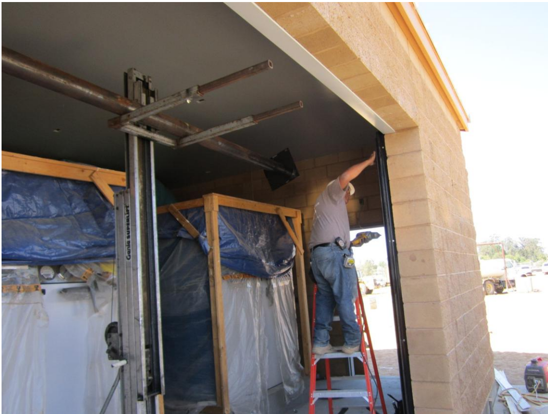
Hamon Overhead Doors installing roll-up door to blower room.
