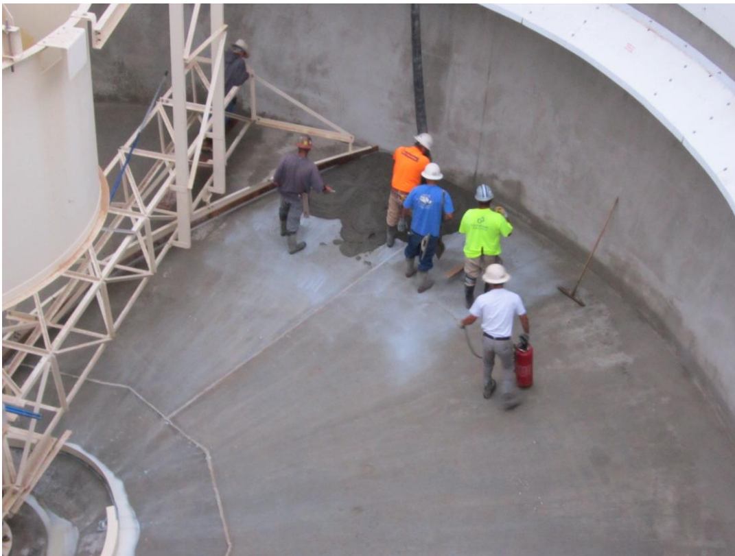
Cushman beginning grouting of Clarifier #1.
