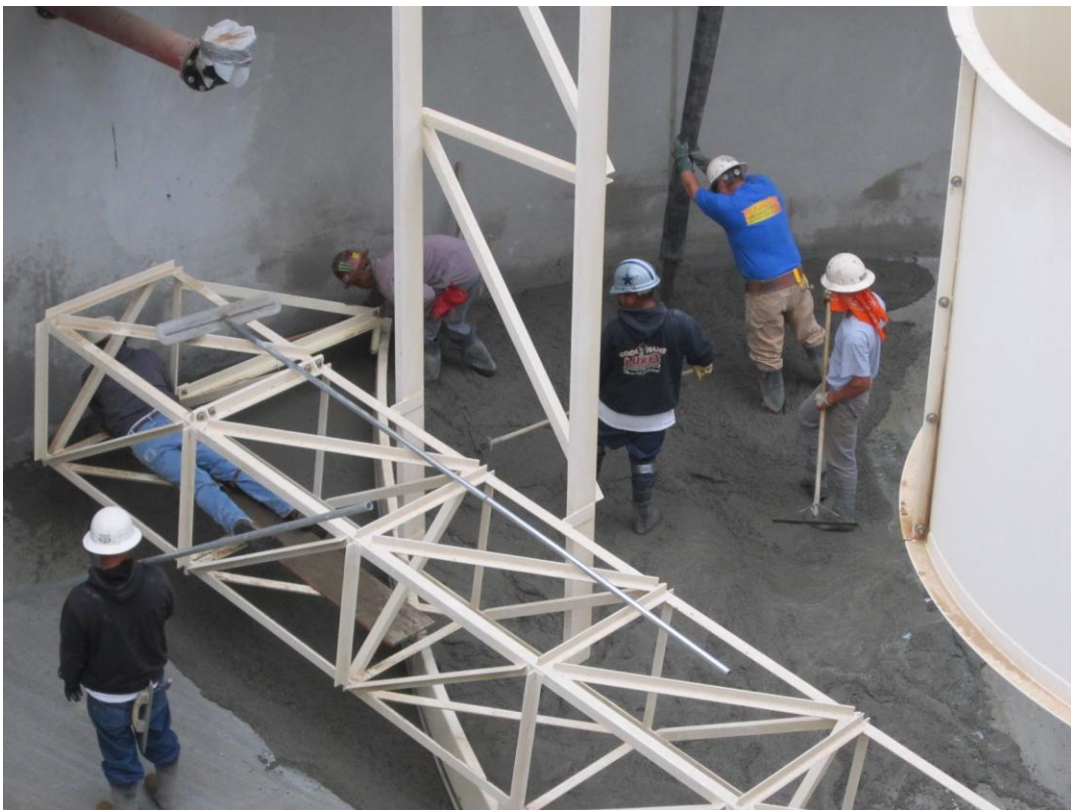
Cushman grouting Clarifier #2.
