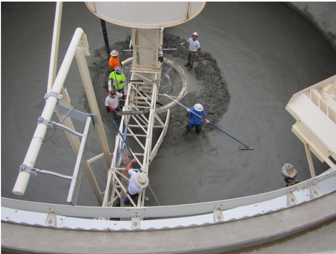
Cushman finishing grout in Clarifier #1.
