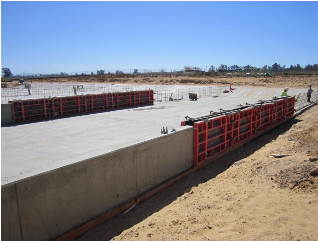
Cushman installing wall forms at Sludge Drying Beds for continued pours.
