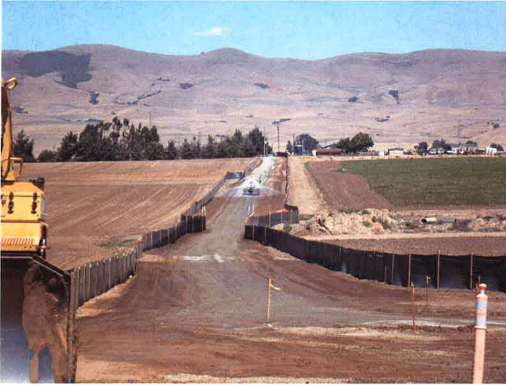
View from future pump station site of temporary access road and silt fence installed.
