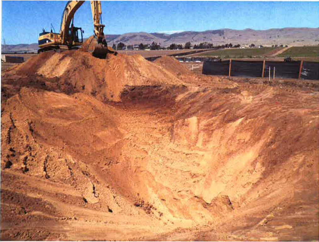
ARB excavating to install the 54-inch diameter casing.
