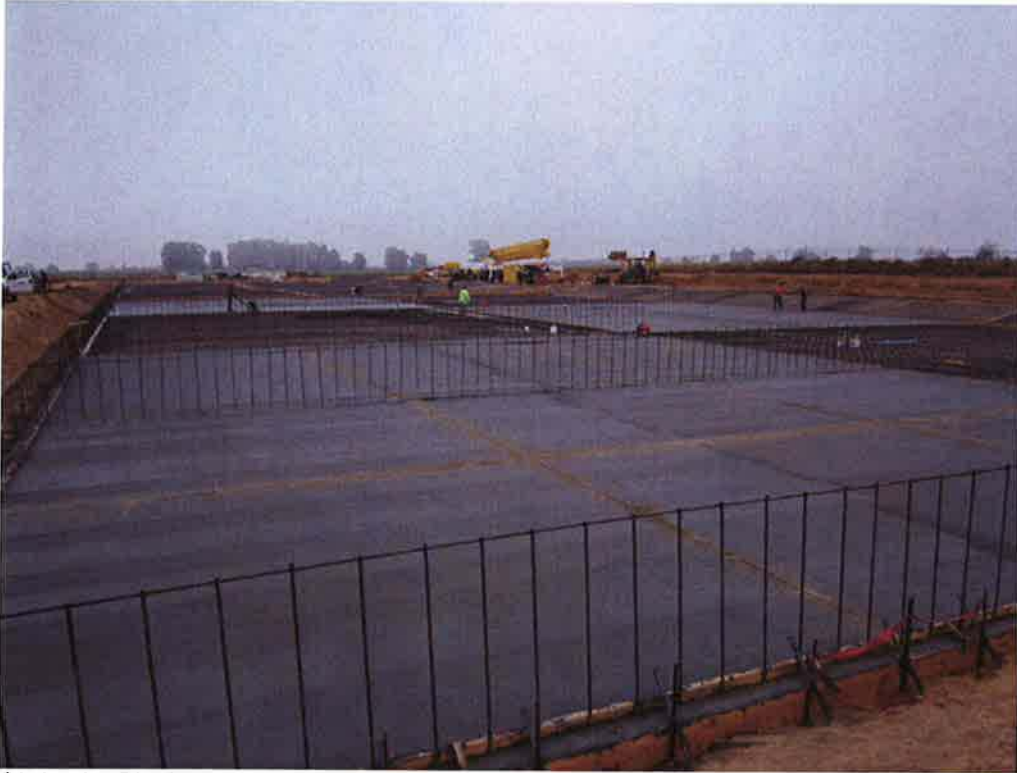
Slabs in Sludge Drying Bed #1 curing after first concrete pour.
