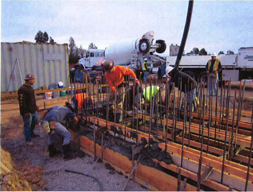
Cushman pouring concrete for slab at Headworks Screening System.
