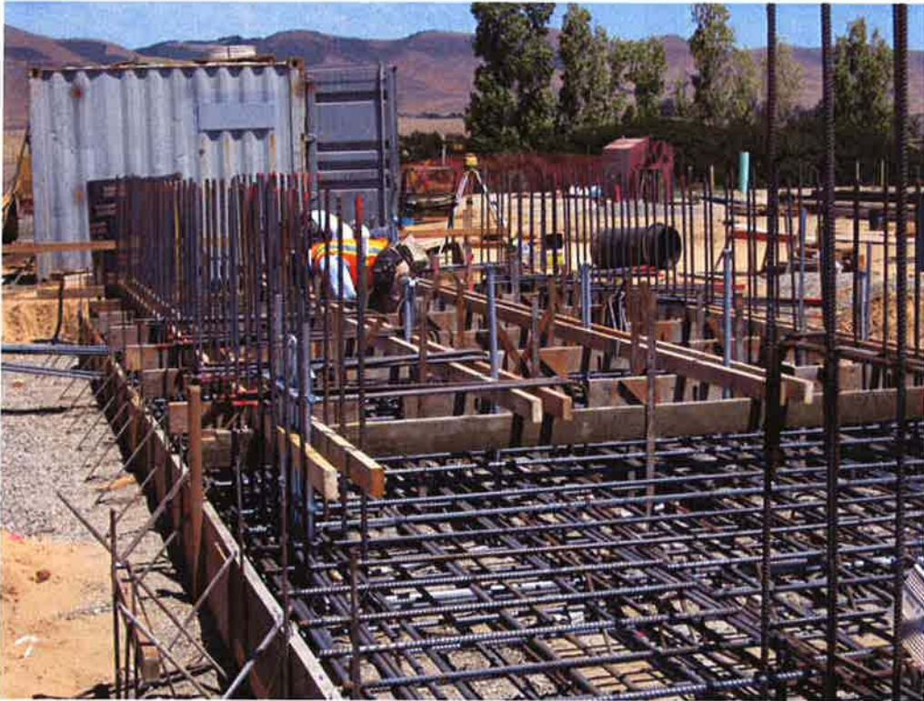
Forming starter walls at Headworks Screening System.
