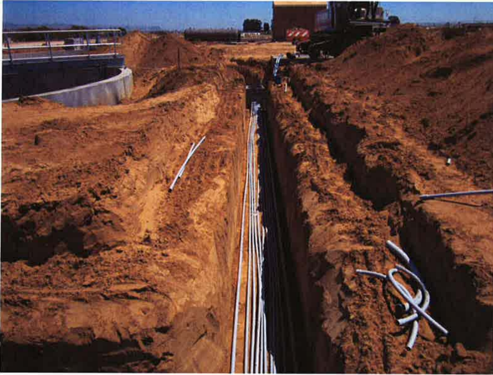
Bergelectric installing Duct Bank 24 (DB-24).
