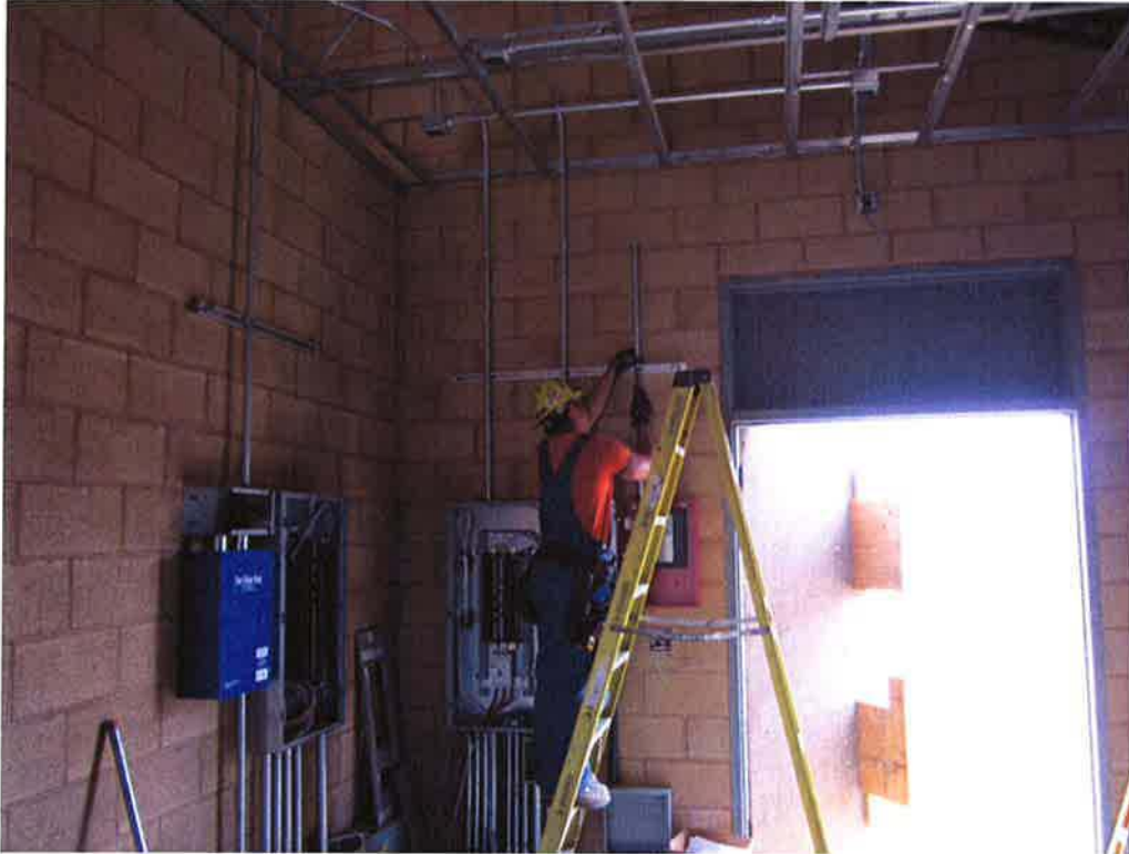
Bergelectric installing fire alarm panel inside the MCC room.
