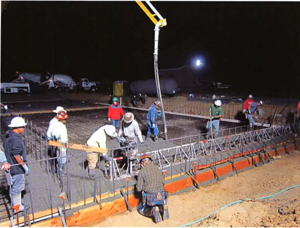
Cushman pouring first slab section of Drying Bed #1.
