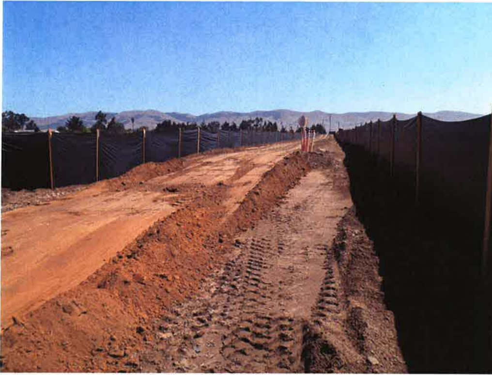
Building up road to protect existing Phillips 66 oil line.
