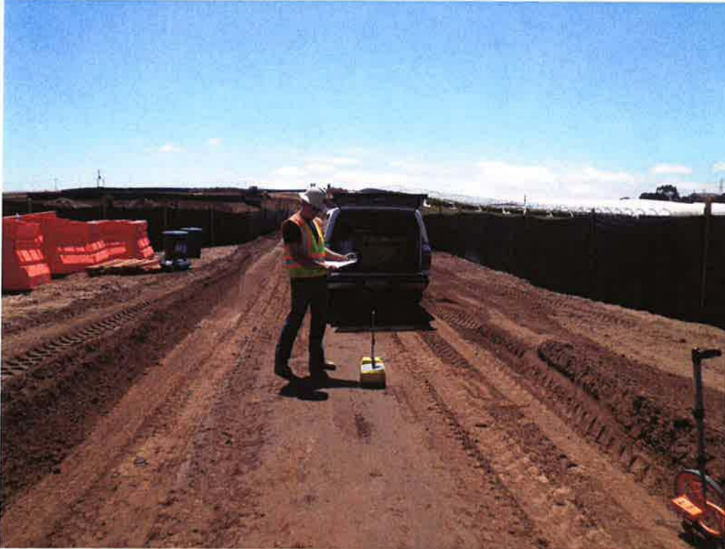
Fugro taking compaction tests for the base under the temporary access road.
