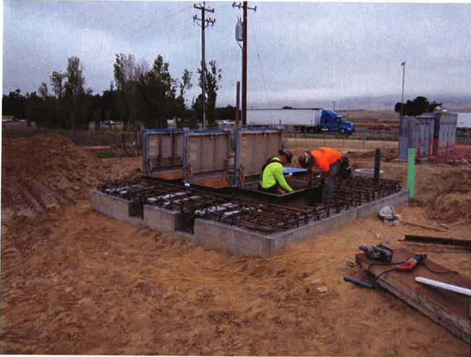
Cushman forming Influent Pump Station deck.
