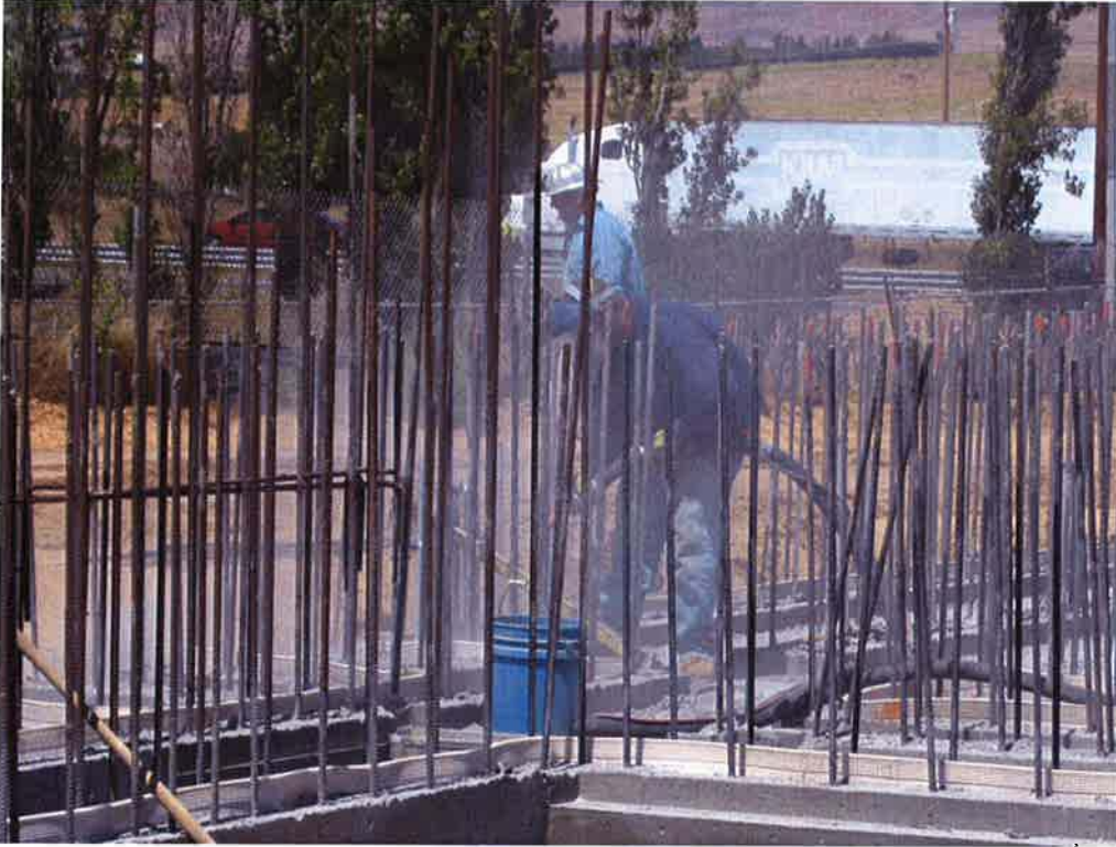
Cushman sand blasting base of starter walls in preparation for forming interior walls of the Headworks Screening System.
