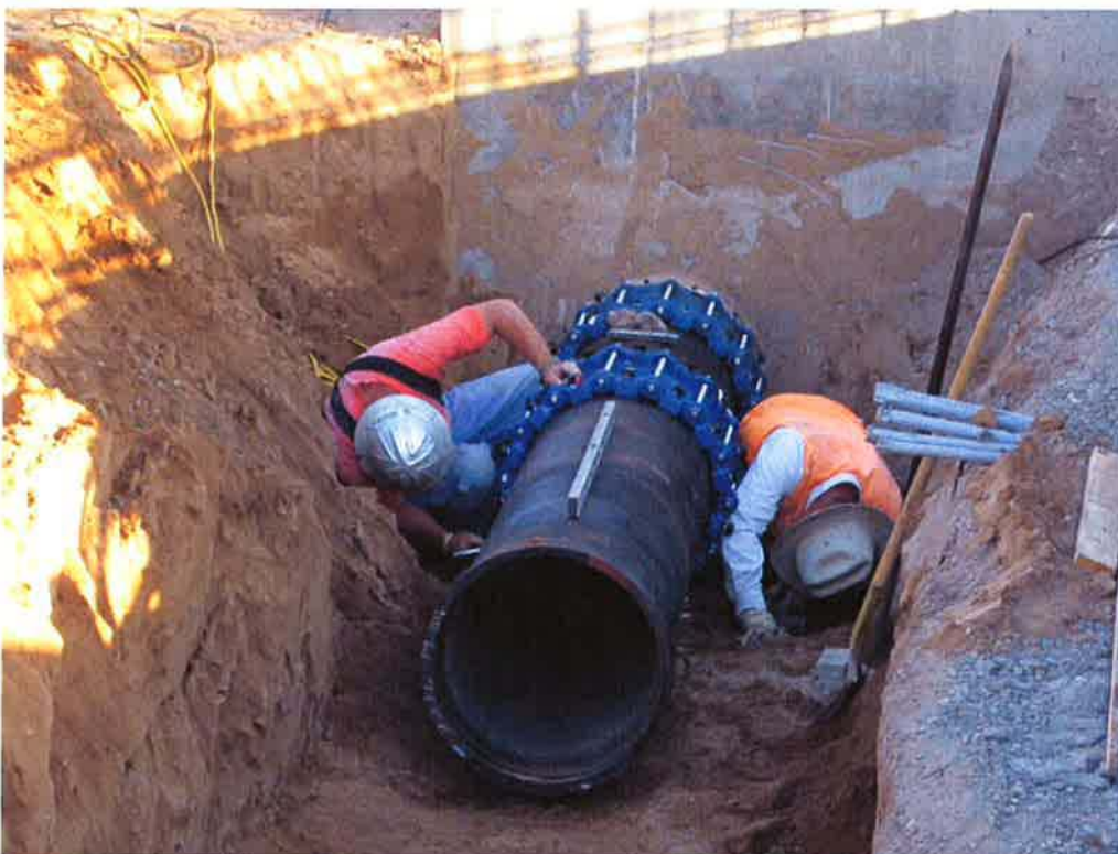
Cushman installing 20-inch SI pipe from Headworks to Distribution Box #1.
