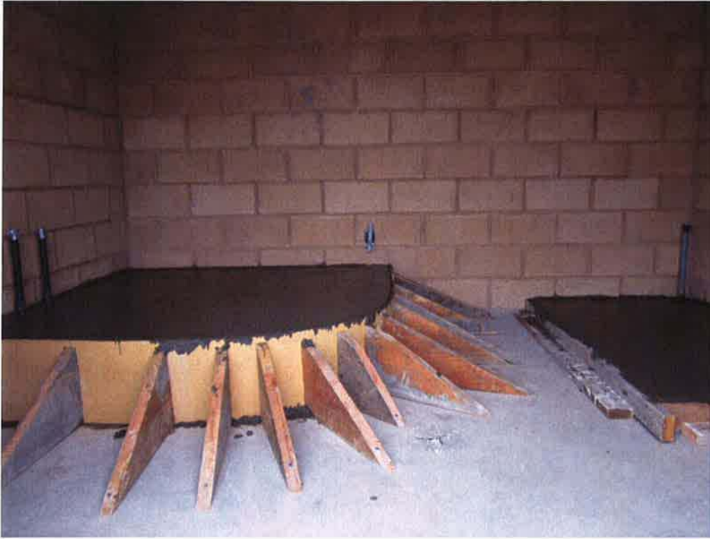
Pouring equipment slabs inside Sodium Hypochlorite Building.
