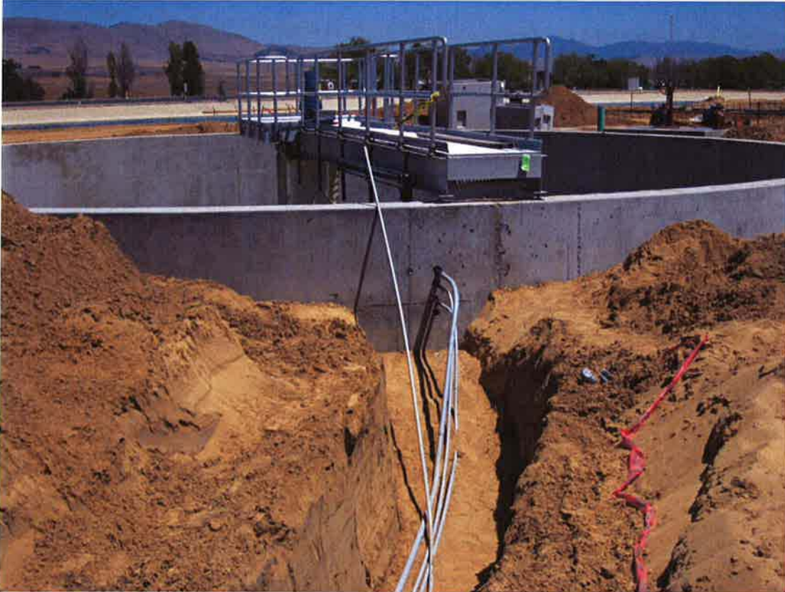
Conduit being installed to Clarifier #1.
