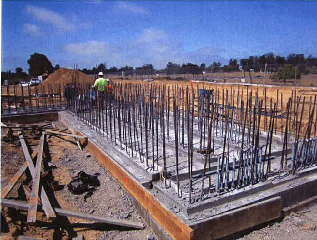
Stripping forms from slab pour at Headworks Screening System.
