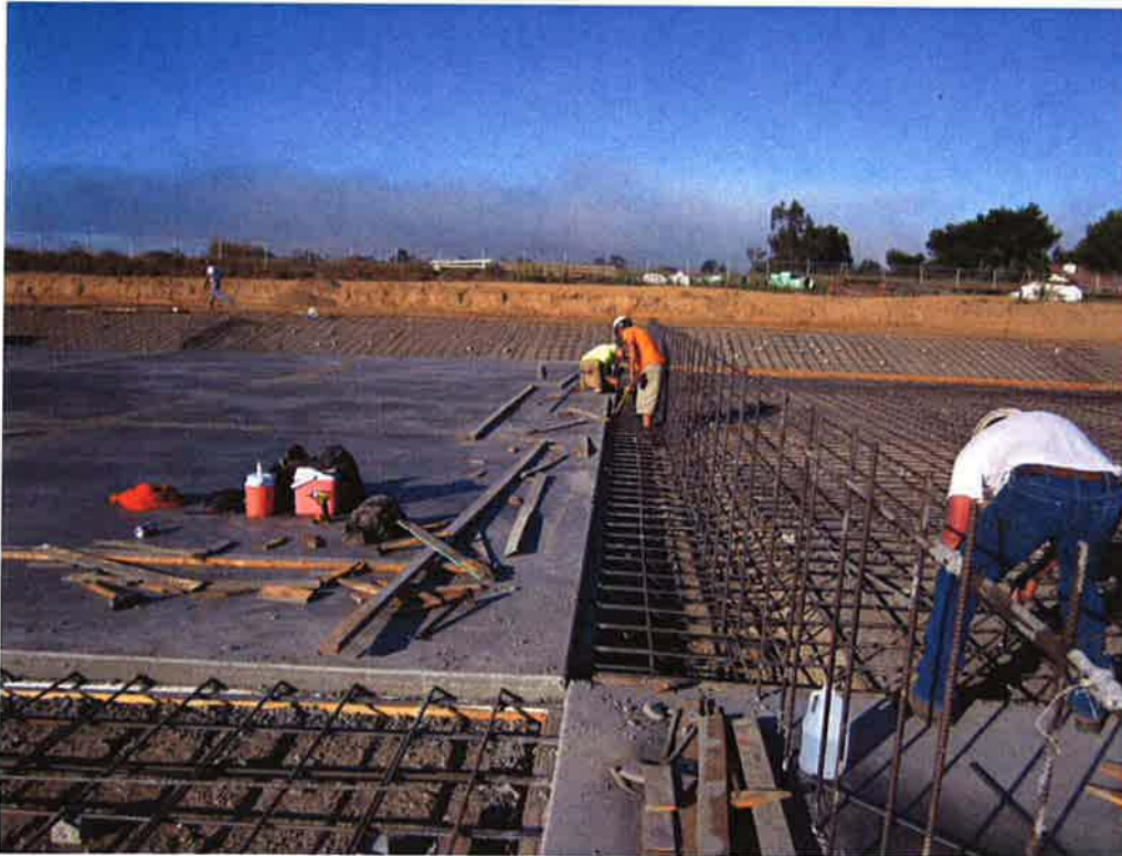
Cushman stripping forms after night pours at Sludge Drying Beds.
