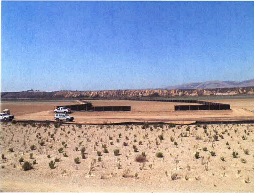
Silt fence installed on south side of project.
