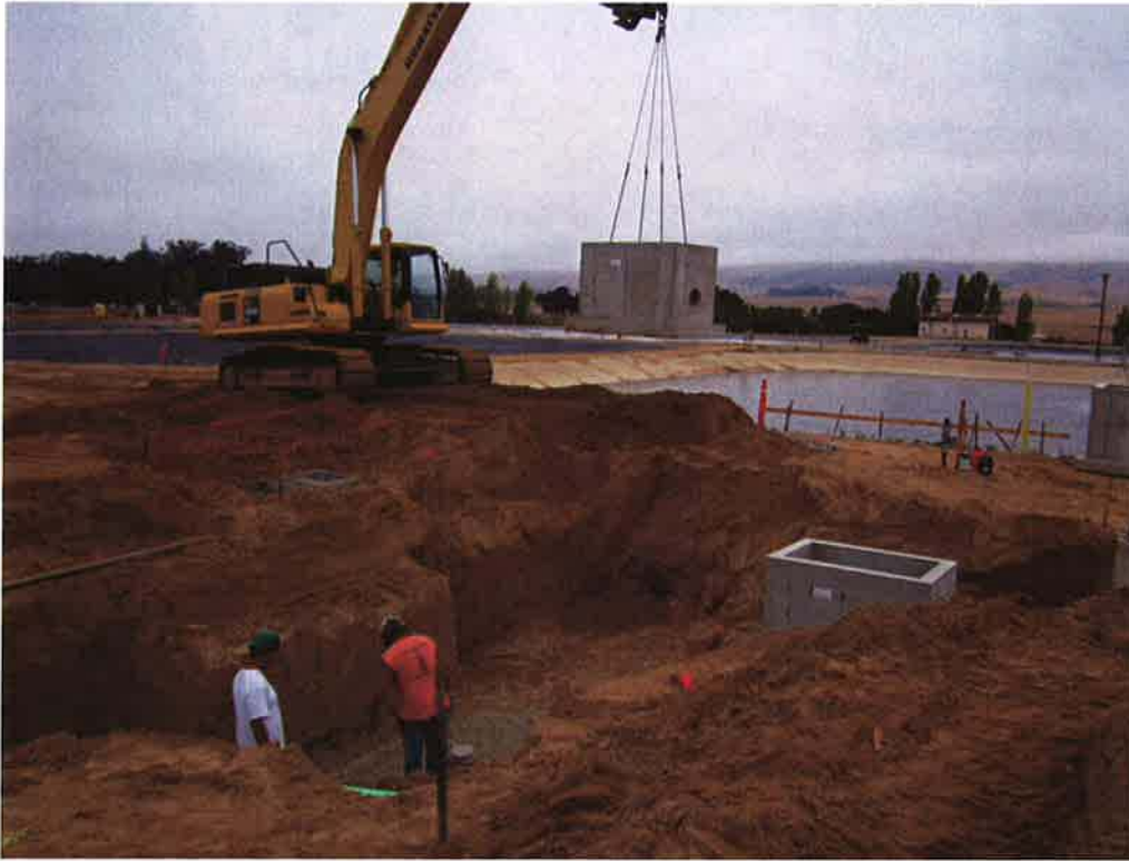
Cushman installing flow meter vaults.
