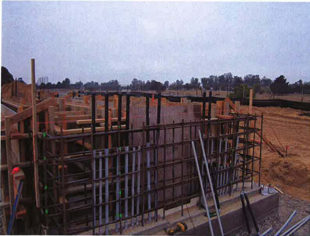
Bergelectric installing through-wall conduit at Headworks Screening System
