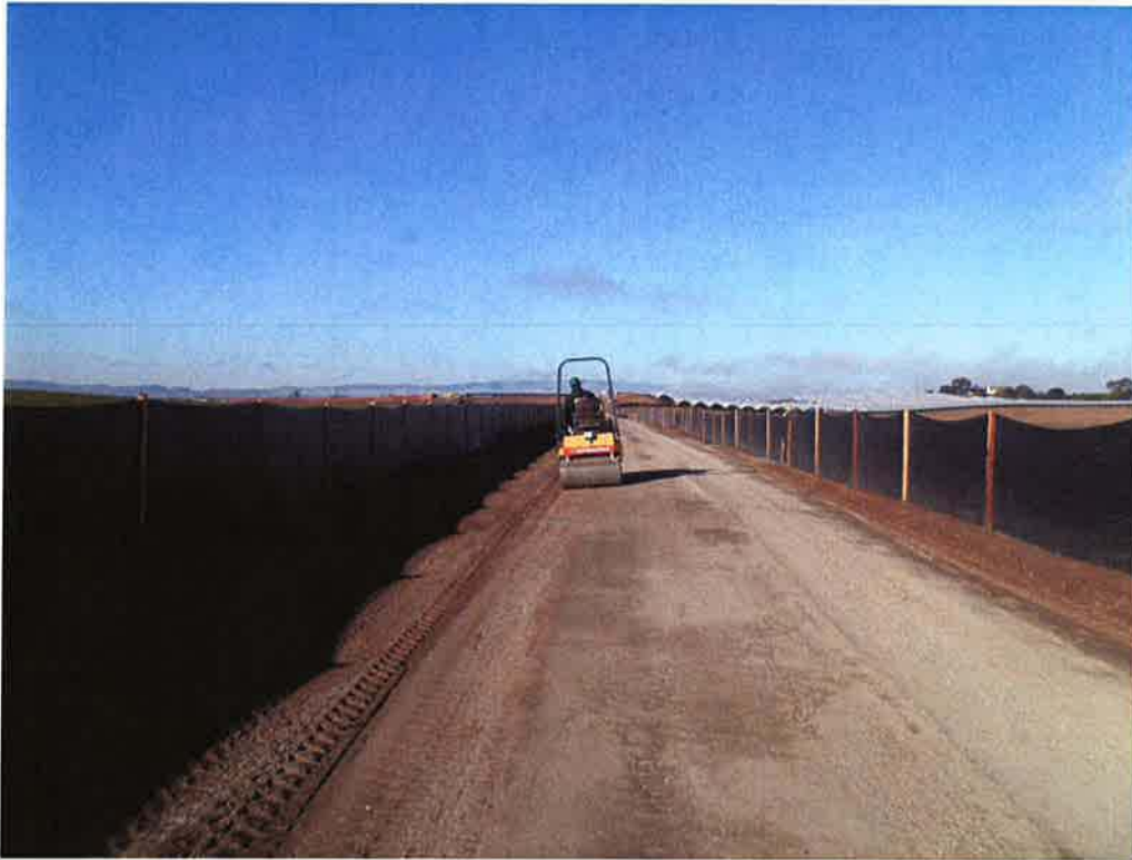
Burke compacting recycled aggregate base on temporary access road.
