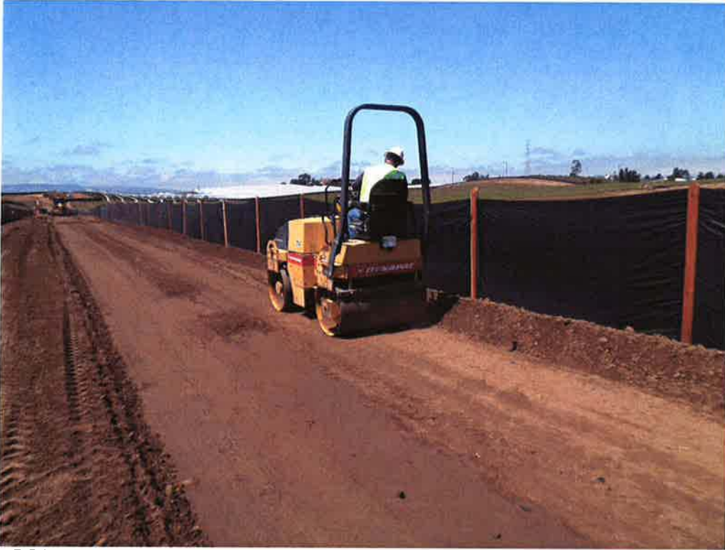
ARB's subcontractor Burke Construction building temporary access road to the pump station site on the north side of the project.
