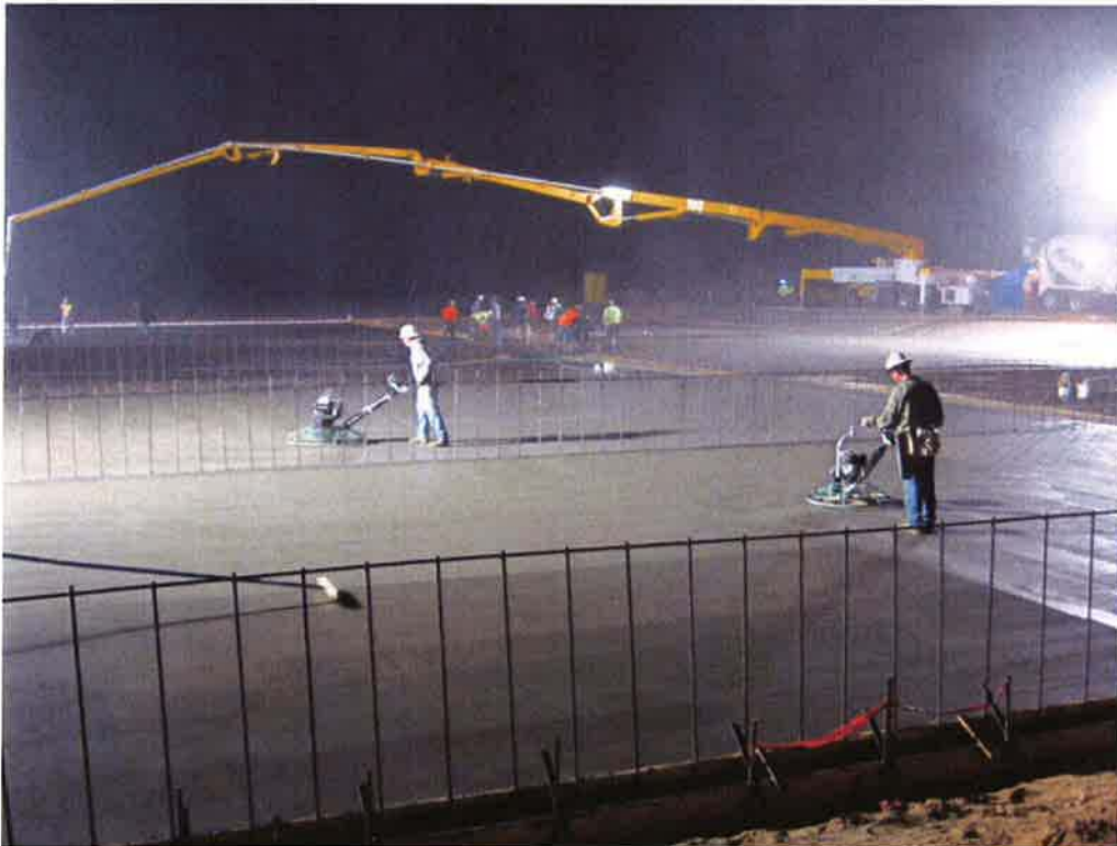
Cushman starting finish work on concrete slabs at Sludge Drying Beds during first night pour.
