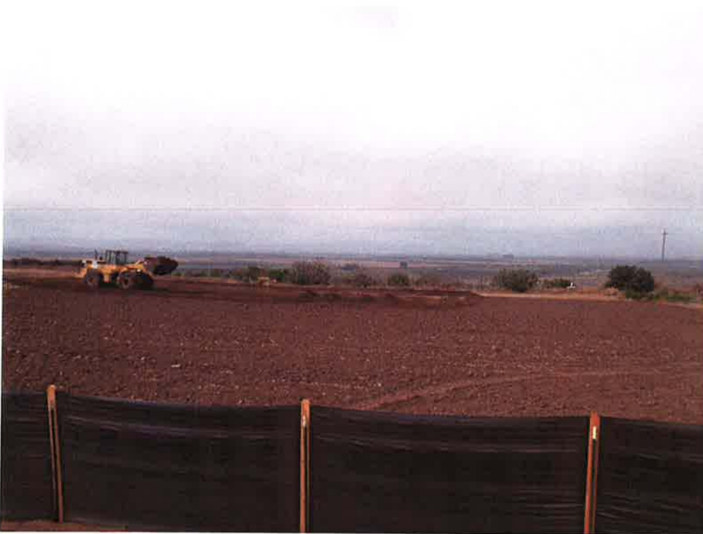
Burke spreading excavated and preserved top soil to the west of the future pump station as directed by Linda Vista Farms.
