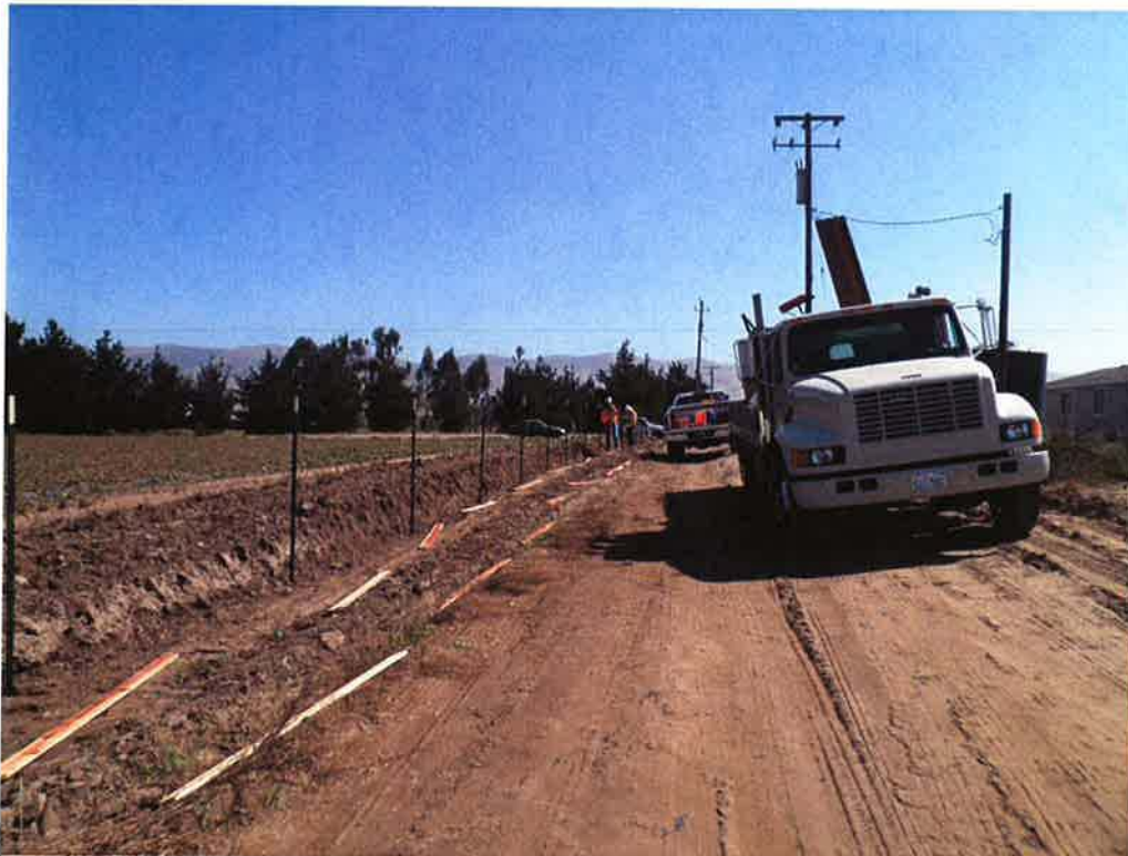
Marborg and ARB installing tee posts for the silt fence along the access road to the pump station site on the north side.
