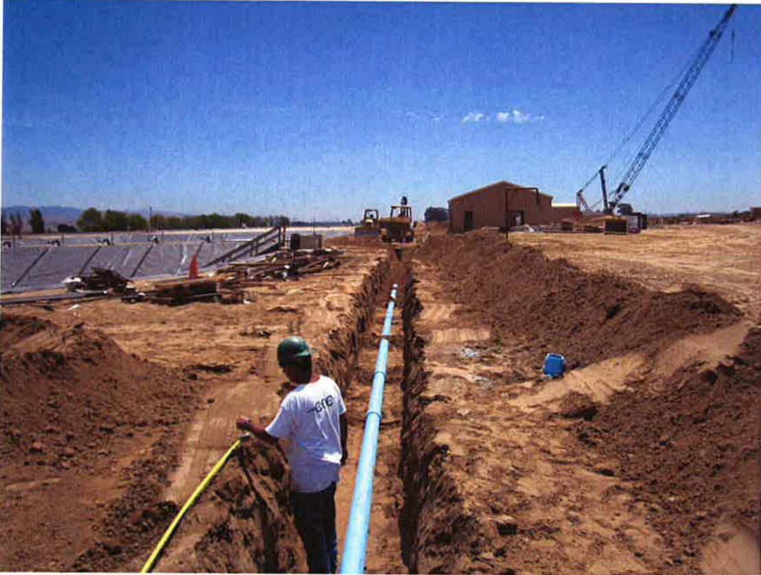
Cushman installing 6-inch water line.
