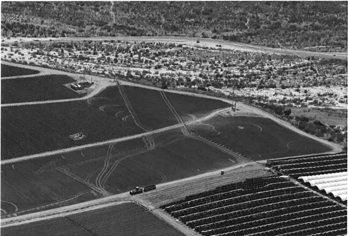
Aerial view of the north side of the project at the future pump station site.
