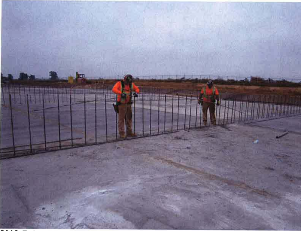
CMC Rebar tying reinforcement for walls at Sludge Drying Beds.
