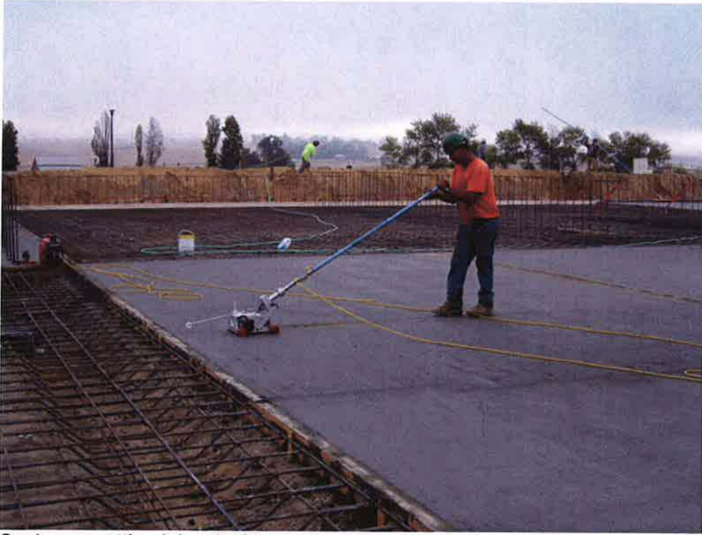
Cushman cutting joints in Sludge Drying Bed #1 after first concrete pour.
