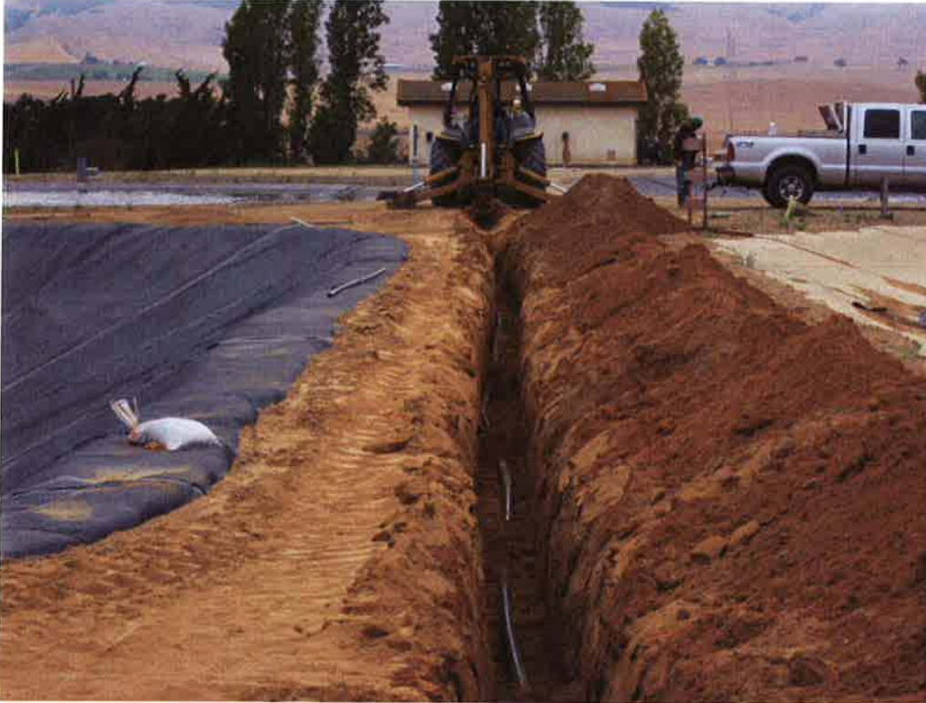
Installing 2-inch NPW line.
