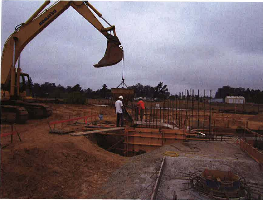
Cushman pouring concrete for lower walls of Headworks Screening System.
