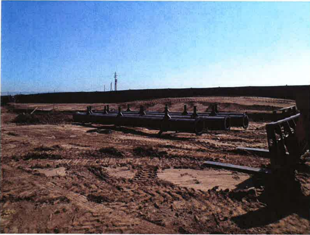
Casing centralizers on site for installation inside the 54-inch diameter casing.
