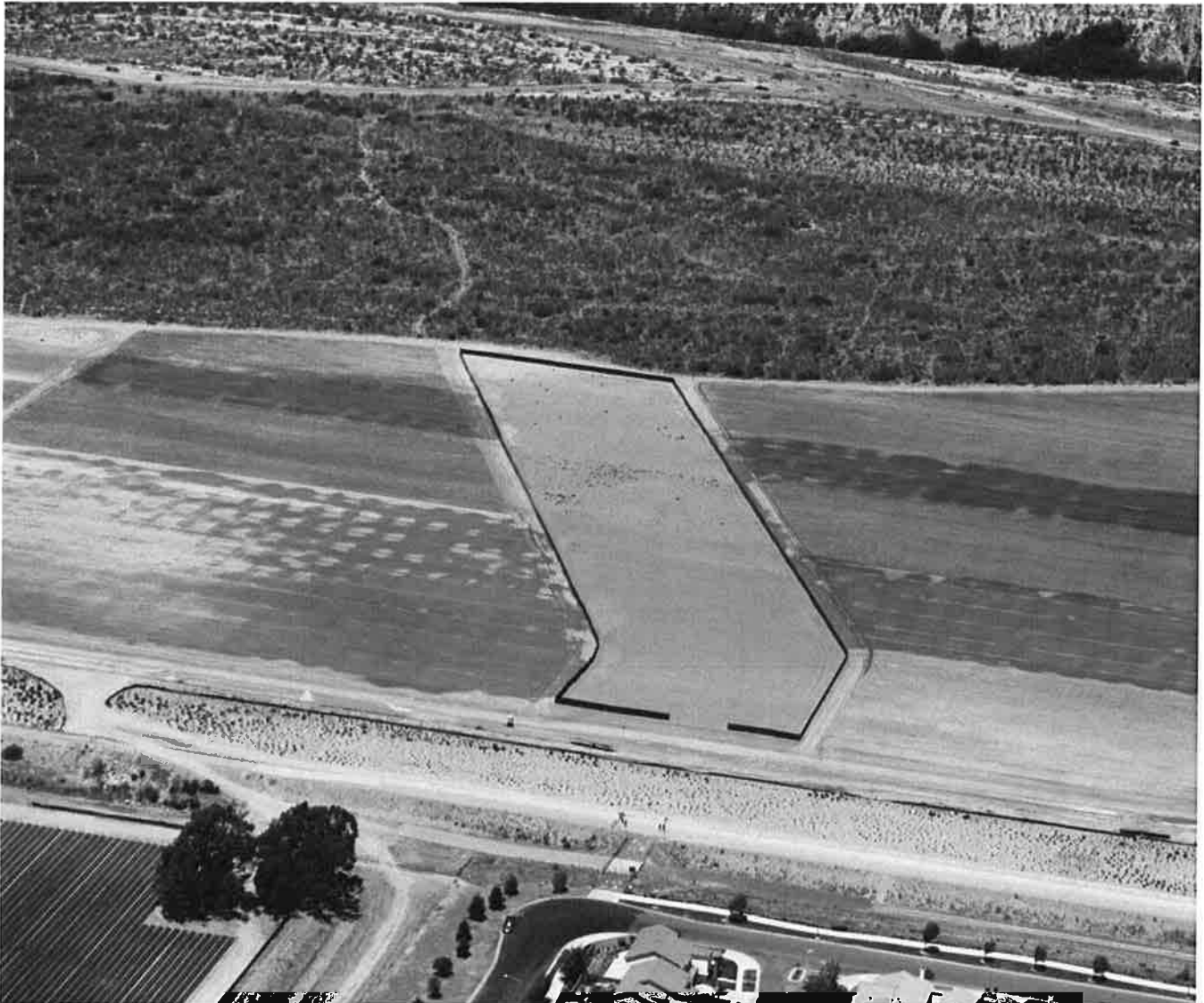
Aerial photo of the south side with silt fence installed at temporary construction easements.
