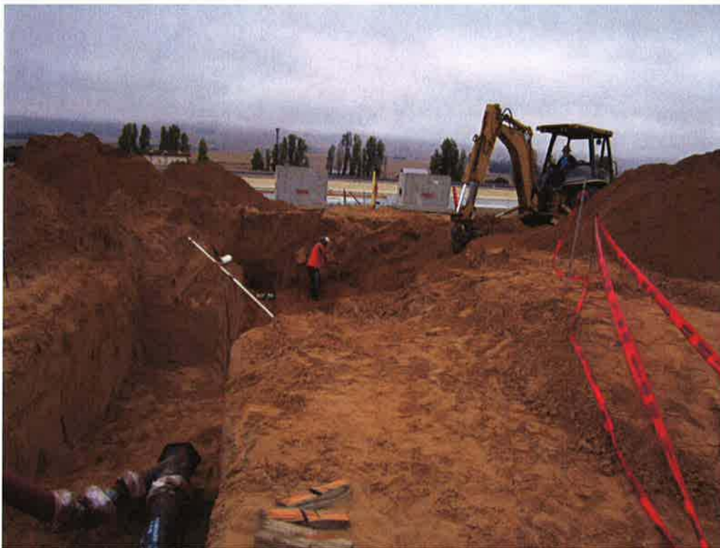
Cushman excavating for flow meter vaults.
