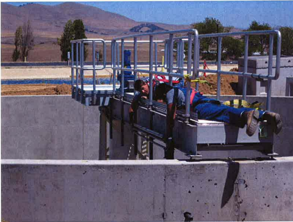
Bergelectric installing rigid conduit along the bridge at Clarifier #2.
