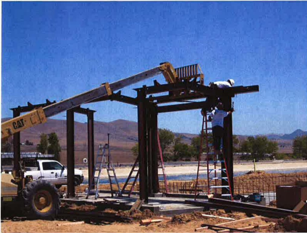
Dueck Construction erecting steel structure to support canopy.
