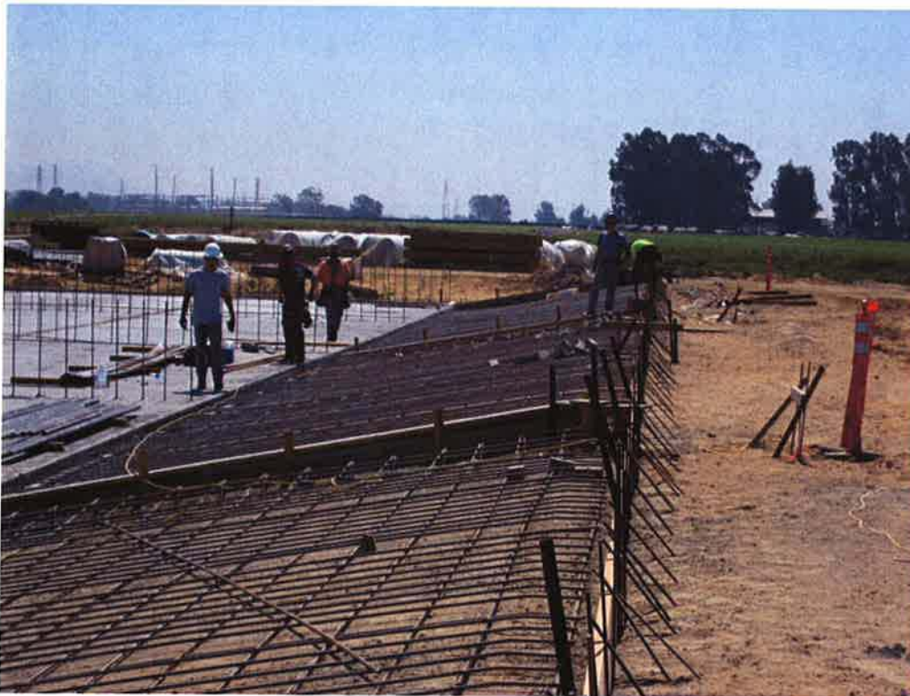
Cushman setting footing edge board along ramp at Sludge Drying Beds.
