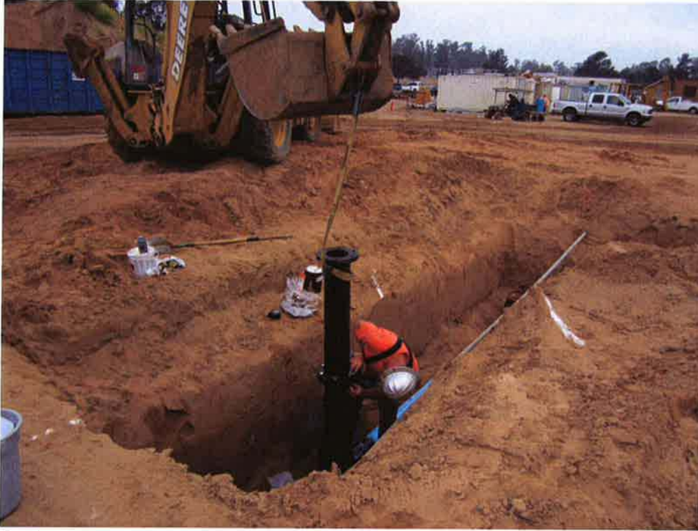
Cushman installing riser for fire hydrant off 6-inch waterline.
