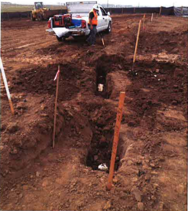
ARB potholing for existing irrigation lines crossing the future pump station site and HDD work area.
