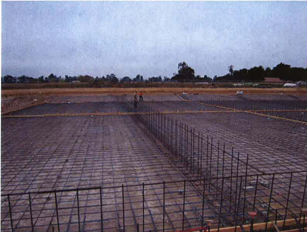
Cushman forming construction joints at Sludge Drying Beds.
