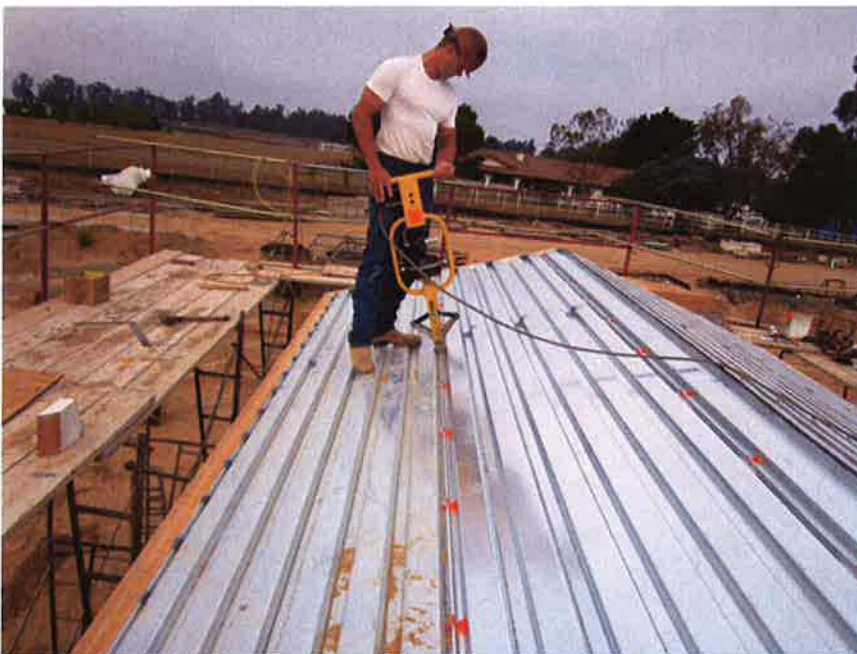
Cushman crimping metal deck on Sodium Hypochlorite Building.
