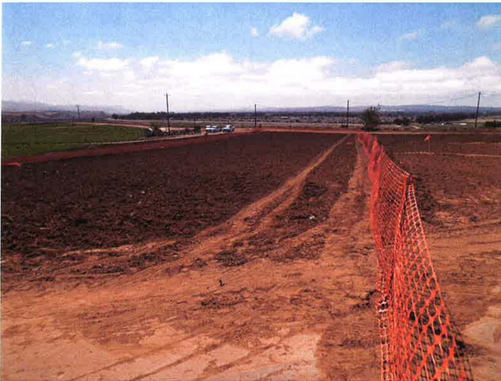
ARB installing temporary orange snow fence on boundaries of temporary construction easement to protect HDD tracing wires during drilling.
