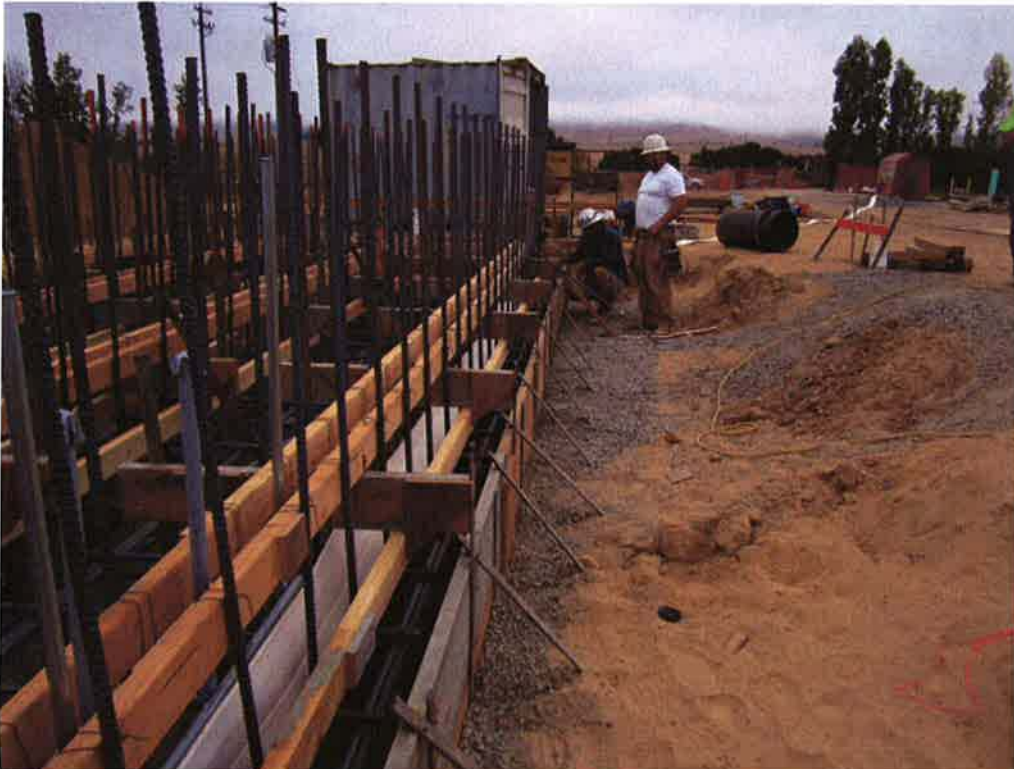
Cushman installing water stops at the Headworks Screening System walls.
