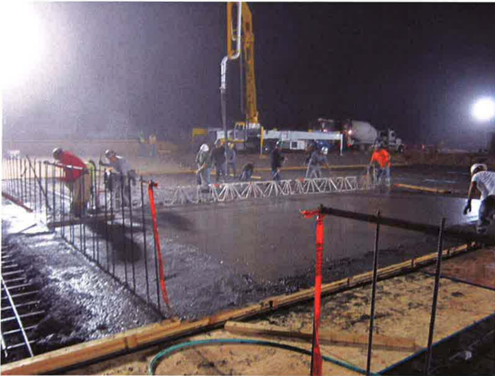
Skreeding concrete of first slab section in Drying Bed #1.
