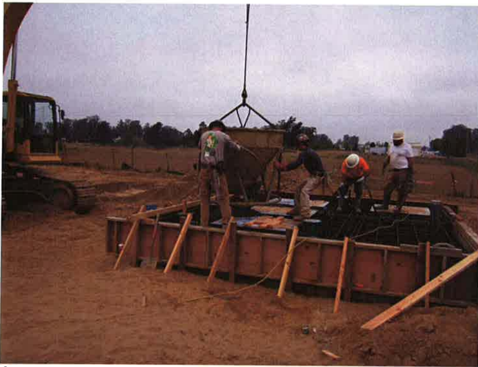
Concrete placement for deck of Influent Pump Station.
