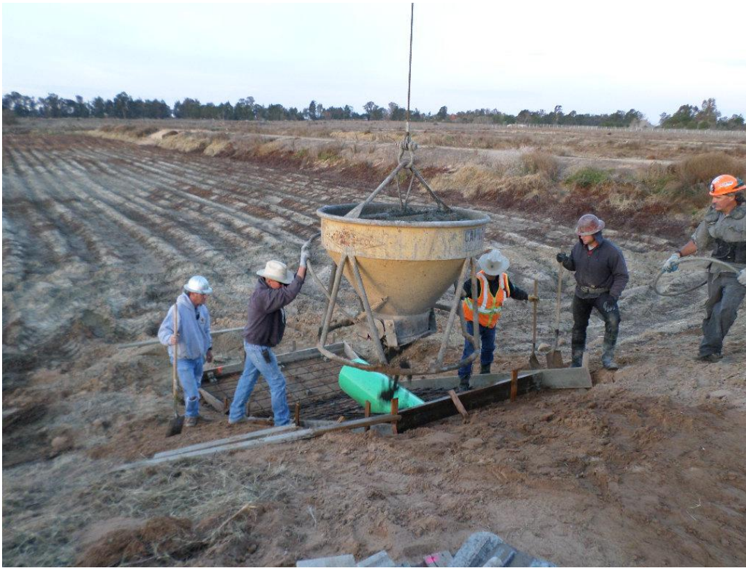
Cushman pouring 4,000 psi concrete at inlet structure splash pads.
