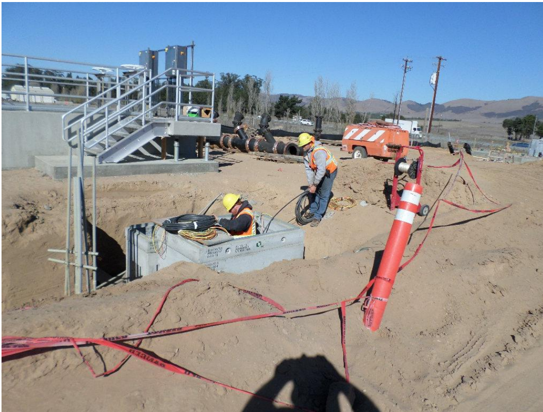
Bergelectric pulling wires to the Headworks.
