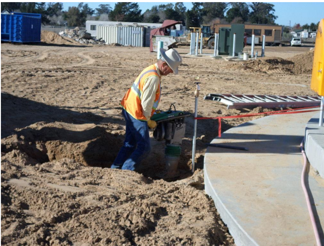
Cushman installing NPW and hose bibs at Clarifiers.
