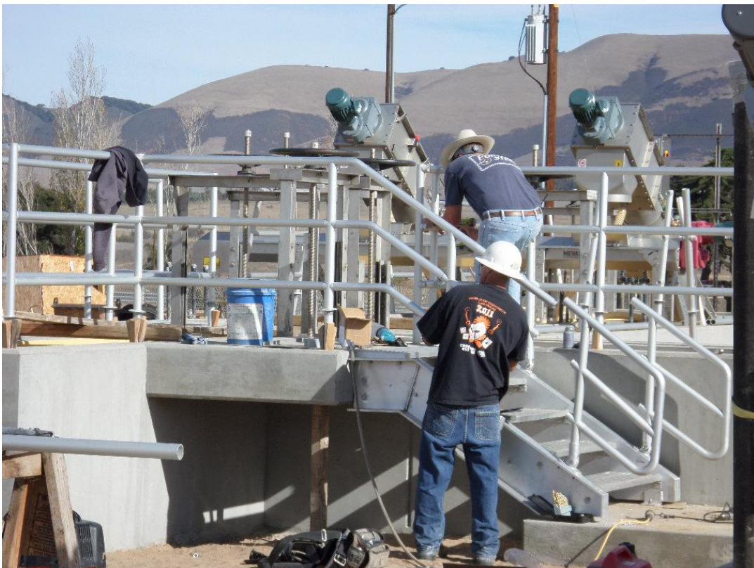
Cushman installing the aluminum handrail.
