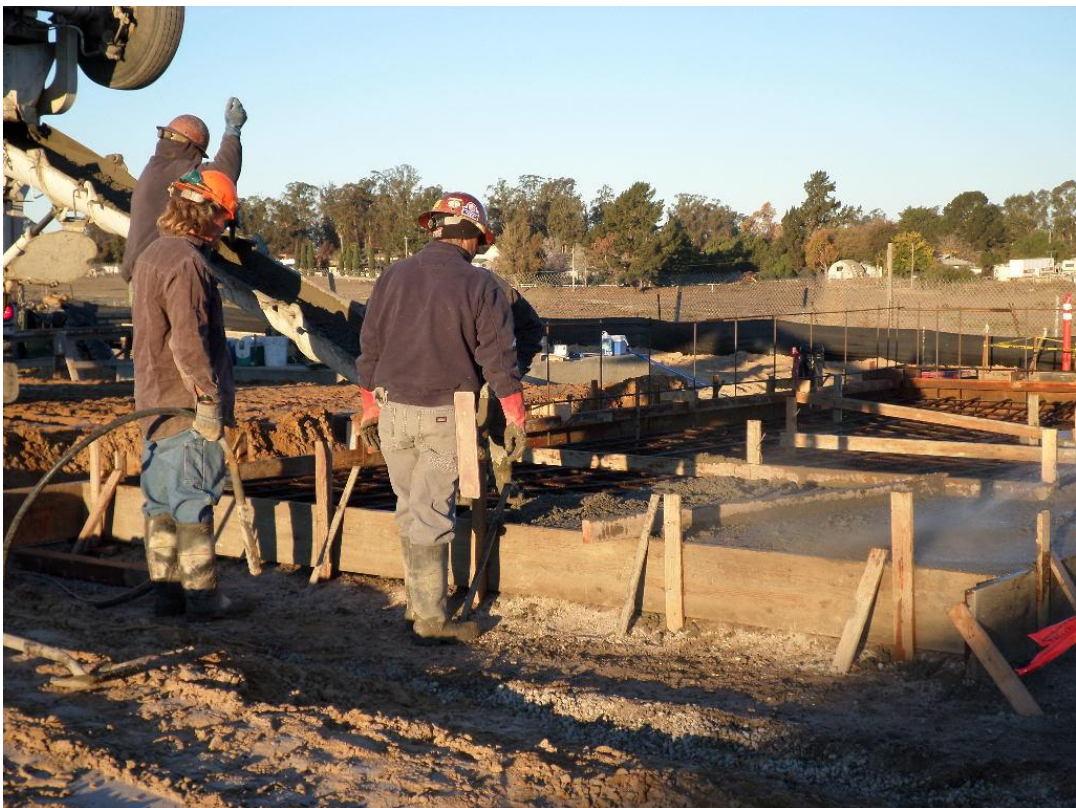
Cushman pouring 4,000 psi concrete for the truck wash down station slab.
