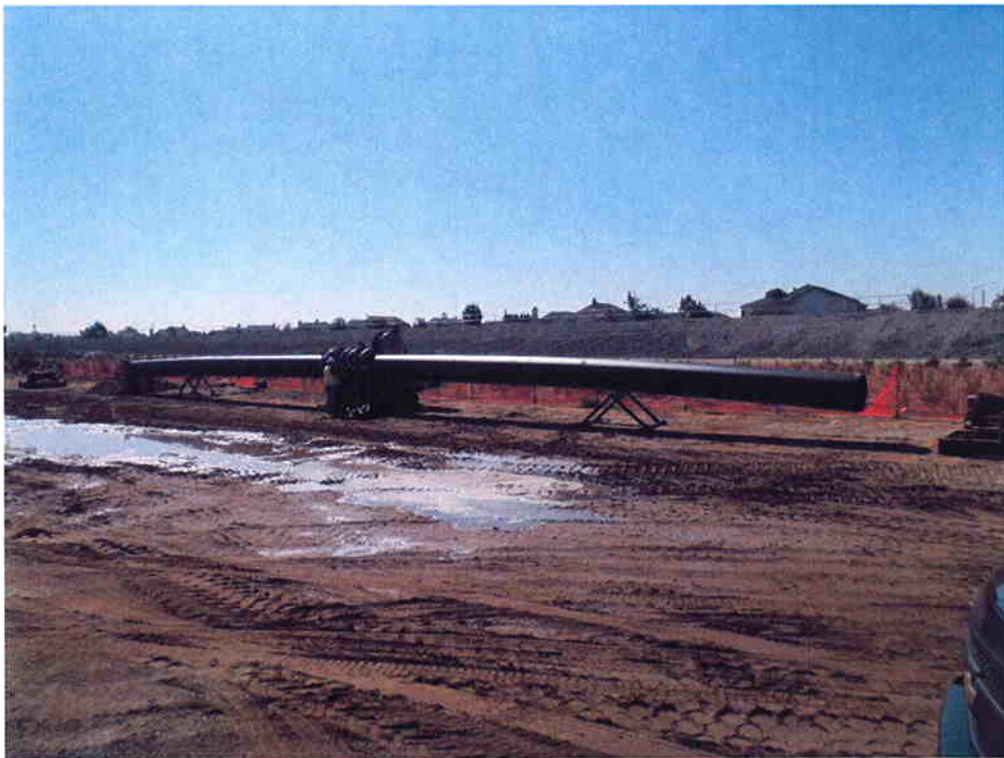
ARB starting fusion welding of the 24-inch diameter HDPE carrier pipe.
