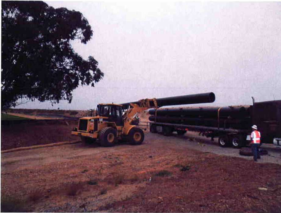
HDPE pipe being unloaded.
