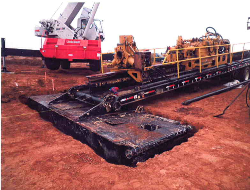
ARB positioning drill rig on front deadman.
