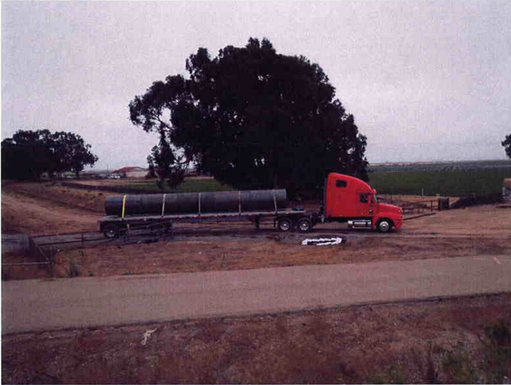
Delivery of 54-inch diameter steel casing, 40 foot section.
