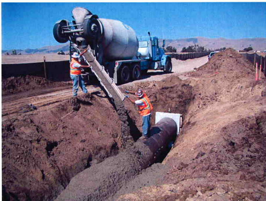
ARB pouring slurry over steel casing before backfilling to install the 18-inch RCP pipes.
