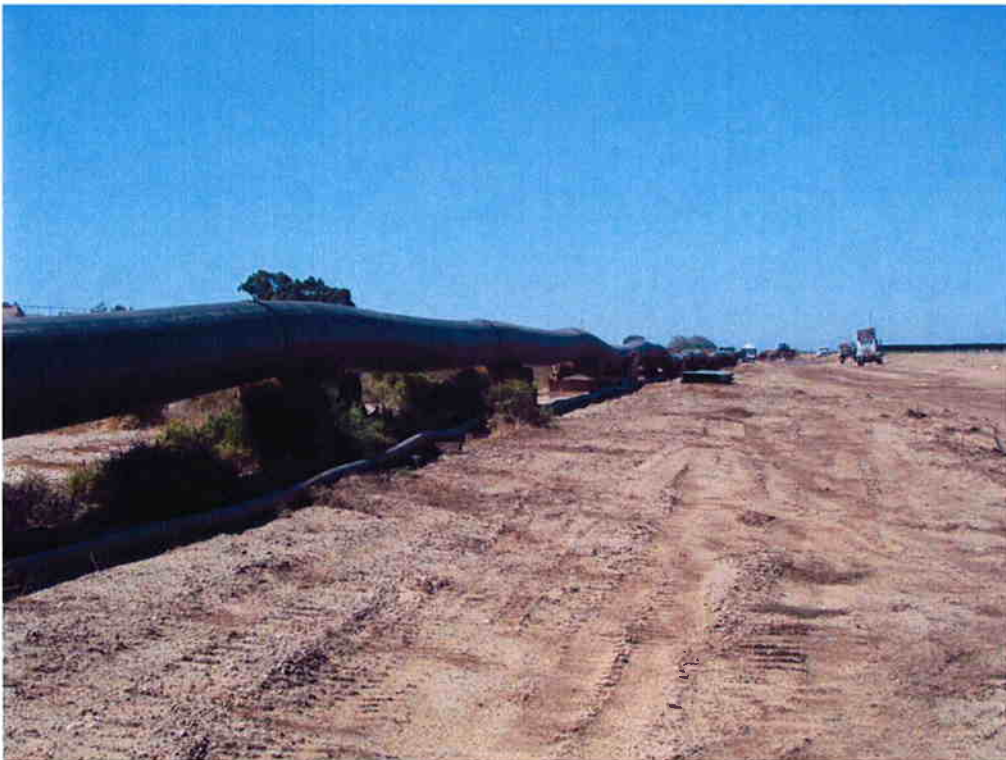
HDPE pipe with one of the 4-inch pipes next to it which will be inserted into the HDPE carrier pipe to provide a ballast and vent to prevent a vacuum when the pipe is pulled into place.
