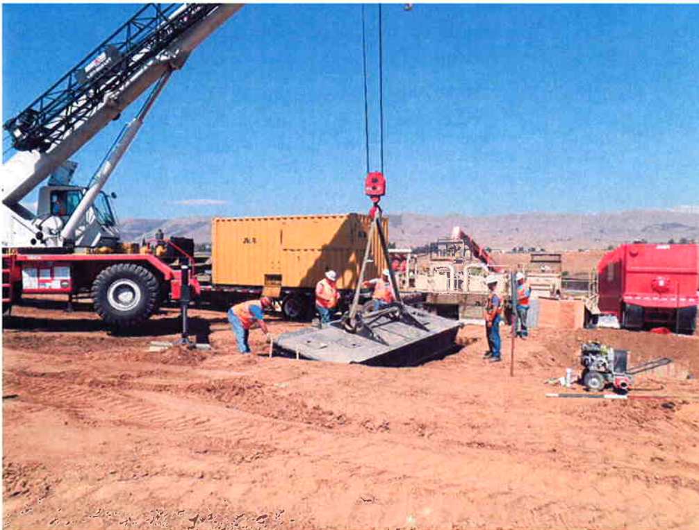
ARB unloading deadman front section which supports the drill rig.
