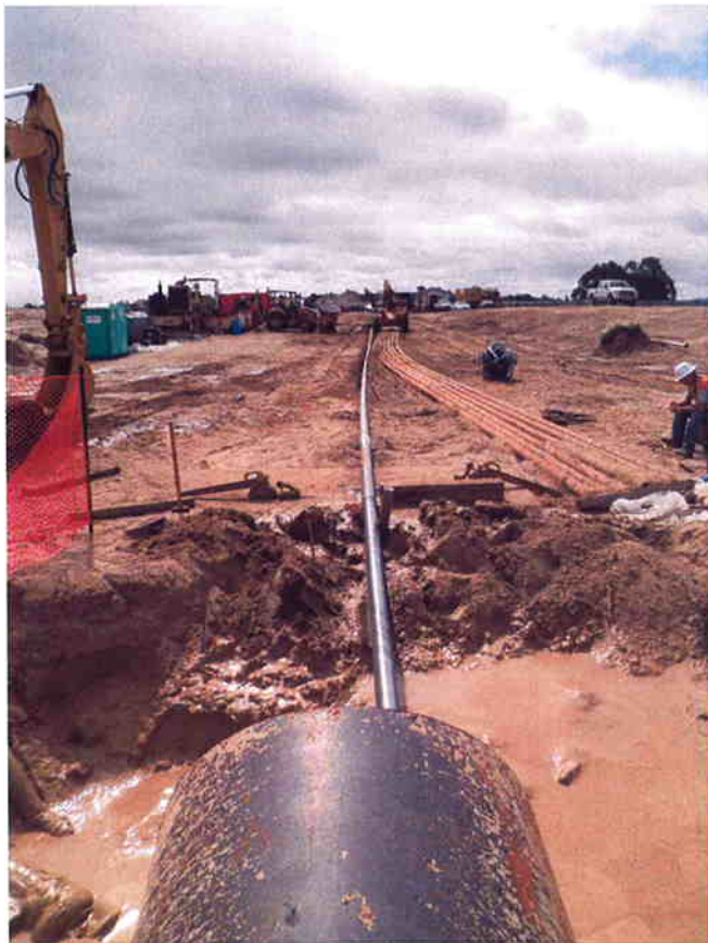
"Tail string" of pipe following the 36-inch drill being pulled from south to north.
