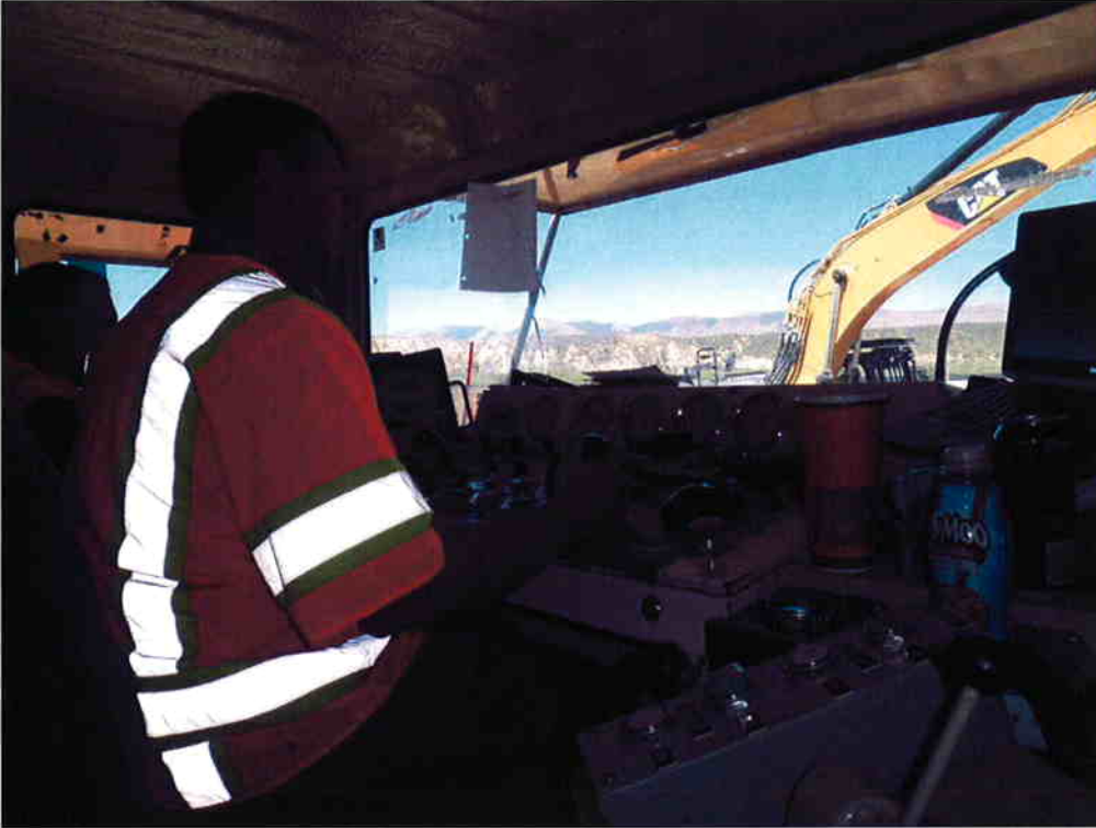
ARB drill operator and manager in control room during pilot hole drill.
