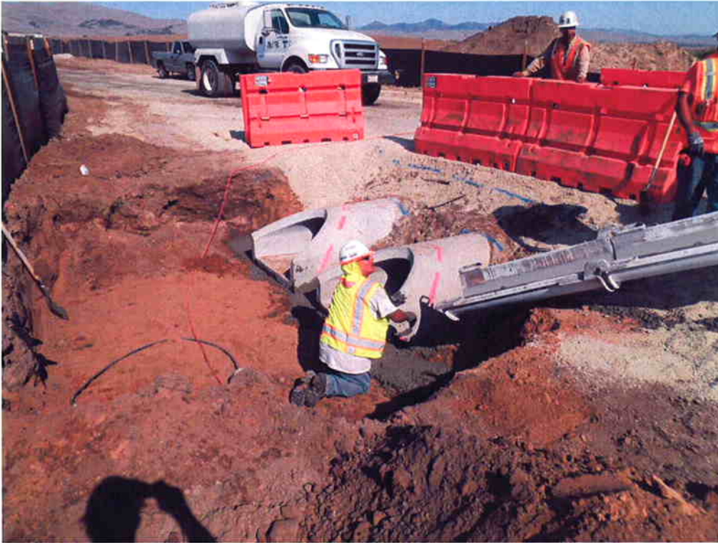
ARB pouring concrete cut-off wall at the end of the 18-inch RCPs.
