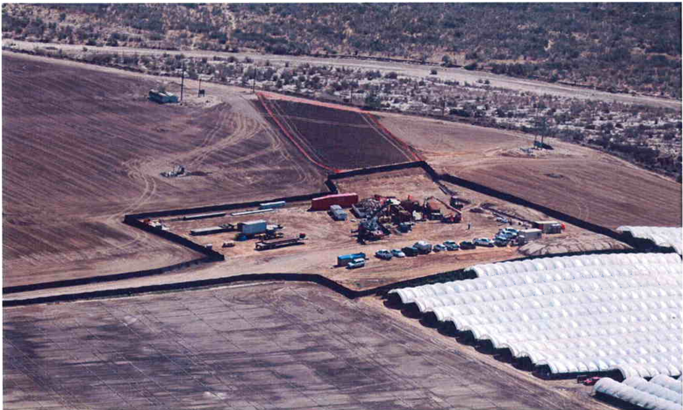
Aerial view of the north side of the project with ARB drill rig and equipment mobilized.
