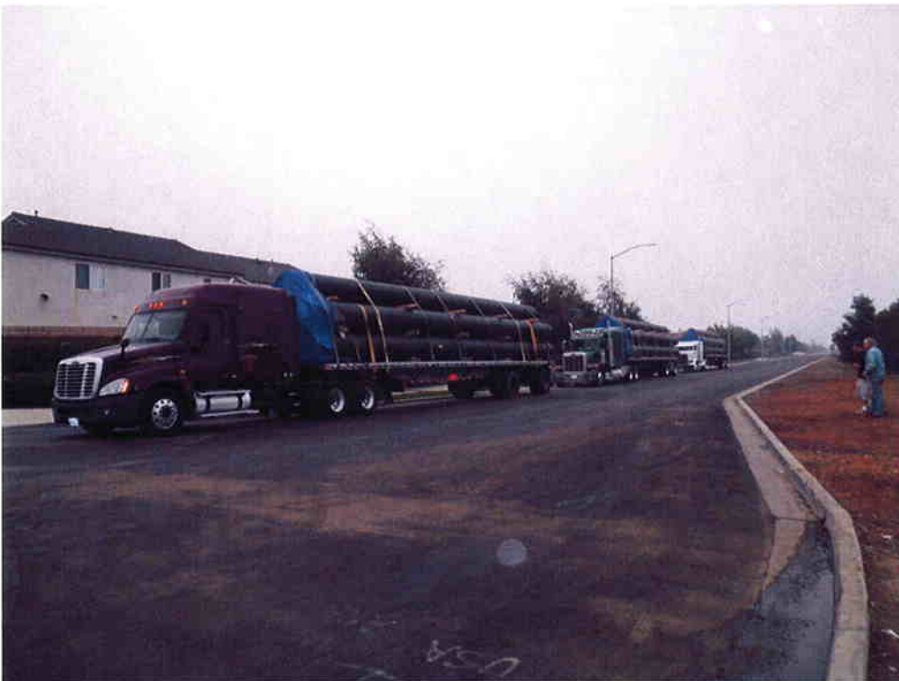
HDPE pipe arriving on site.
