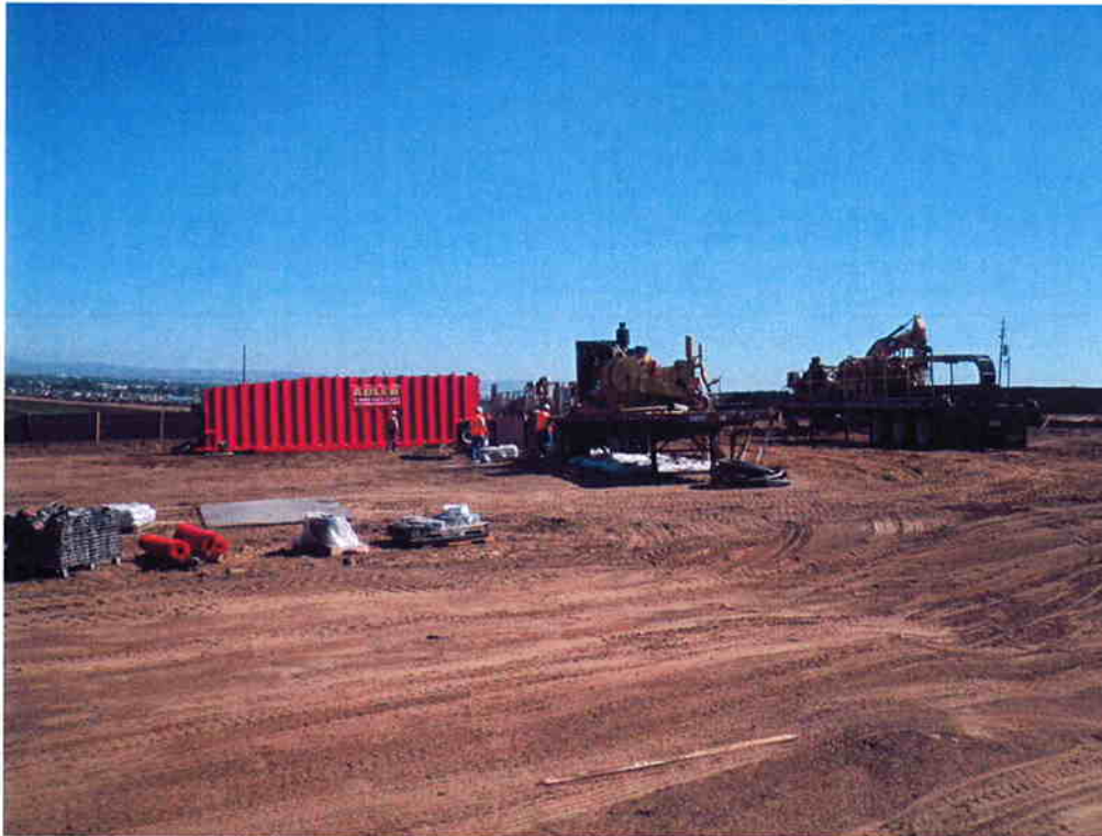
ARB drill equipment mobilizing to north site.
