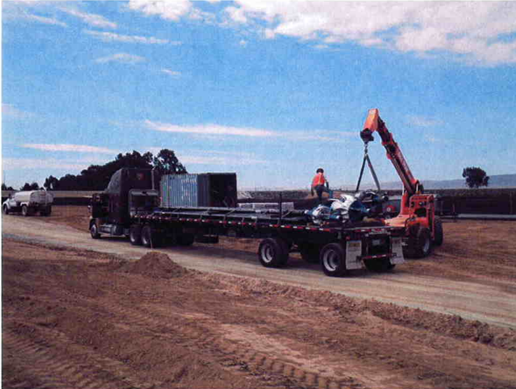
Drill heads delivered to site.
