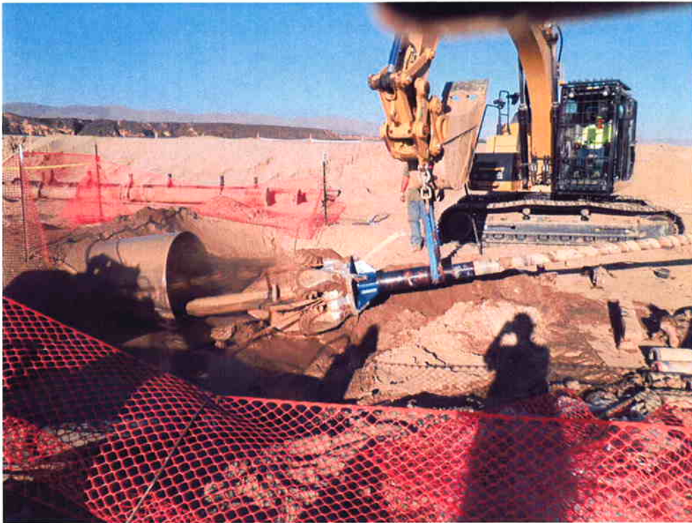
The 42-inch drill entering the 54-inch casing.
