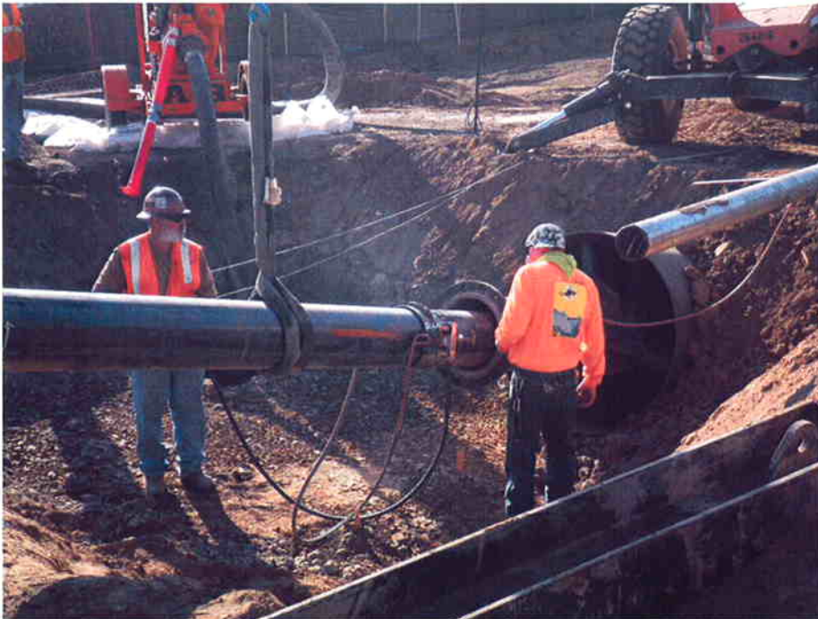
ARB welder cutting excess 12-inch casing once it was in place.
