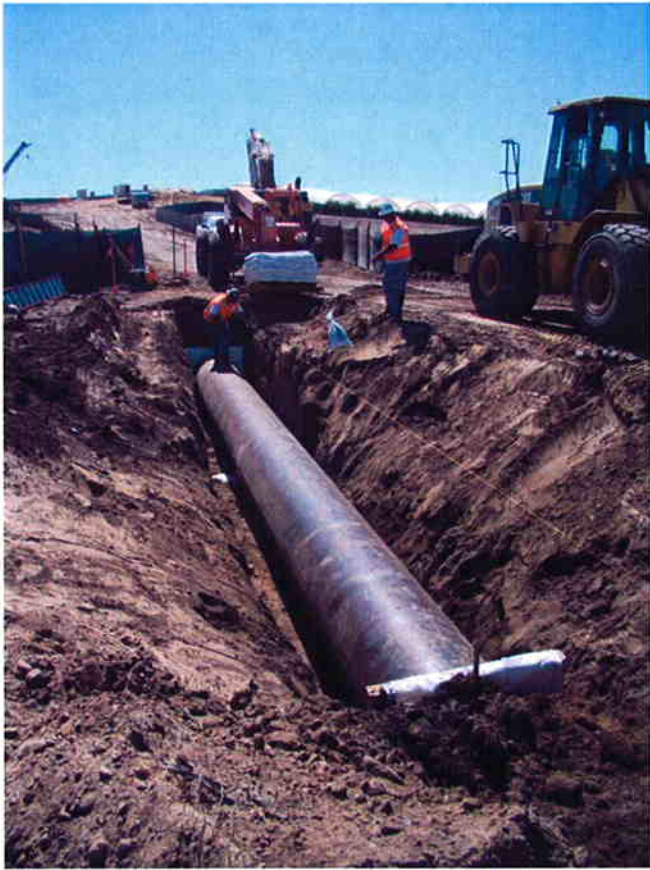
Steel casing installed with ends blocked.
