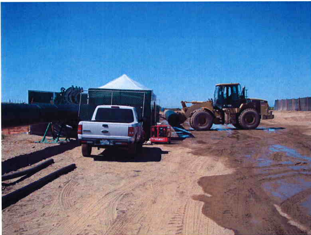
ARB moving another 50 foot section of HDPE pipe into place for fusion welding.
