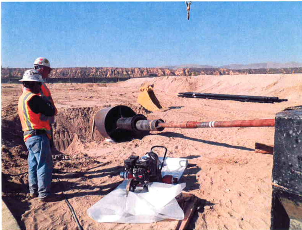
12-inch casing drilled into place inside the centralizer and 54-inch casing.
