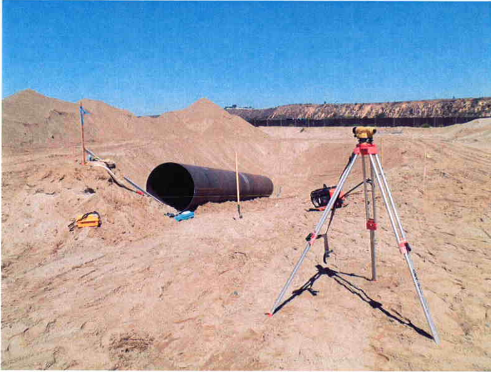
54-inch casing being installed at entry point on the south site.
