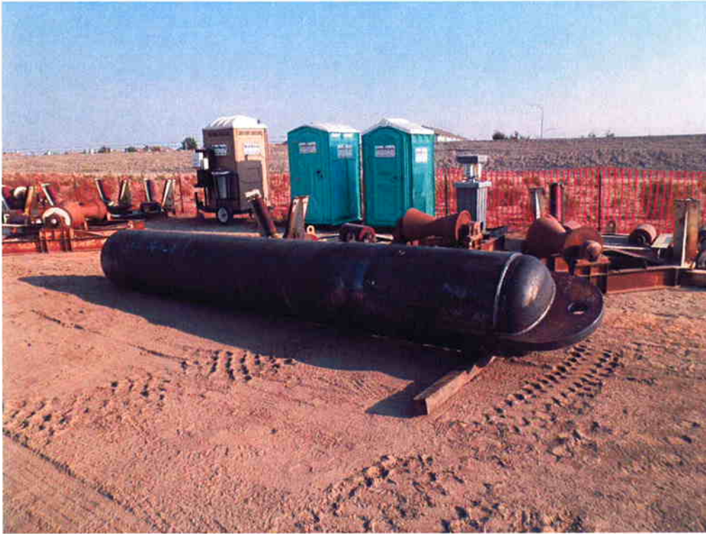
Pull head delivered to site.
