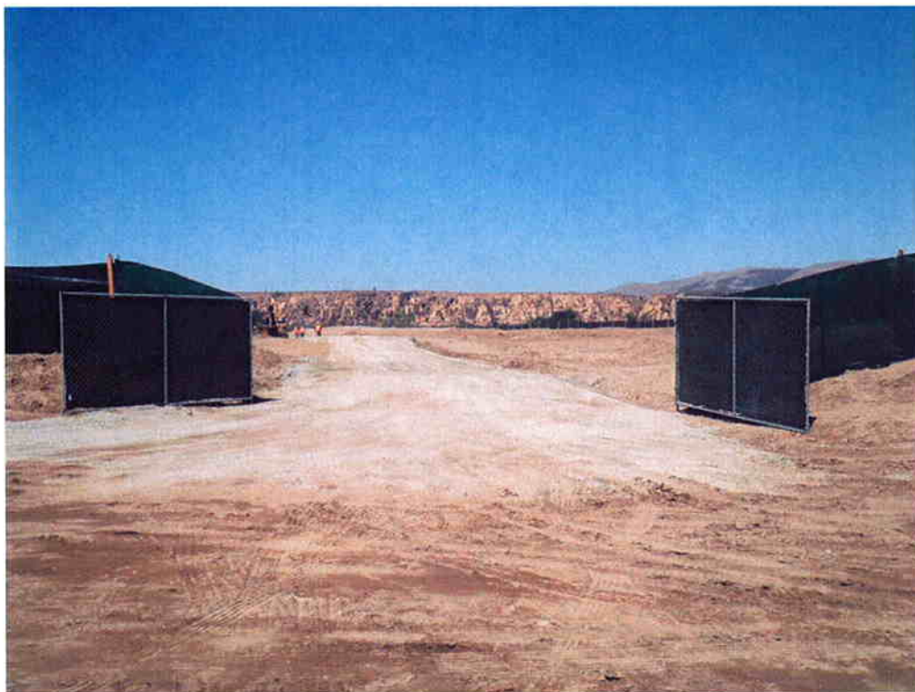
Gates installed at entrance of the south site.
