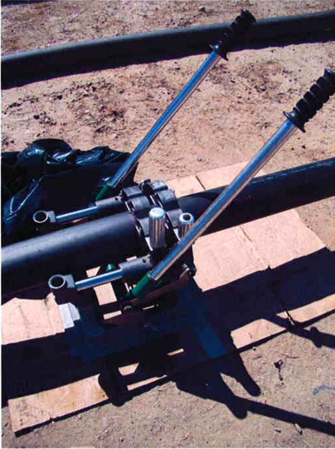
Small machine used to fuse weld the 4-inch ballast and vent pipes.
