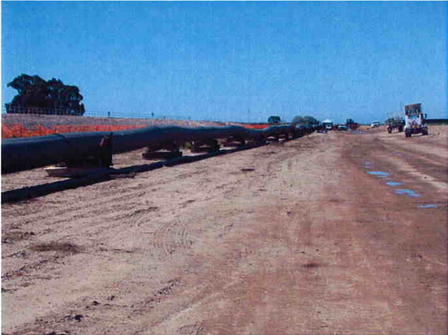
HDPE pipe laid out to the east of the site on rollers along the north side of the levee after being fusion welded.
