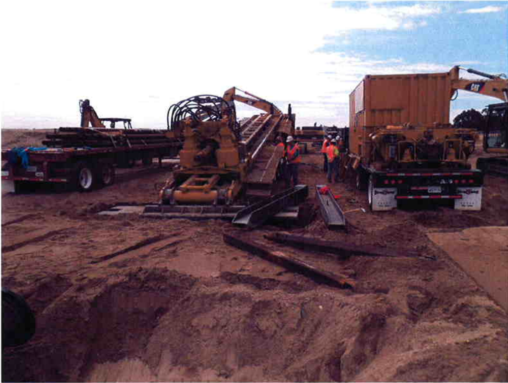
ARB positioning front of drill rig on deadman at south site.
