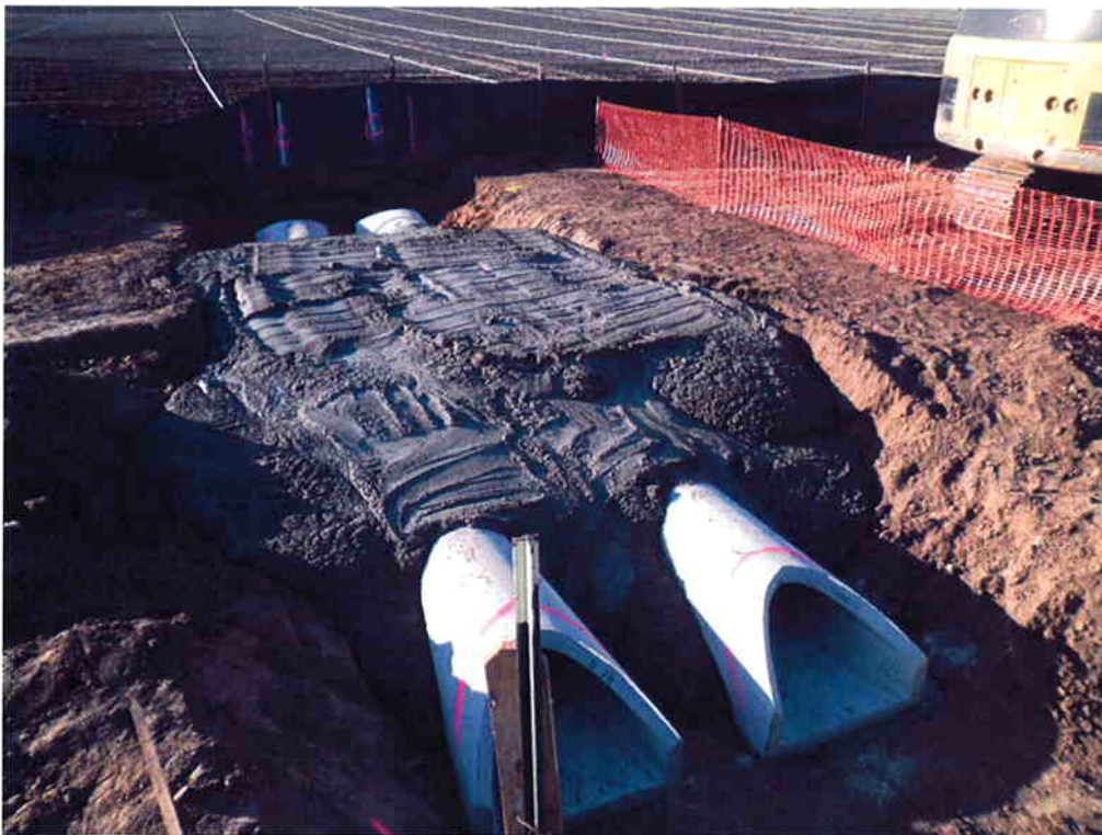
Slurry placed over the 18-inch RCPs.
