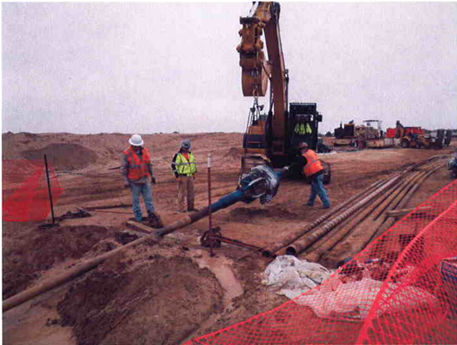
ARB positioning 36-inch drill.
