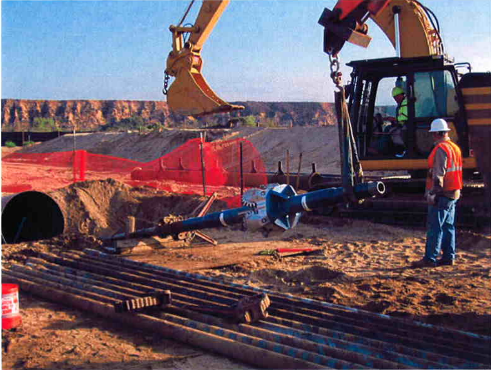
ARB preparing for the 26-inch reaming pass from the south site to the north site.
