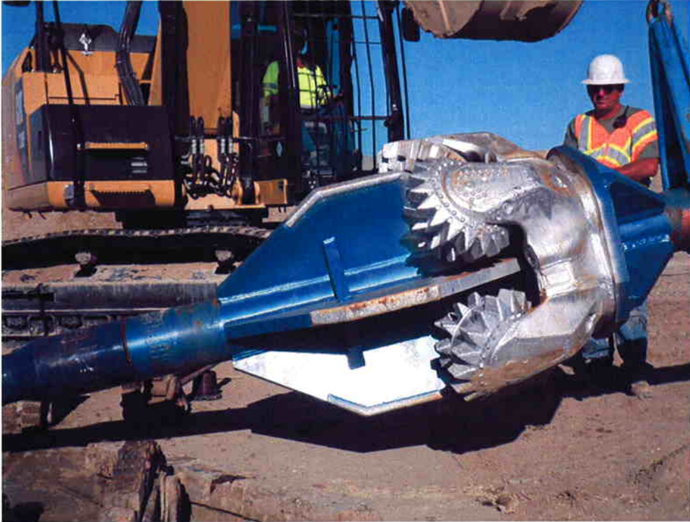
The 42-inch drill being positioned to start reaming.
