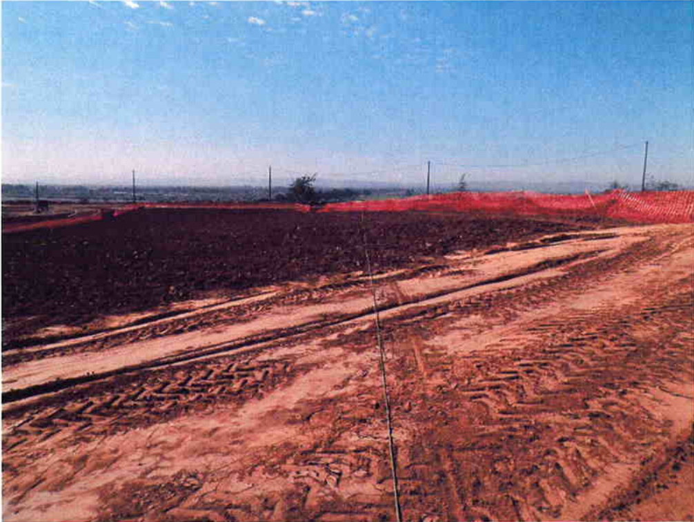
Tracer wire laid out across temporary construction easement from the north site to the bluff edge.
