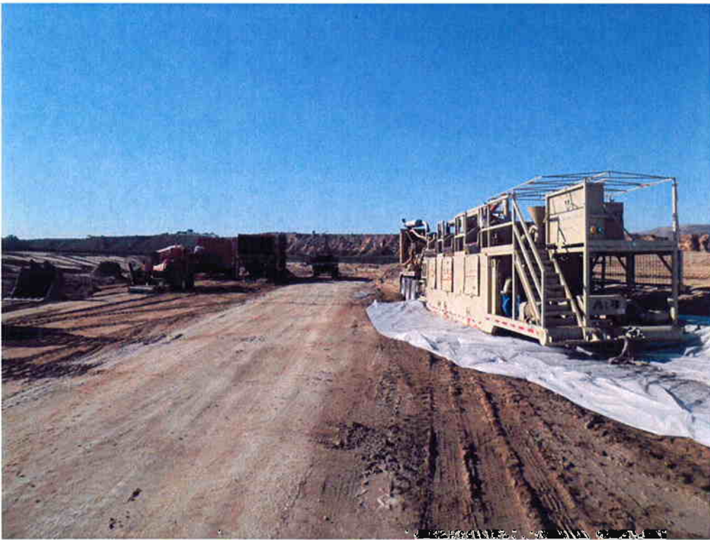
Mud cleaning equipment placed on plastic for environmental protection.
