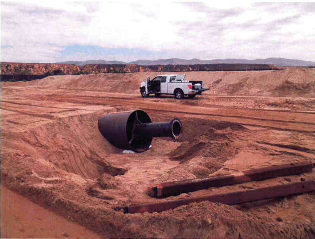
54-inch casing with centralizer installed.
