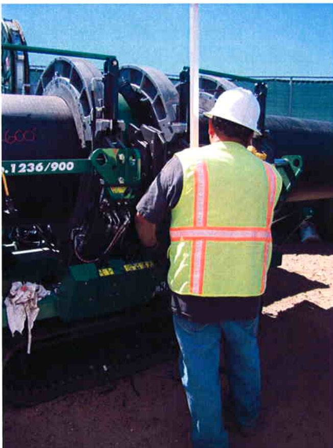
ARB welding operator cutting the pipe ends to achieve a smooth surface for fusion welding.
