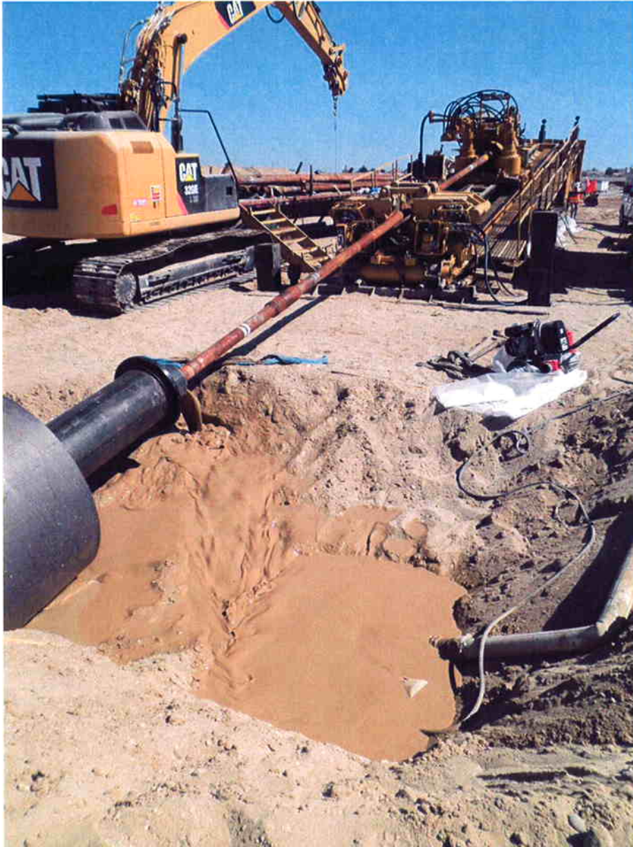
Pilot hole drilling in progress.
