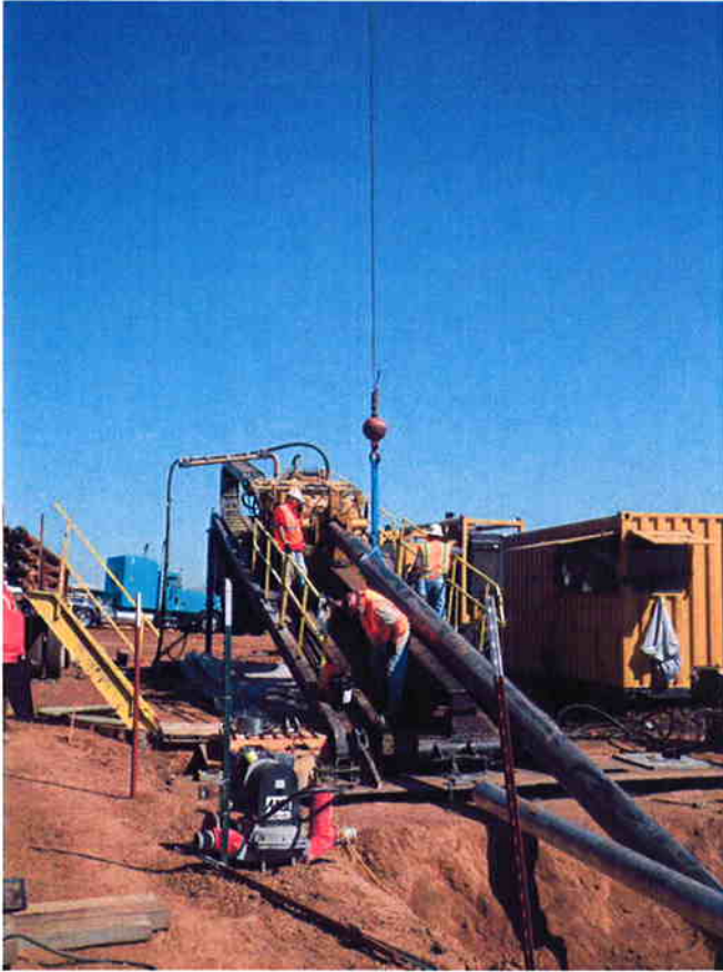
ARB installing 12-inch casing inside centralizer and 54-inch casing.
