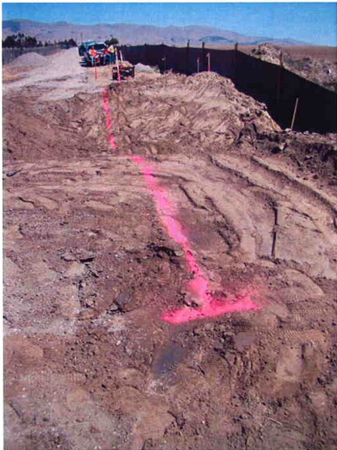
ARB layout for 36-inch diameter steel casing.
