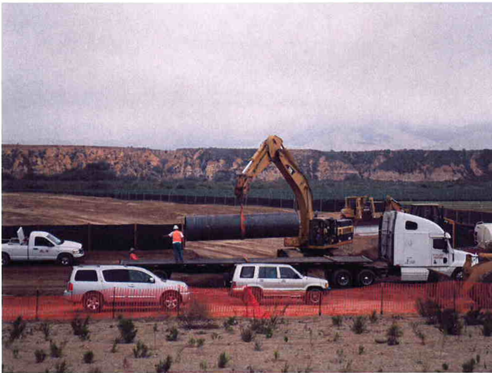
ARB unloading 20 foot section of 54-inch diameter steel casing.
