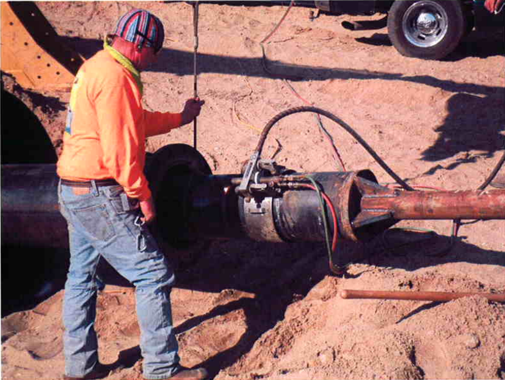
ARB's welder cutting the end of the 12-inch casing after it is in place.
