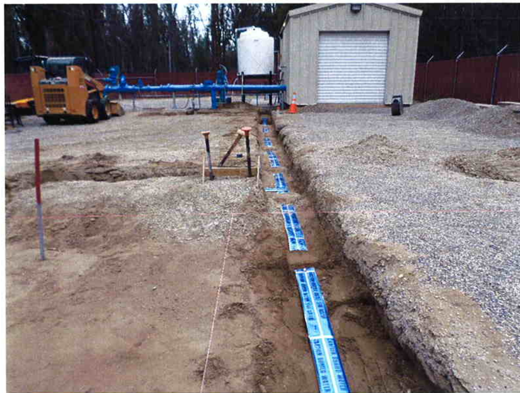
Spiess backfilling and placing tape over chemical tubing pipe.
