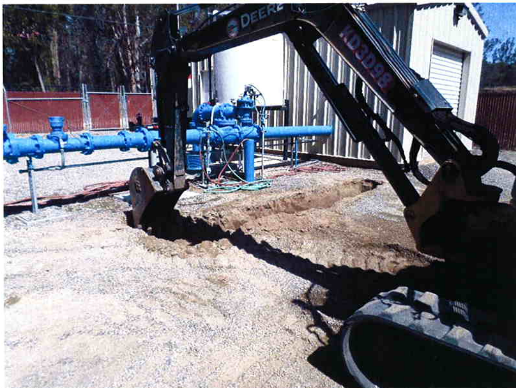
Spiess excavating to install plant water pipe.
