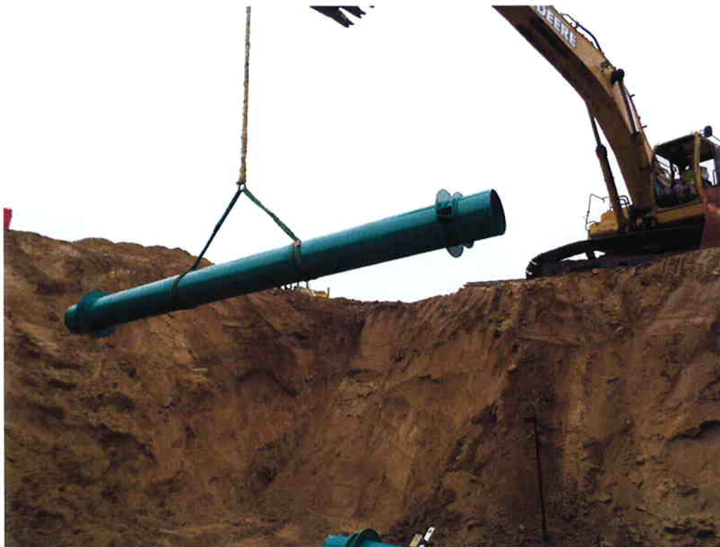
Installing suction piping.
