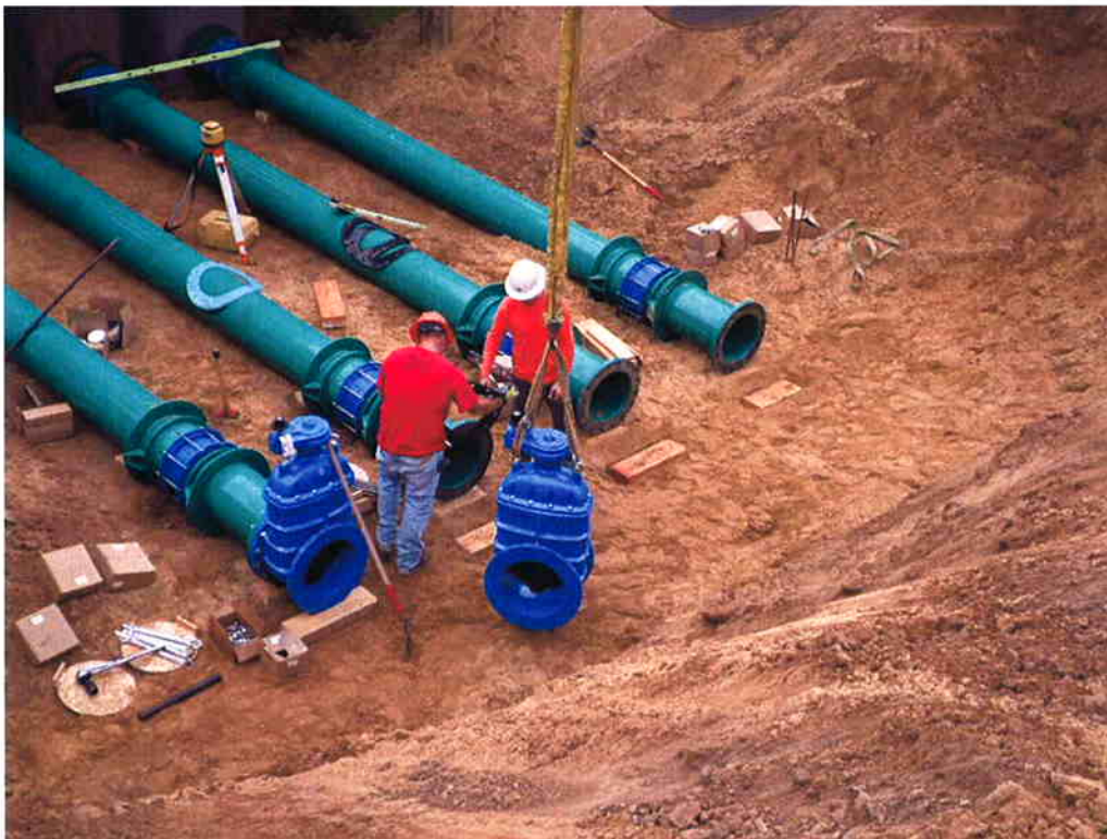
Spiess installing 16-inch valves.
