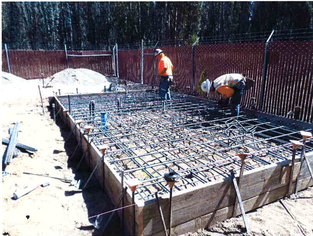
Vista Steel installing reinforcing at Chemical Building.
