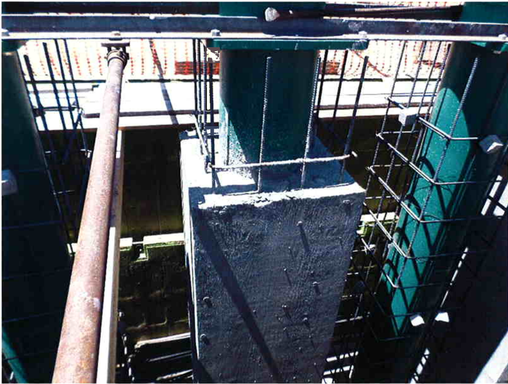
Forms stripped from around first encasement pour at pump cans.
