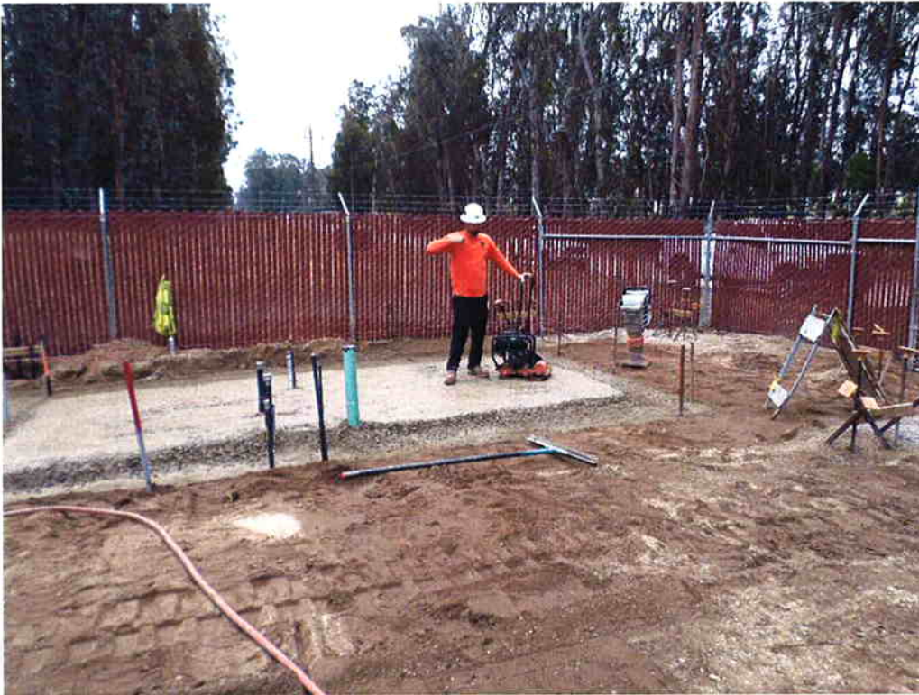
Spiess compacting base material for the Chemical Building slab.
