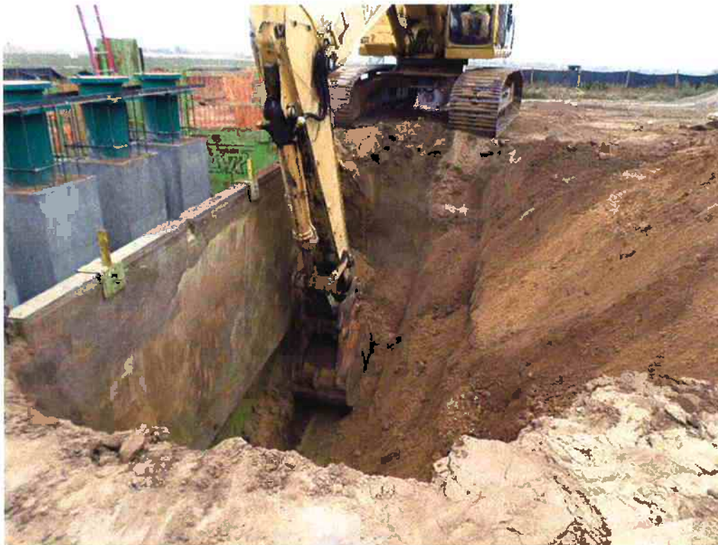
Spiess excavating and cutting back sides for installation of the suction piping and manifold.
