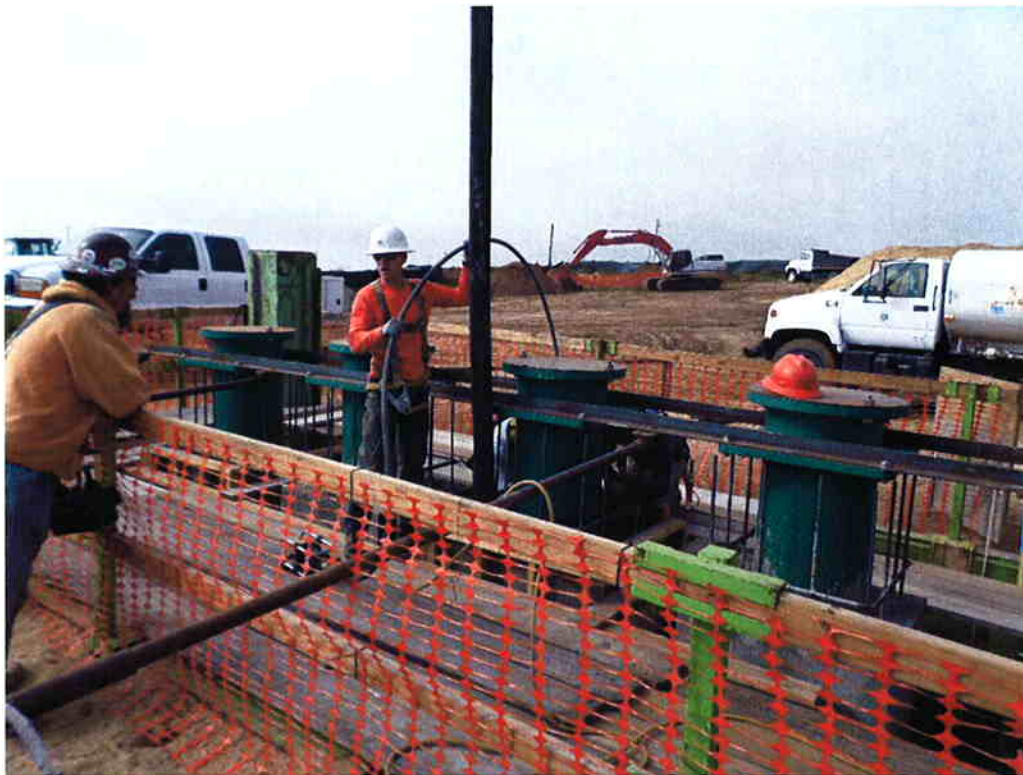
Spiess pouring last two pump can encasements.
