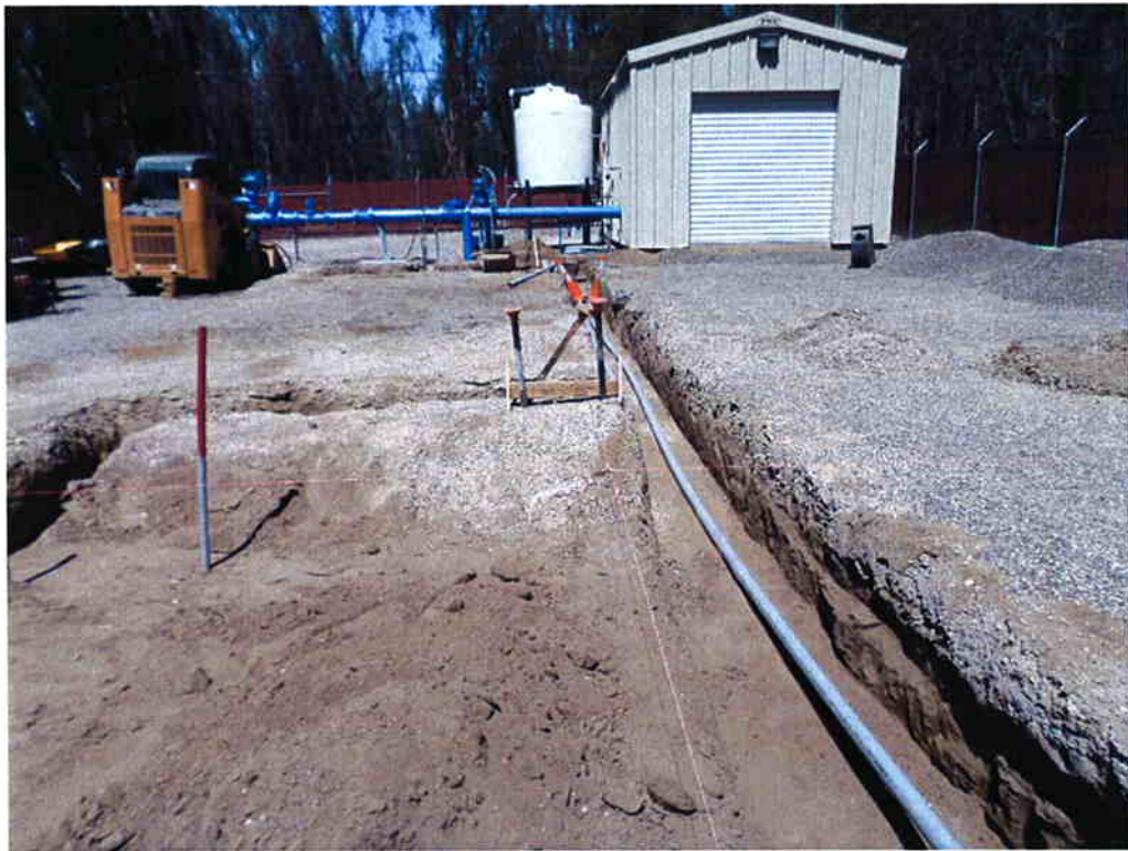
Spiess installing 2-inch PVC conduit for chemical tubing.
