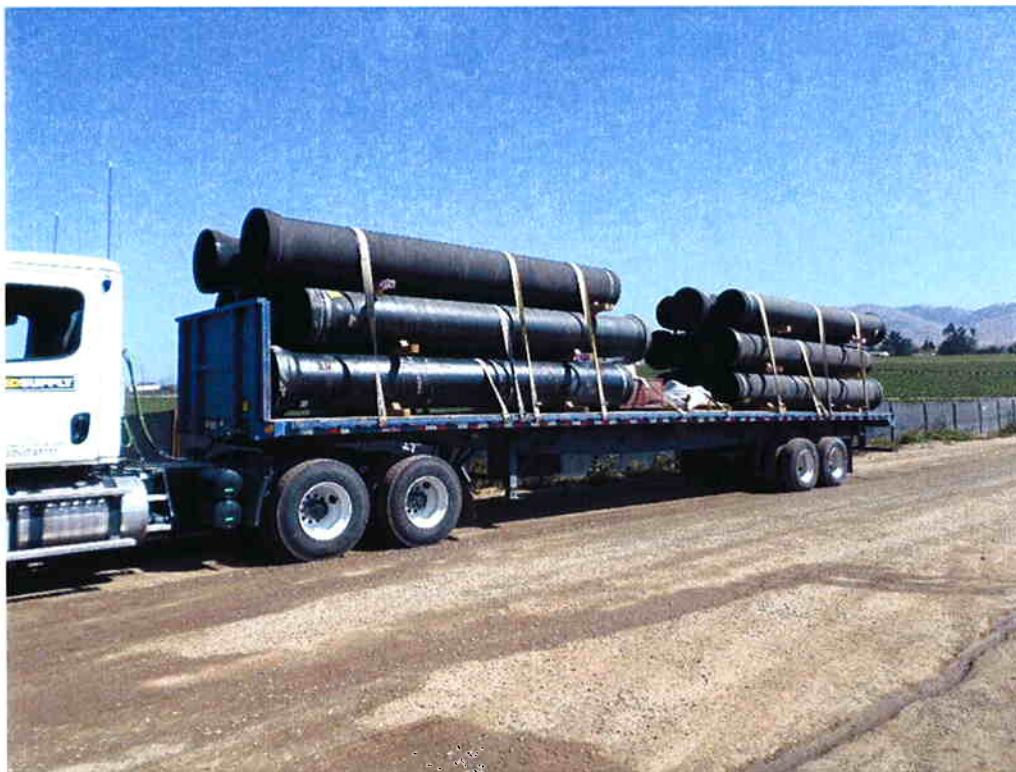
Delivery of 24-inch ductile iron pipe.
