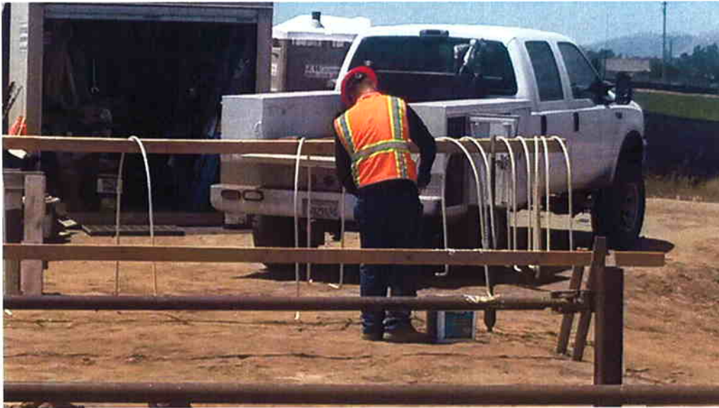
Spiess coating rebar for valve anchors.
