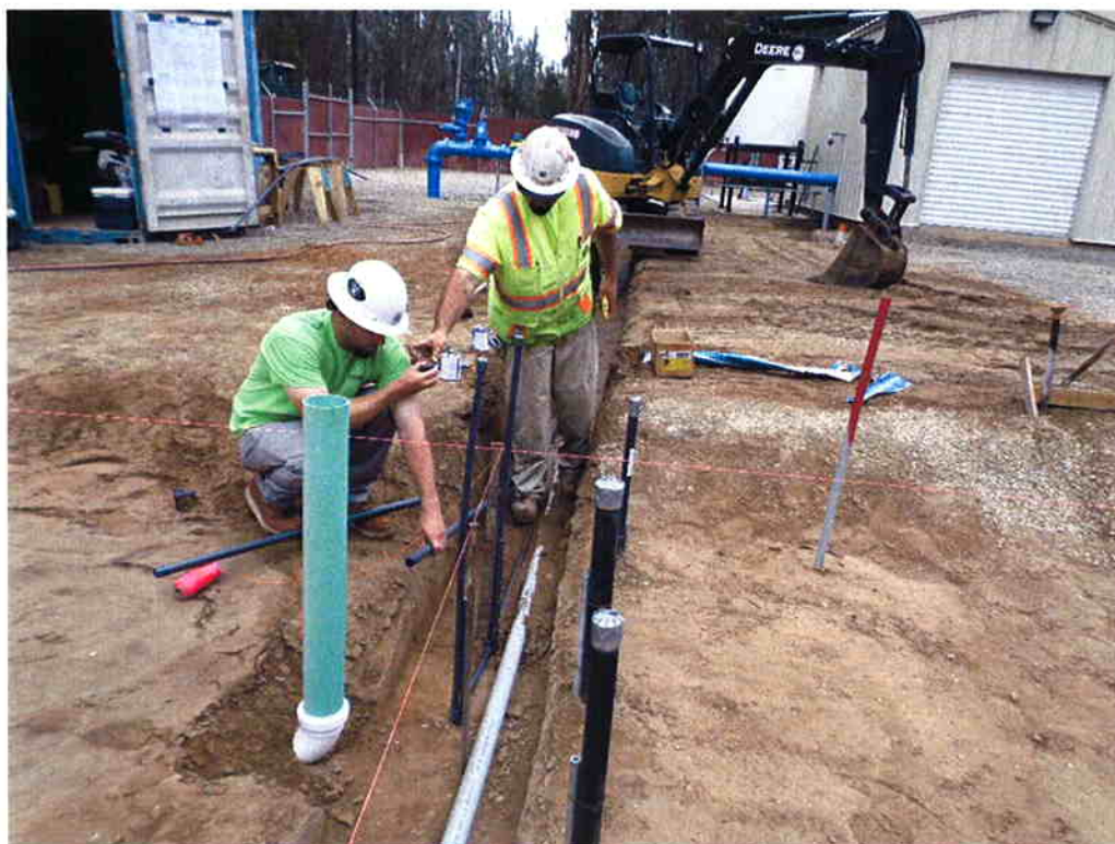
Spiess installing 1/2-inch PVC plant water line and 2-inch PVC chemical tubing line.
