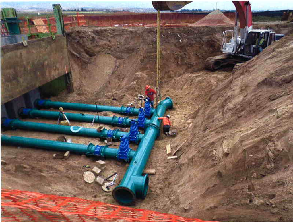
Spiess installing 24-inch manifold onto 16-inch valves.
