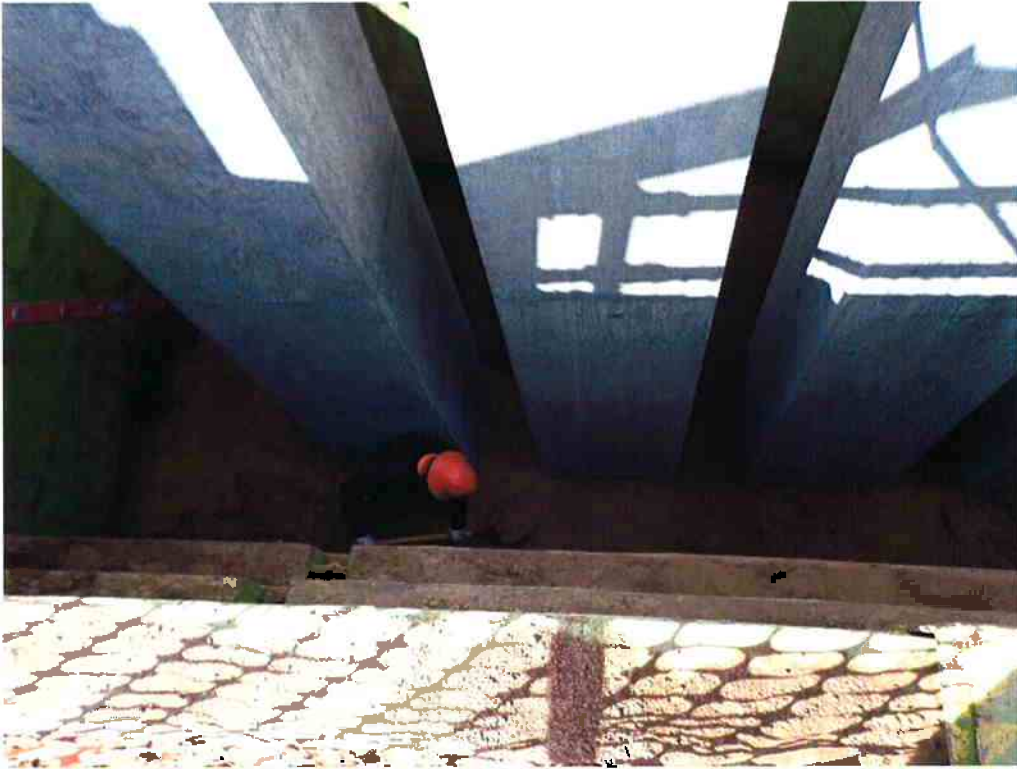
Spiess spreading native material backfill around the base of the pump cans.
