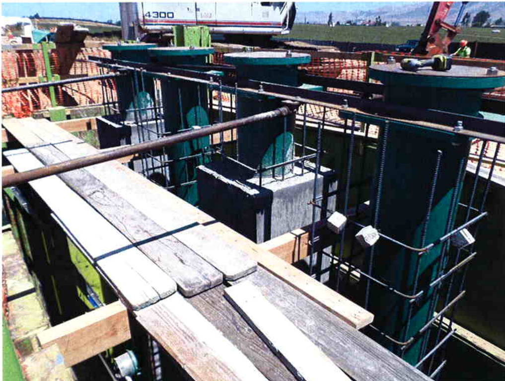
Stripping forms after first pour of encasements around pump cans.
