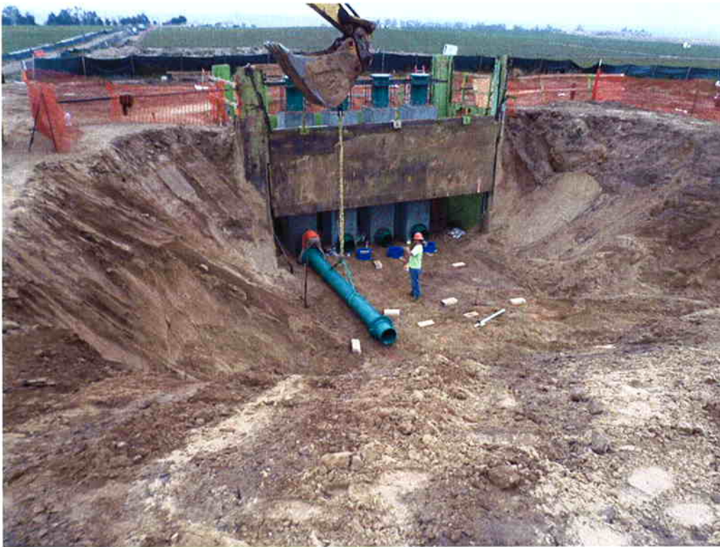
Spiess starting installation of 16-inch coated steel suction piping.
