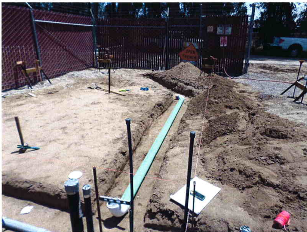
Spiess installing 4-inch PVC drain piping under the Chemical Building slab.
