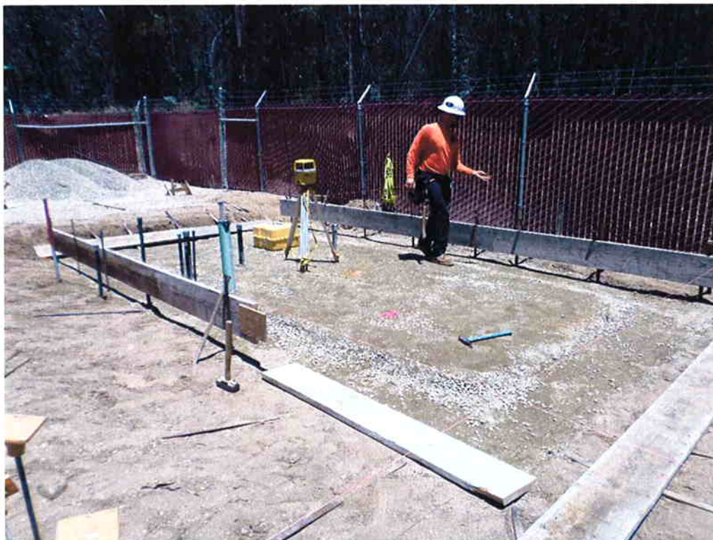
Spiess installing forms for the Chemical Building slab.
