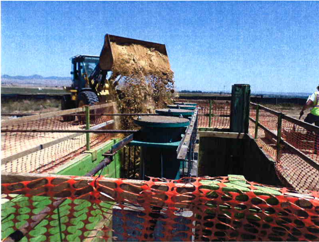
Spiess backfilling around concrete encased pump cans in order to remove some of the shoring before work on the suction pipes.
