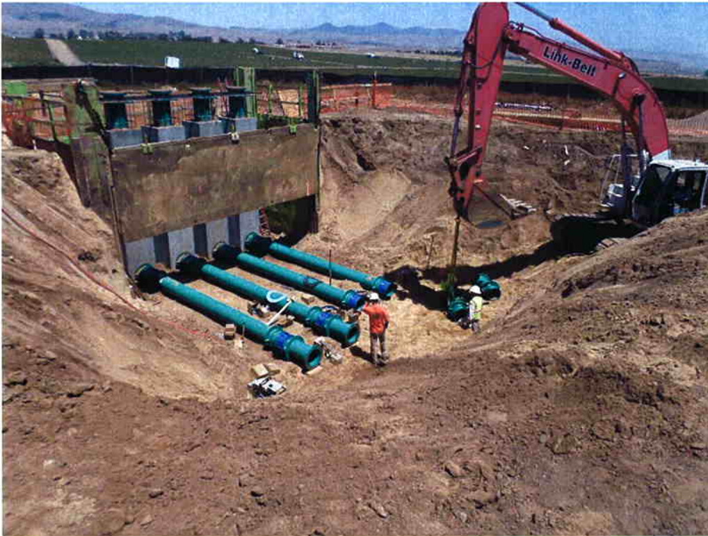
Spiess installing 16-inch coated steel suction piping and fittings.
