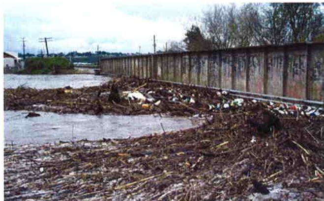
High flows and debris in Arroyo Grande Creek at the railroad bridge (1999 flood event).
