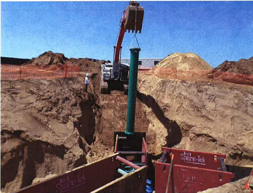
Spiess setting the pig launcher riser.
