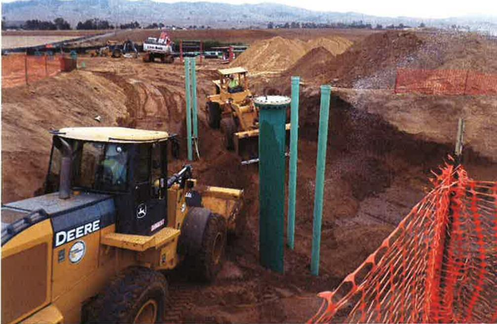
Spieß backfilling around installed valve can risers.
