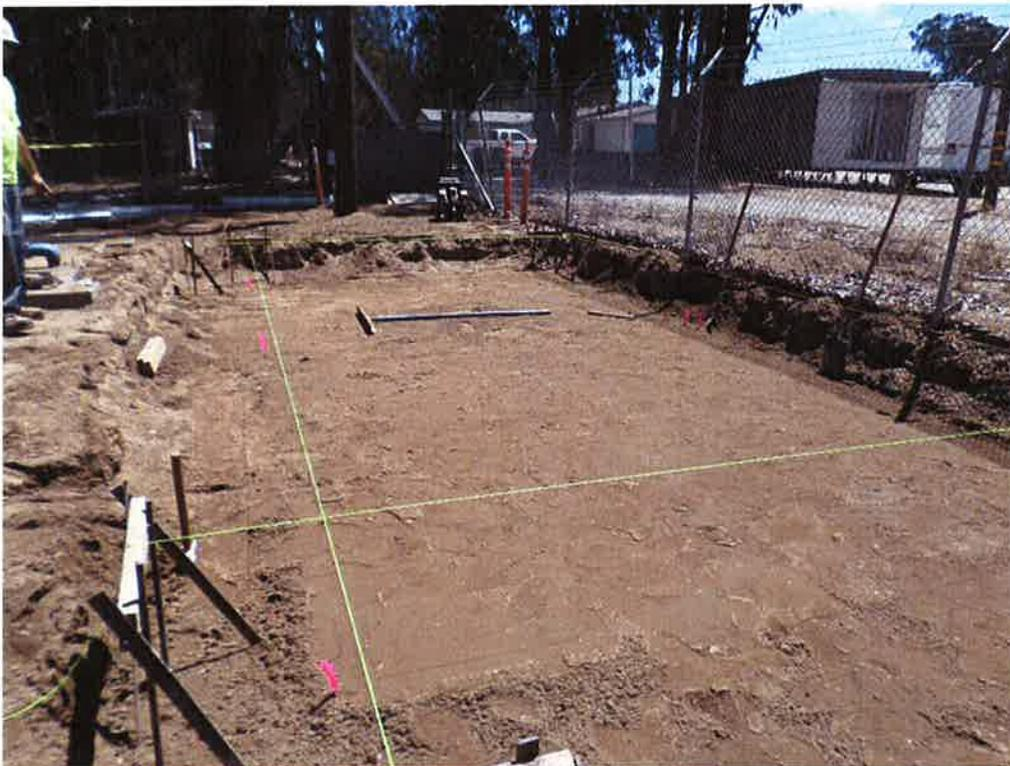
Laying out the chemical building slab foundation.
