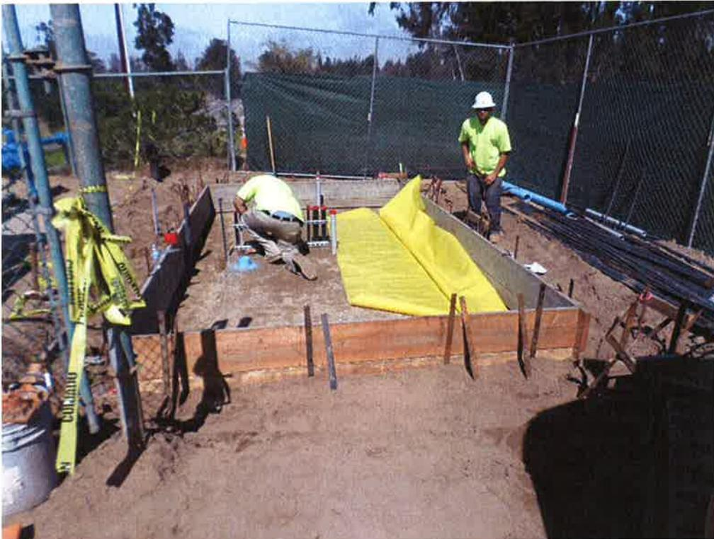
Spiess installing underslab vapor barrier.
