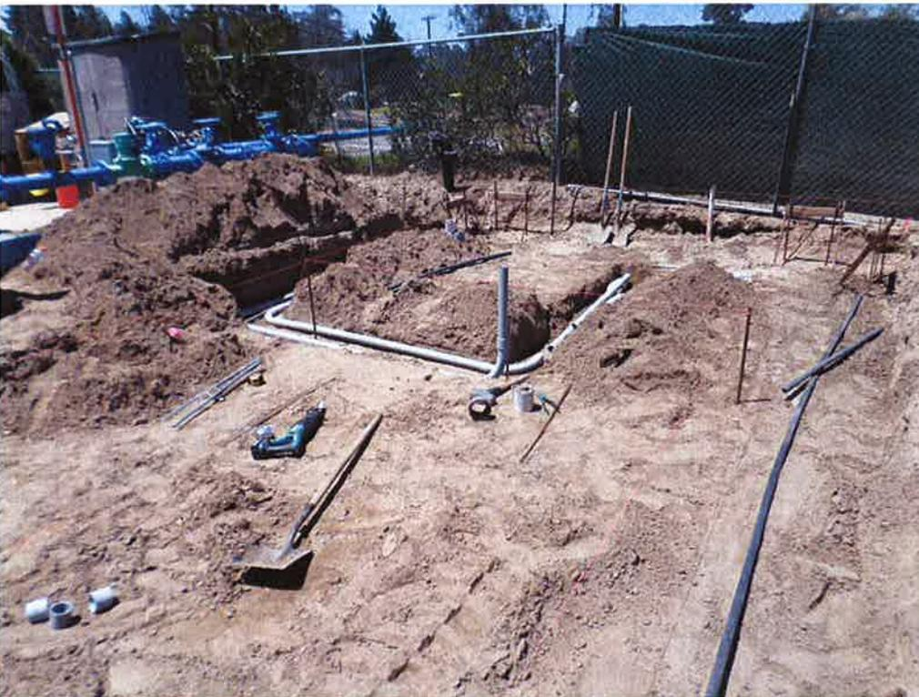
Spieß installing underslab piping.
