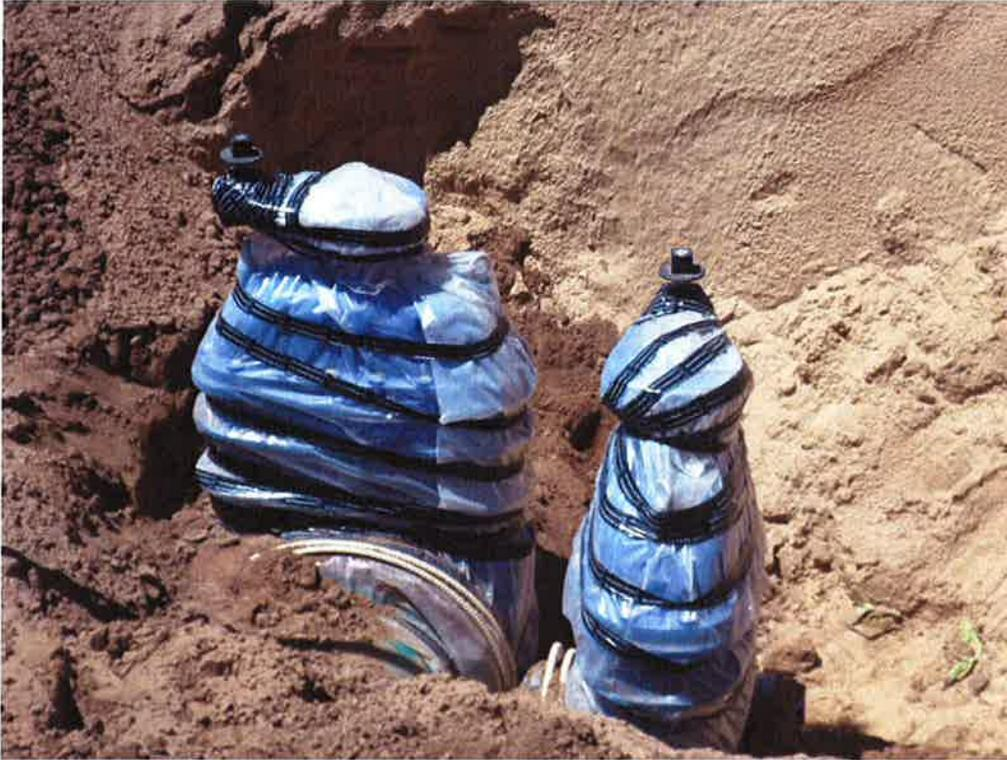
Spiess wrapping valves with plastic before backfilling.
