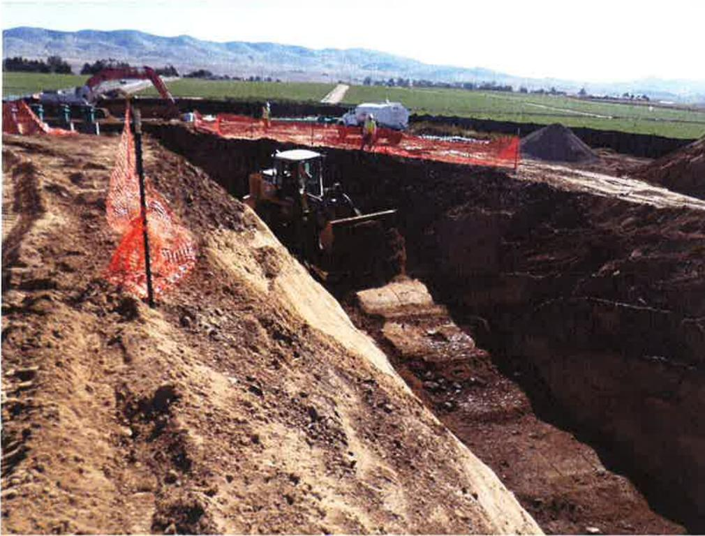
Spiess backfilling over 24-inch DIP.
