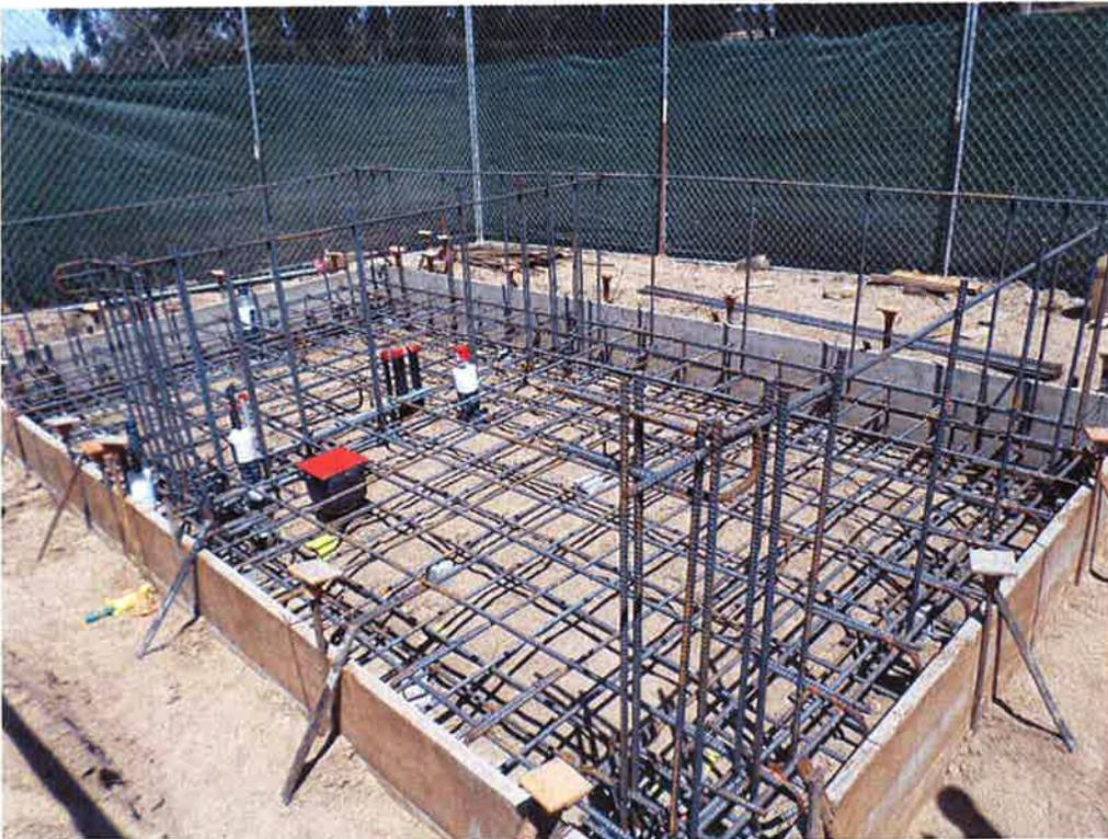
Reinforcing installed for chemical building slab.
