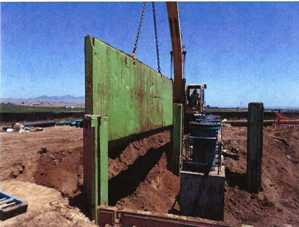
Removing shoring from around the pump cans.
