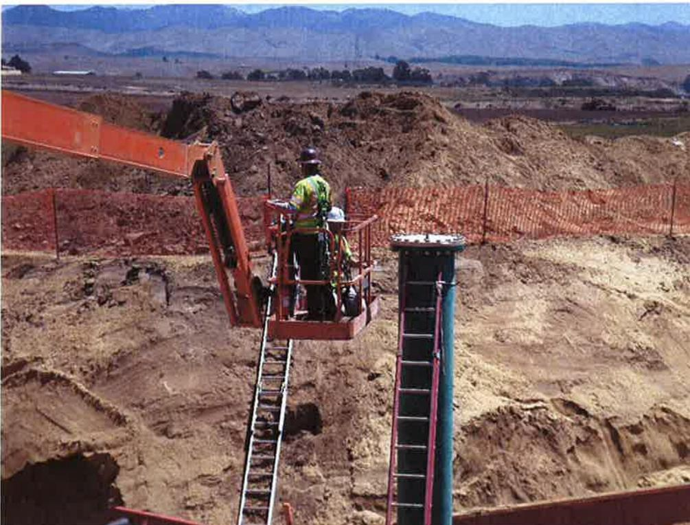
Spiess tightening bolts at the top of the pig launcher riser during pressure testing.
