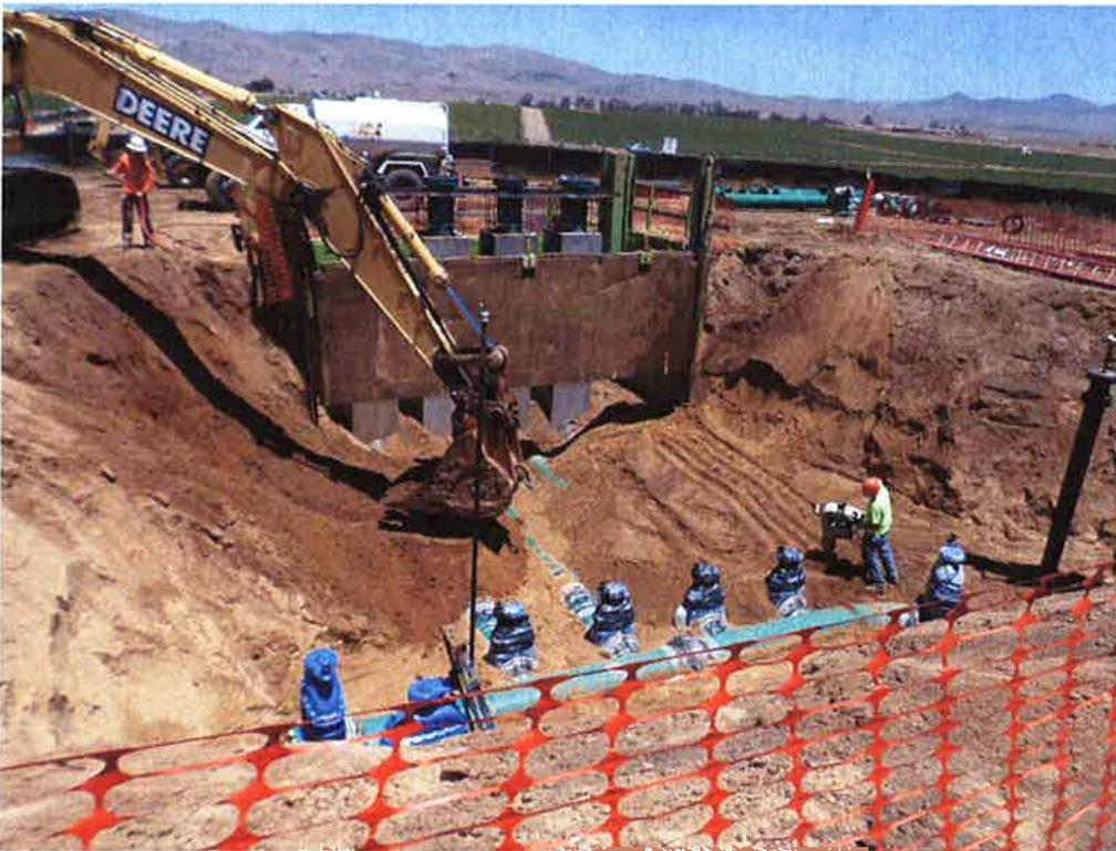
Spiess continuing backfill and compaction over inlet piping.
