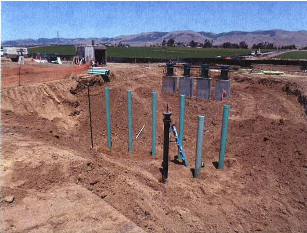
Spieß installing valve can risers on inlet manifold.
