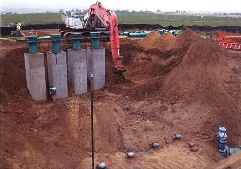
Spieß continuing backfill around the pump cans.
