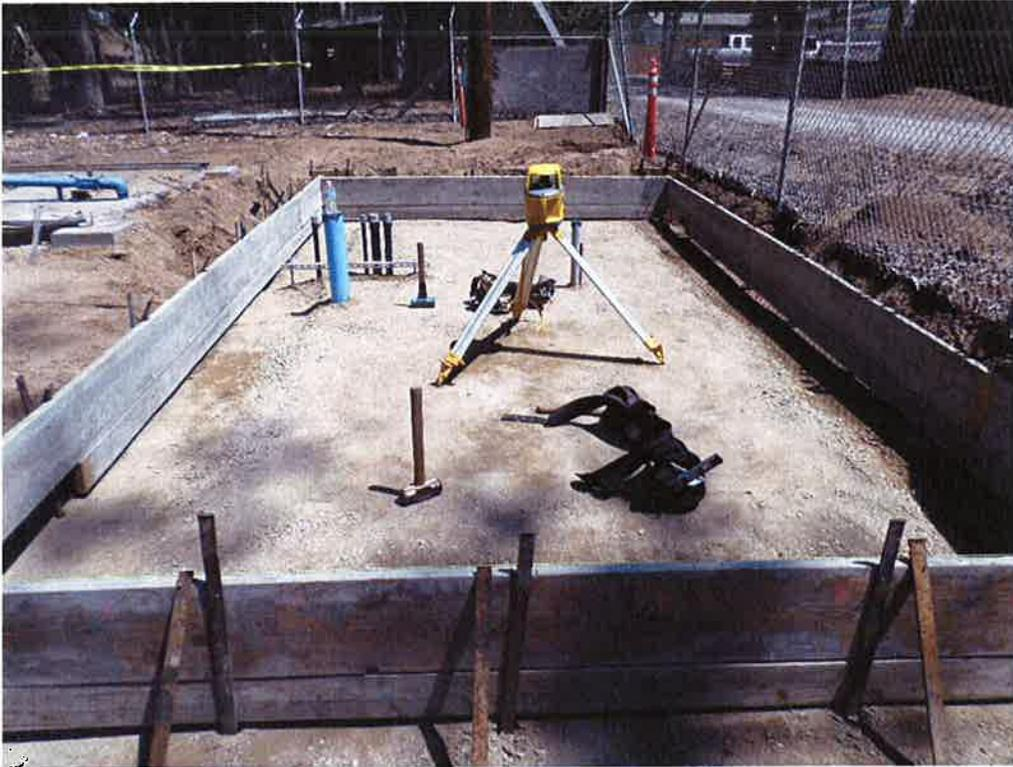
Forming the chemical building slab foundation.
