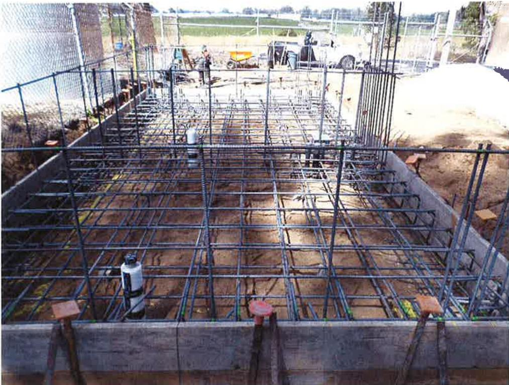
Chemical pad reinforcing installed by Vista Steel.
