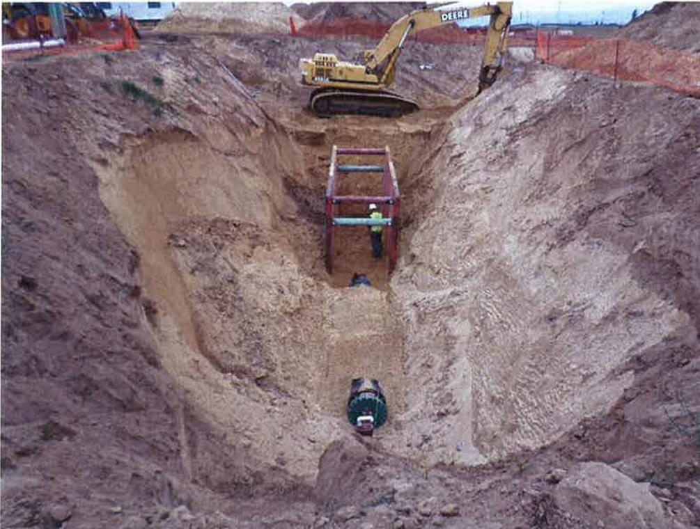
Spies continuing installation of 24-inch DIP from the future connection point at the HDPE pipe to the pump station inlet manifold.
