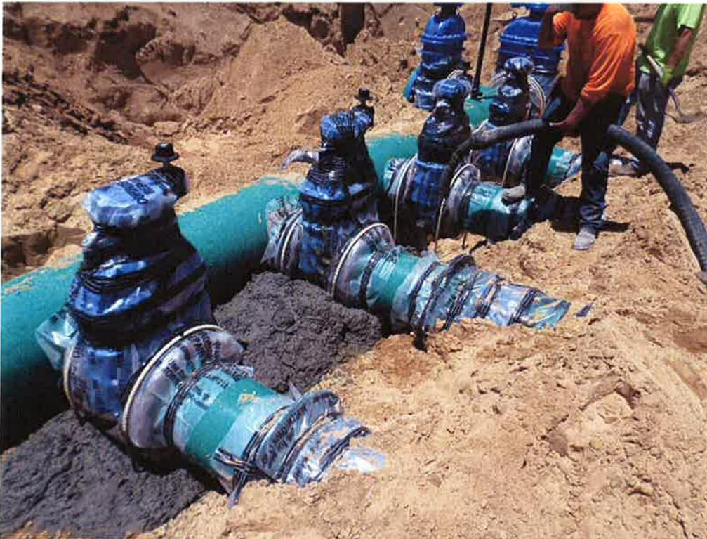
Pouring concrete valve anchors on inlet piping.
