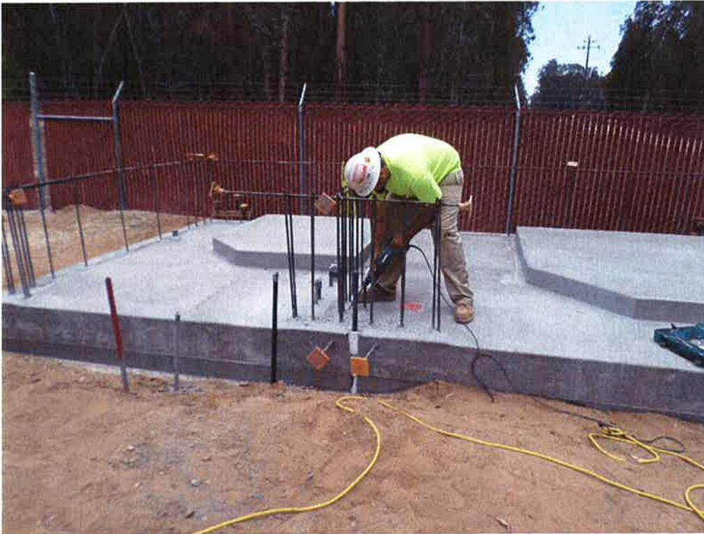
Spiess roughening concrete on building slab in preparation for placement of the concrete block.
