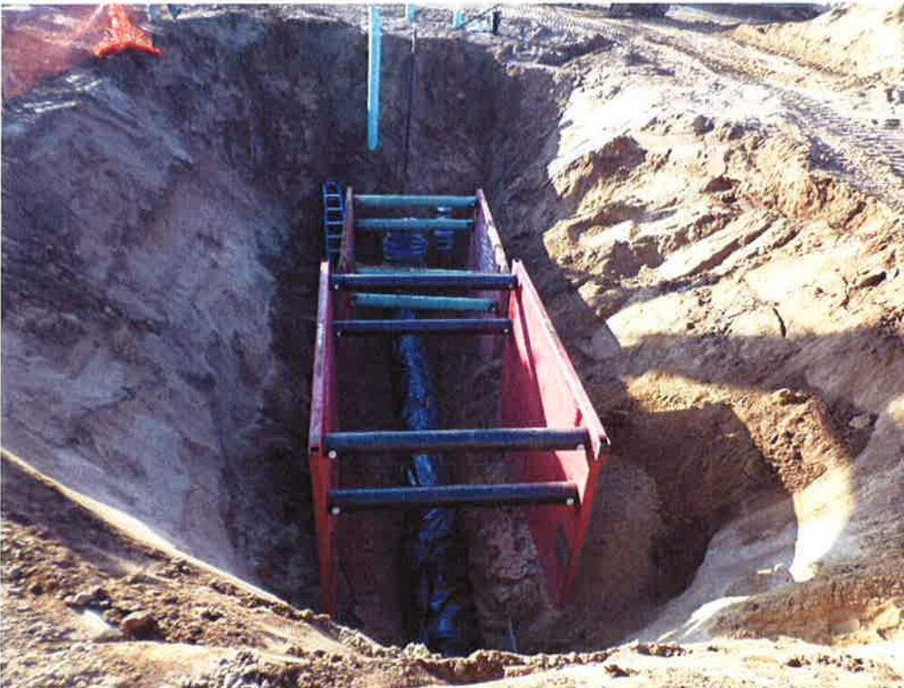
Spieß installing pipe extension to future tank outlet piping.
