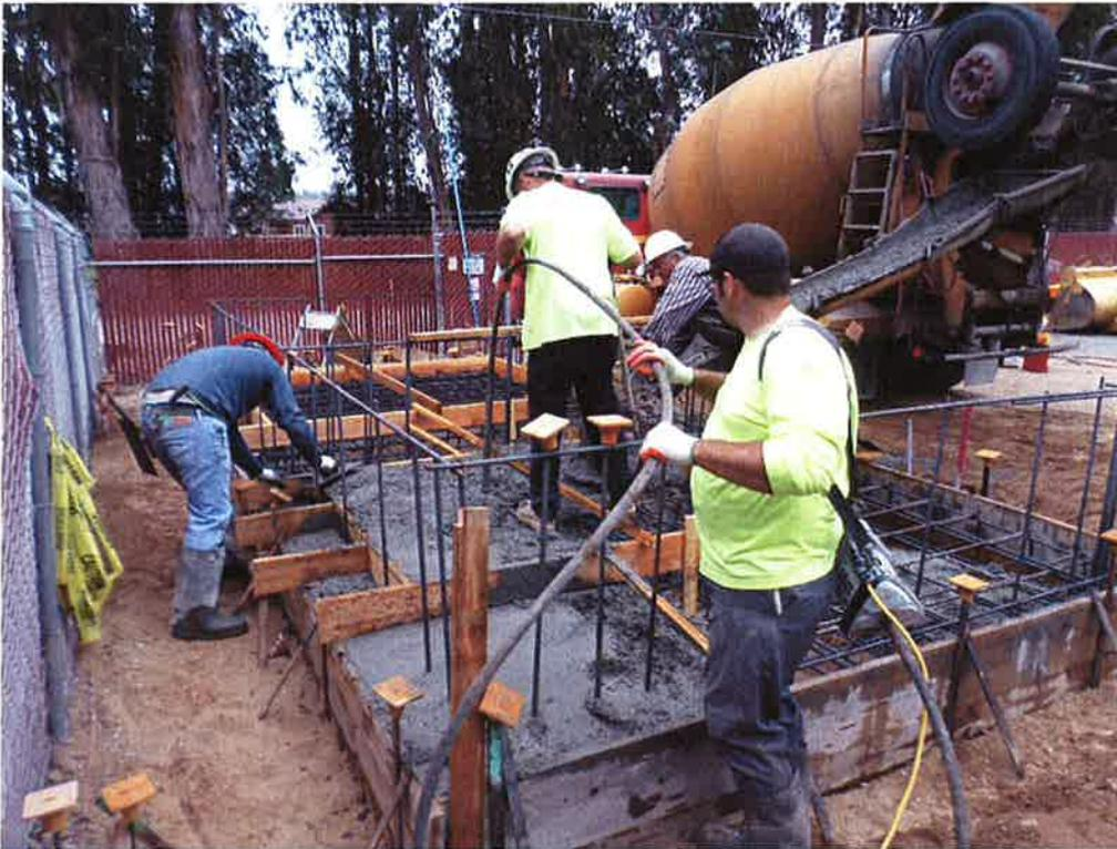
Spiess placing concrete for chemical building slab.
