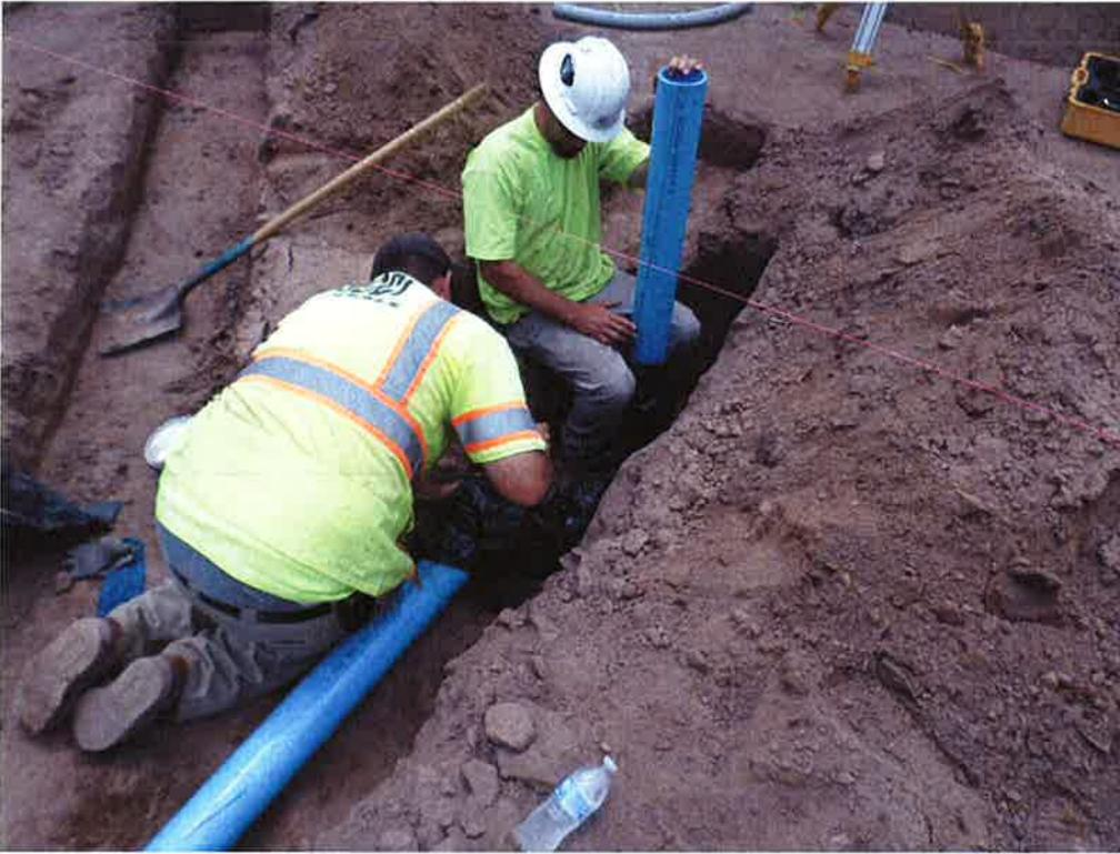
Spiess installing 4-inch drain line.
