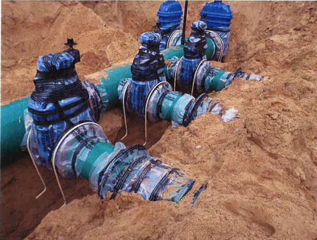
Spies excavating for concrete blocks and placing epoxy rebar anchors over valves on inlet piping.
