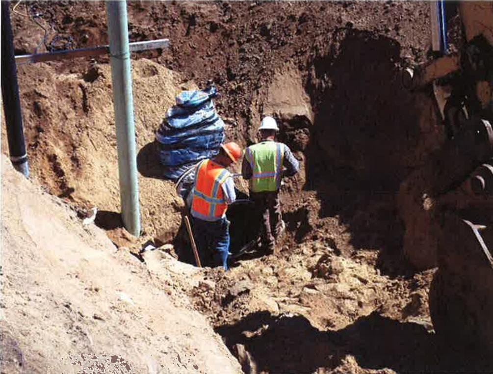
Spieß installing flange adapter on 24-inch DIP.
