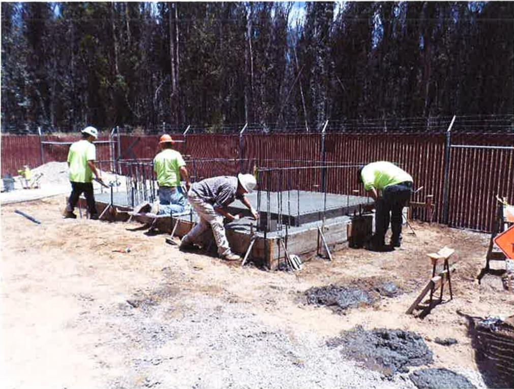
Spiess finishing concrete at chemical building slab.
