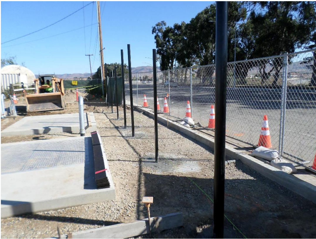
Post for new perimeter fence installed around metering vaults.
