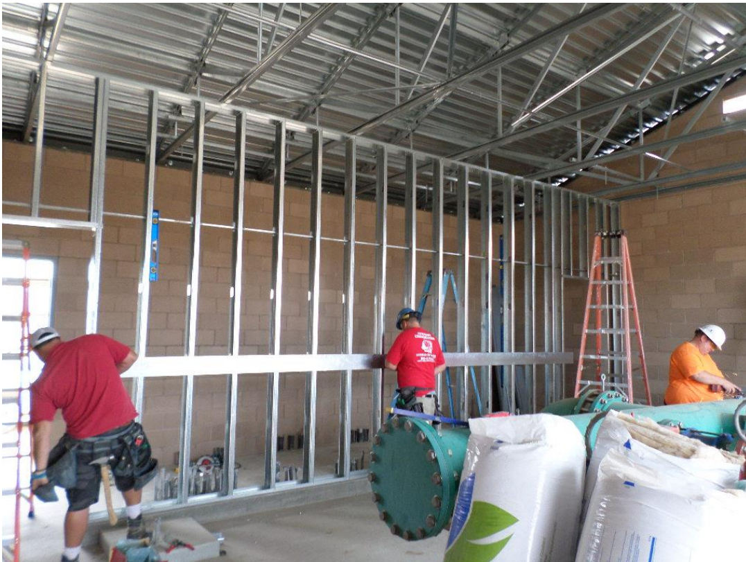
Ely Dodson Construction installing interior steel stud wall at pump station.
