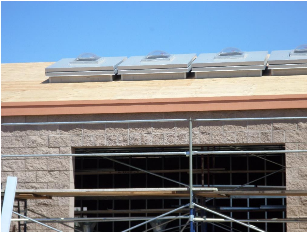
Coast Painting applying coating to fascia at pump station building.
