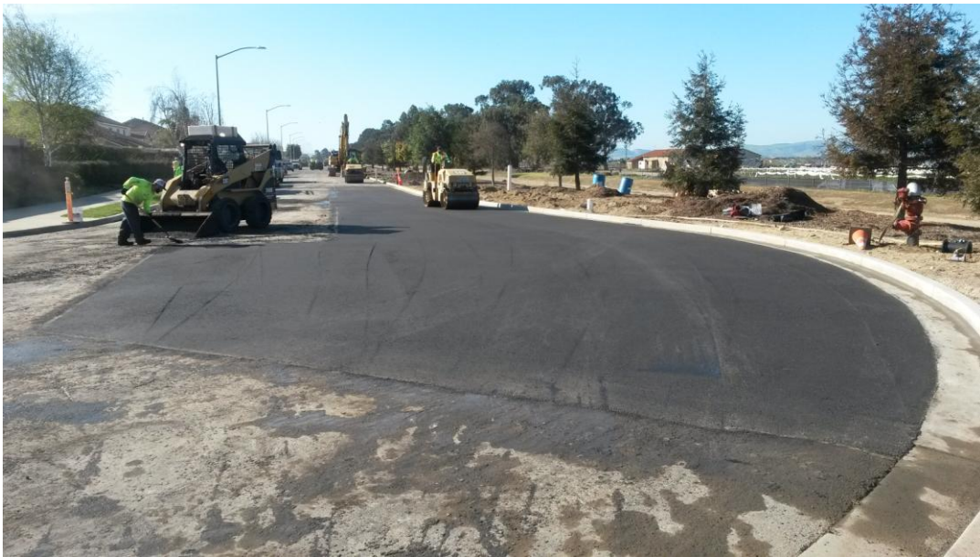
Ramsey Asphalt completing final paving at Blosser and Atlantic.
