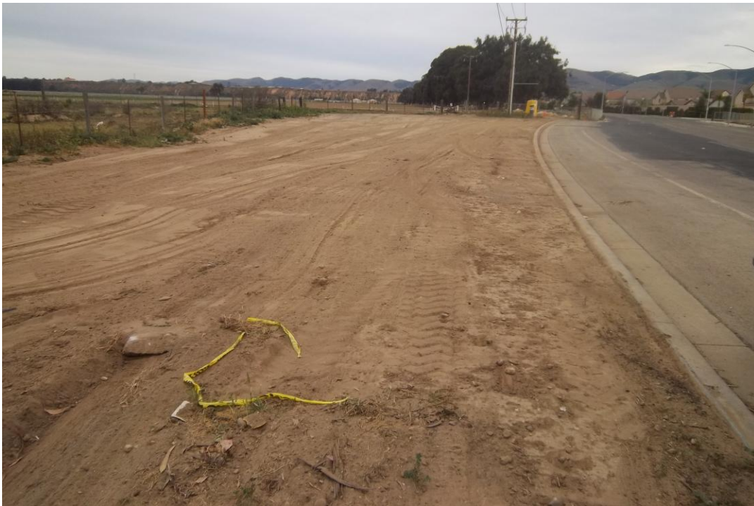
Staging area being cleaned up and regraded.
