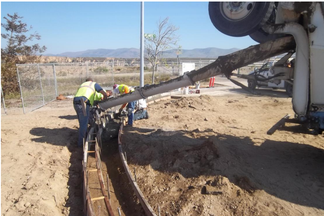
D-KAL pouring curb and gutter.
