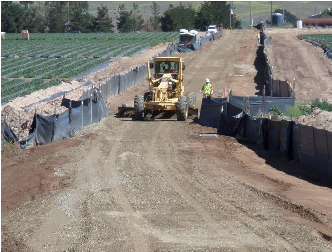
Spiess grading the permanent access road.
