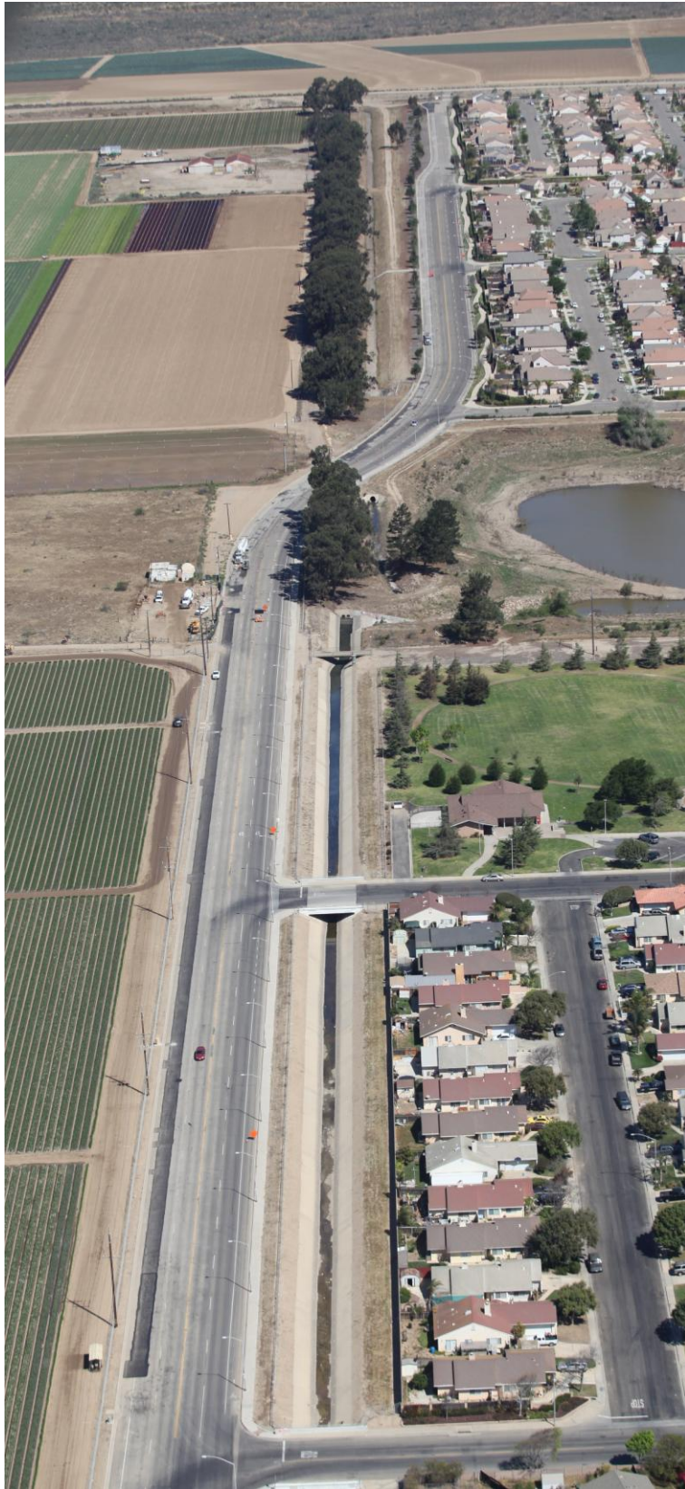
Entire length of Blosser Road Water Main completed. Ramsey Asphalt grinding and oiling trench paving near Blosser Flow Meter Vaults.
