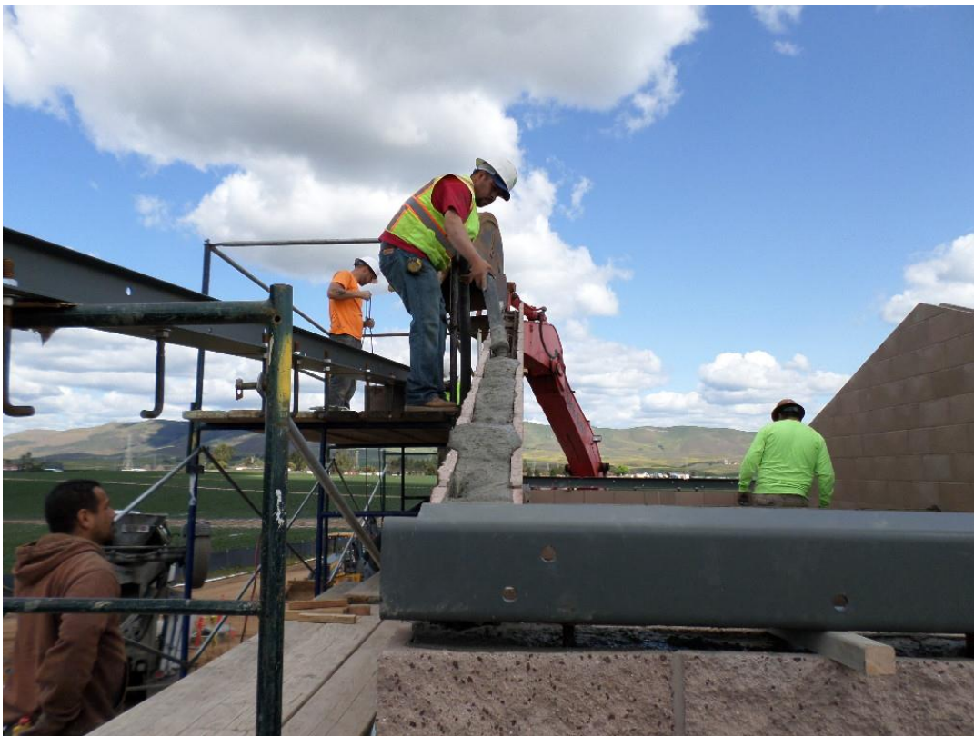
Spieß setting steel roof plates during final wall grout.
