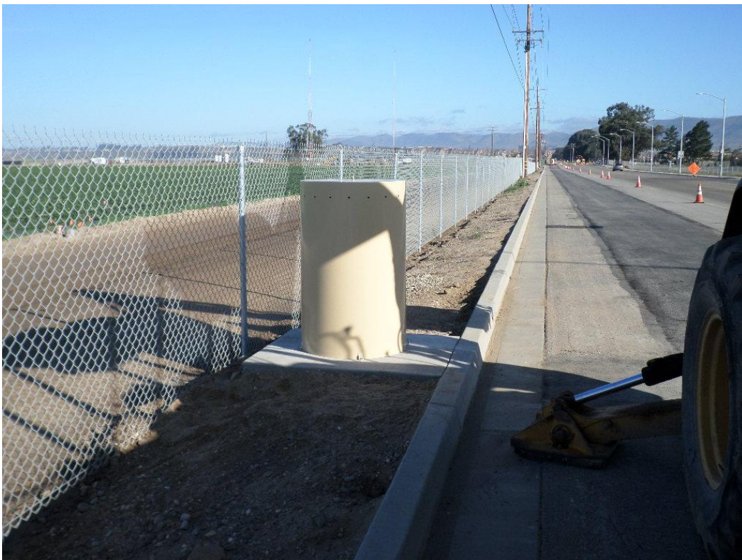
Enclosure installed over CAV.
