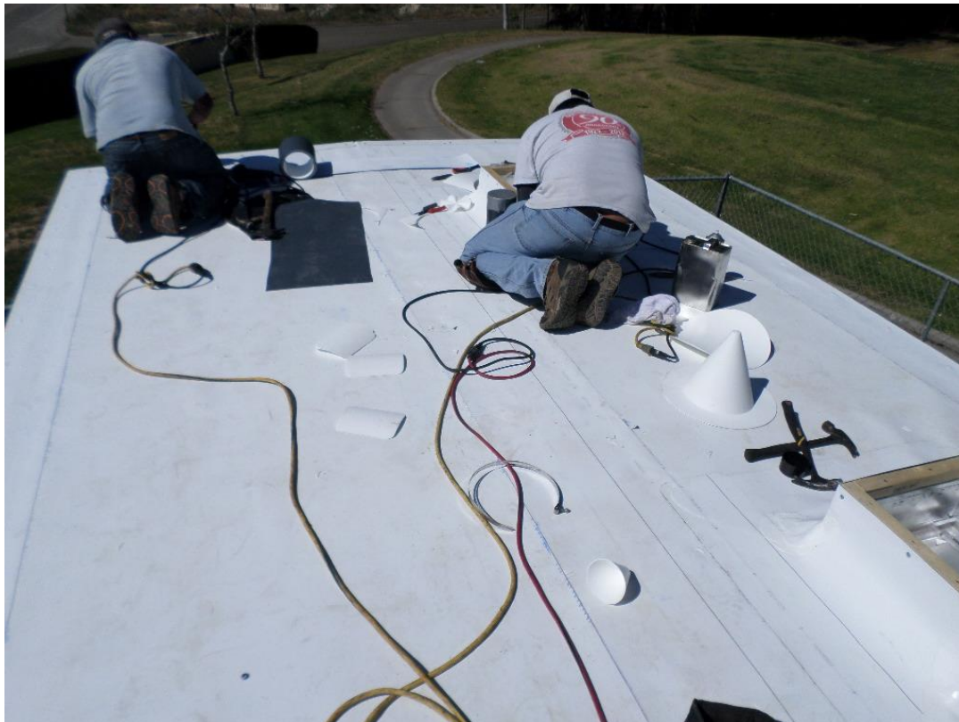
Quaglino Roofing installing roof membrane.
