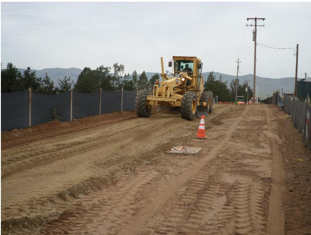
Spies placing base to construct permanent access road.
