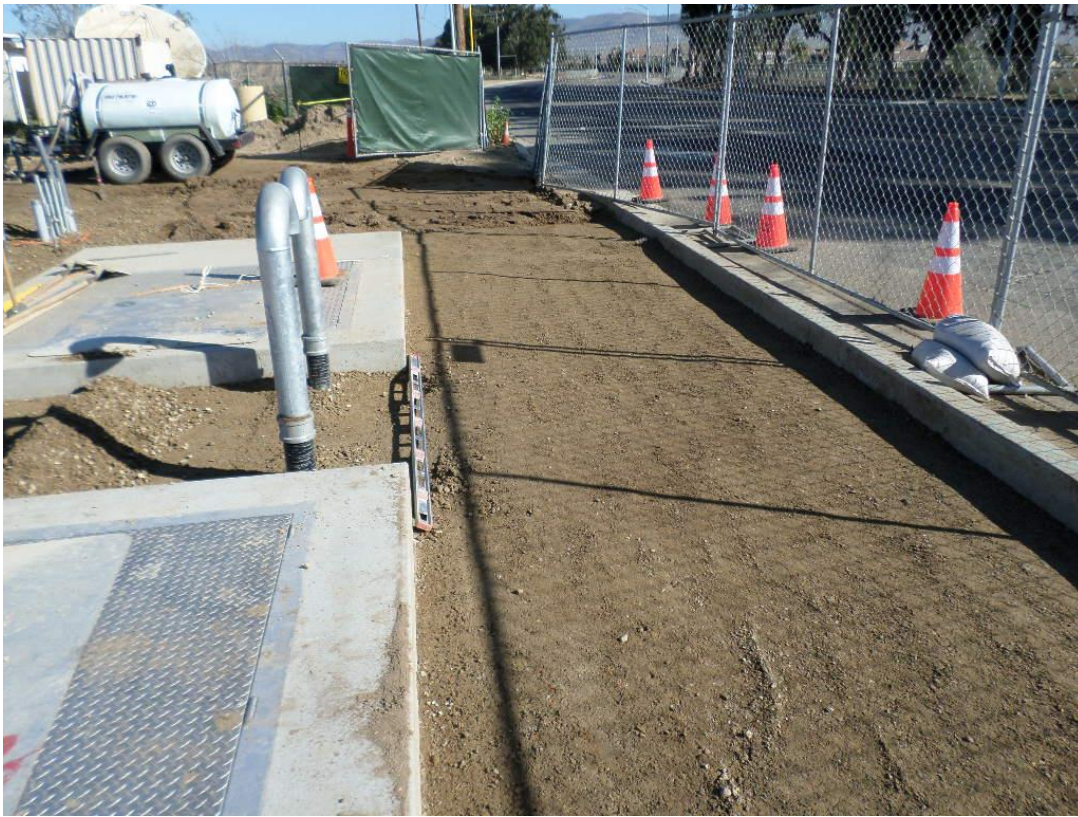
Placing base material around metering vaults.
