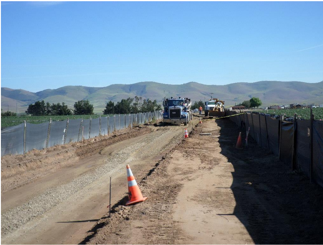
Base delivered for construction of permanent access road.
