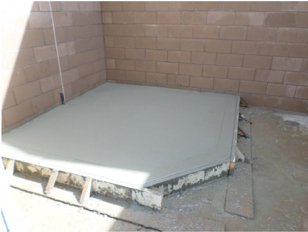
Chemical tank pad in Sodium Hypochlorite Room poured.
