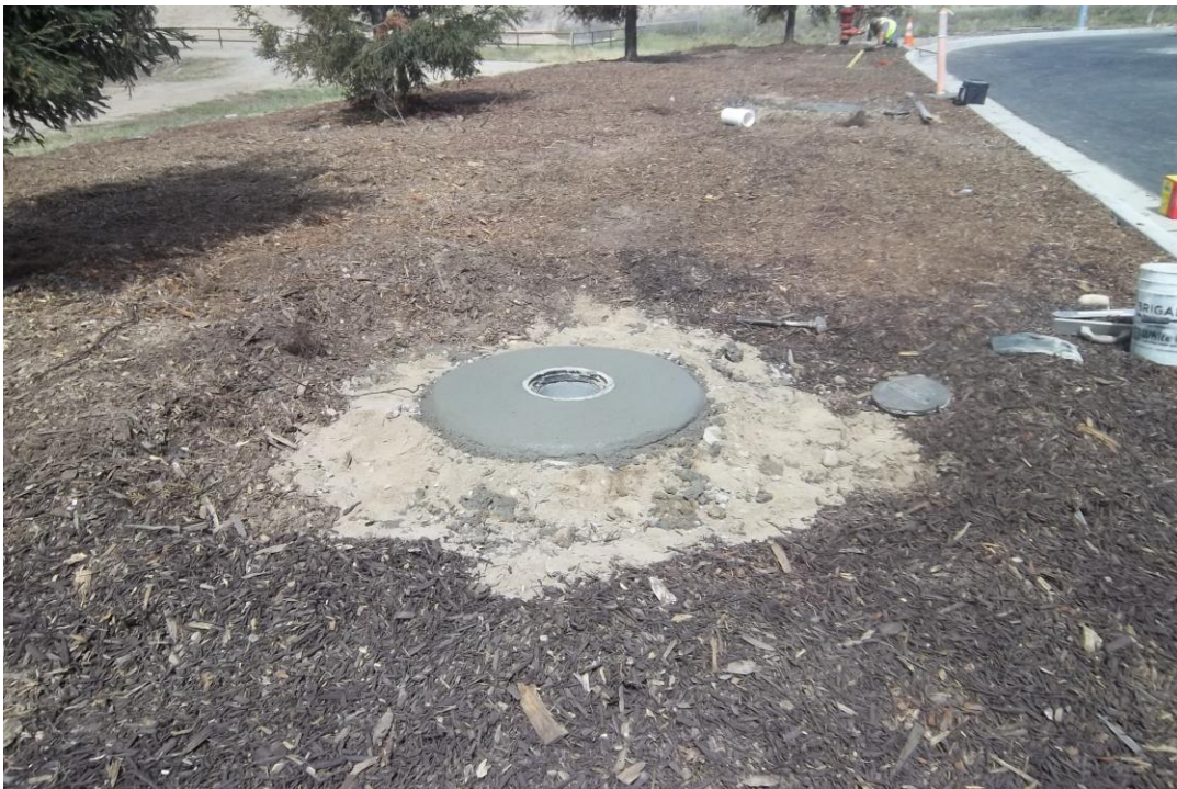
D-KAL finishing concrete collar at pig launcher.
