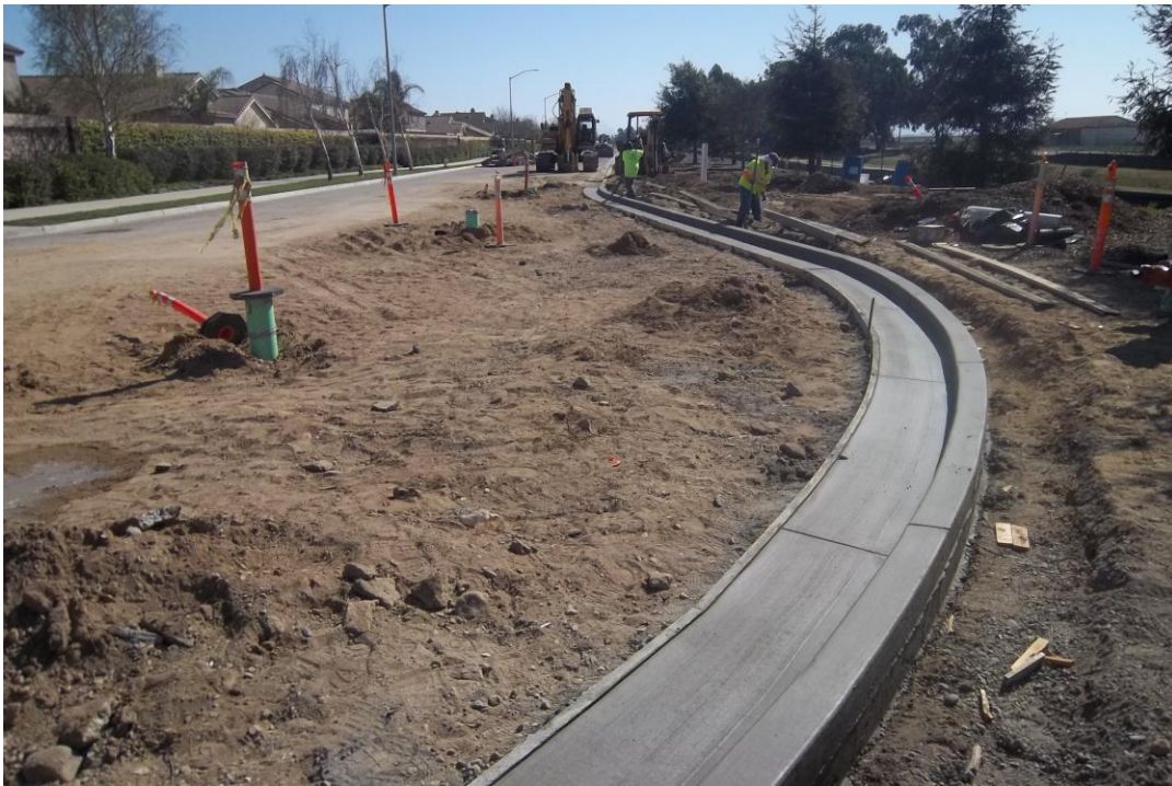
Curb and gutter replacement poured at Blosser Road and Atlantic Place.
