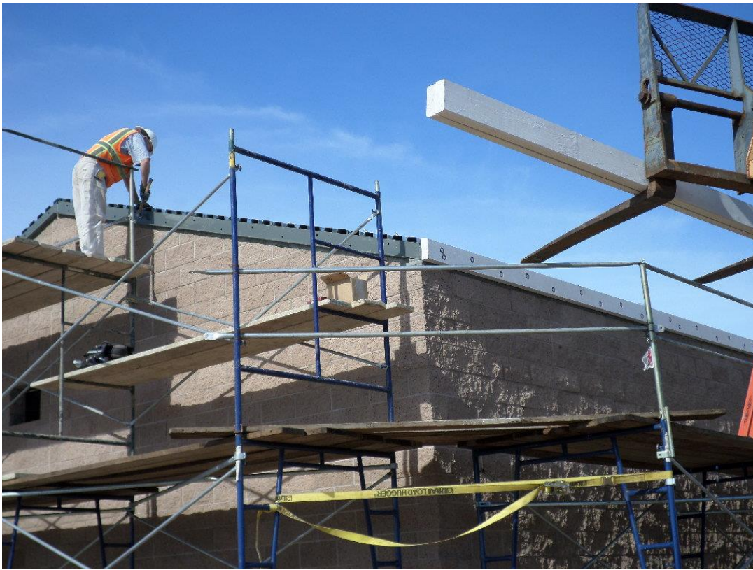
Spiess installing fascia backing.
