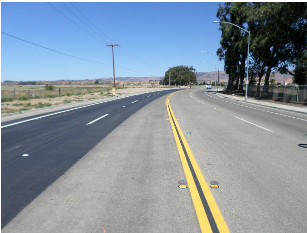
Blosser Road with project completed.
