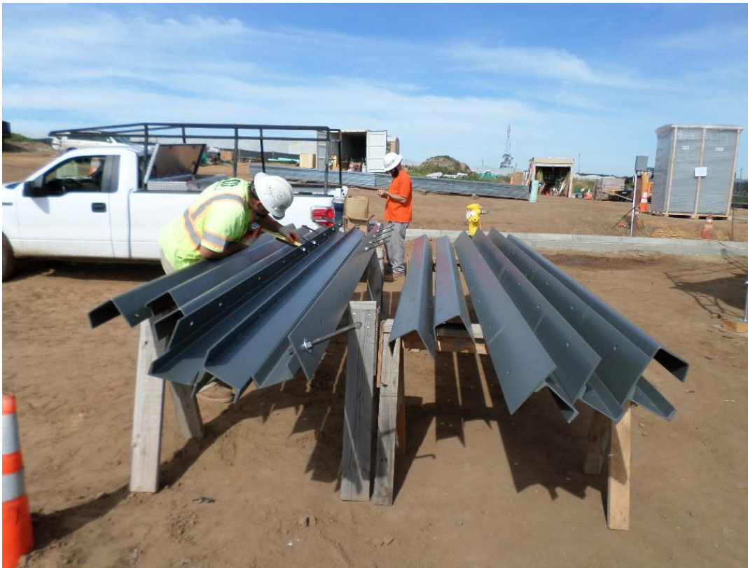
Spiess attaching bolts to roof steel plates.
