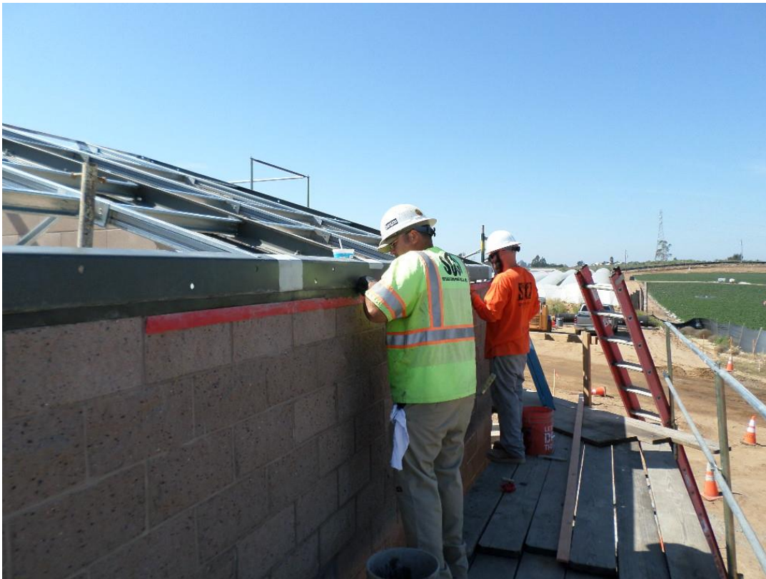
Spies dry packing grout under steel roof frame plate.
