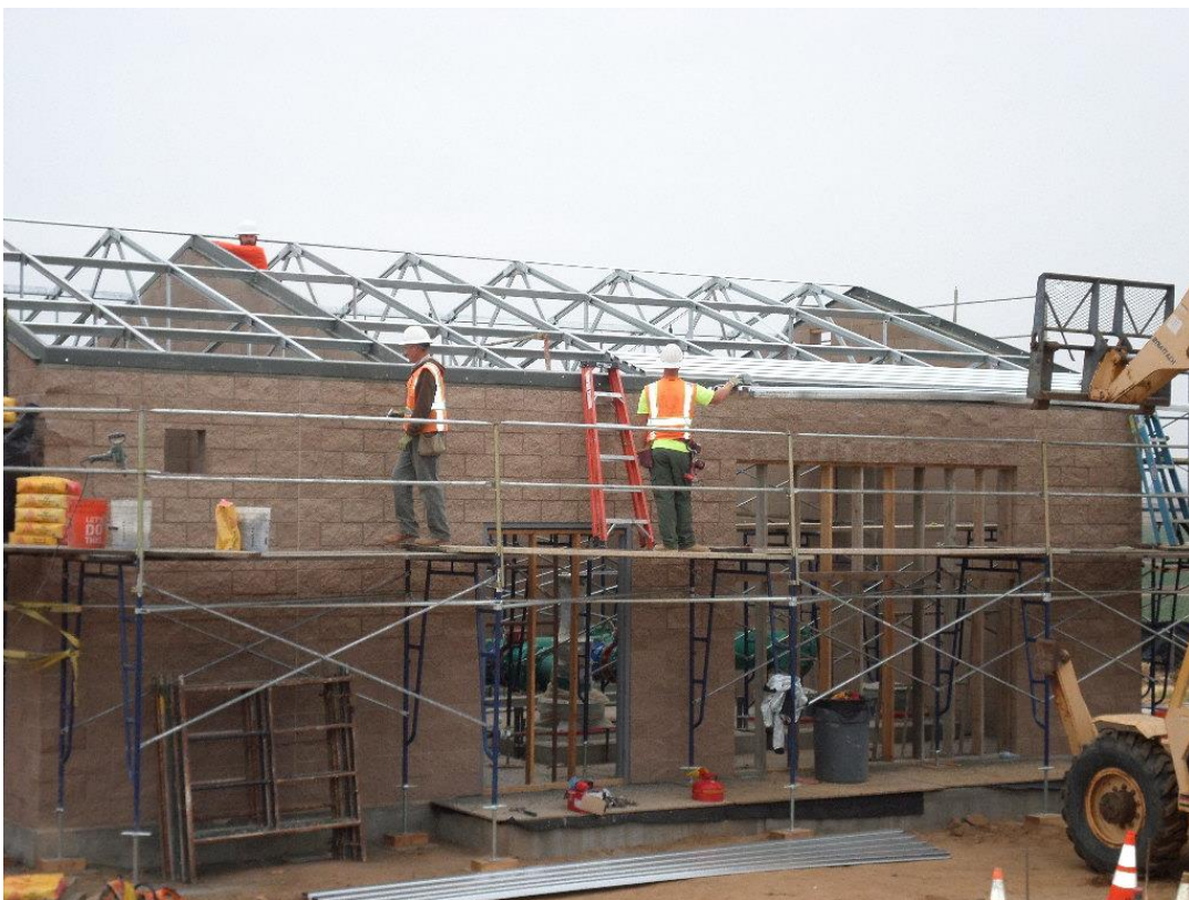
Spies installing the steel deck for the roof.
