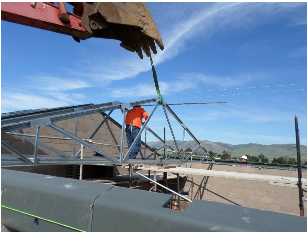
Spieß setting trusses at pump station.
