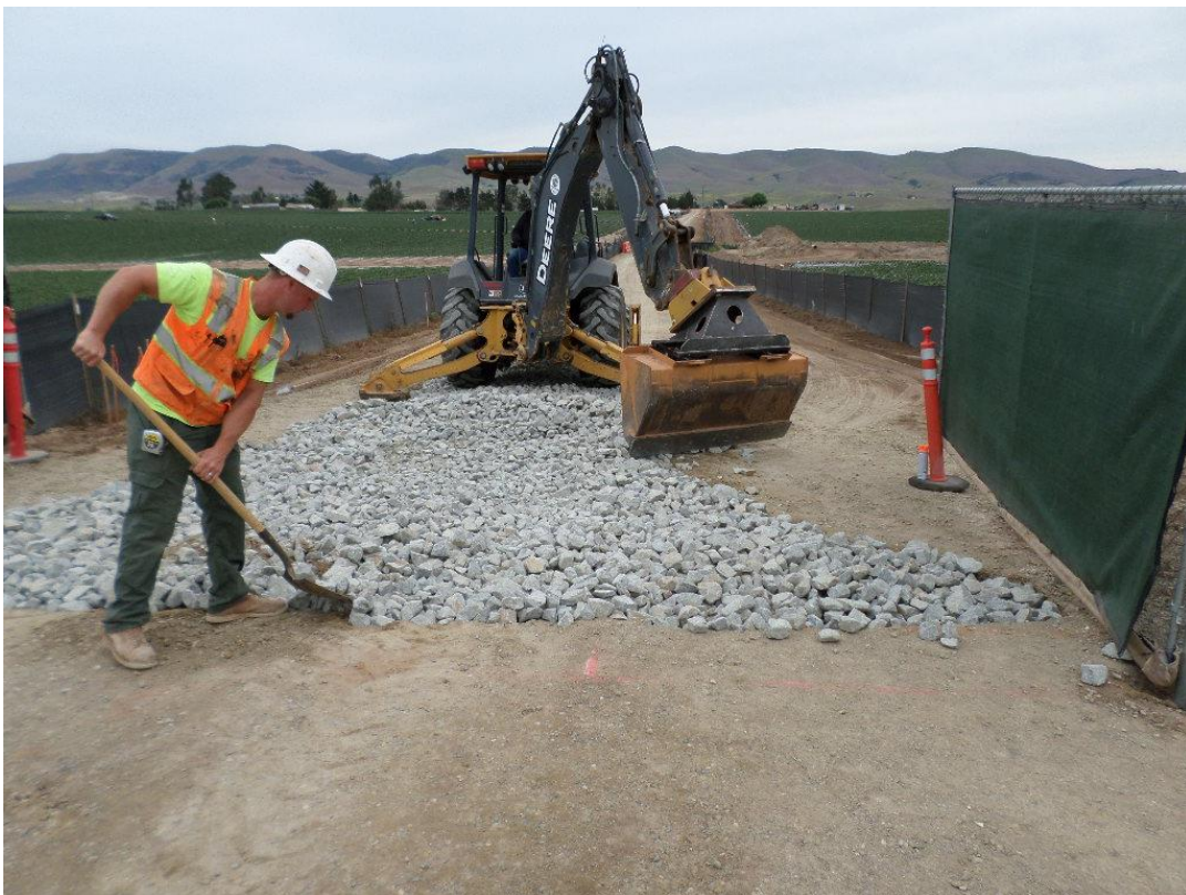
Spiess installing tracking control at relocated site entrance.
