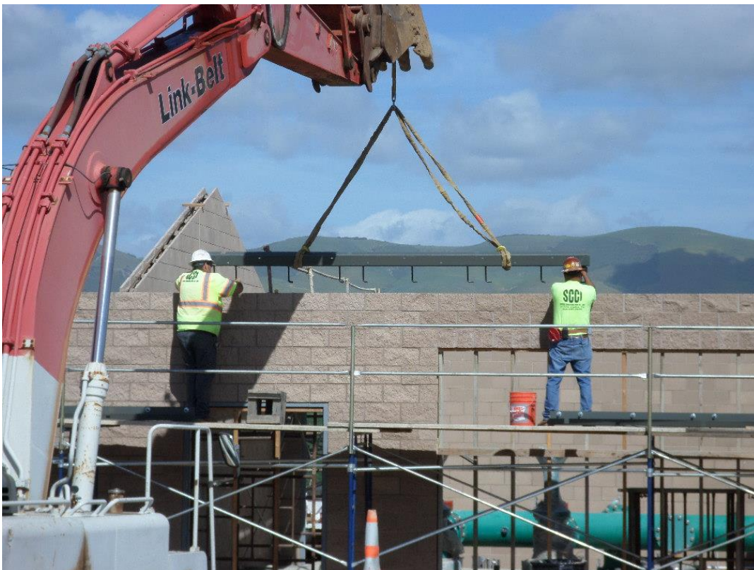
Spiess verifying hold down bolt locations prior to final grouting.
