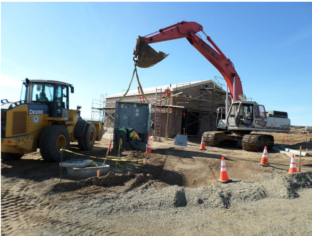
St. Denis Electric installing PG&E metering station.
