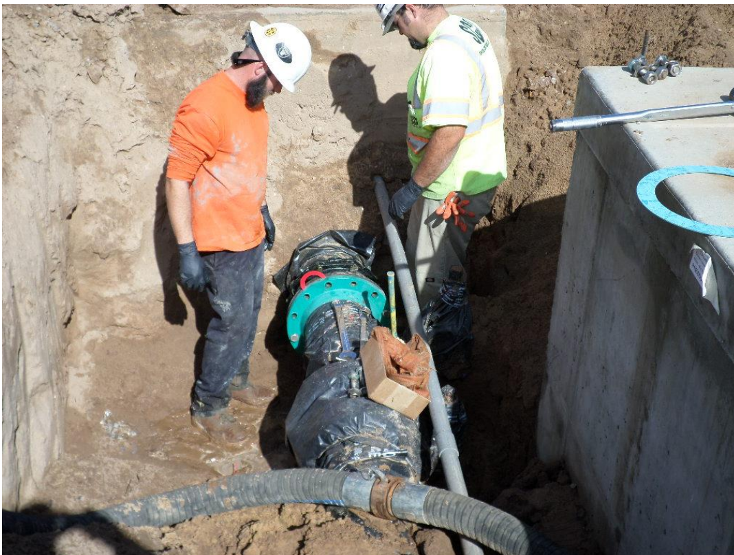
Spieß removing the test plate from piping at the PRV vault.
