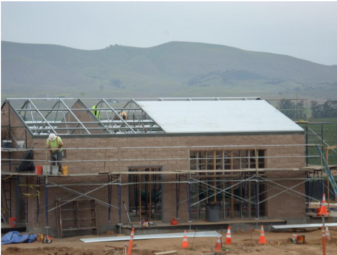
Spieß installing the steel deck for the roof.
