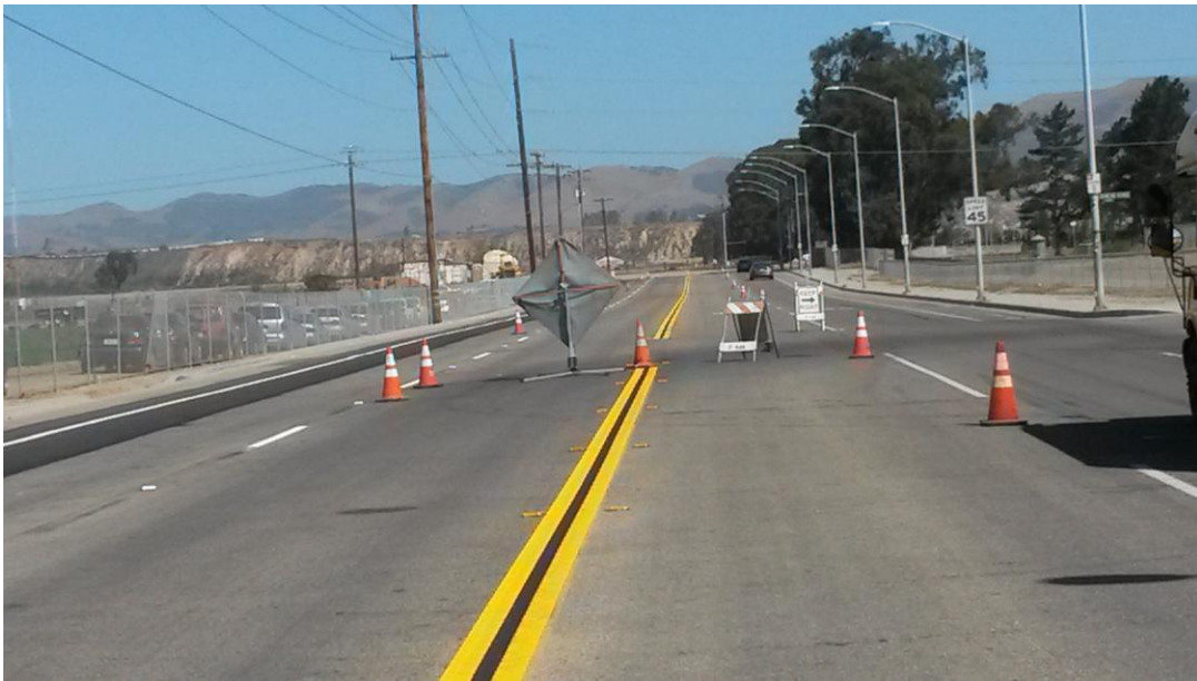
Traffic control during restriping.
