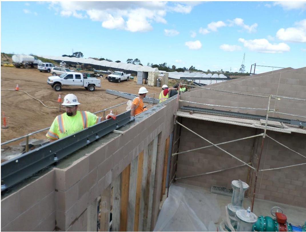
Spieß setting steel roof plates in grout.
