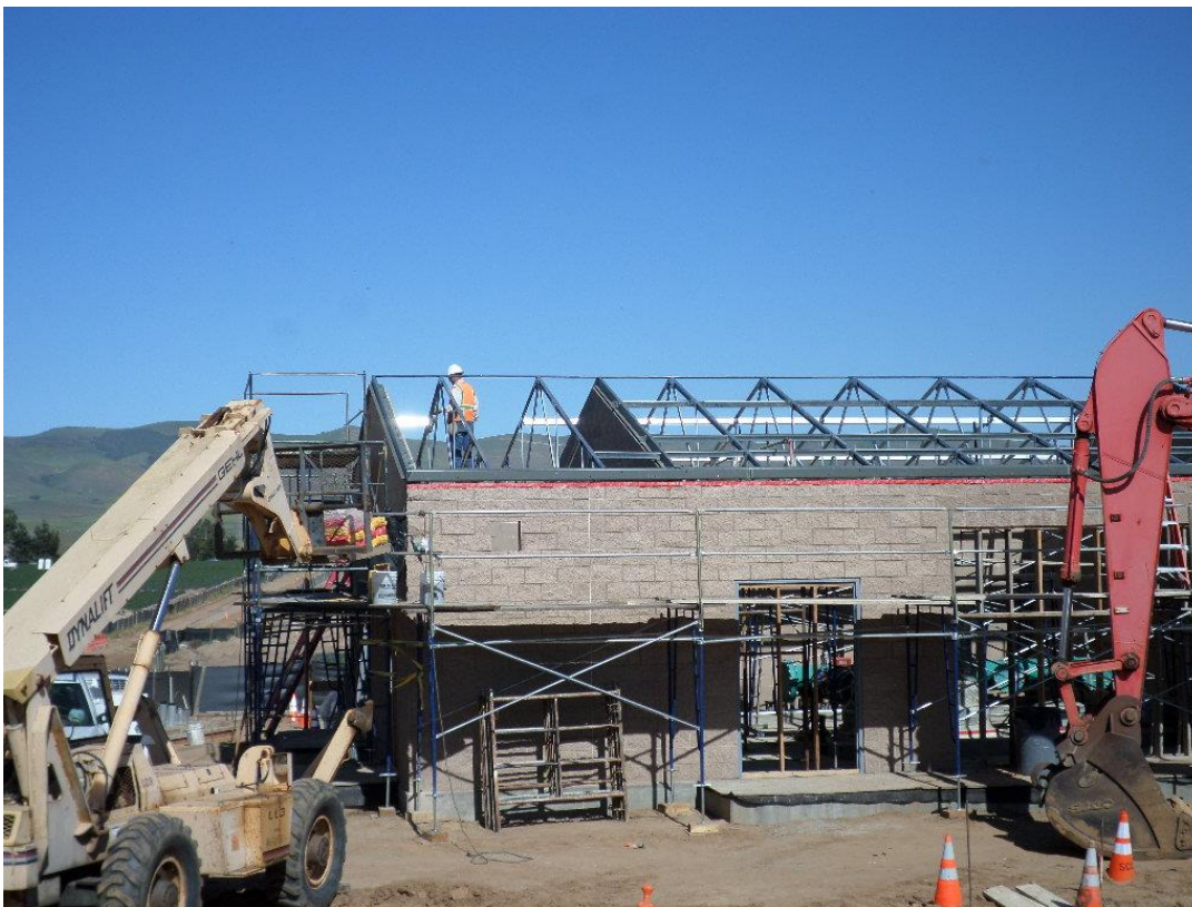
Spiess installing truss framing.
