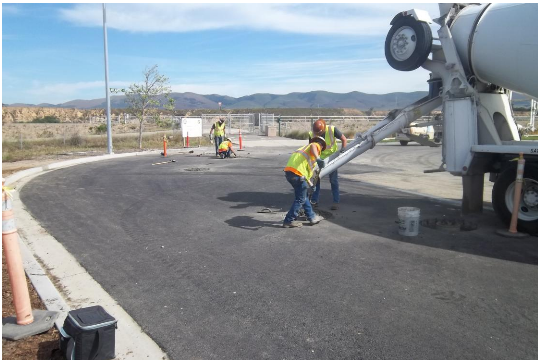
D-KAL pouring concrete collars around valve cans.
