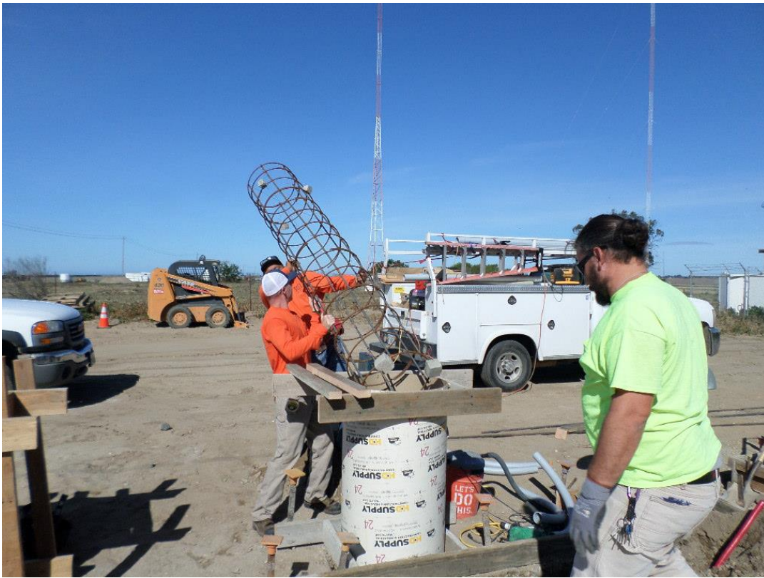
Spieß installing forms and reinforcement for light pole base.
