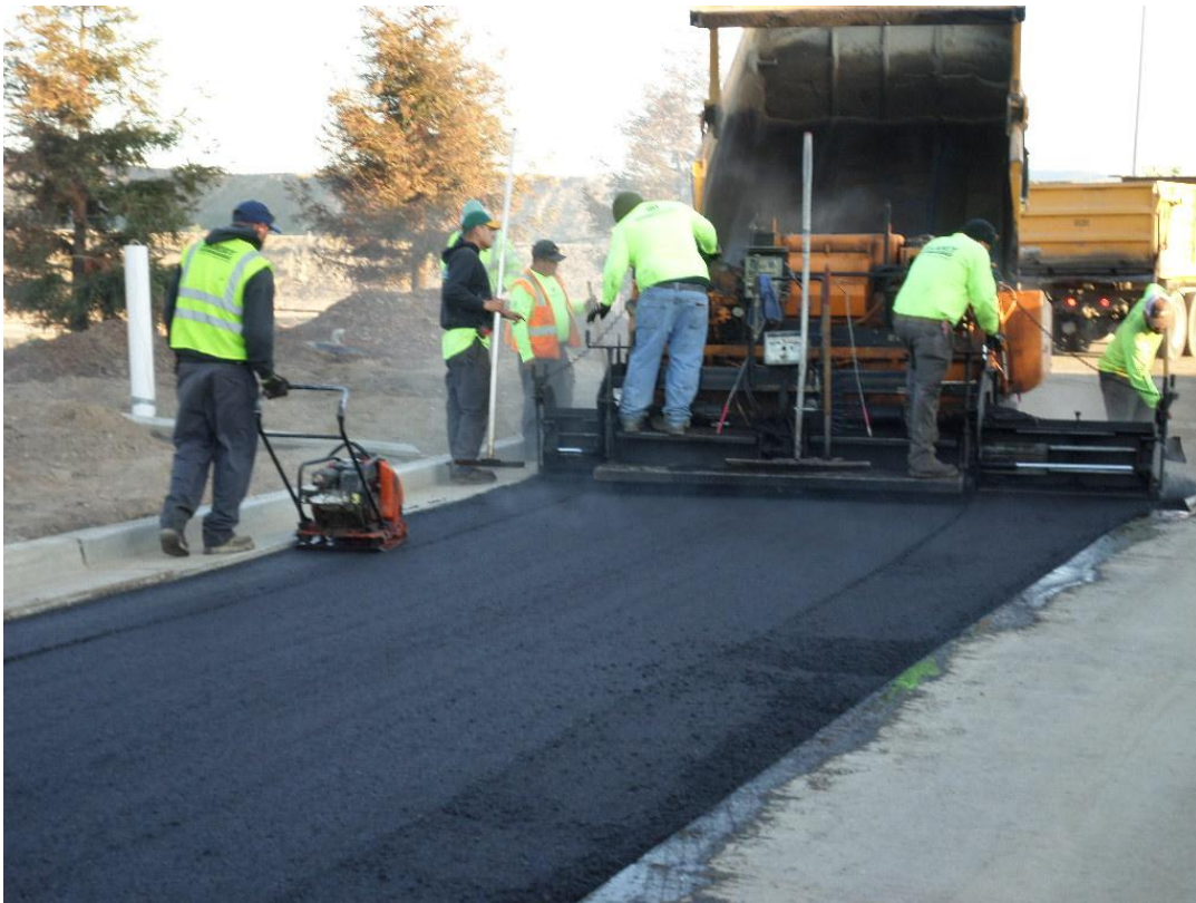
Ramsey Asphalt performing final paving of Blosser and Atlantic.
