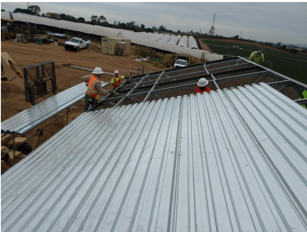
Spieß installing the roof deck at the pump station.
