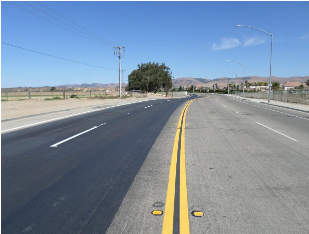
Blosser Road with project completed.
