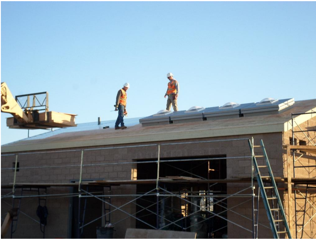
Spiess installing plywood sheeting on pump station roof around hatches.
