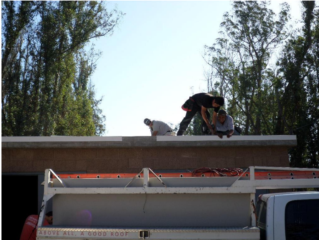
Quaglino Roofing installing the roof membrane.
