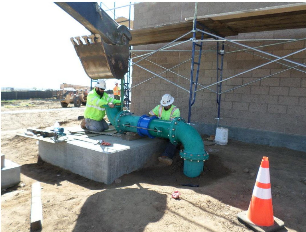
Spieß assembling surge tank piping.
