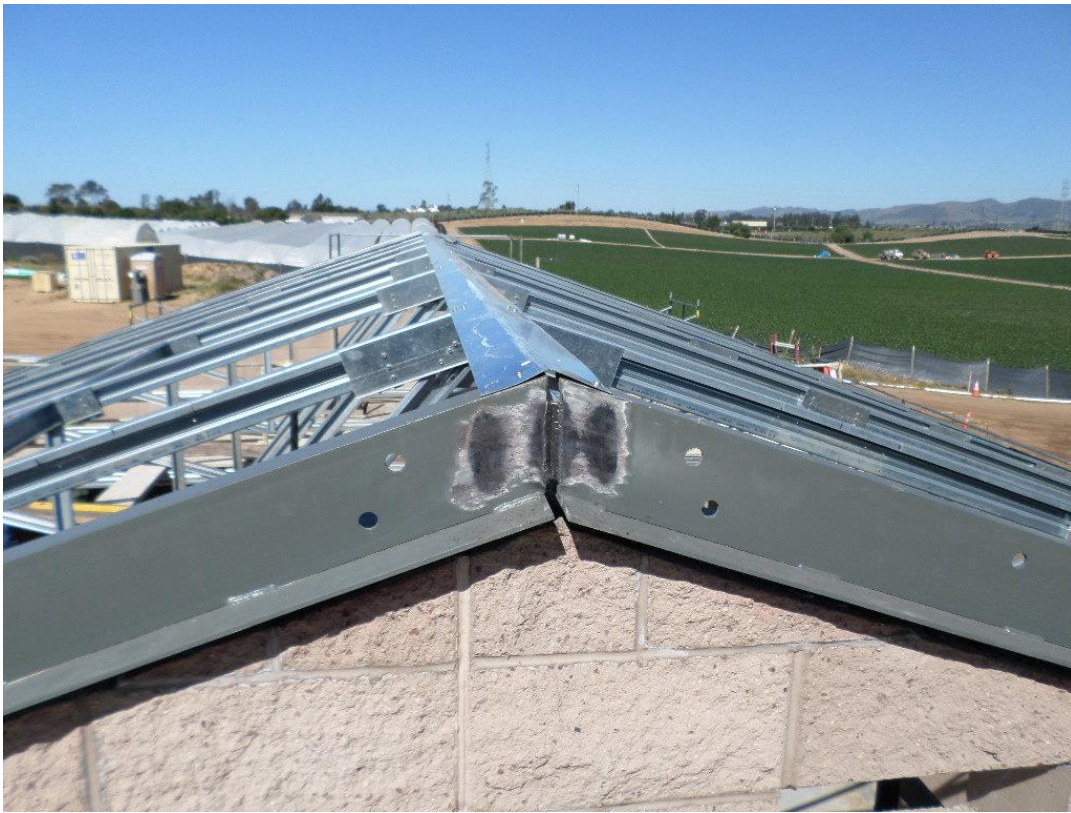
Welding steel plate connections at pump station.
