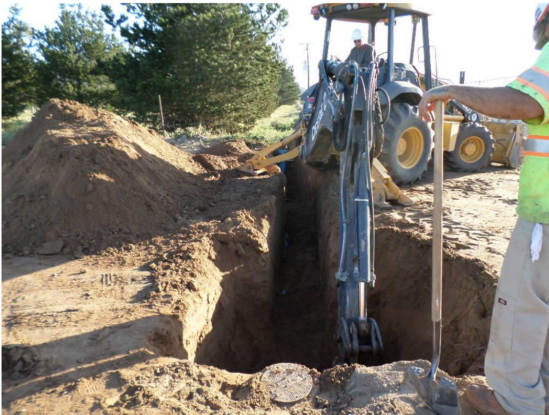
Spieß excavating to remove temporary bypass piping at PRV vault.
