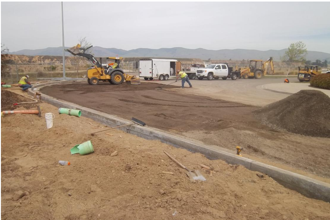
D-KAL spreading aggregate base in preparation for final paving.
