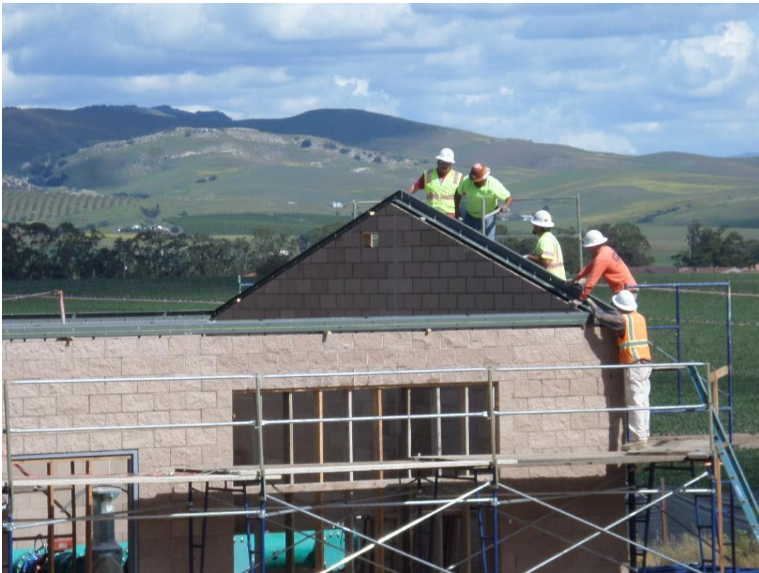
Spieß installing steel roof plates during final wall grout.
