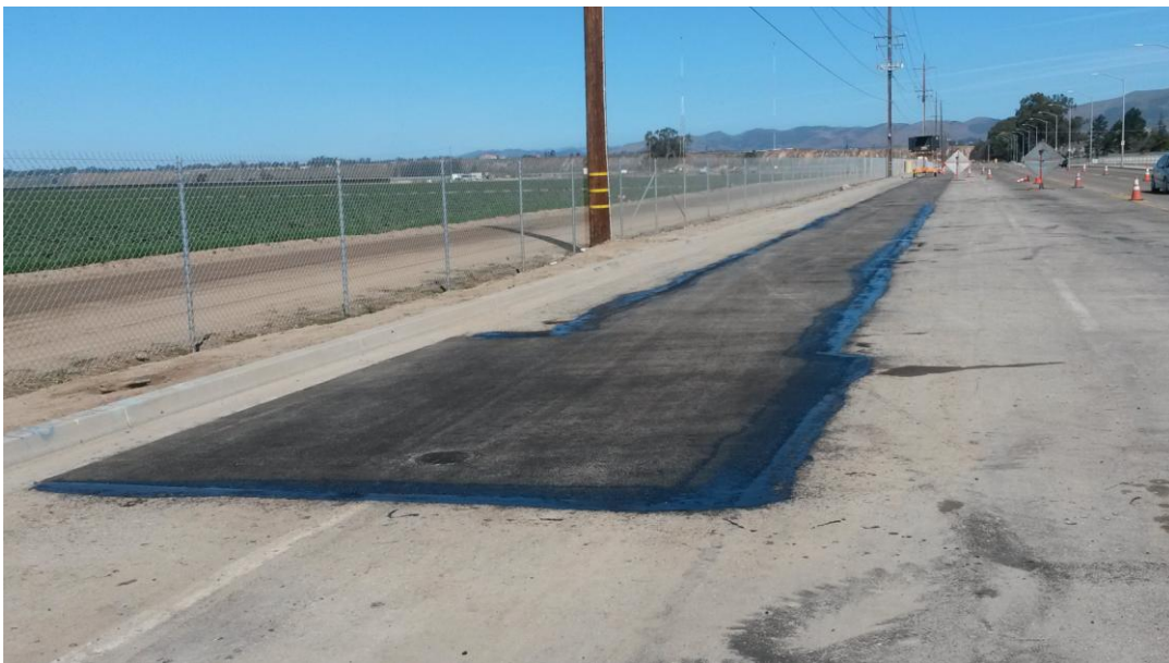
Final paving completed at Blosser and Taylor, and trench edges oiled.
