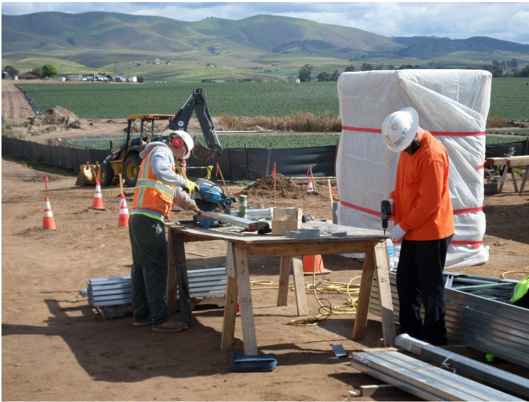
Spieß fabricating steel framing for roof at pump station.
