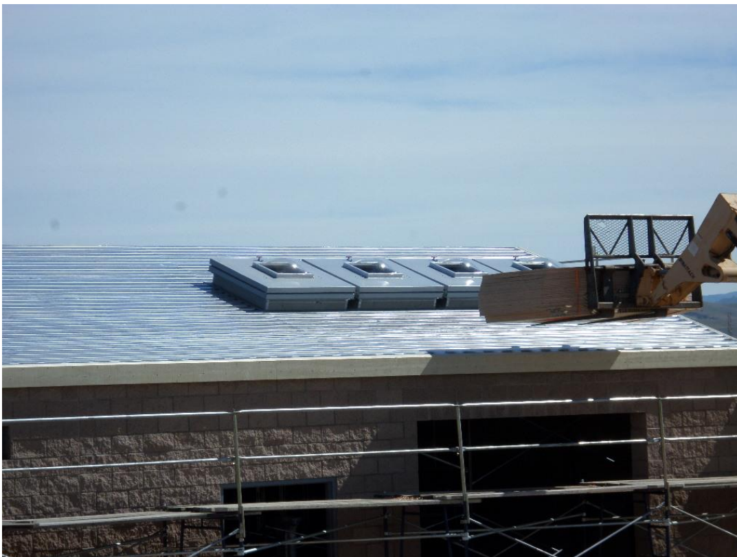
Roof hatches installed.
