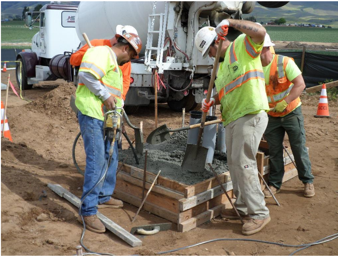
Spiess pouring for PG&E metering station.
