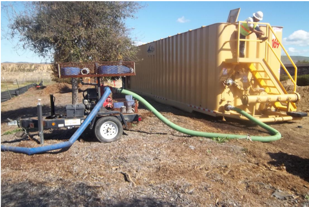
D-KAL using Baker tank to dechlorinate water from chlorinating prior to bacteria test and flushing from tank into SBCFC channel at Blosser and Atlantic with their permission.
