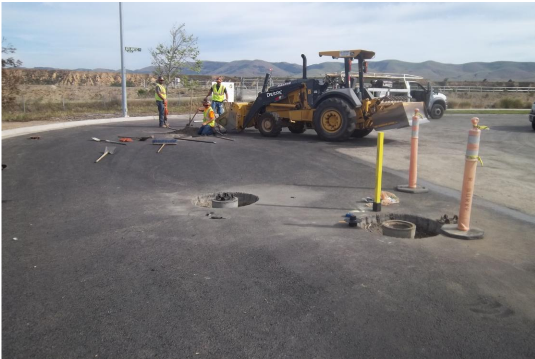
Valve cans installed and ready for pouring concrete collars.
