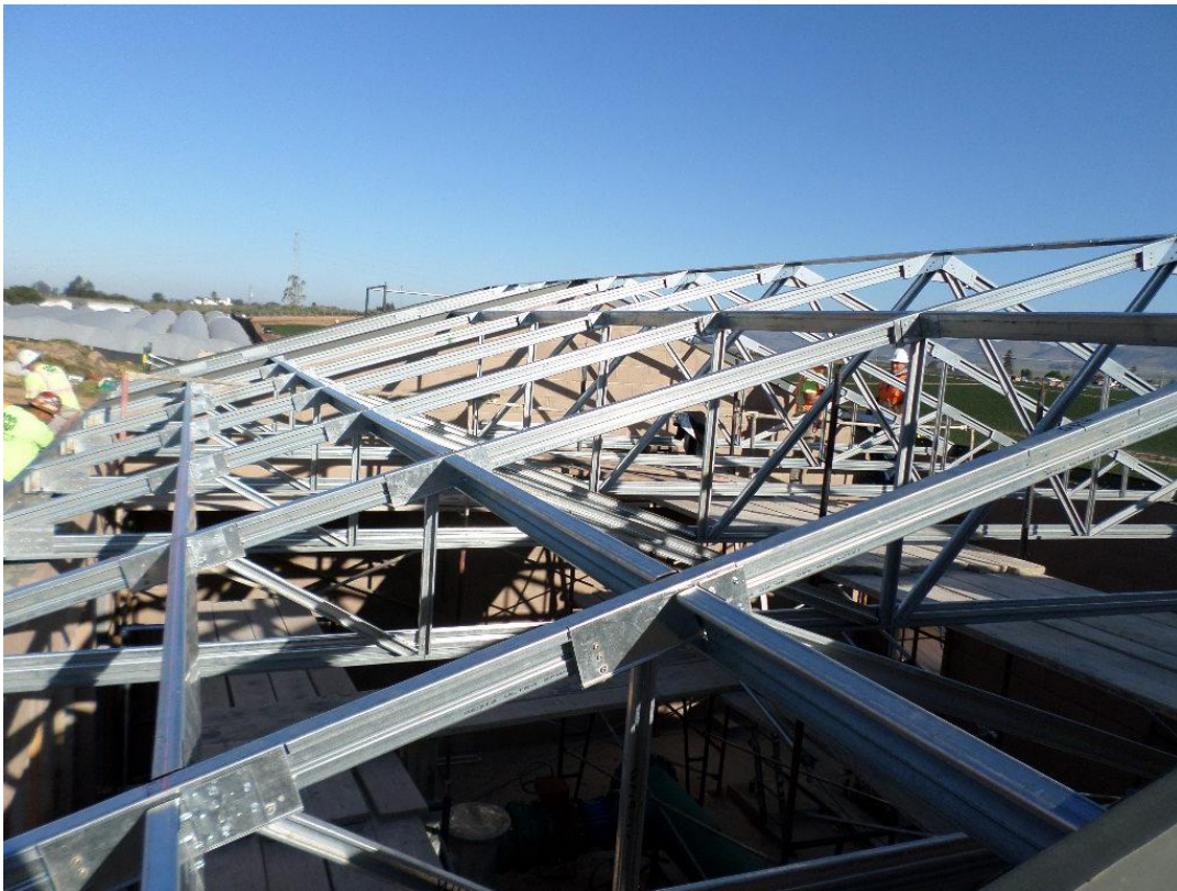
Spiess installing truss framing.
