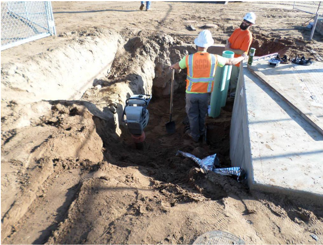
Backfilling and compacting over piping at the PRV vault.
