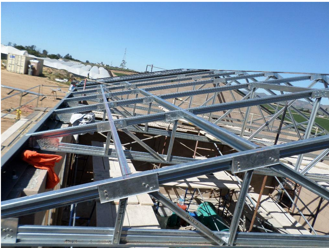
Spieß installing truss framing.
