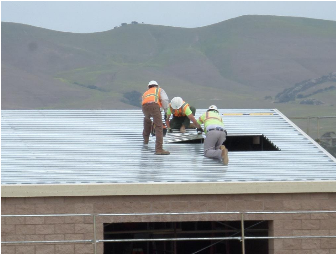
Spies cutting openings for roof hatches.
