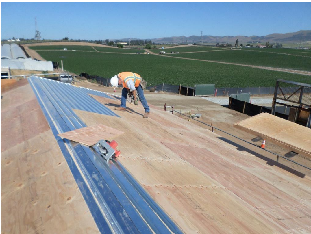
Spiess installing plywood sheeting on pump station roof.
