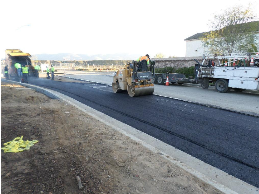
Ramsey Asphalt performing final paving at Blosser and Atlantic.
