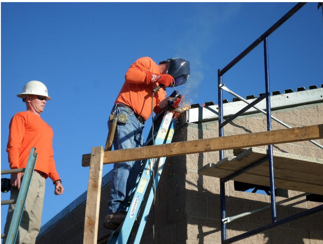
Puddle welding at steel roof plates.
