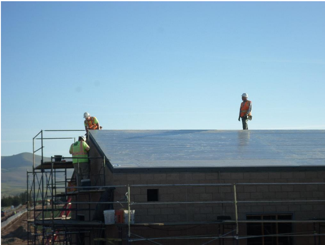
Steel roof deck installed.
