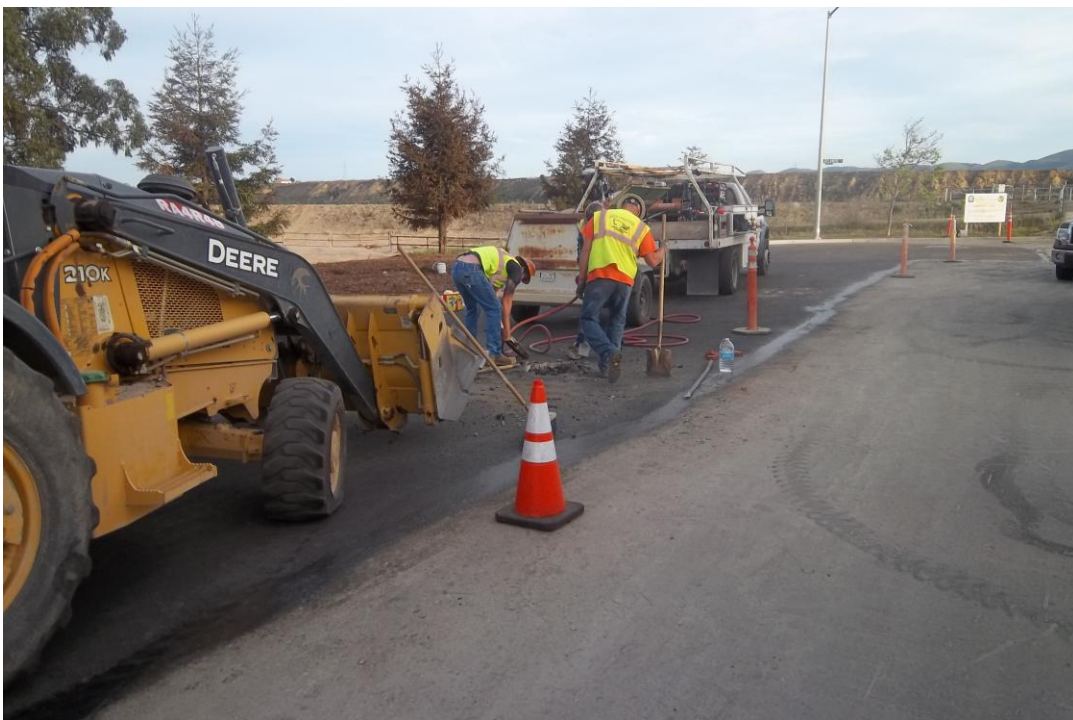
D-KAL removing paving to install valve cans and concrete collars.
