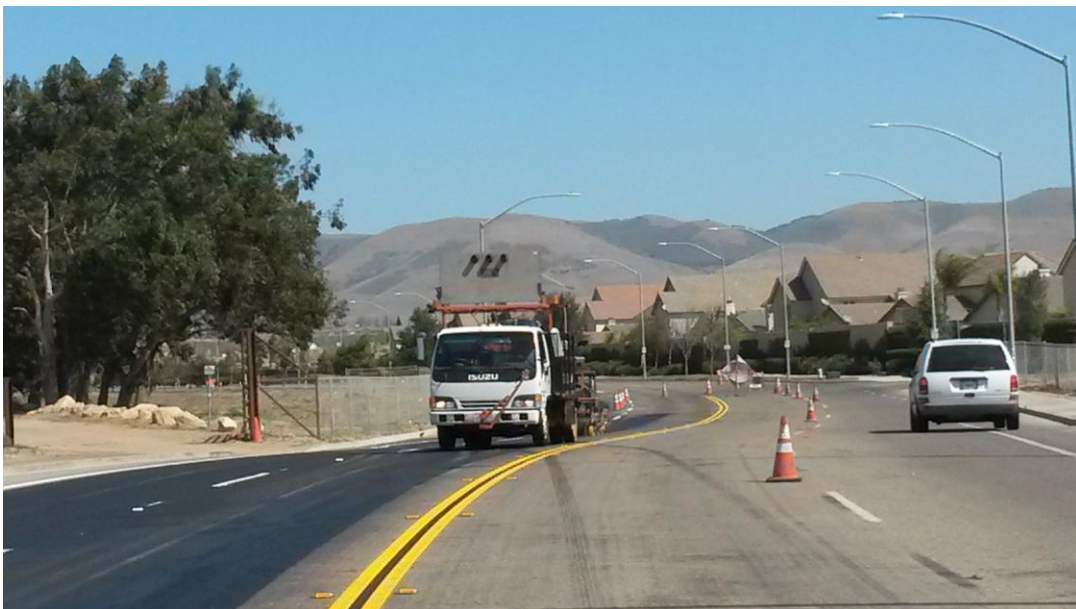
Toste restriping Blosser Road and replacing delineators.
