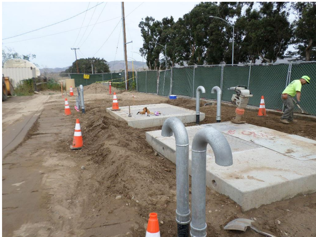
Spiess installing vent piping at metering vaults.
