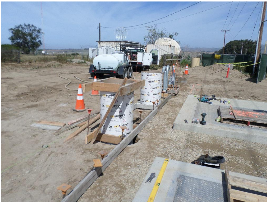
Spiess installing forms for electrical pad, light pole and SCADA antenna.
