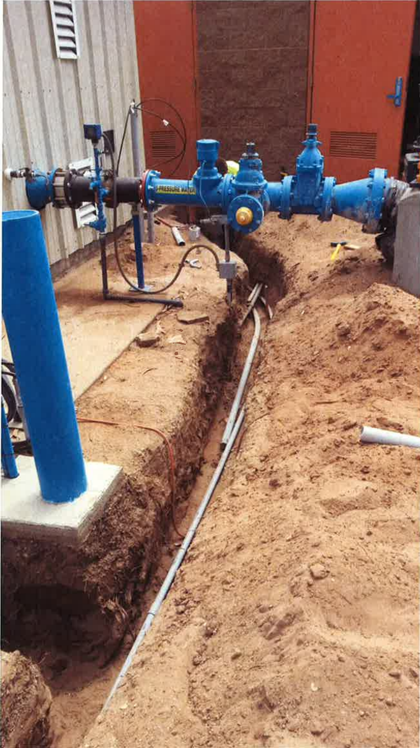
St. Denis Electric installing underground conduit.
