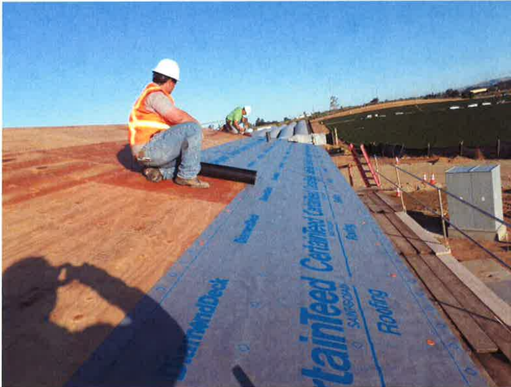
Quaglino Roofing installing moisture barrier on pump station building roof.
