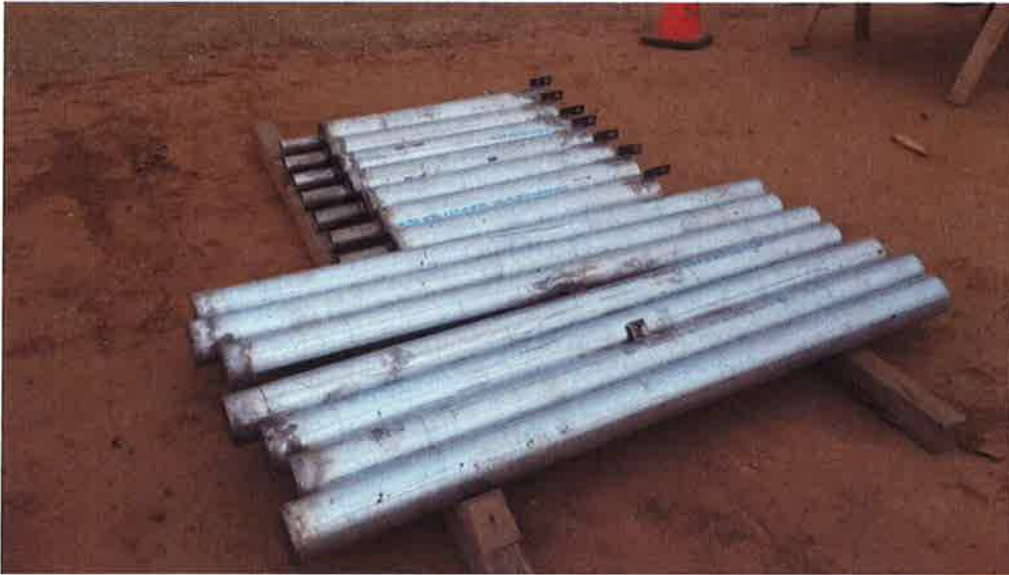
Removable bollards fabricated and delivered to pump station site.
