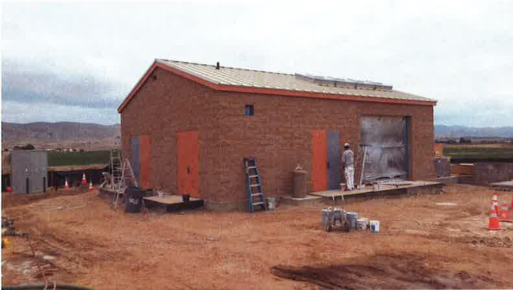
Coast Painting priming metal doors at pump station building.
