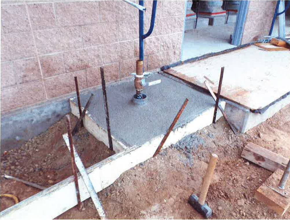
Concrete pad poured for air release valve at pump station.
