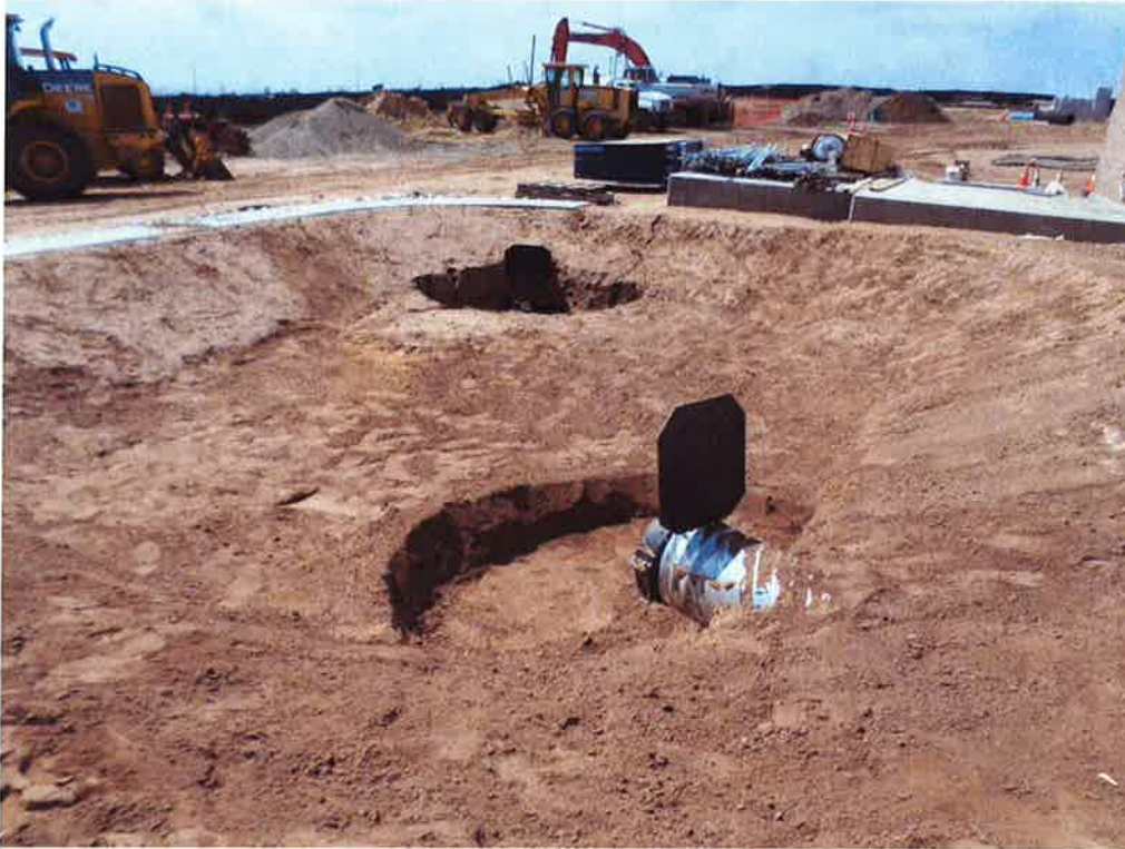
Excavation for rip rap at storm drain inlets in retention basin.
