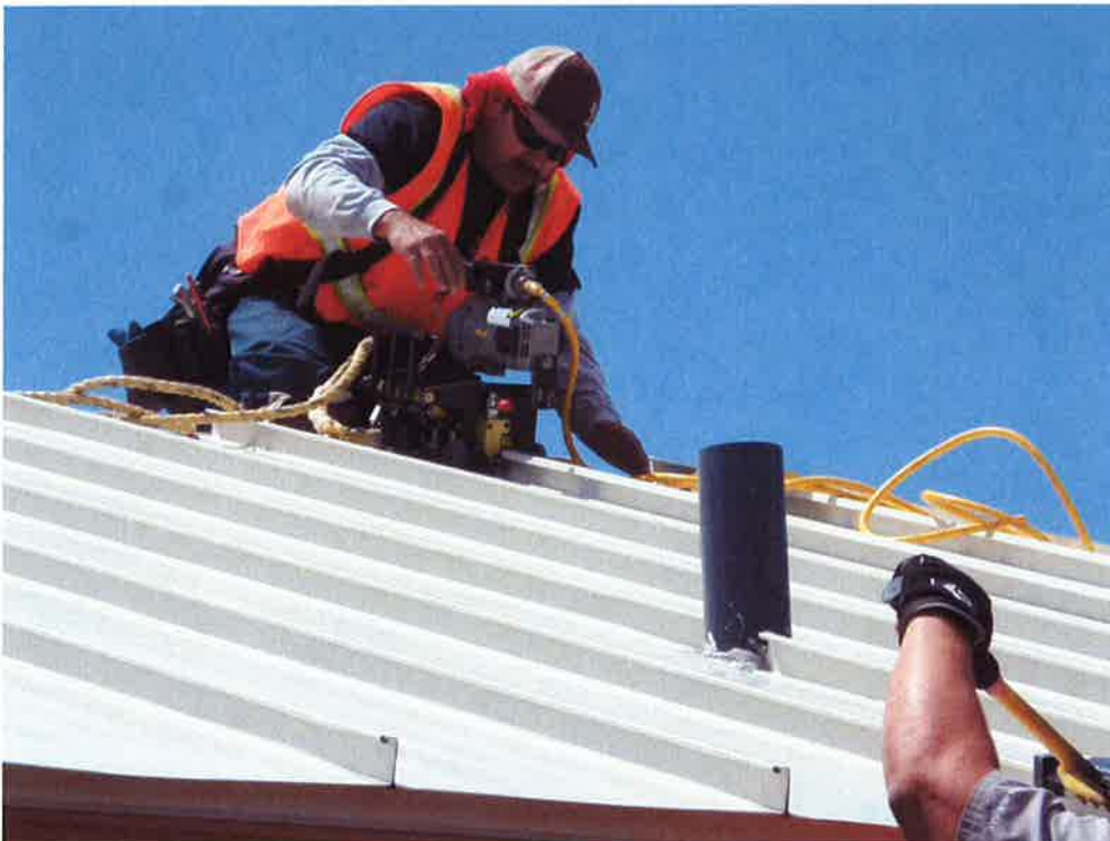
Quaglino Roofing installing seamless metal roof on pump station building.
