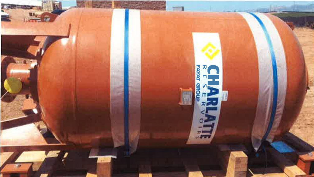
Surge tank delivered to pump station site.
