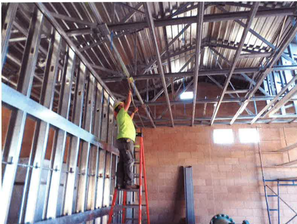
St. Denis Electric installing conduit and receptacles inside pump room.
