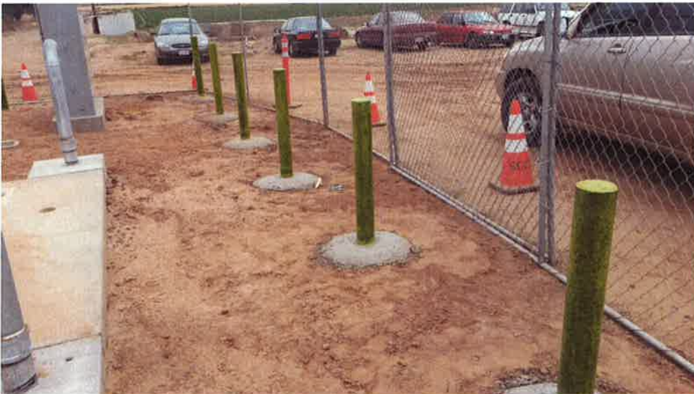
Coast Painting priming stationary bollards at the PRV vault.
