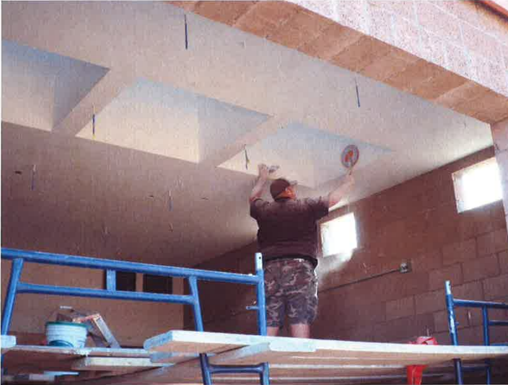
Ely Dodson Construction sanding the finish on the pump room ceiling.
