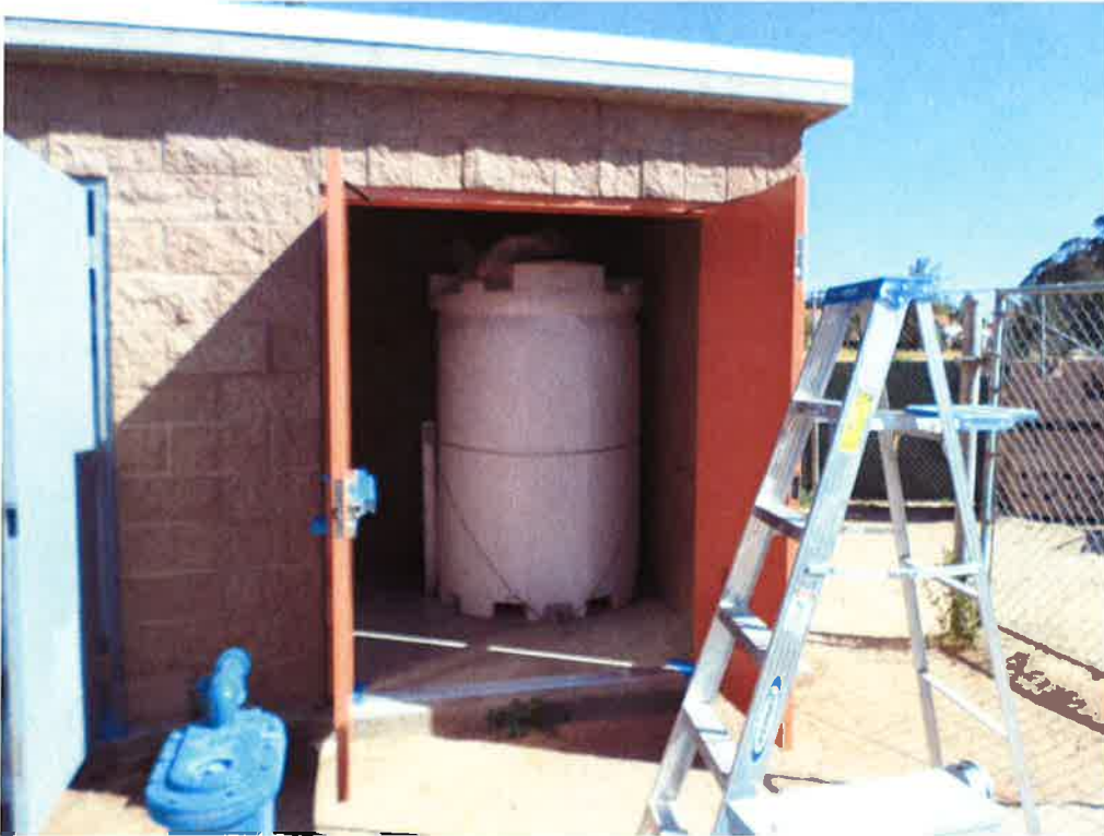
Coast Painting applying primer on doors.
