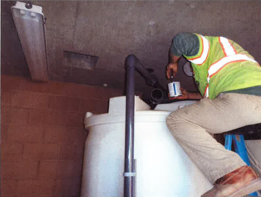
Spieß installing overflow piping on the chemical tanks.
