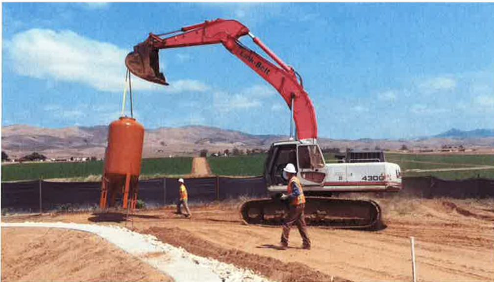
Spiess moving surge tank into place on concrete pad.
