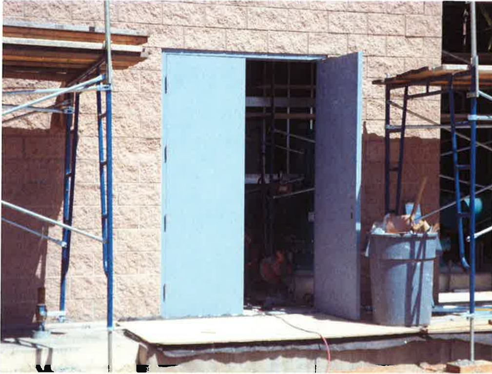
Martin Doors installing metal doors on pump station building.
