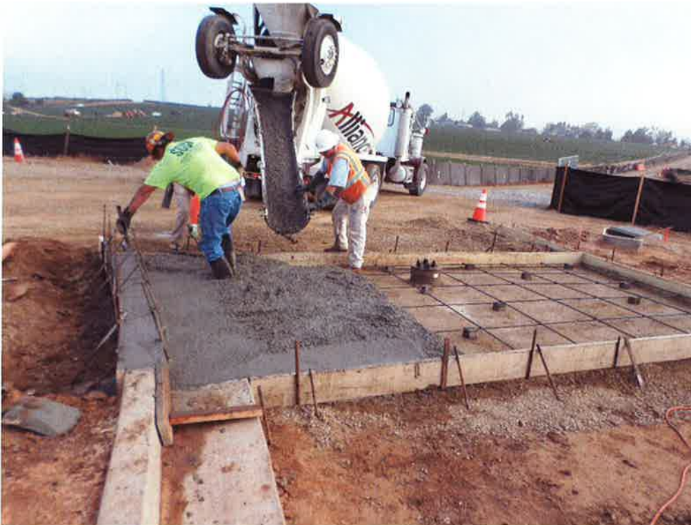
Spies pouring concrete for driveway approach.
