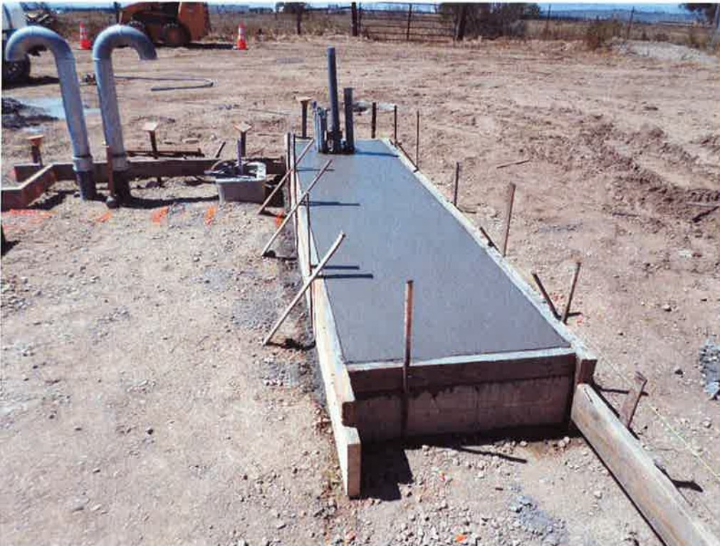
Completed pad for electrical panel.
