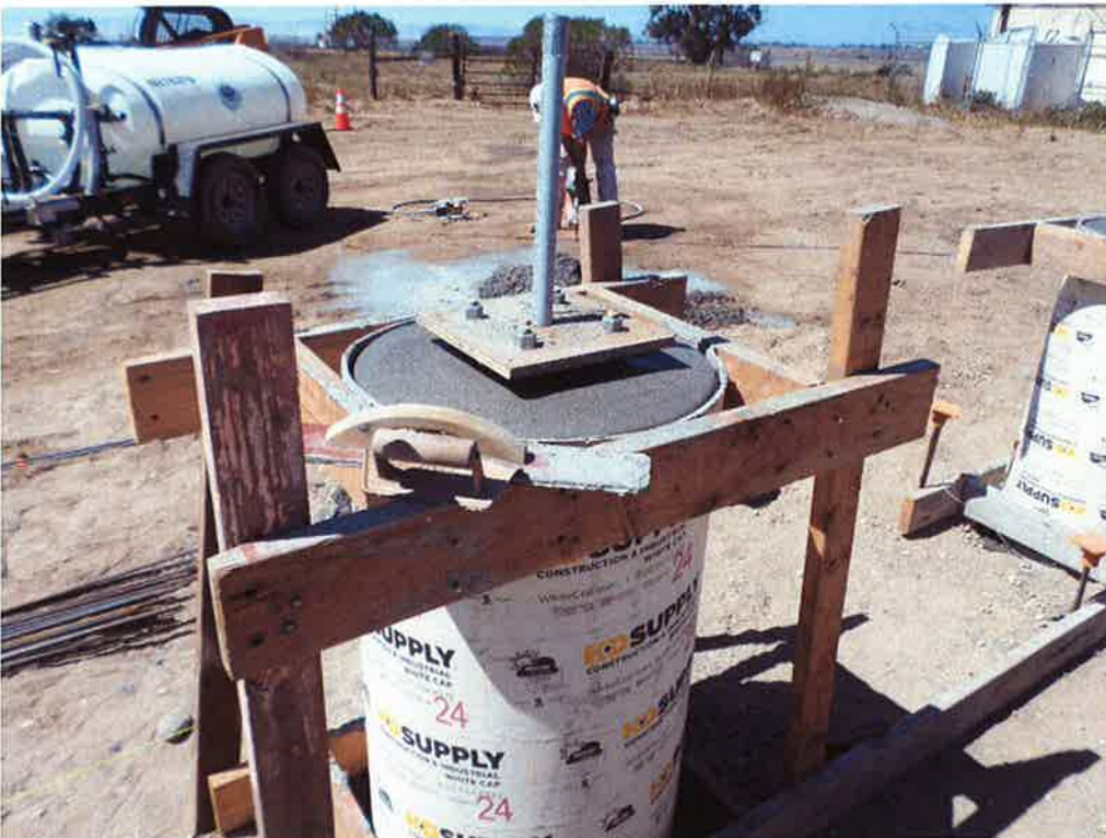
SCADA tower base poured.
