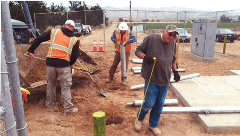
Spiess setting removable bollards at PRV vault.
