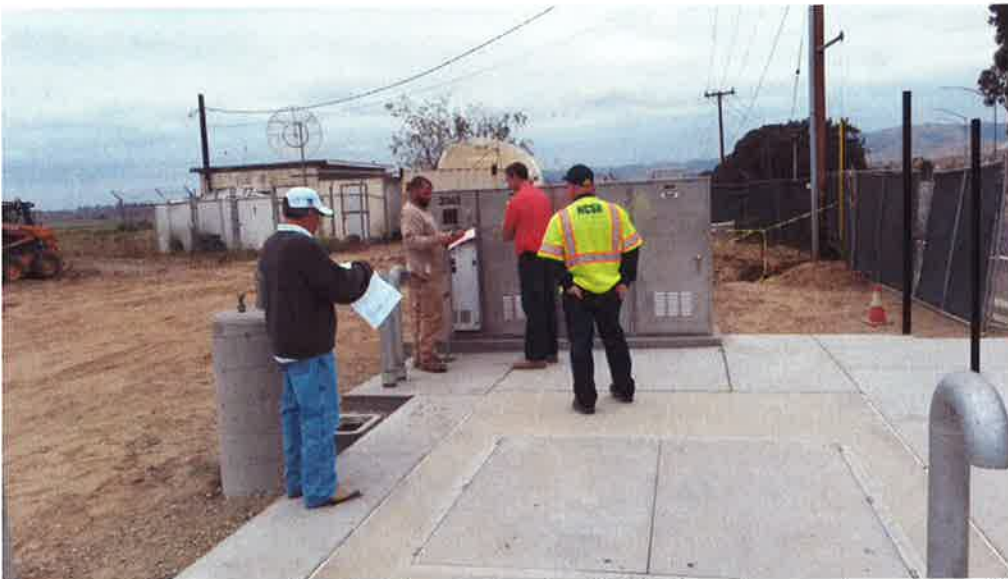
AECOM performing electrical inspection for PG&E to allow service connection.
