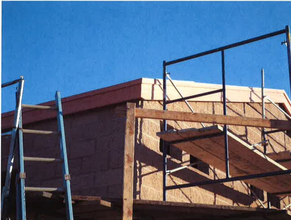
Coast Painting coating the pump station building fascia.
