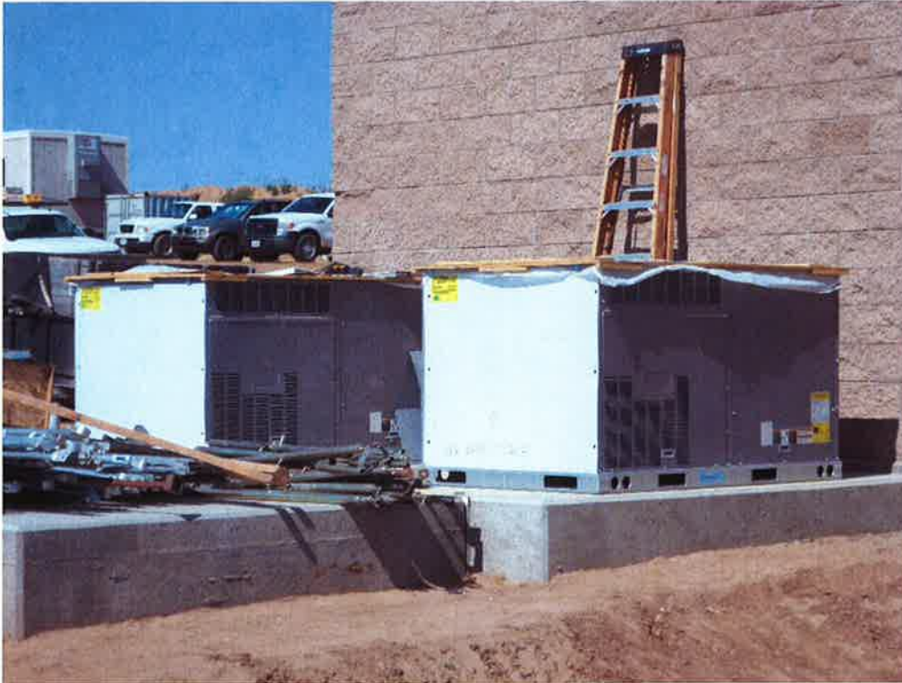
AC units delivered, set and anchored by Dahl Air Conditioning.
