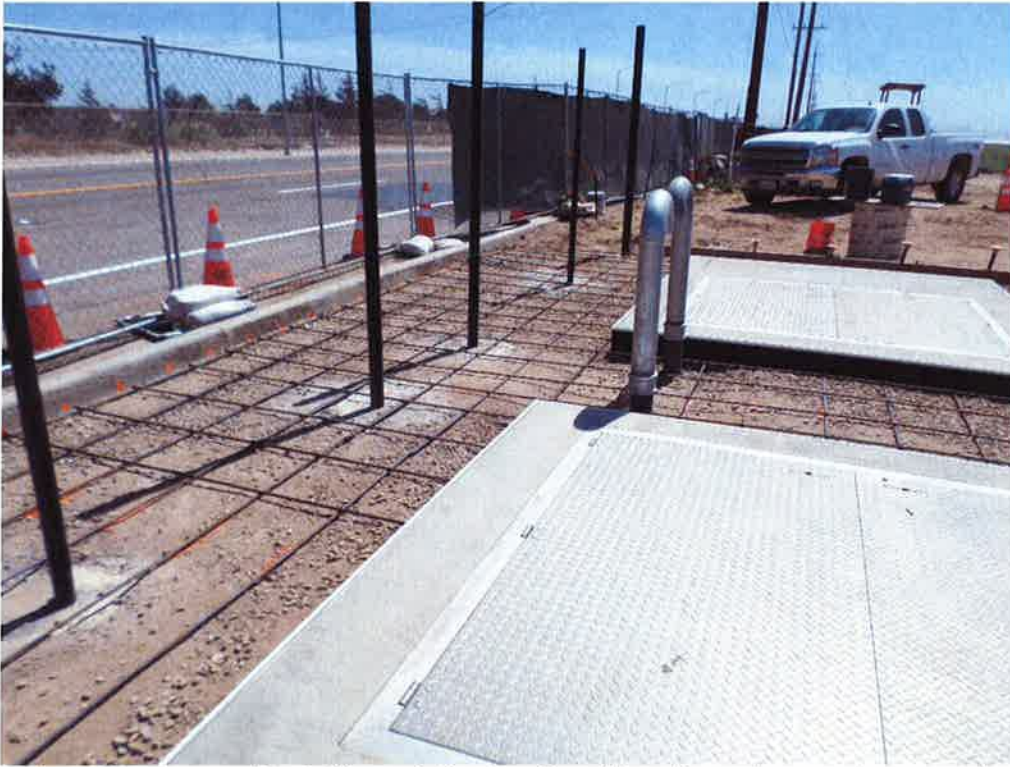
Spiess forming and installing reinforcing for sidewalk and concrete around vaults.
