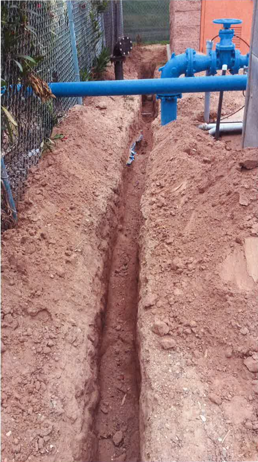
St. Denis Electric working on trench and installation of underground conduit.
