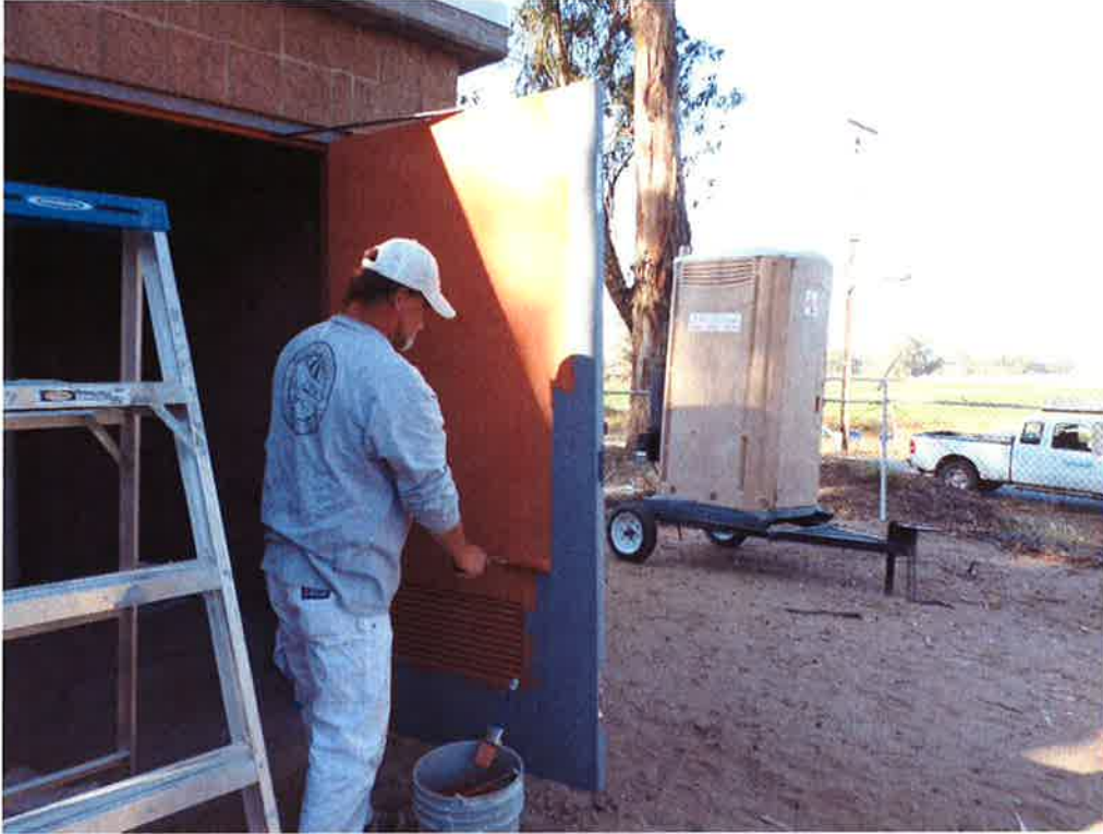
Coast Painting applying prime coat to metal doors.
