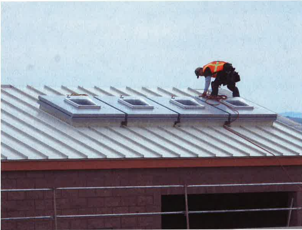
Quaglino Roofing completing seamless metal roof on pump station building.
