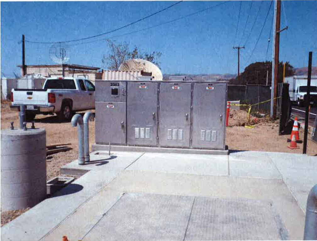
Electrical panels installed.
