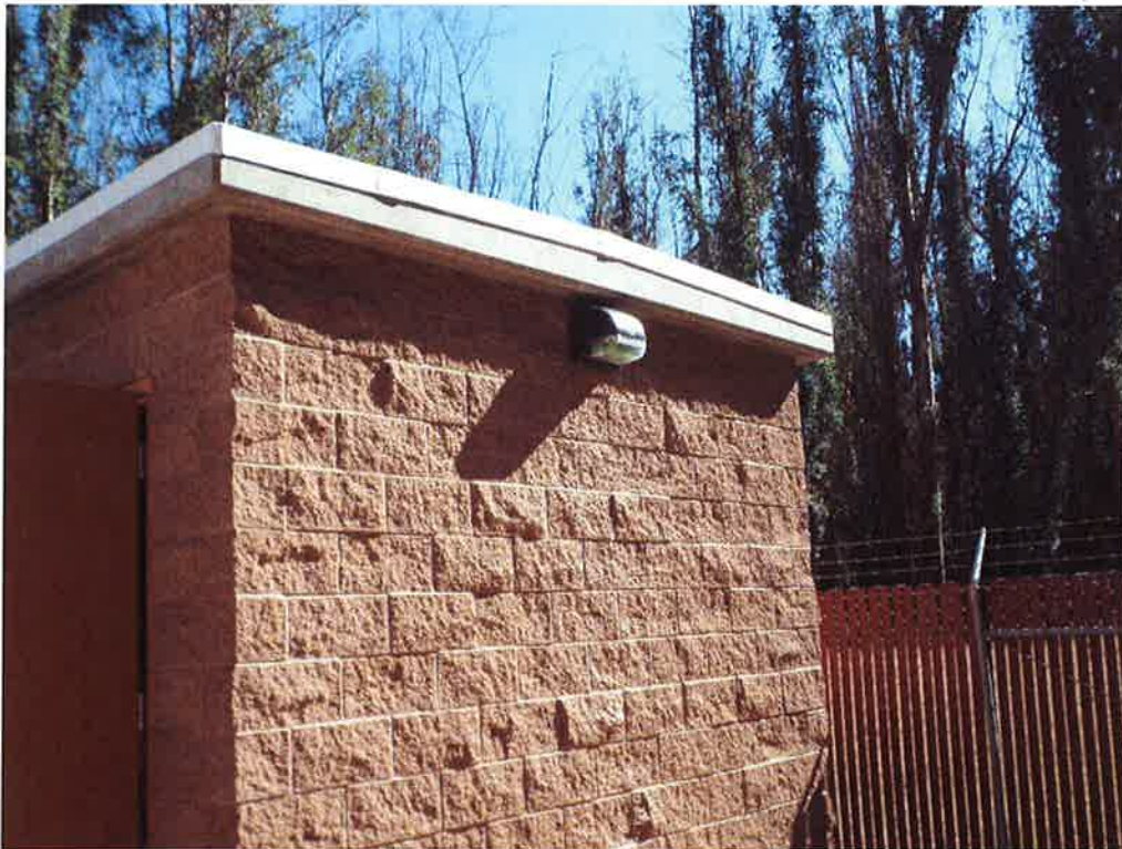
Exterior lighting installed.
