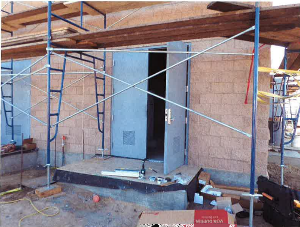
Martin Doors installing metal doors at pump station building.
