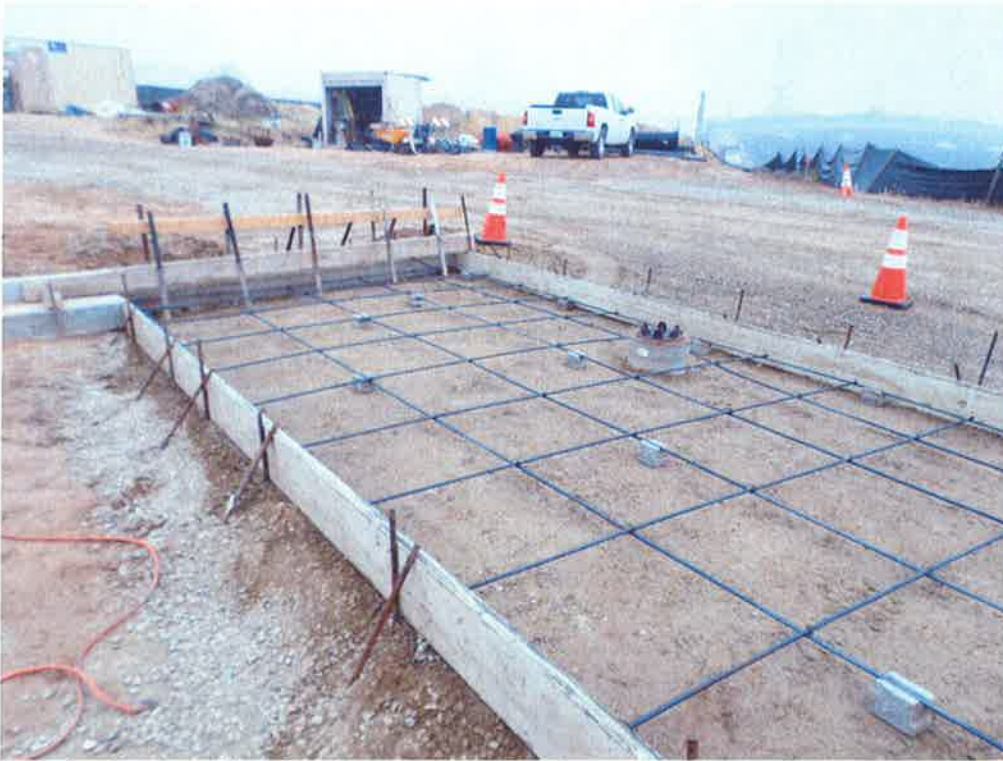
Reinforcing installed for driveway approach.
