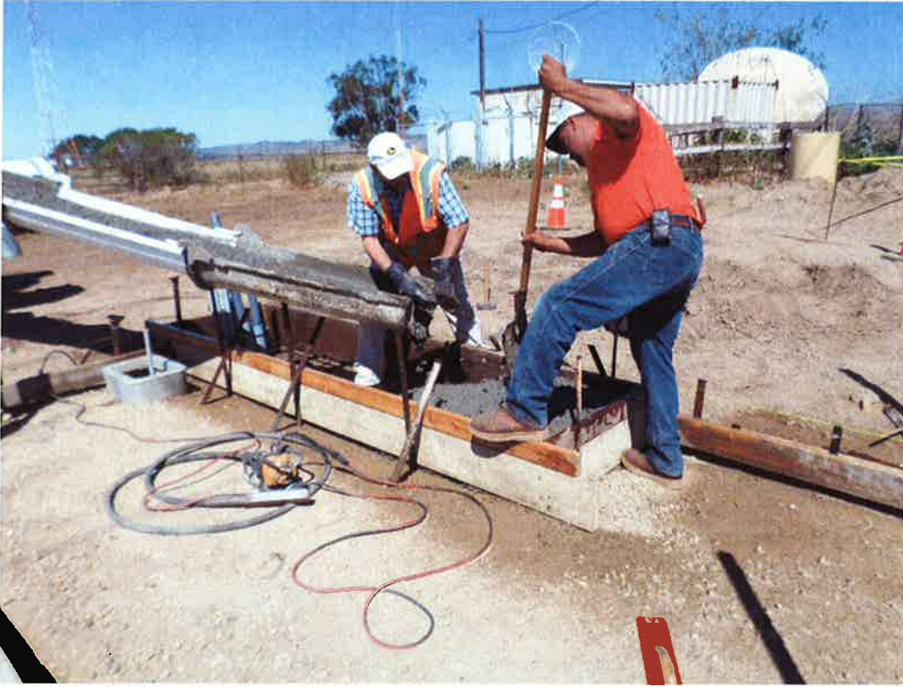
Spieß pouring concrete for the electrical panel pad.
