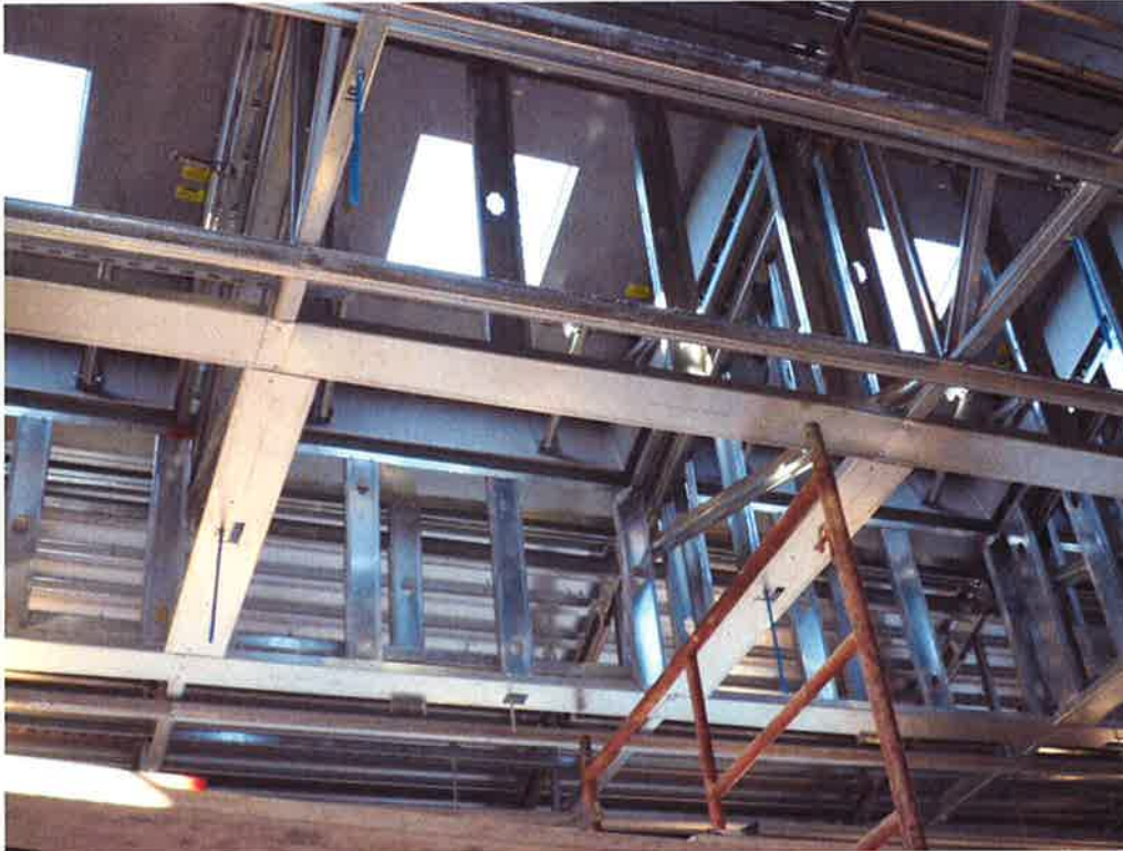
Ely Dodson Construction framing walls and ceiling at the roof hatches.
