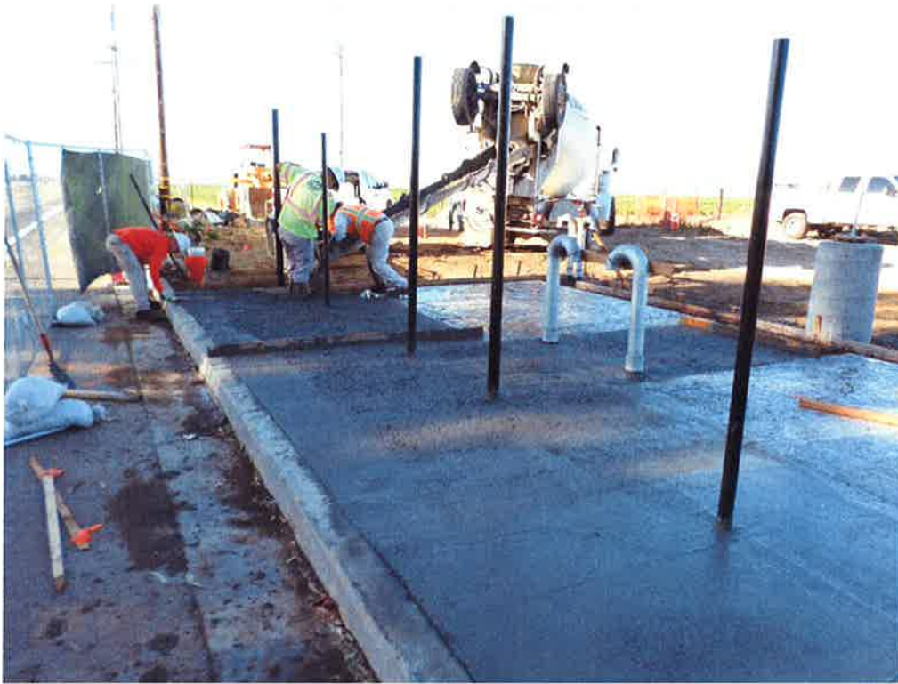
Spieß pouring concrete around vaults.
