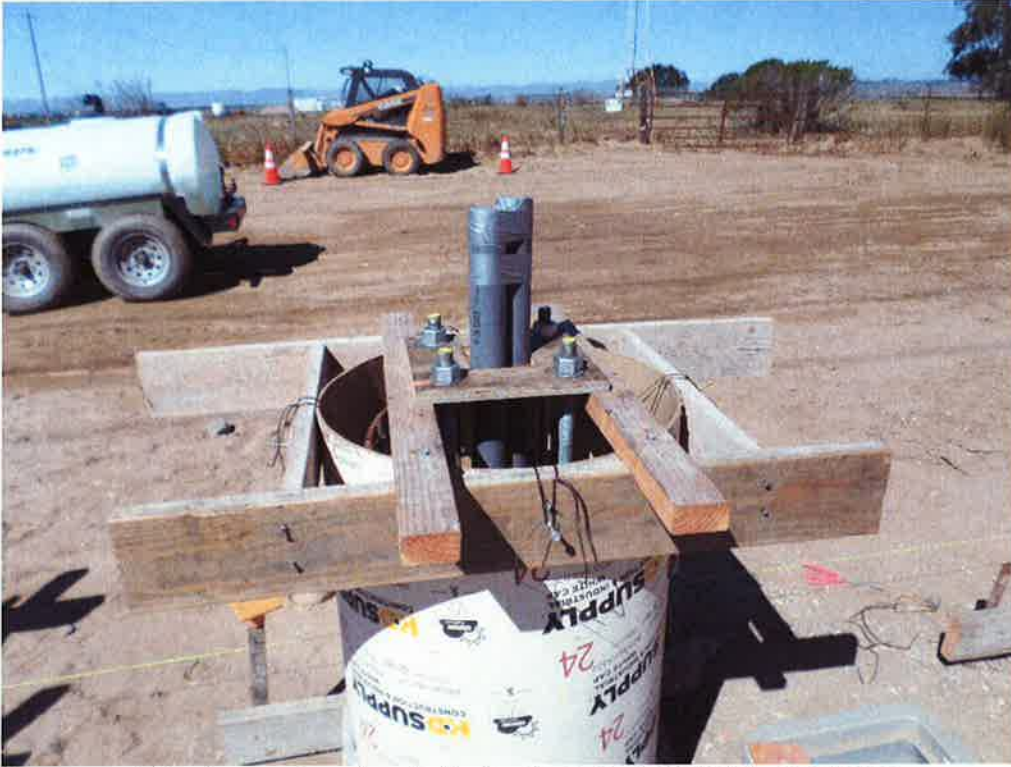
Forms, reinforcing and anchor bolts in place for SCADA tower base.
