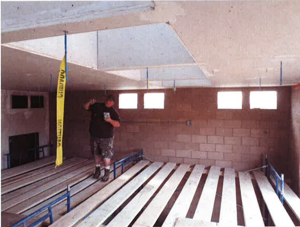
Ely Dodson Construction installing sheet rock inside pump station.
