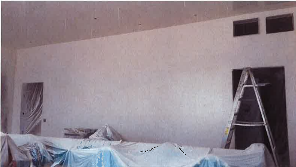
Coast Painting coating wall between pump room and electrical room.
