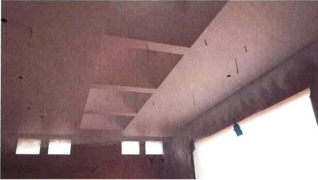
Coast Painting coating pump room ceiling.
