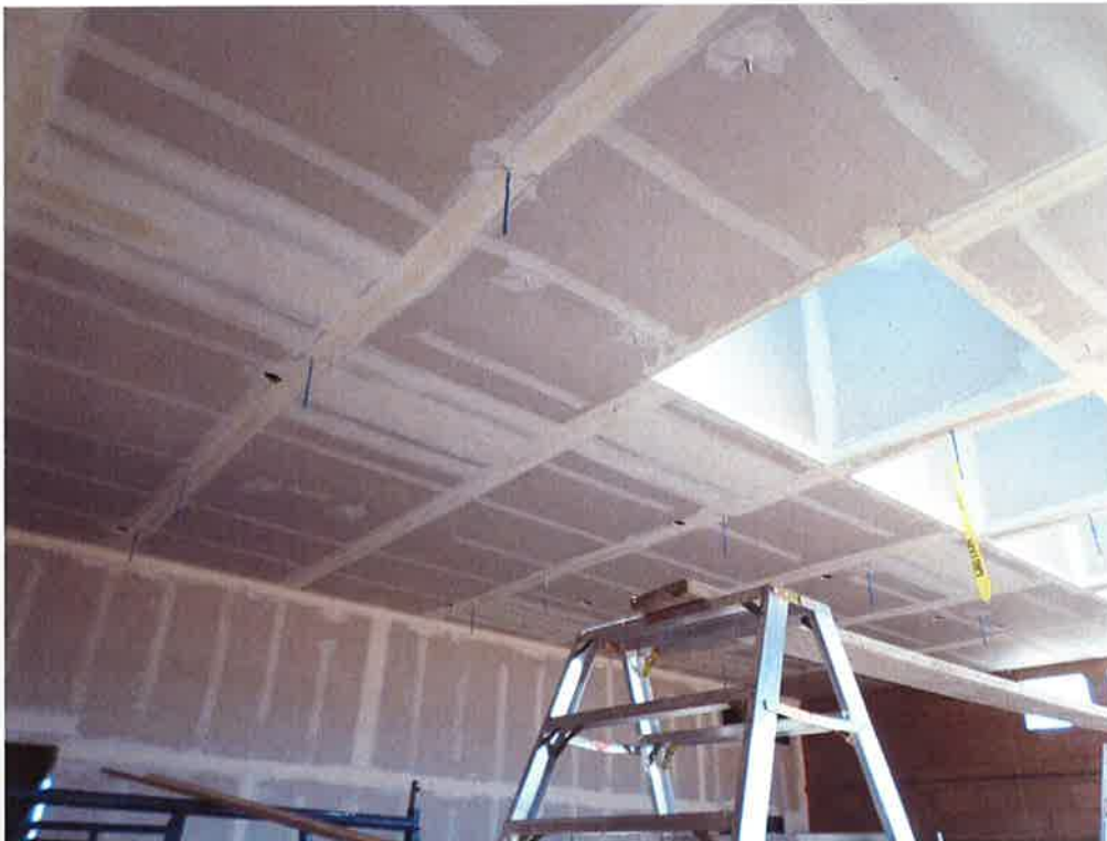
Ely Dodson Construction taping sheet rock inside pump station.
