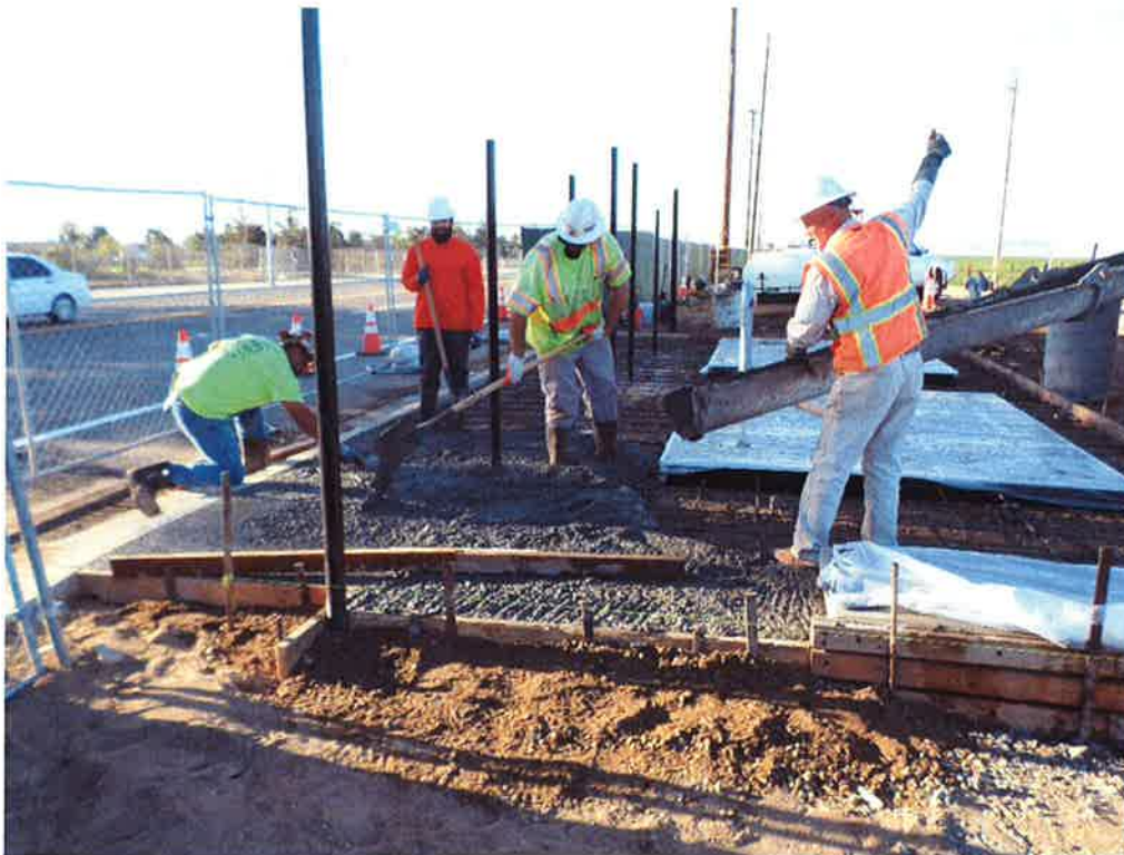
Spiess pouring sidewalk and concrete around vaults.
