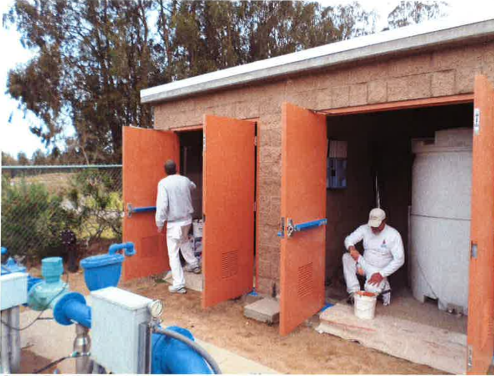
Coast Painting applying final coating to doors.
