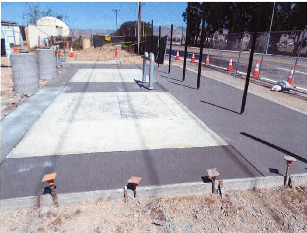
Completed sidewalk and concrete around vaults.
