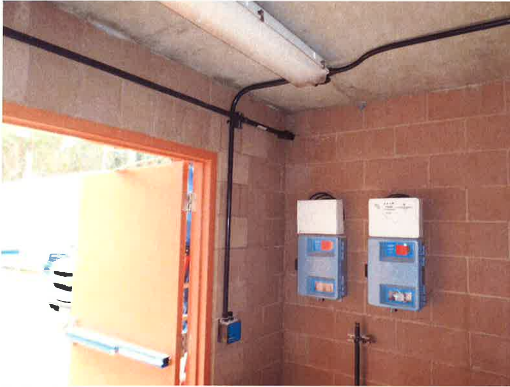
St. Denis Electric installing conduit and receptacles in chemical building.
