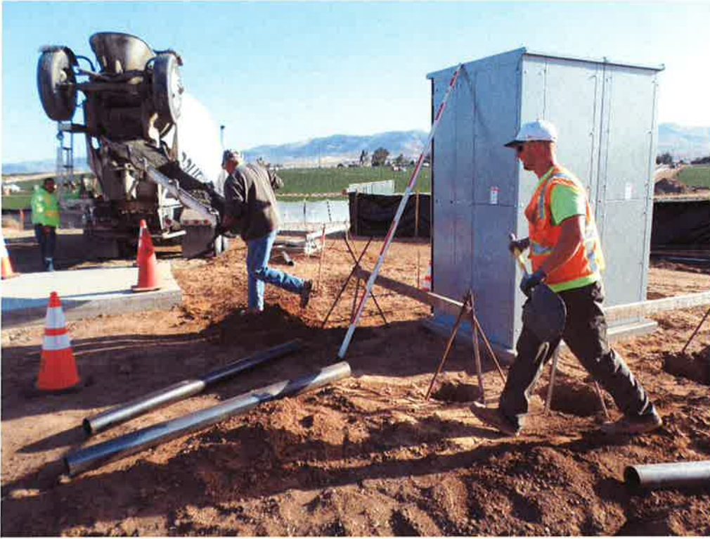
Spieess pouring bases for stationary bollards at pump station site.
