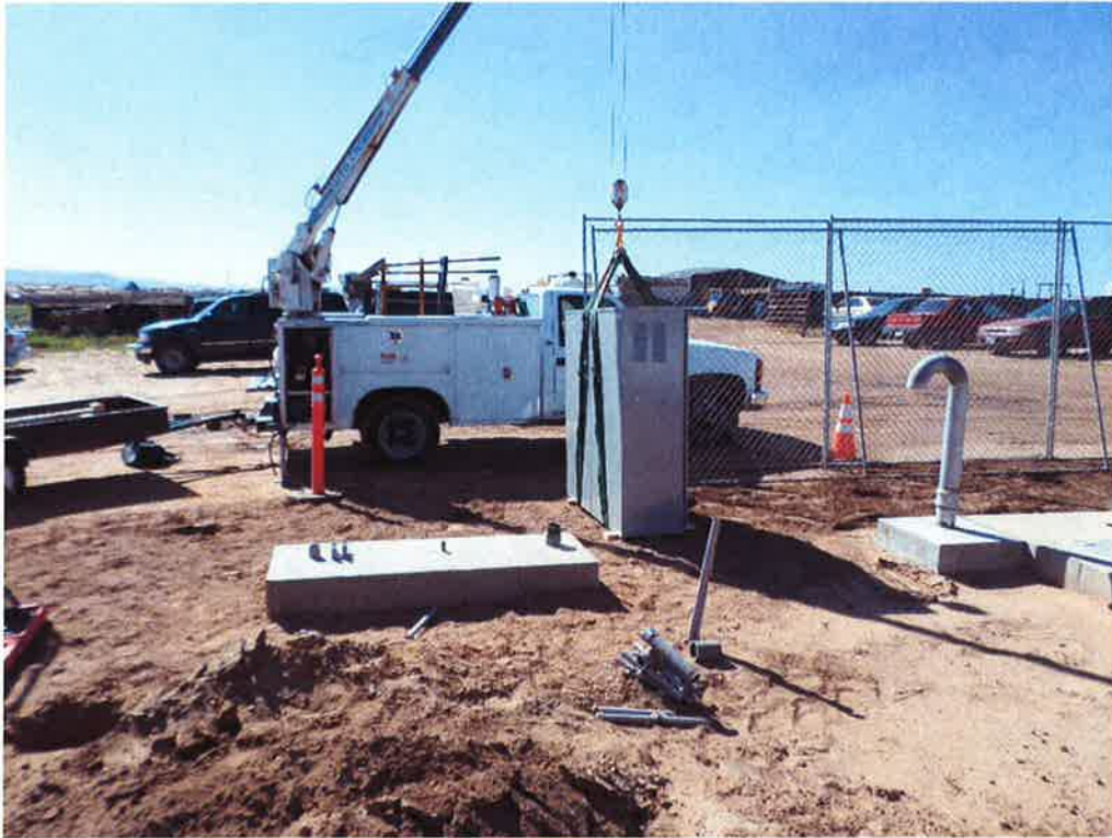
St. Denis Electric installing PLC at PRV vault.
