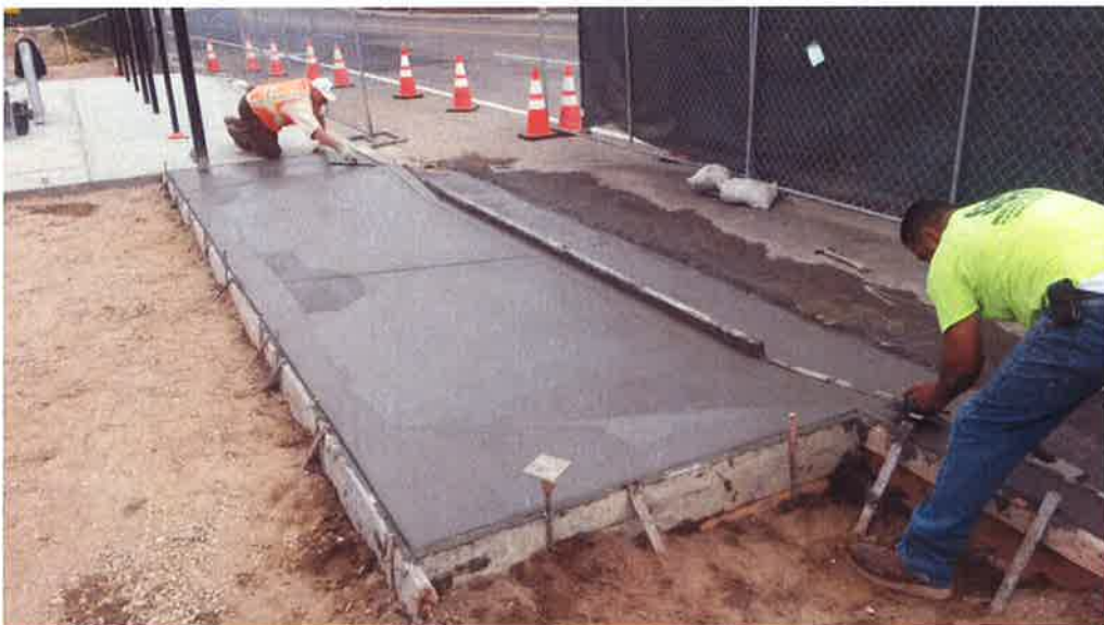
Spiess finishing concrete for driveway approach.
