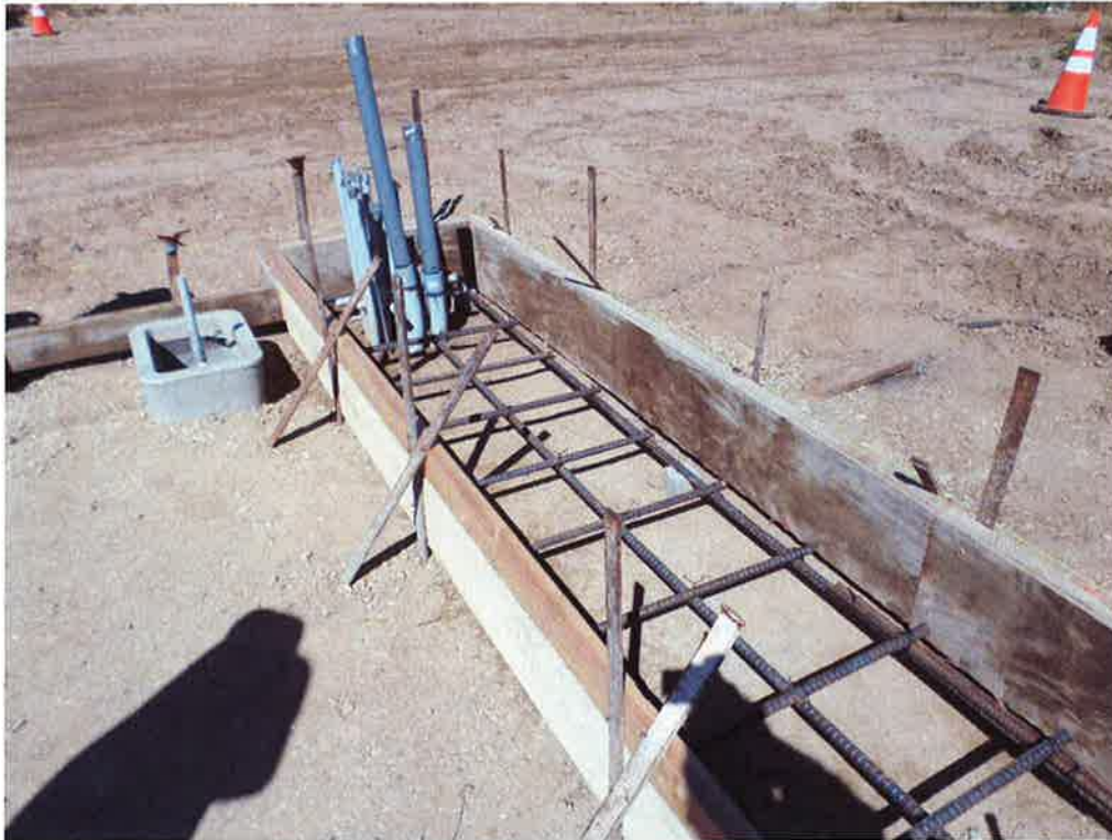
Forms and reinforcing for electrical panel pad.
