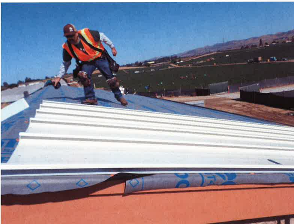
Quaglino Roofing installing seamless metal roof on pump station building.
