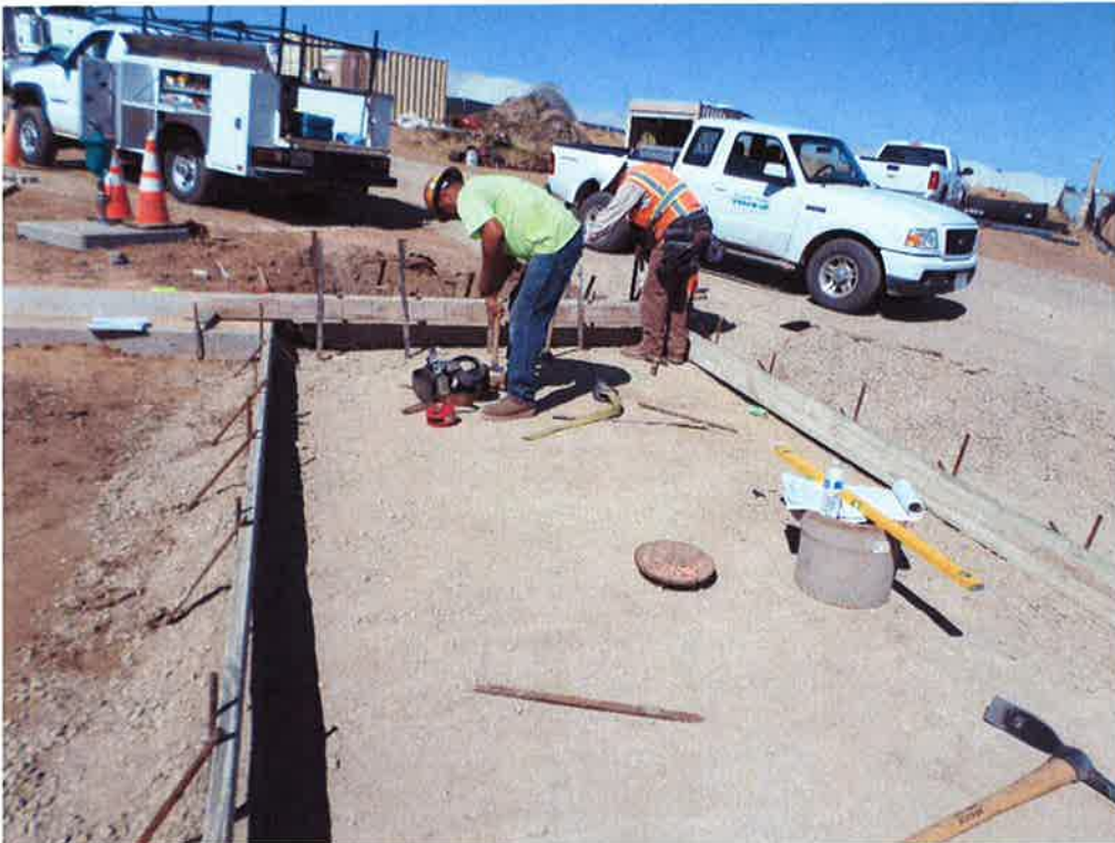
Spiess forming driveway approach at pump station.
