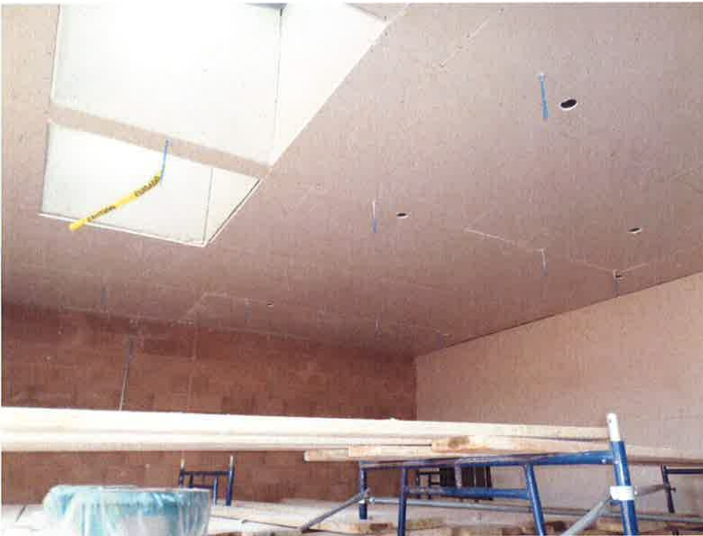
Ely Dodson Construction installing sheet rock inside pump station building.
