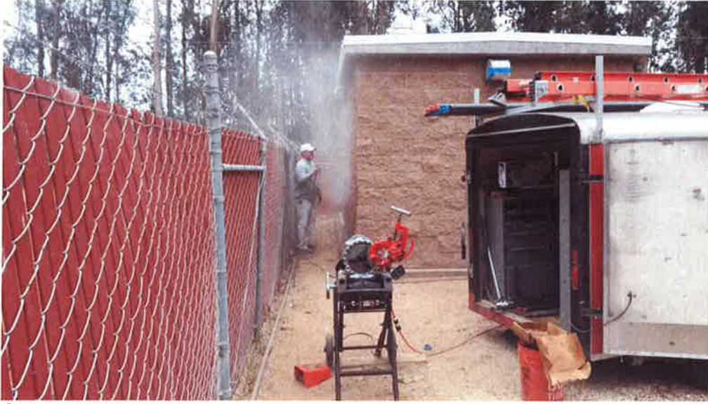
Coast Painting sealing outside of building.
