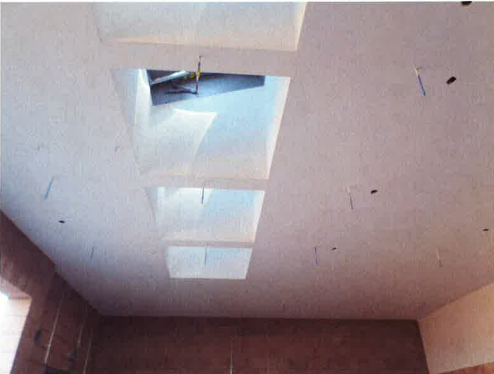
Pump room ceiling completed and ready for coating.
