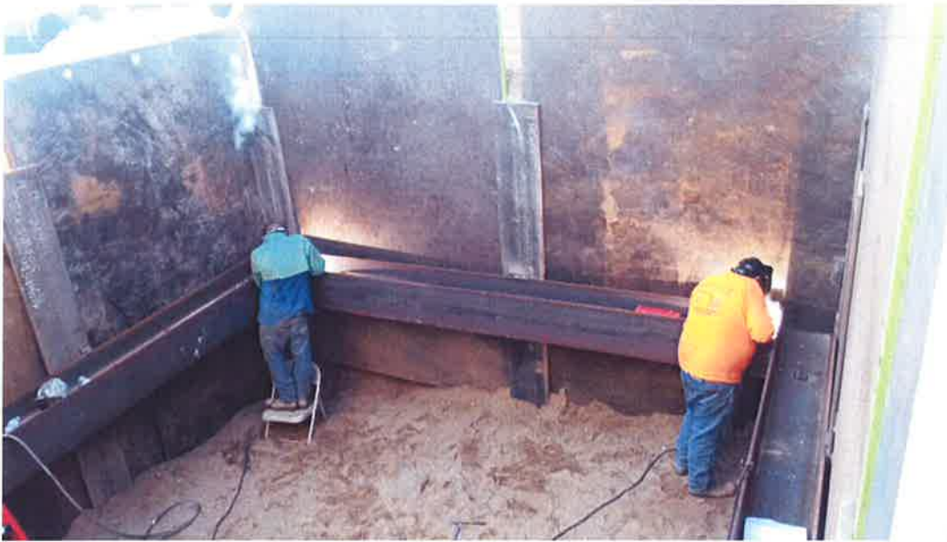
D-KAL welding horizontal supports for shoring inside receiving pit.
