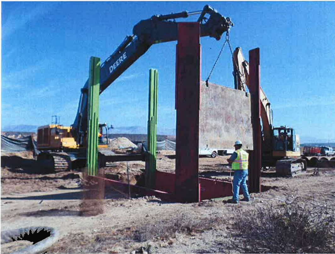
D-KAL installing slip shoring at bore and jack pit.
