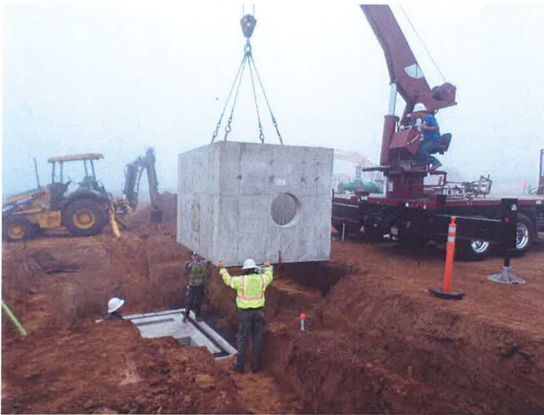
Spiess setting metering vault onto base.
