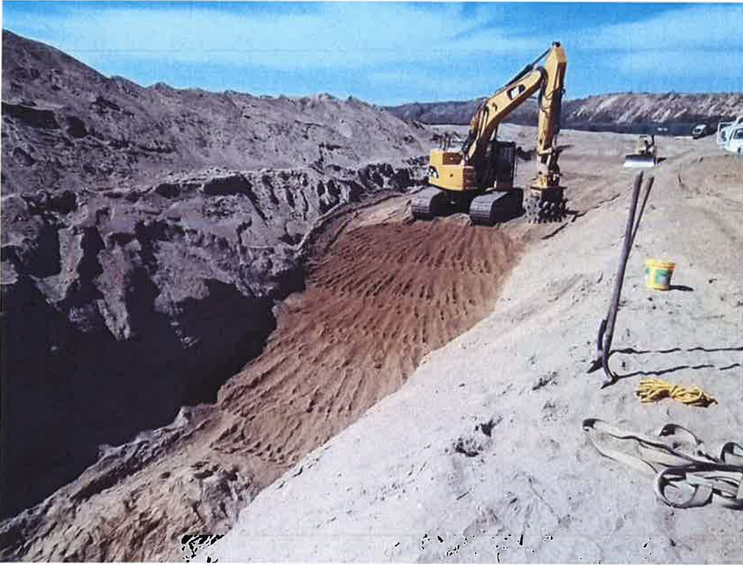
D-KAL backfilling and compacting over 24-inch DIP in river area.
