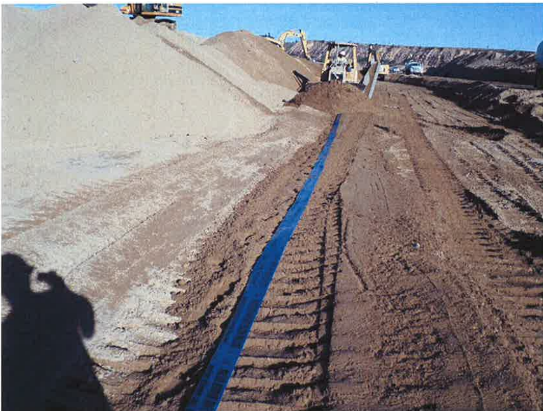
D-KAL installing top layer of pipe locating tape.
