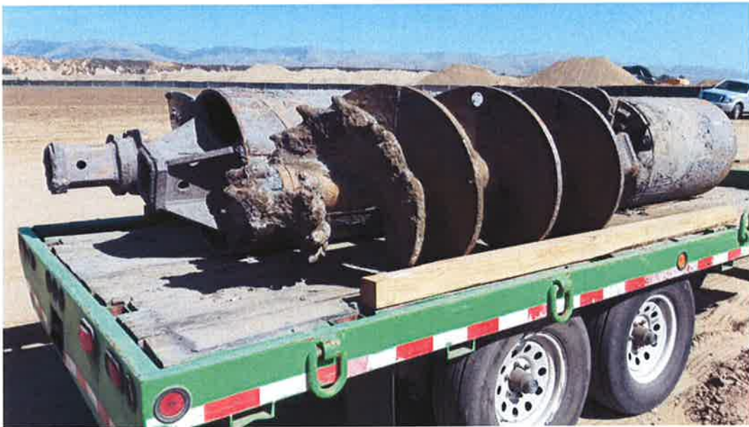
Pacific Boring mobilizing drill heads for bore and jack.
