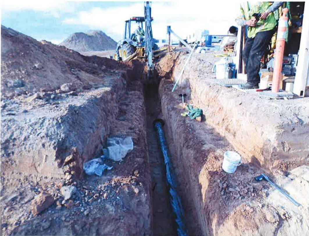
Spieß installing 6-inch DIP for the fire hydrant located on site.
