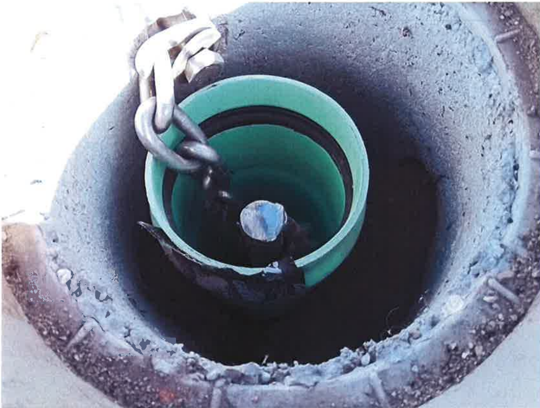
Settlement monitor installed.
