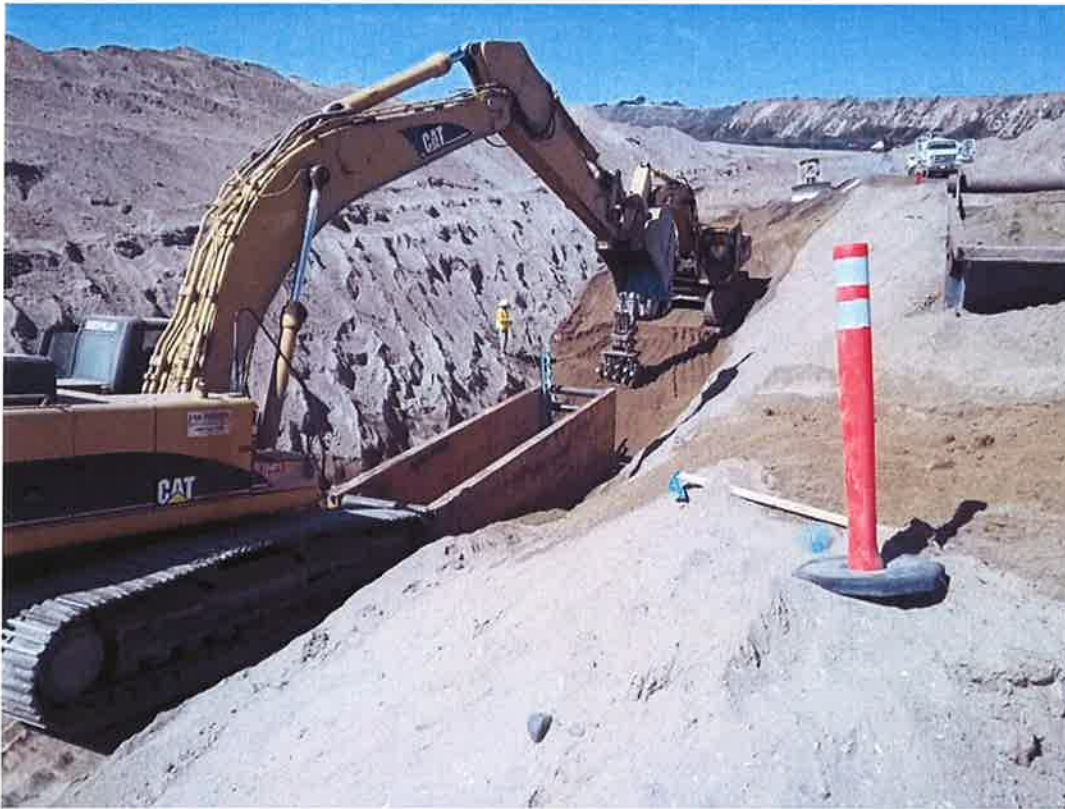
D-KAL continuing excavation and installation of 24-inch DIP in river area.
