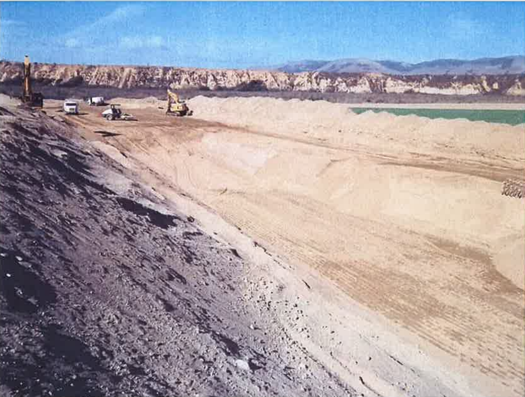
Backfilling of deep trench pipe section in river area.
