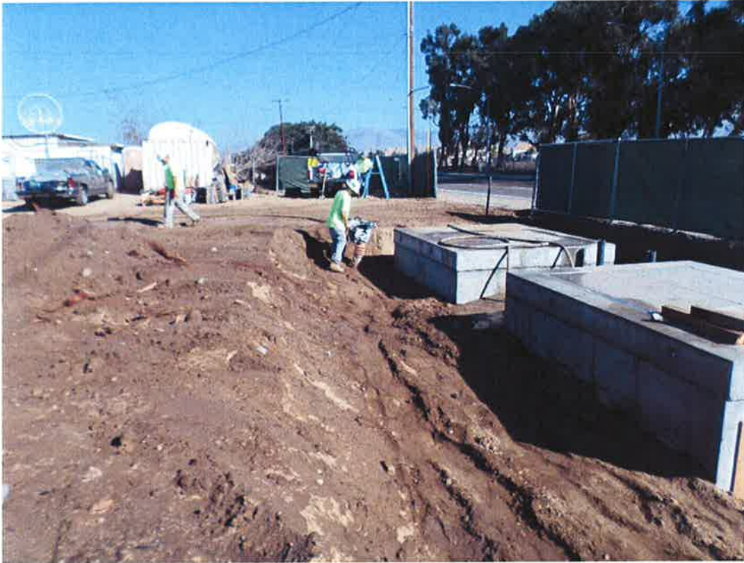
Spiess completing backfill and compaction around vaults.
