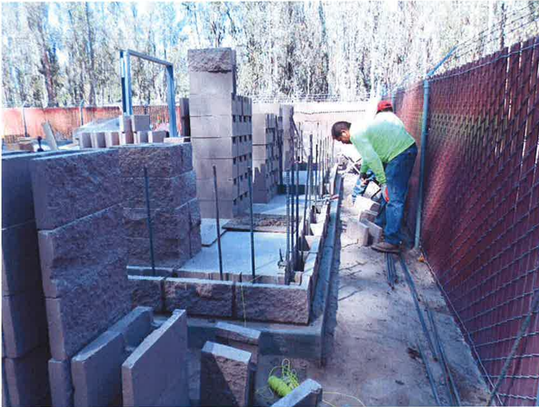
Rocky Boydston Masonry installing first course of block for chemical building.
