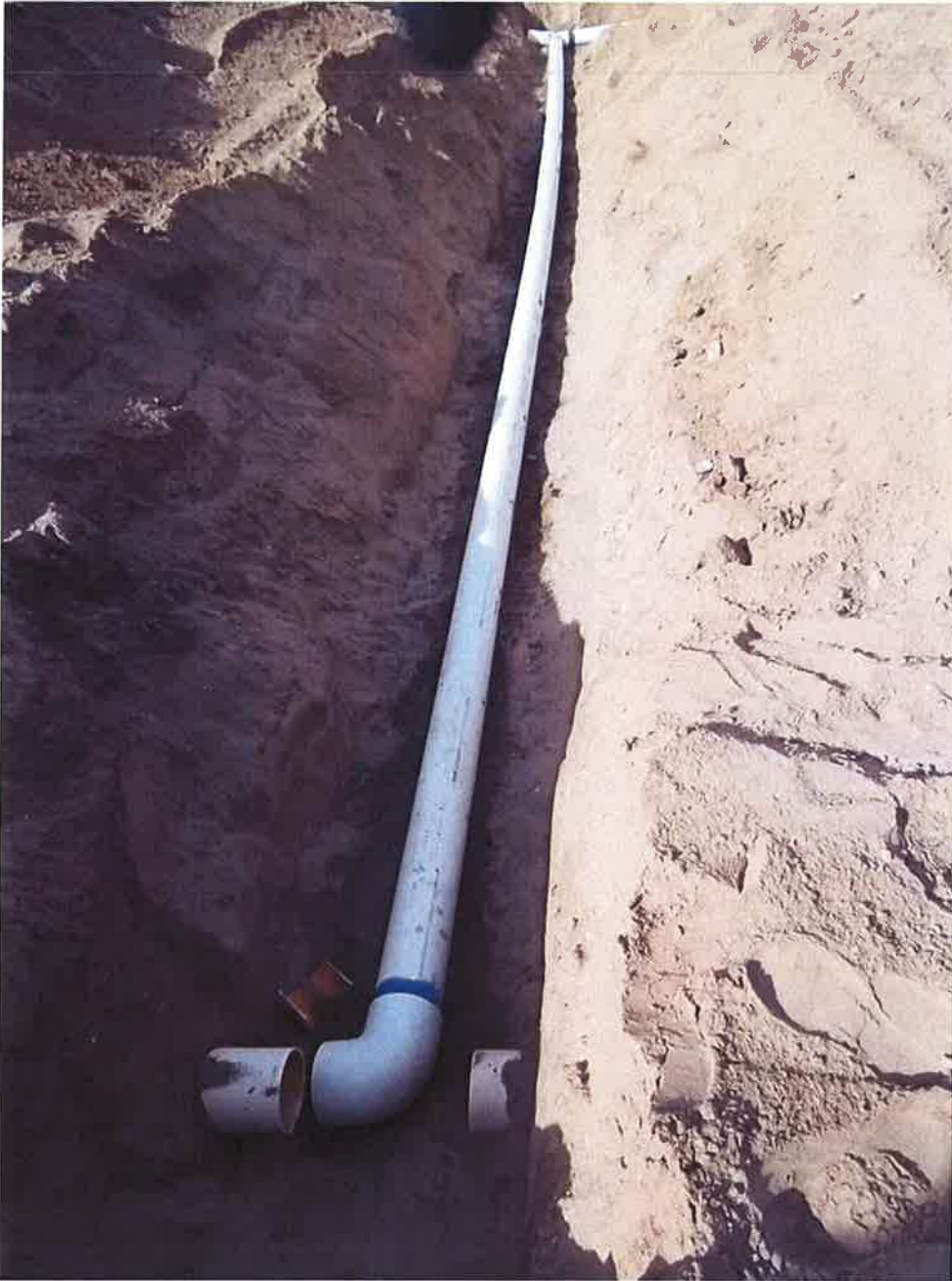
Relocated 8-inch PVC farm irrigation line.
