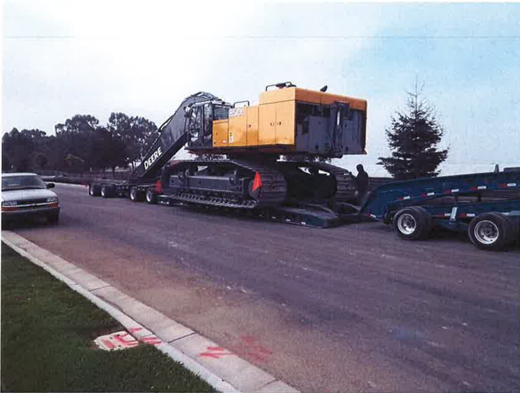
John Deere 850 excavator being delivered to site for bore and jack pit excavation.
