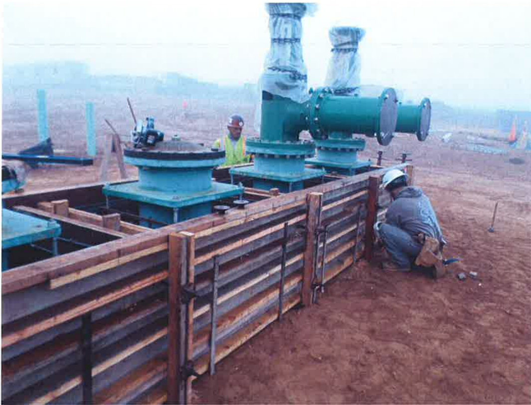
Forms installed for pump pedestals.
