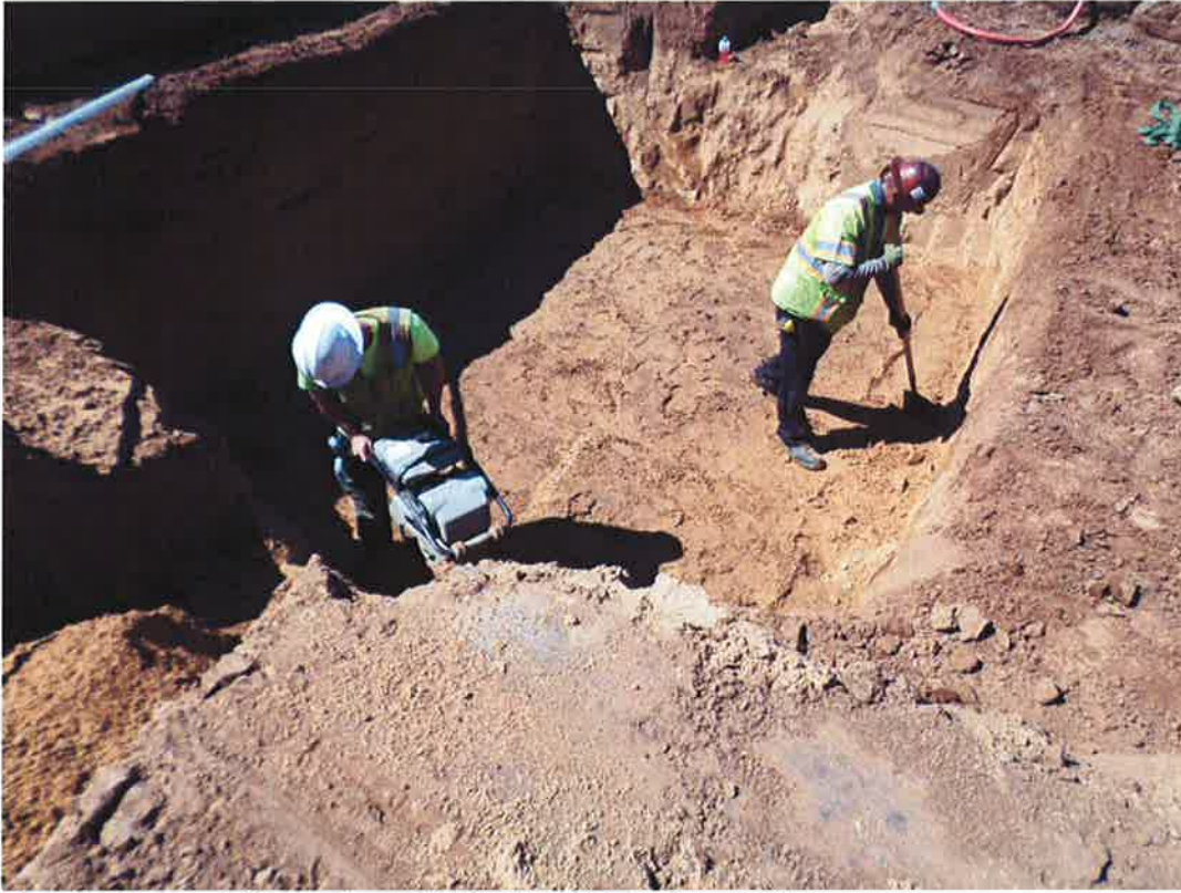
Spies compacting subgrade for the metering vault.
