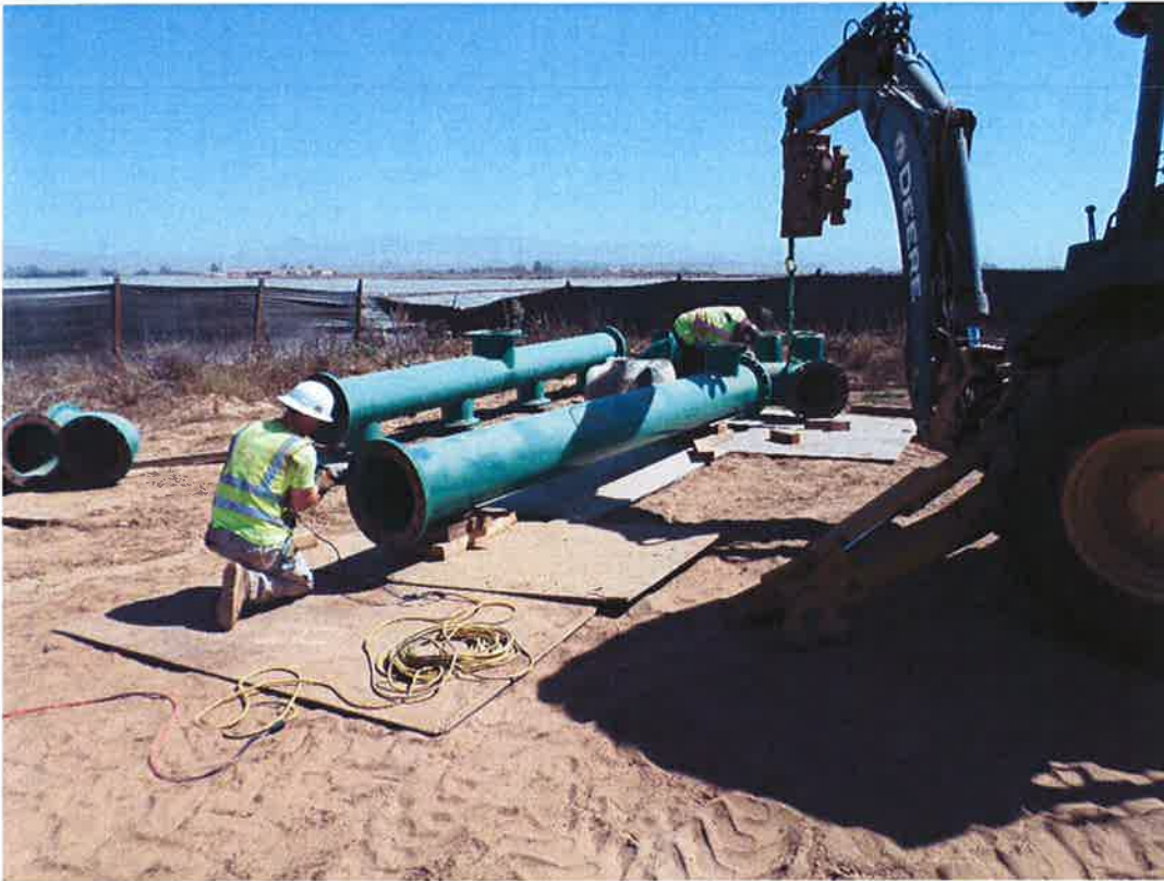
Spiess assembling discharge piping.
