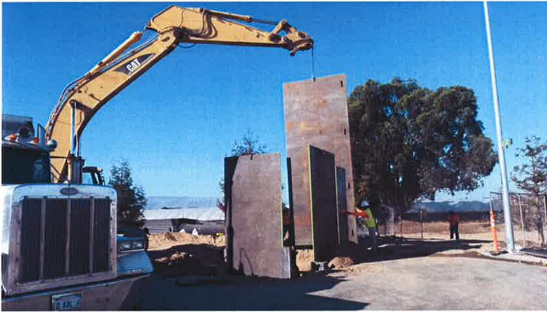
D-KAL installing steel plates as part of shoring in receiving pit.
