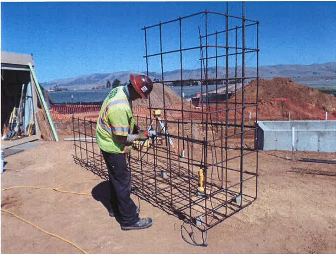
Spiess building rebar for concrete encasement of discharge pipe.
