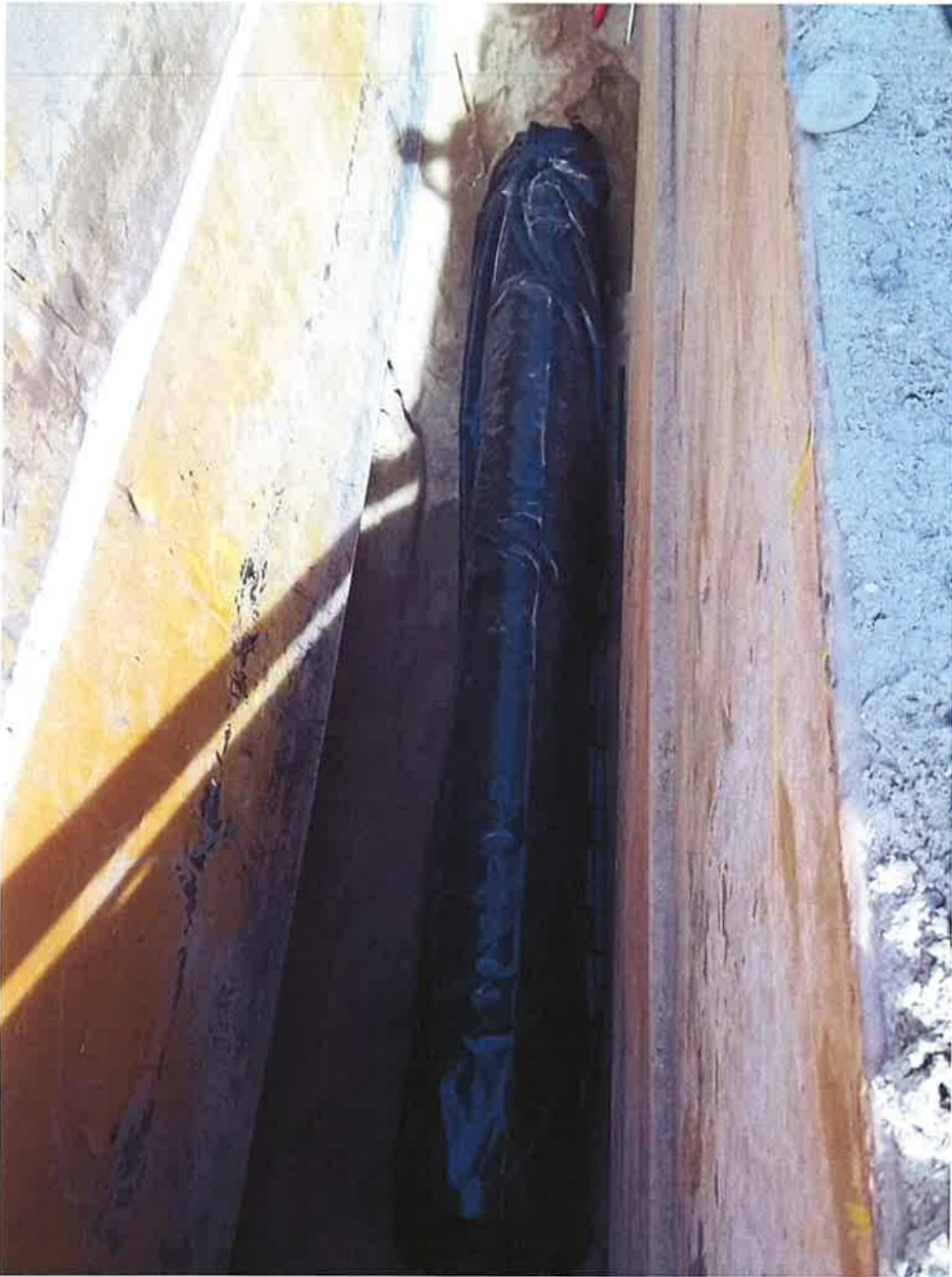
24-inch DIP wrapped in plastic and installed inside shoring.
