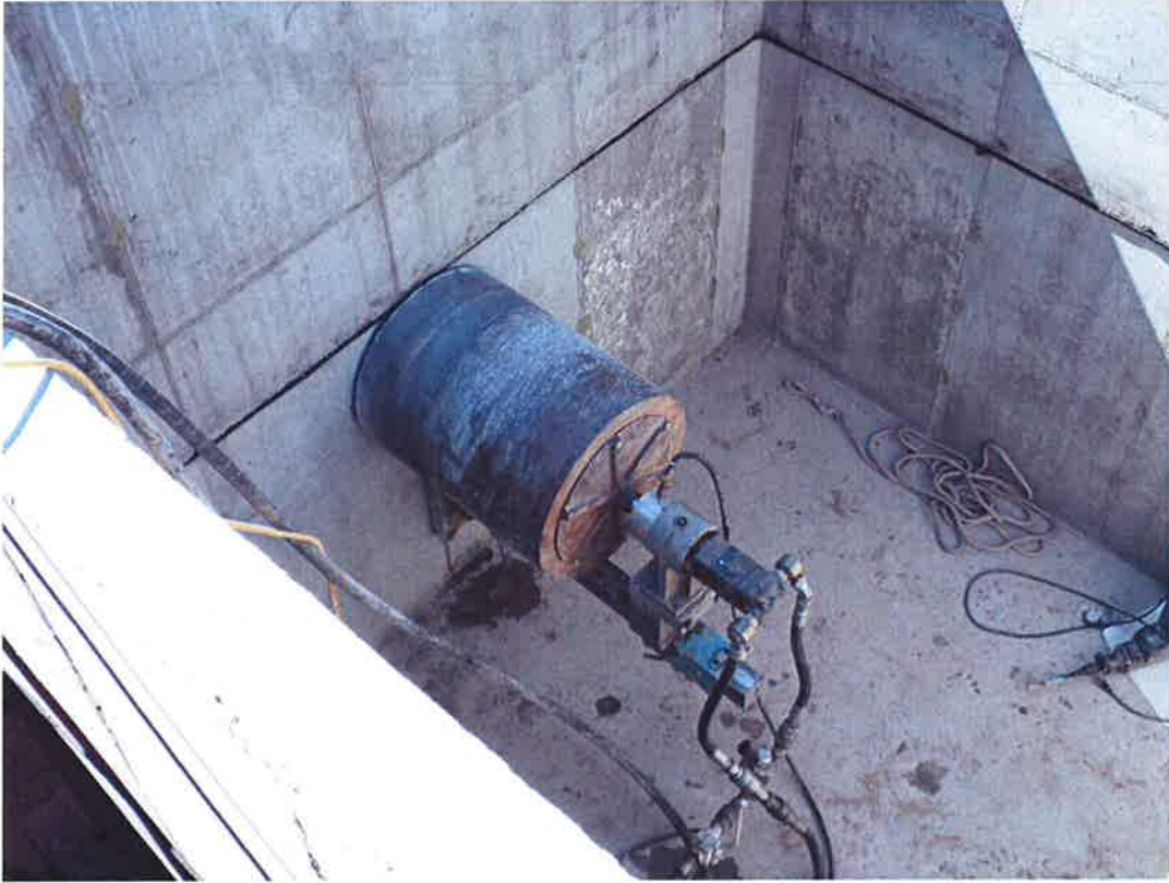
Spieß coring for pipe opening in vaults.
