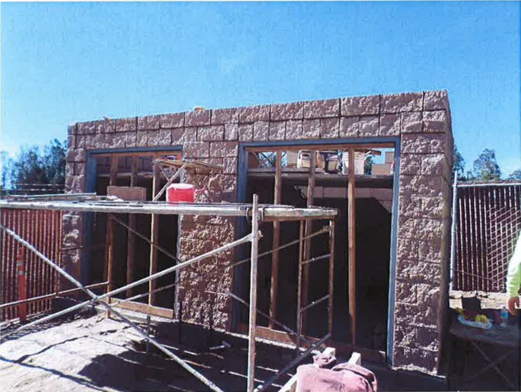
Final course of masonry being completed for the chemical building.
