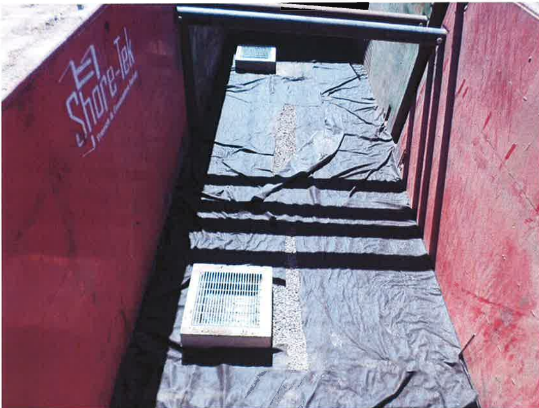
Rock and fabric installed and ready for vault placement.
