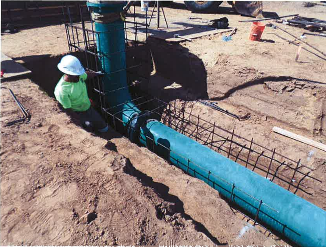
Spieß placing setting discharge pipe inside rebar cage for concrete encasement.
