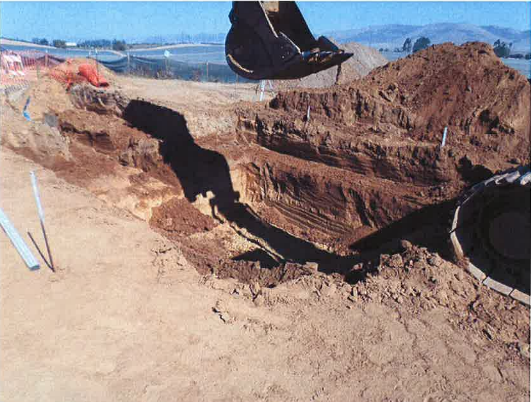
Excavating for metering station vault.
