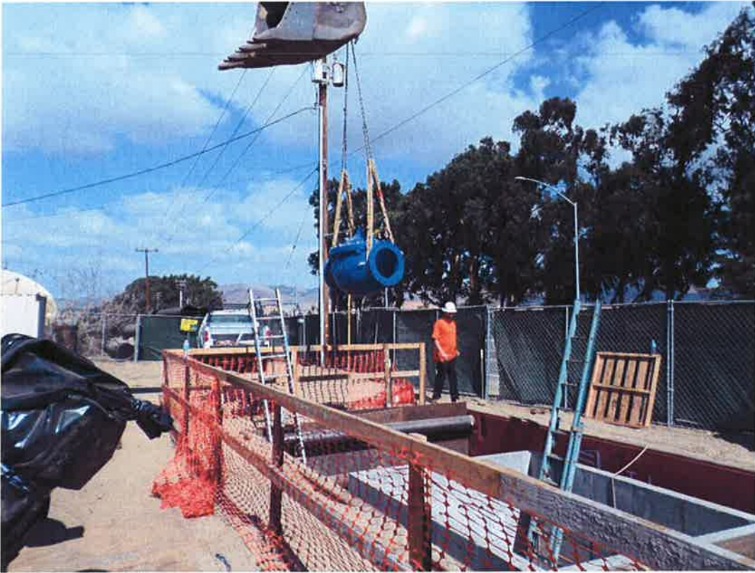
Spieß installing flow control valve.
