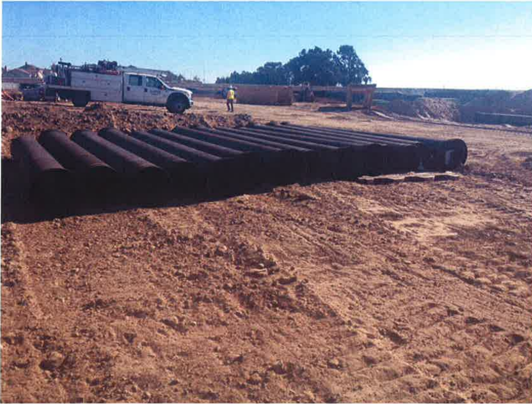
Ductile iron pipe delivered to the river area.
