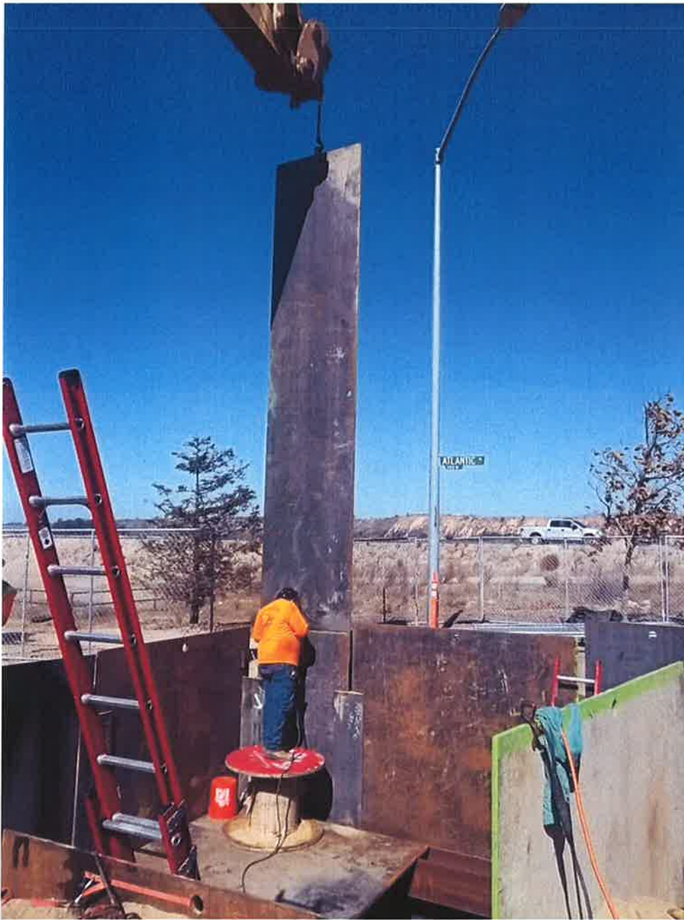
D-KAL welding second layer of steel plates at receiving pit.
