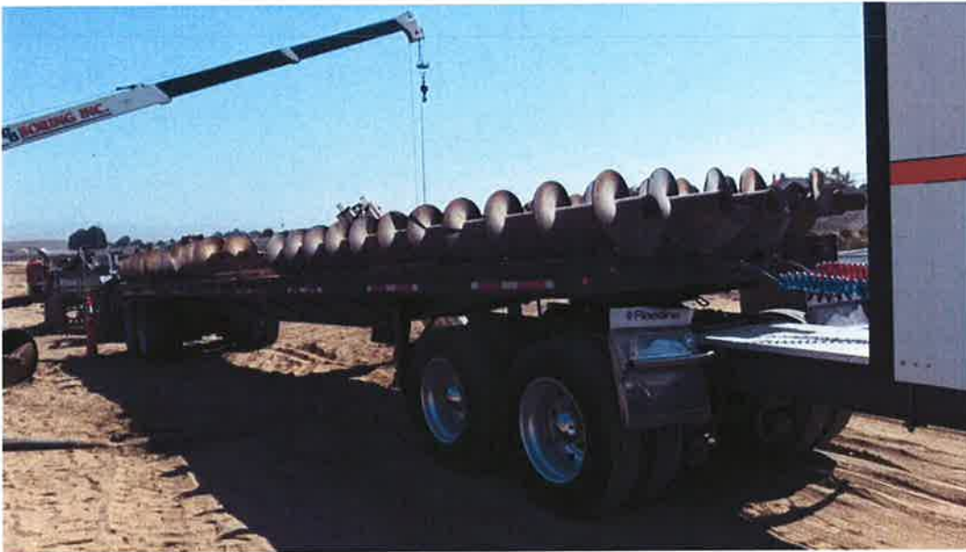
Augers for bore and jack under levee arriving on site.
