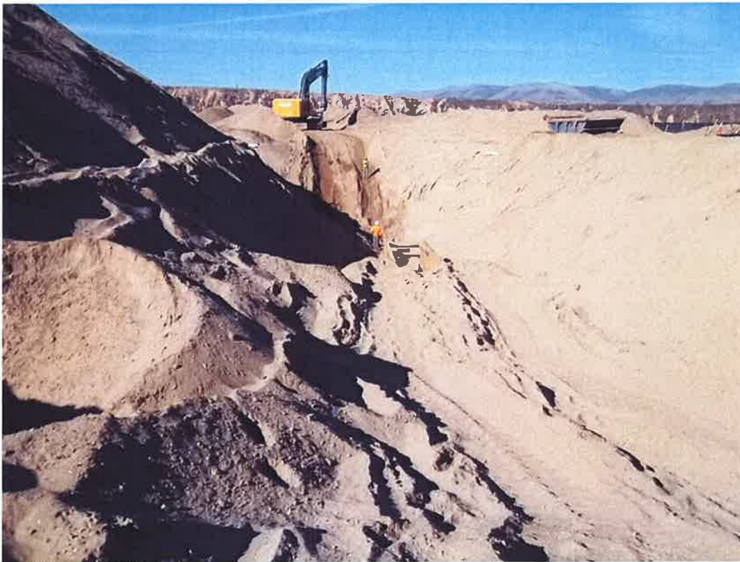
D-KAL backfilling deep trench pipe installation in river area.
