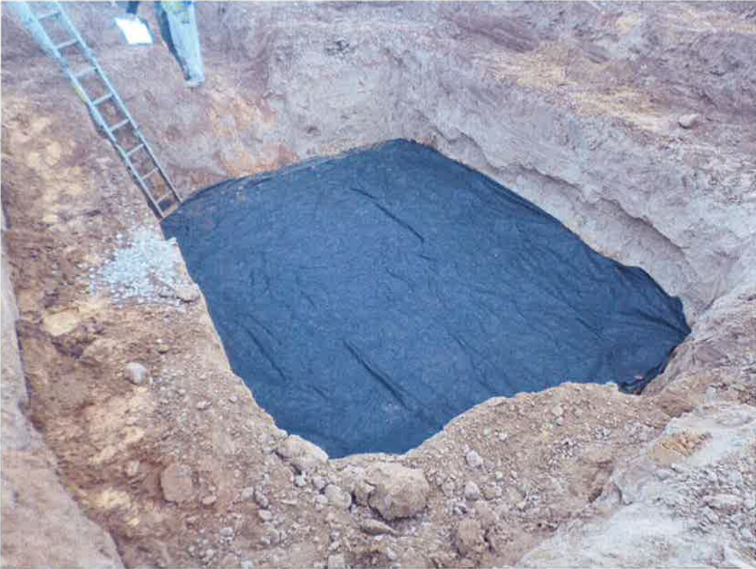
Rock and filter fabric for underneath vault in place.
