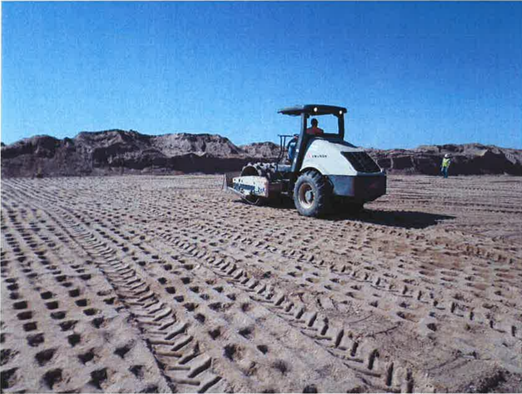
D-KAL compacting area over trench in preparation for top soil restoration.
