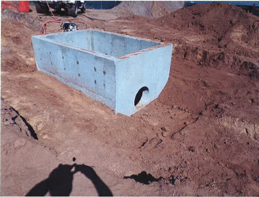
Spiess backfilling around the metering vault.
