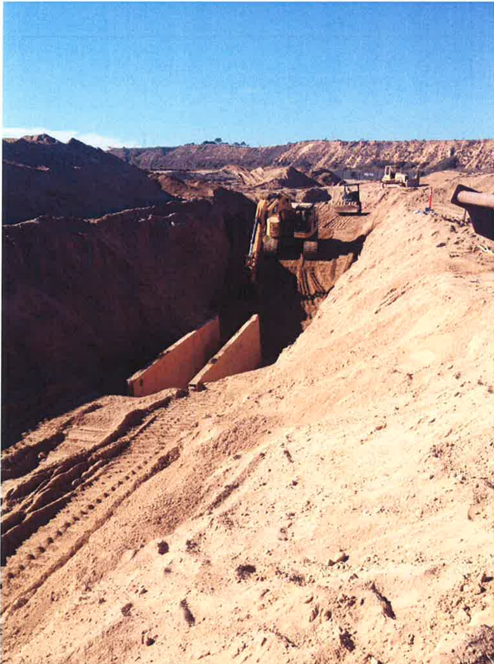
D-KAL installing 24-inch DIP in river area deep trench section.
