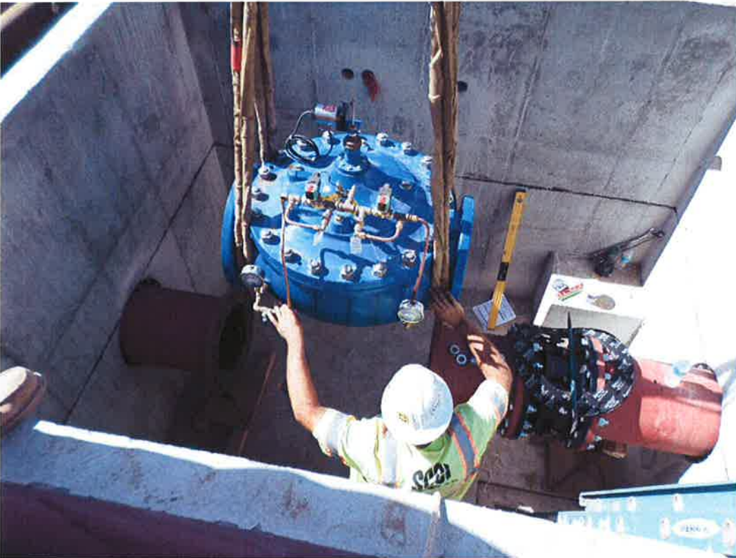
Spieß installing flow control valve.
