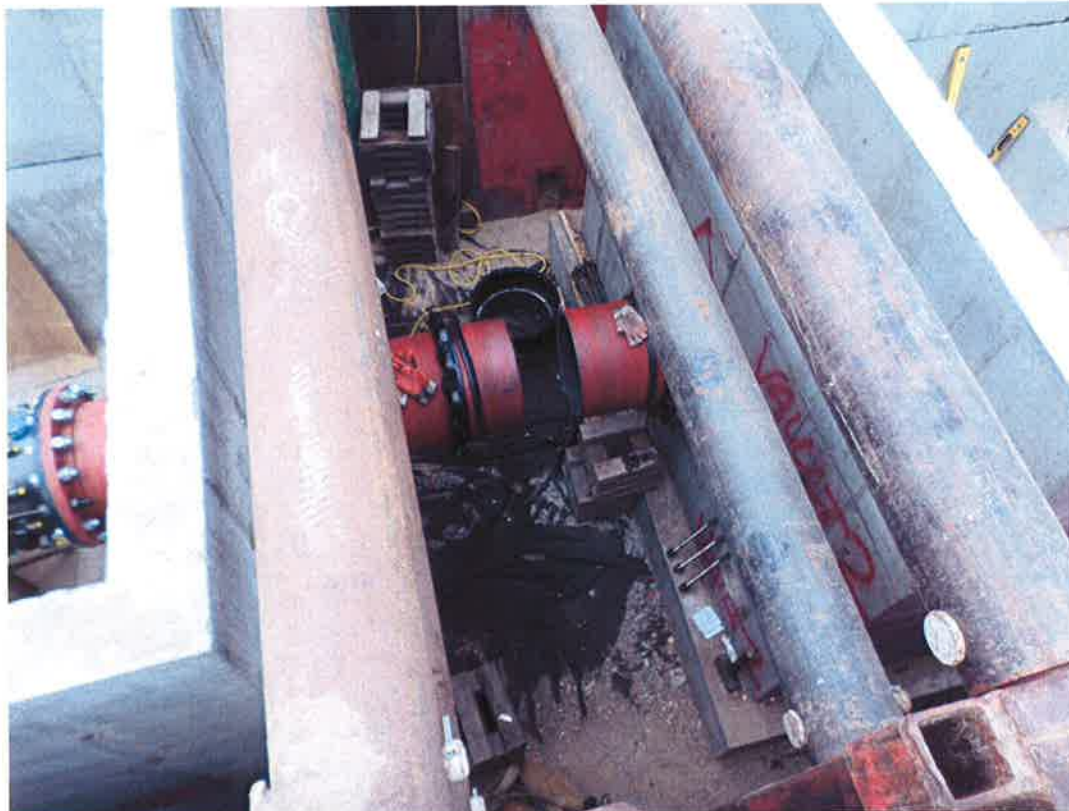
Spiess assembling piping between vaults.
