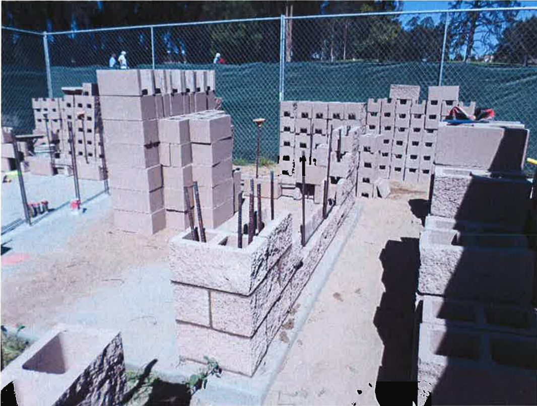
First course of rock being installed at the chemical building.
