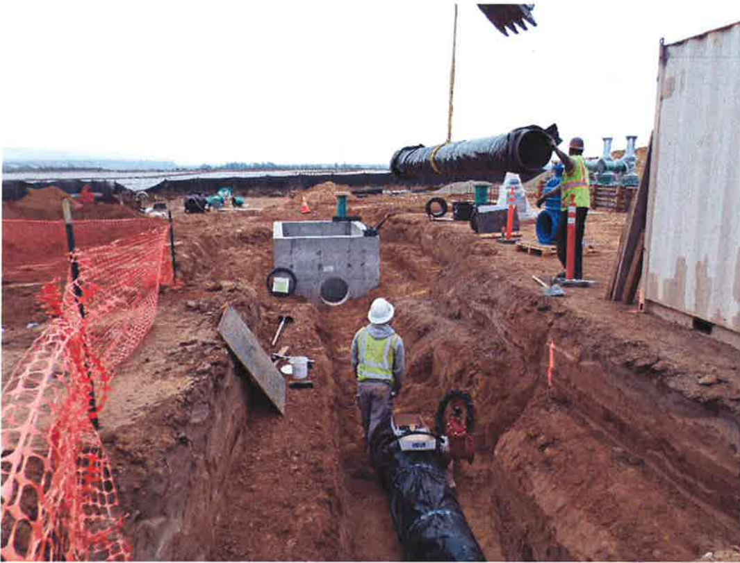
Spiess installing pipe to metering vault.
