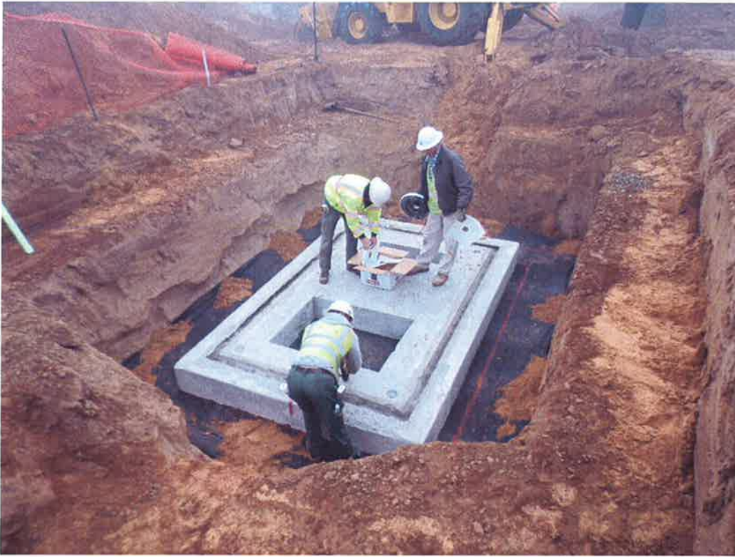
Spiess setting base of metering vault.
