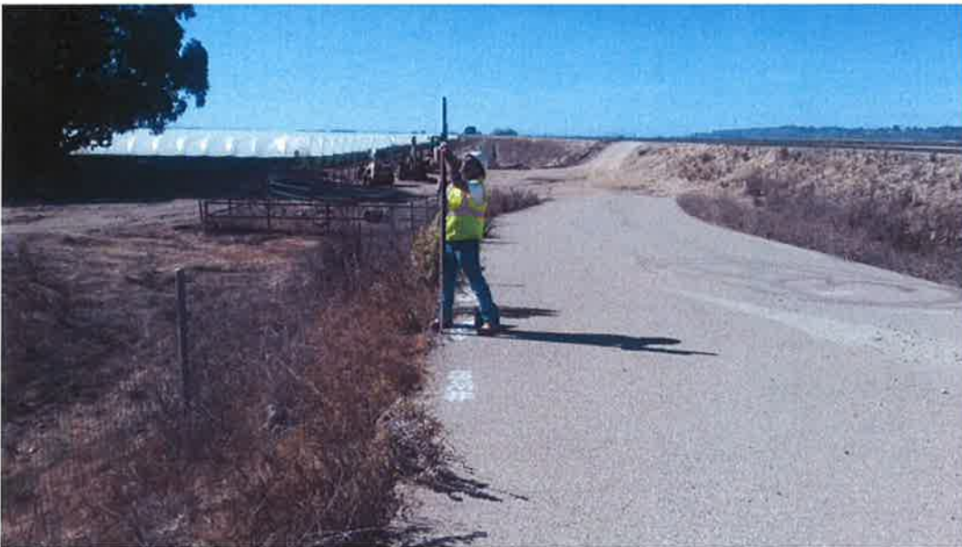
D-KAL taking settlement monitor readings.
