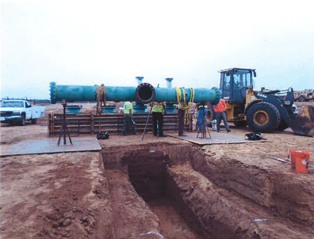
Spies aligning manifold and excavating for discharge pipe and encasement.
