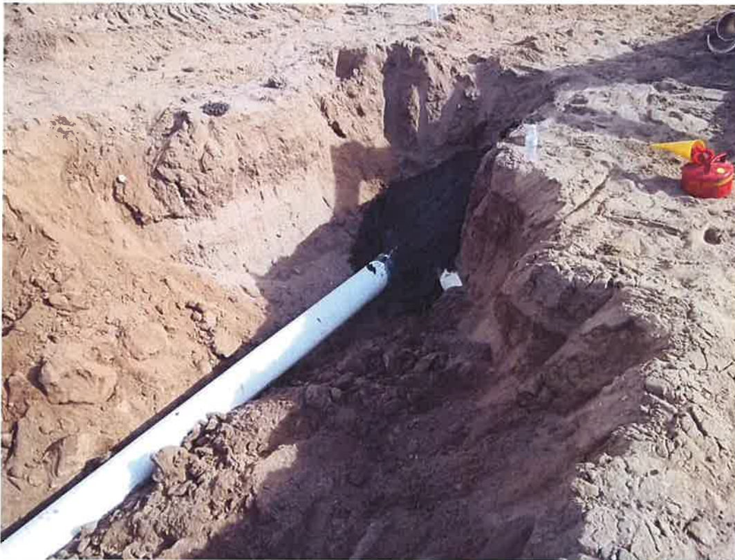
D-KAL pouring temporary thrust blocks on relocated irrigation line.
