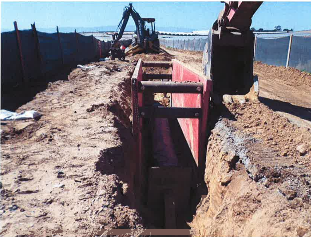
Spieß continuing installation of 24-inch DIP in access road.
