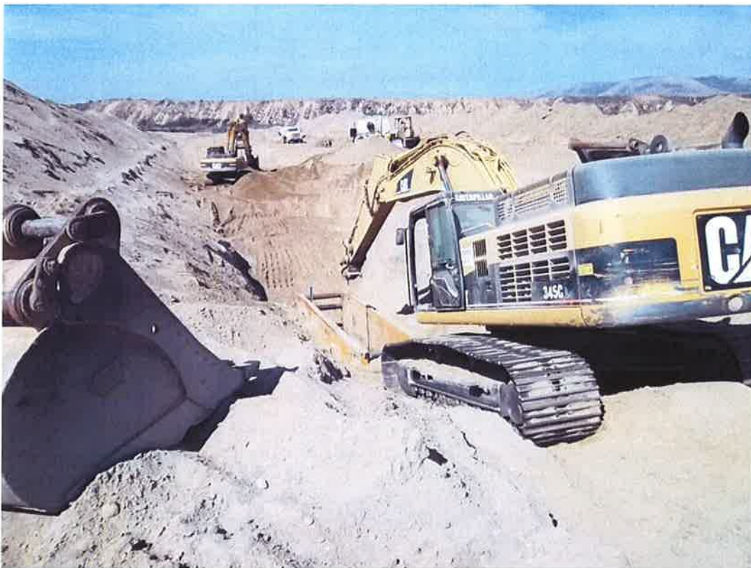
Ductile iron pipe installation in river area.
