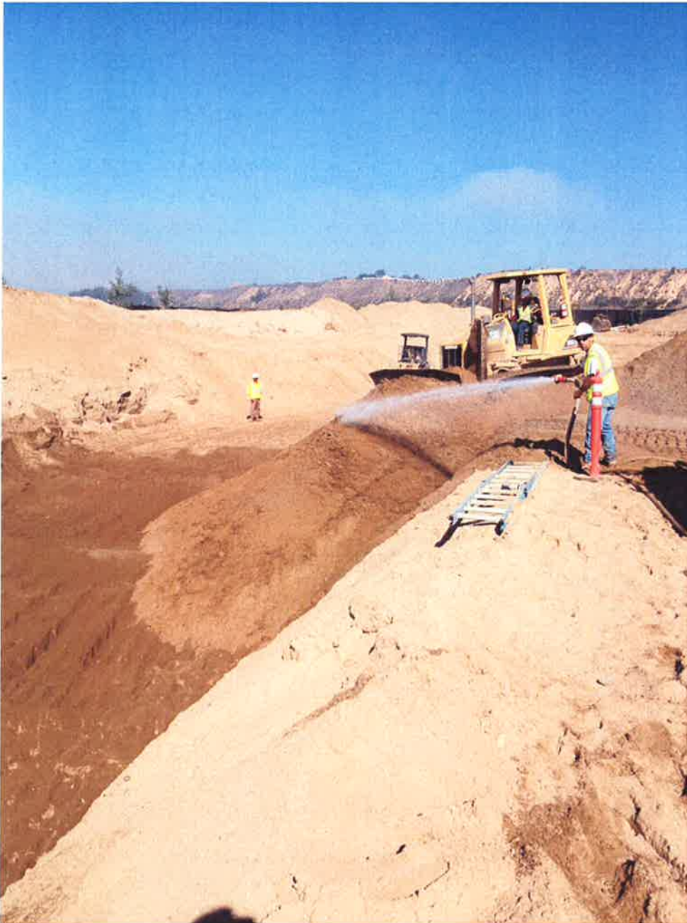
Moisture conditioning backfill material for compaction over 24-inch DIP.
