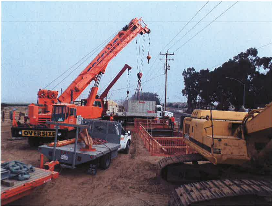
Spieß setting vaults which weigh approximately 26,000 lbs each.
