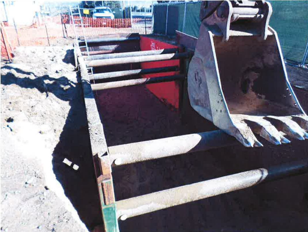
Spiess installing shoring for vaults excavation.
