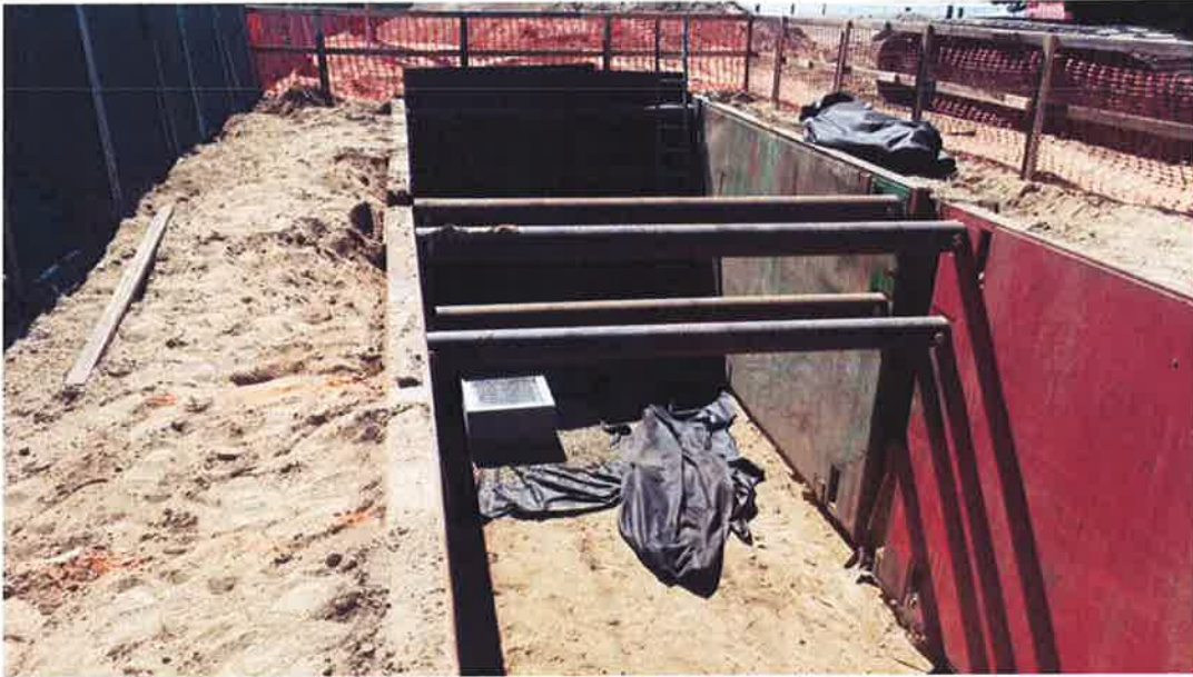
Sump boxes positioned and set for vault placement.
