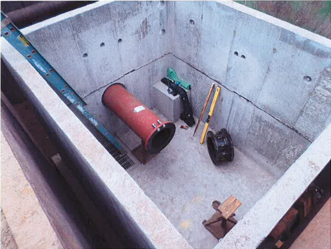
Assembling vault piping.
