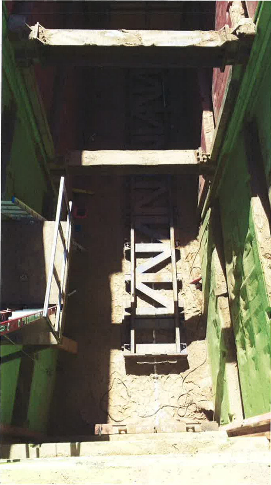
Pacific Boring setting track inside bore and jack pit.
