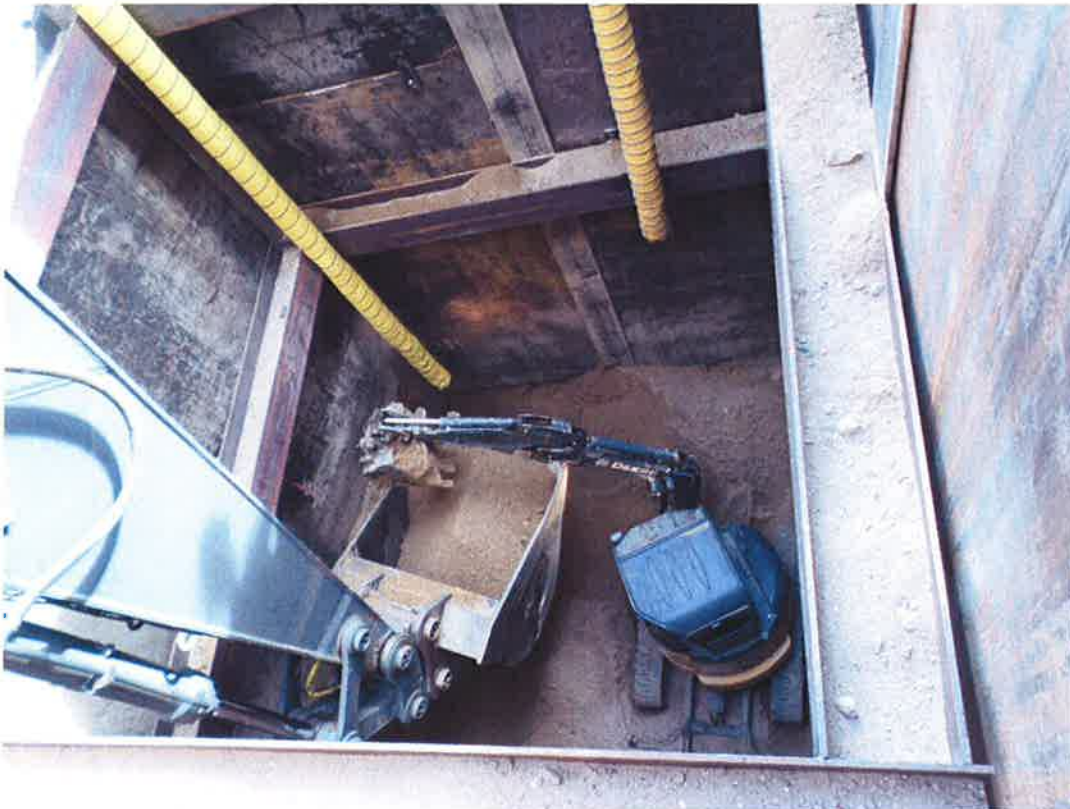
D-KAL using John Deere 850 excavator to excavate material from the receiving pit.
