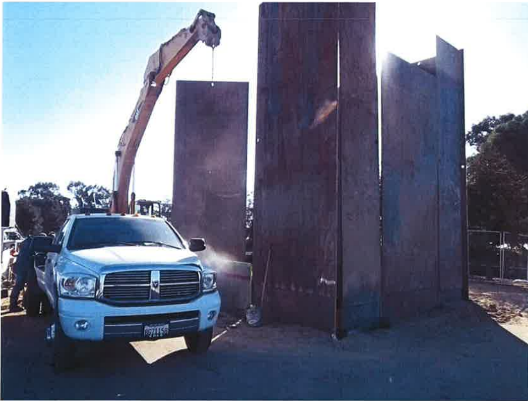
Second layer of steel plates being installed at receiving pit.
