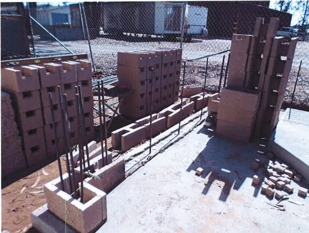
Rocky Boydston Masonry starting first course of block installation.
