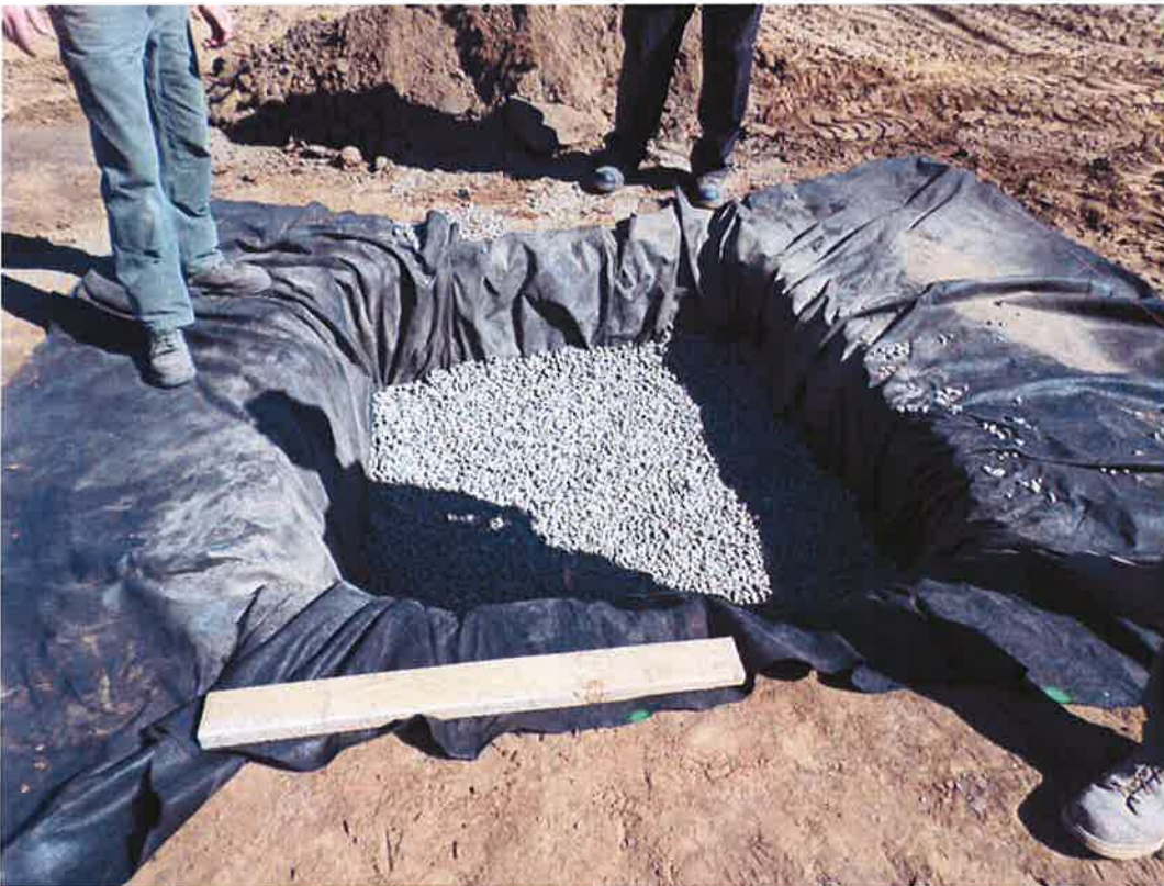
Spiess rock and fabric installed for base underneath catch basin.
