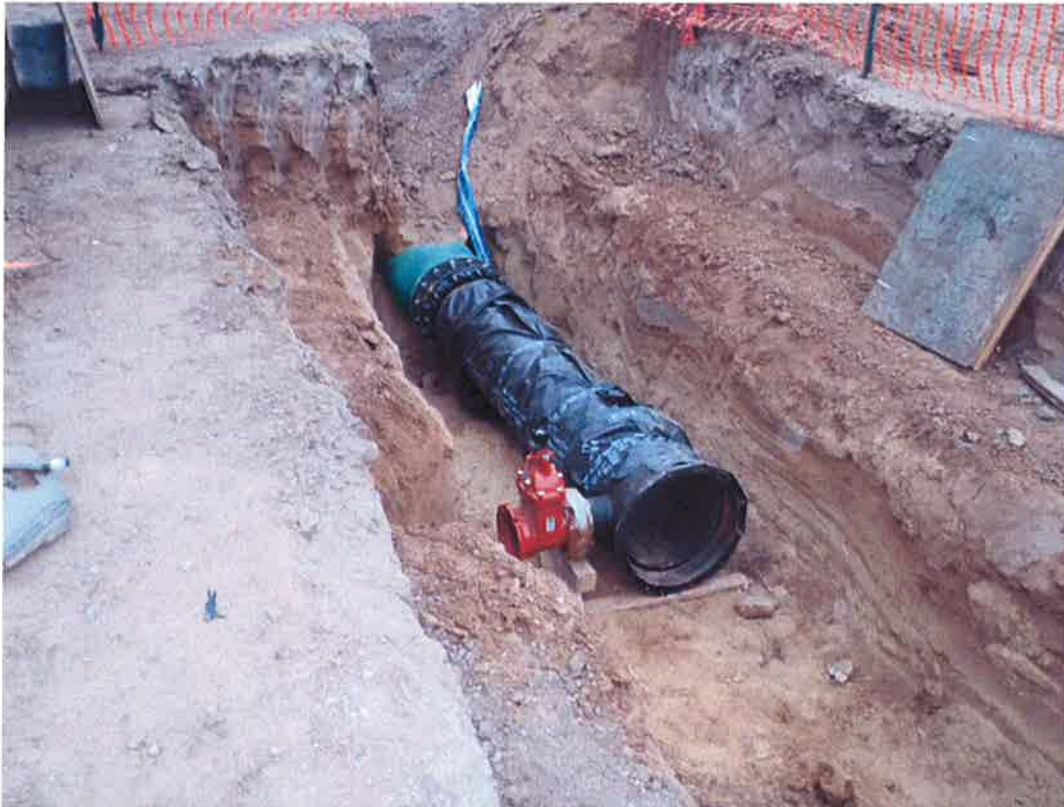
Spiess installing piping toward metering vault.
