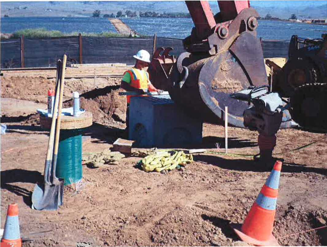
Spiess setting catch basin for site drainage.
