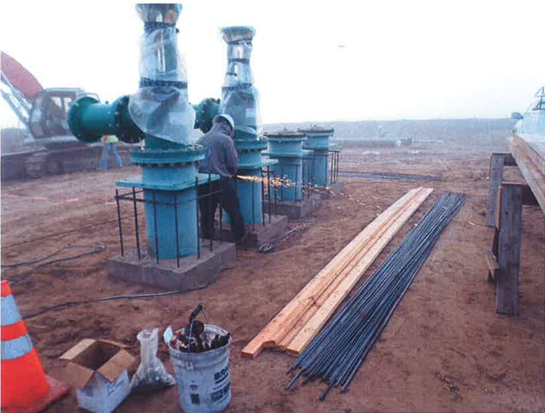
Spies preparing reinforcing for pump pedestals.
