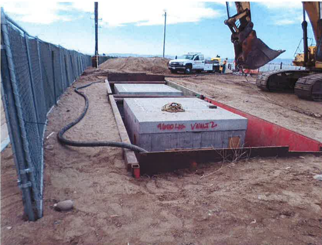
Lids placed on vaults.
