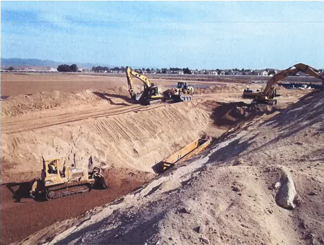
Ductile iron pipe installation in river area.
