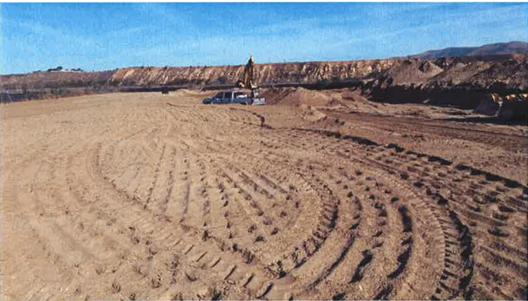
D-KAL restoring agricultural topsoil behind the pipe installation operation.
