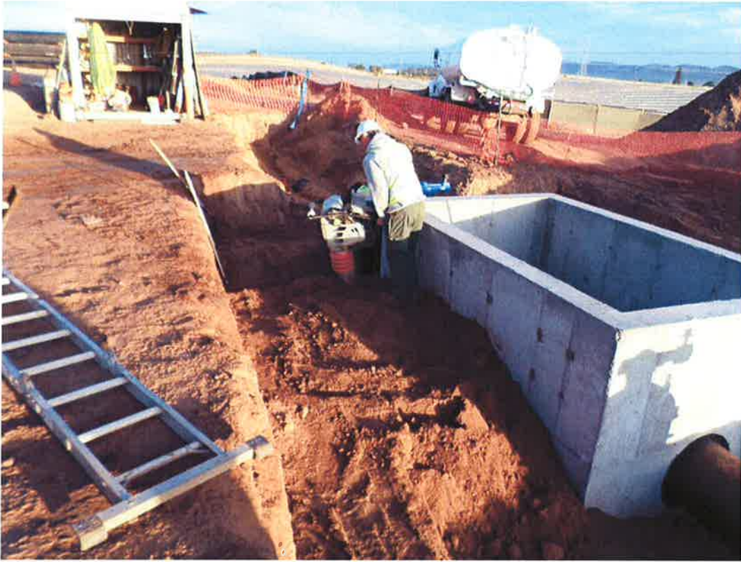
Spieß compacting around the metering vault.
