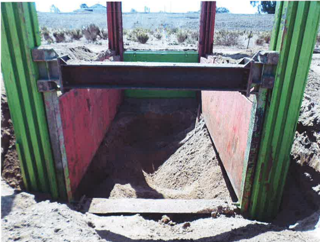
Slip shoring installed during bore and jack pit excavation.
