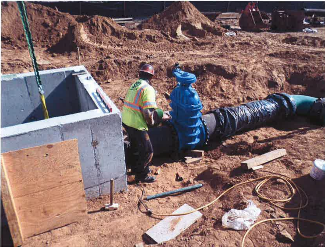
Spiess installing discharge piping and valve to metering vault.
