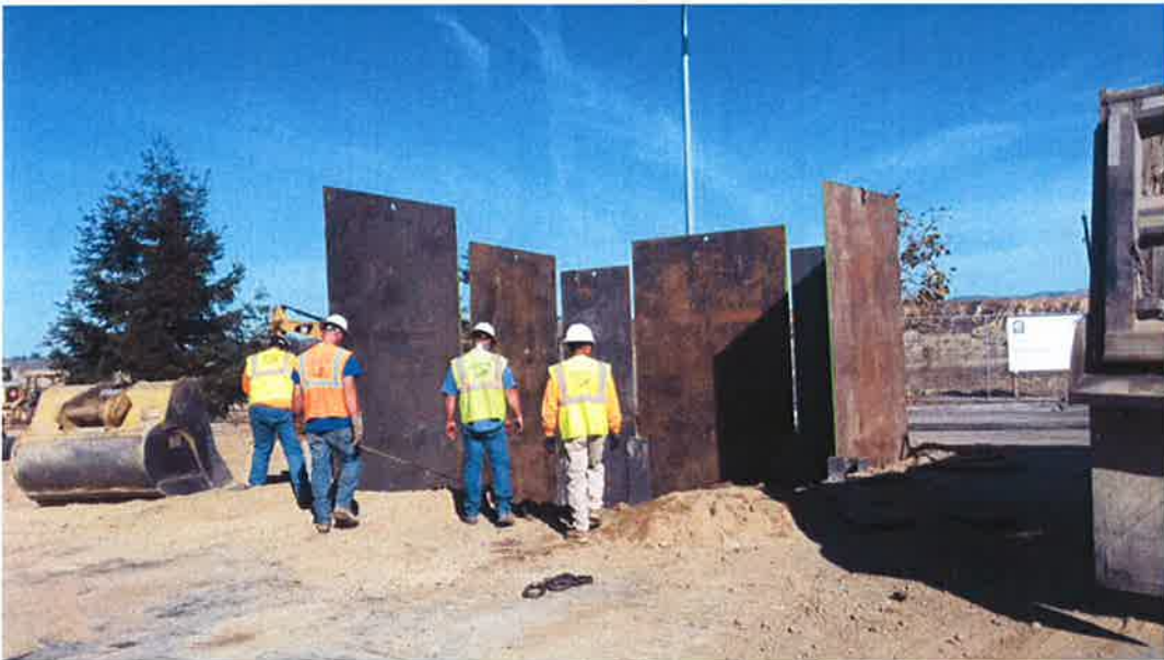
D-KAL installing receiving pit shoring in Blosser Road.
