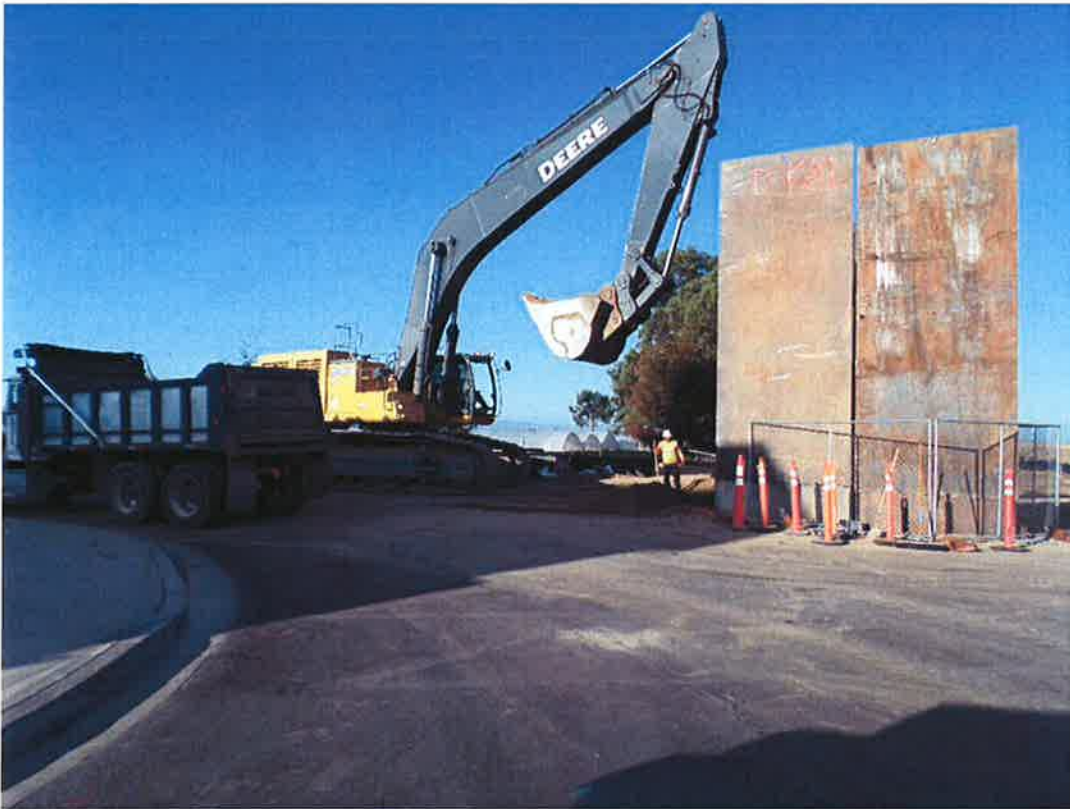
D-KAL using John Deere 850 excavator to excavate material from the receiving pit.
