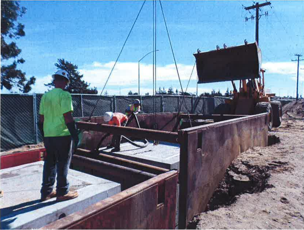
Spieß pouring slurry around vaults for backfill.
