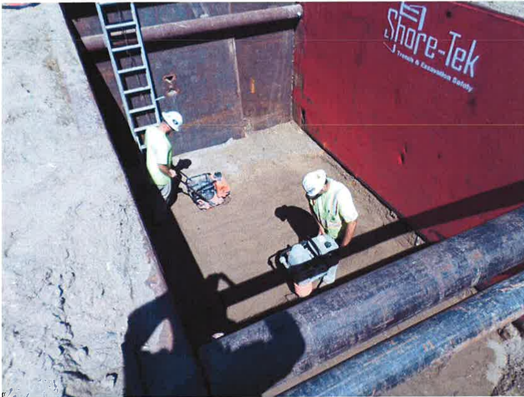
Spieß compacting the base underneath the vaults.
