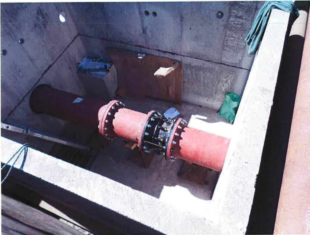
Spiess assembling piping in metering vault.
