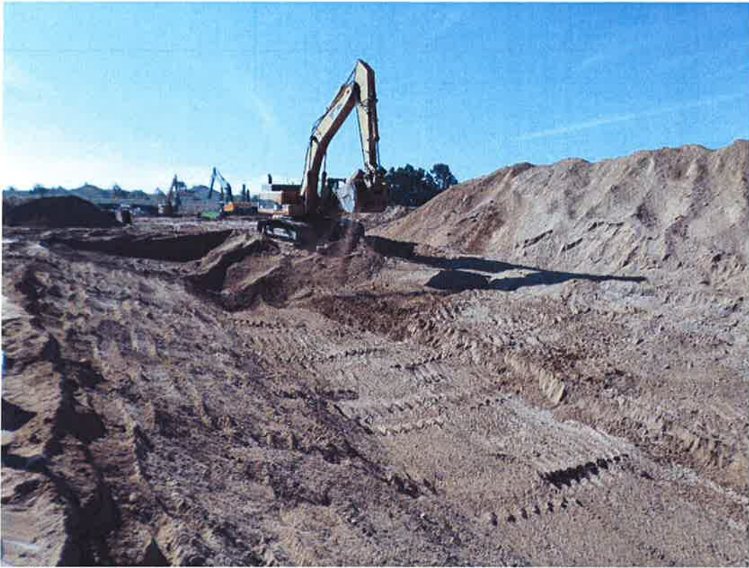
D-KAL creating bench for deep pipe trench in river area.
