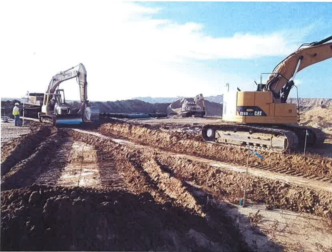
D-KAL removing and preserving agricultural topsoil.
