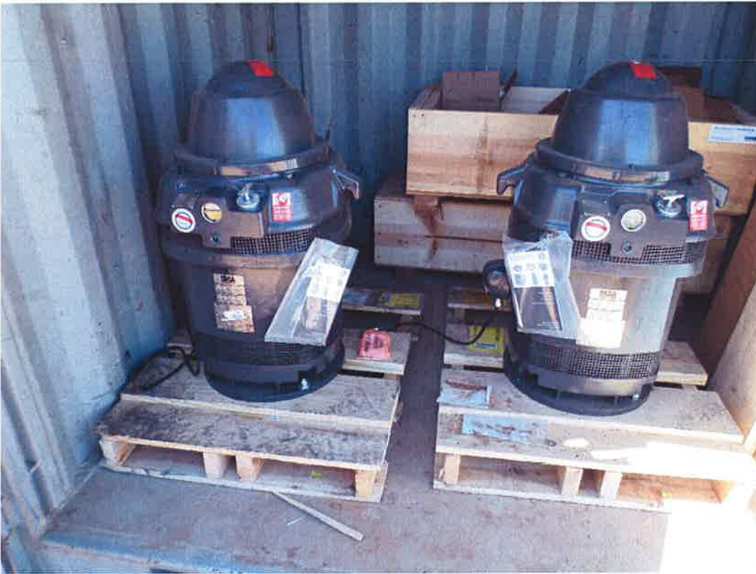
Pump motors being energized while being stored on site.
