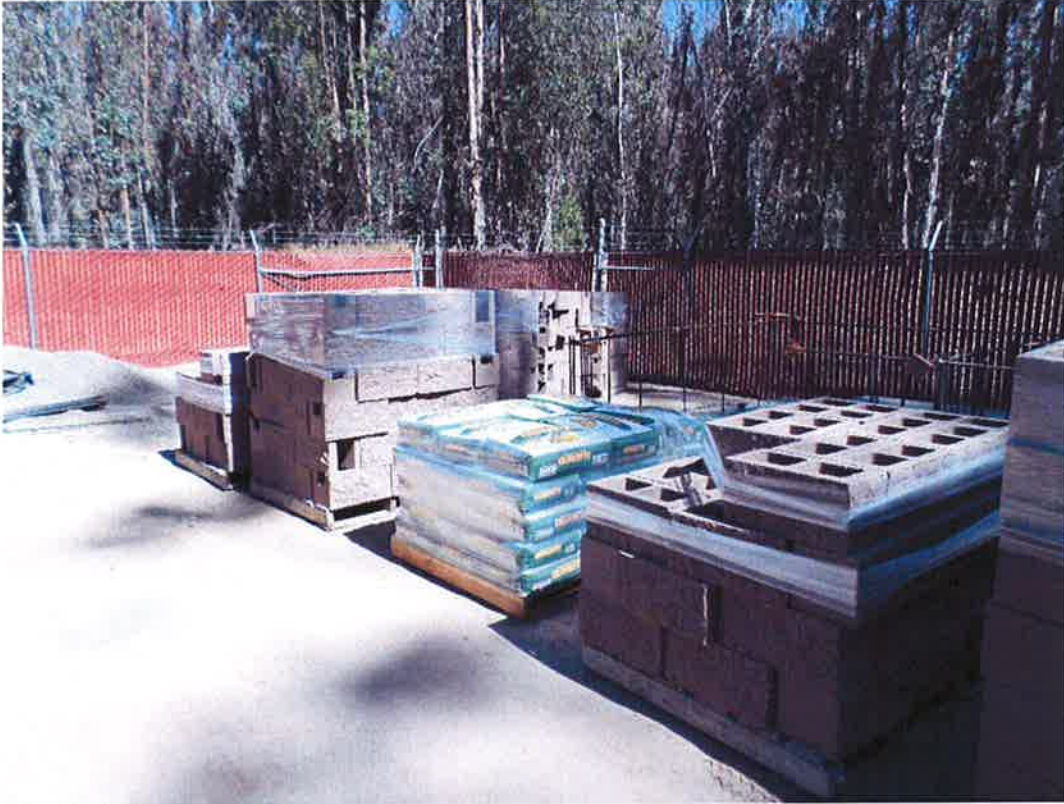
Block delivered to the site.
