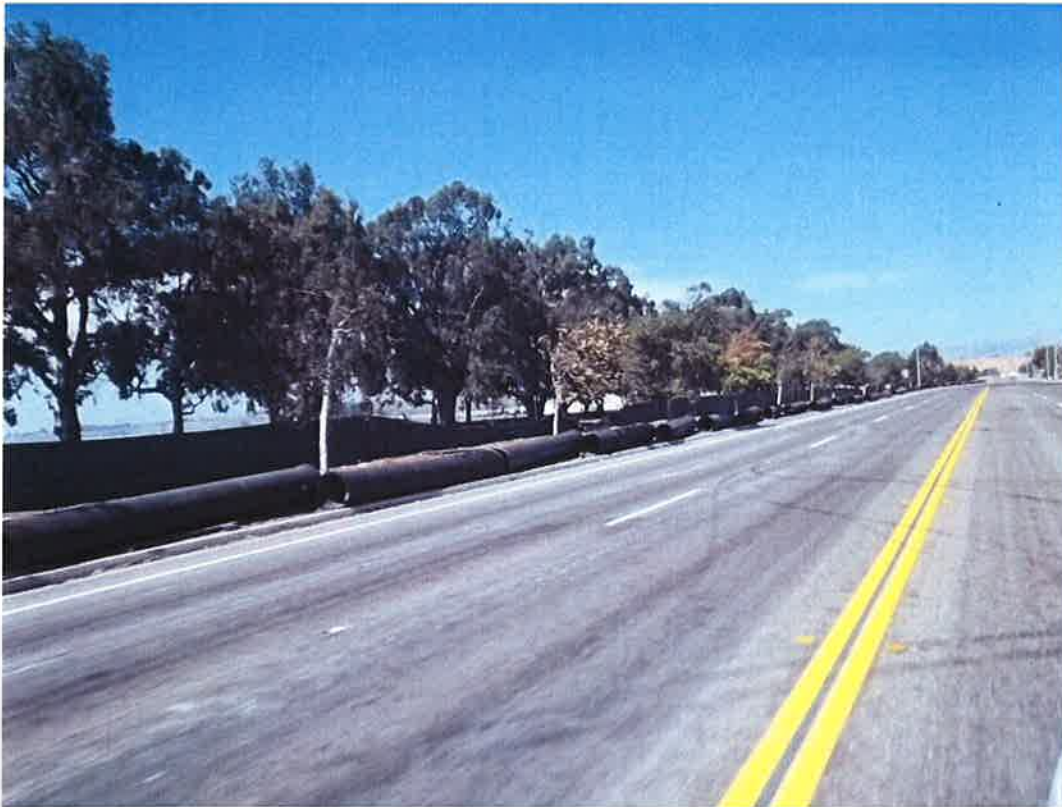
Ductile iron pipe delivered and staged along Blosser Road.
