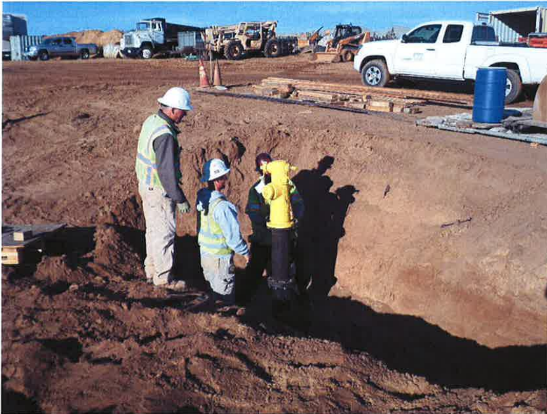
Spiess installing the fire hydrant.
