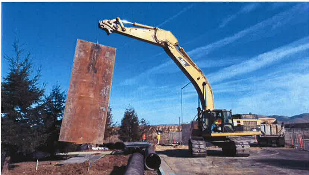
D-KAL installing steel plates for shoring in receiving pit.
