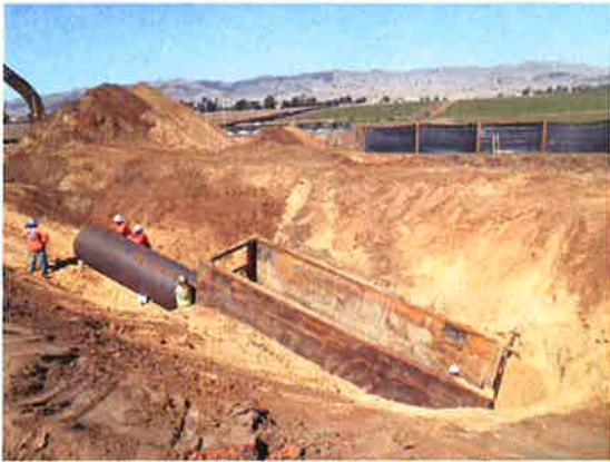
Figure 4. Conductor barrel in side-sloped trench.
