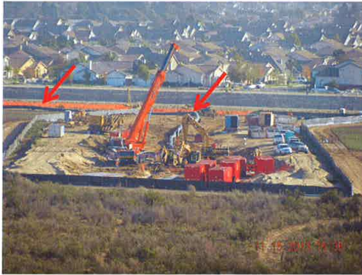
Figure 11. Pipe snaked along access road prior to pullback.
