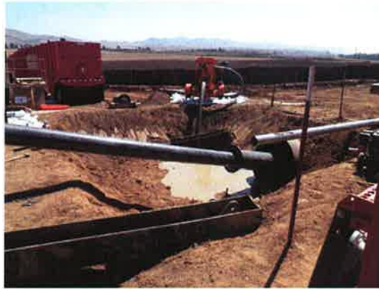
Figure 5. 16-inch (405 mm) casing centralized in the conductor barrel .
