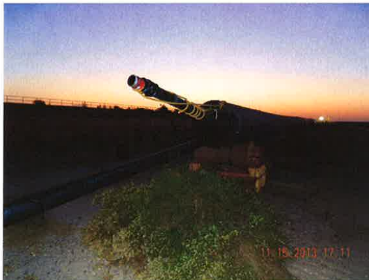
Figure 9. Water fill bottom line and rope-restrained air line top.
