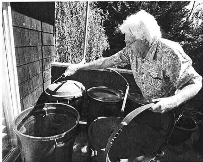
Bill Seavey of Cambria with one of his rainwater catchment systems that he built himself. The pipe he is holding is connected to the house's rain gutter and swivels so it can fill up any of these 32 gallon garbage cans. JOE JOHNSTON — jjohnston@thetribunenews.com | Buy Photo
