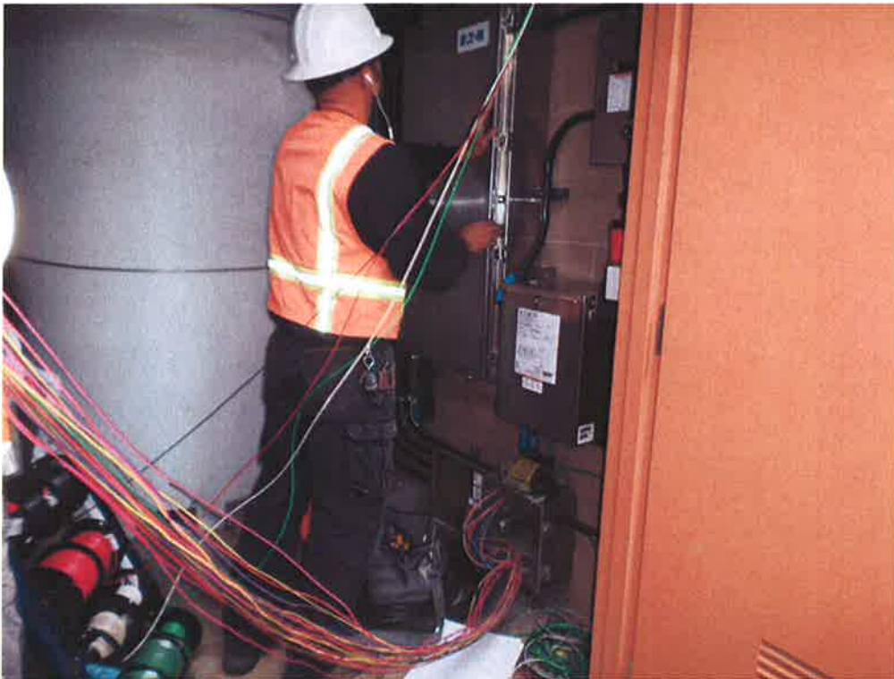
St. Denis Electric pulling wire.
