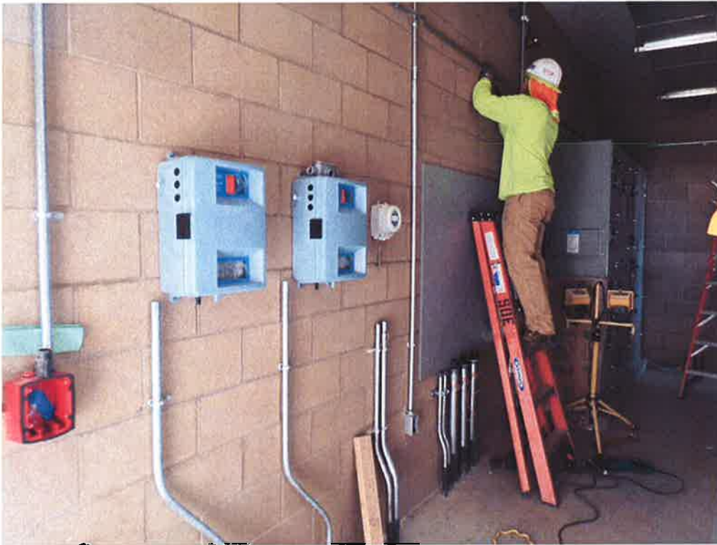
Installing exposed conduit in electrical room.
