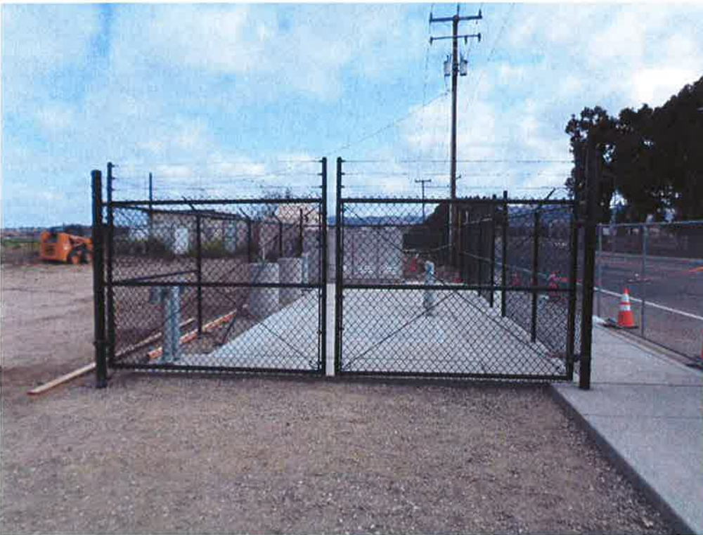
Vehicle access gate installed.
