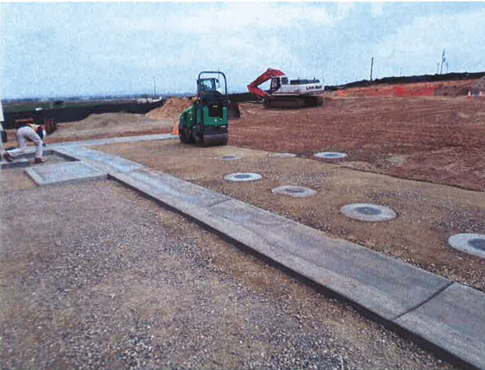
Compacting aggregate base.
