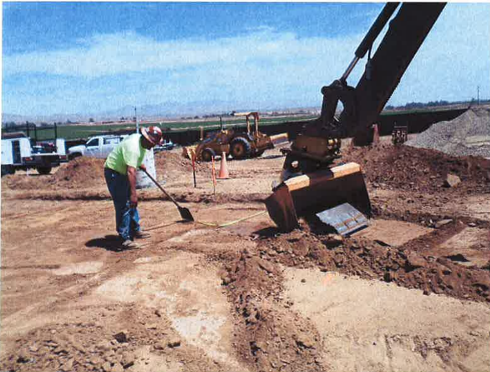
Spiess starting excavation for V-ditch.
