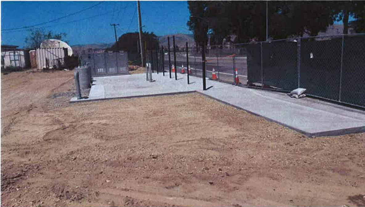
Driveway with forms removed and site graded.
