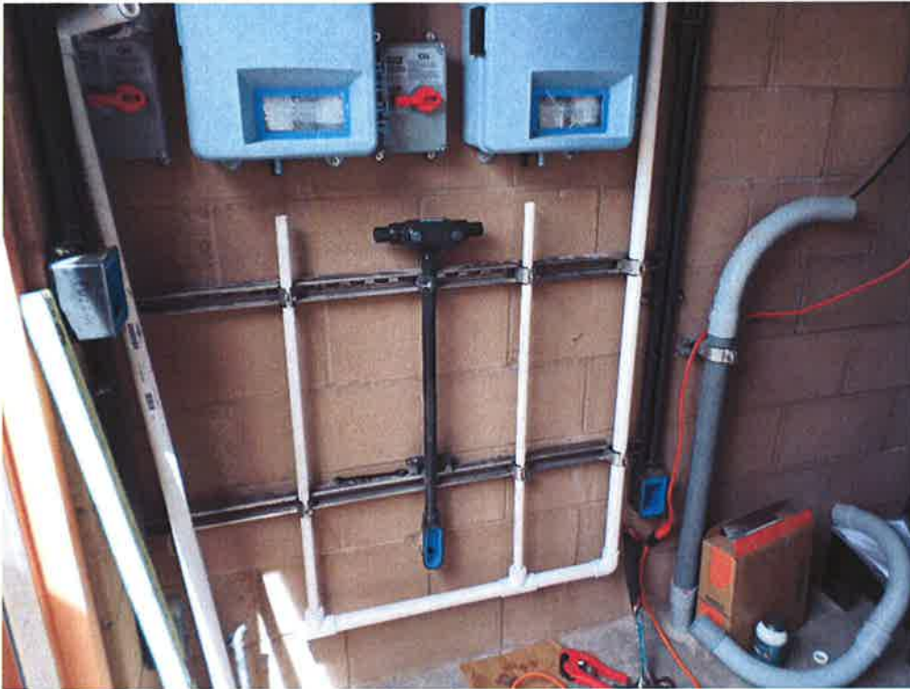
Chemical analyzer piping being installed.
