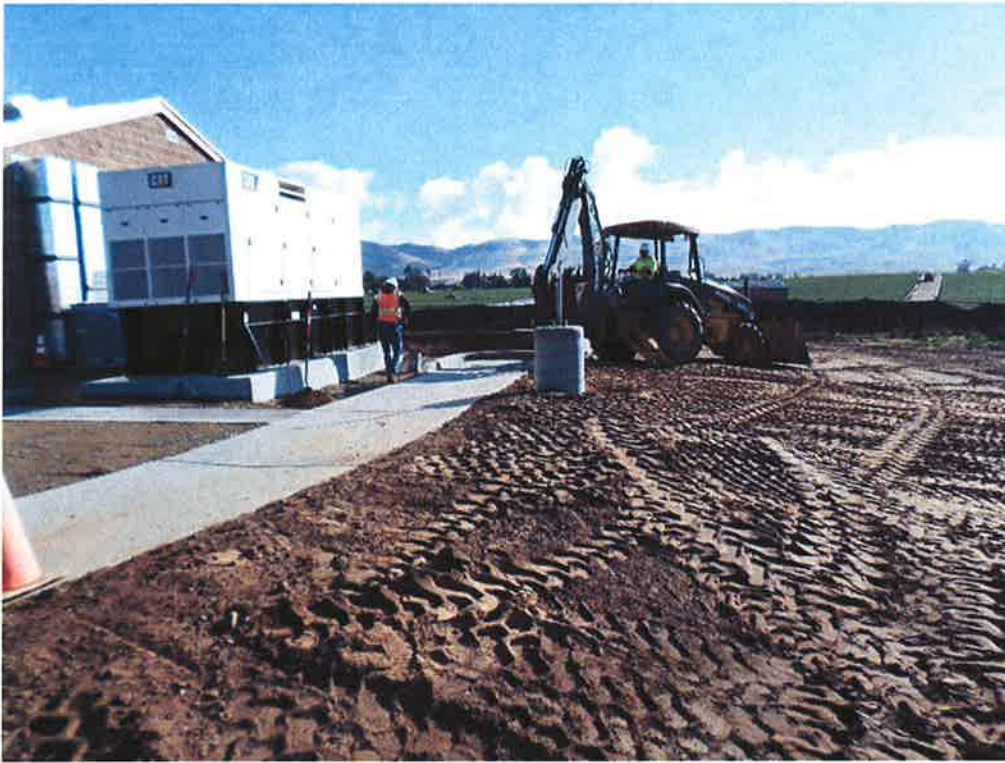
Grading bank between facilities and future fence.
