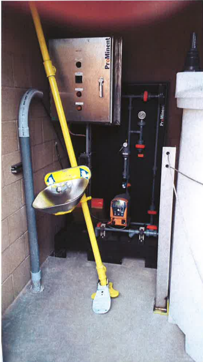
Ammonium sulfate chemical skid installed (eye wash station assembled).
