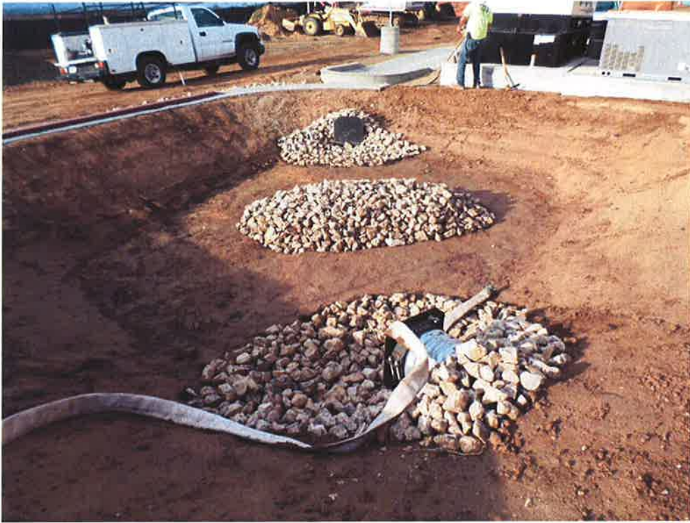
Fabric lined rock drain in retention basin completed.
