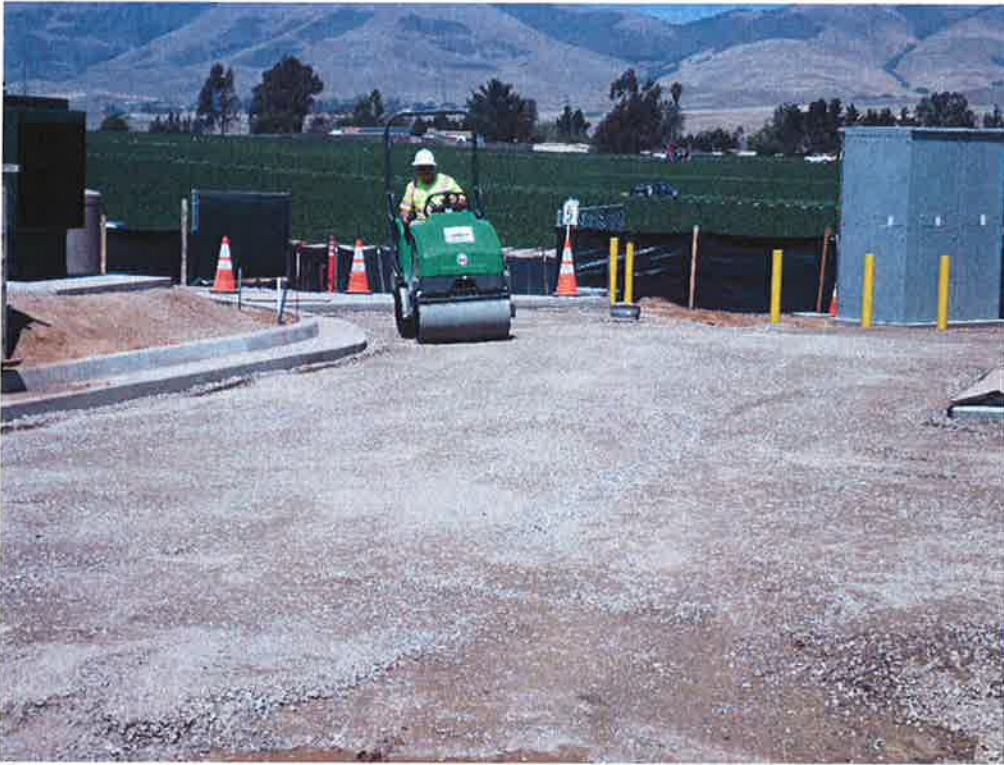
Spiess compacting aggregate base for driveway around building.
