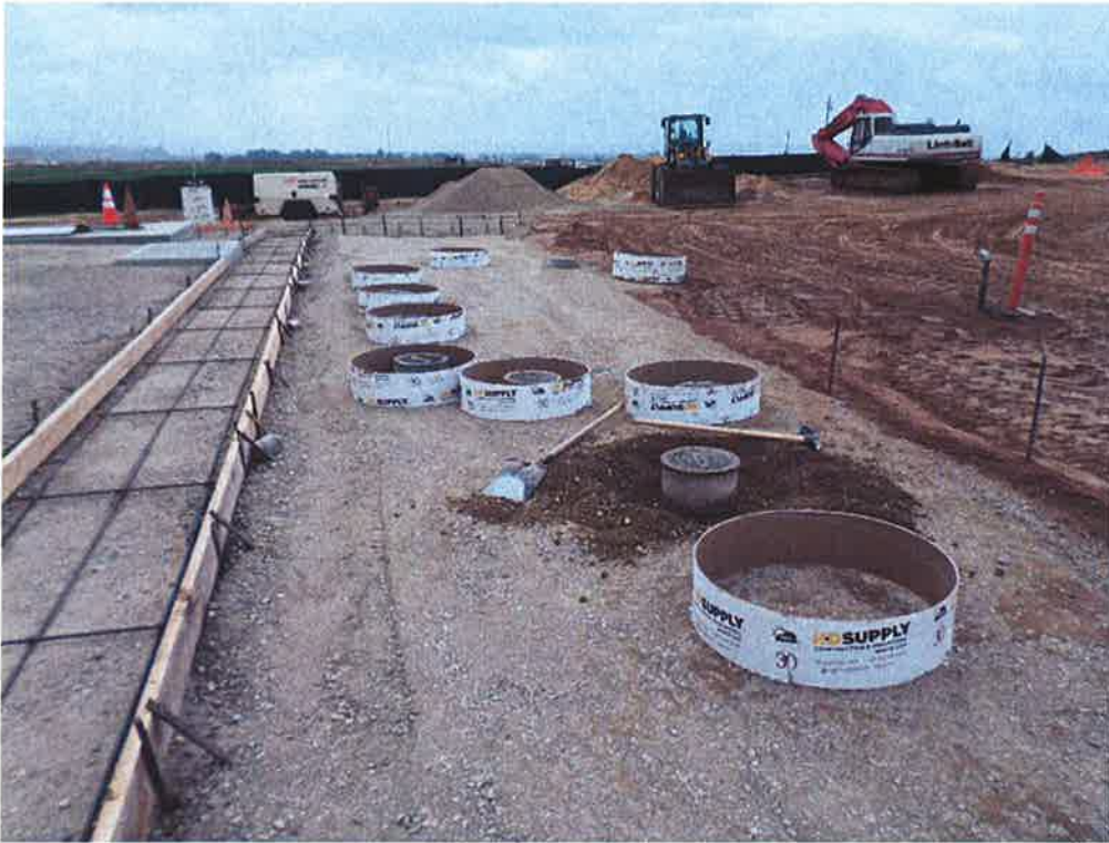
Forms for pouring valve can collars.
