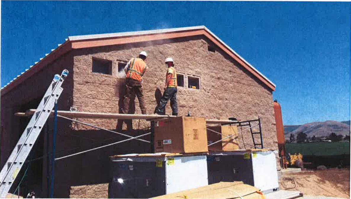
Spies removing rough face from block to allow flush HVAC installation.
