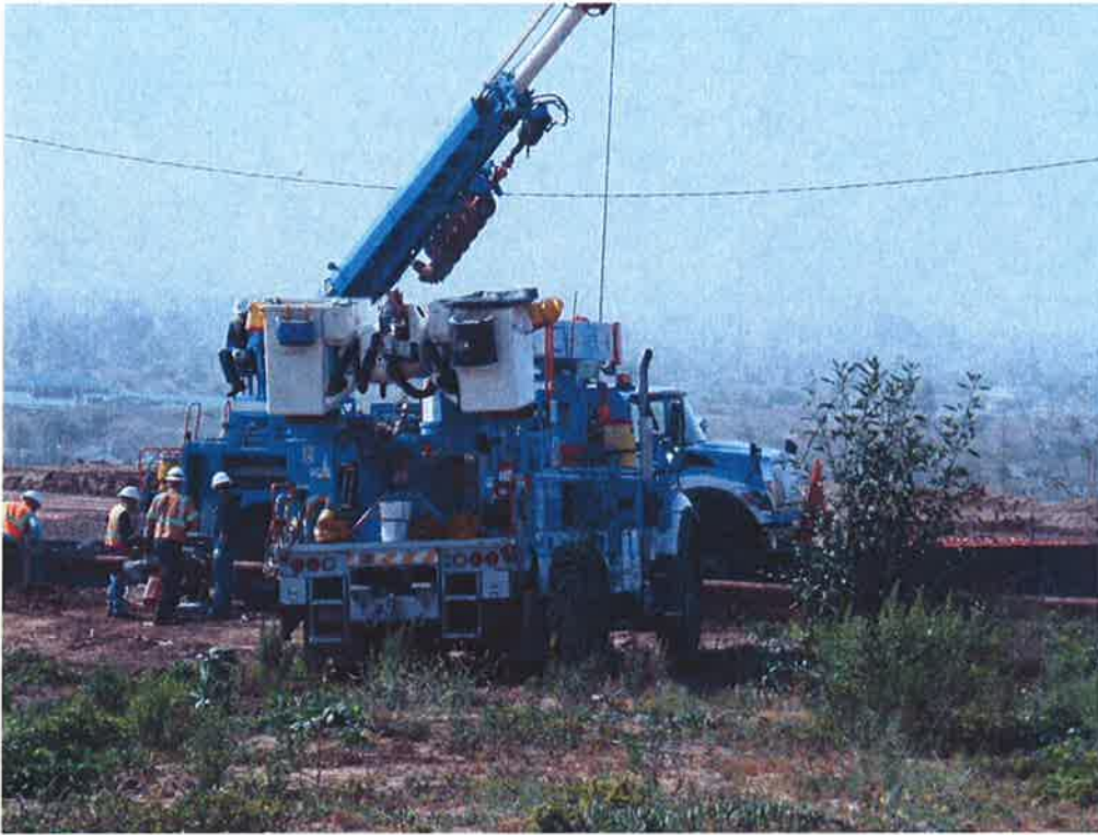
PG&E installing power pole for electrical service to the pump station.
