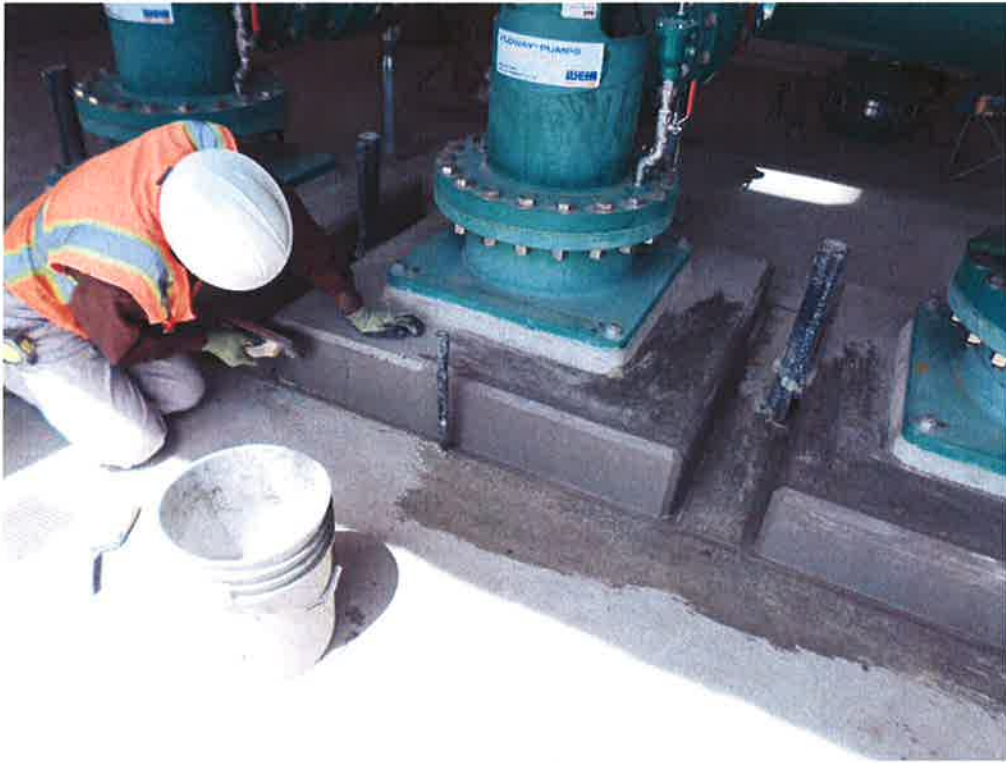
Spiess patching surface defects in concrete pump pads.
