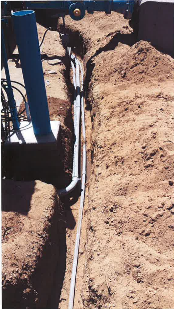
Underground conduit being installed by St. Denis Electric.
