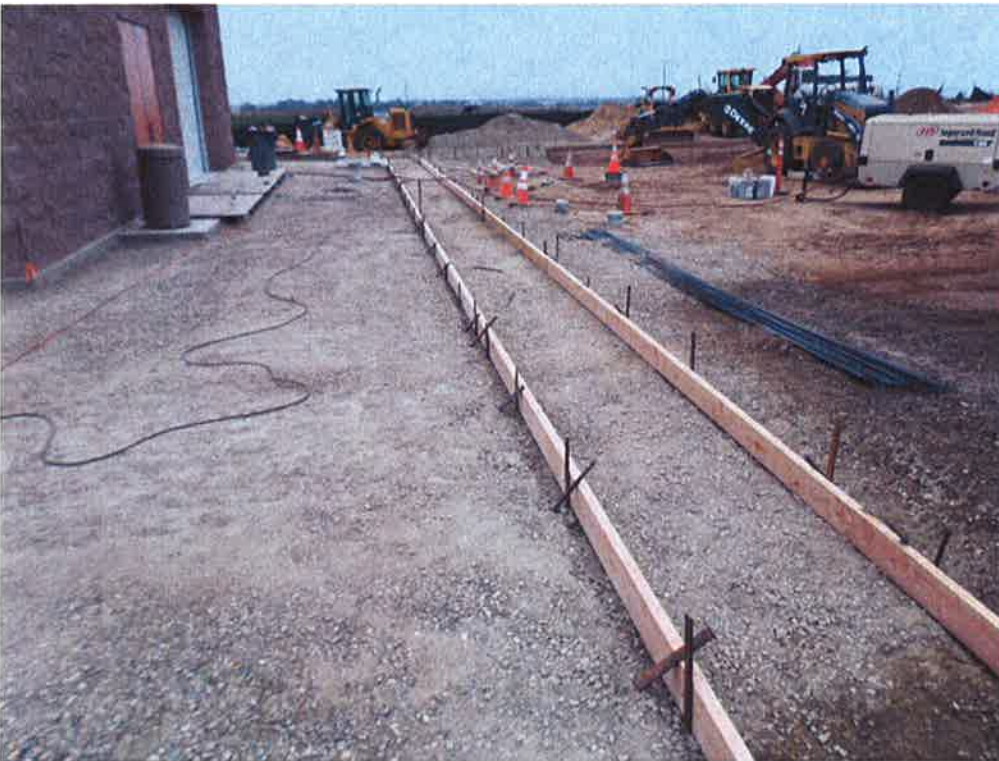
Three foot V-ditch formed.
