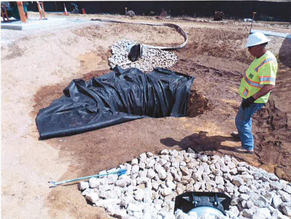
Spiess installing fabric lined rock drain in retention basin.
