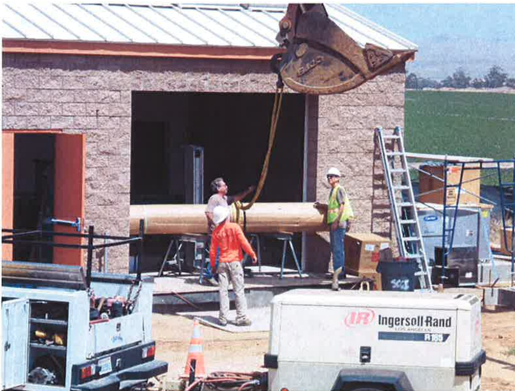
Installing the roll-up door for the pump room.
