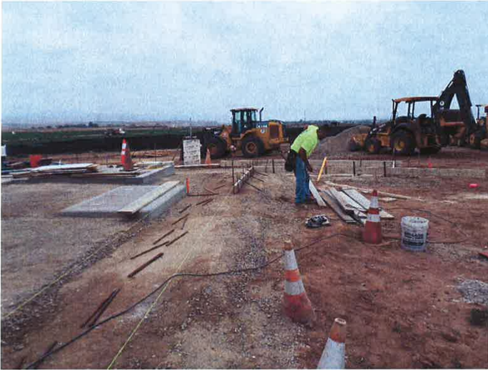
Spies forming three foot V-ditch.
