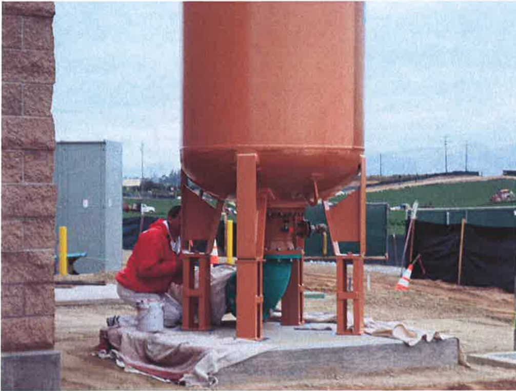
Coast Painting coating supports for surge tank.
