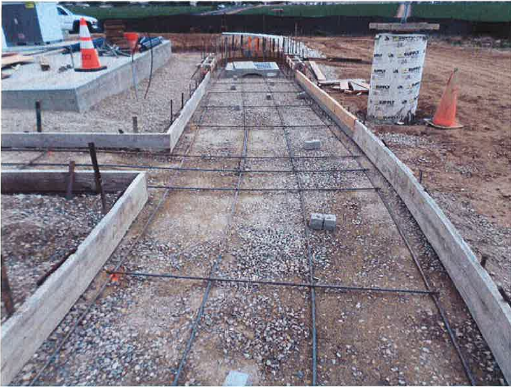
Reinforcing installed in six foot V-ditch.
