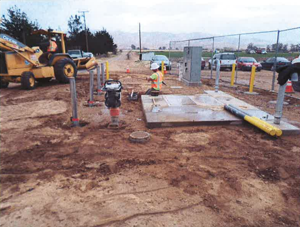
Spiess raising valve cans around PRV vault.
