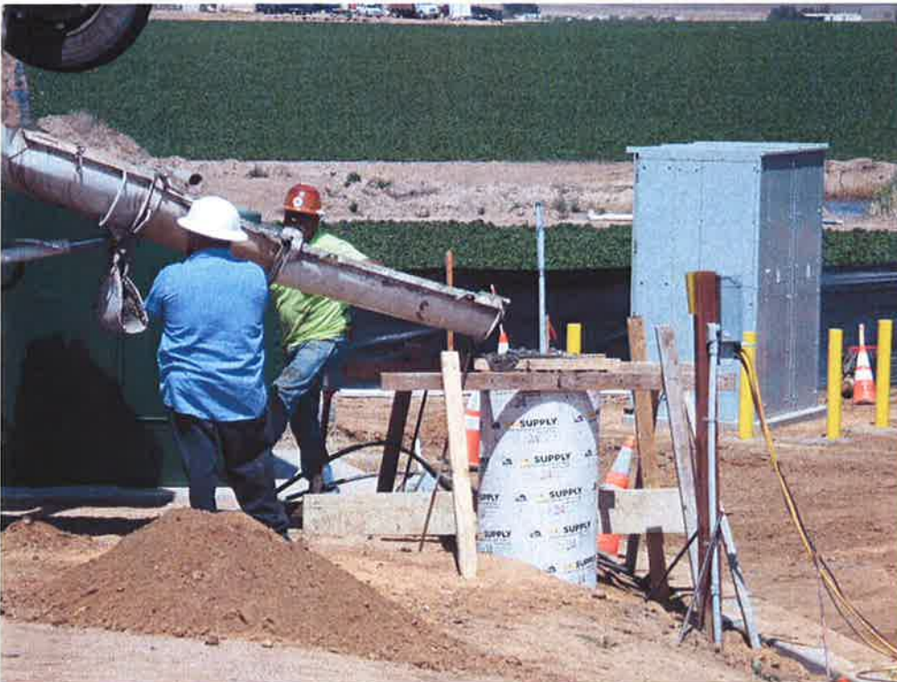
Pouring the light pole base.
