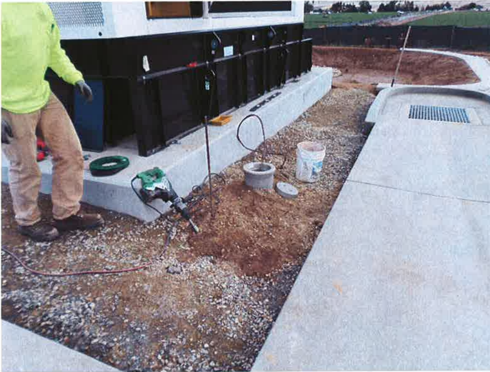
Installing grounding rod for emergency generator.
