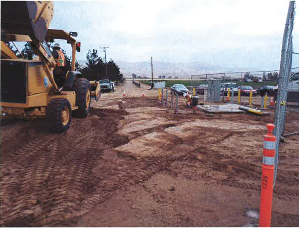
Spiess grading around PRV vault.
