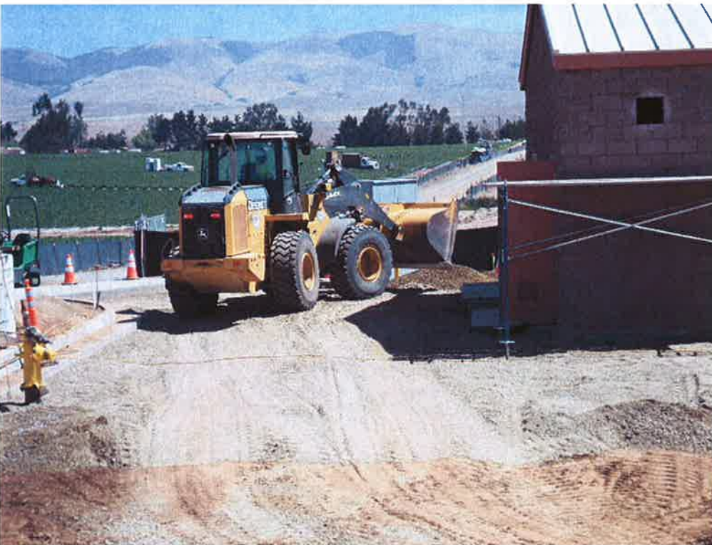
Spiess spreading aggregate base around the building.
