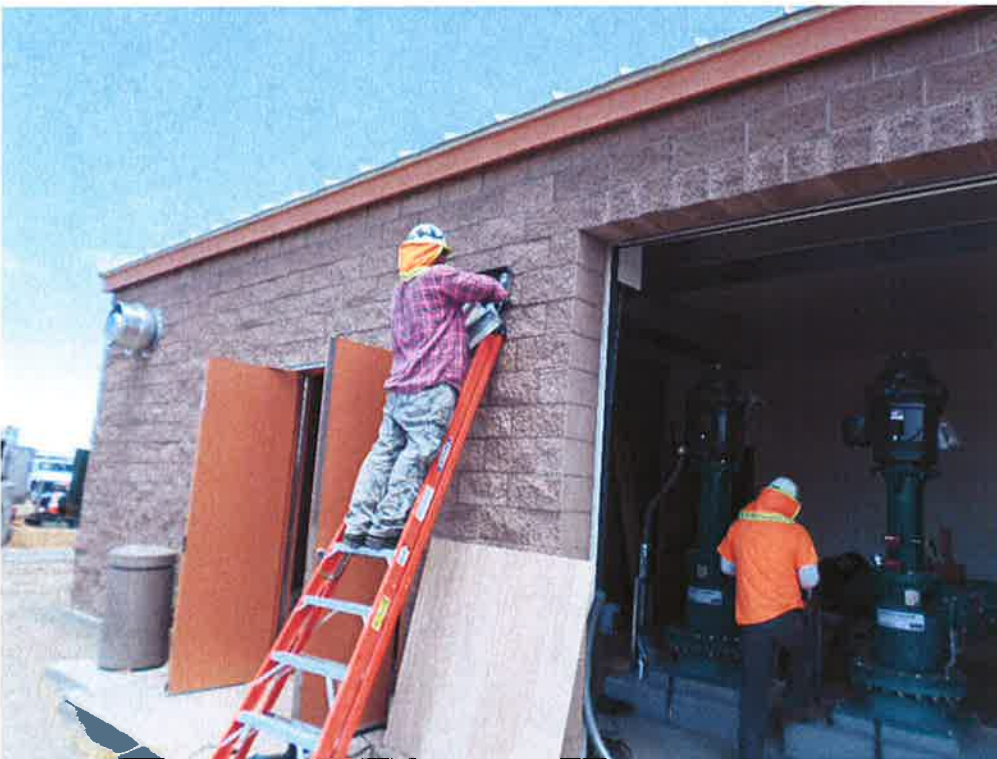
St. Denis Electric installing exterior lights around pump station building.
