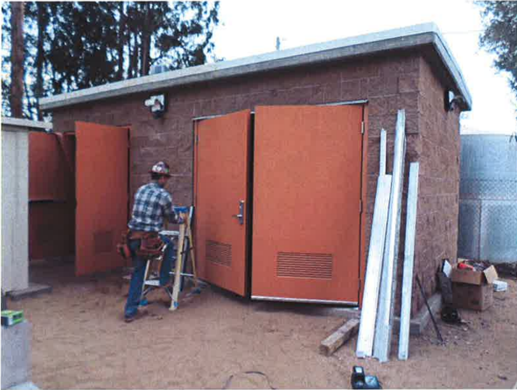
Installing door hardware.
