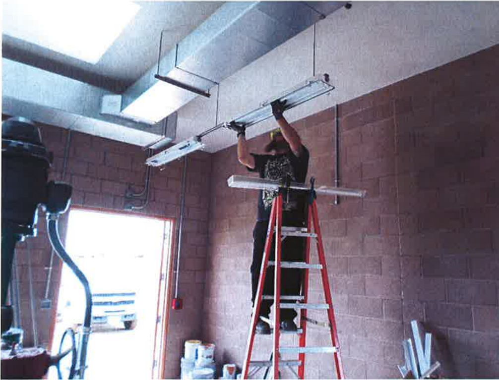
St. Denis Electric installing lighting in pump station.
