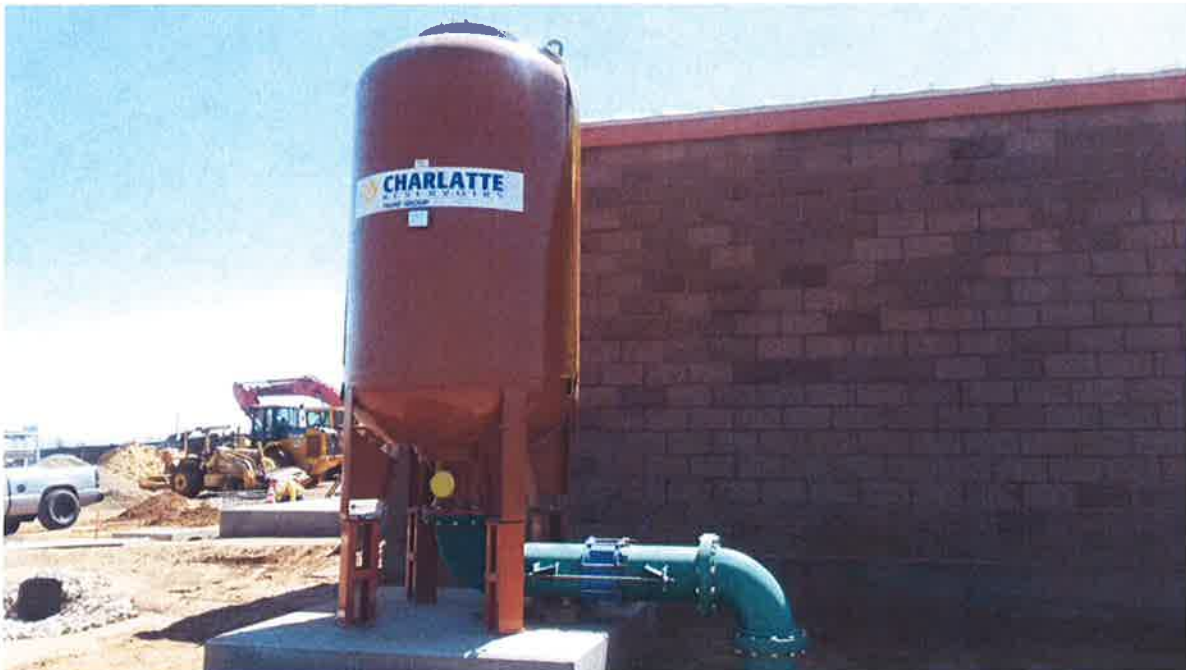
Surge tank anchored.
