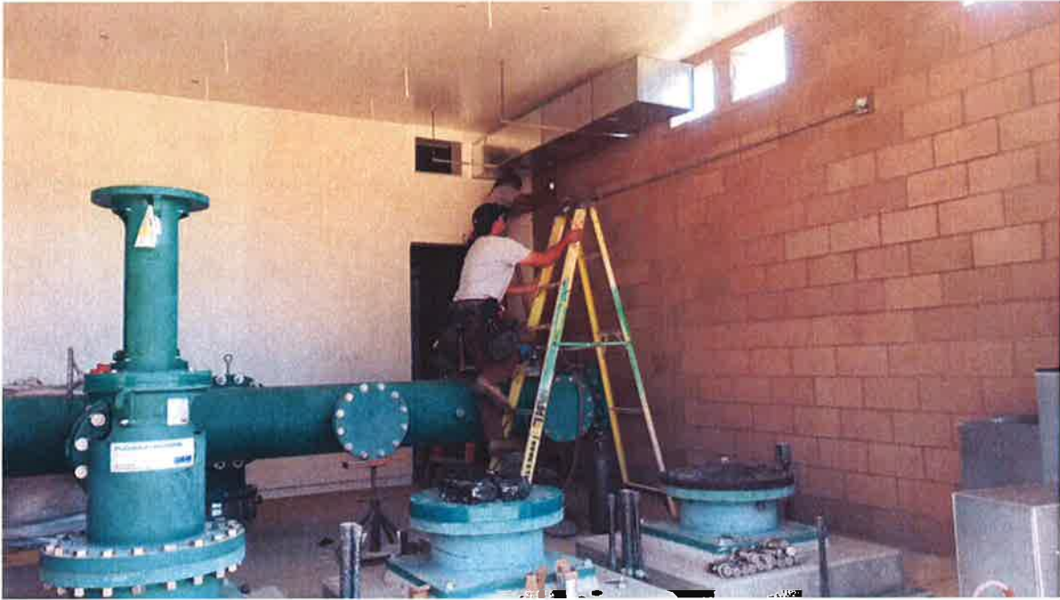
DAHL Air Conditioning installing the HVAC ducts in the pump room.
