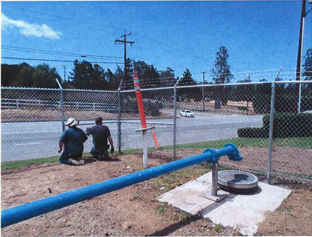
Central Coast Fence installing new fence.
