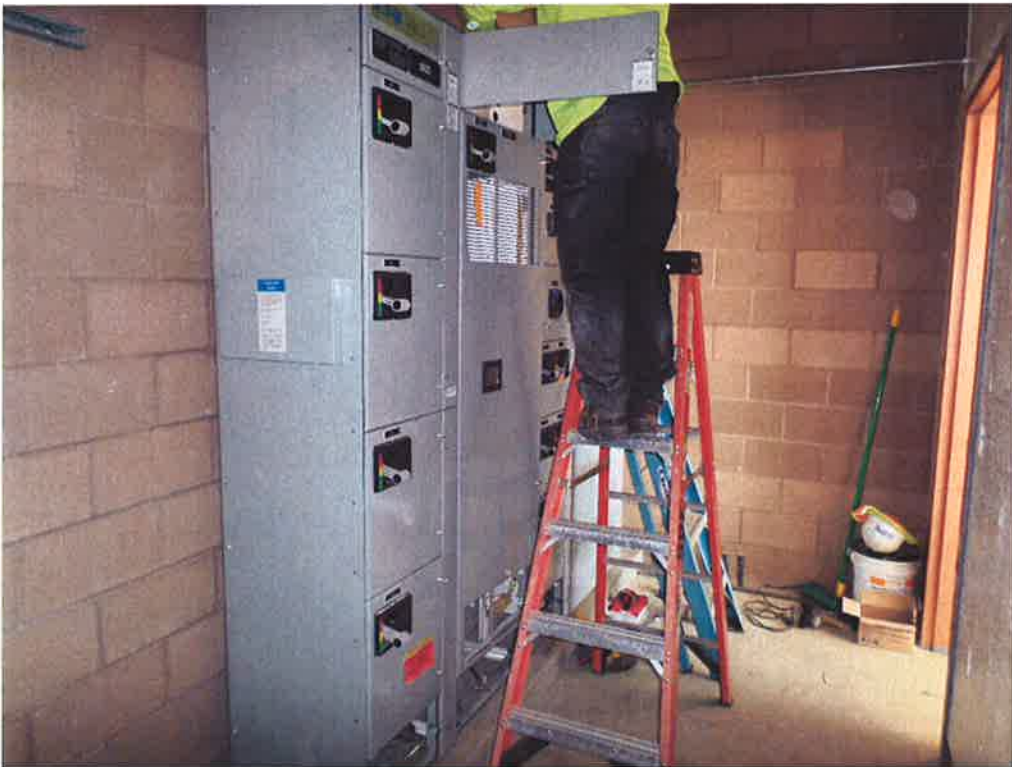
St. Denis Electric setting MCC in electrical room.
