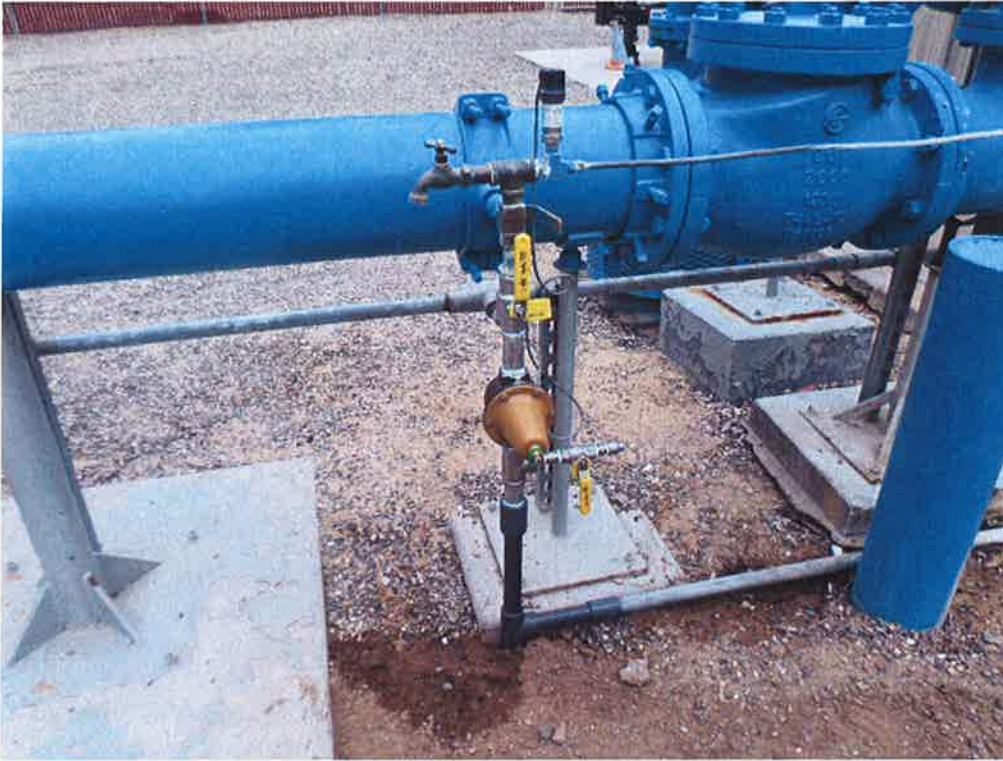
Spiess installing pressure reducer.
