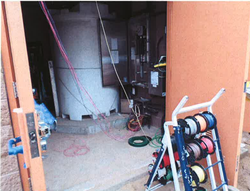
St. Denis Electric pulling wire.
