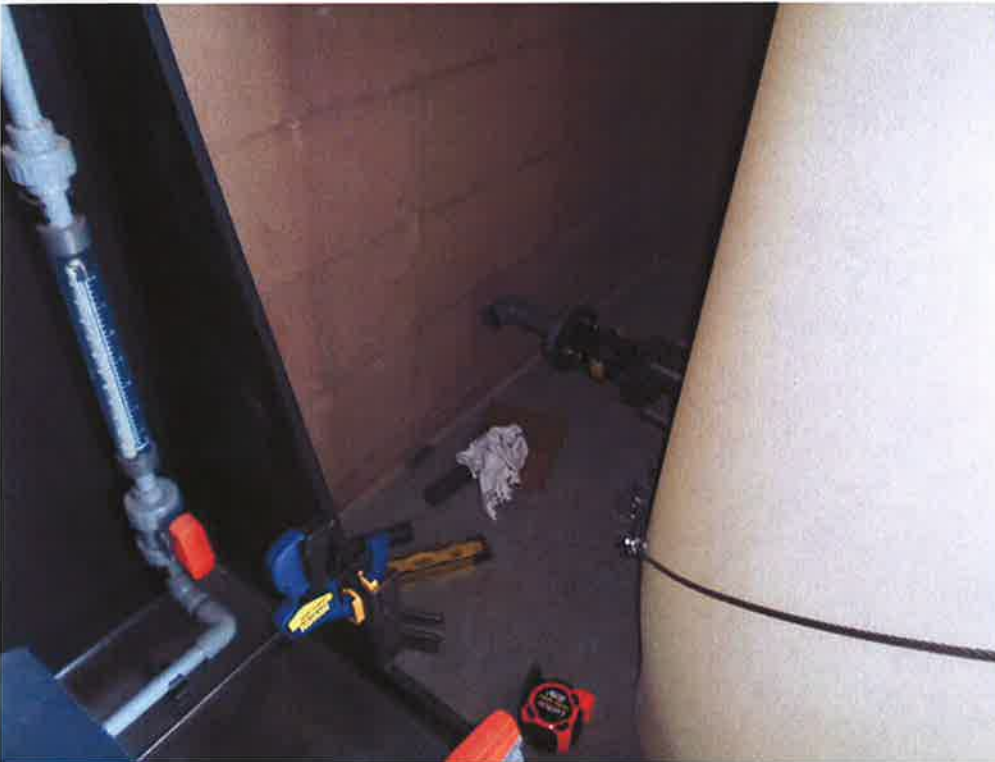
Spiess installing chemical piping at Eureka.
