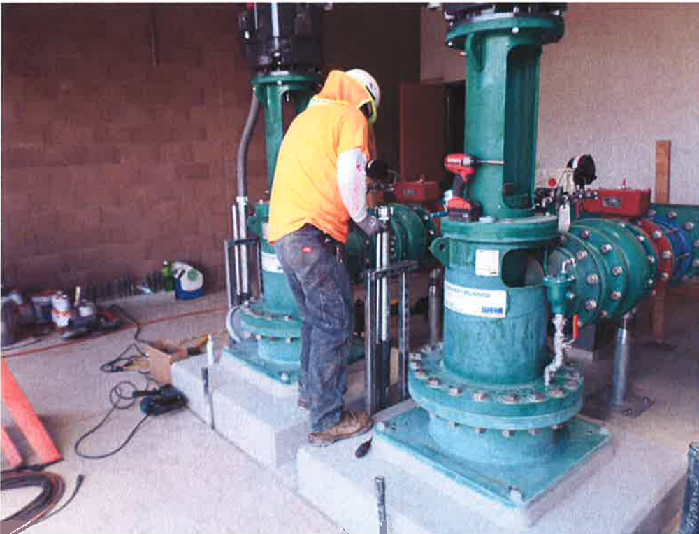
Spiess installing rack and conduit at pumps.
