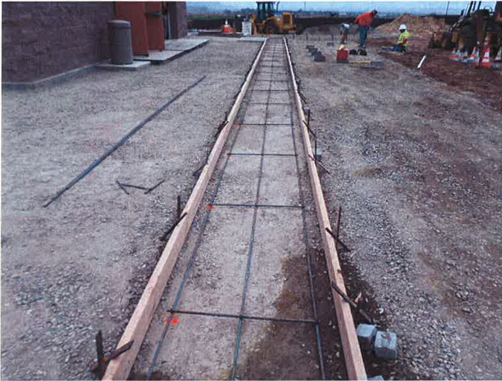
Reinforcing installed at three foot V-ditch.
