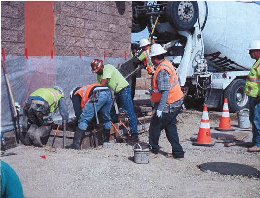
Spieß pouring side walk to electrical room.
