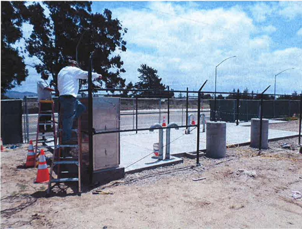
Central Coast Fence installing perimeter fencing.
