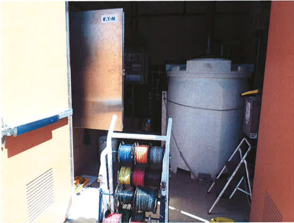
St. Denis Electric pulling wires.
