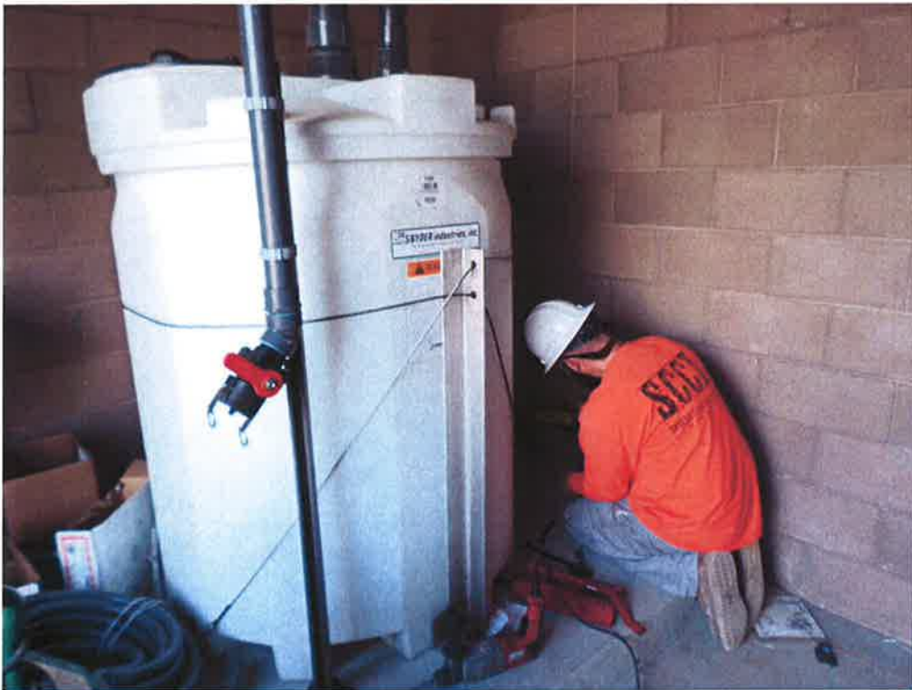
Spiess installing chemical tank piping.
