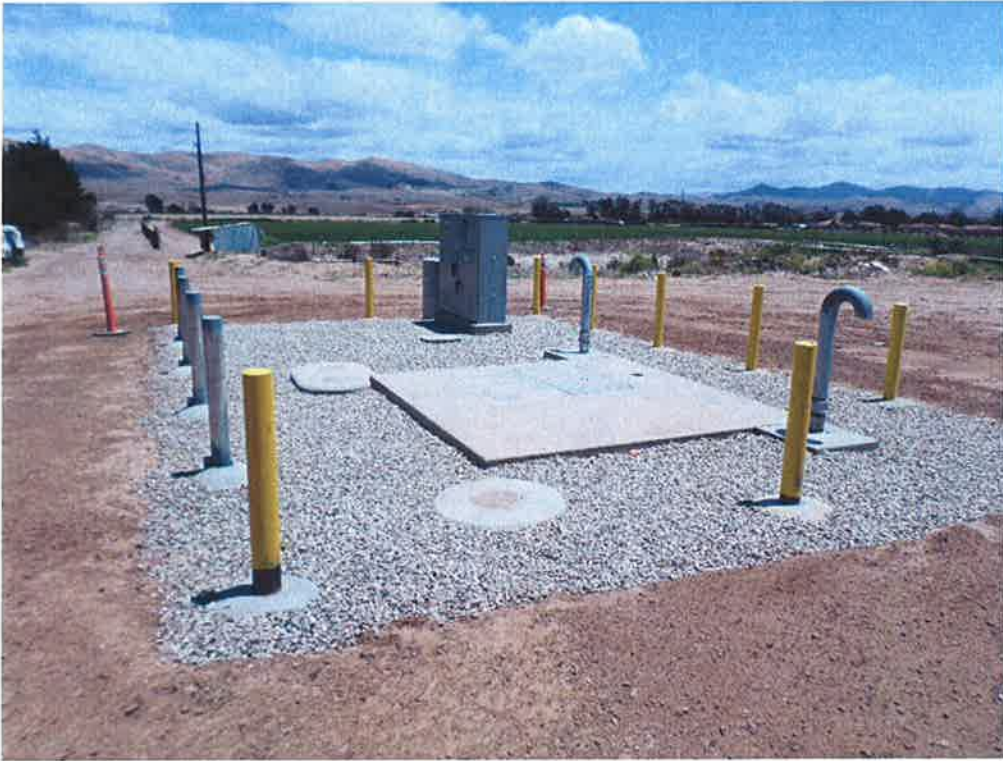
Rock placed around PRV vault site.
