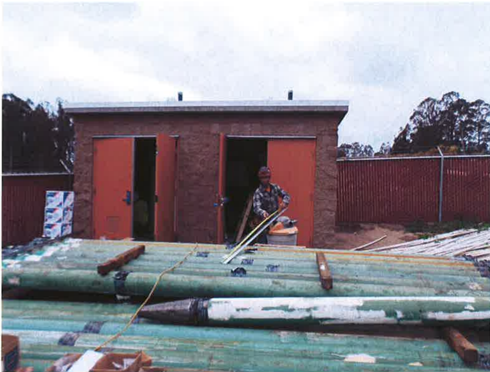
Martin Doors installing hardware on doors.
