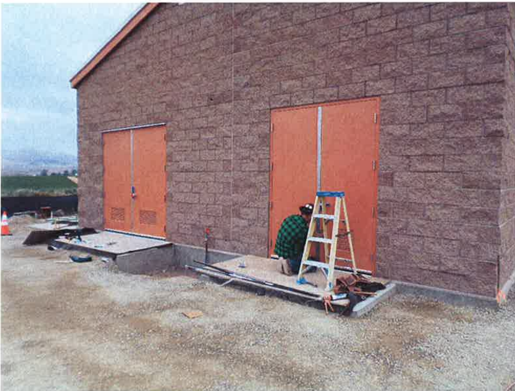
Martin Doors installing hardware on doors.
