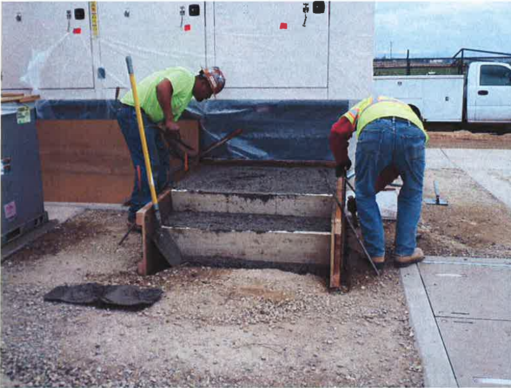
Spieß pouring emergency generator access steps.
