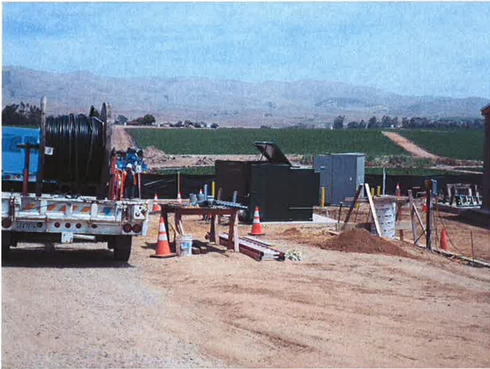
PG&E on site to set the new transformer.
