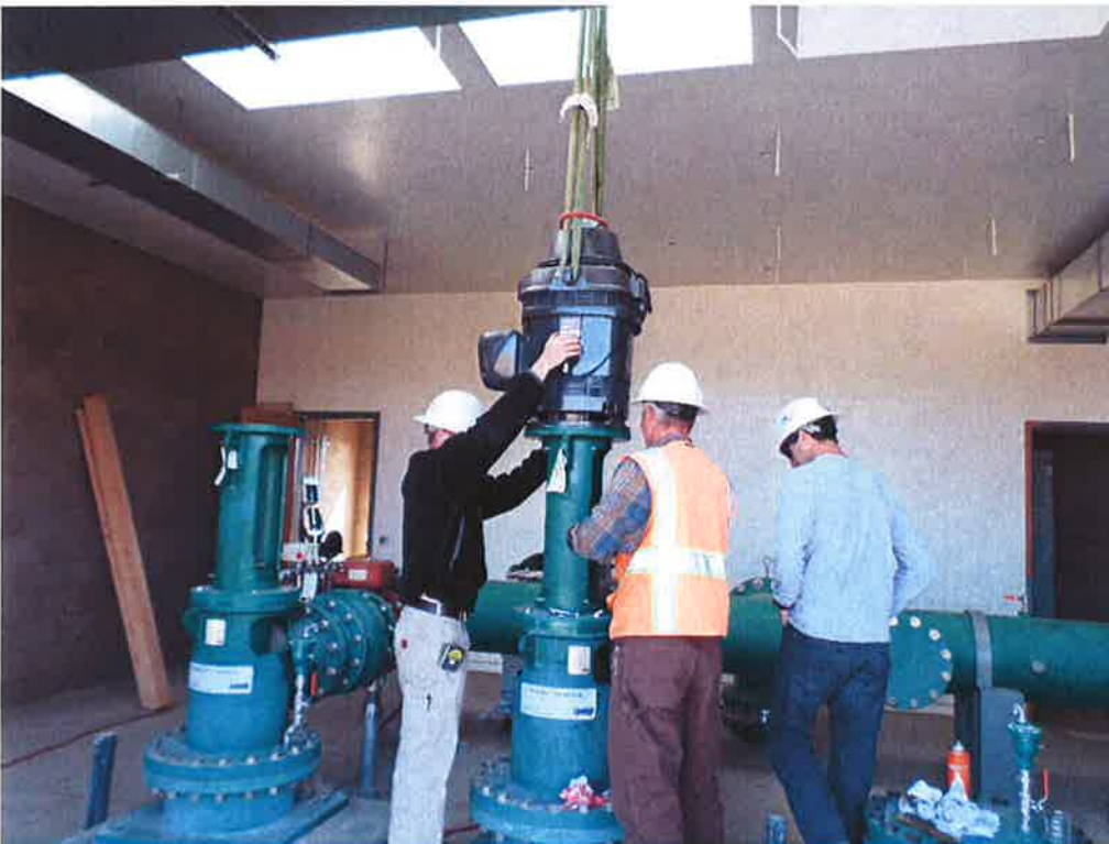
Spiess installing pump motors.
