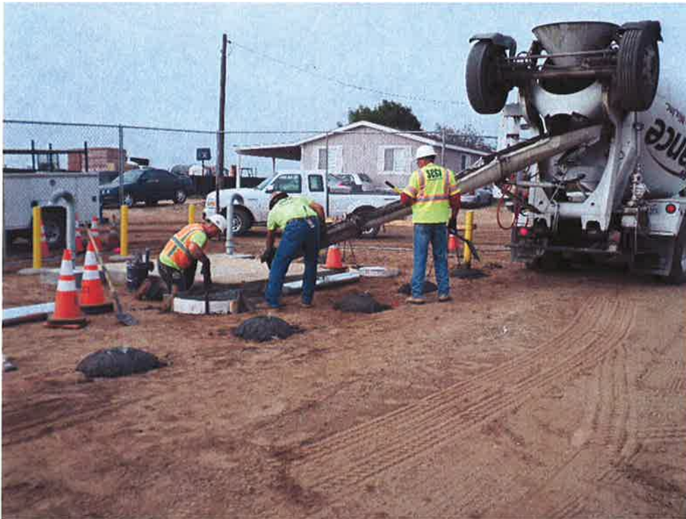
Spies pouring bollards and valve can collars.
