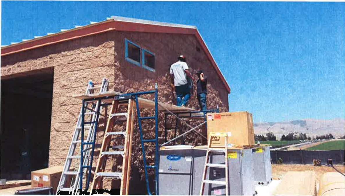
DAHL Air Conditioning installing exterior HVAC ducts to units.
