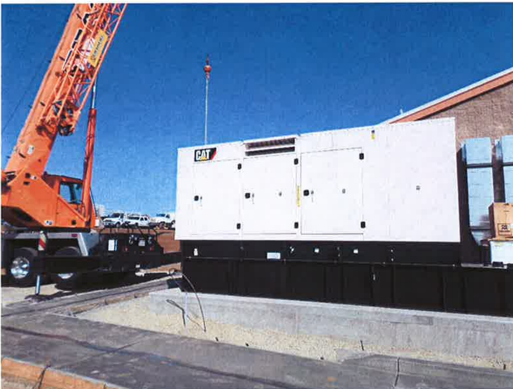
Spiess setting emergency generator onto pad.
