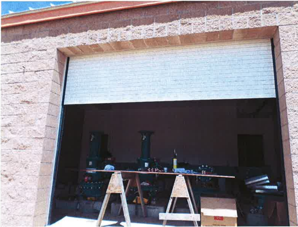
Roll-up door installed for the pump room.
