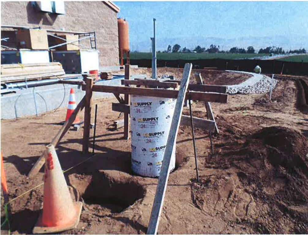
Light pole base formed and reinforcing and conduit installed.
