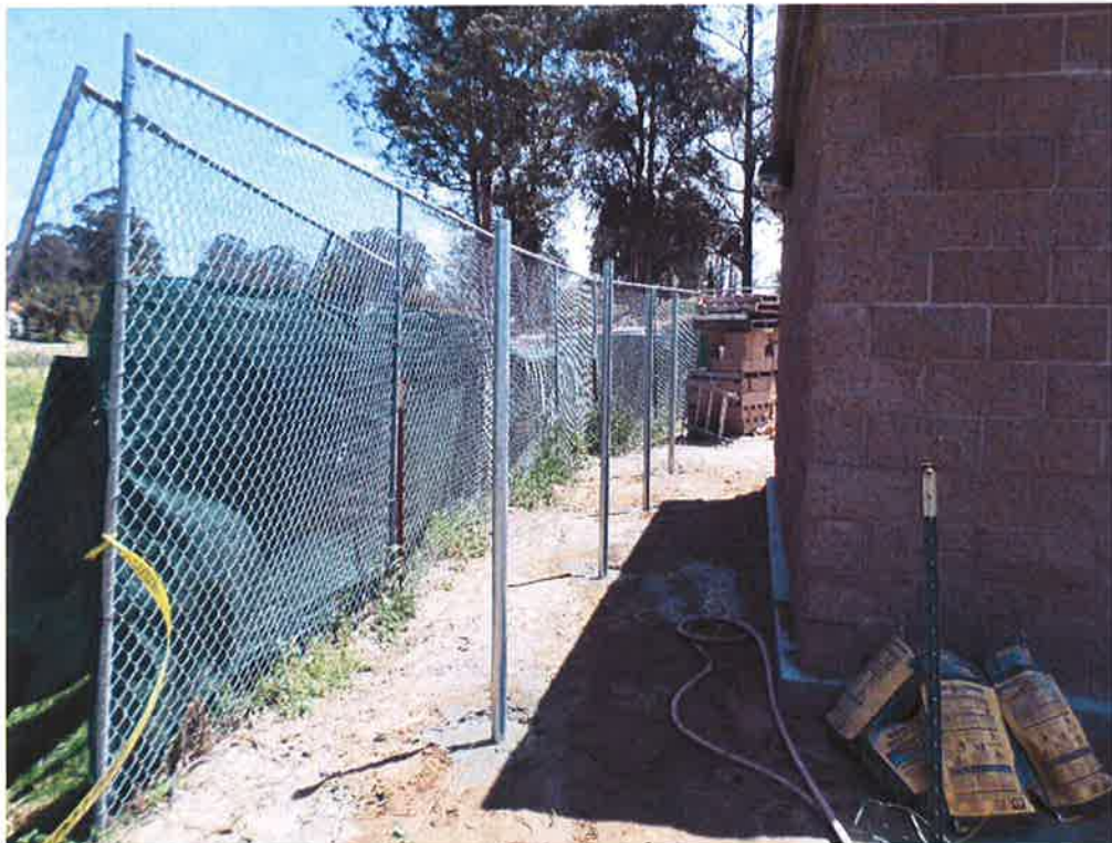
Central Coast Fence installing fence posts.
