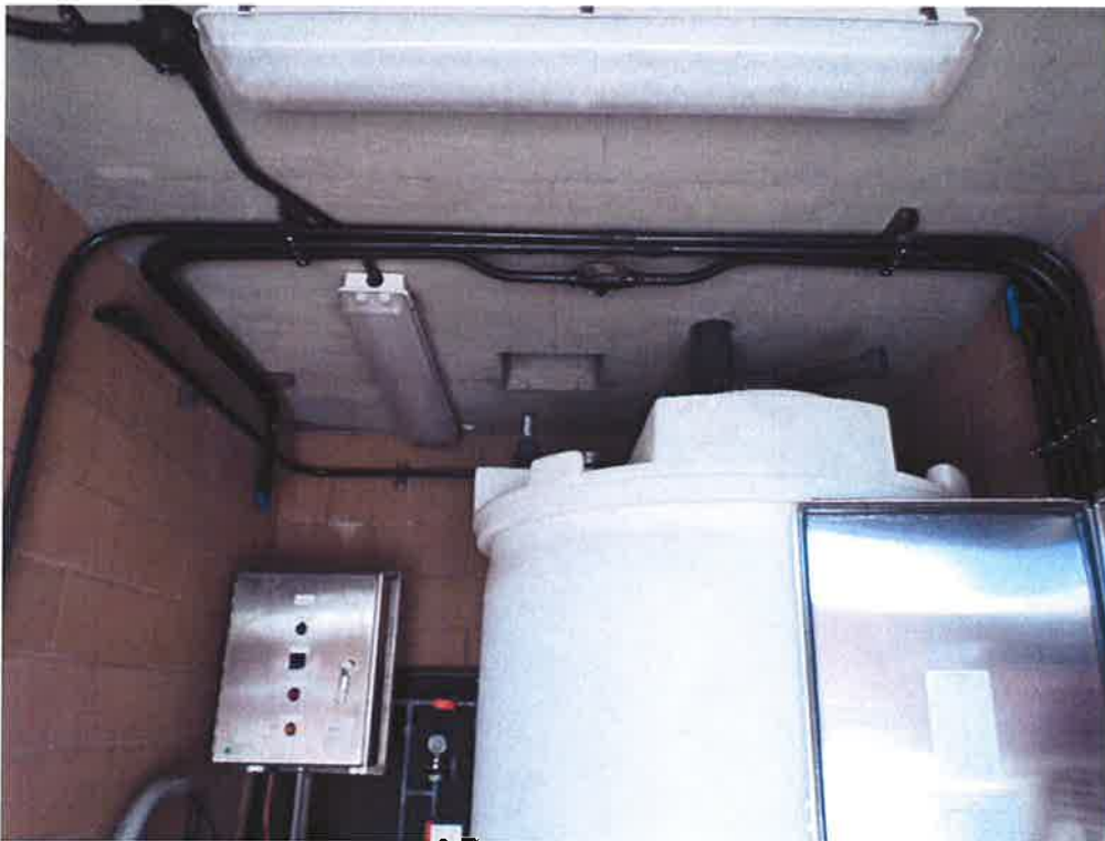
Conduit being installed by St. Denis Electric.
