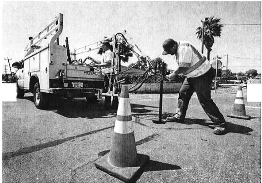
Casey Stewart, left, and Jason Carlile with the Oceano Community Services District perform a valve-turning maintenance procedure on one of the water lines in Oceano. JOE JOHNSTON — jjohnston@thetribunenews.com | Buy Photo
