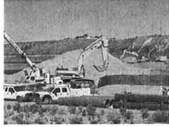
Project progress at the Santa Maria River - October 2014
