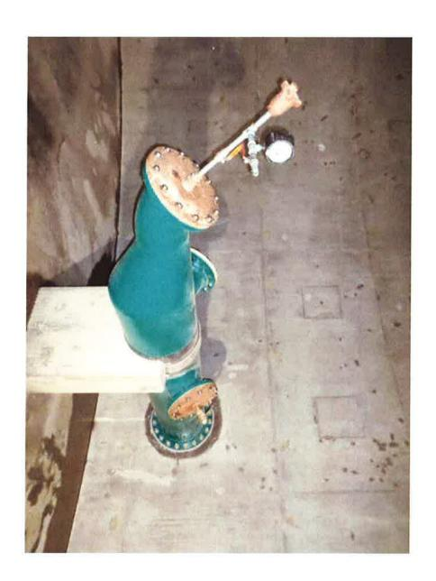
Pressure test of inlet pipe from inside tank
