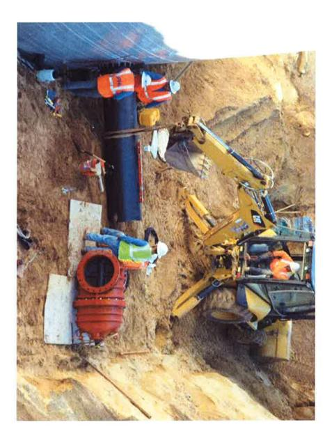
Installing inlet piping and 24-inch valve
