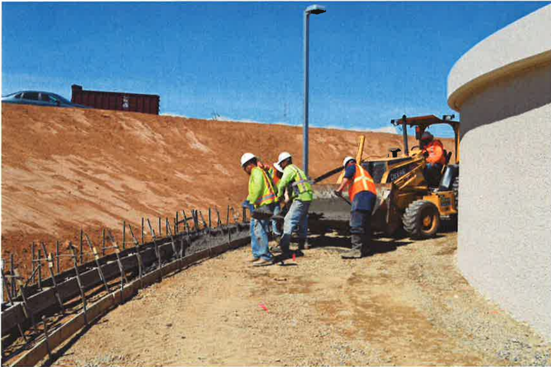
PHC and Lopez Engineering pouring concrete curb and gutter.
