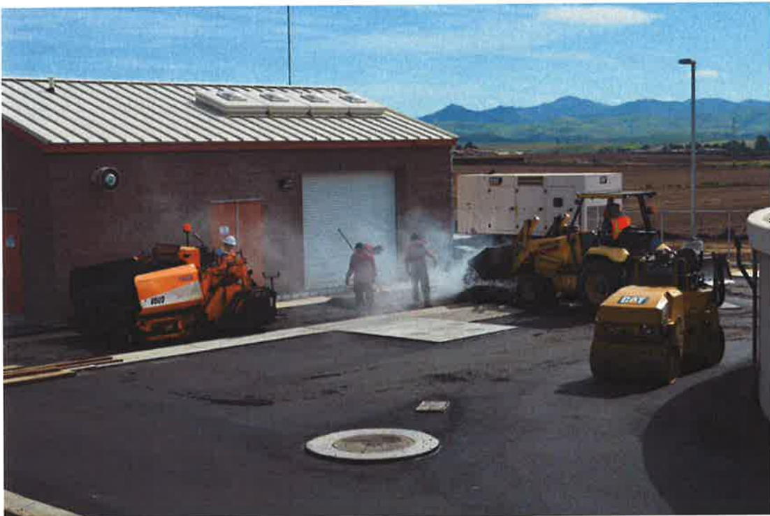
Pav-Kote applying second layer of asphalt.
