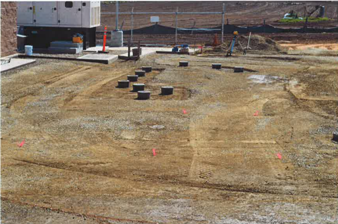
PHC preparing site for concrete work and paving.
