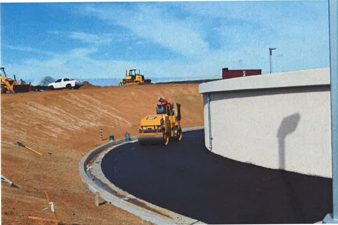
Pav-Kote rolling first layer of asphalt.
