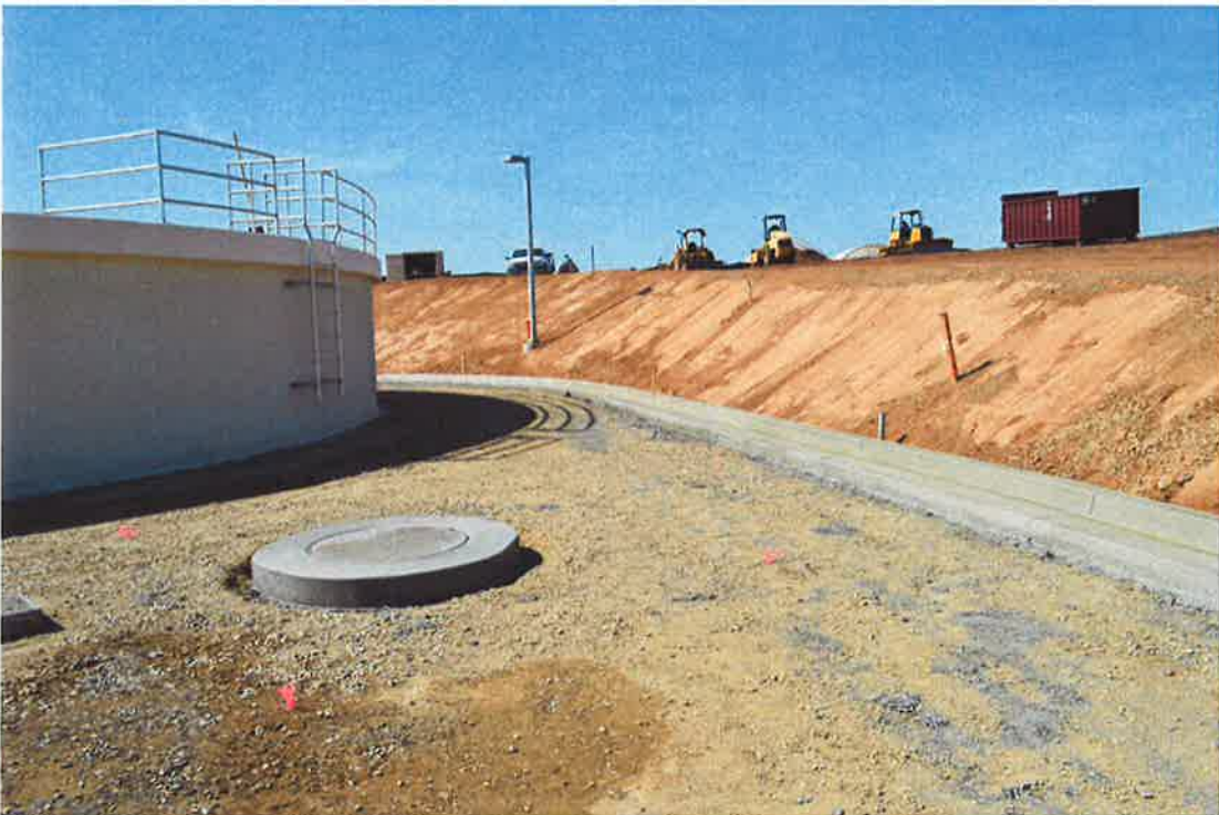
Concrete work curing.
