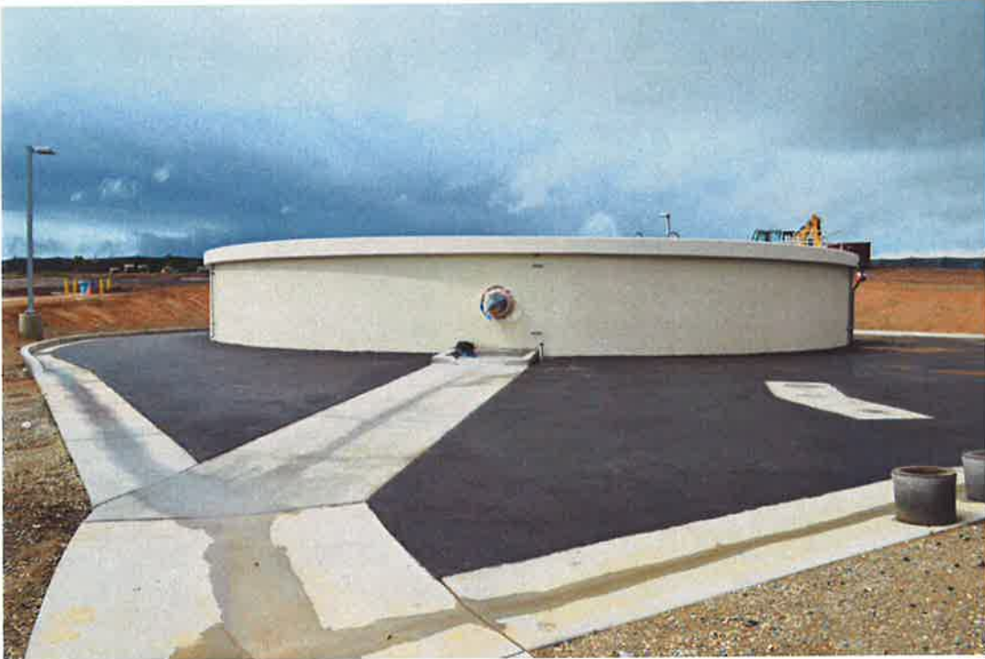
Concrete v-ditches and gutter flowing after rain.
