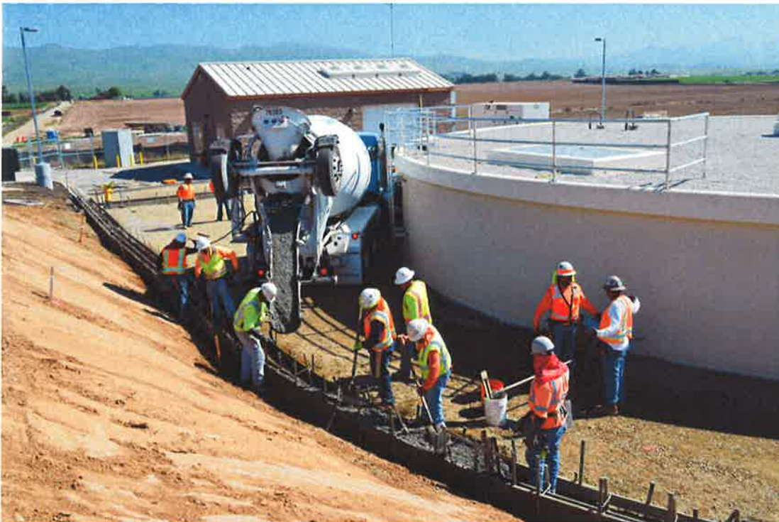
Lopez Engineering starting to pour concrete curb and gutter.
