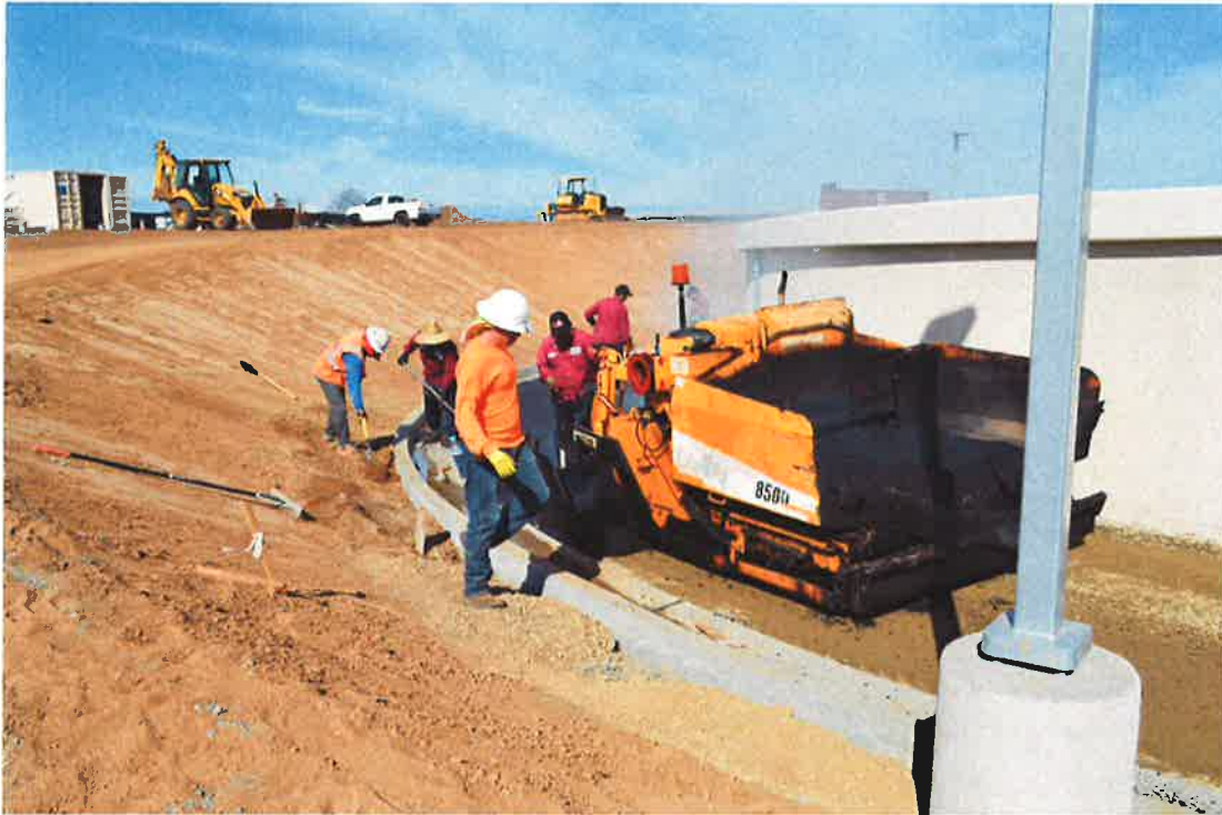
Placing first lift of asphalt around reservoir.
