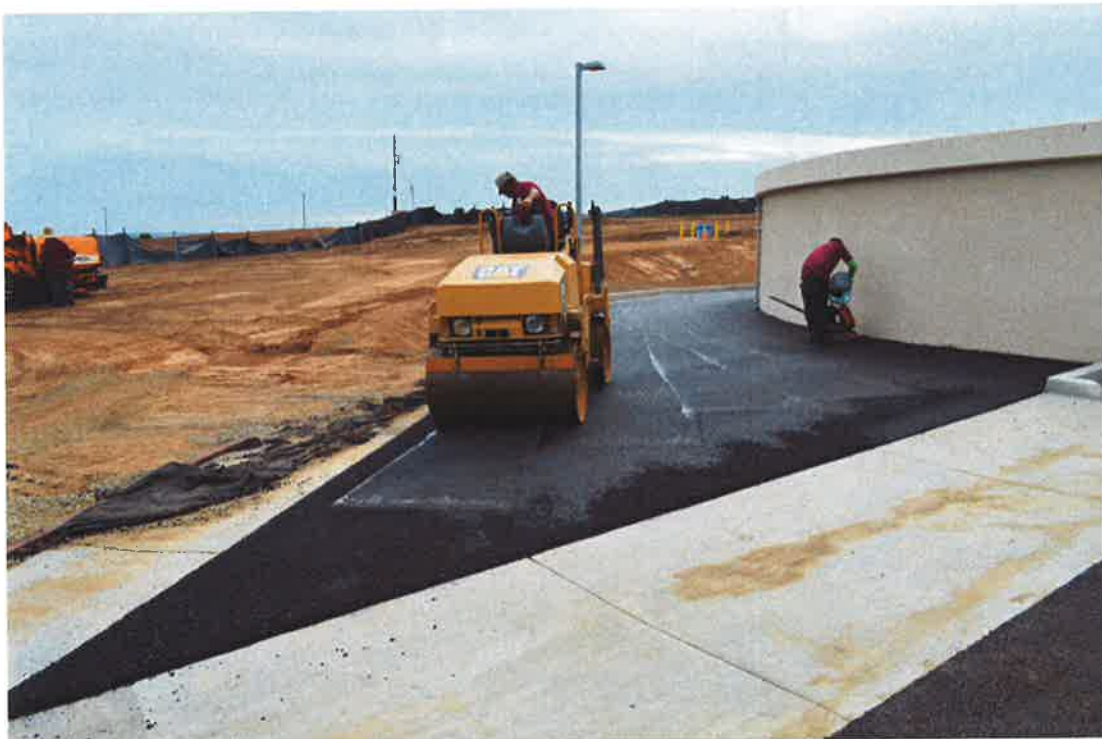
Final rolling of asphalt.
