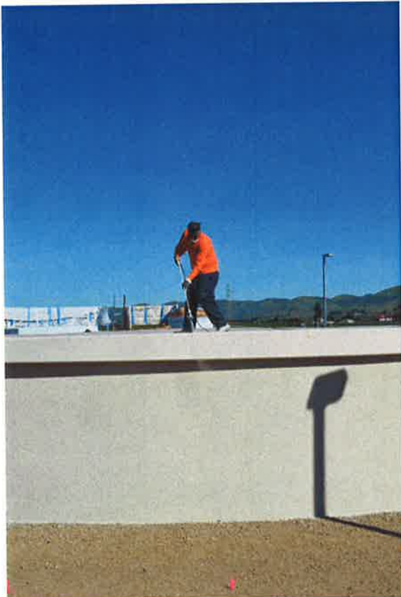
National Coating applying second layer of coating to reservoir.
