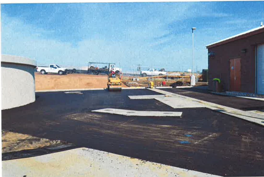
Pav-Kote placing first lift of asphalt.
