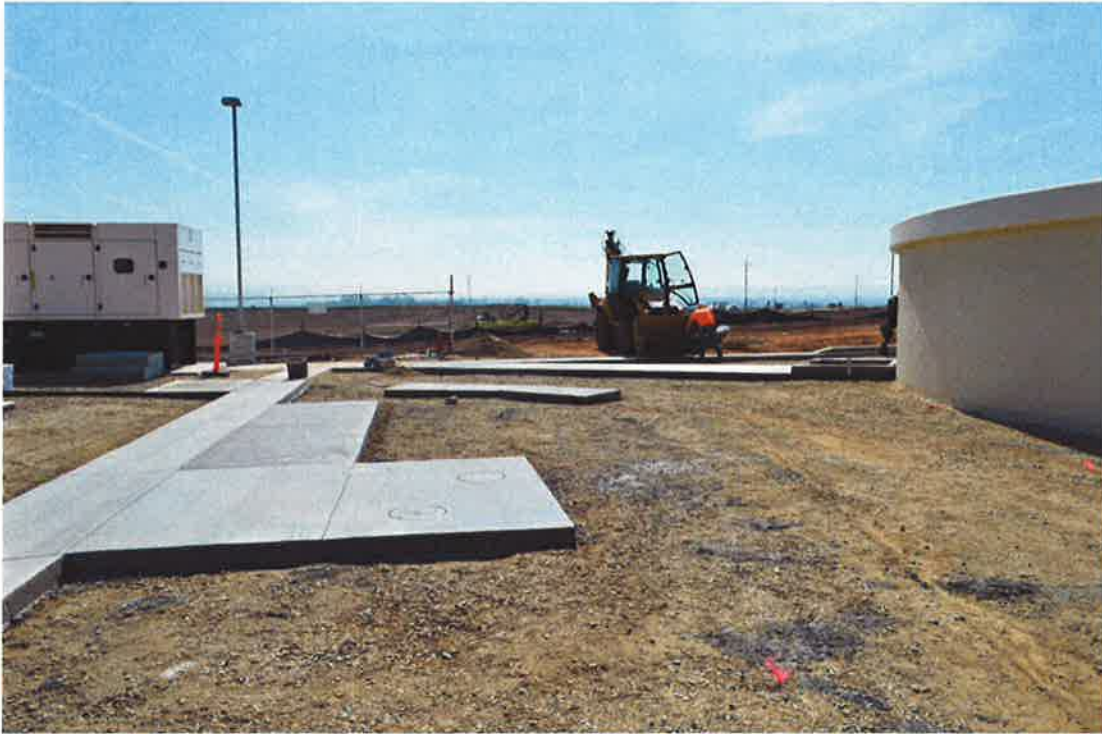
Concrete work curing, PHC cleaning up site.
