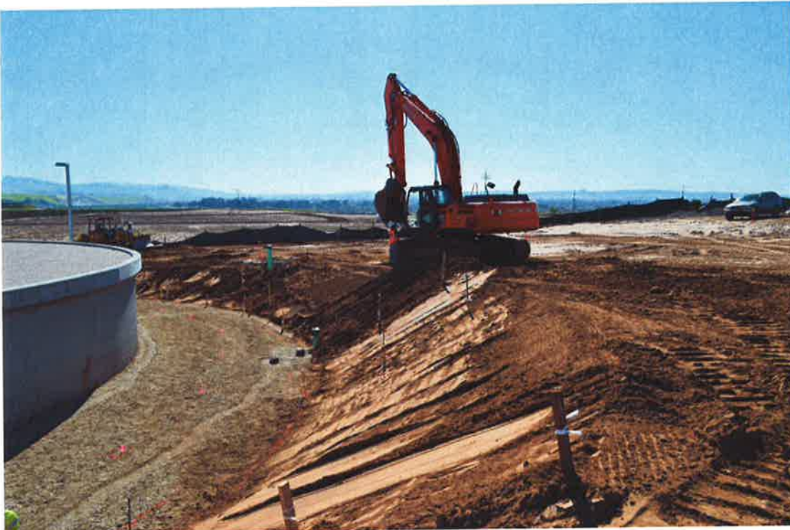
PHC cutting slope around reservoir to a 3:1.
