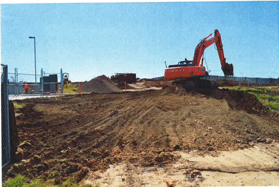
PHC construction Class II AB fire truck turn around.
