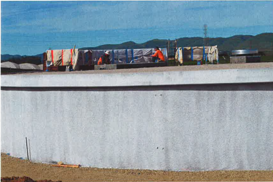
National Coating prepping surface of reservoir and applying primer.
