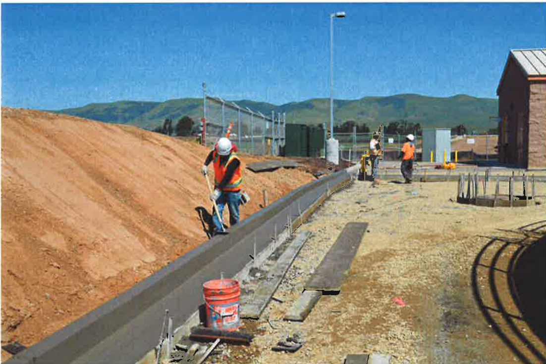
Lopez Engineering finishing concrete curb and gutter.
