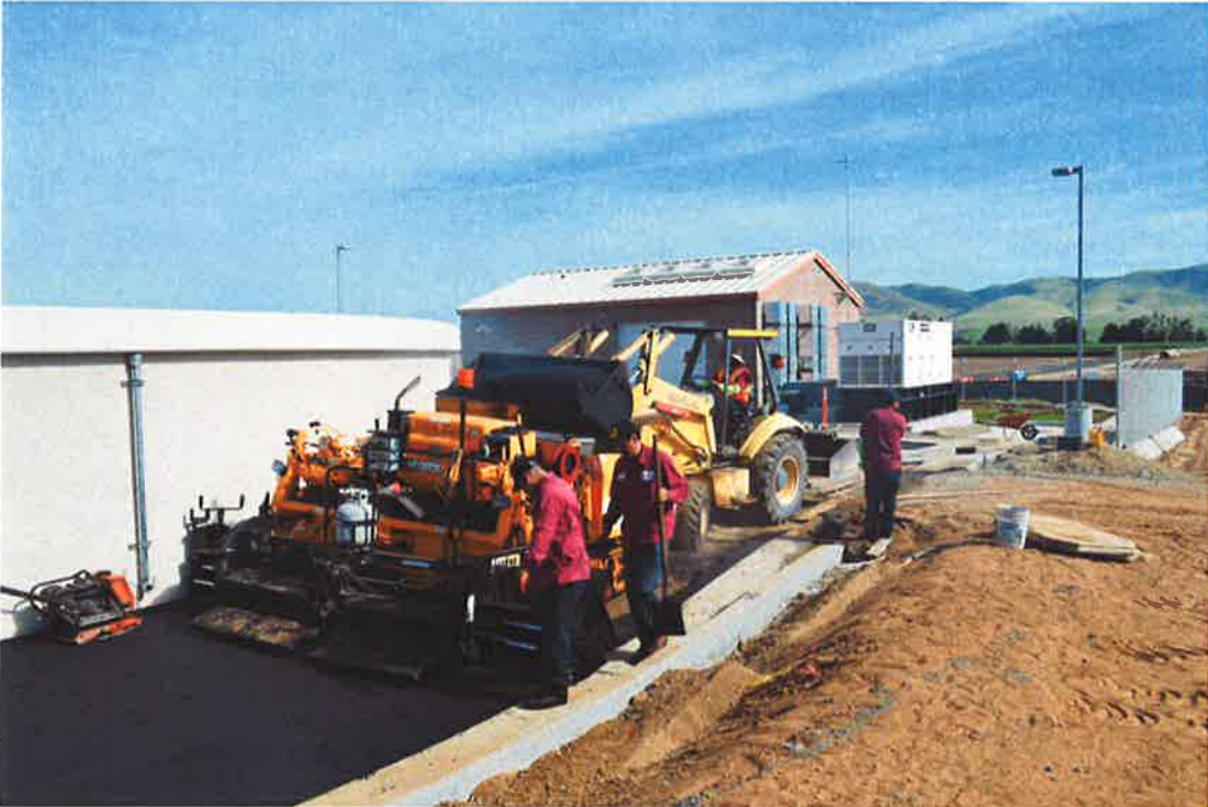
Pav-Kote placing first lift of asphalt around reservoir.
