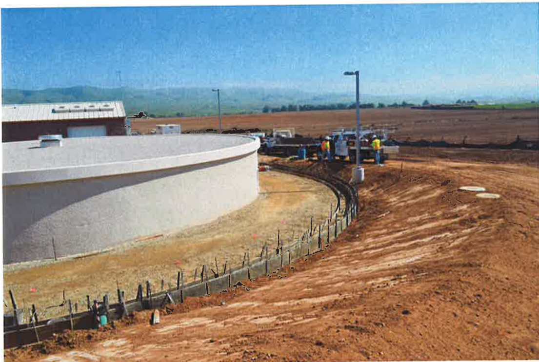
Concrete curb and gutter formed.
