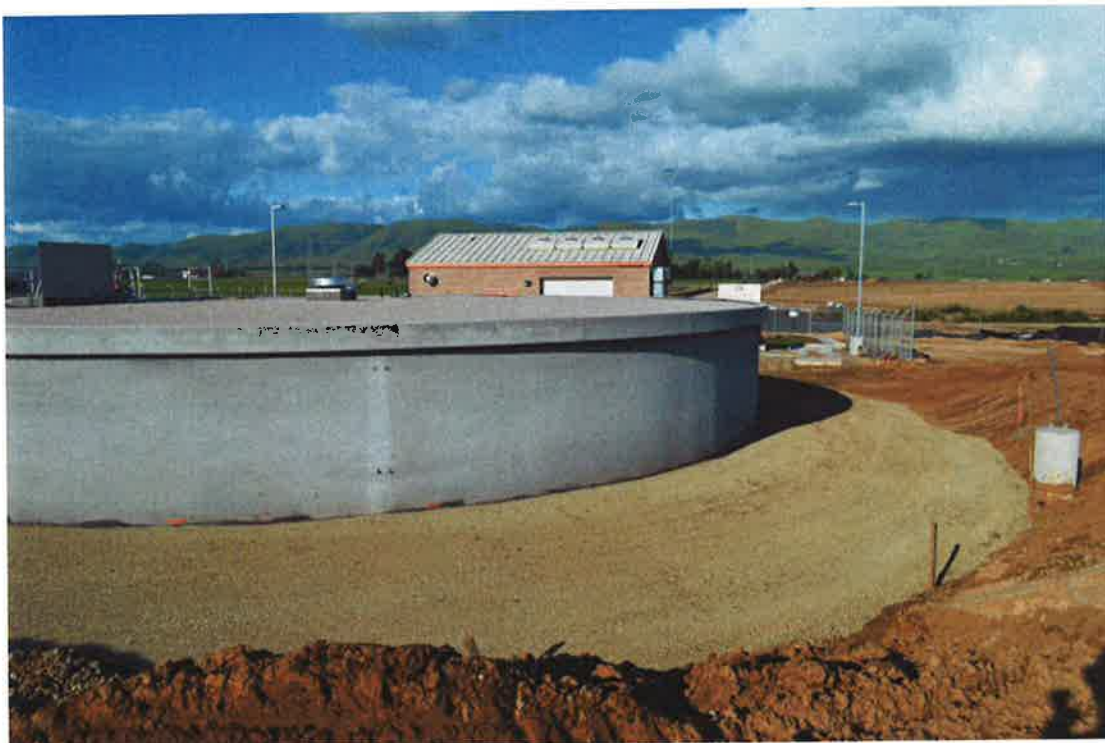
Class II AB to grade around reservoir.
