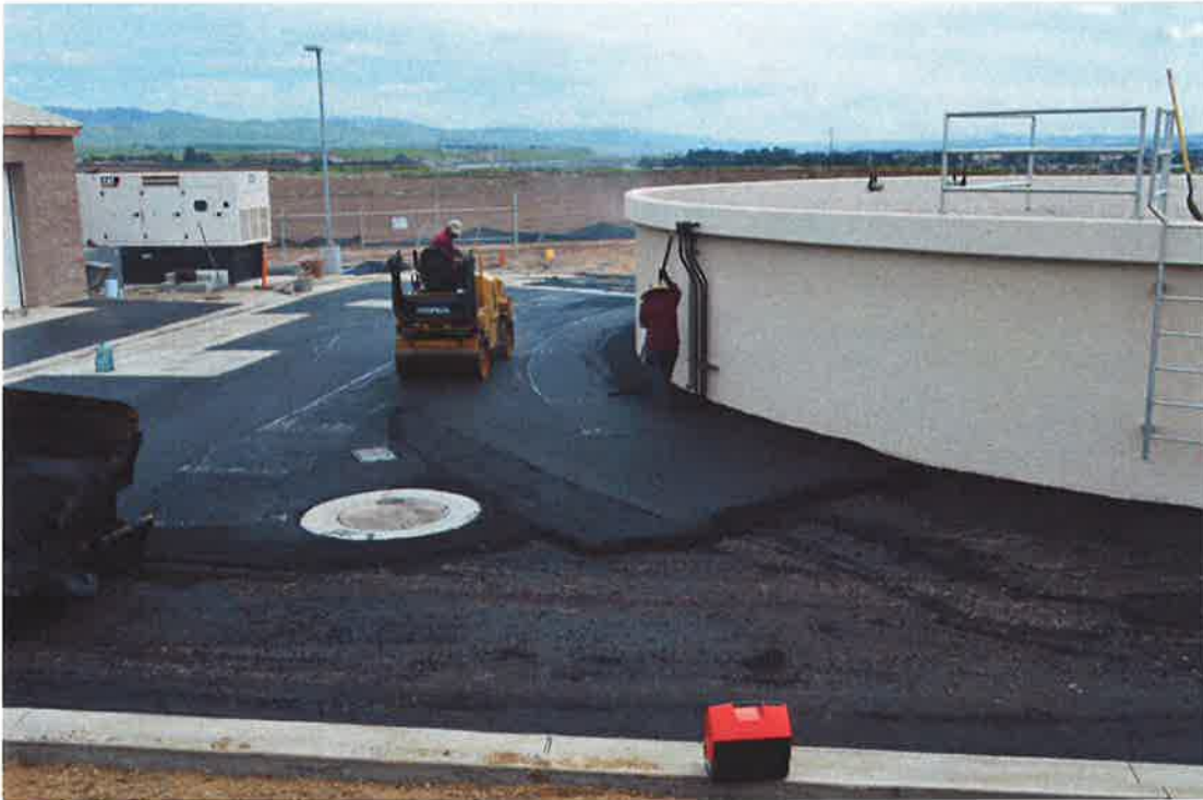
Placing second layer of asphalt.
