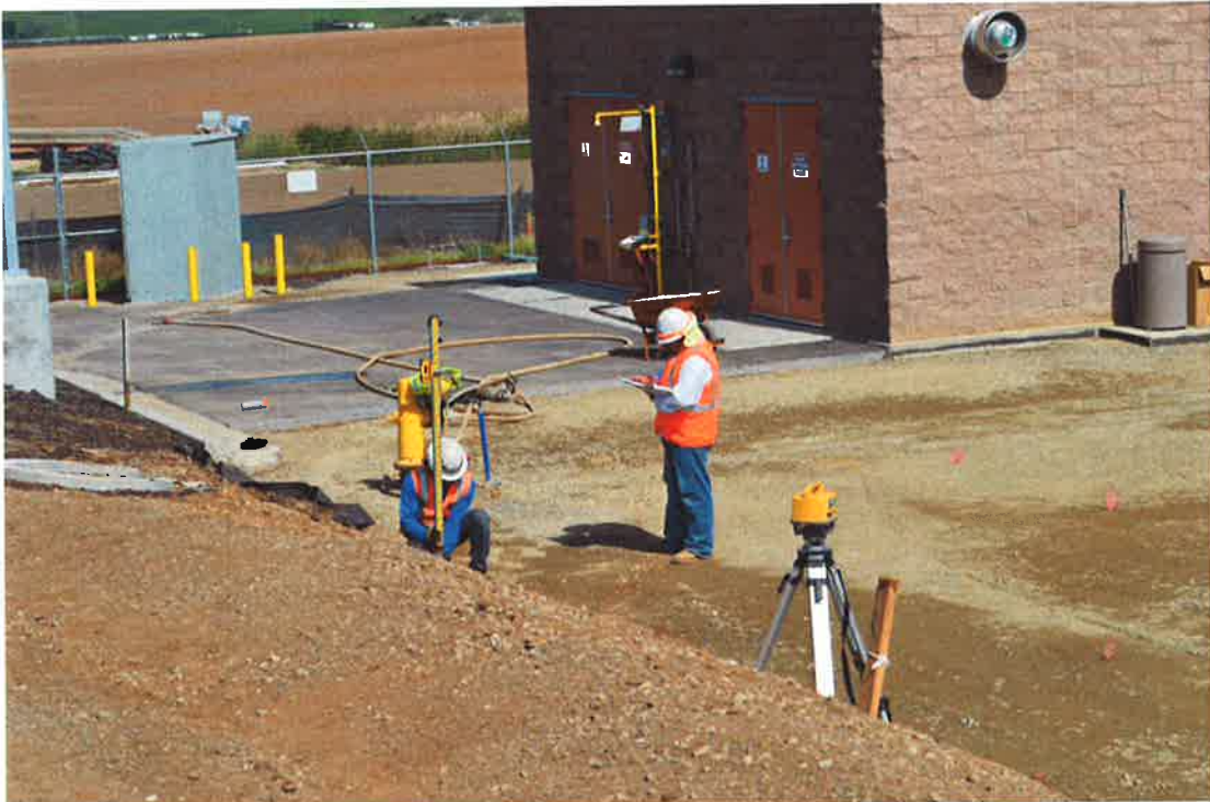
PHC checking grades to prepare for concrete work and paving.
