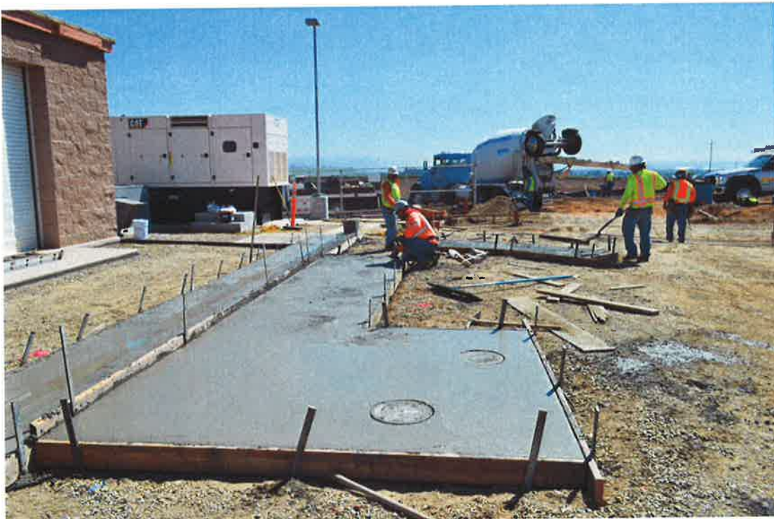
Pouring concrete around valve collars and v-ditch.
