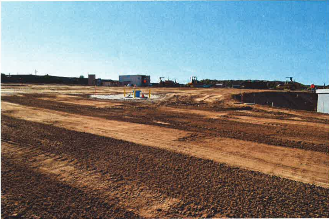
Clean-up of temporary construction easement and restoration of top soil.
