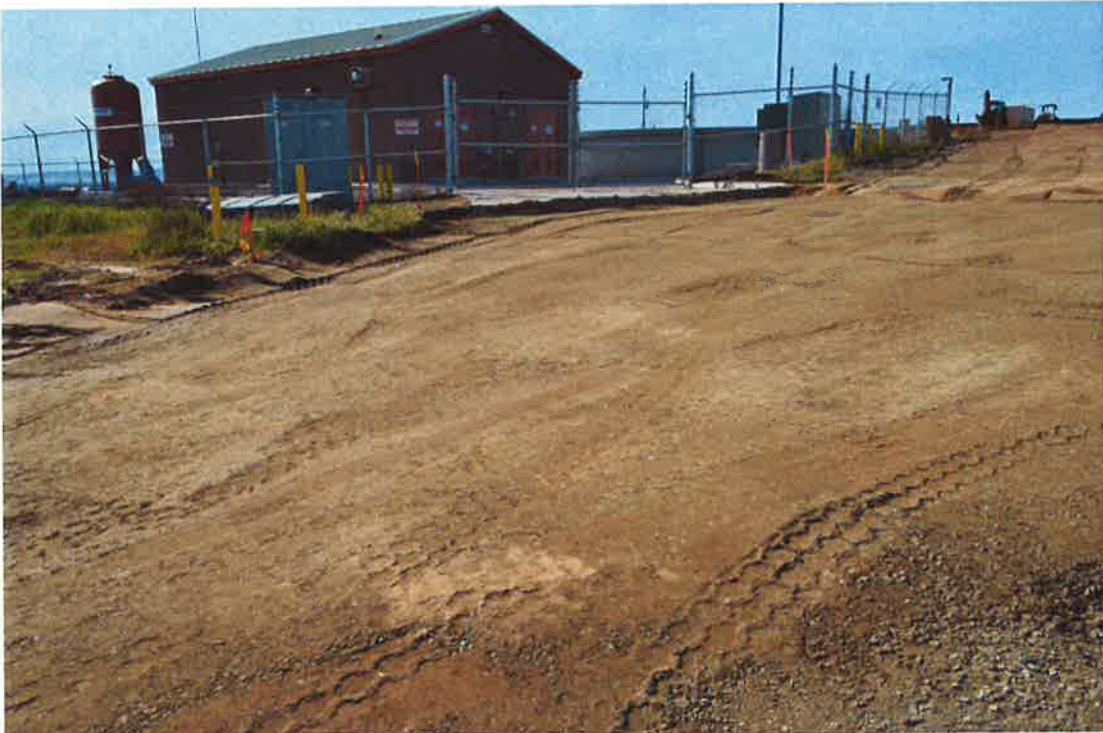
Construction of Class II AB fire truck turn around.
