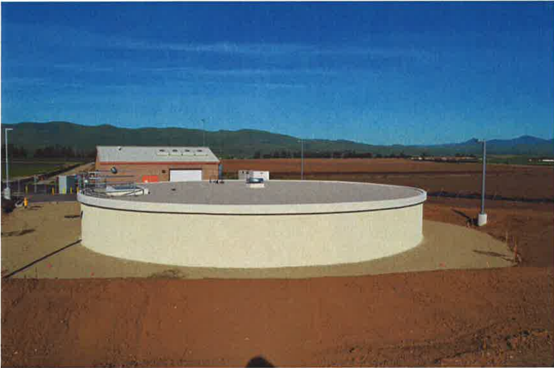
Reservoir coating completed.
