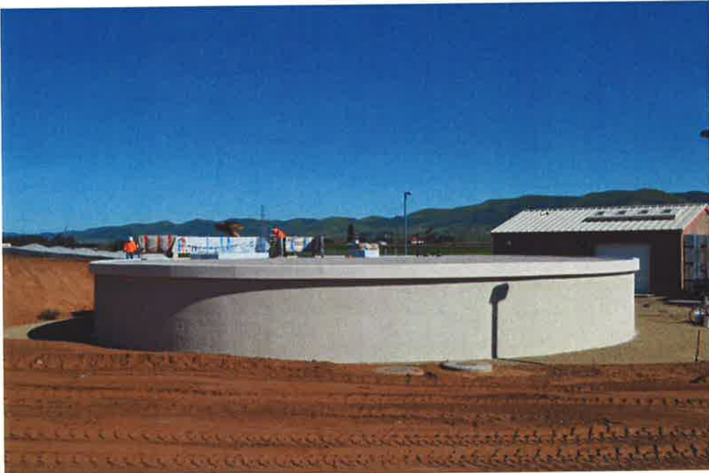
National Coating applying first layer of Carboline coating on reservoir.
