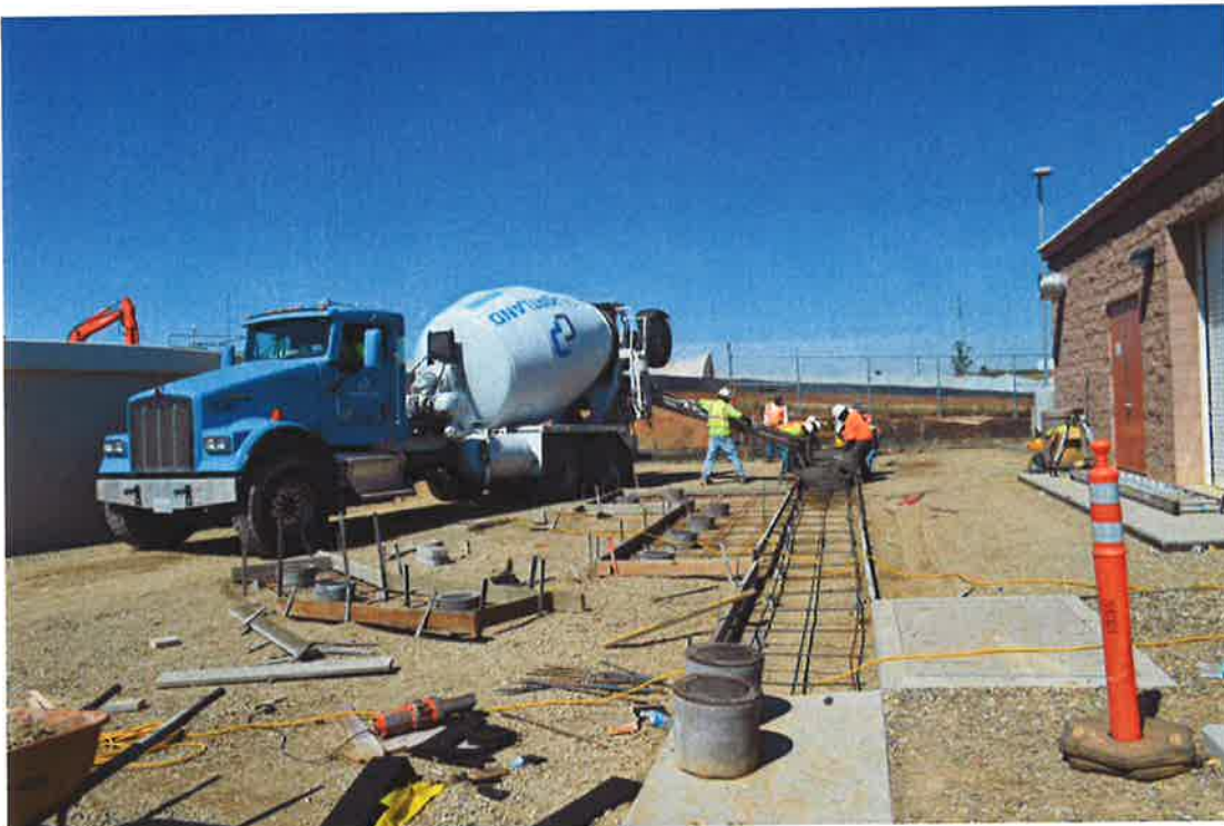
Lopez Engineering pouring concrete v-ditch.
