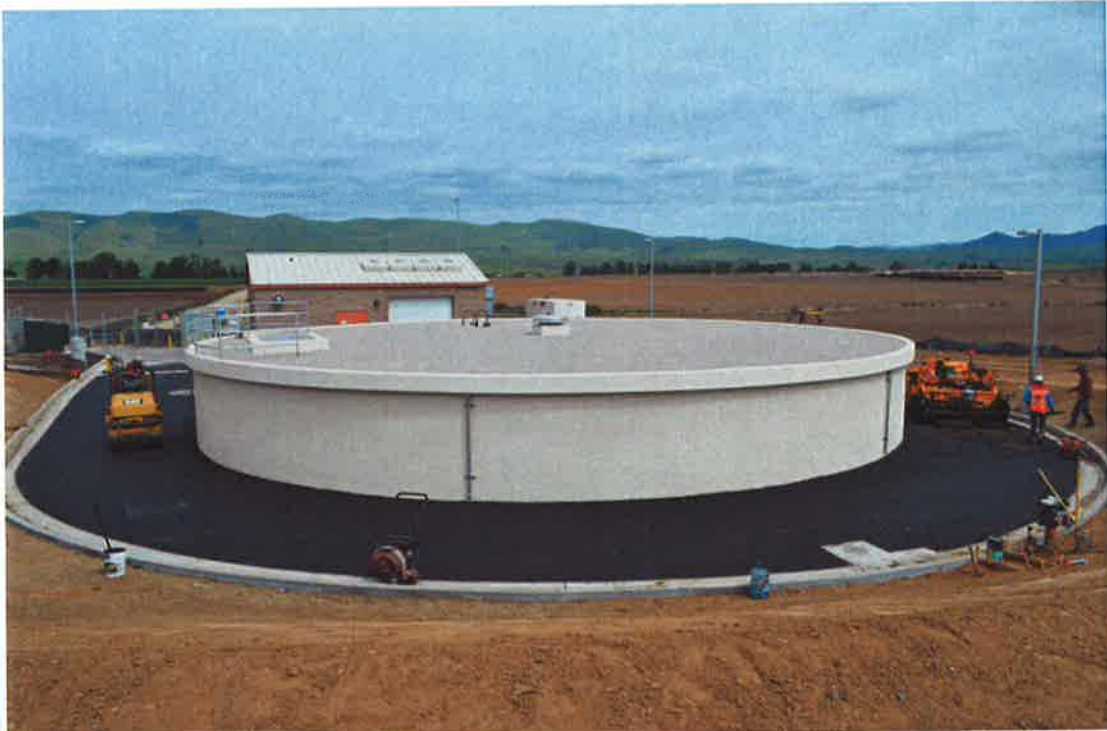
Pav-Kote finishing second layer of asphalt around reservoir.
