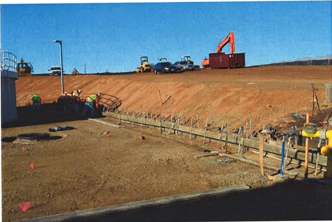
Lopez Engineering forming concrete curb and gutter.
