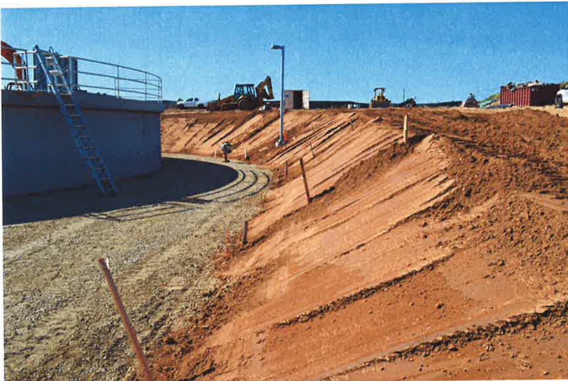
Slope around reservoir cut to a 3:1.
