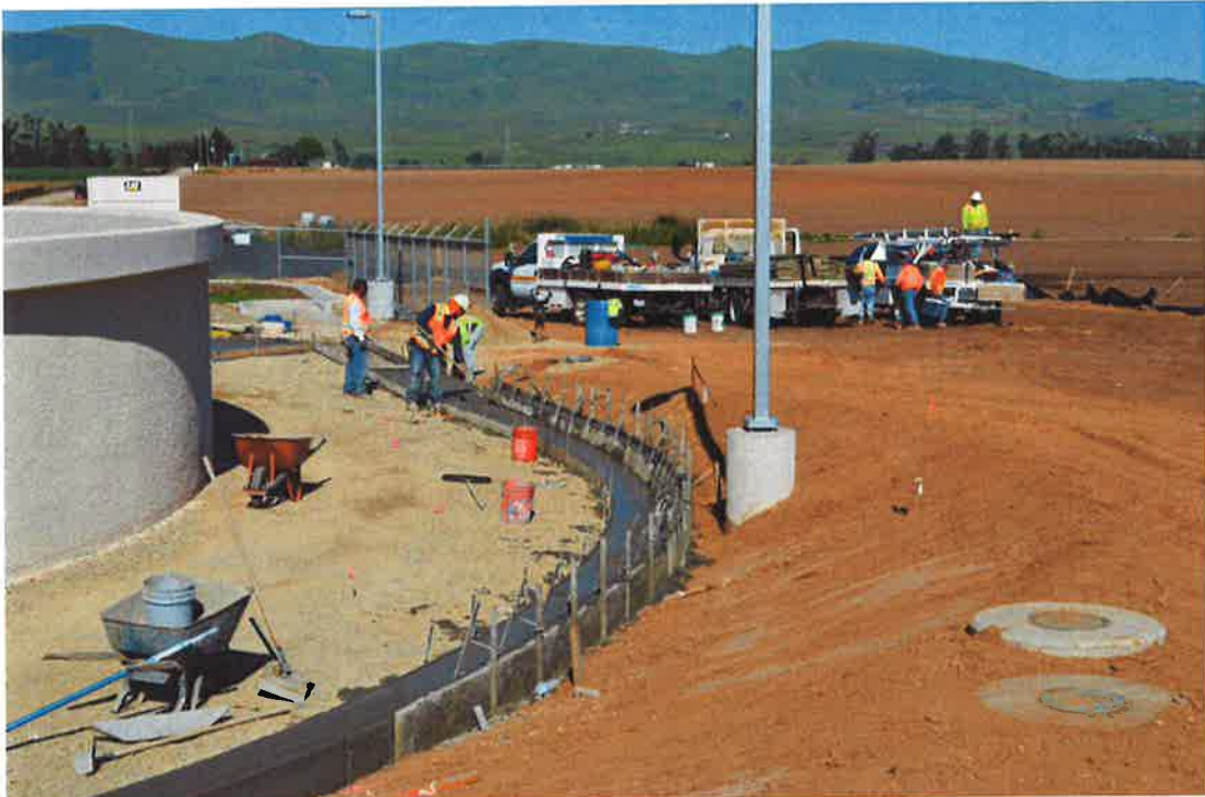
Finishing concrete curb and gutter.
