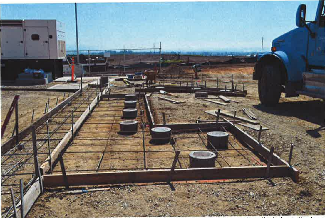
Forms and reinforcement for concrete around valve collars and v-ditch installed.
