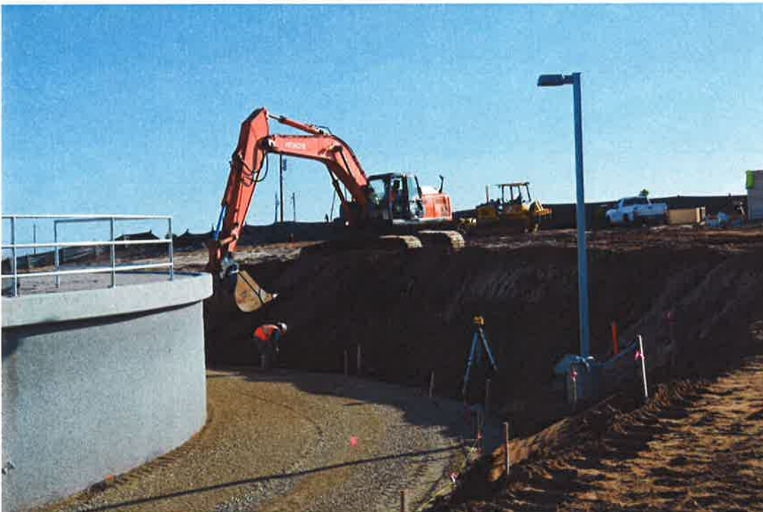
PHC continuing work to shape slope around reservoir.
