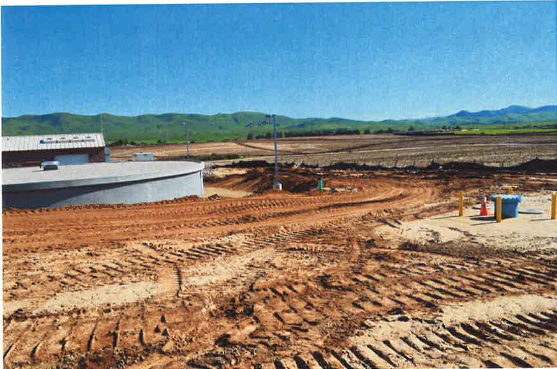
PHC grading area above slope around reservoir.
