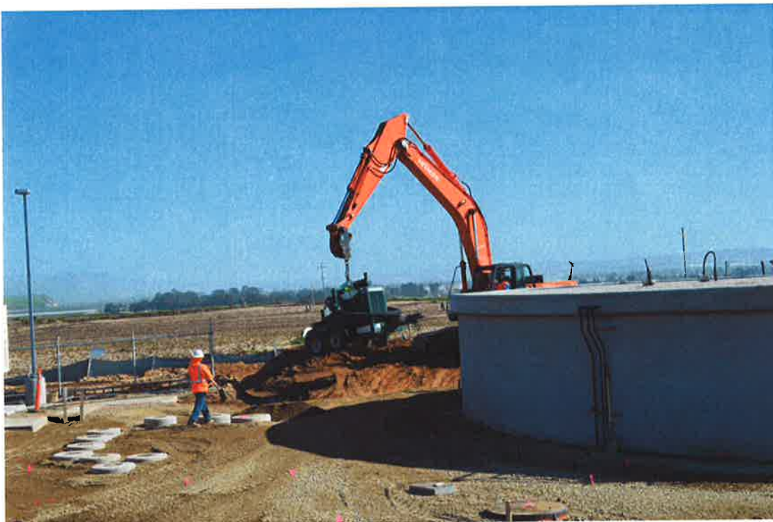
PHC setting pump on AB to prepare to drain the reservoir.
