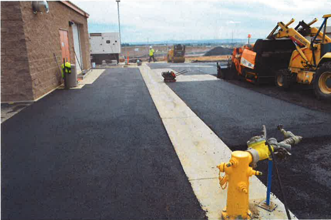
Placing second layer of asphalt.
