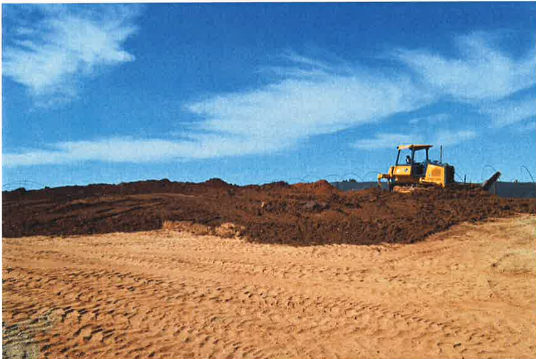
PHC restoring top soil in temporary construction easement.
