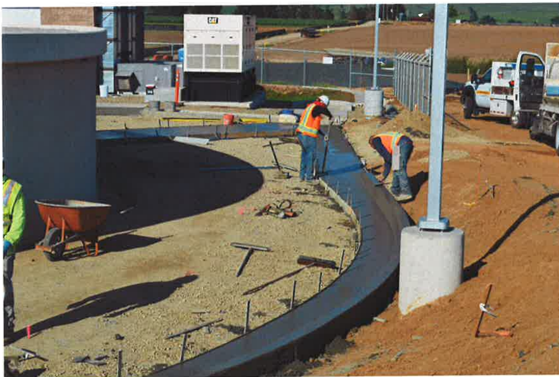
Lopez Engineering finishing concrete curb and gutter and overflow v-ditch.
