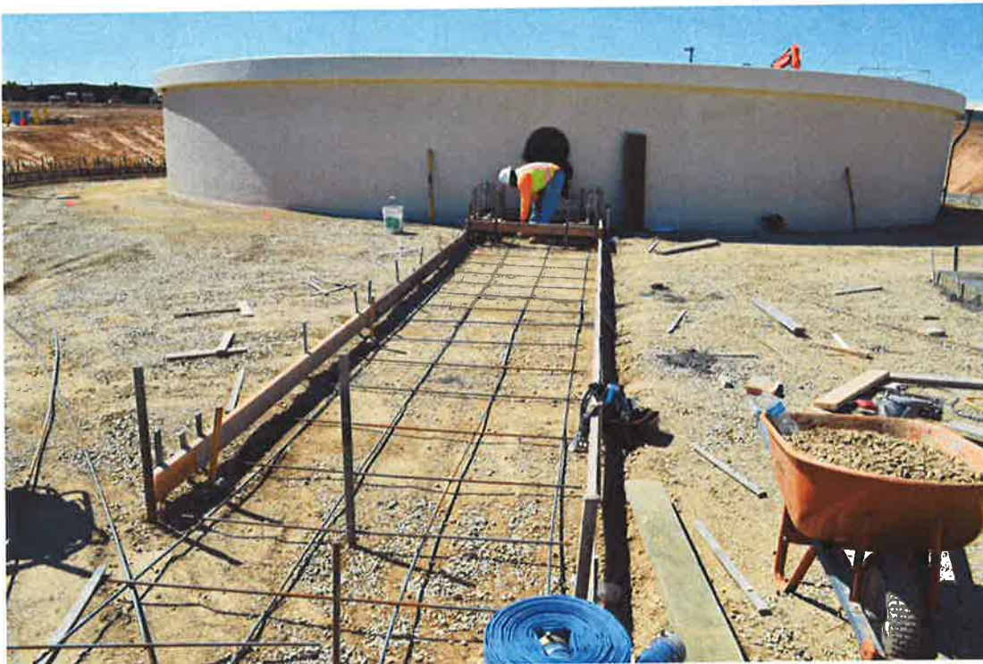
Lopez Engineering forming overflow v-ditch.
