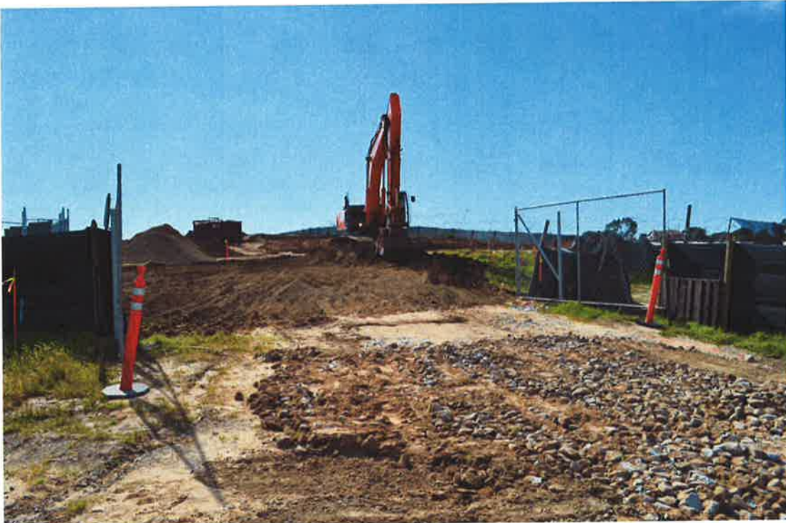
PHC installing Class II AB fire truck turn around.
