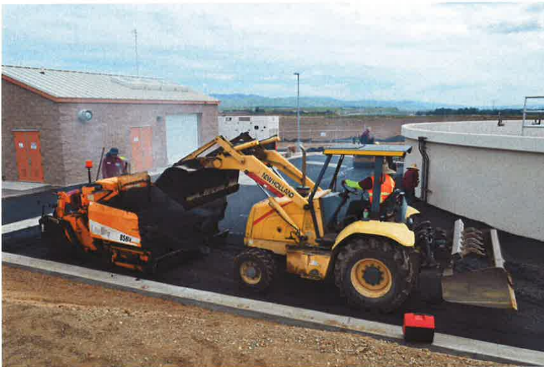
Placing second layer of asphalt.
