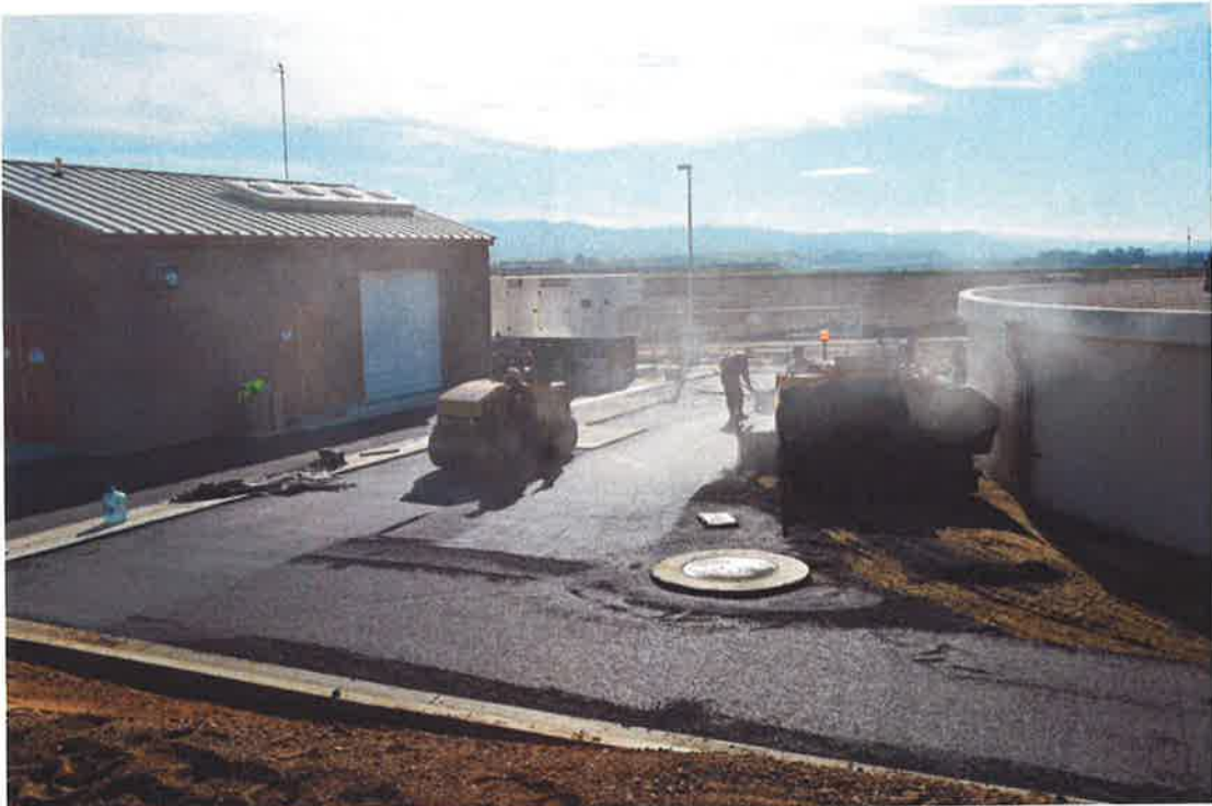
Pav-Kote placing first lift of asphalt.
