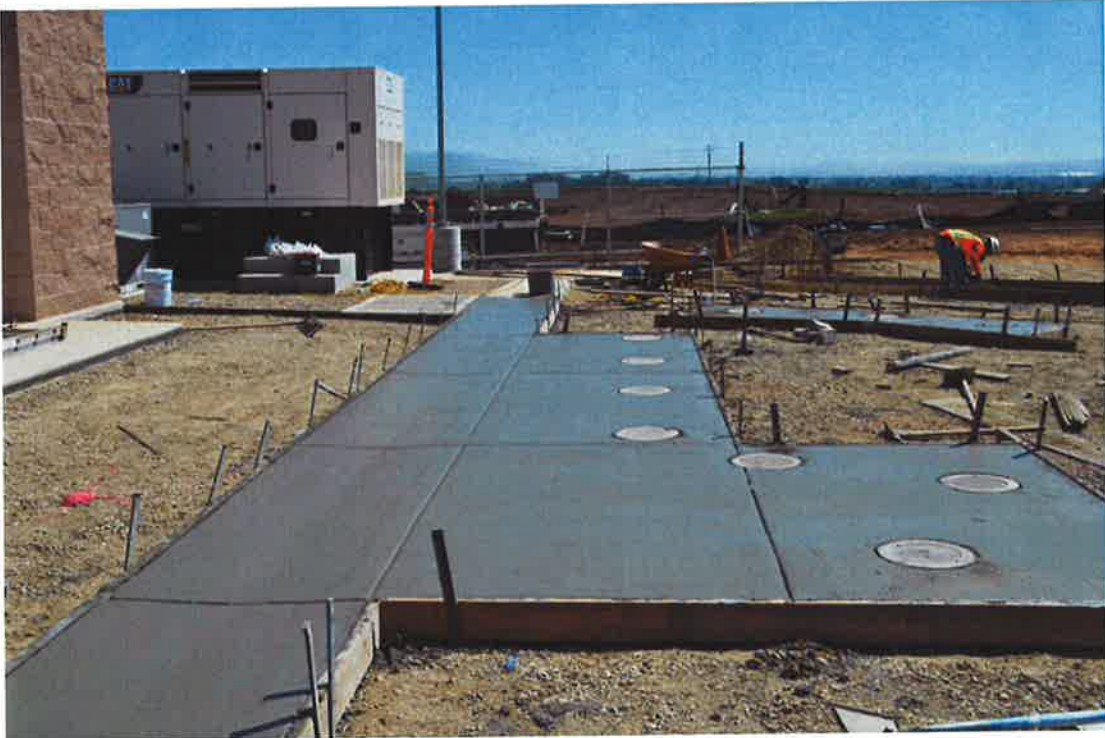
Finishing concrete v-ditch and concrete around valve collars.
