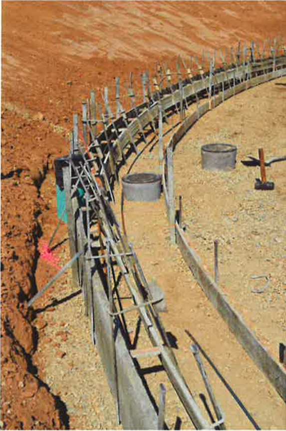
Concrete curb and gutter formed around valve cans.
