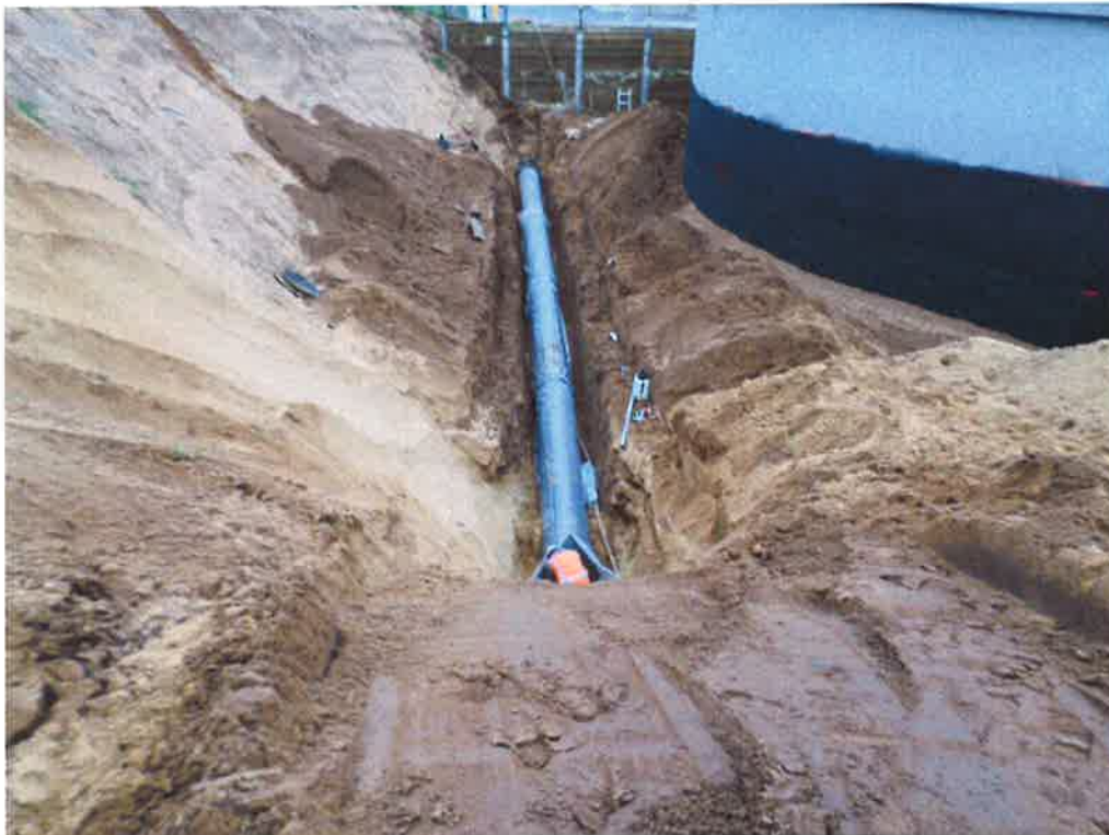
Future reservoir connection installed.
