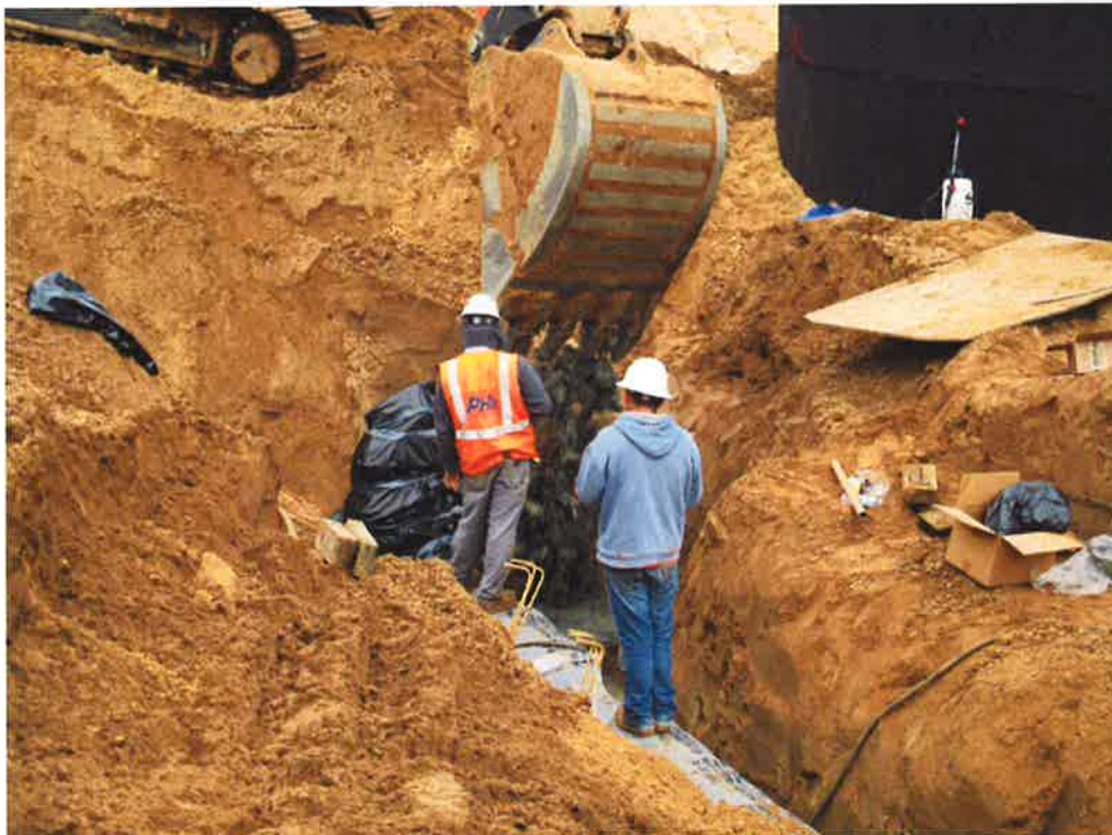
PHC pouring concrete thrust block at valves on reservoir inlet piping.
