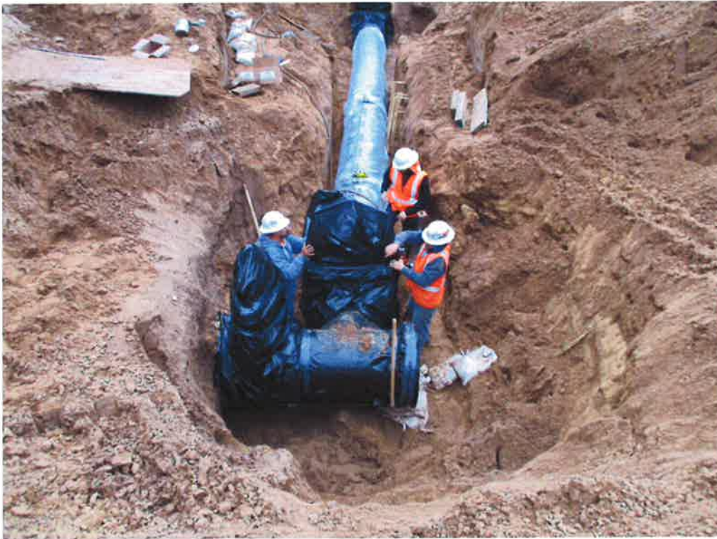
PHC wrapping reservoir inlet piping with plastic.
