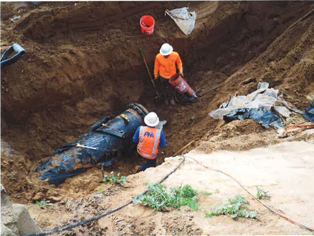
End of future reservoir piping exposed to install extension.
