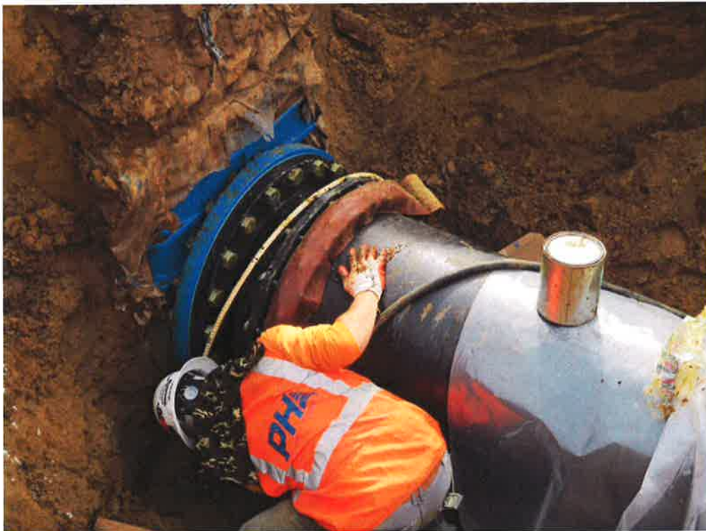
PHC applying wax tape to reservoir inlet line connection.
