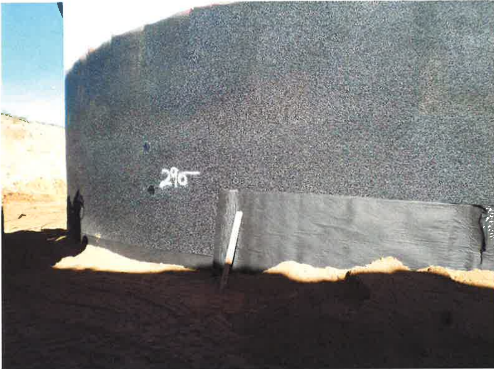
PHC installing third row of Miradrain.
