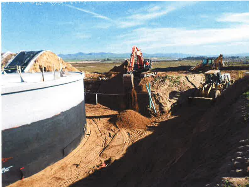
PHC backfilling after installing third row of Miradrain around reservoir.
