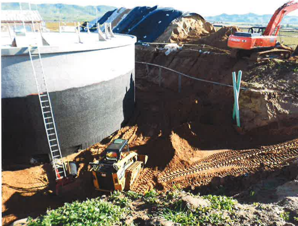
PHC backfilling around reservoir after installing second row of Miradrain.
