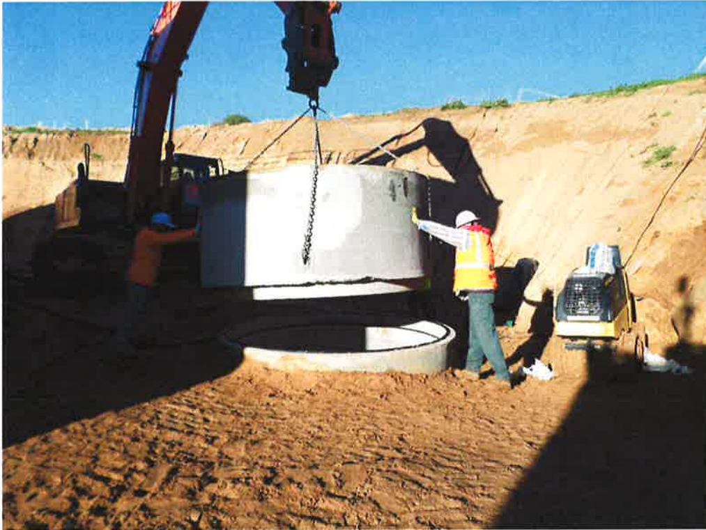
PHC adding another ring to the dewatering manhole.
