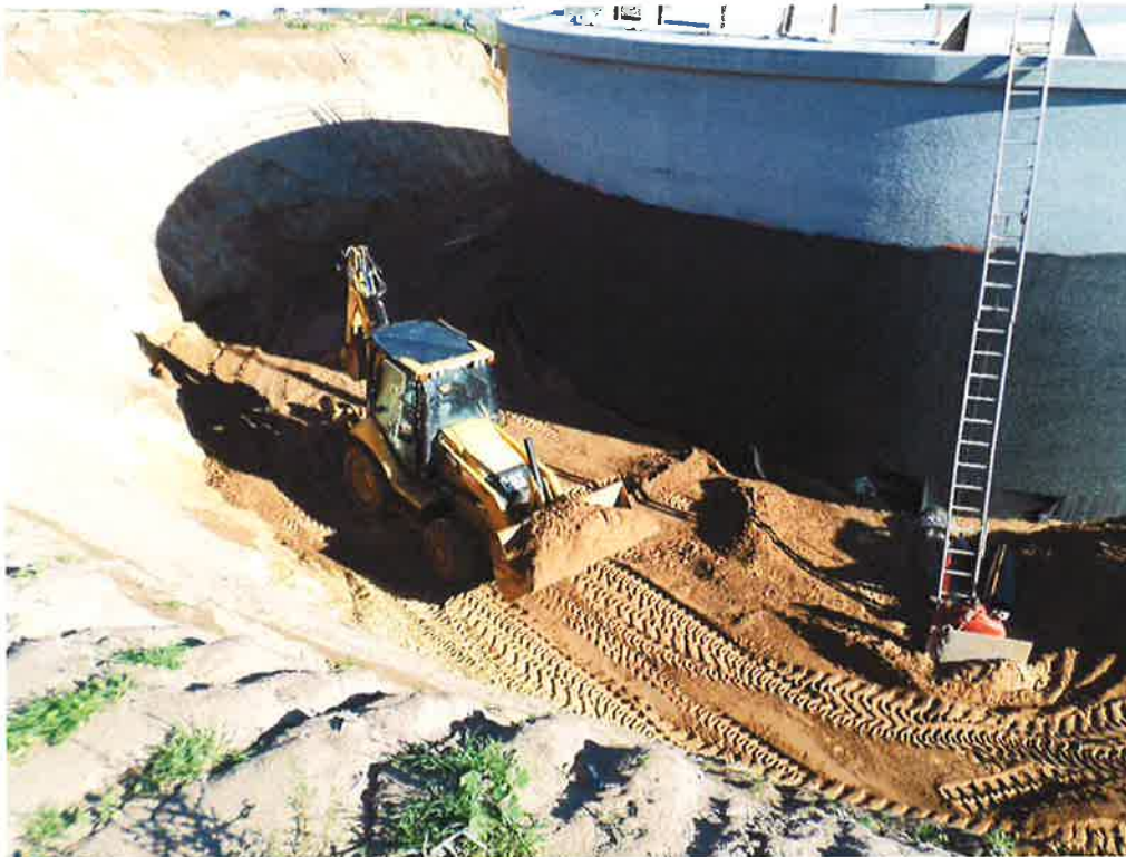
Backfilling around reservoir after second row of Miradrain was installed.
