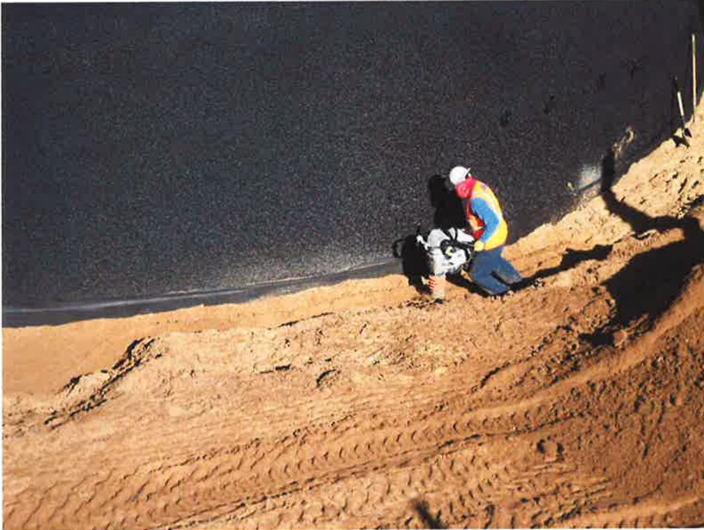
PHC compacting with whacker after installing second row of Miradrain.
