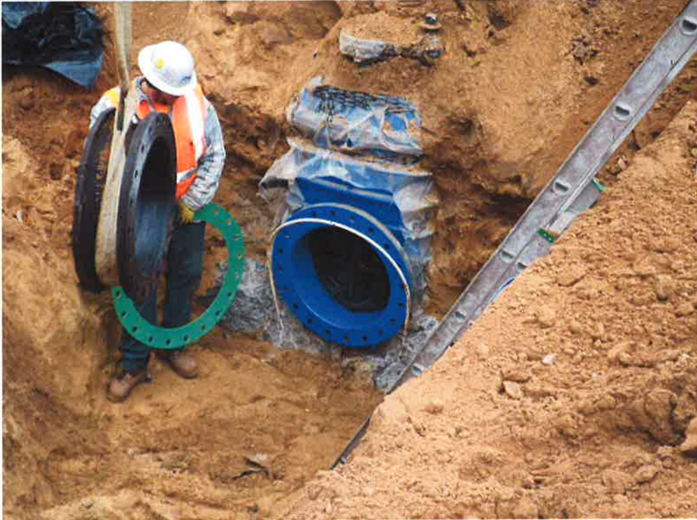
Installing flange adapter to existing valve on reservoir inlet piping.
