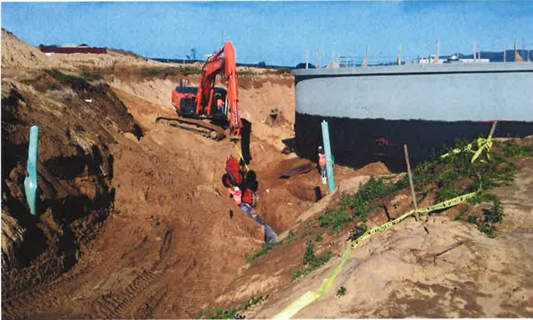
PHC installing tee and valve on reservoir inlet piping.
