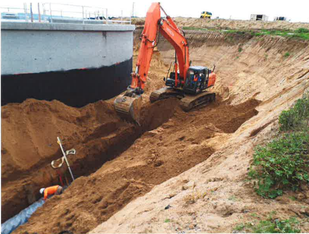
PHC excavating to continue to extend future reservoir connection.
