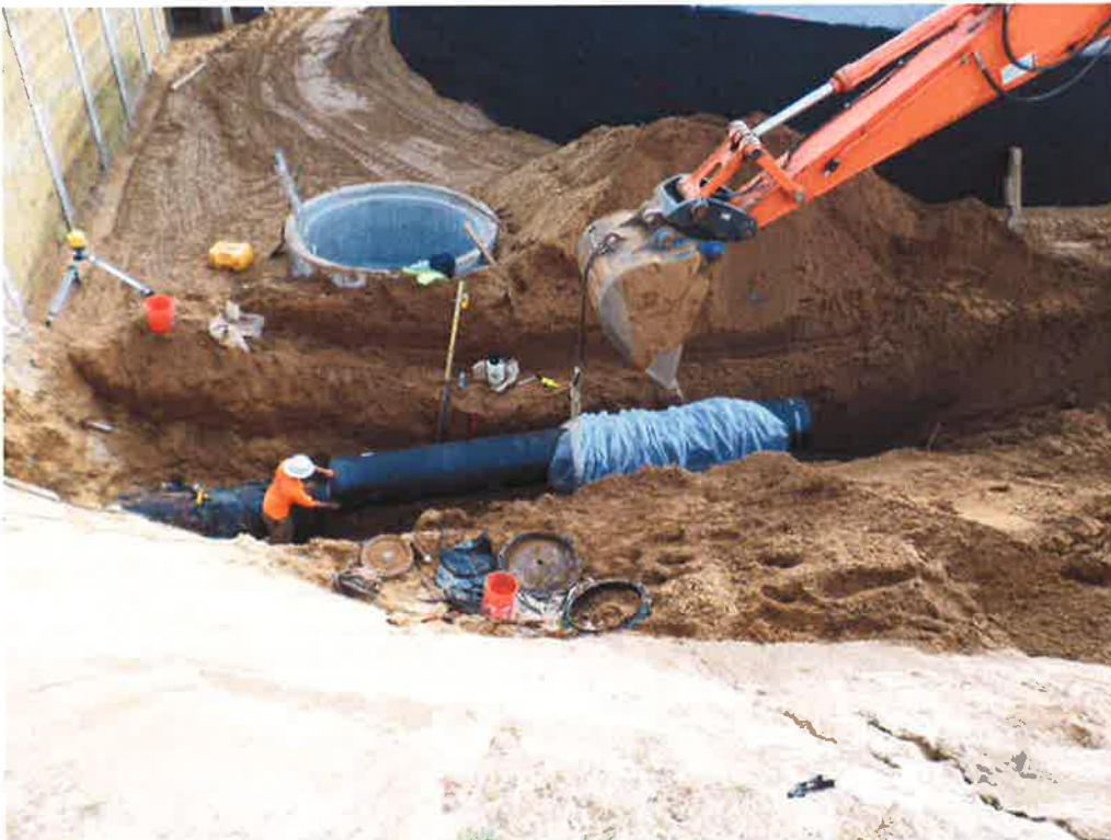
PHC installing 24-inch ductile iron pipe to extend future reservoir connection.
