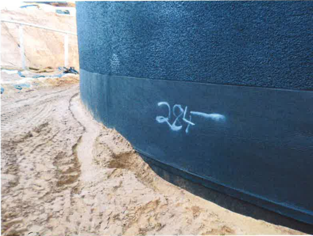
PHC installing second row of Miradrain.
