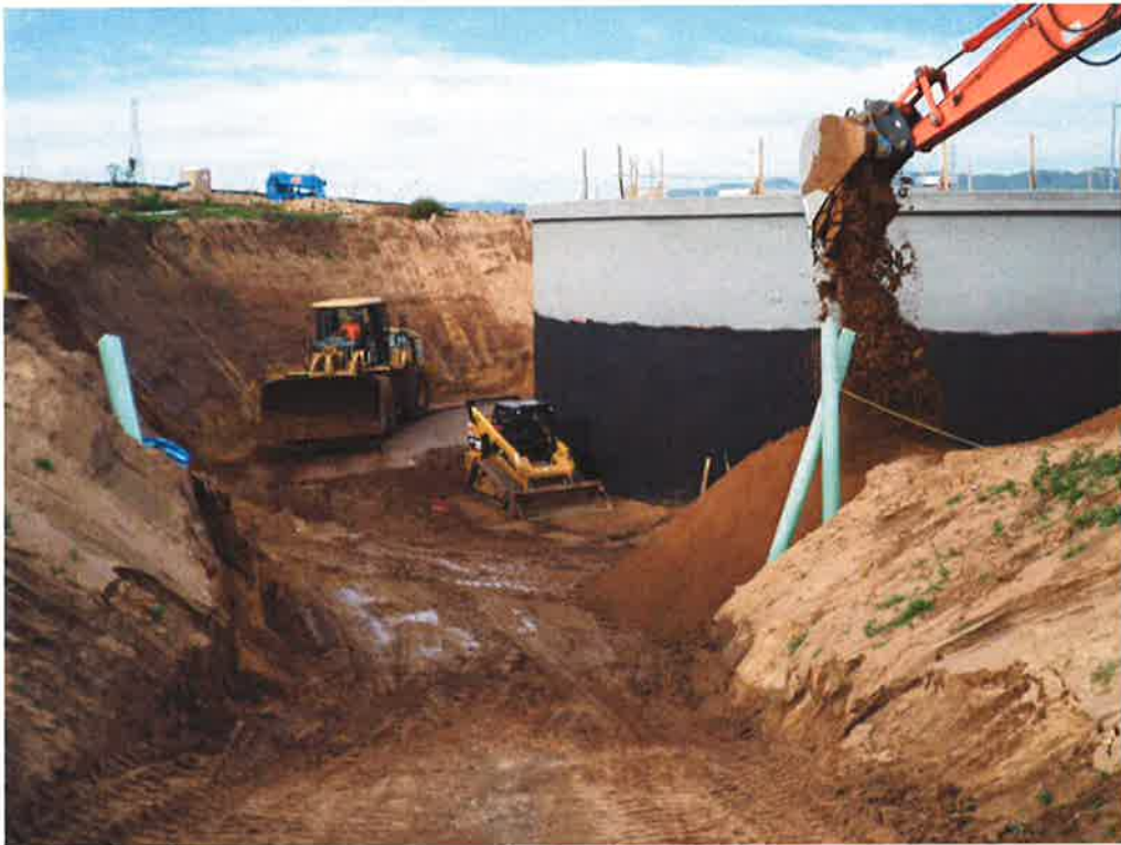
Backfilling after installing third row of Miradrain around reservoir.
