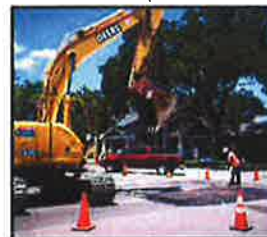
Site Repairs see pages 24-29
