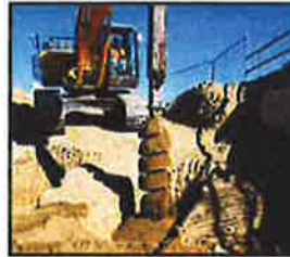
Lift Station Replacement and Rehabilitation see pages 24-27
