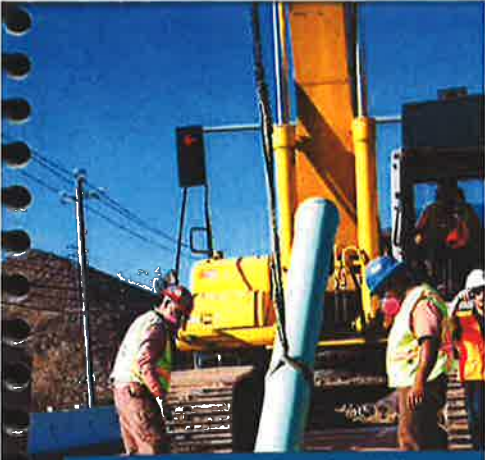
This project involved the construction of a new regional lift station.
