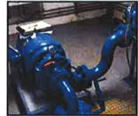
Piping and Pump Replacement and Rehabilitation see pages 24-27
