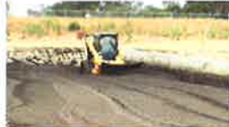
Nipomo's wastewater treatment plant. (KSBY photo)
