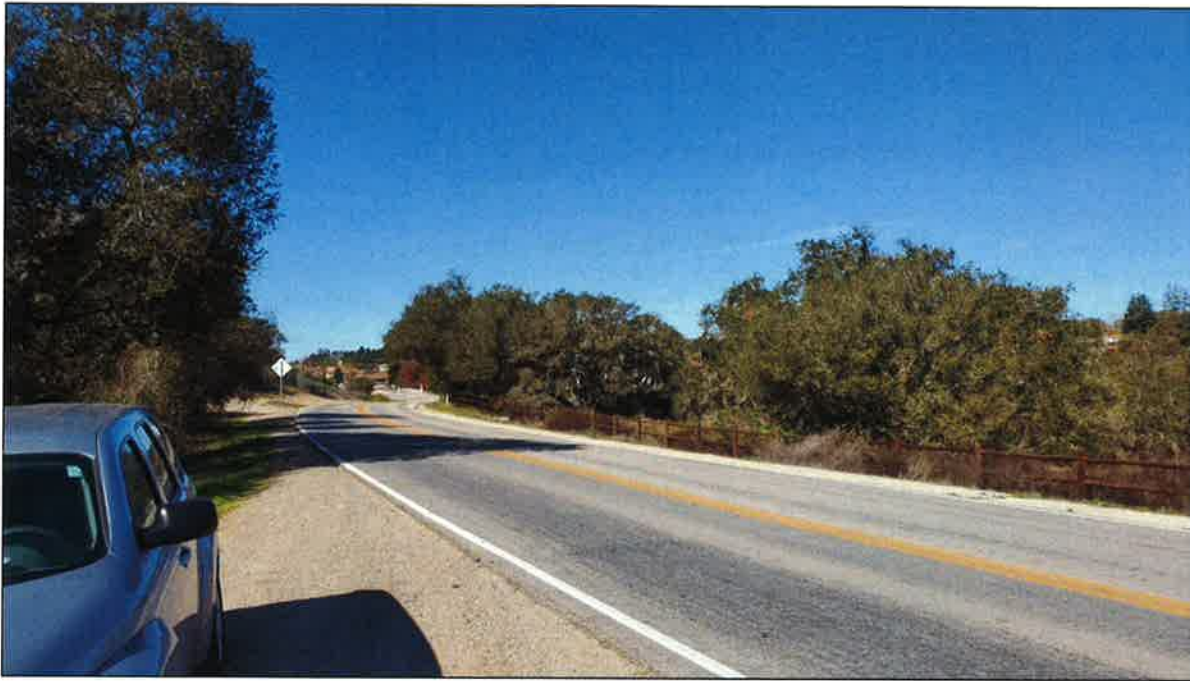
Figure 6. View of Camino Caballo near Camino Caballo/Pomeroy Road intersection, facing west (February 19, 2021).
