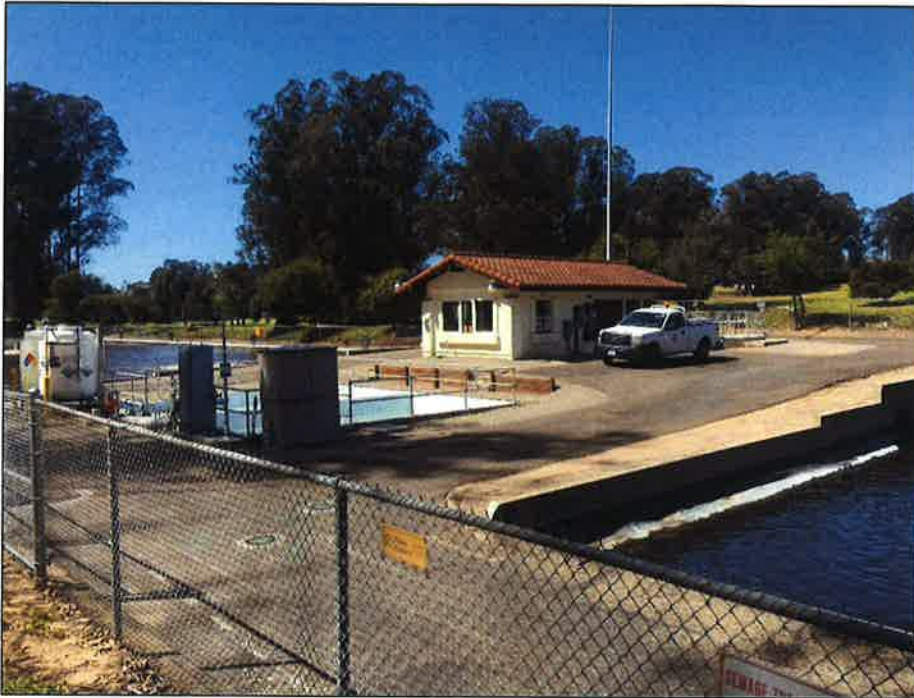
PHOTO 5. View facing northwest of the Blacklake Water Reclamation Facility control building.
