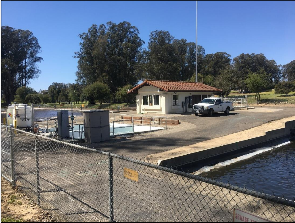
PHOTO 5. View facing northwest of the Blacklake Water Reclamation Facility control building.
