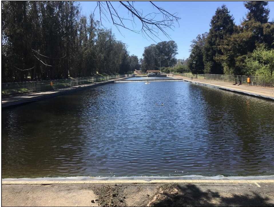
PHOTO 1. View facing west of the Blacklake Water Reclamation Facility and sewage treatment ponds.
