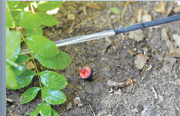
Missing drip emitter
