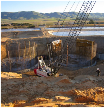
Southland Wastewater Treatment and Reclamation Facility Upgrade Under Construction
