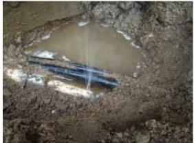
Most of these extreme cases involved landscape irrigation systems - including lateral lines to remote hose connections. On this sand dune we affectionately call 'The Mesa', water infiltrates very quickly and even large leaks can go undetected. Many smaller leaks or simply overwatering occur routinely in many homes.
