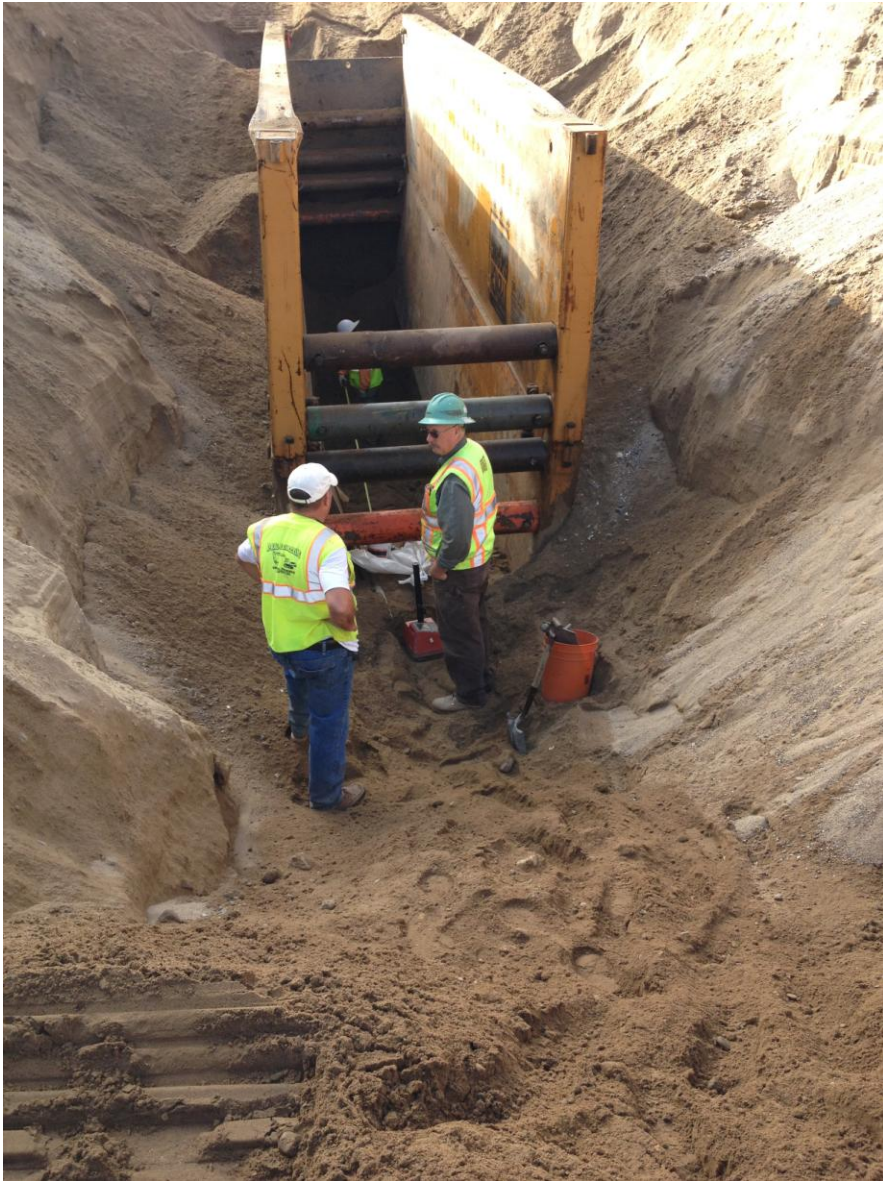
Furgo testing backfill compaction.
