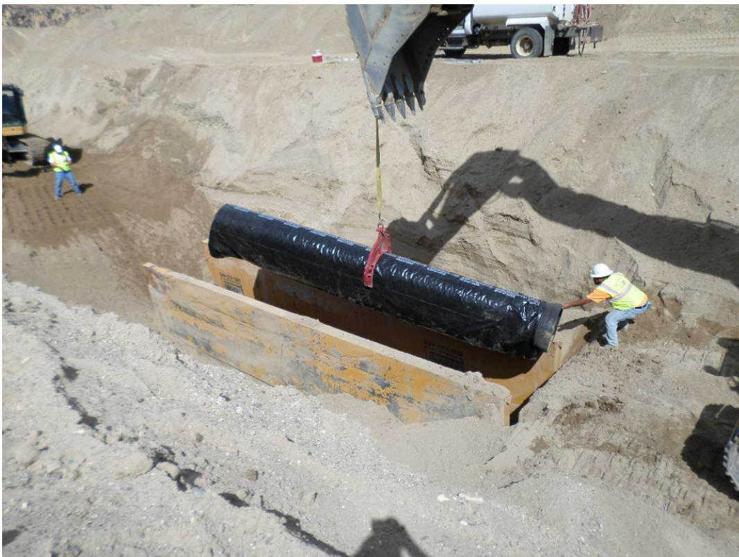
D-KAL installing 24-inch DIP.
