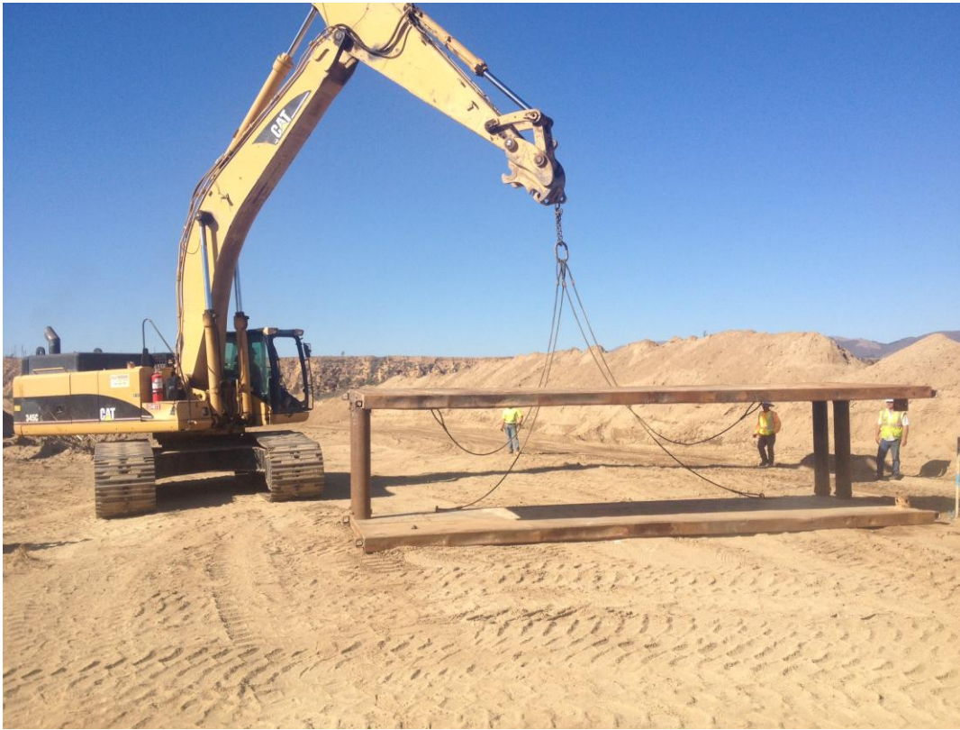
D-KAL assembling trench shoring.
