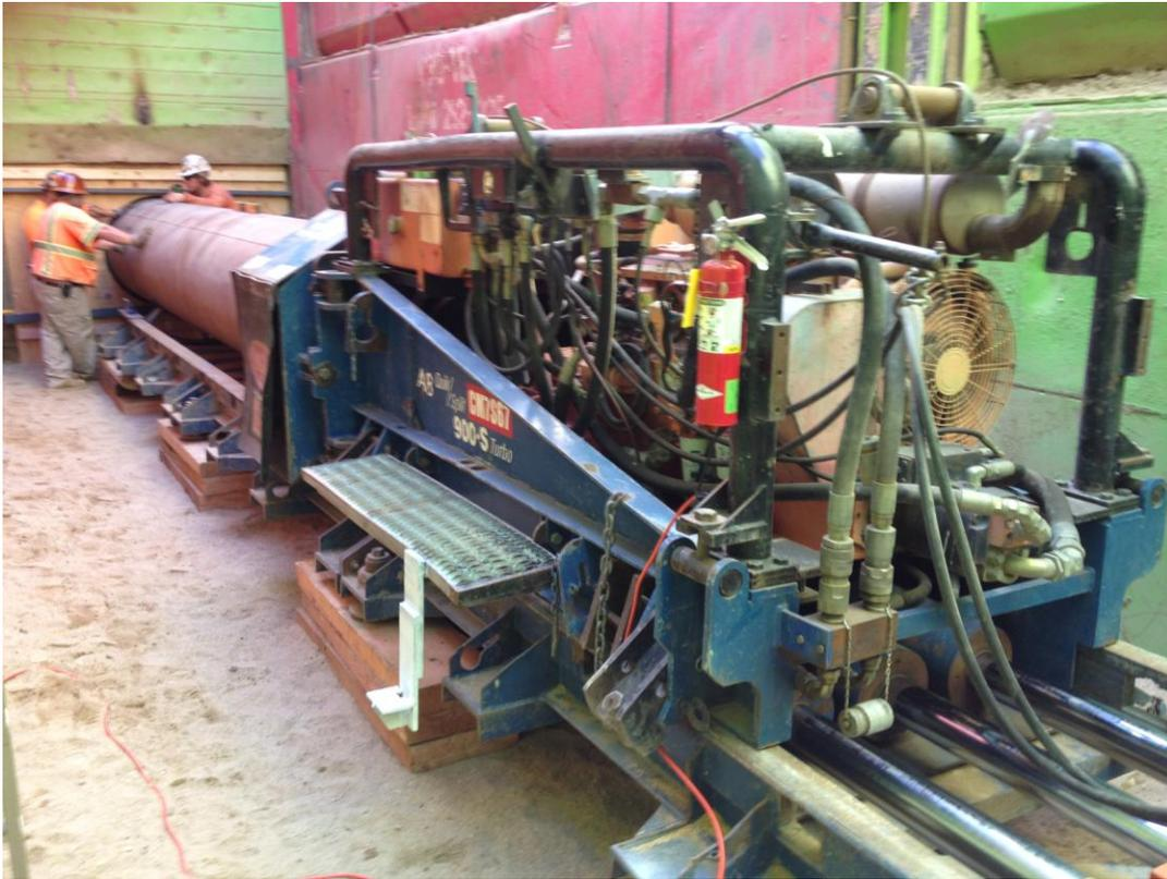
Pacific Boring operating bore and jack machine to begin boring first 36" steel casing section.
