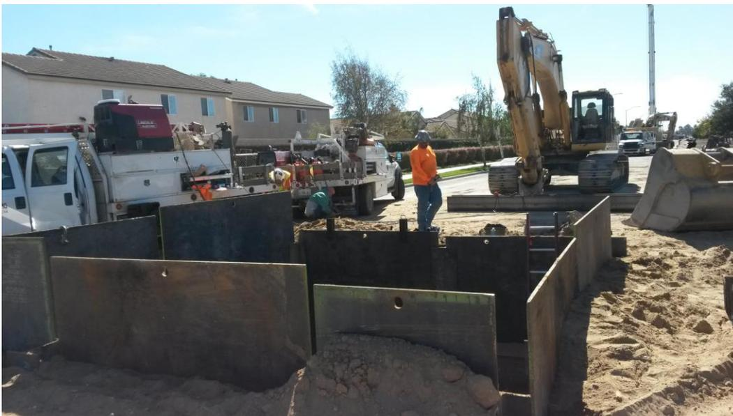
First layer of steel plates driving down between I-beams at receiving pit.
