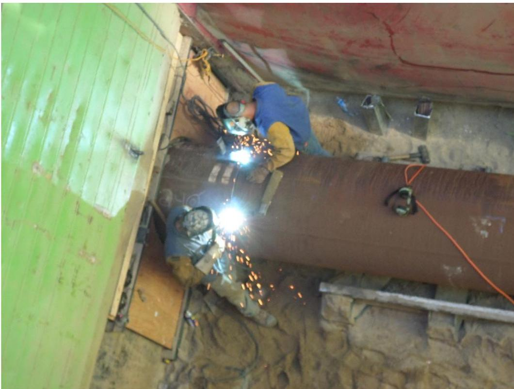
Pacific Boring welding another section of 36-inch casing to the one installed.
