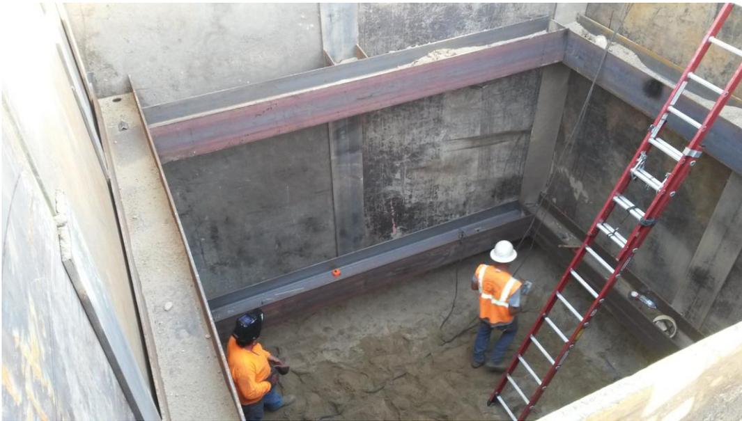
D-KAL welding second layer of horizontal supports inside the receiving pit at approximately 16 feet.
