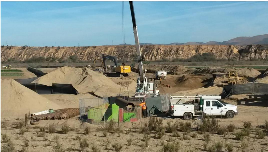
Pacific Boring placing another section of 36-inch steel casing pipe and auger into bore and jack pit.
