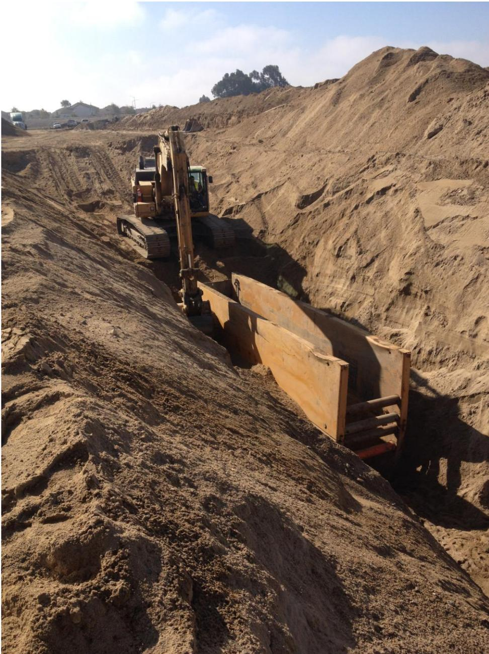
D-KAL excavating beside trench shield to set it in place for more pipe installation.
