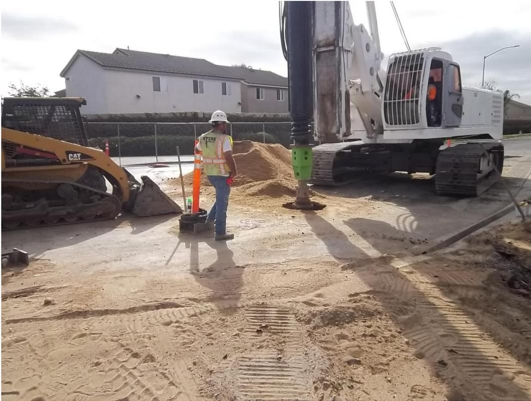
D-KAL subcontractor Meyers Drilling installing steel I-beams in Blosser Road for the receiving pit.
