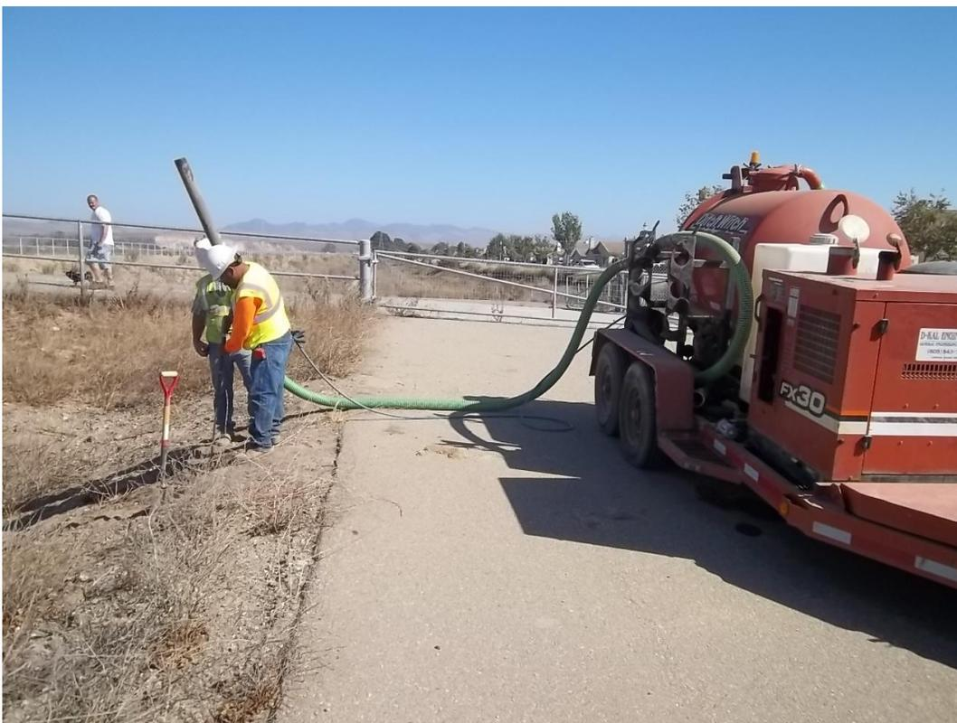
D-KAL installing settlement monitors on the levee to monitor any changes during the bore and jack operation.
