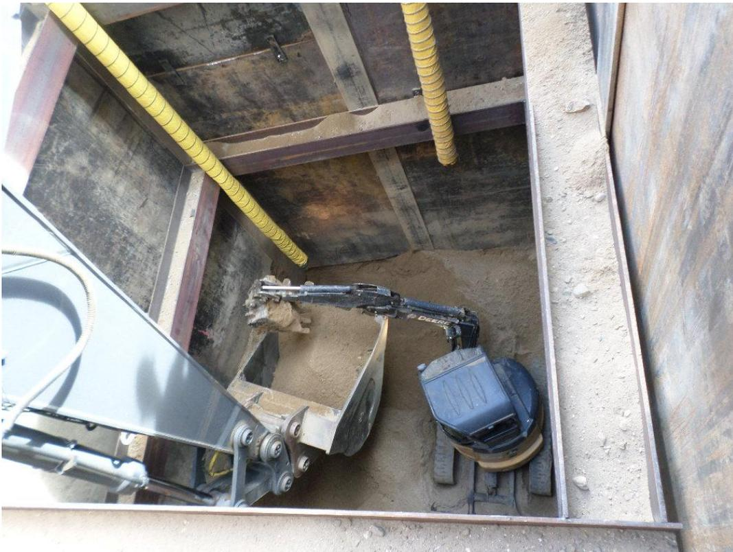
D-KAL using mini-excavator and JD 850 excavator in receiving pit at approximately 27 feet deep, digging to final grade of 37 feet.
