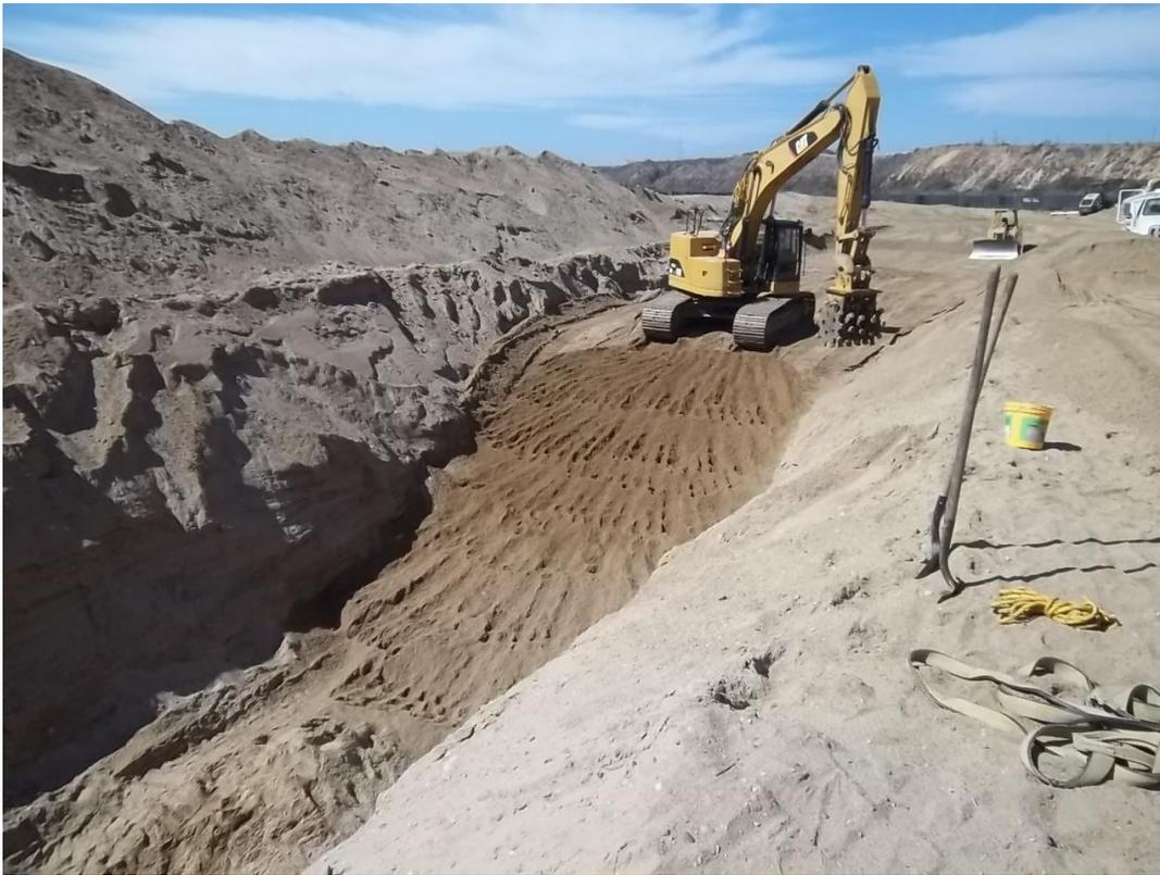
D-KAL backfilling and compacting over 24-inch DIP in river area.
