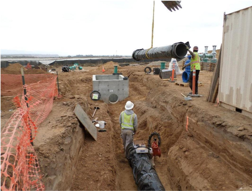
Spieß installing pipe to metering vault.
