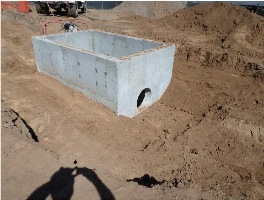
Spieß backfilling around the metering vault.
