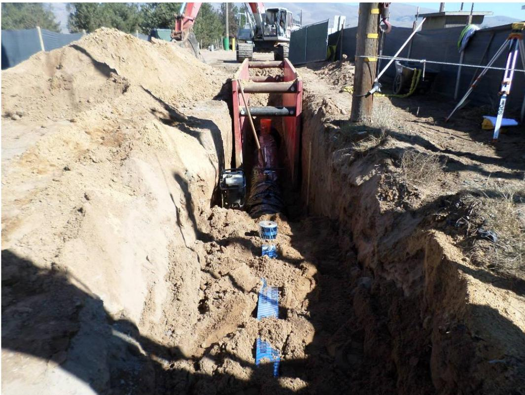
Spiess installing the 24-inch DIP past the PG&E power pole at the edge of the access road while the pole is supported by PG&E.
