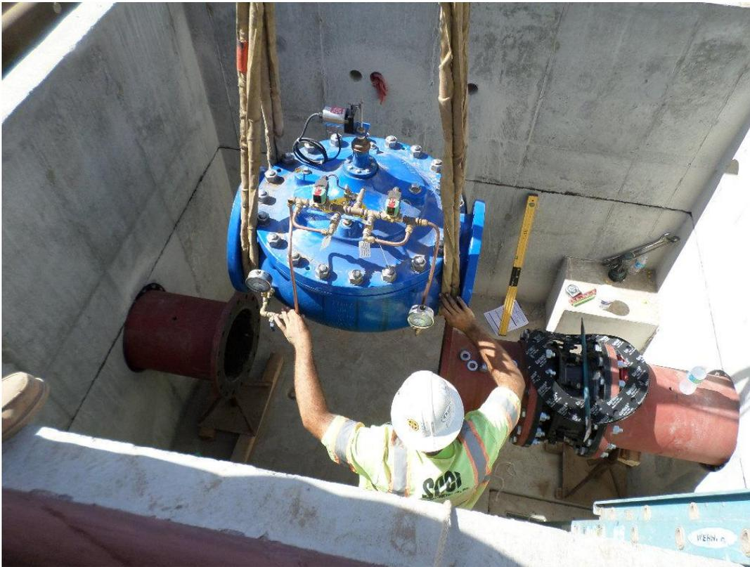
Spiess installing flow control valve.
