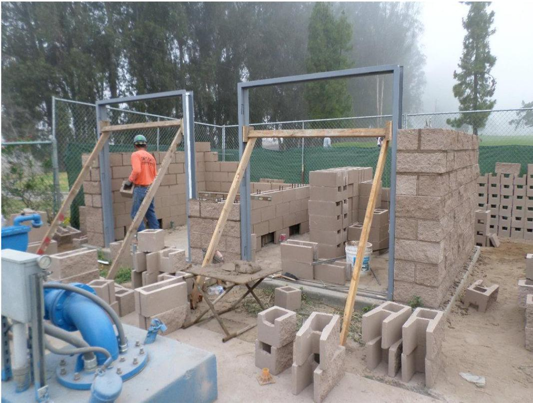
Door frames installed by Spiess and Rocky Boydston Masonry installing block walls at the chemical building.
