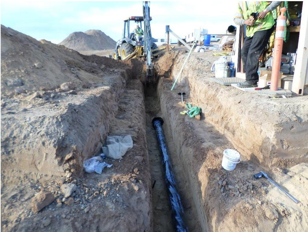
Spieß installing 6-inch DIP for the fire hydrant located on site.
