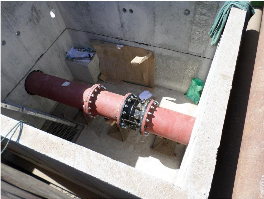
Spiess assembling piping in metering vault.
