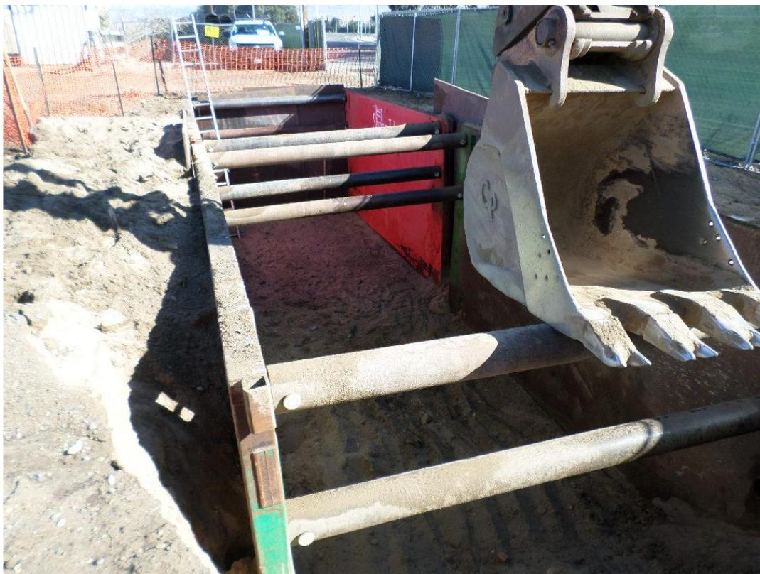
Spiess installing shoring for vaults excavation.
