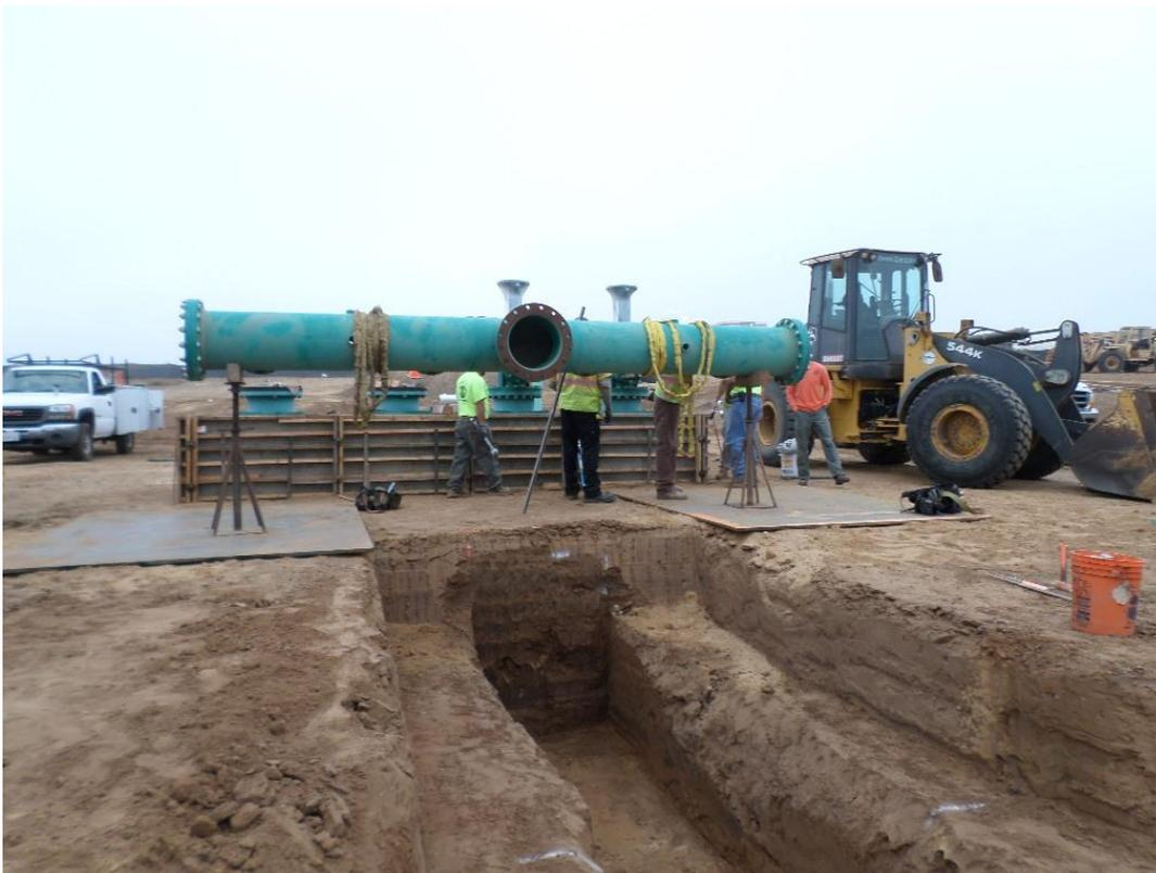
Spies aligning manifold and excavating for discharge pipe and encasement.
