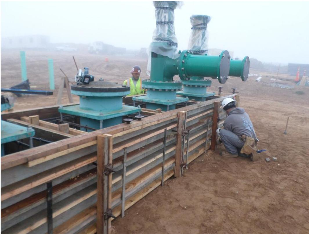
Forms installed for pump pedestals.
