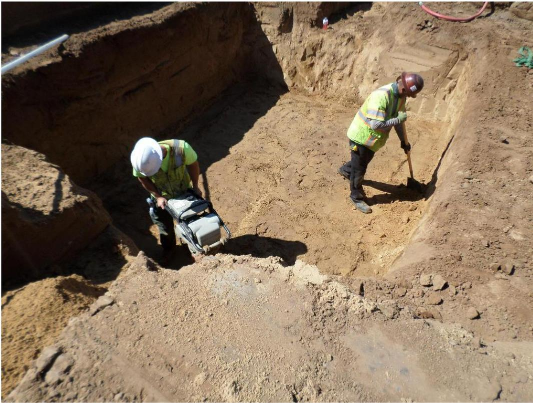
Spiess compacting subgrade for the metering vault.
