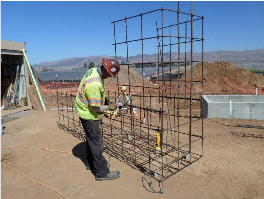
Spieß building rebar for concrete encasement of discharge pipe.
