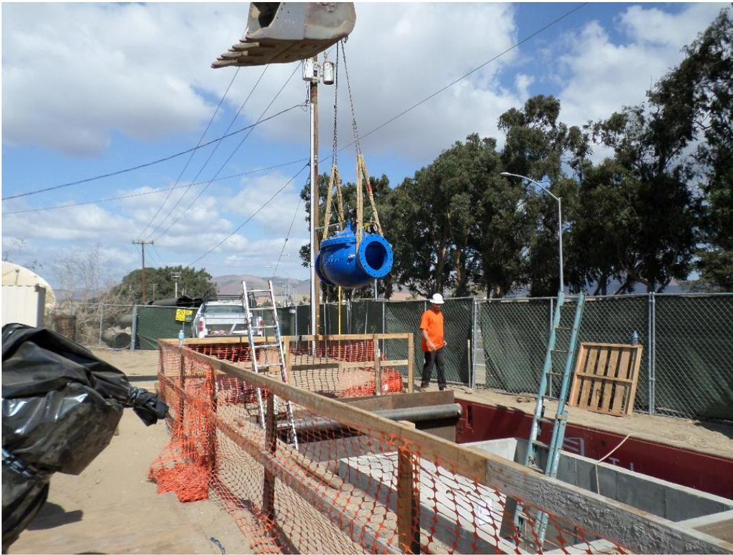
Spiess installing flow control valve.
