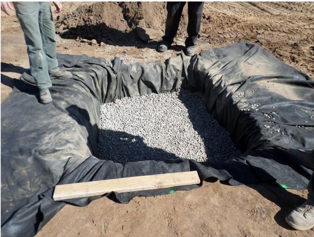
Spieß rock and fabric installed for base underneath catch basin.
