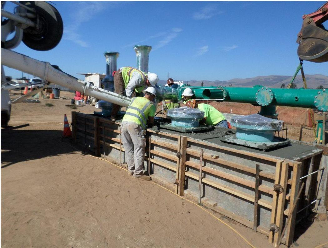
Spiess pouring the pump pedestals at the same time as the discharge pipe encasement.
