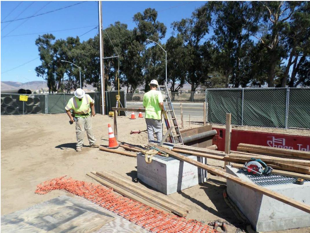
Spiess installing the safety hand rail around the top of the vault shoring.
