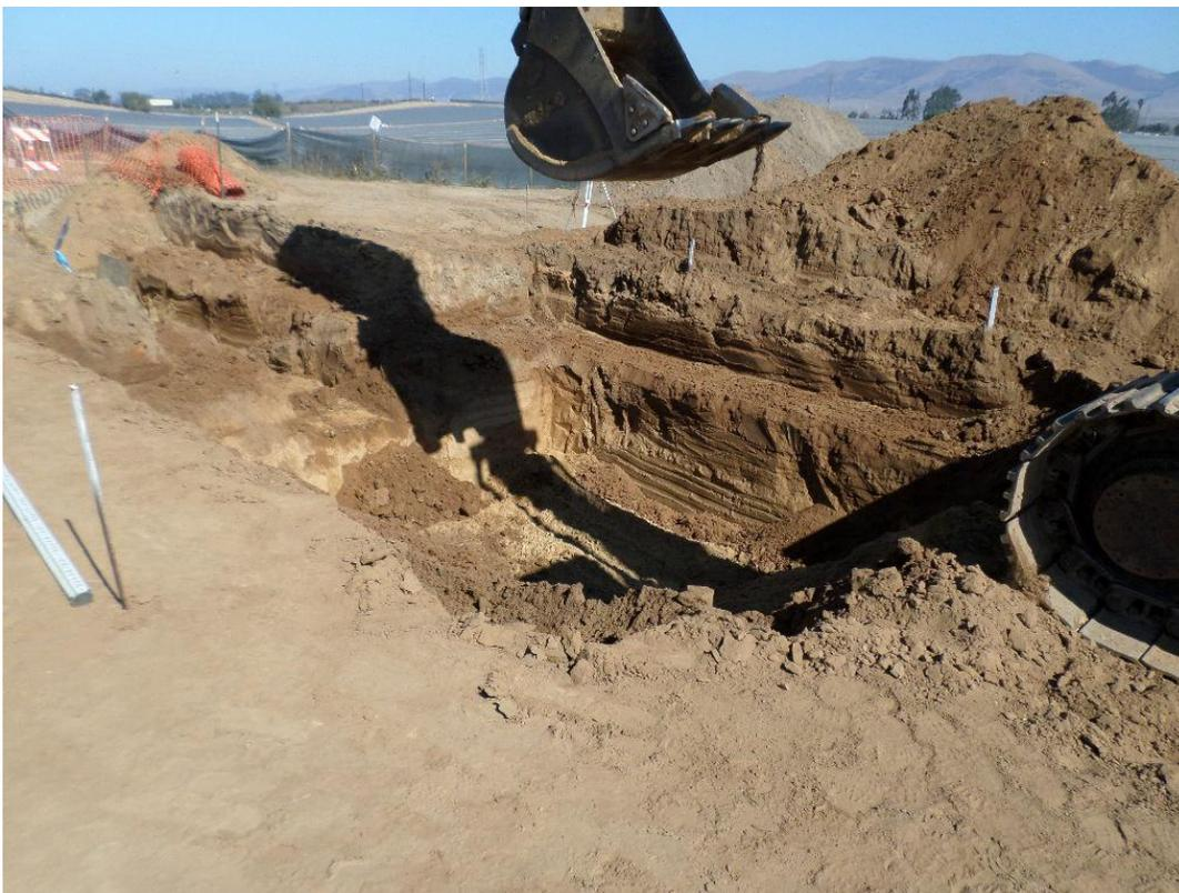
Excavating for metering station vault.
