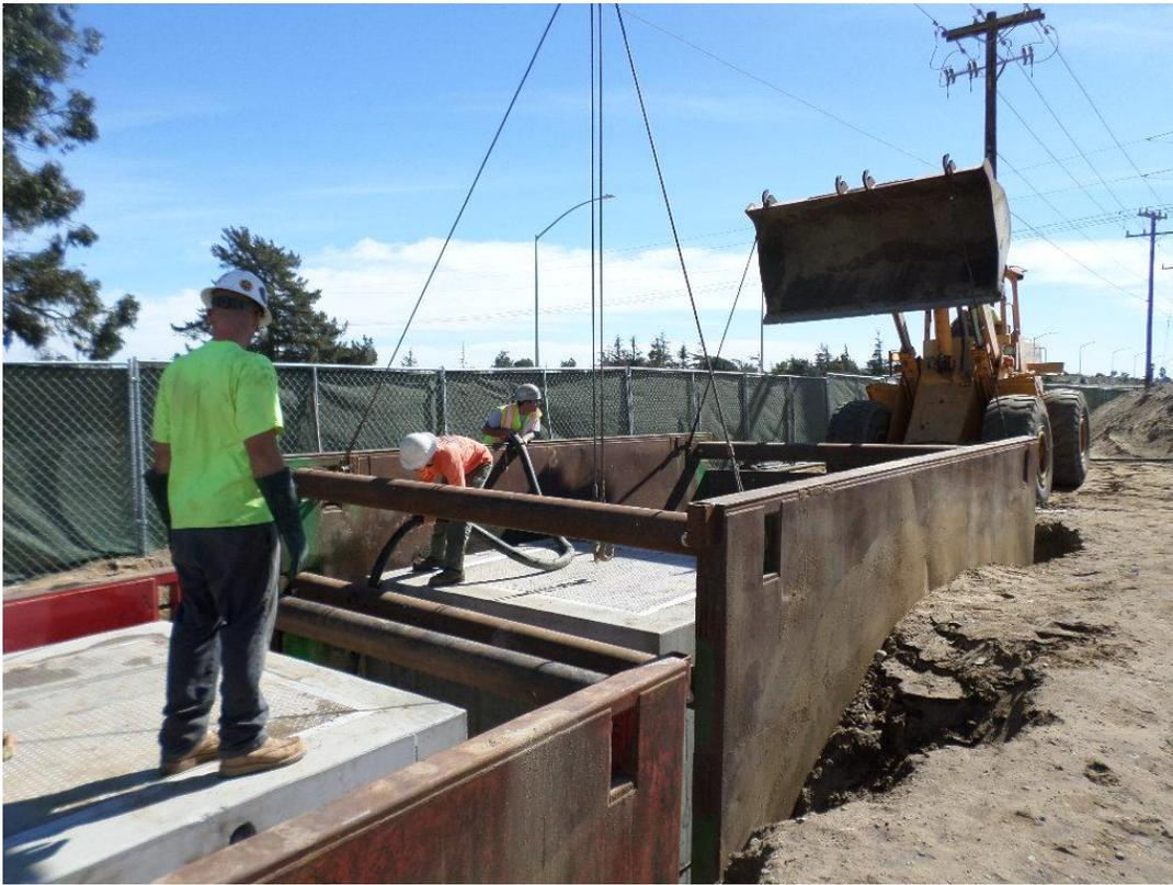
Spieß pouring slurry around vaults for backfill.
