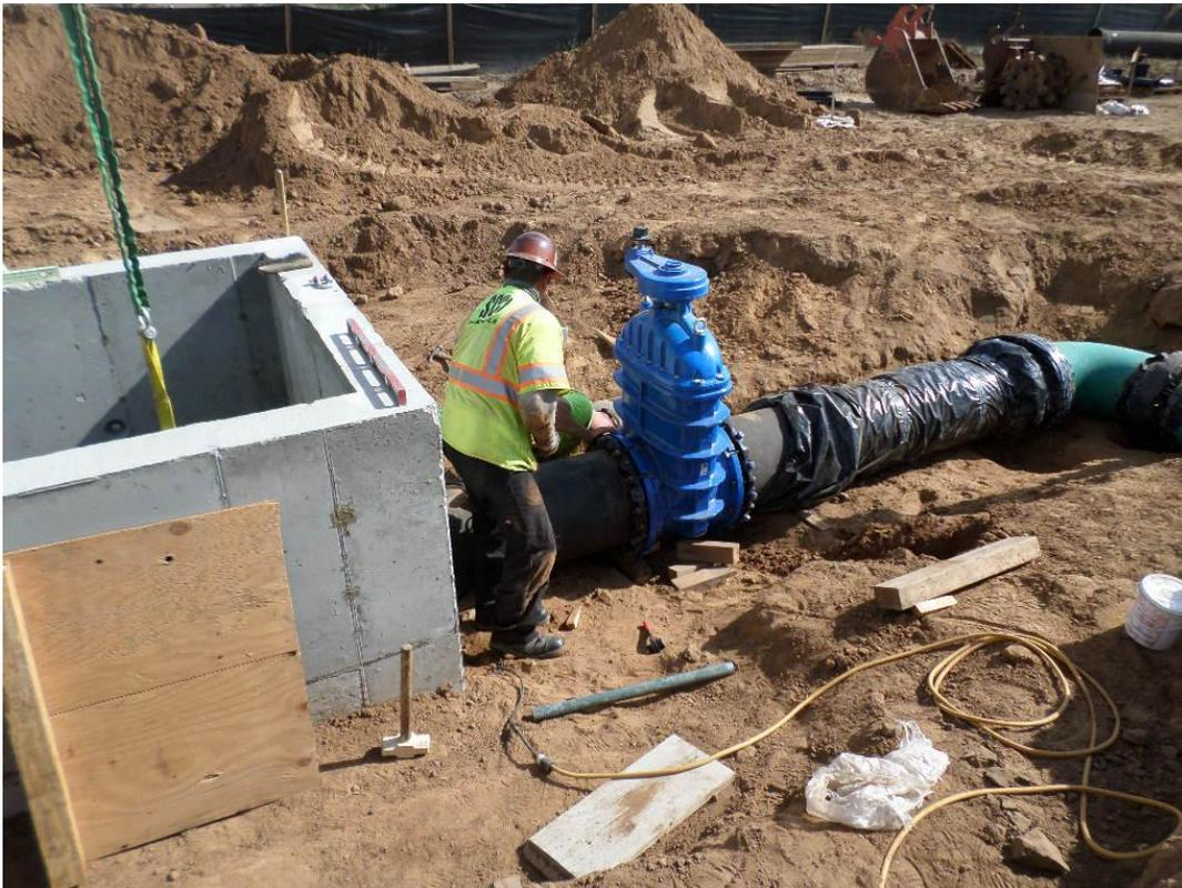
Spieß installing discharge piping and valve to metering vault.
