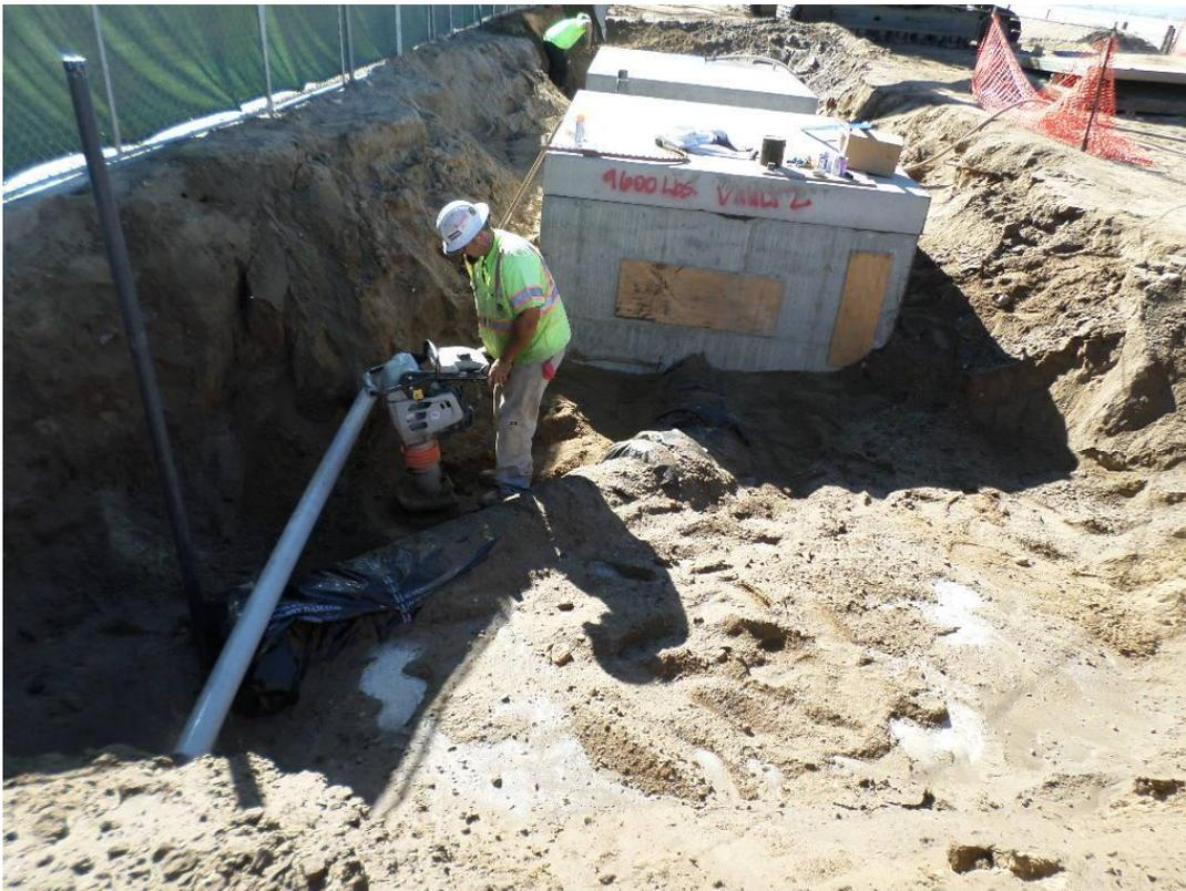
Piping to and from vaults installed and Spieß backfilling and compacting around piping and 4-inch Verizon line.
