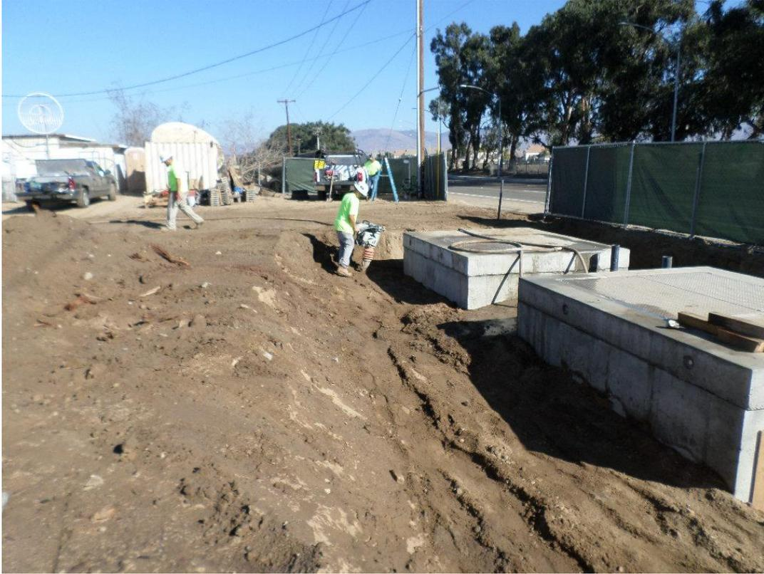
Spiess completing backfill and compaction around vaults.
