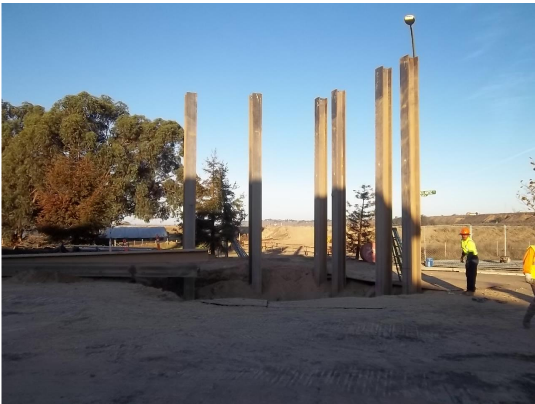
D-KAL removing the I beam piles from the receiving pit shoring.
