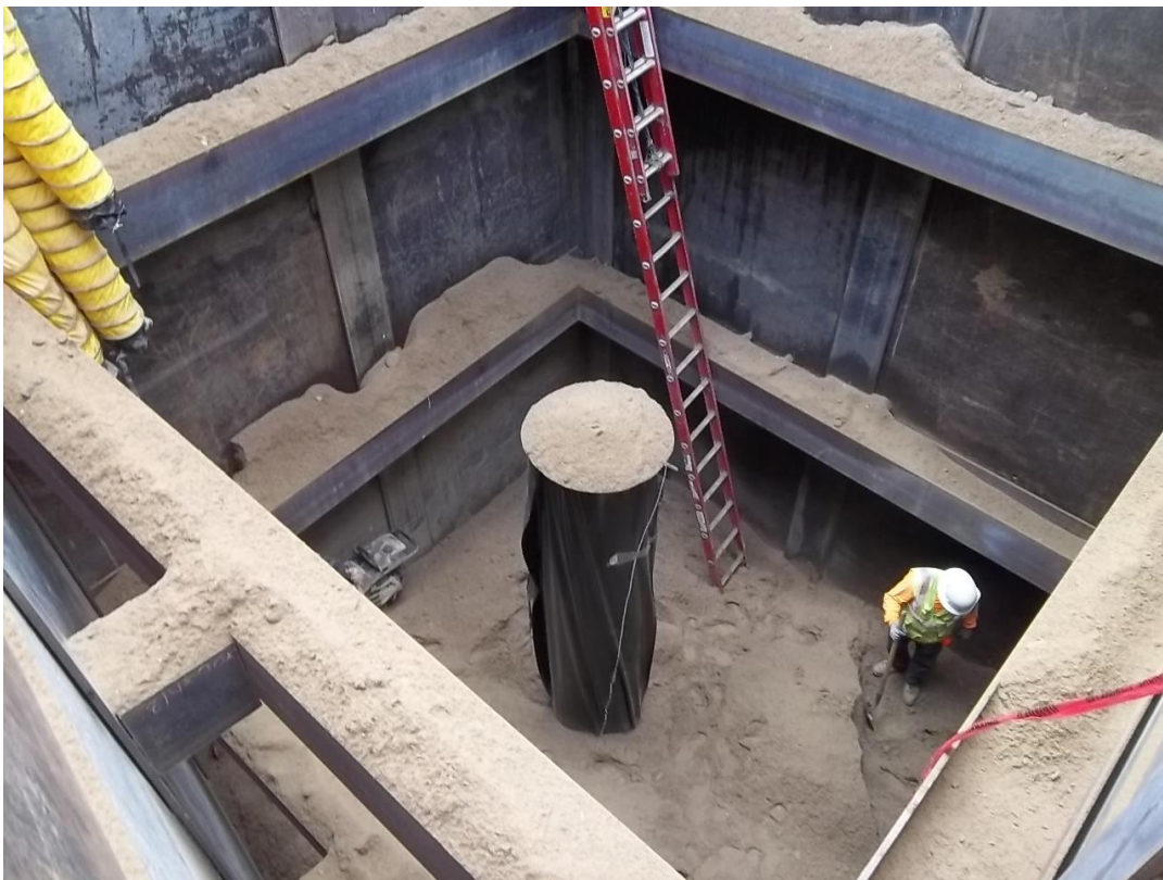
D-KAL backfilling around vertical pipe inside receiving pit.
