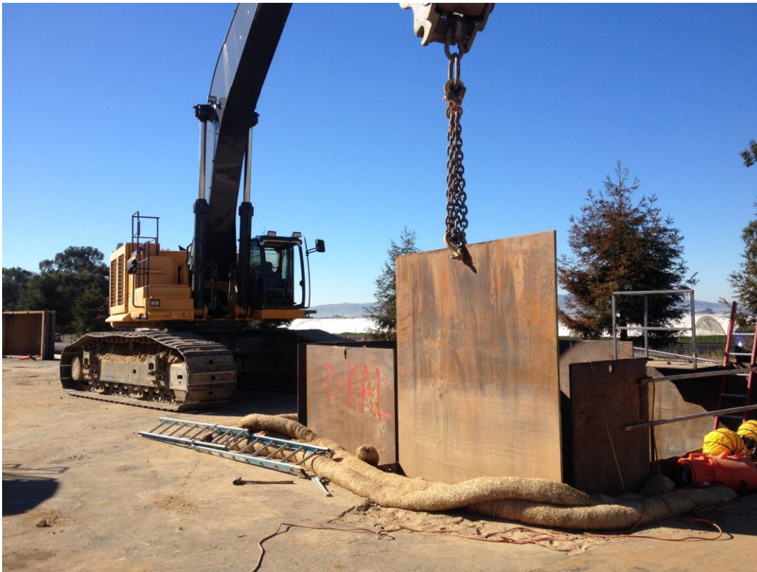
D-KAL pulling shoring plates out of receiving pit as they backfill.
