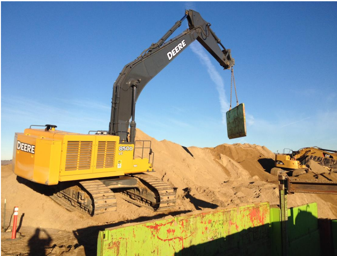
D-KAL disassembling the bore and jack pit.
