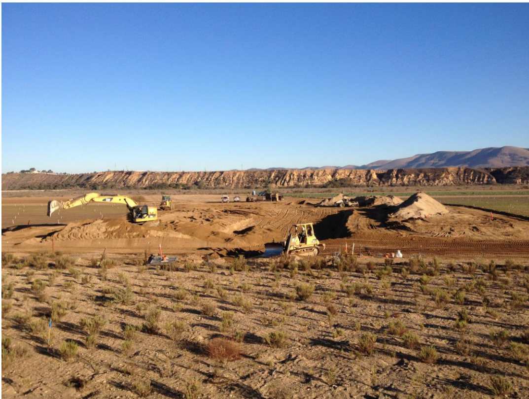
D-KAL completing backfill and agricultural topsoil restoration in the river area.
