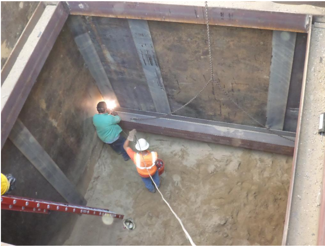
D-KAL welding whalers in final horizontal supports for the receiving pit.
