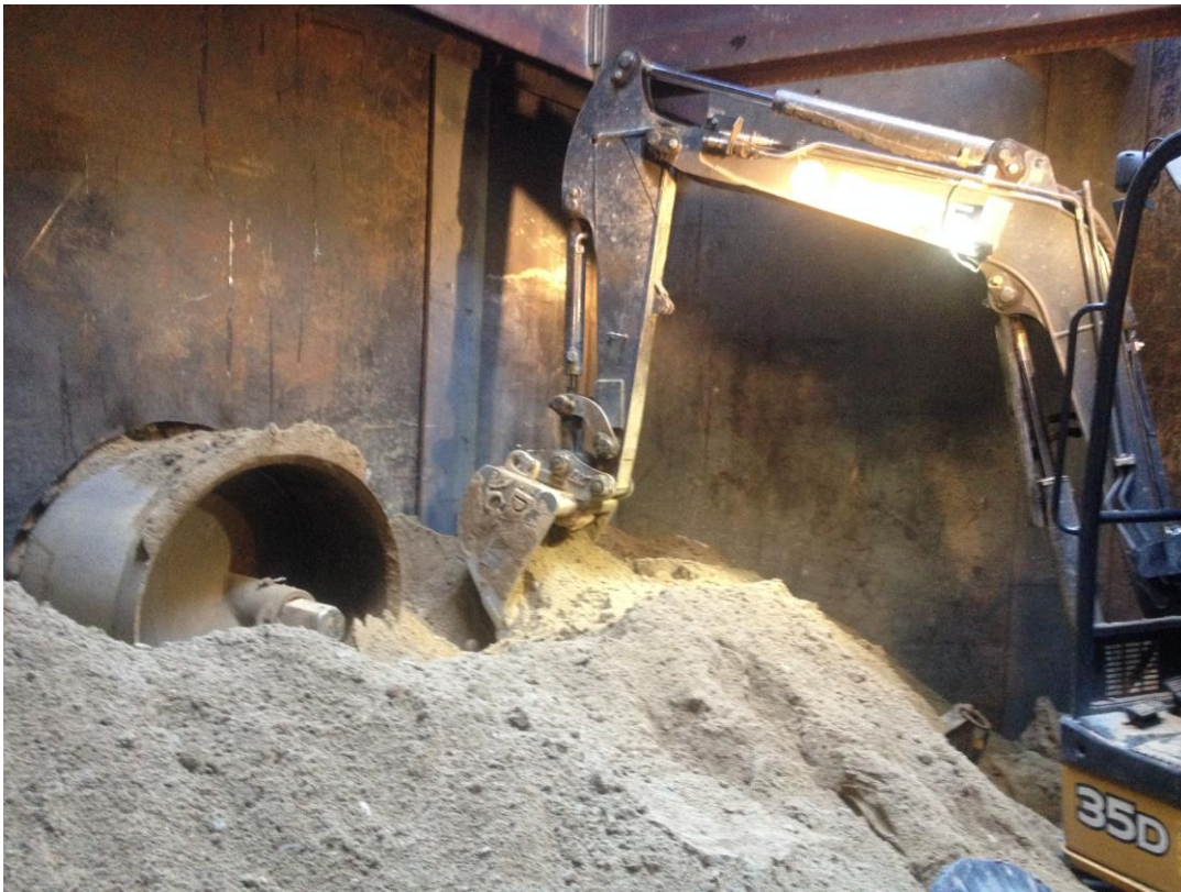
Casing received after bore and jack under the levee.
