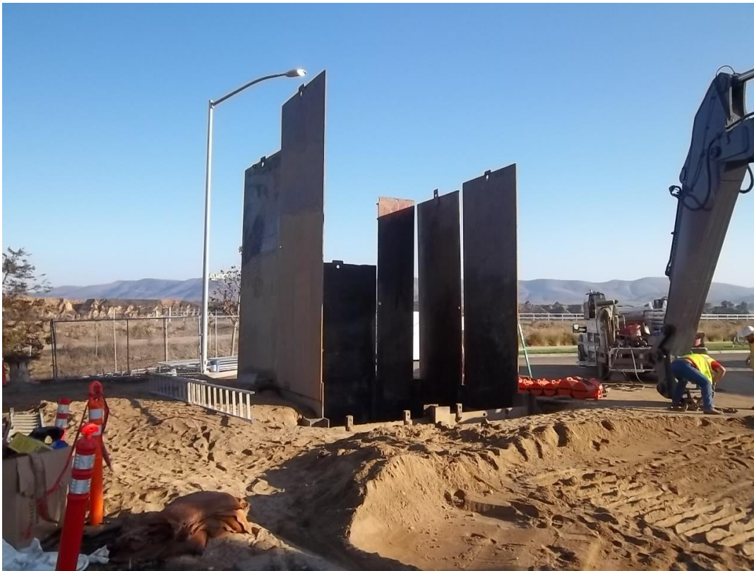
D-KAL continuing the backfill receiving pit and remove the shoring plates.
