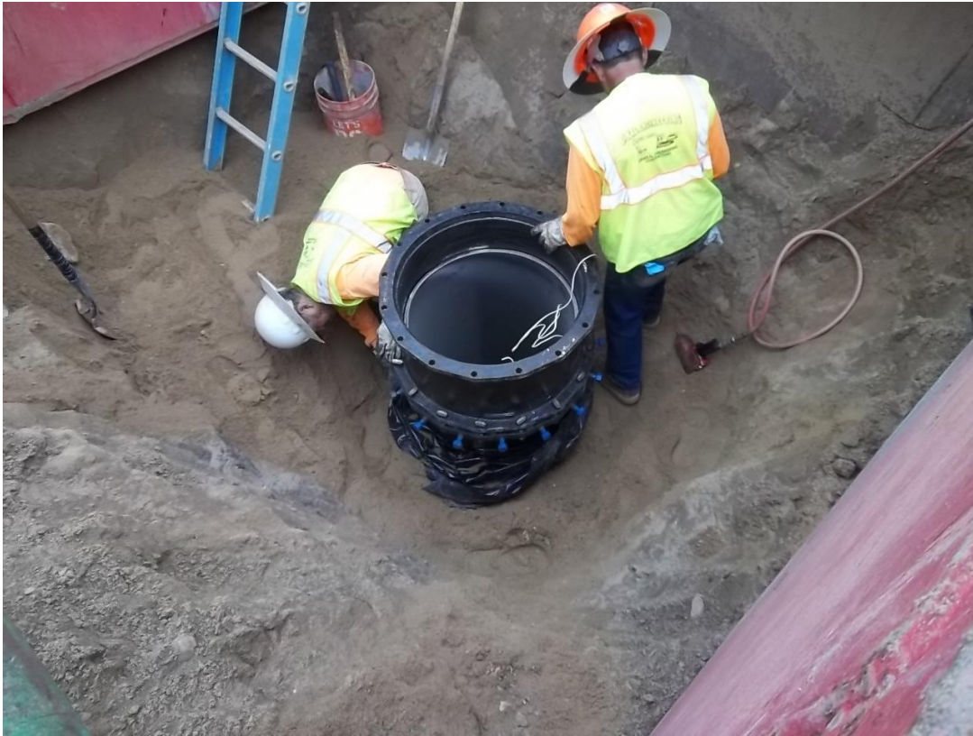
D-KAL installing the sleeve with megalugs.
