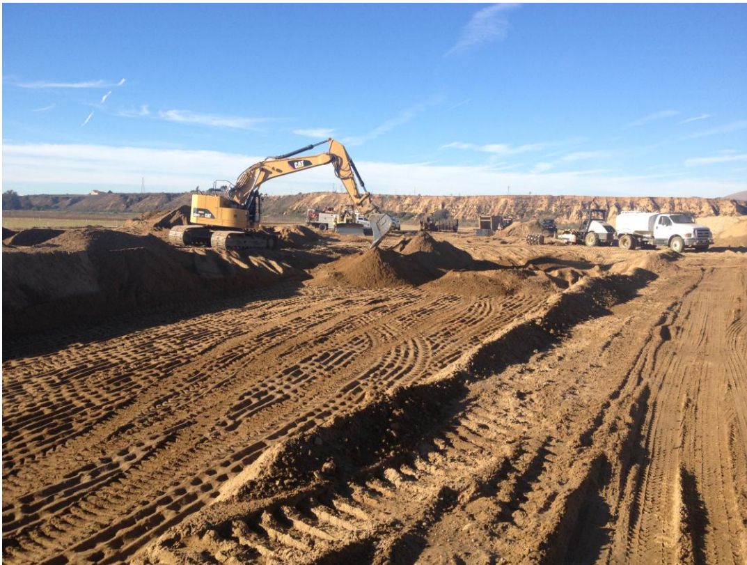
D-KAL backfilling and compacting over final trench segment in river area.
