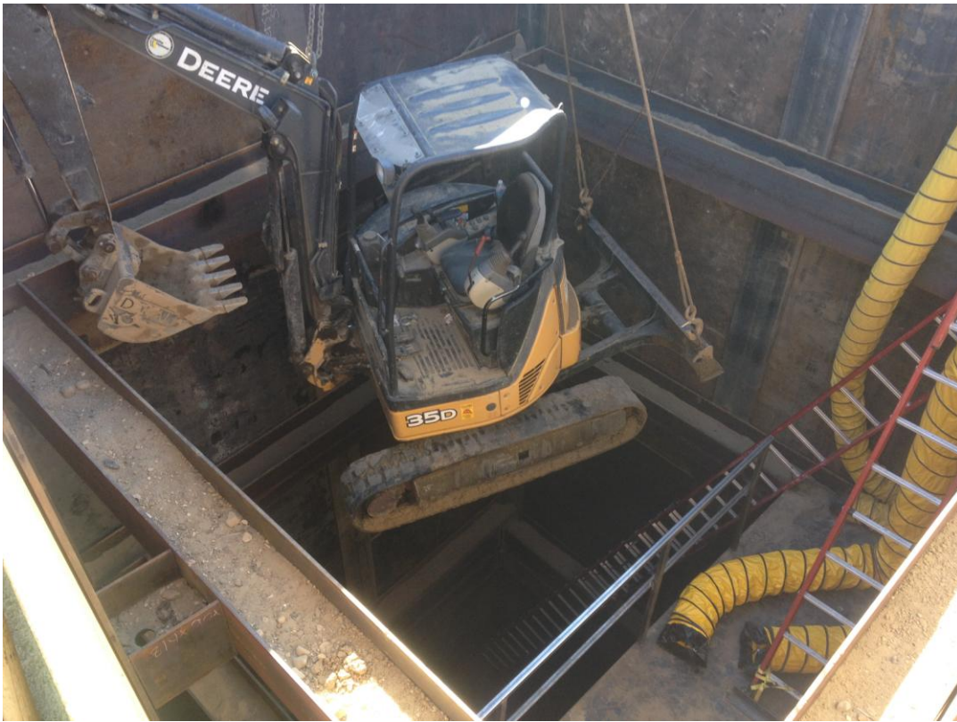
Removing mini excavator from the receiving pit.
