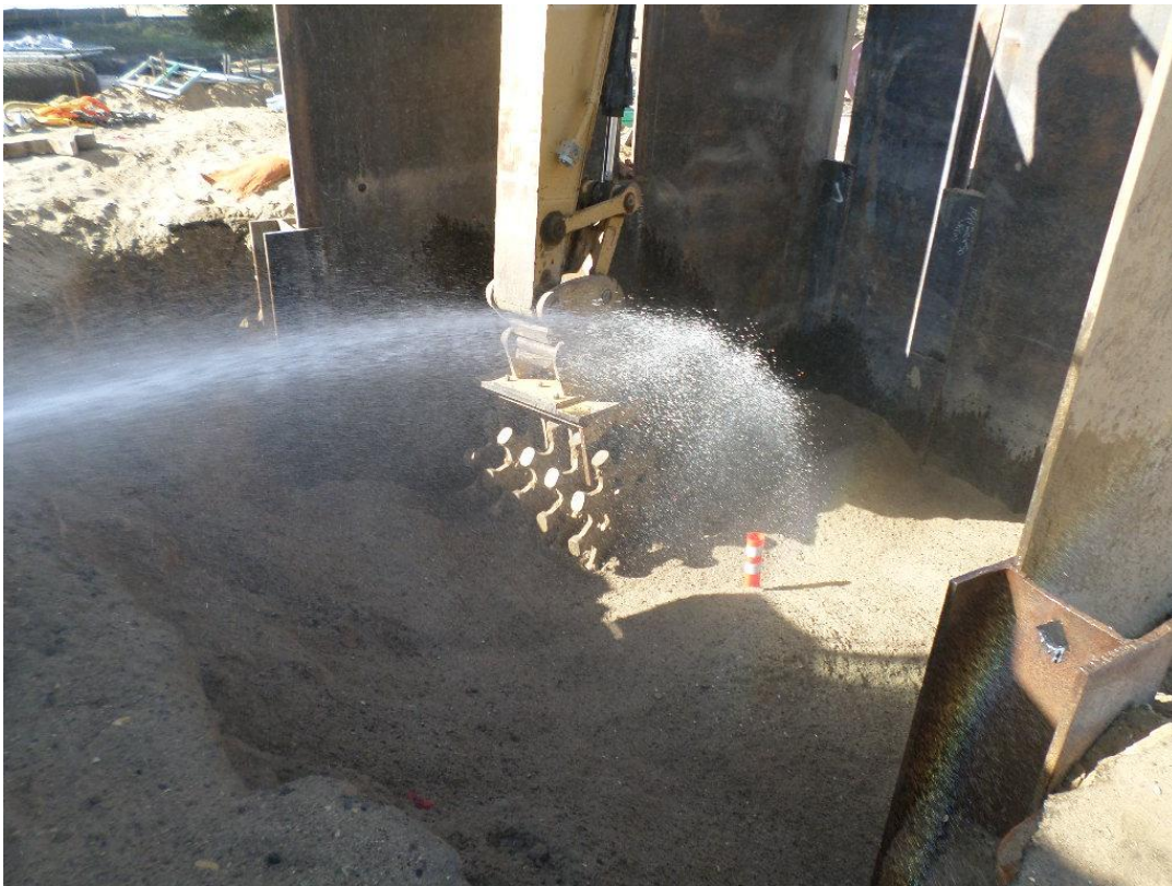
Compacting top of receiving pit excavation with sheep's foot roller.
