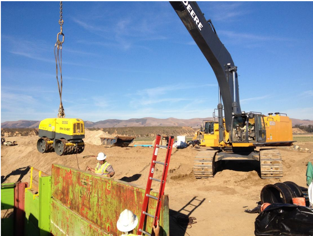
D-KAL lowering remote control compactor into the bore and jack pit.
