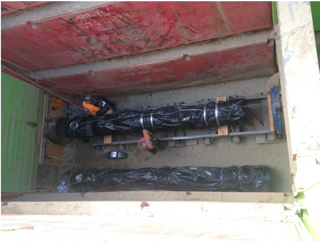
Pacific Boring pushing pipe into casing under the levee.
