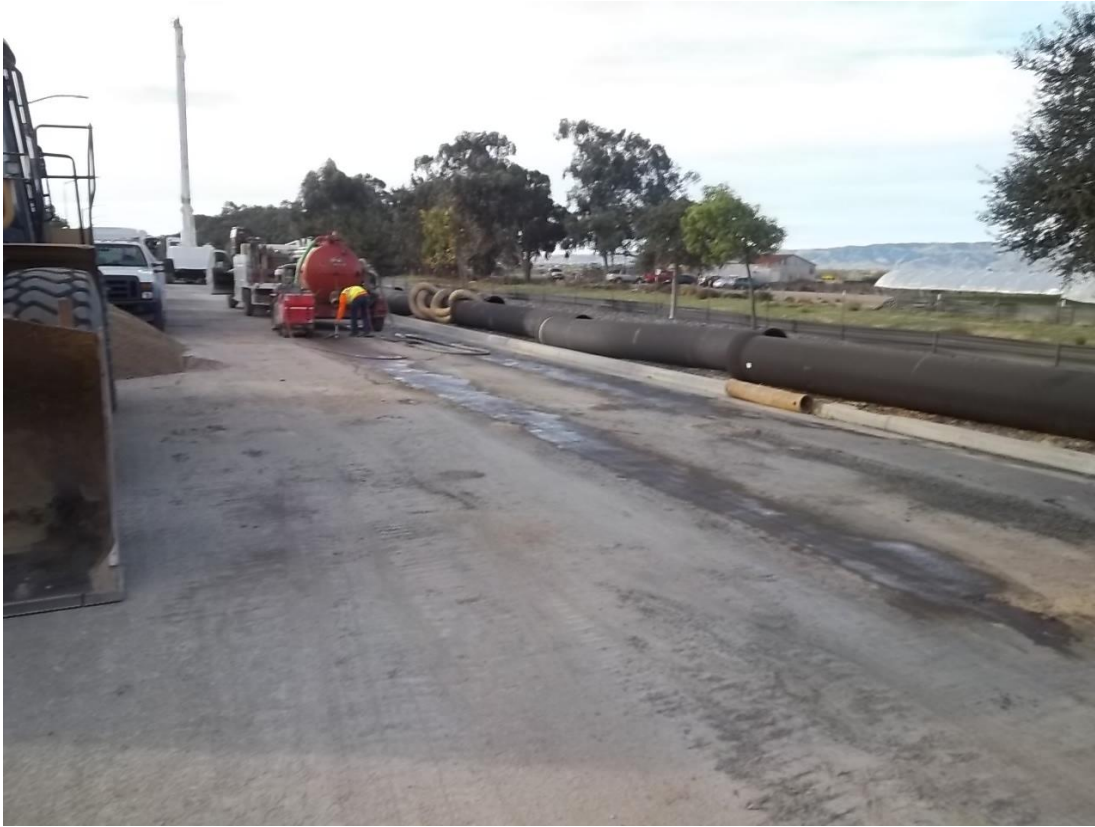
D-KAL sawcutting pavement for the trench in Blosser Road.
