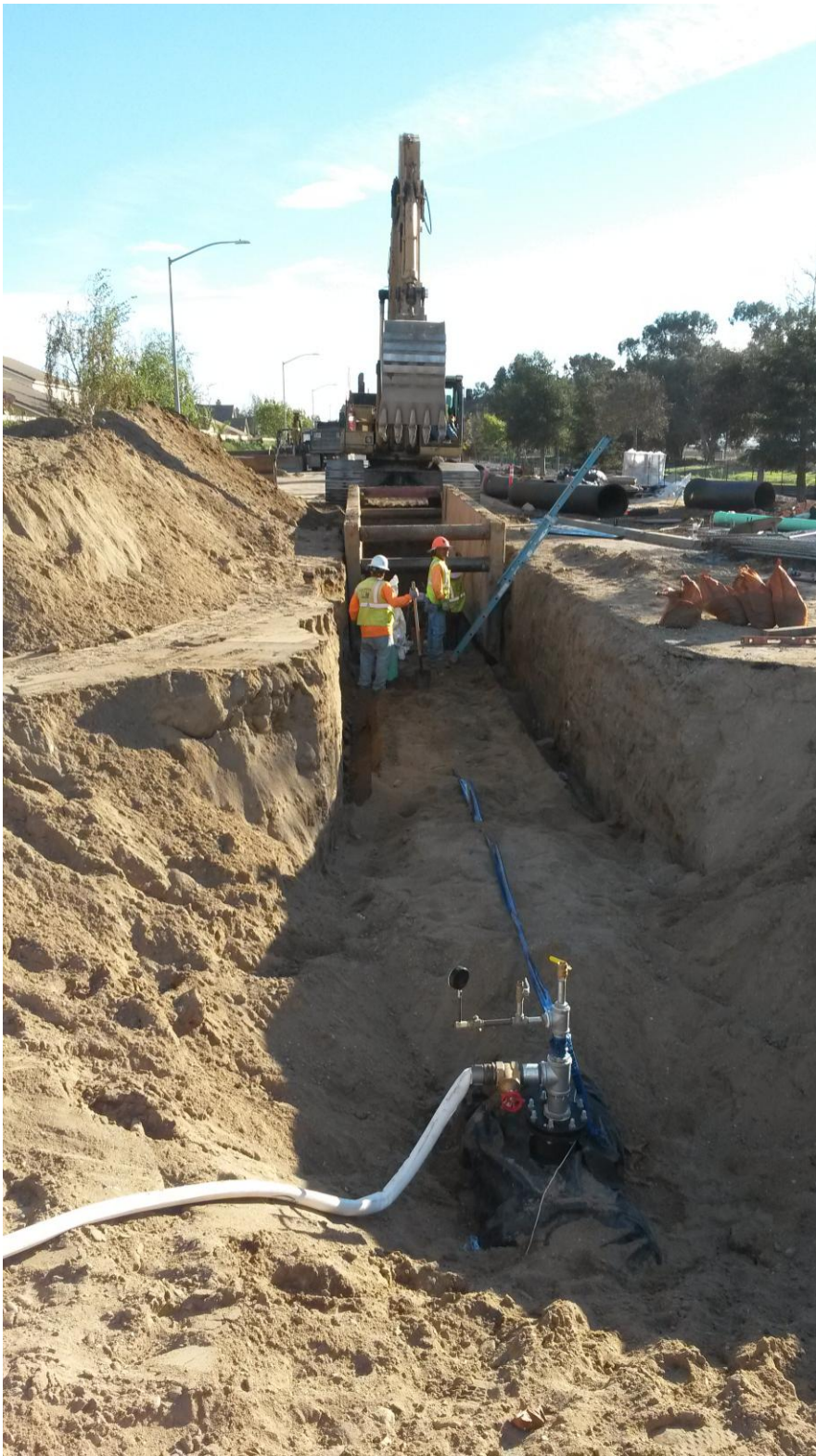
Installing pipe from the 90 degree elbow south in Blosser Road.
