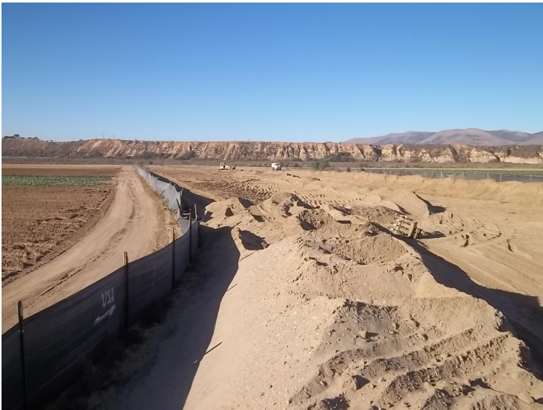
D-KAL removing silt fence and restoring the agricultural top soil.
