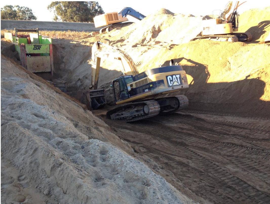
D-KAL removing trench shields and backfilling 24-inch DIP after final connection.
