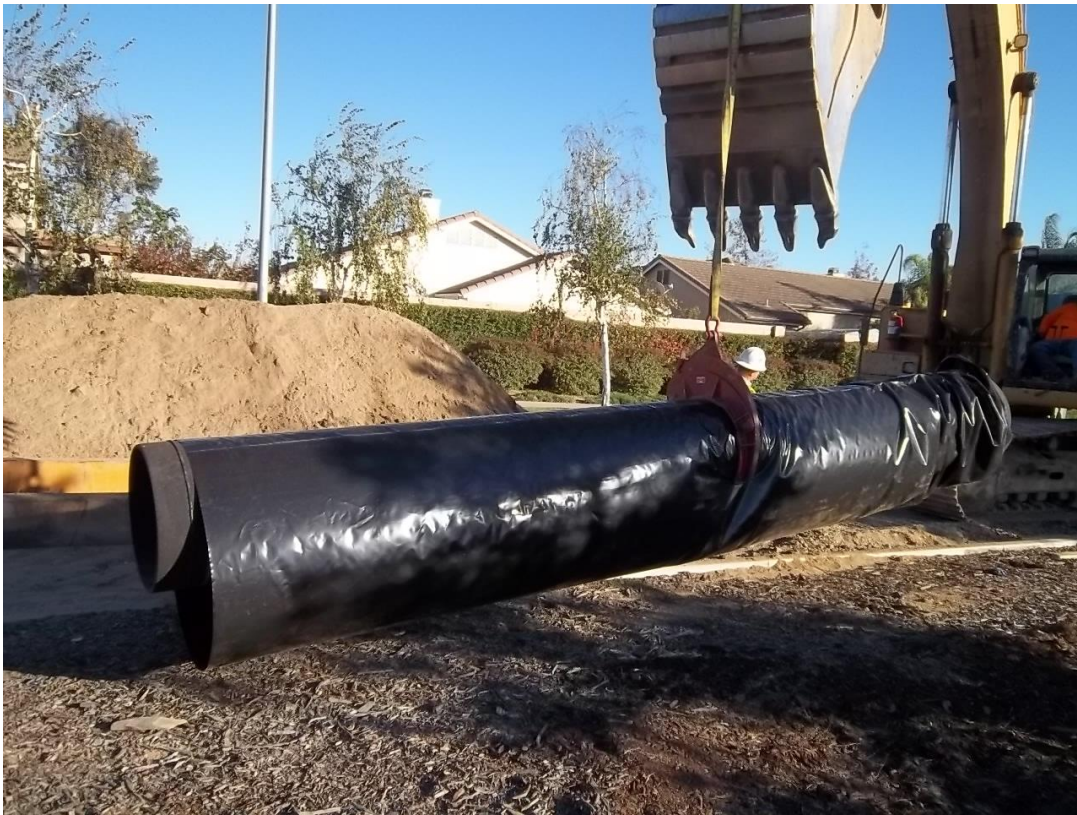
24-inch DIP wrapped in plastic and ready for installation.
