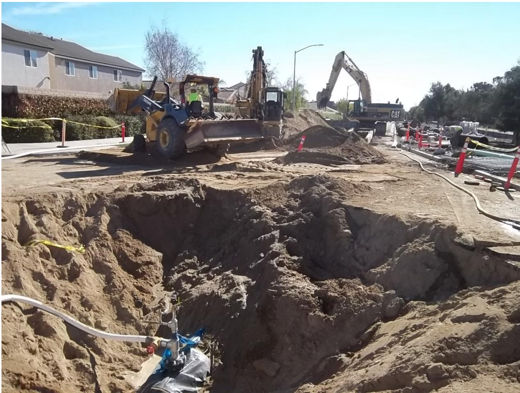
D-KAL backfilling in Blosser Road.
