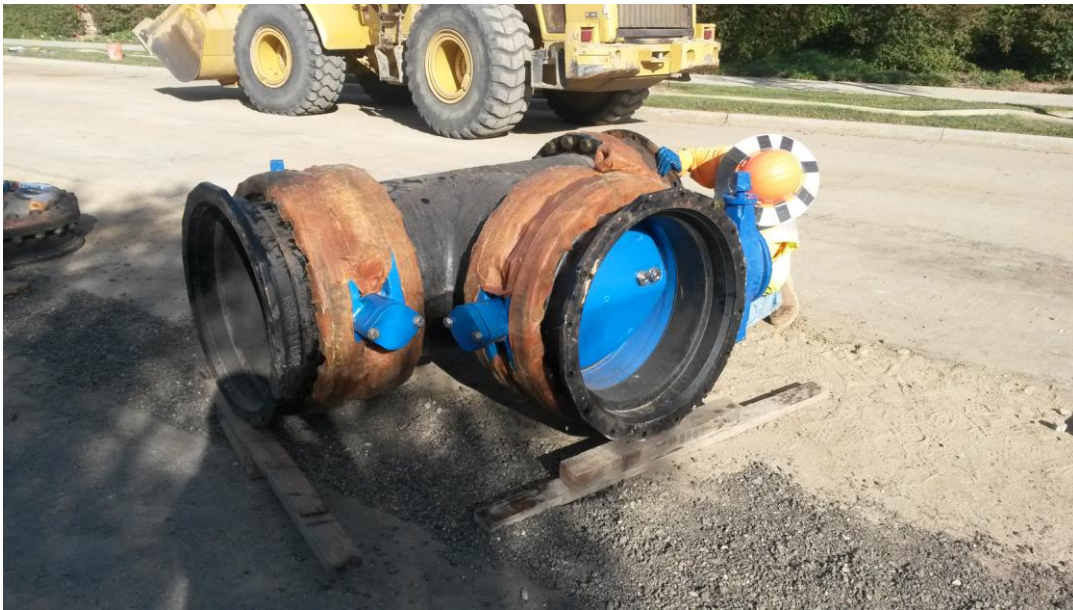
D-KAL applying wax tape to the 24-inch tee.
