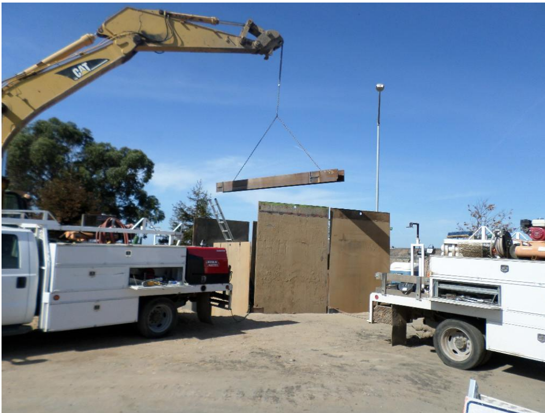
D-KAL removing beams from horizontal shoring inside the receiving pit.
