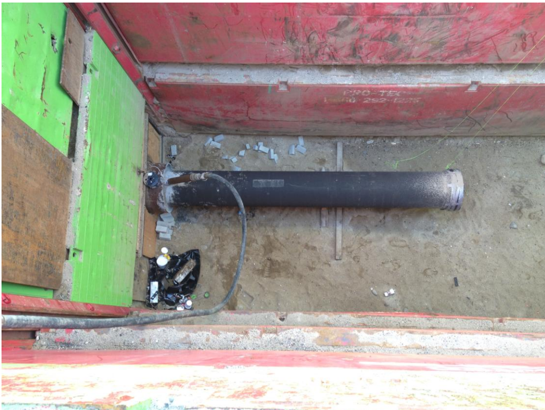
Grouting the casing.
