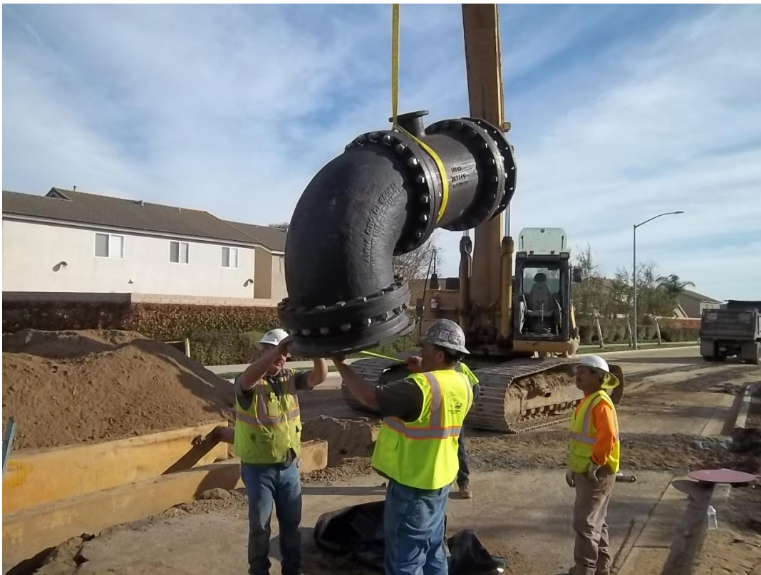
D-KAL preparing to install the 90 degree bend.
