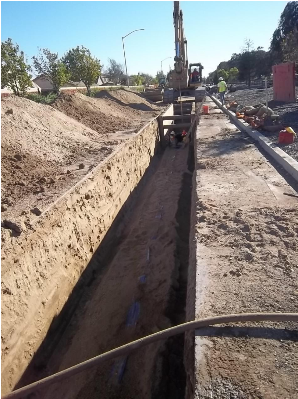
Marking tape placed and D-KAL backfilling pipe in Blosser Road.
