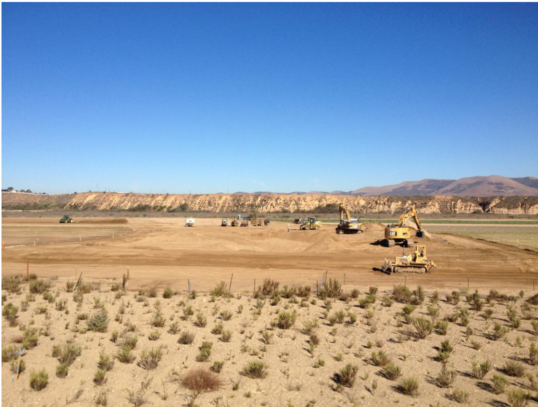
Restoring agricultural topsoil and farm access road to grade.
