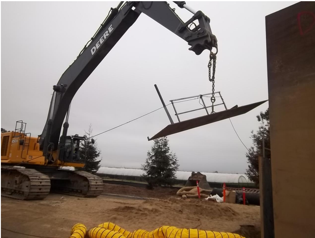
Removing scaffolding from receiving pit during backfill.
