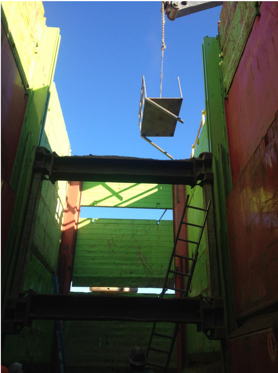
D-KAL removing scaffolding from the bore and jack pit.
