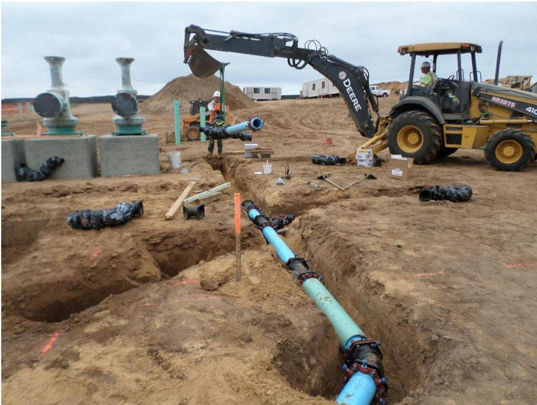
Spieß installing drain pipe for underneath the pump station slab.
