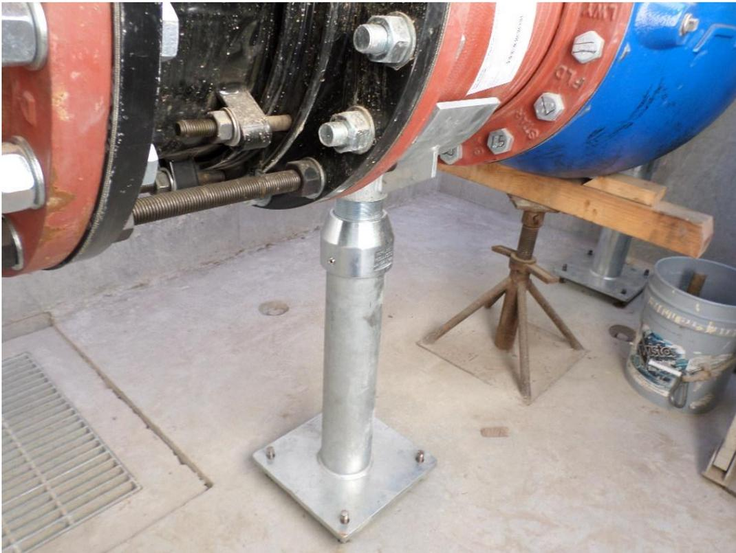
Pipe supports being installed inside the metering vaults.
