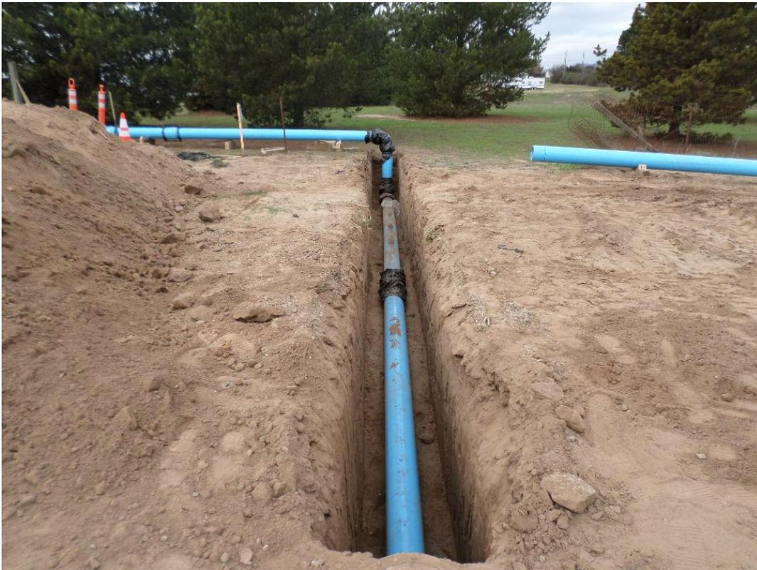
Spiess installing the 8-inch PVC bypass line.
