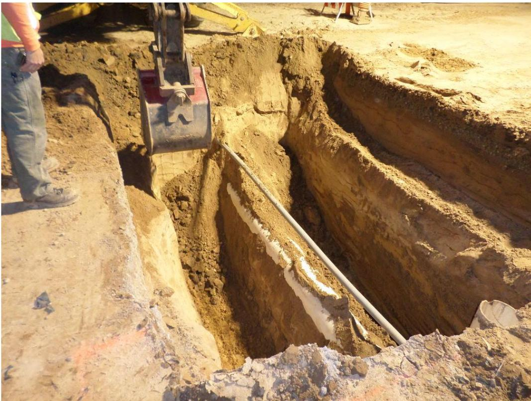
Spieß exposing the 12-inch PVC waterline for installing the temporary bypass.
