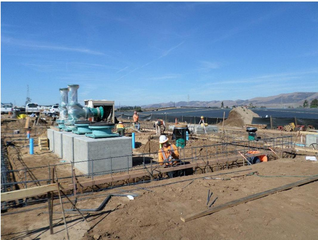
Vista Steel installing reinforcing for the pump station footing and stem wall.
