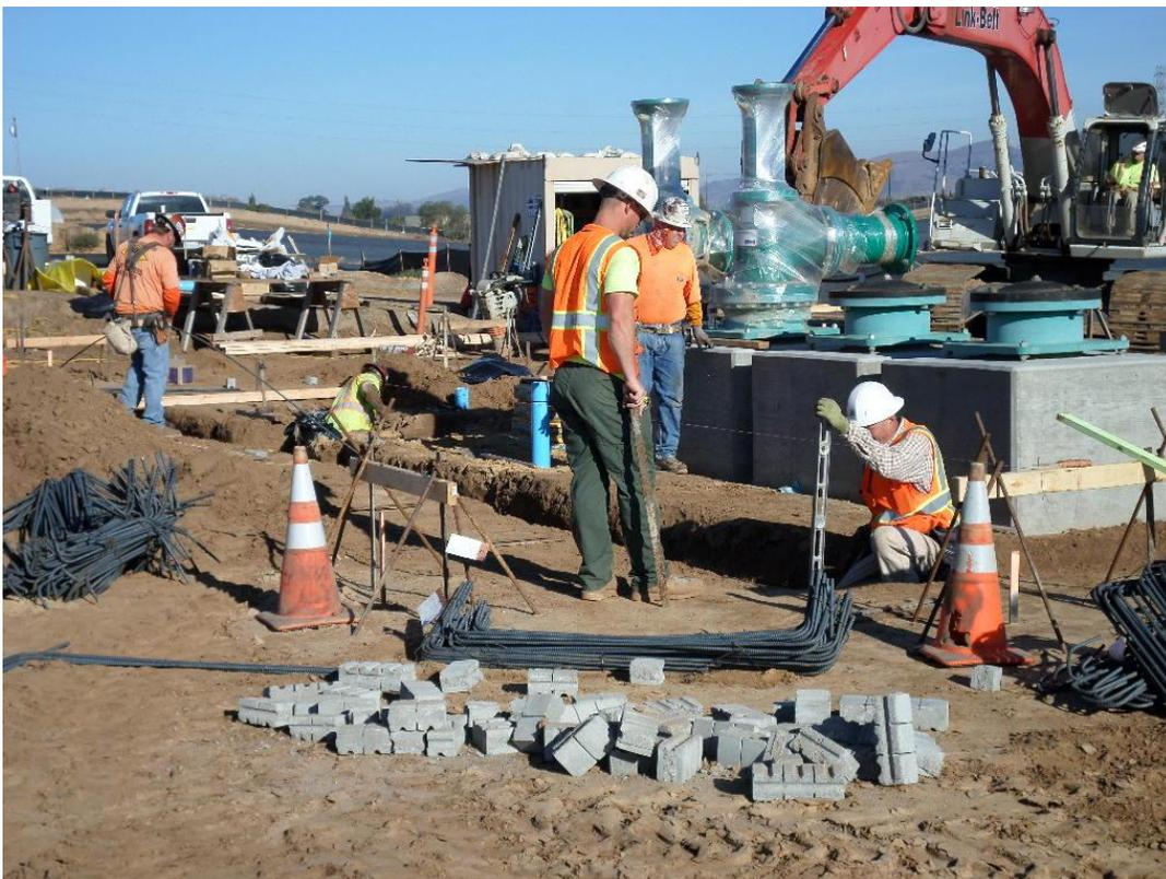
Spieß laying out and excavating the pump station footing.
