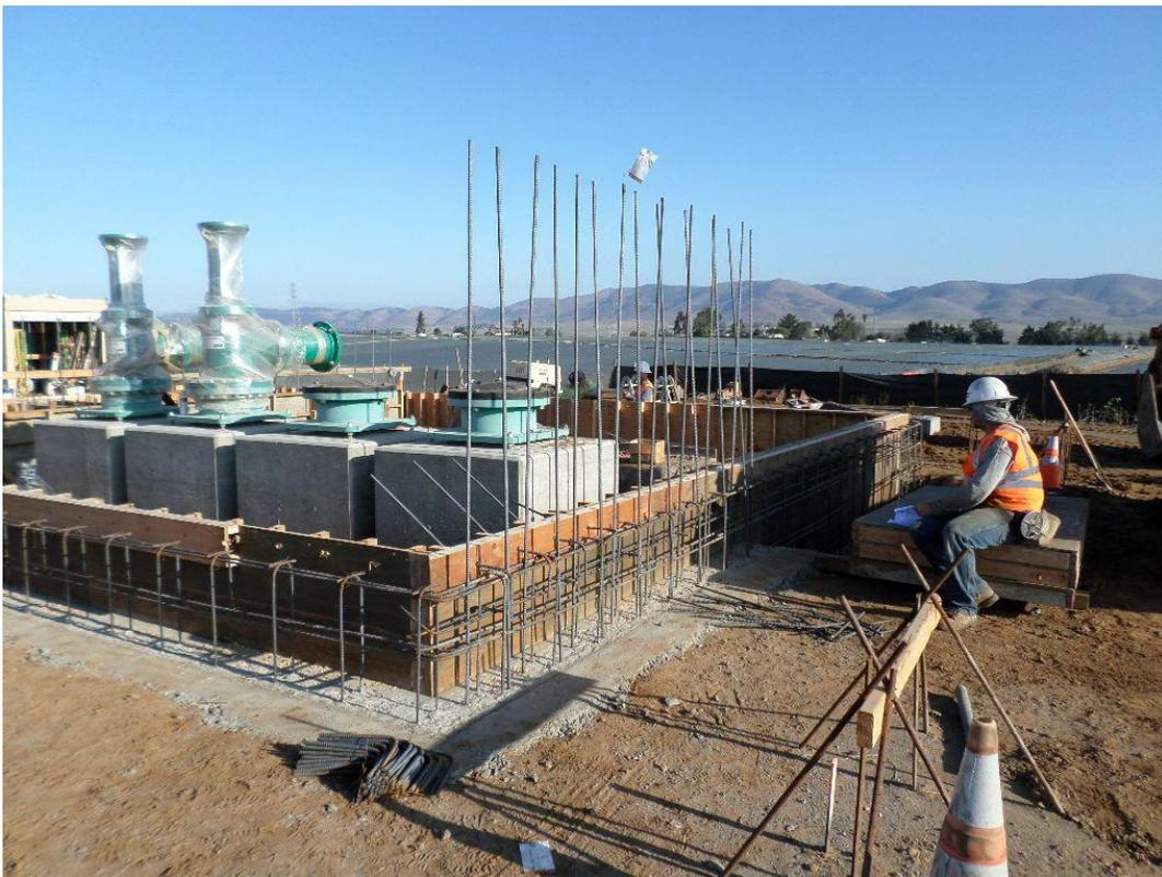
Vista Steel installing more reinforcing at the stem walls of the pump station.
