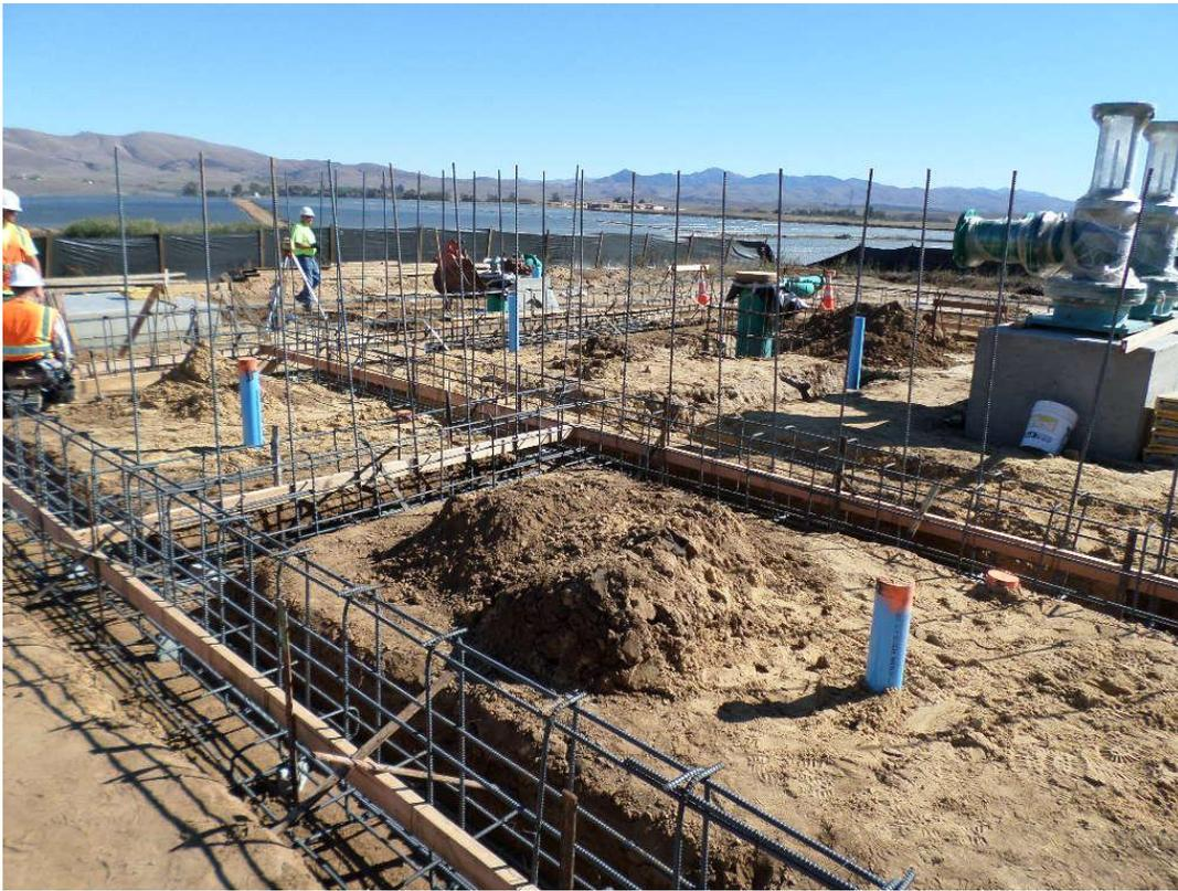
Installing forms for pump station foundation.
