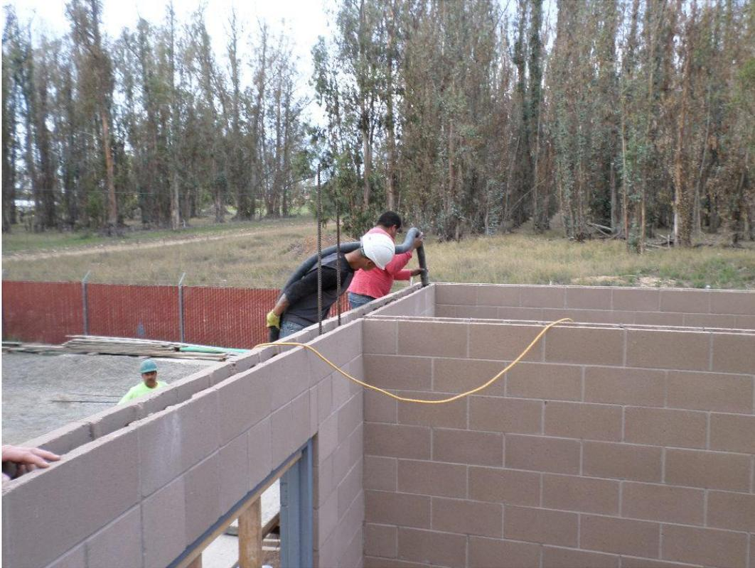
Boydston Masonry grouting block walls at Sundale.
