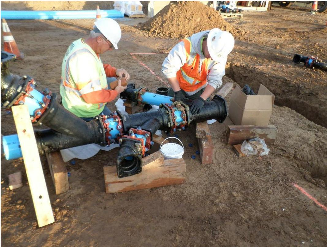
Applying wax tape to drain piping.
