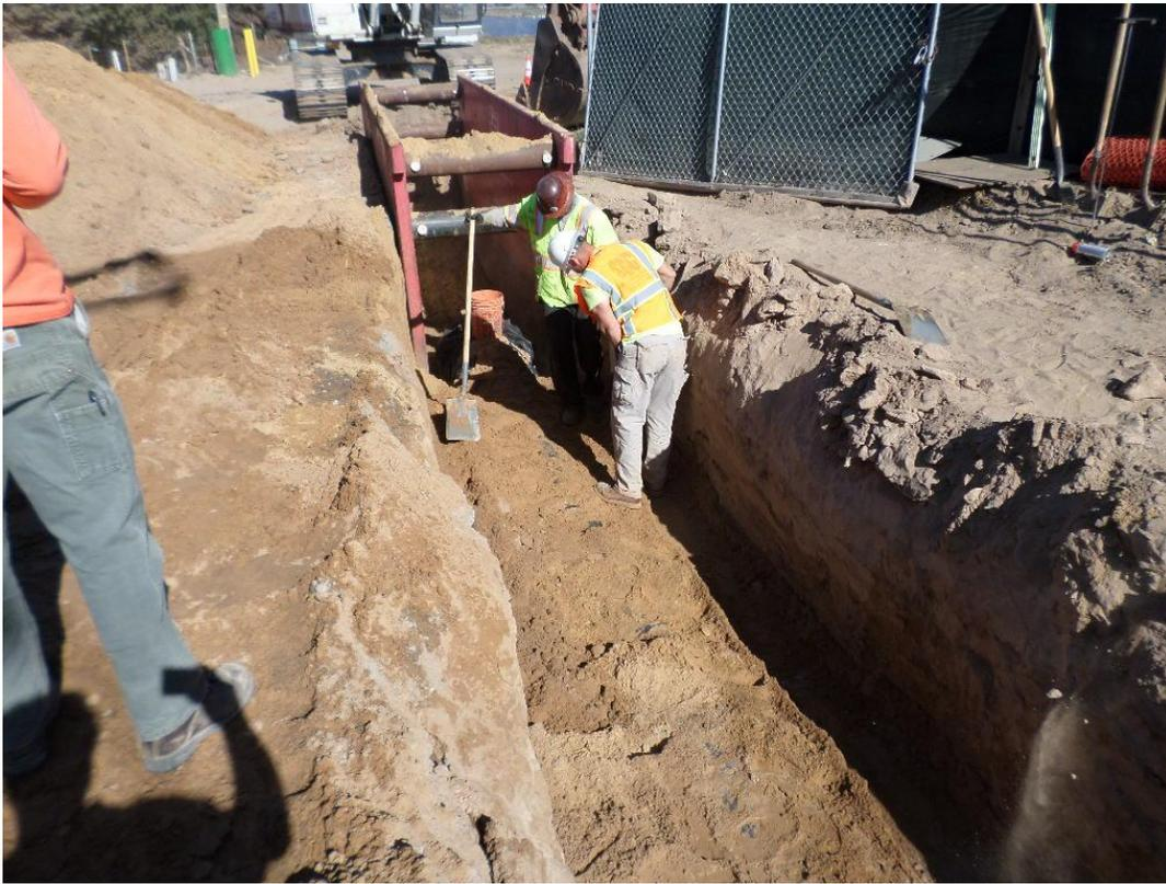
Spieß compacting last section of 24-inch DIP installed in the access road.
