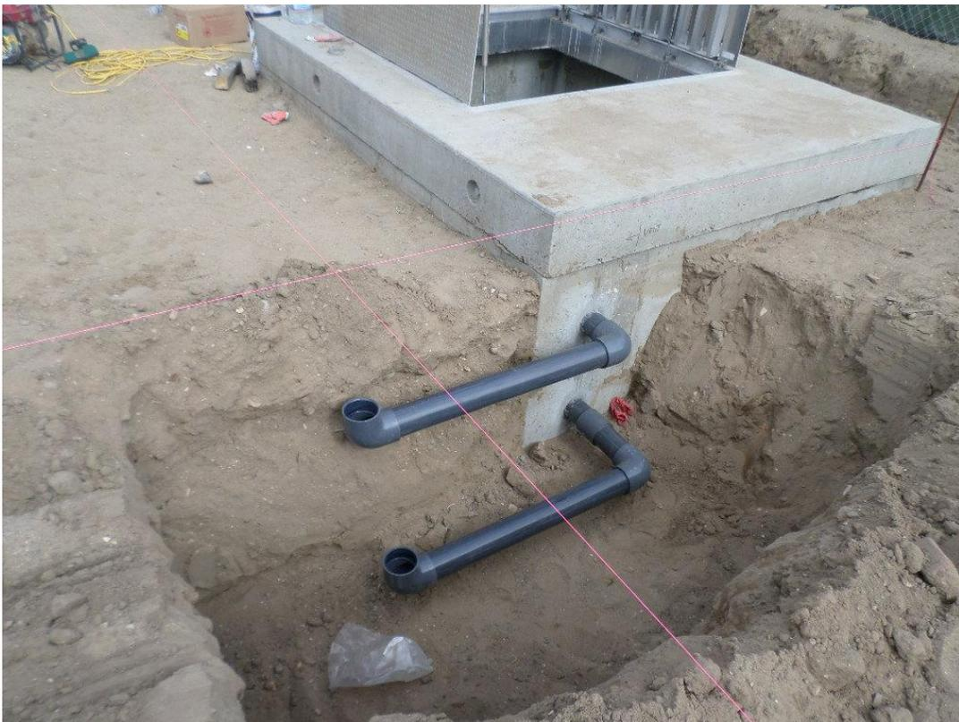
Vent pipes installed at the metering vaults.
