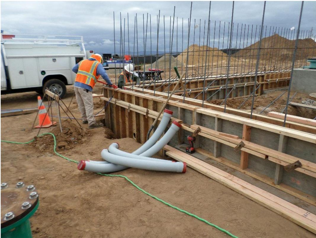
Spieß forming stem wall and St. Dennis Electric installing conduit underneath the future pump station slab.
