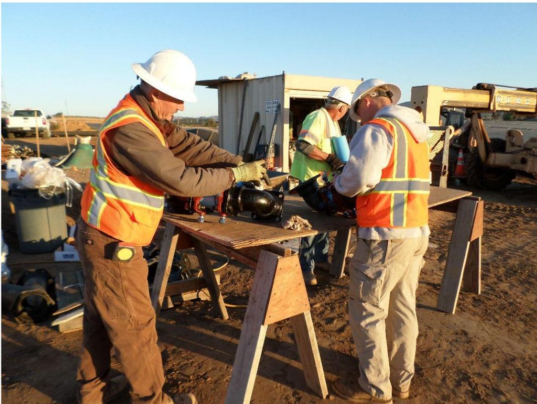
Spiess assembling drain pipe for under pump station slab.
