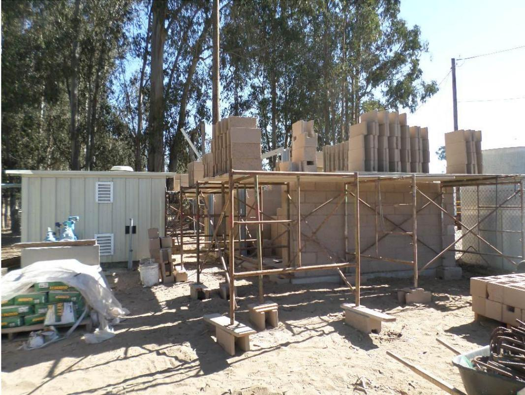
Boydston Masonry installing scaffolding and staging block for next wall course.
