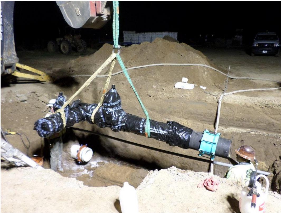
Spiess installing second section of bypass on the existing 12-inch PVC waterline.
