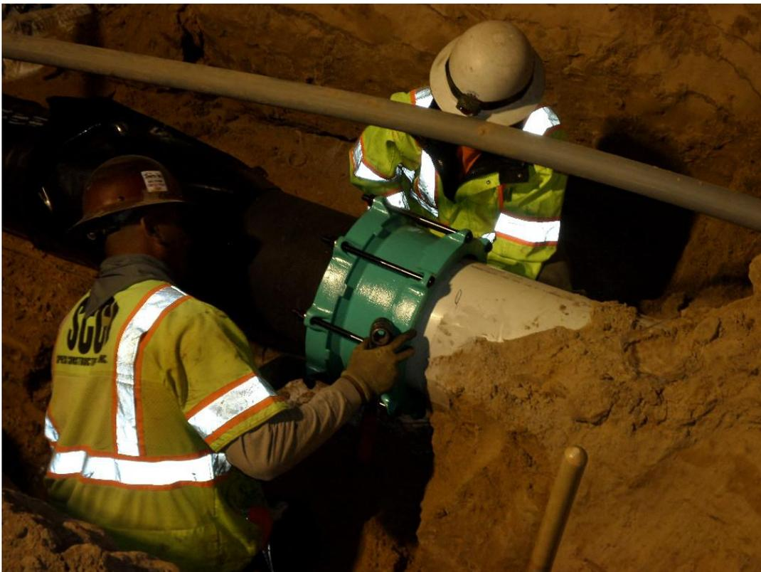
Spiess installing 12-inch transition coupler to connect to existing PVC waterline.
