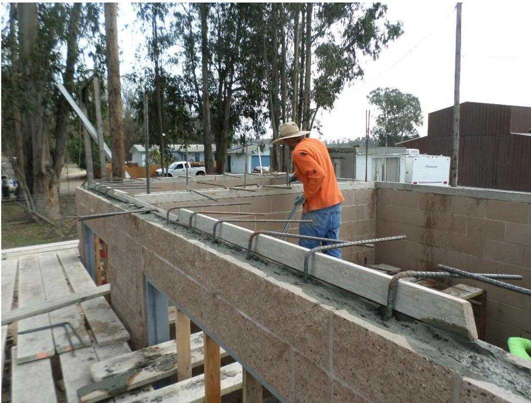
Boydston grouting and installing rebar to connect future roof to walls.
