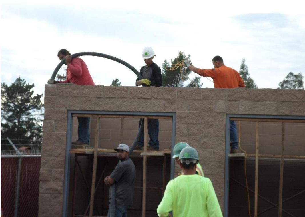
Boydston Masonry grouting block walls for the chemical building.
