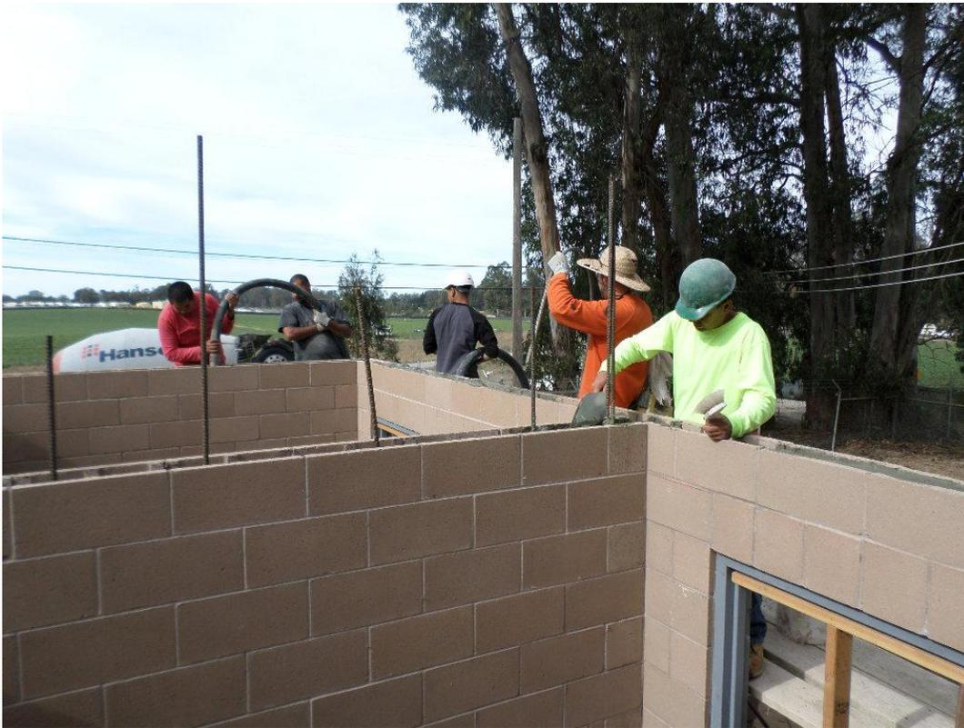
Boydston Masonry grouting walls of chemical building.
