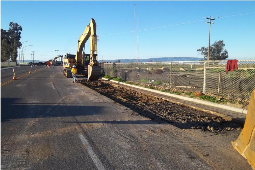
D-KAL excavating to install 36-inch casing under 48-inch and 72-inch storm drain pipes which cross Blosser Road.
