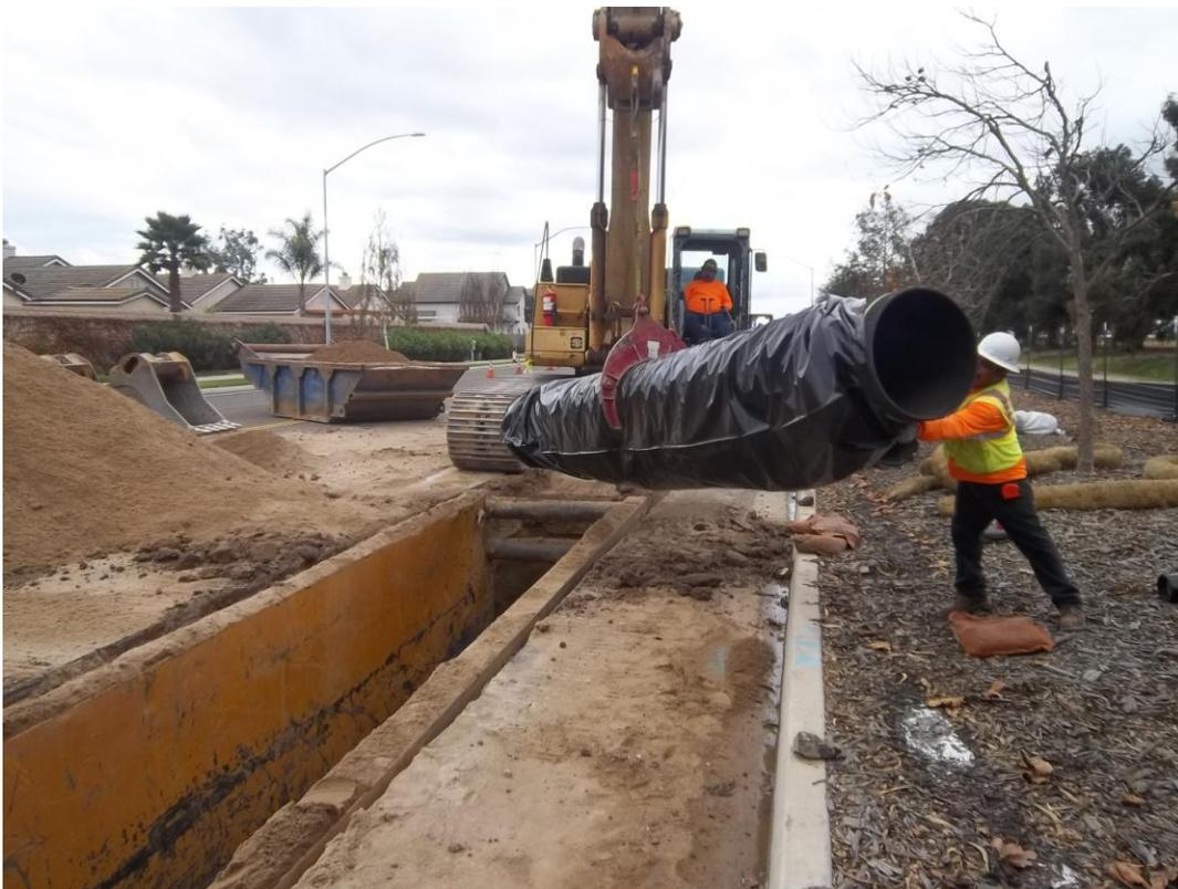
D-KAL installing a section of 24-inch DIP.
