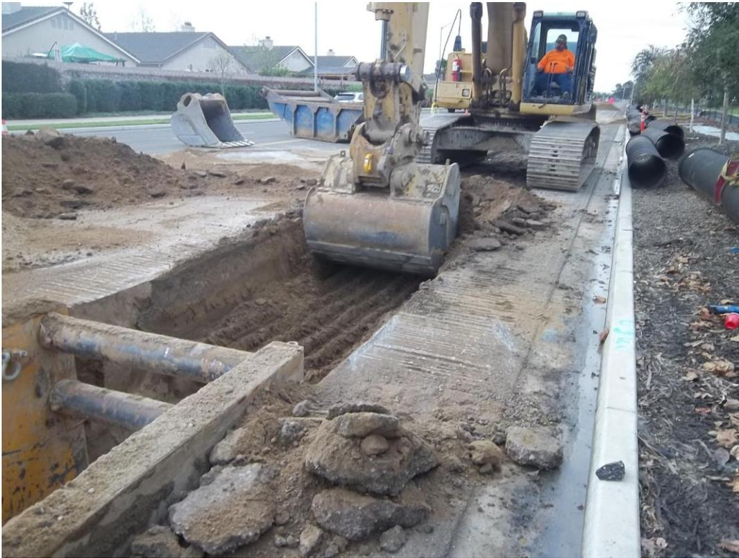
D-KAL removing existing AC and road base to excavate trench for 24-inch DIP.
