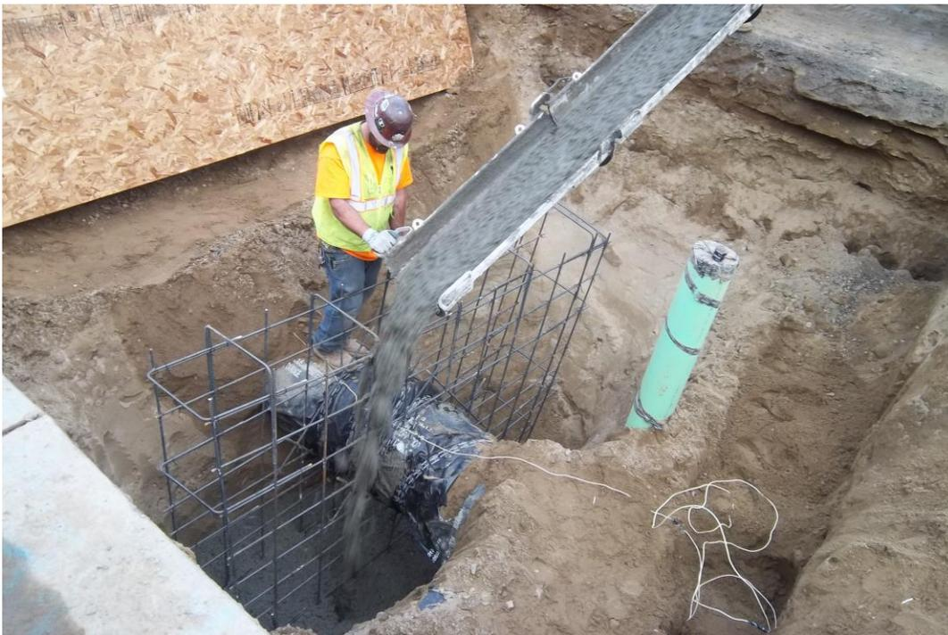
Pouring thrust collar for butterfly valve at Station 42+42.
