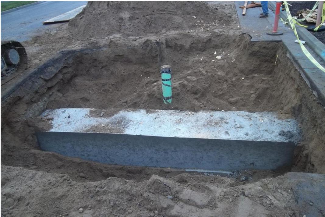
Top of thrust collar with forms removed prior to backfill.
