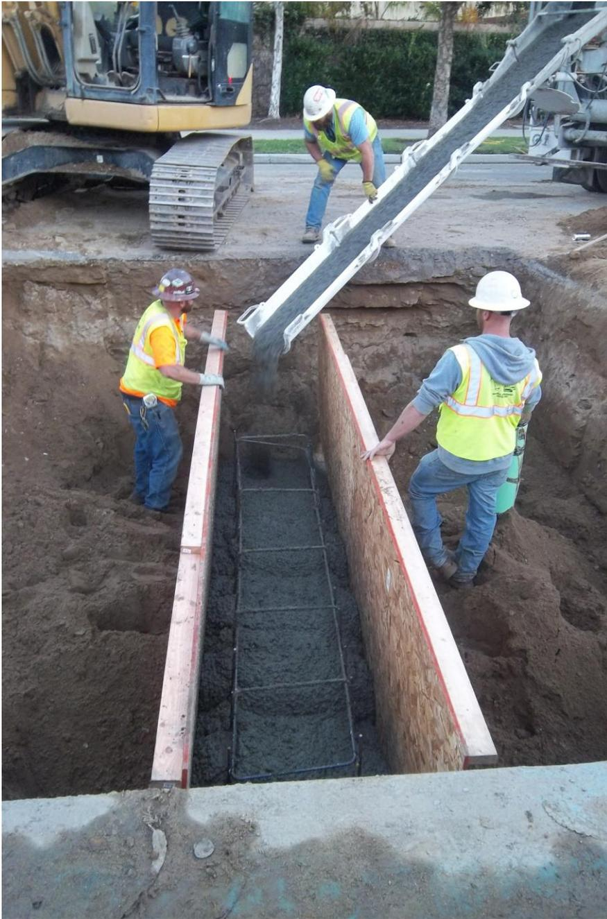
Top forms in place at thrust collar for concrete pour at Station 42+42.
