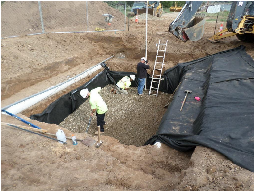
Spiess installing drain rock and fabric for underneath the PRV vault.
