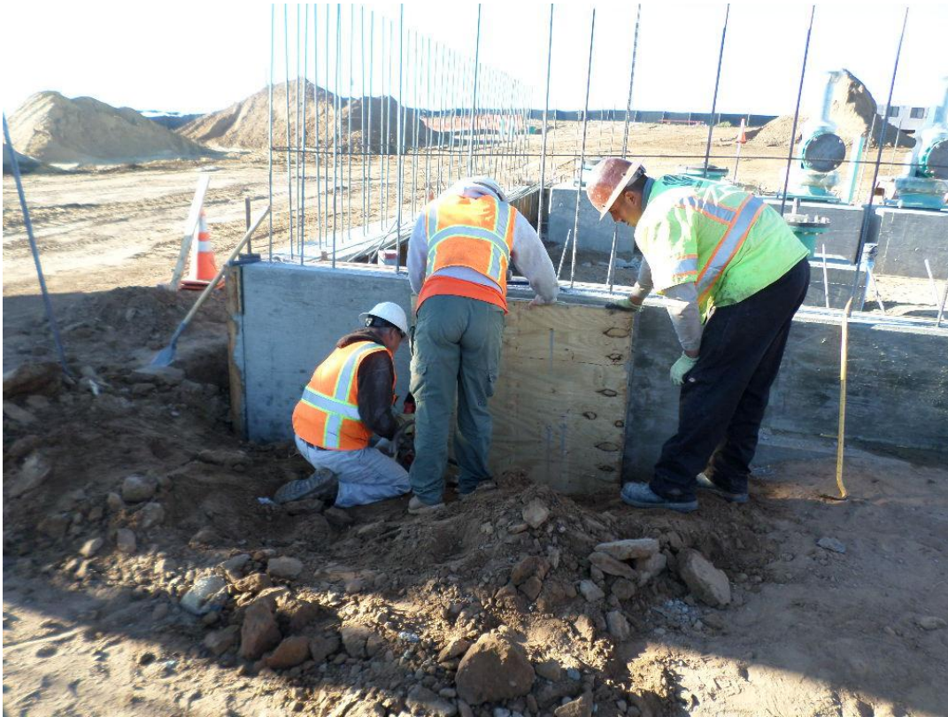
Spieess stripping forms from stem wall pour at the pump station.
