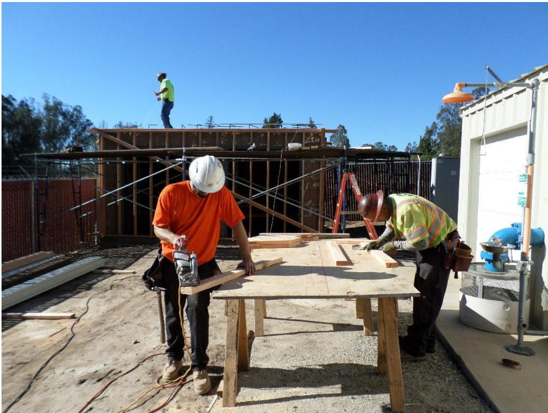
Spies forming falsework for concrete pour of the roof.
