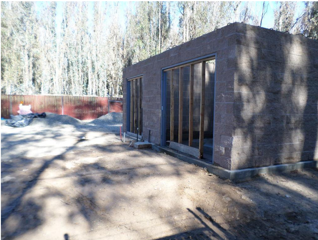
Sundale Well Site with the masonry complete.
