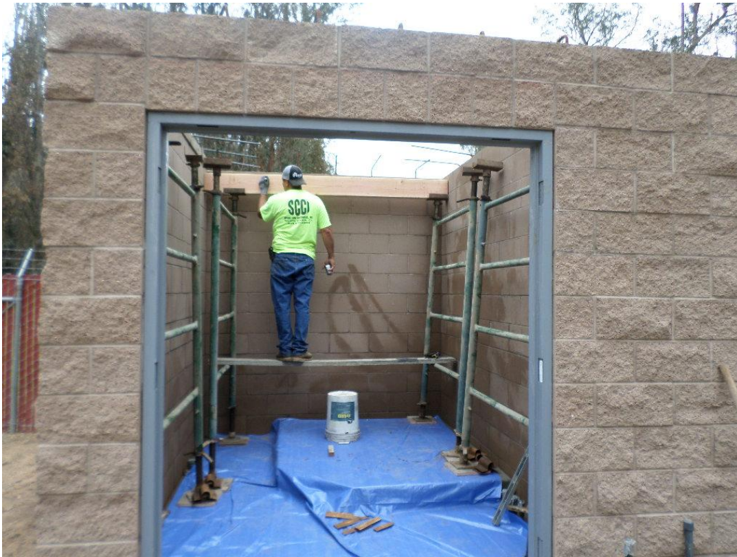
Spiess installing falsework for roof construction.
