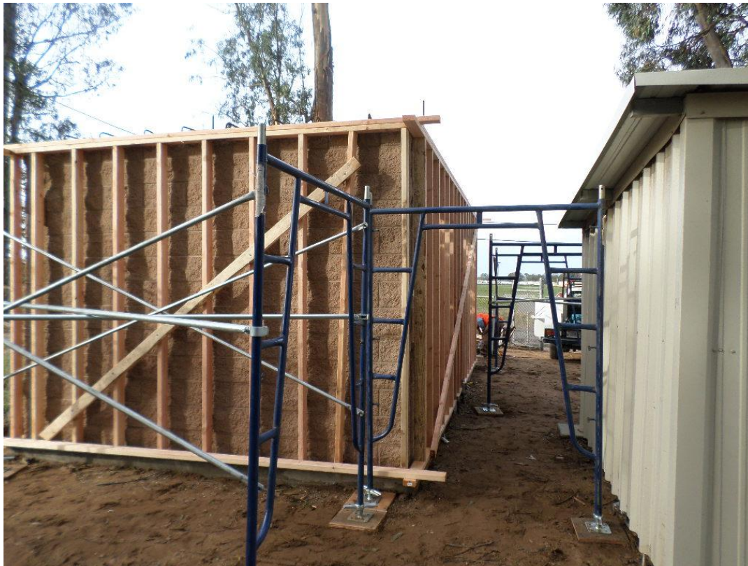
Exterior falsework, forms and scaffolding installed for roof pour.
