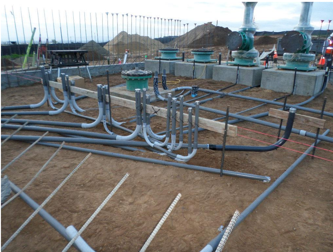
St. Dennis Electric installing underslab conduit.
