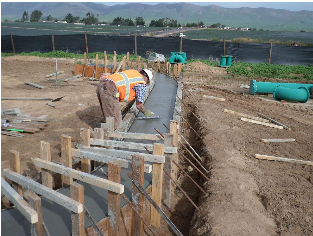
Spieß finishing the concrete spillway.
