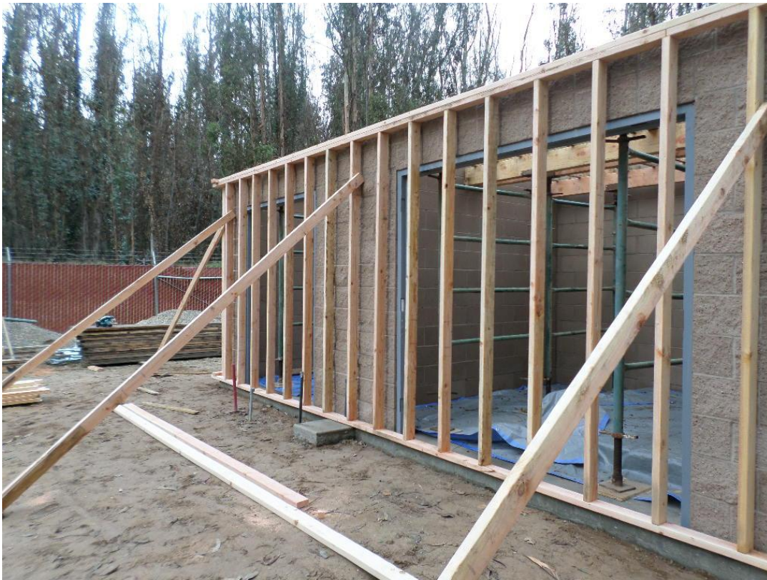
Exterior falsework installed.
