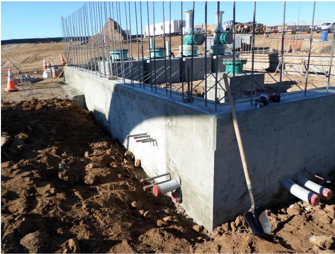
Forms stripped from stem wall at the pump station.
