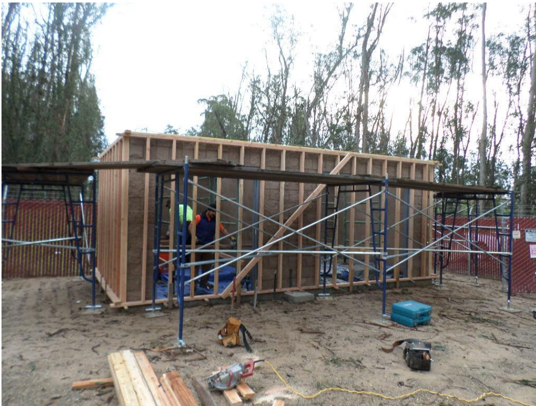
Spiess installing scaffolding.
