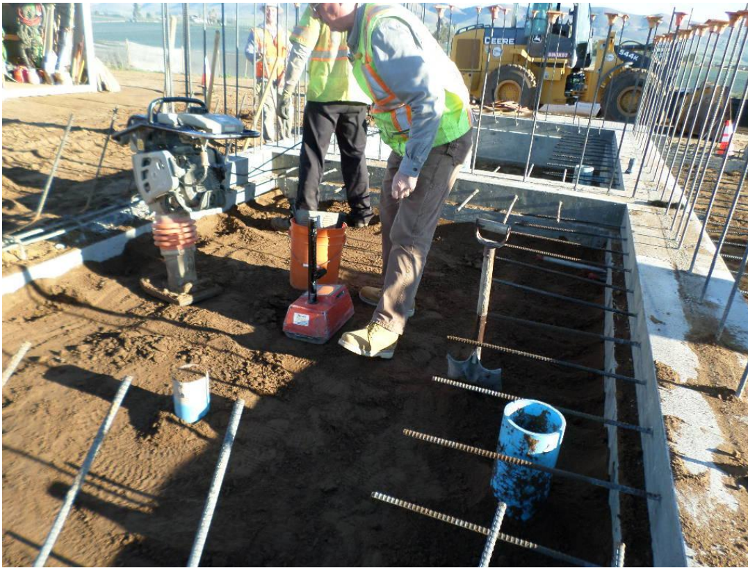
Furgro testing compaction for subgrade under pump station slab.
