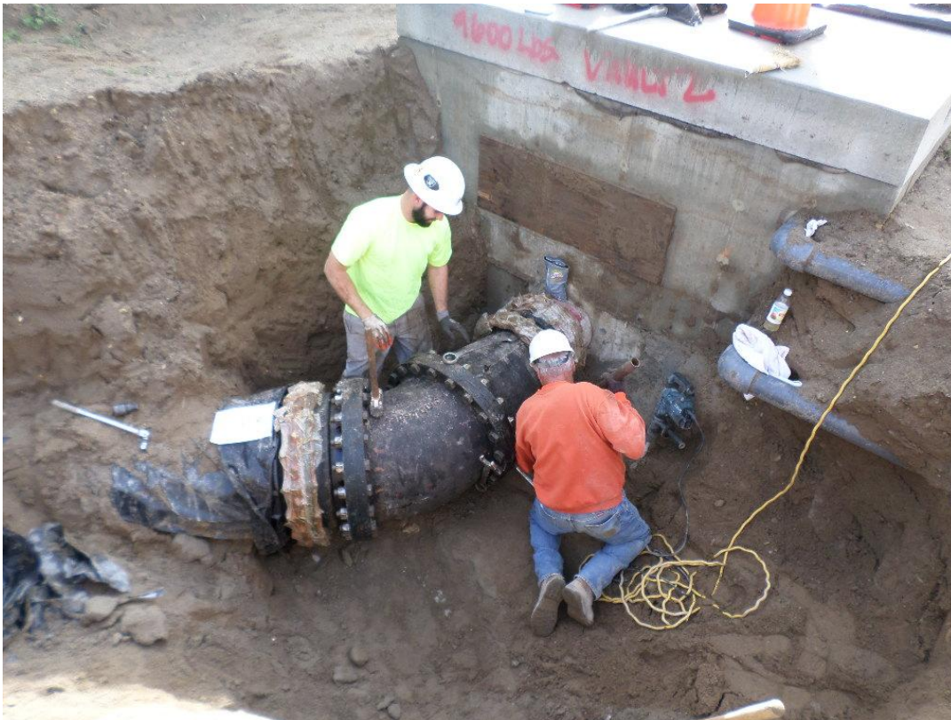
Spiess reinstalling 45 degree elbows to replace defective elbows.
