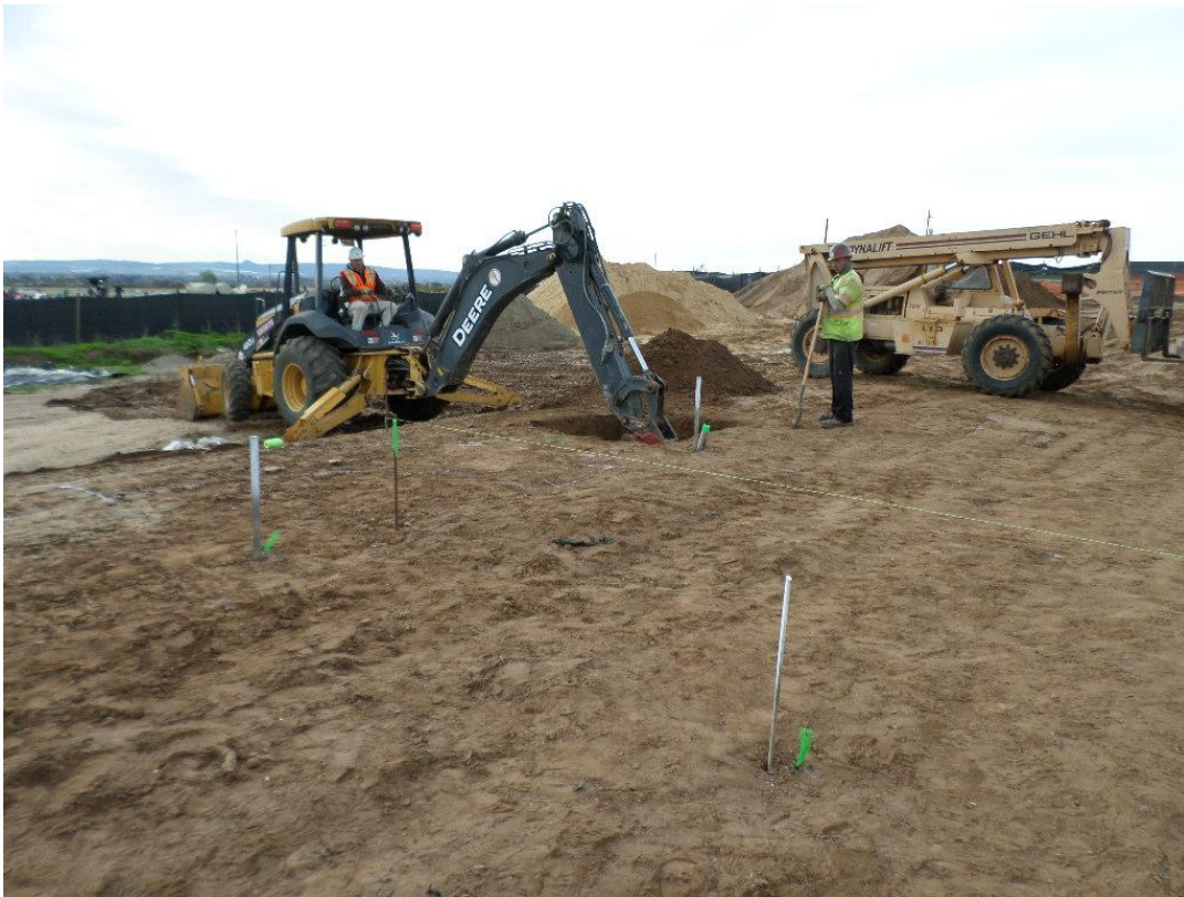
Spieß starting excavation for concrete spillway at retention basin.
