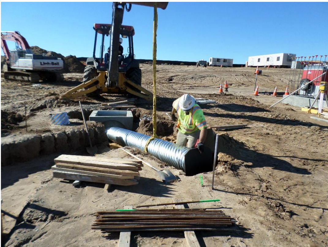
Spieß installing 15-inch CMP for site drainage.
