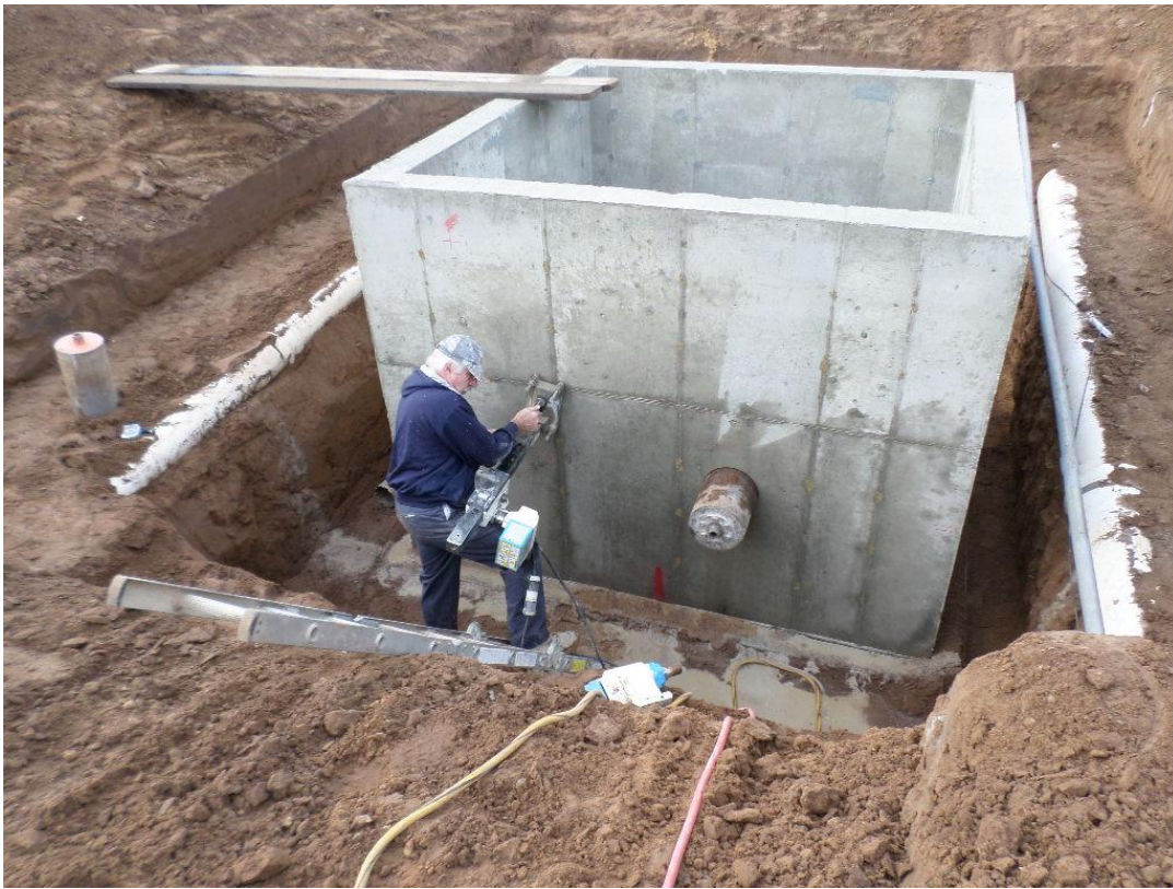
Subcontractor, Russ Concrete Cutting, coring PRV vault walls for pipe penetrations.
