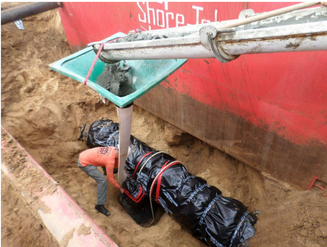
Spieß pouring thrust block at butterfly valve on the 24-inch bypass.
