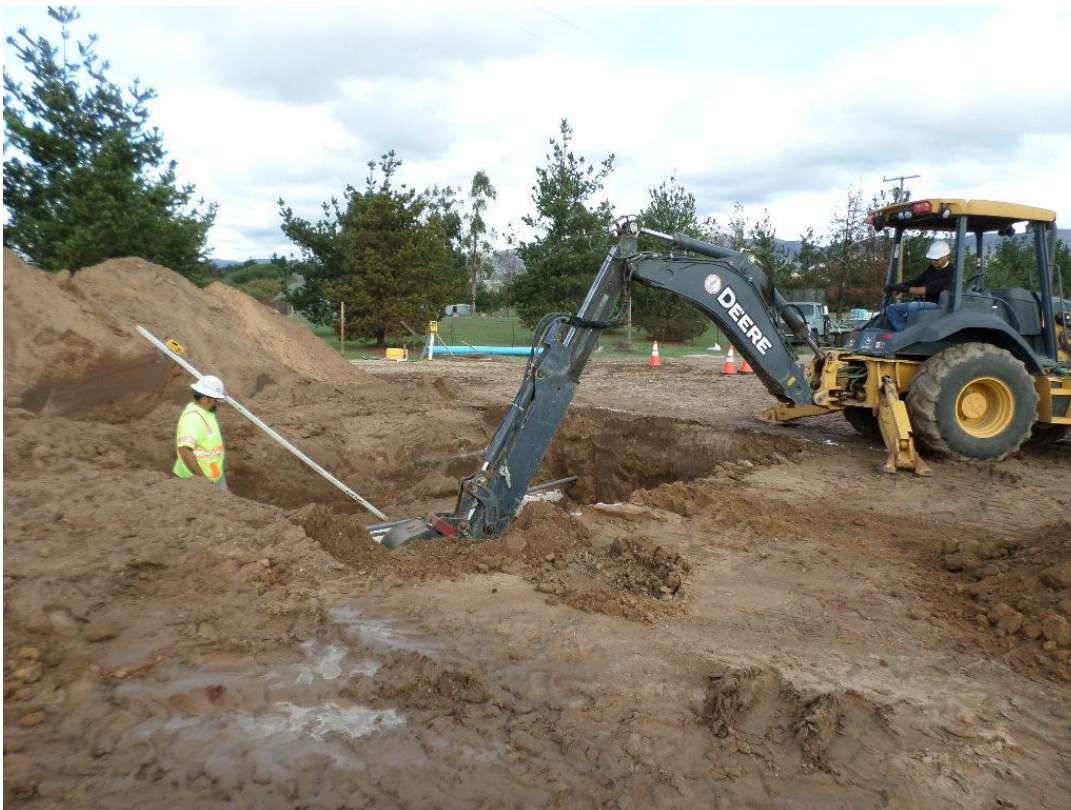
Spieß excavating for the PRV vault in Santa Maria Vista Way.
