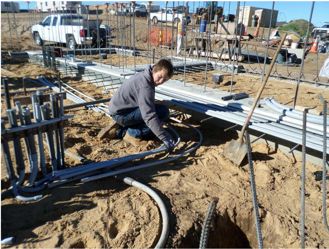
St. Dennis Electric continuing under slab conduit installation at pump station.
