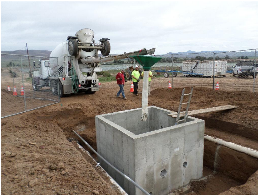
Spieß pouring pipe support pads inside PRV vault.
