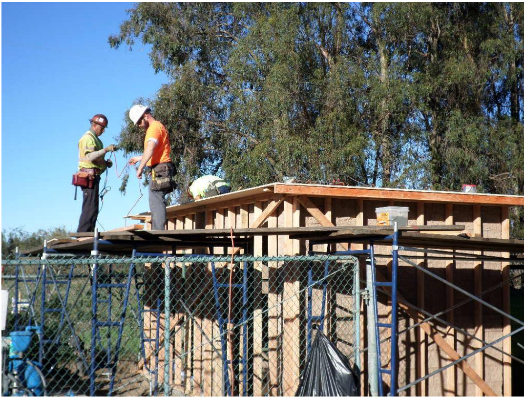
Spieß installing roof forms.
