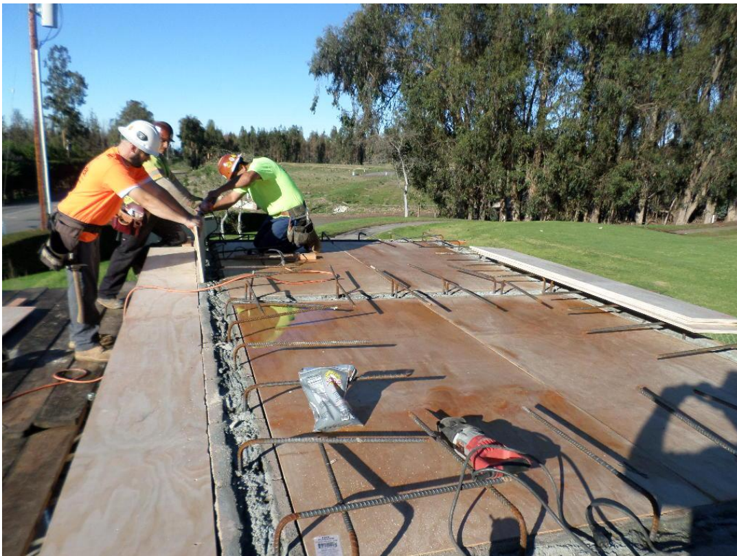
Spieß installing roof forms.
