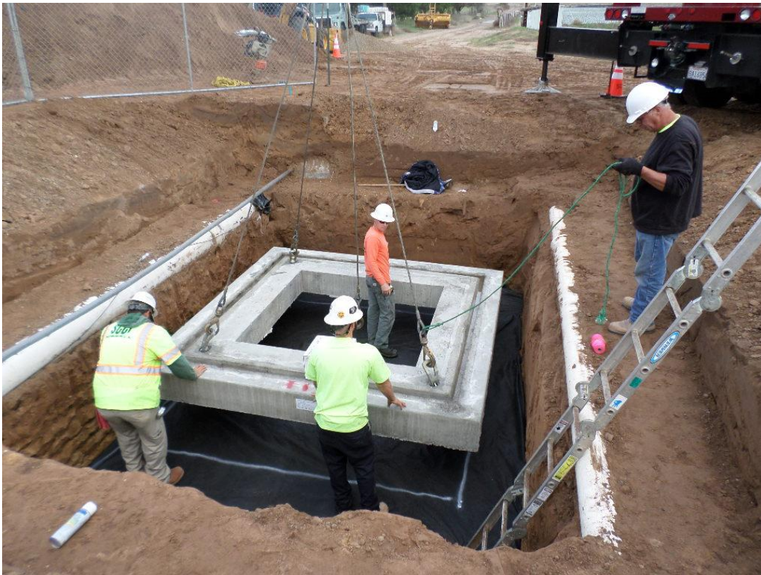
Spiess setting the PRV vault base.
