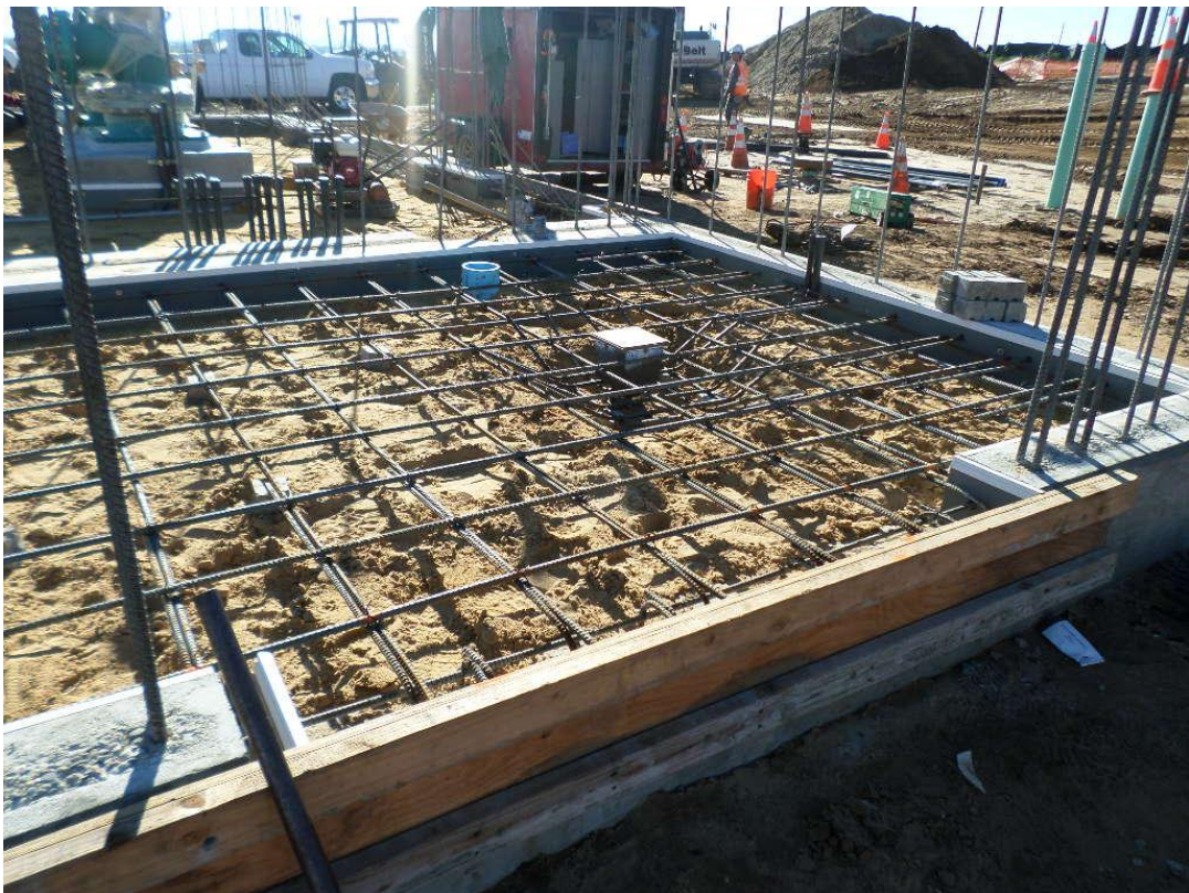
Rebar installed for slab at ammonium sulfate room in pump station.
