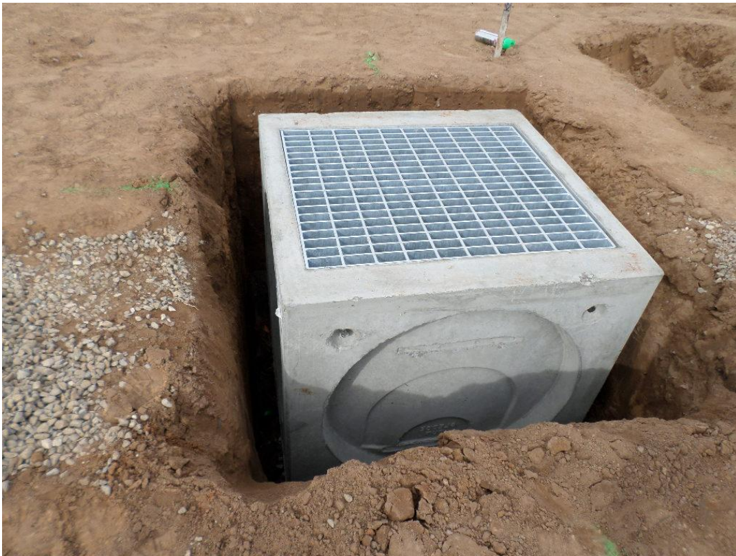
Catch basin installed.
