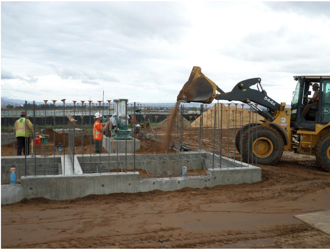
Spiess backfilling under slab subgrade at pump station.
