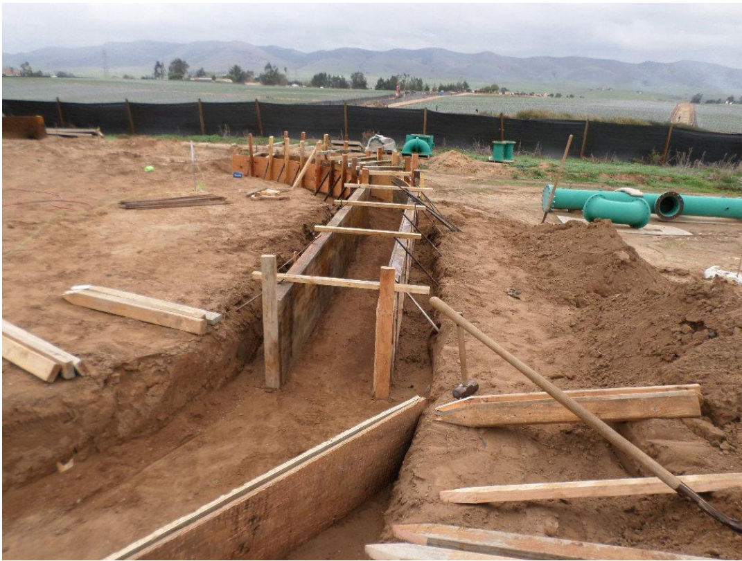
Forming the concrete spillway.
