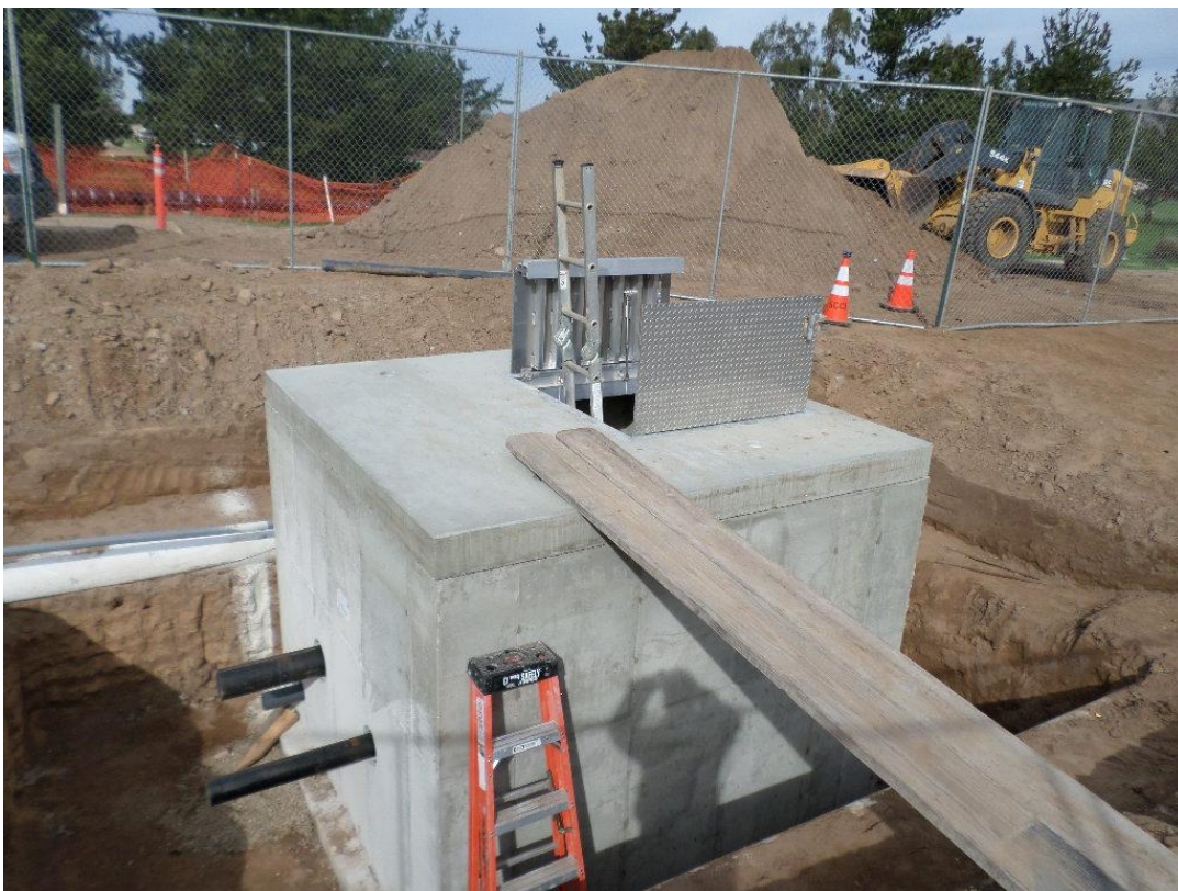
PRV vault lid installed.
