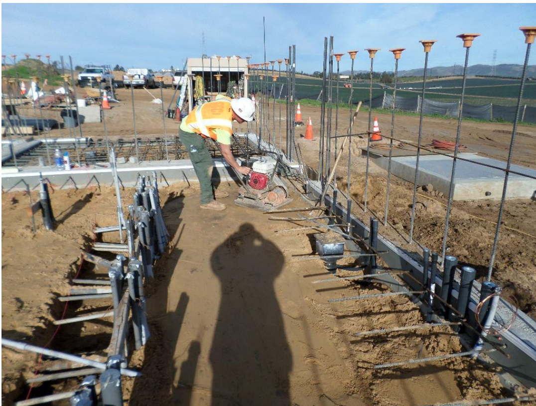
Spiess compacting subgrade fill at pump station.
