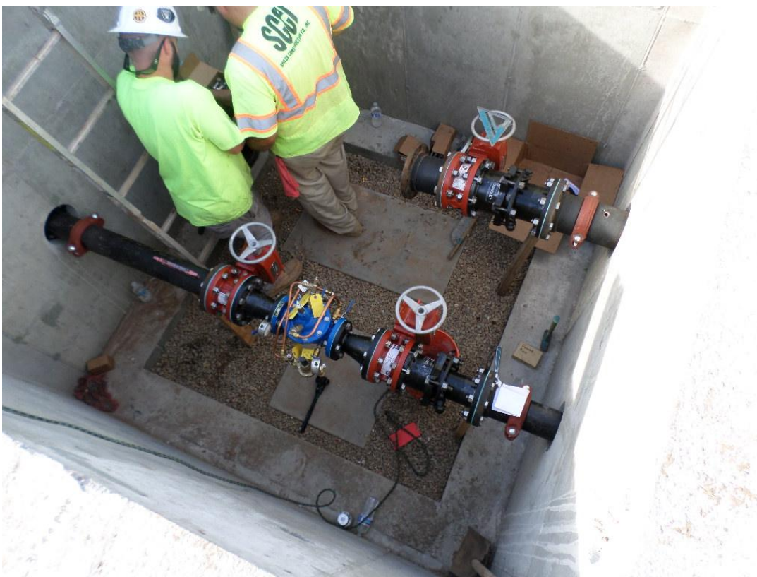
Spiess installing pipes inside the PRV vault.
