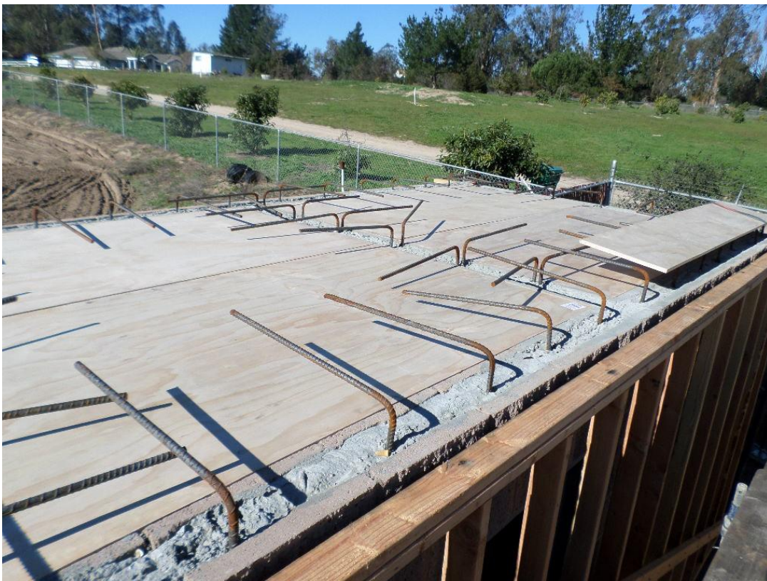
Forming for roof pour.
