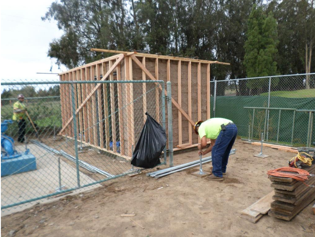
Spiess installing exterior forms and scaffolding for the roof pour.
