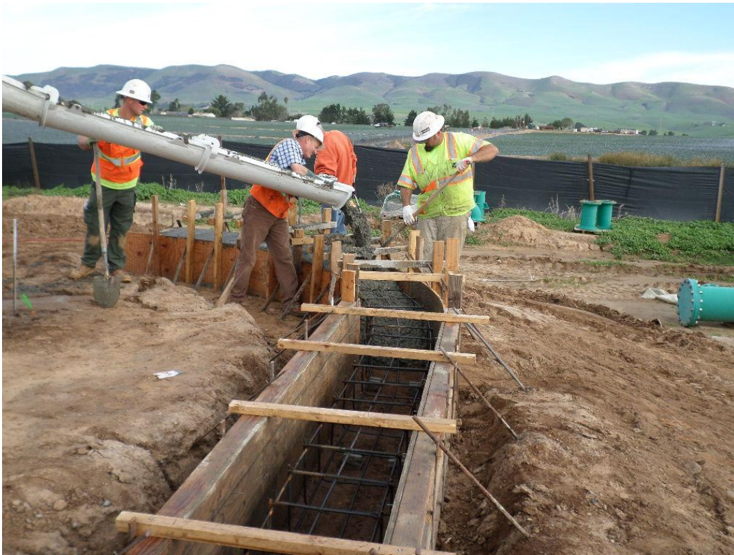
Spieß pouring the concrete spillway.
