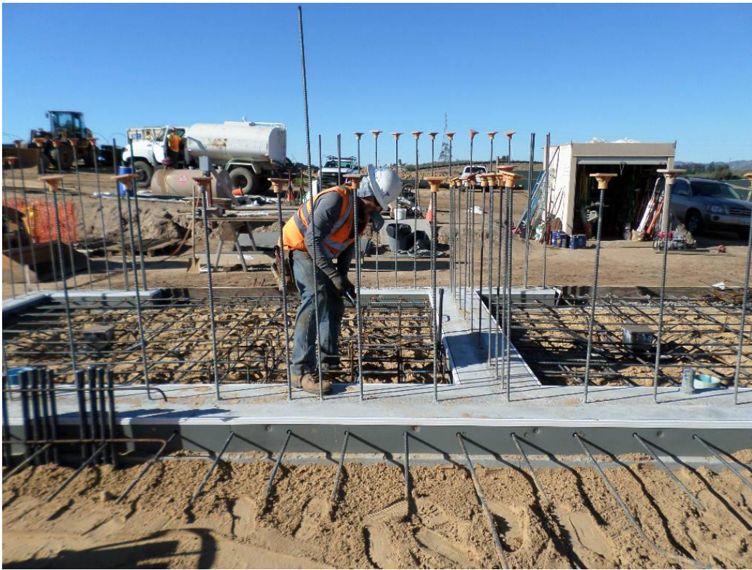
Vista Steel tying reinforcing at pump station.
