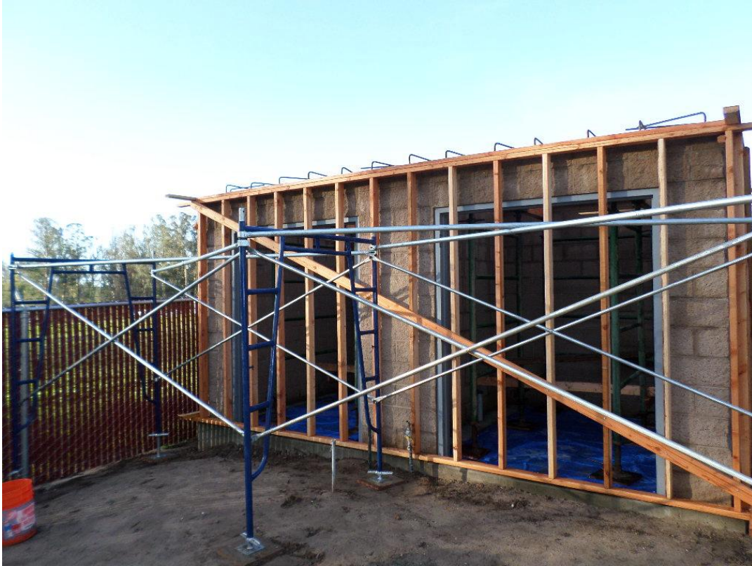
Exterior forms and scaffolding installed.
