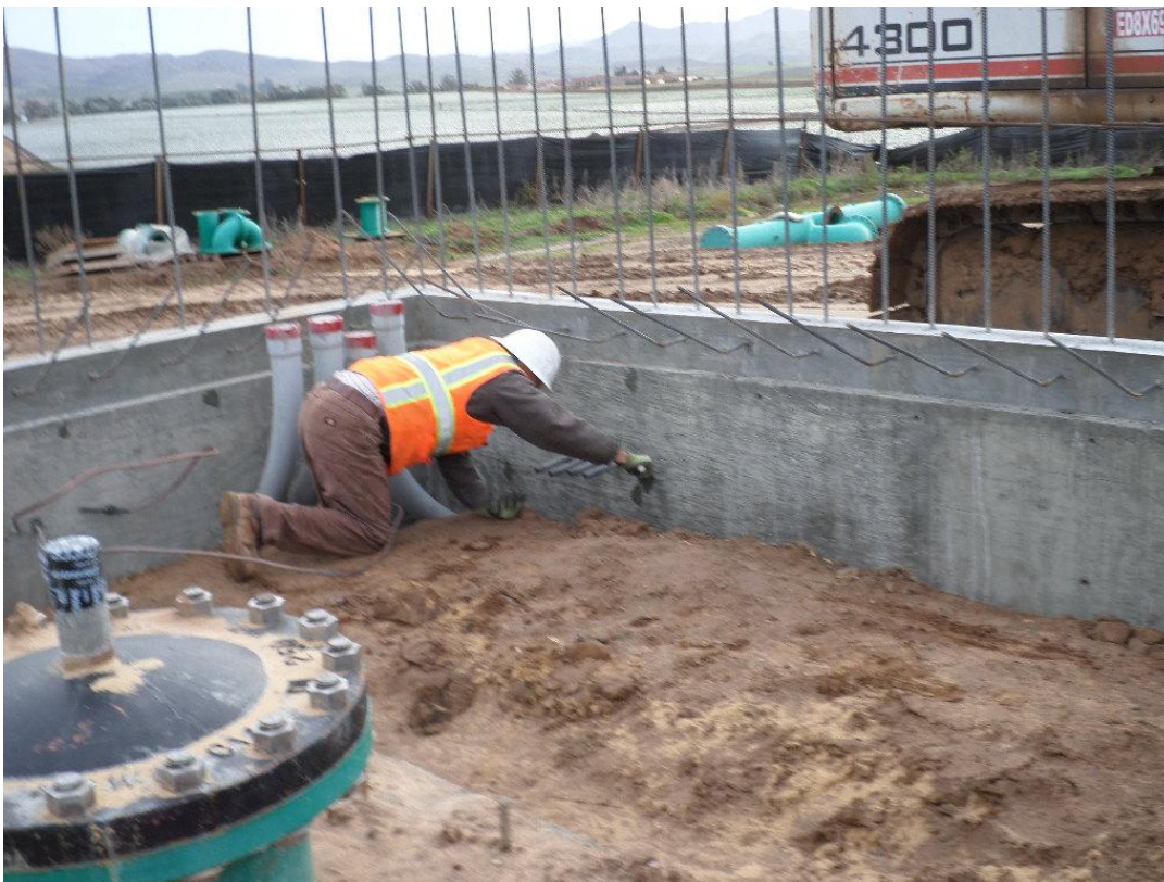
Spieß patching form tie holes in stem wall at pump station.
