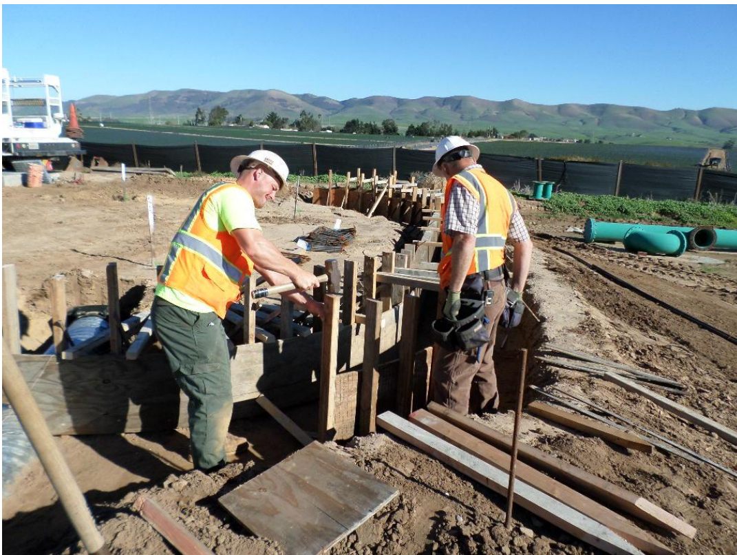
Spies forming the concrete spillway.
