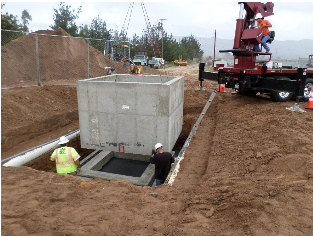
Spiess setting the PRV vault in Santa Maria Vista Way.
