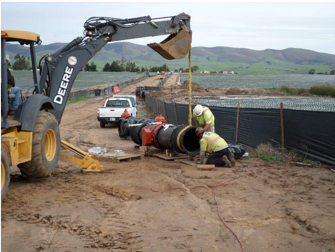
Spieß assembling 24-inch DIP bypass piping.
